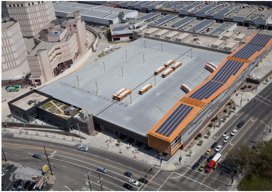
Photo Credit: Roof Maintenance Design Group
