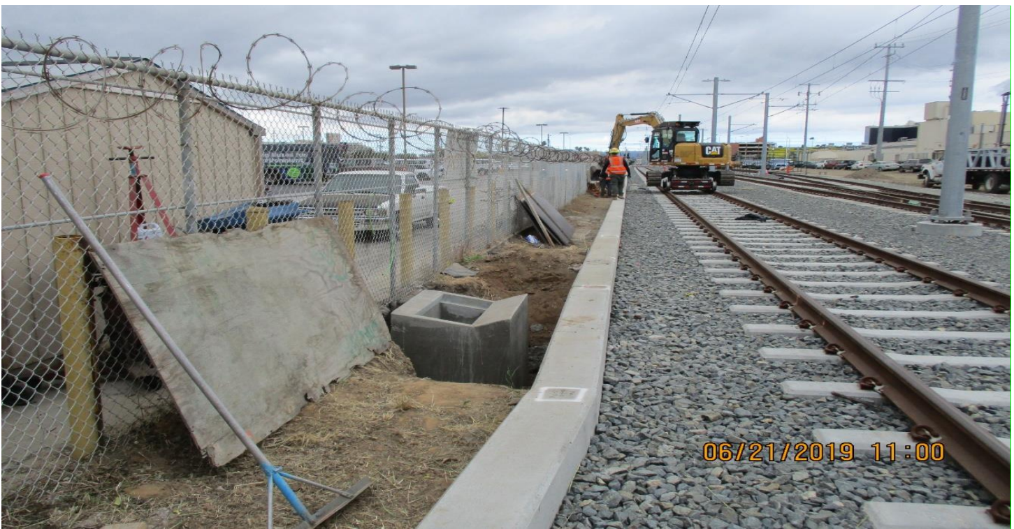
GUIDEWAY-ARBOR VITAE- A Guideway north Arbor Vitae clearing and grubbing and prep for drainage swale.
