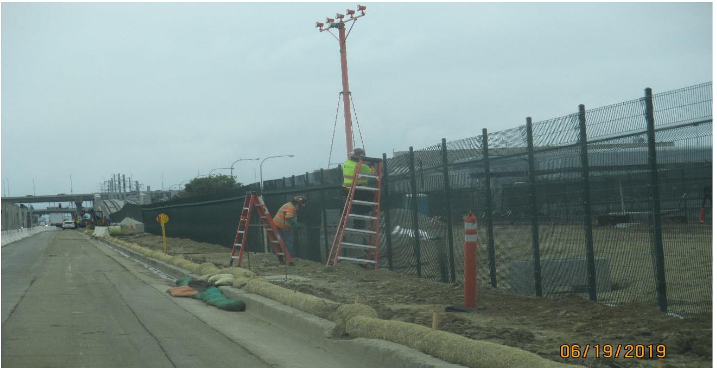
UG1- Wire mesh fence installation at UG-1.
