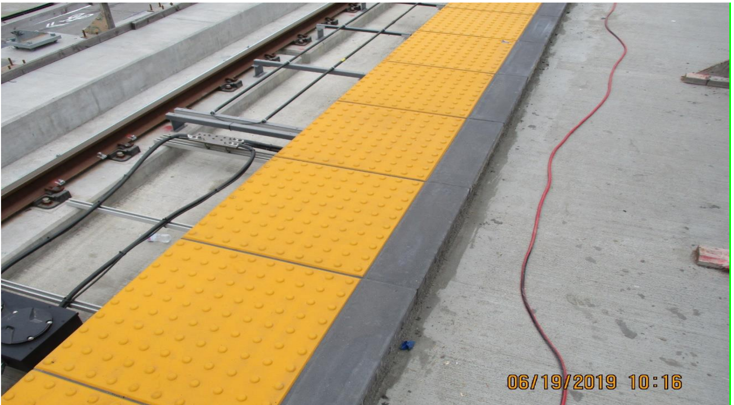
AVIATION/CENTURY- Grout placement at North Bond track for edge pavers.
