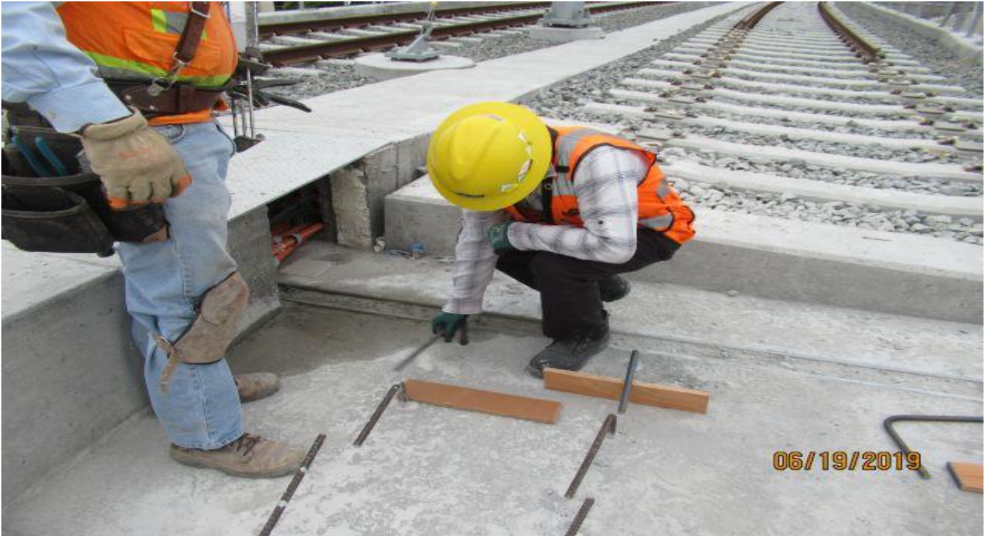
MANCHESTER BRIDGE- WSCC installing rebar after applying epoxy.
