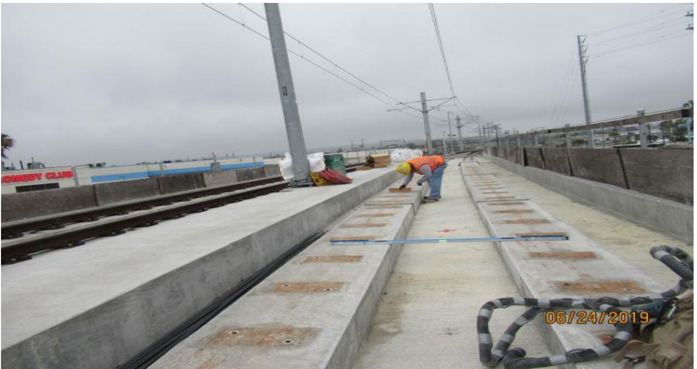
MANCHESTER BRIDGE- WSCC finisher verifying fastener plane on L&R plinths Manchester bridge.
