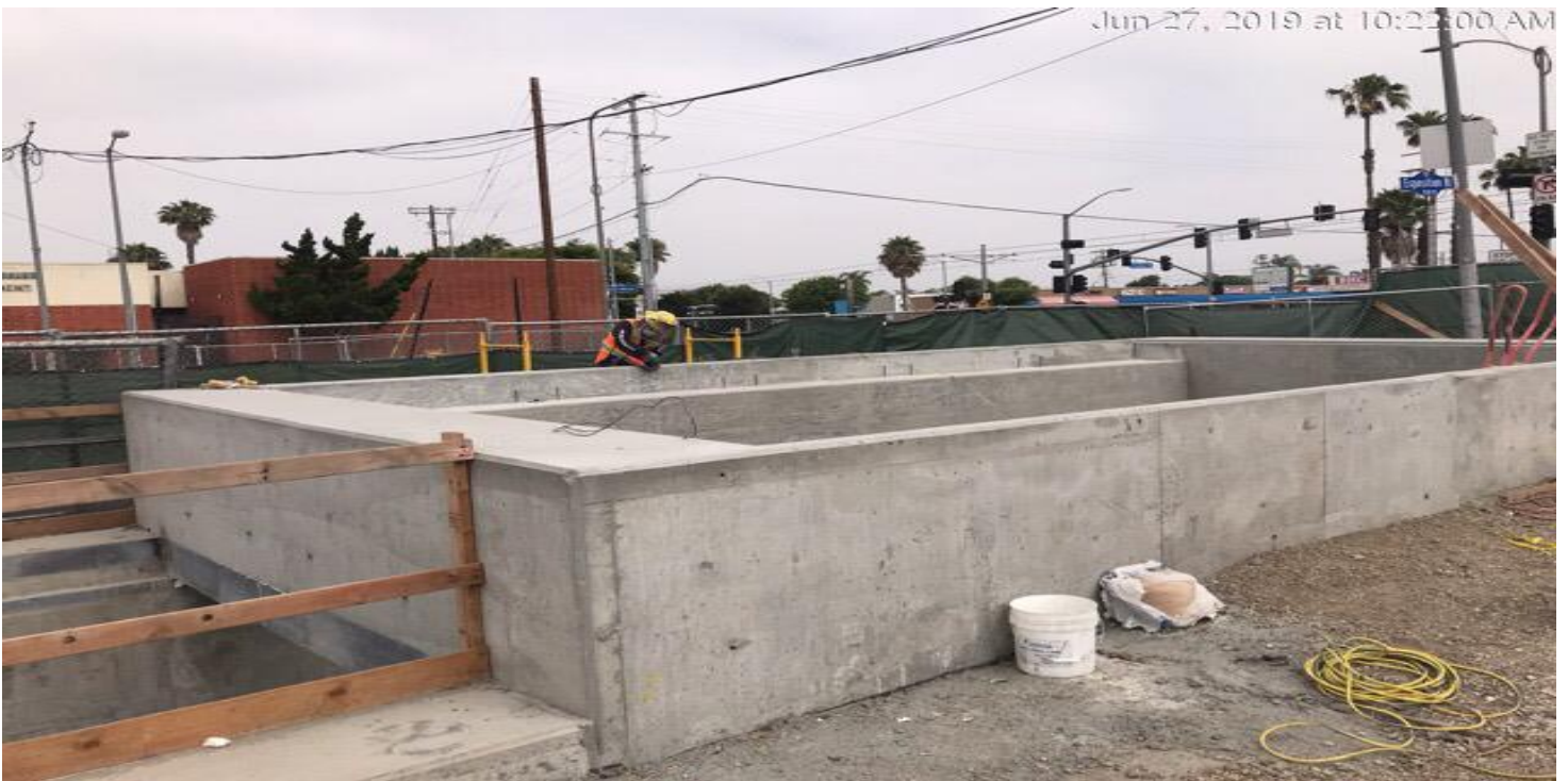
EXPOSITION/CRENSHAW STATION – Continued finish work at the Emergency Ventilation Shaft north.
