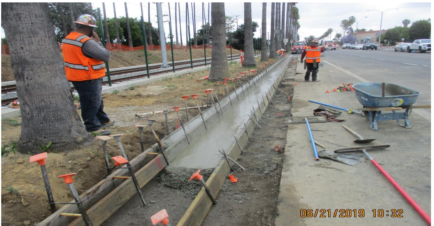
FLORENCE/CENTINELA - Griffith Co-Placing conc C&G on WB Florence east of Centinela.
