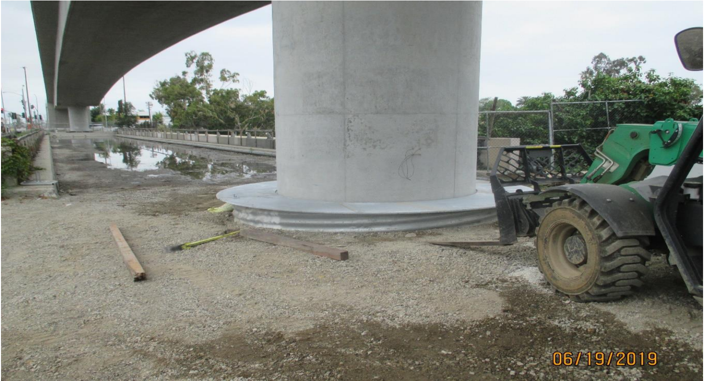
405 BRIDGE - Setting the safety plates for bent 3 of the 405 bridge.
