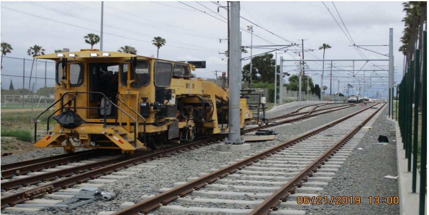
FLORENCE/WEST- Guideway between Q1-Q2 XO track to Fairview Heights Station tamping.
