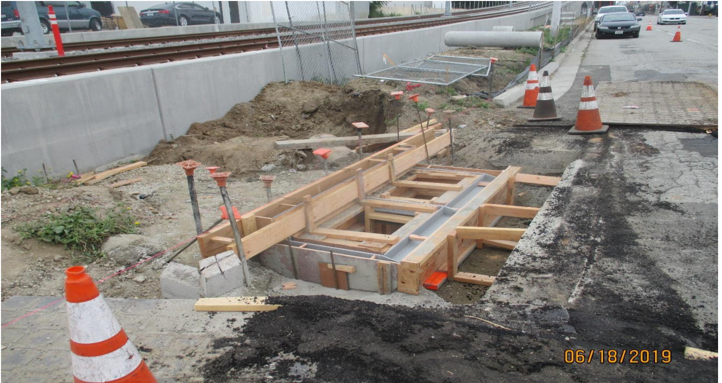
FLORENCE/CENTINELA - Catch basin #1 on Florence prior to concrete today.
