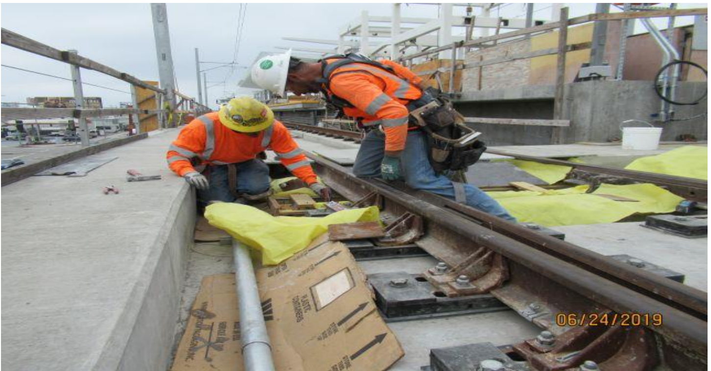
AVIATION/CENTURY- WSCC repairing concrete forms prior to placing concrete on K1LH XO Century bridge.
