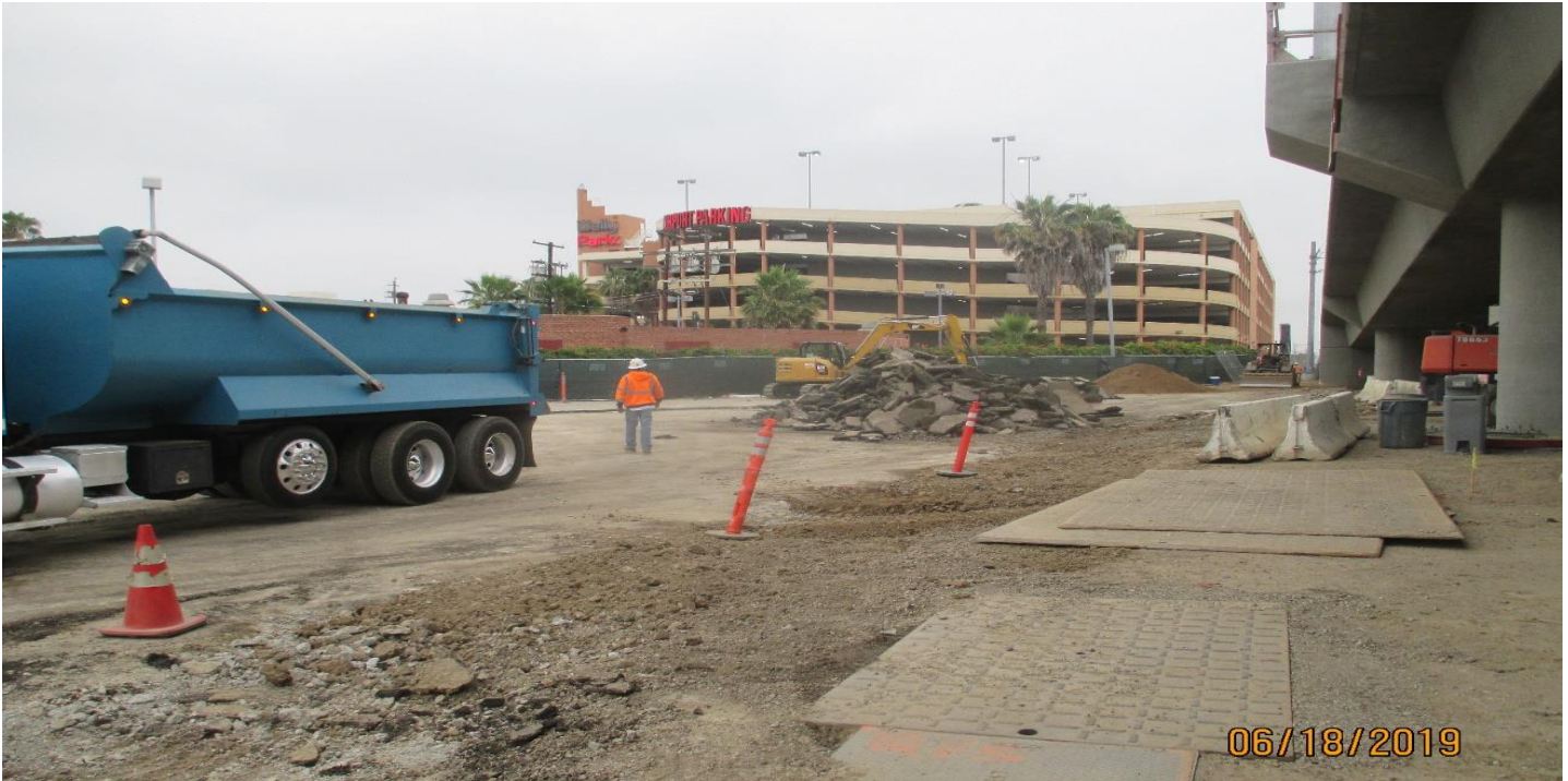
AVIATION/CENTURY- AC demo and removal at the Aviation Station yard.
