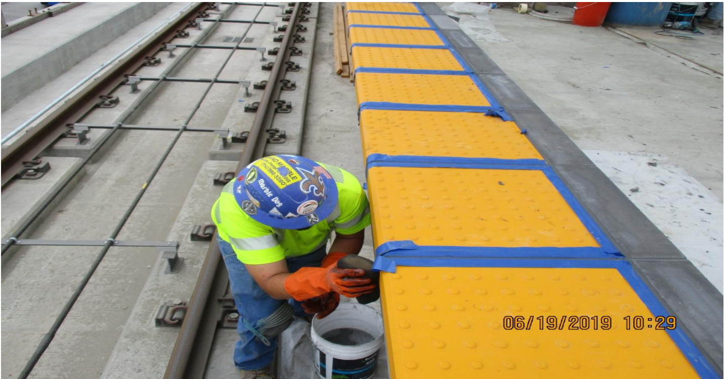
AVIATION/CENTURY- Grout placement at North Bond track for edge pavers.
