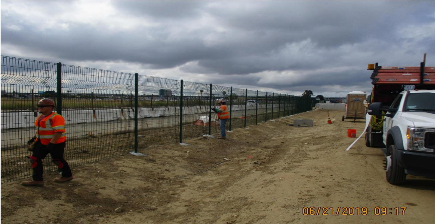
UG-1- A Guideway between UG1 and 104th St. wire fence placement.
