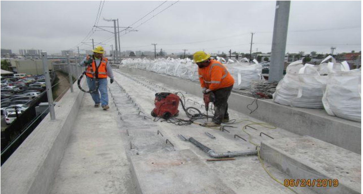
MANCHESTER BRIDGE- WSCC finisher drilling for rebar dowels on Manchester bridge.
