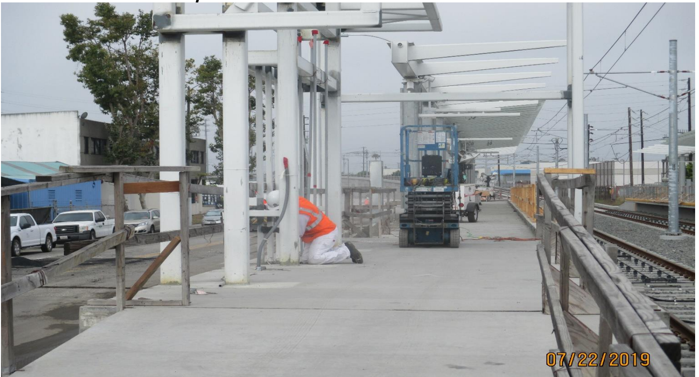
FLORENCE/HINDRY - Sanding and prepping for paint at the Hindry Station.
