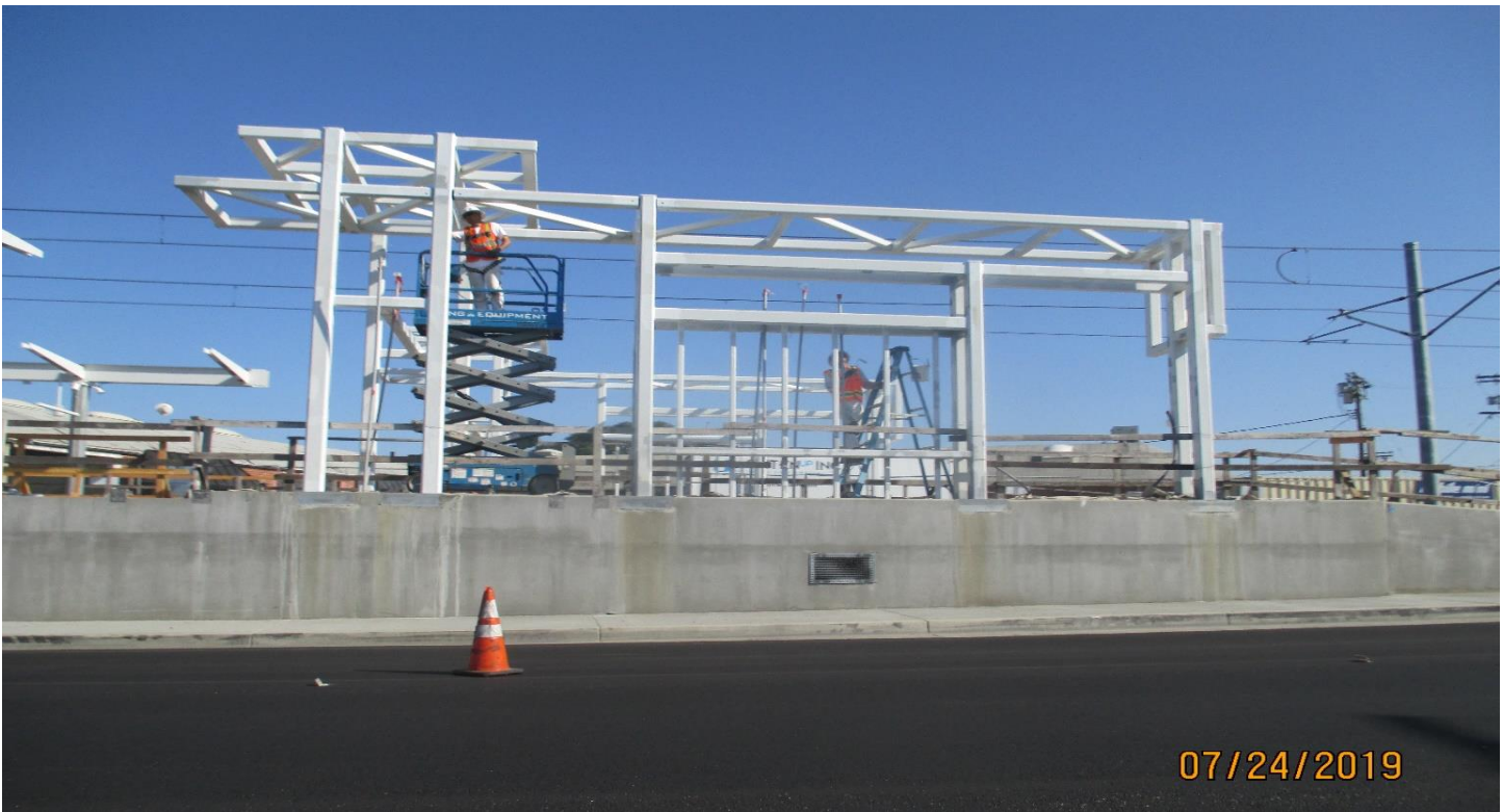
FLORENCE/HINDRY - Painting the ticket vending machine structure at the Hindry Station.
