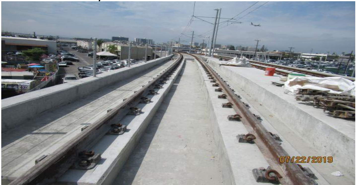
MANCHESTER BRIDGE- SB track at Manchester Bridge DF replacement work.
