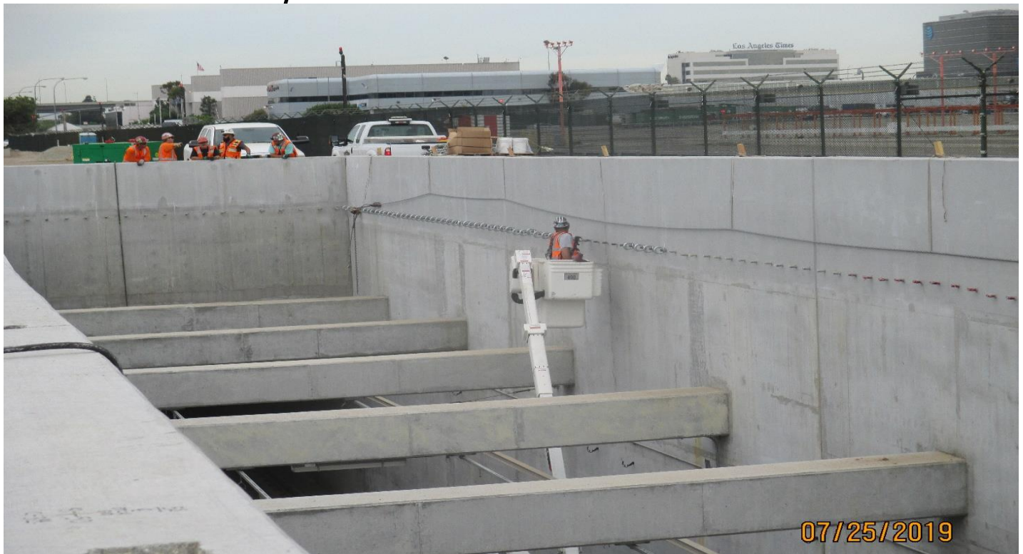
UG1- Cable barrier installation.
