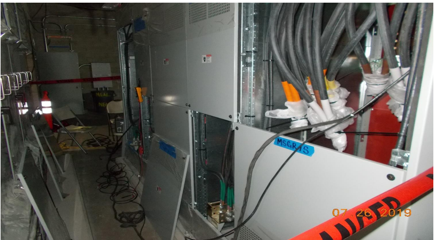
CRENSHAW/VERNON- NETE electrical testing on MSWGR-S, contact resistance.
