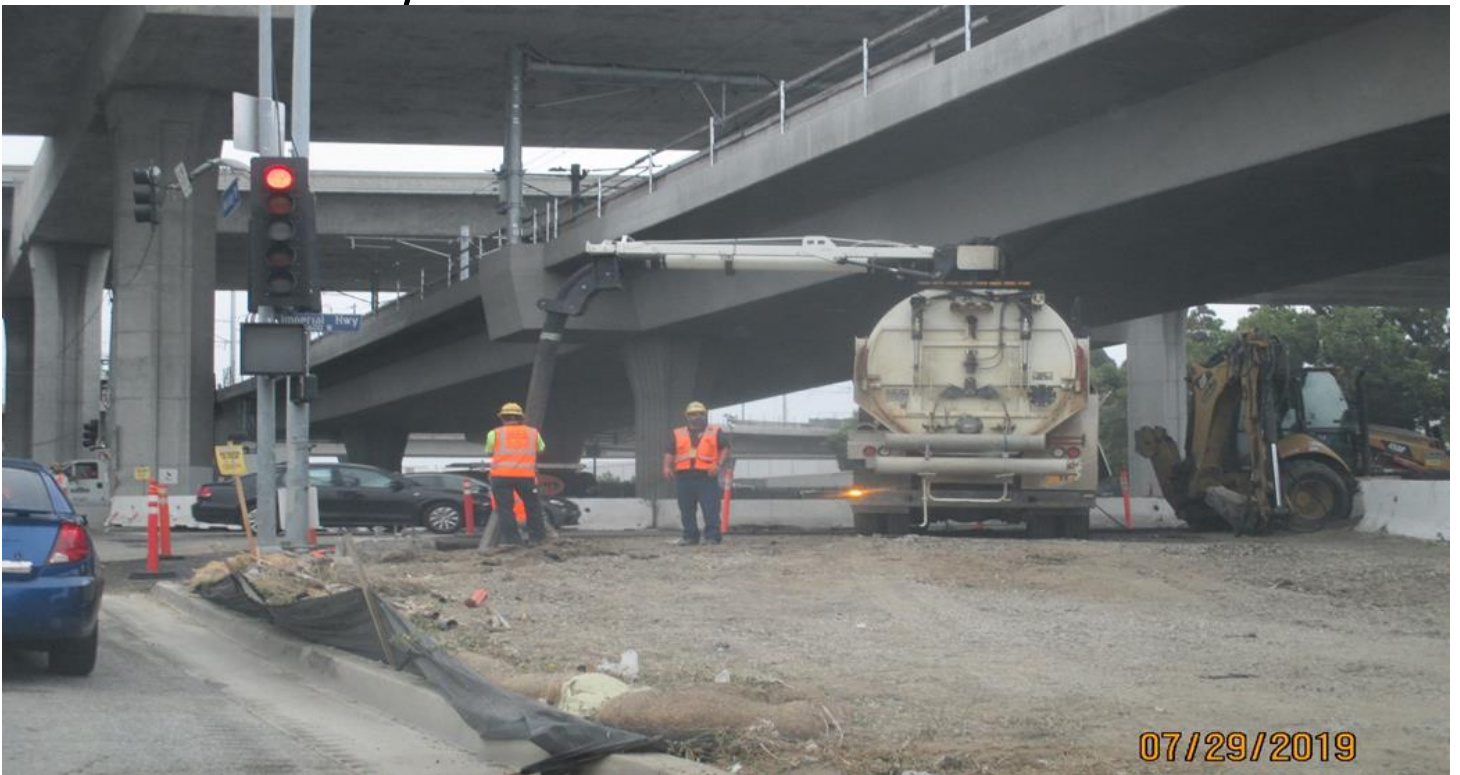
AVIATION/CENTURY- Vacuum truck exposing a foundation to be removed at Aviation.
