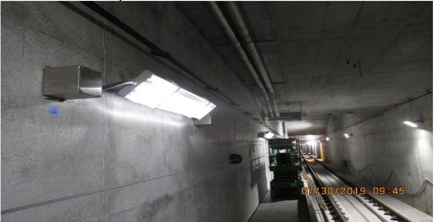
UG3- Continued lighting installation at the southbound tunnel.
