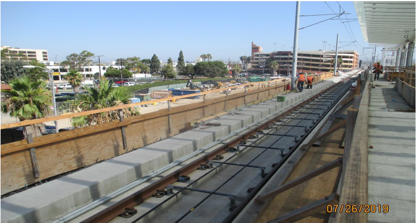
AVIATION/CENTURY- Stripping and setting forms for the galvanized bolt replacement.
