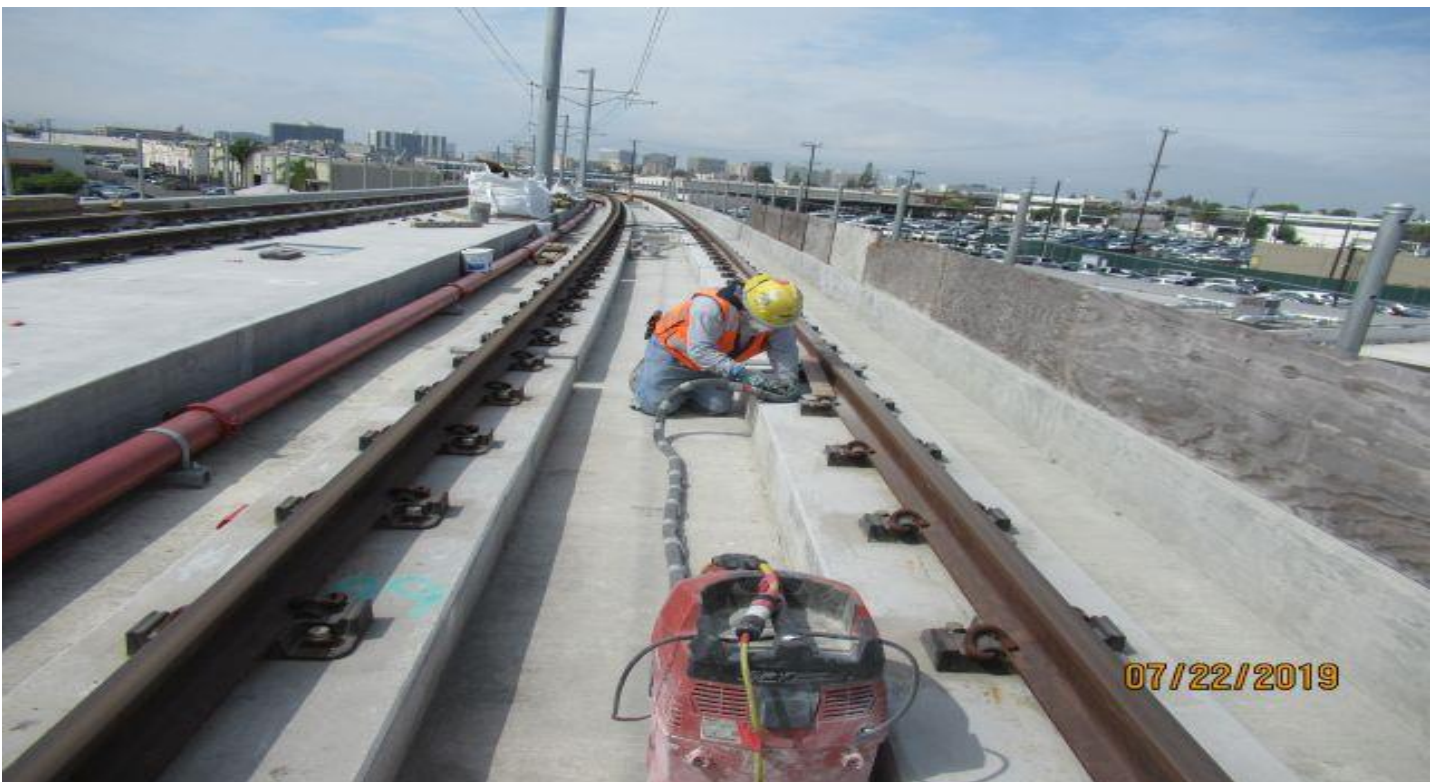
MANCHESTER BRIDGE- NB track WSCC finisher hand grinding plinths for 0" plane.
