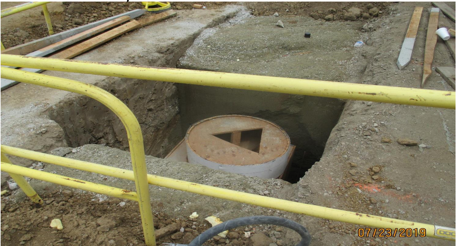
AVIATION/CENTURY- Storm drain manhole prior to concrete placement at the yard.
