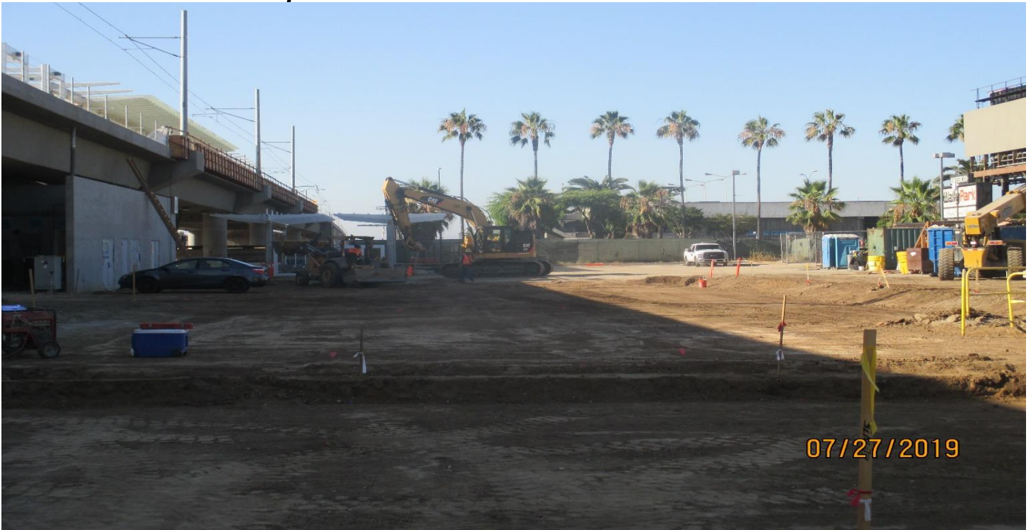
AVIATION/CENTURY- Grading for the plaza and parking lot at Aviation Station.
