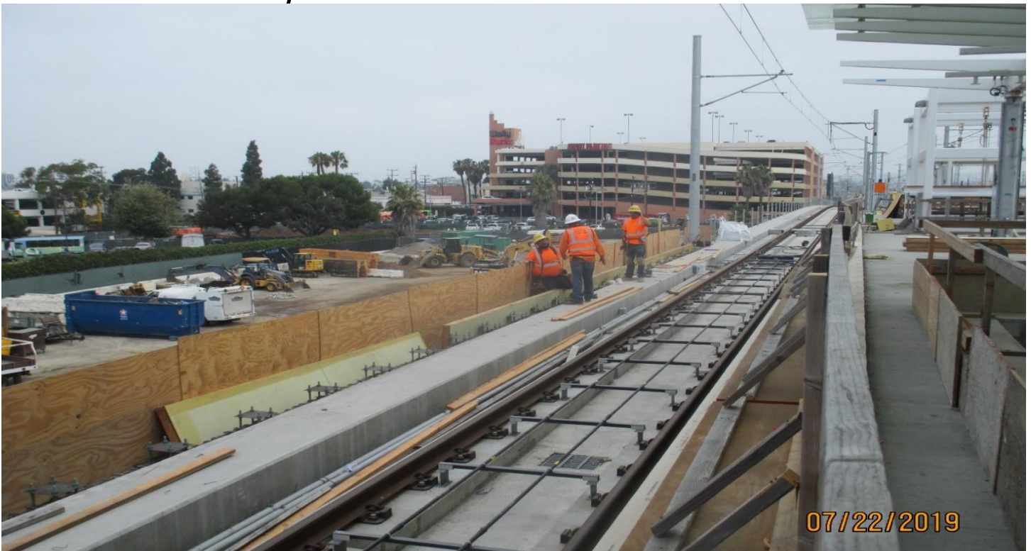
AVIATION/CENTURY- Reinstalling the galvanized fence anchor bolts at the Aviation Station
