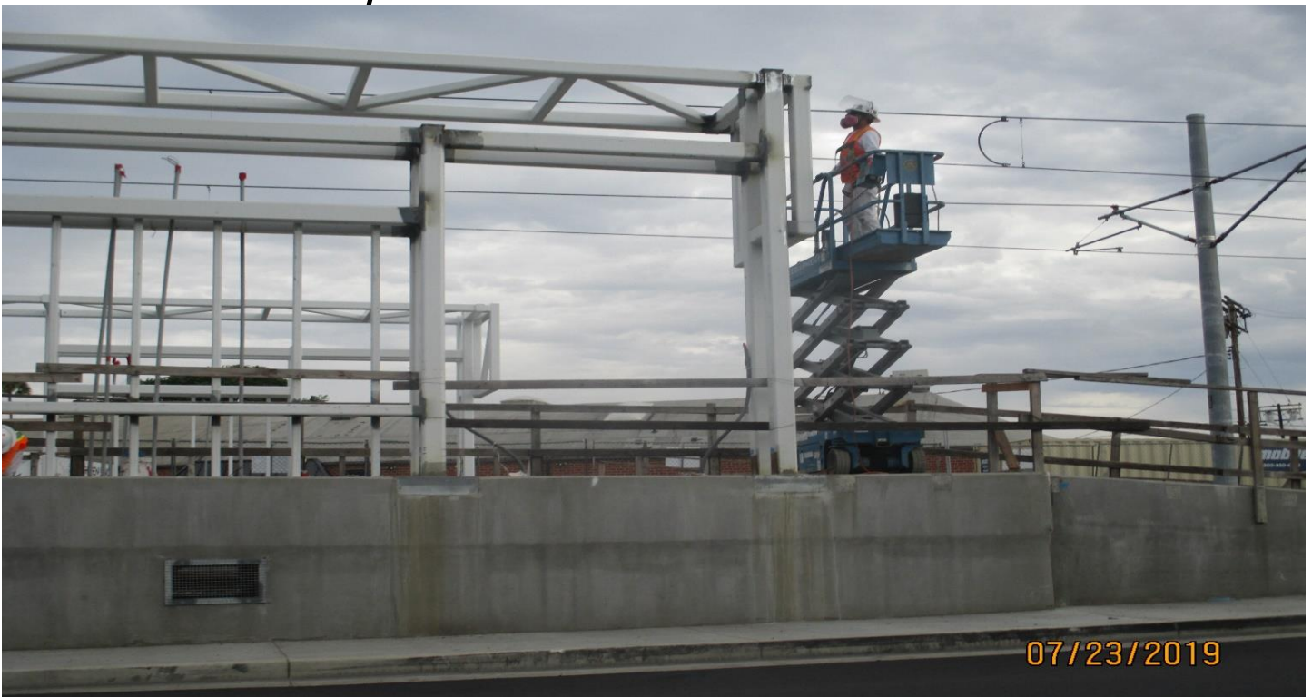
FLORENCE/HINDRY - Painting the TVM structure for the NB Hindry Station platform.
