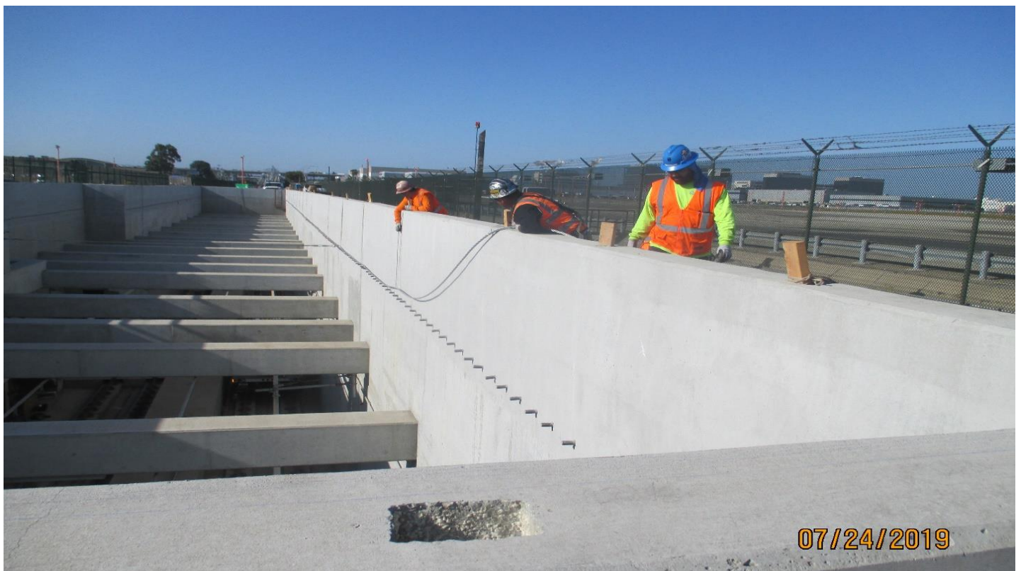
UG1- Cable safety barrier installation.
