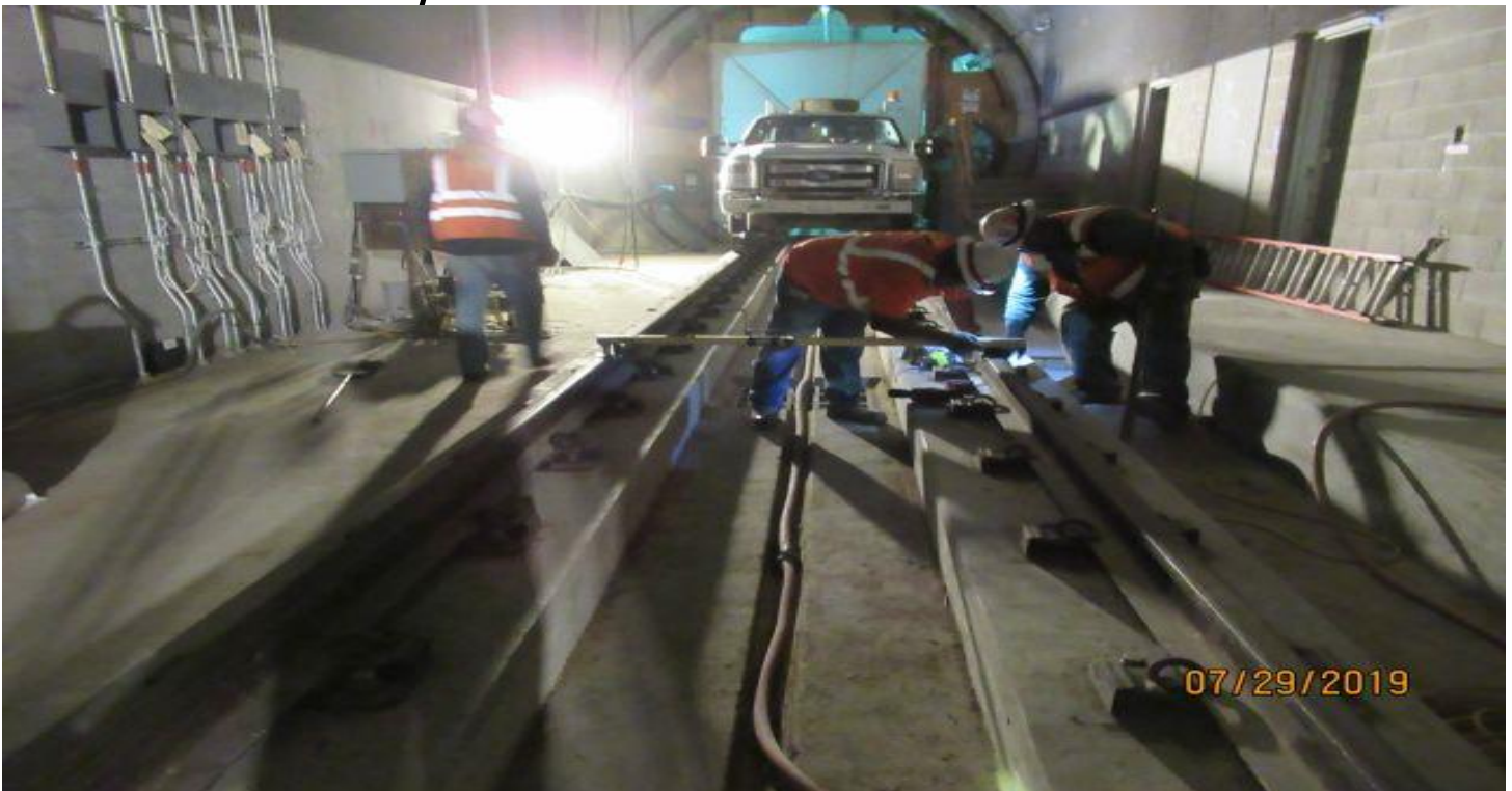
UG4- HCC verifying track gauge on SB track UG4 MLK station.
