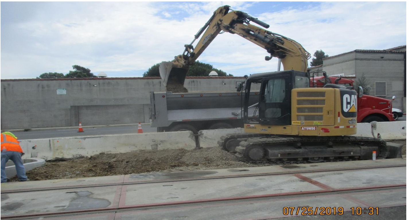
HIGH STREET- WSCC Grading for cross gutter at High ST crossing.
