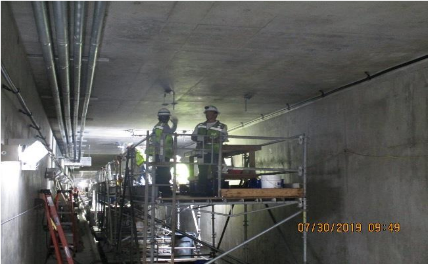
UG3- Continued installation of OCR brackets along the southbound tunnel.
