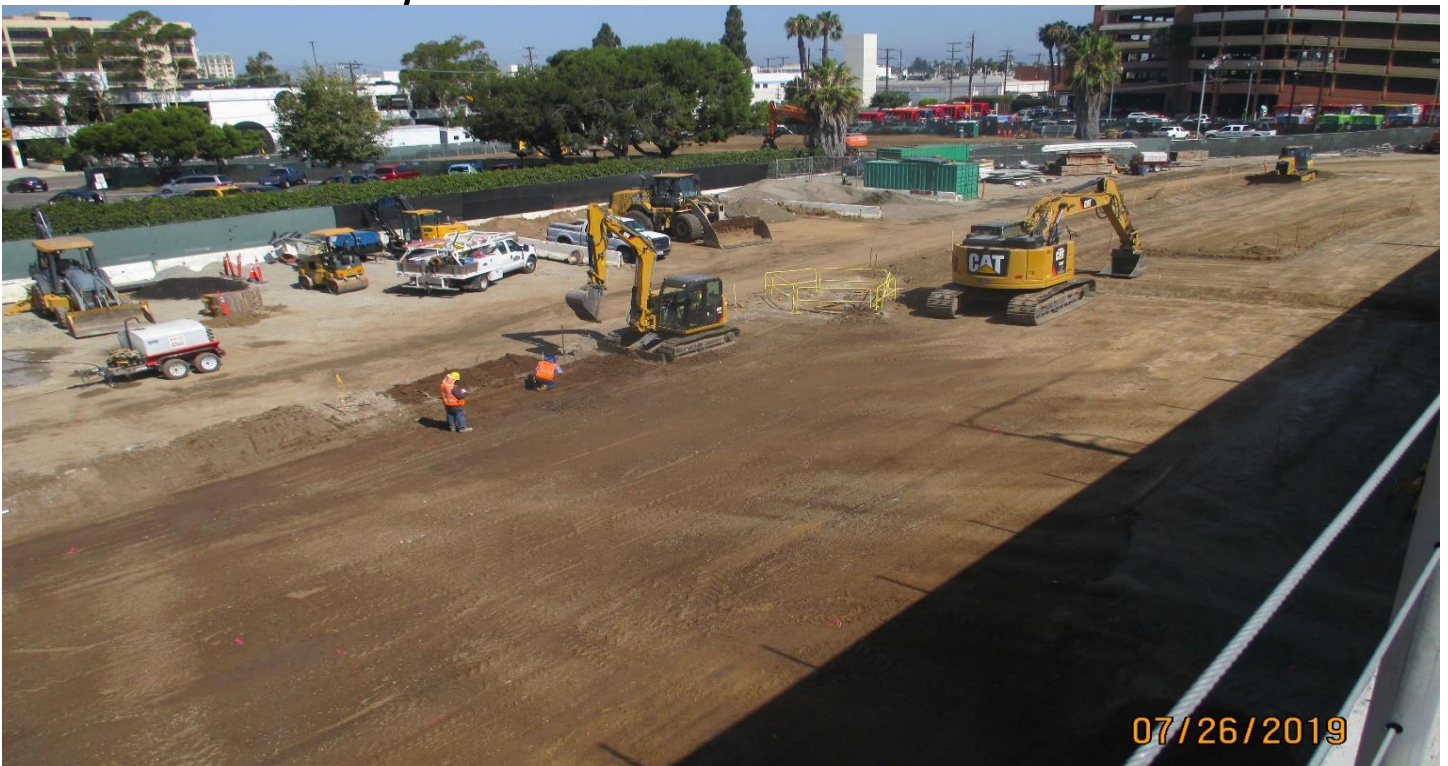
AVIATION/CENTURY- Grading the plaza area at the Aviation Station.
