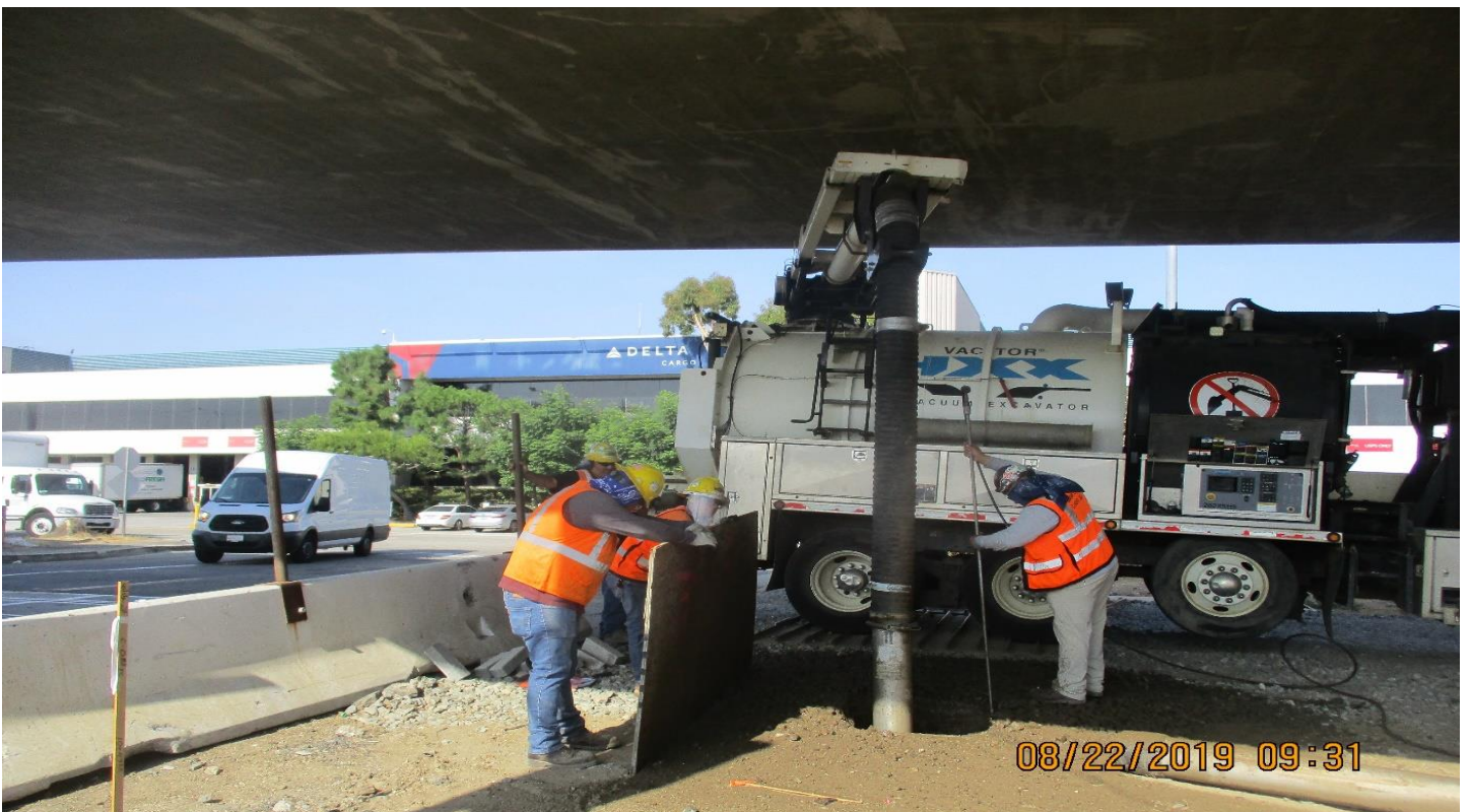
AVIATION/CENTURY- WSCC Pot hole bat 111th St and Aviation.
