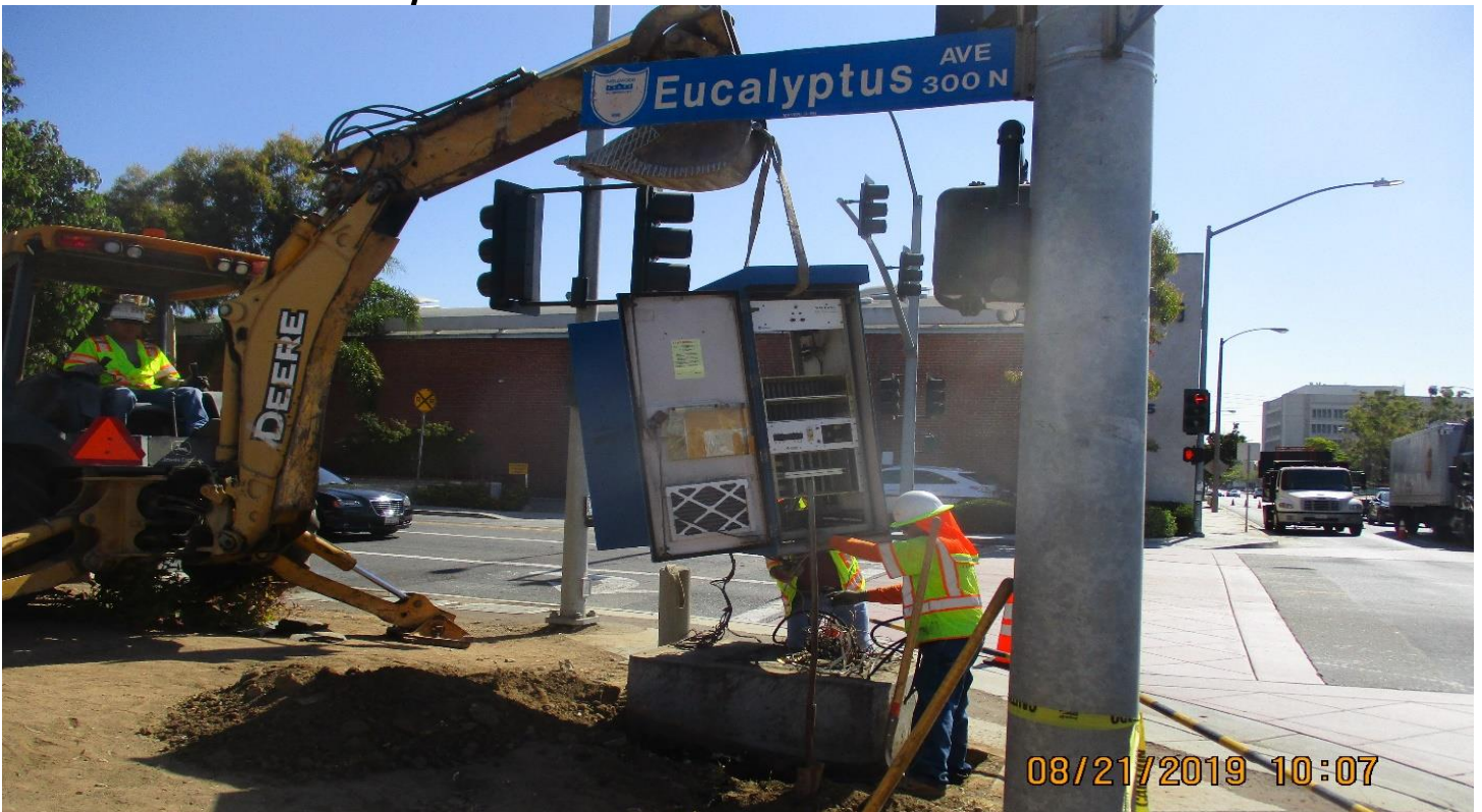
FLORENCE STREET - Select Electric Remove old controler at Eucalyptus and Florence.
