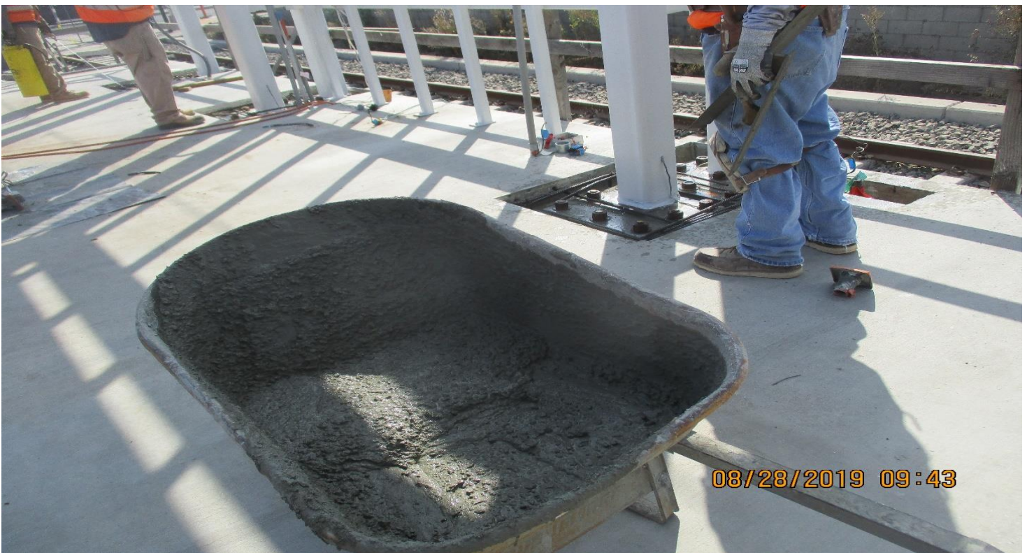
FLORENCE/WEST- WSCC Place Conc in column wells on West Sta platform.st.
