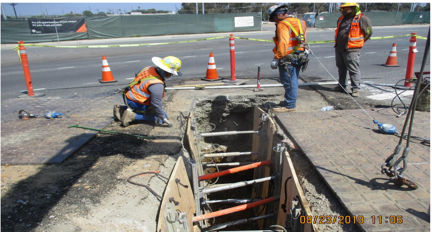
FLORENCE/LA BREA - WSCC Worked on SD lines at Locust and Florence.
