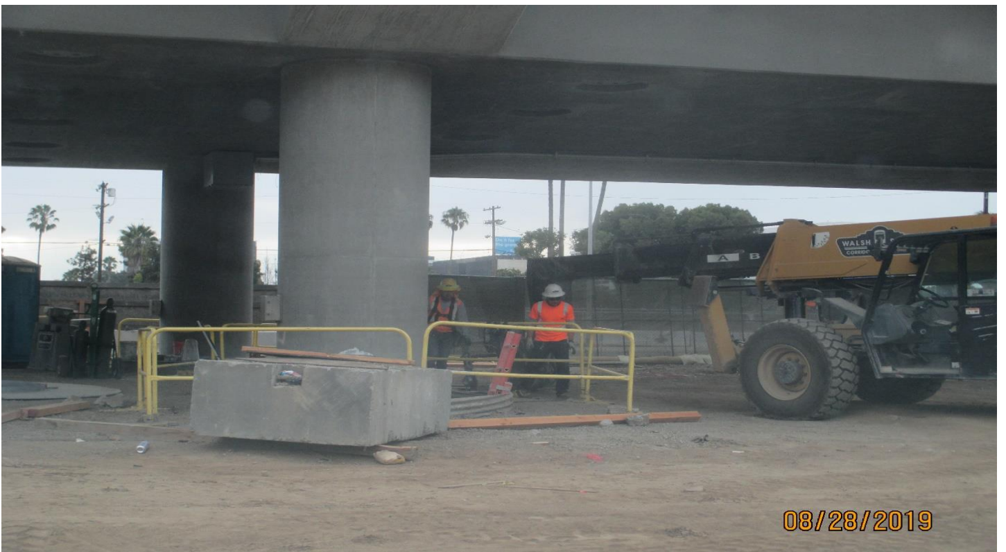
AVIATION/CENTURY- Bent safety cover installation at the Aviation Station bridge.
