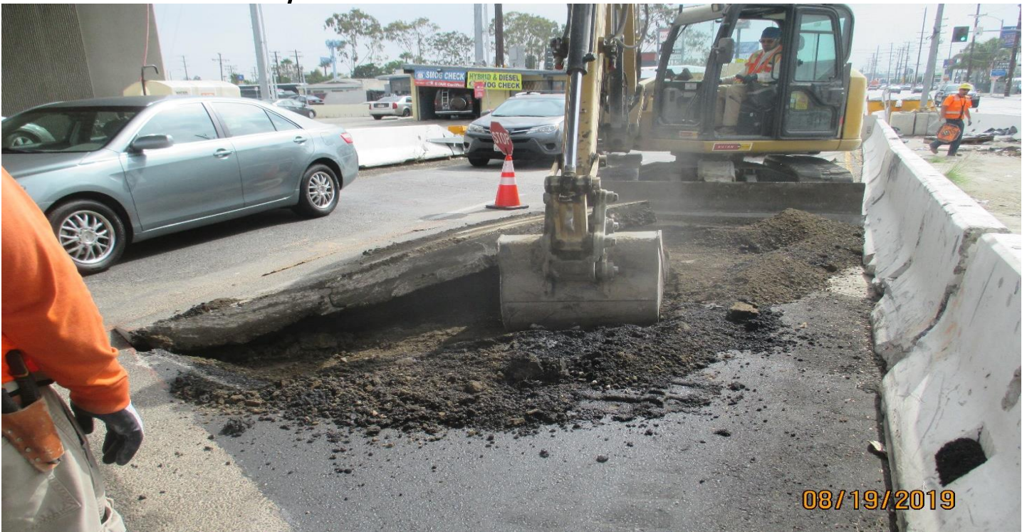
MANCHESTER BRIDGE- Old track removal on Manchester.
