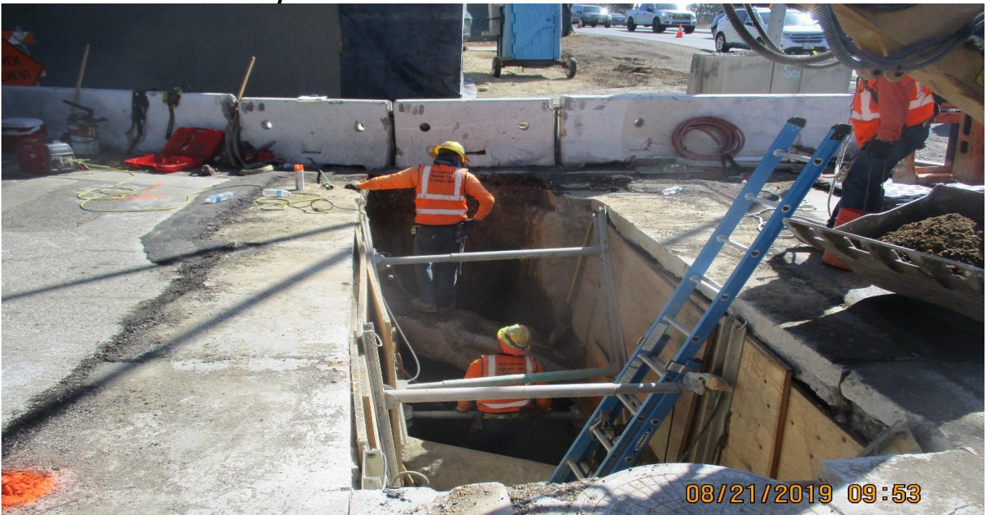
LA BREA BRIDGE- WSCC Relocated SD lines at La Brea bridge.
