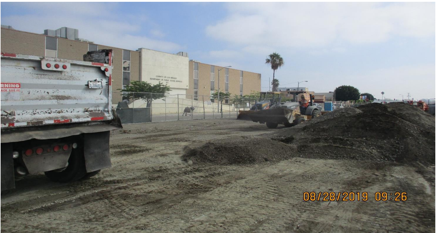
FLORENCE/WEST- WSCC Clean out West Station parking lot.
