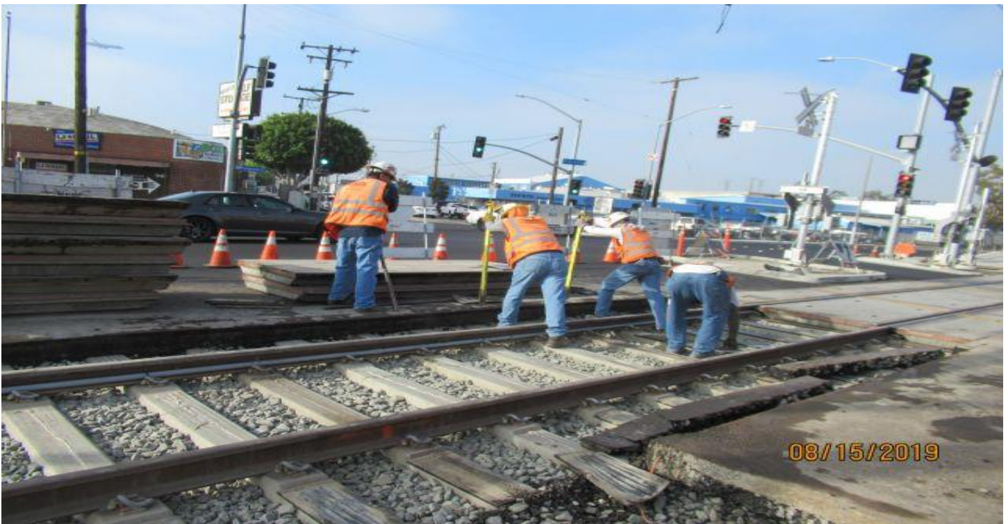
FLORENCE/HINDRY - HCC on NB track at Hindry grade crossing .
