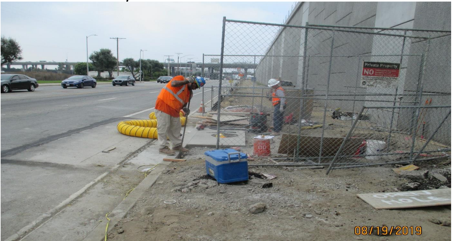
AVIATION/CENTURY- Stripping and finishing catch basin #4 on Aviation.
