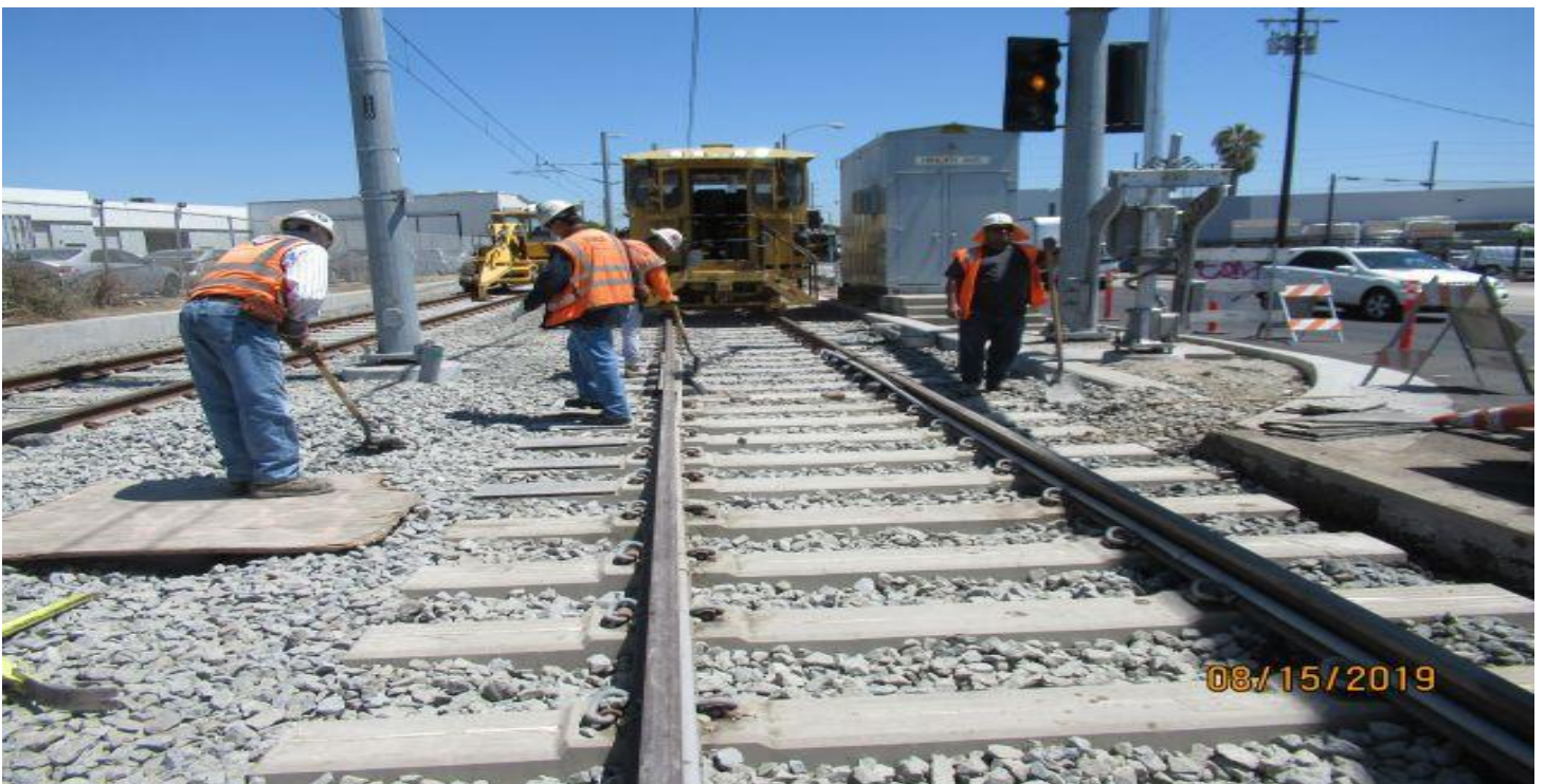
FLORENCE/HINDRY - HCC at Hindry grade crossing dressing tie cribs after re-tamping NB track.
