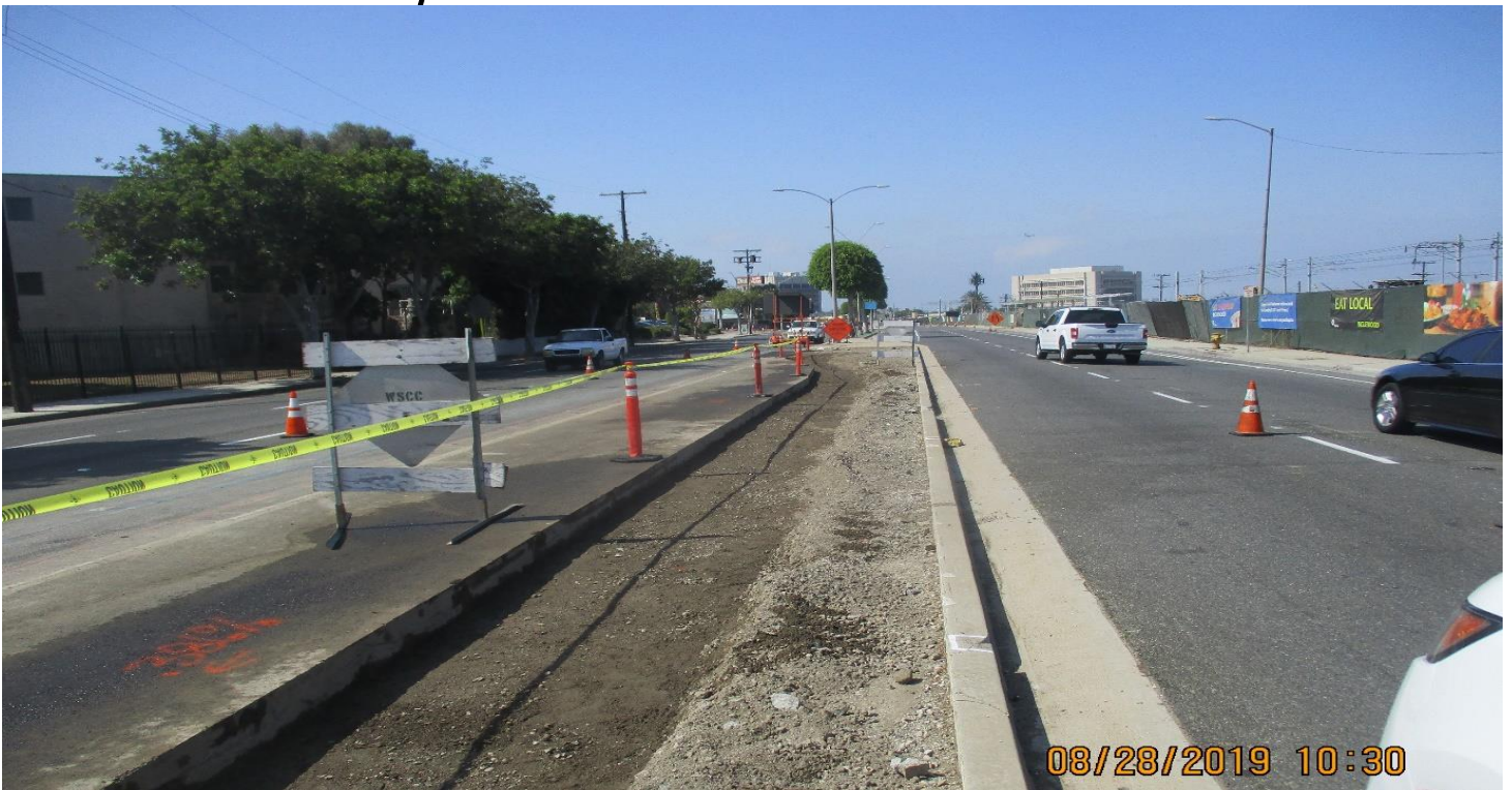
FLORENCE STREET - WSSC Cut and make grade to replace C&G at Florence island w Hillcrest.
