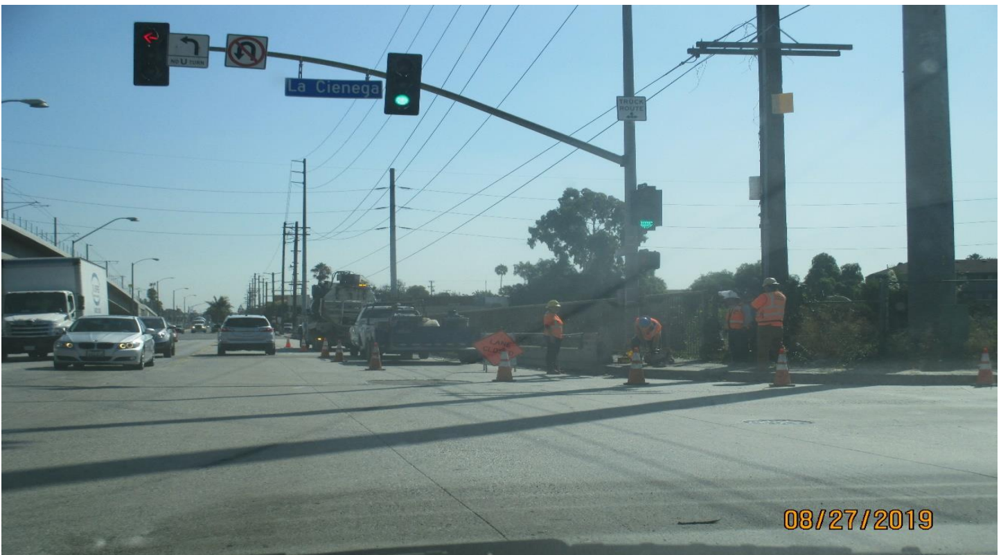
FLORENCE STREET - Potholing for utilities at La Cienega and Florence.
