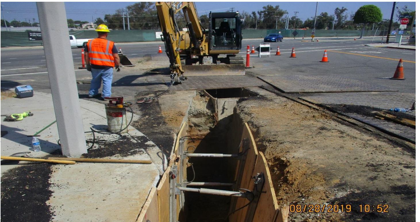
FLORENCE STREET- WSSC Excavate for SD lines at Locust and Florence.
