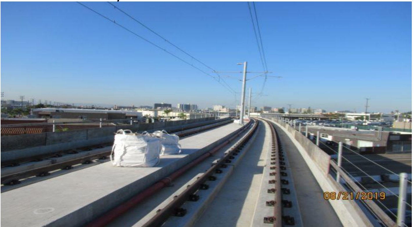
MANCHESTER BRIDGE- Manchester Bridge north end no construction being performed.
