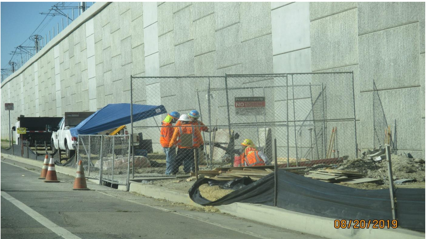
AVIATION/CENTURY- Stripping catch basin #4 on Aviation.
