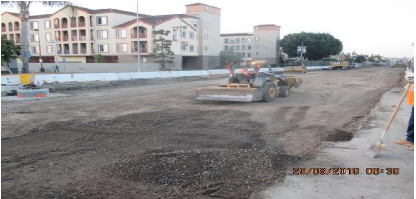
UG3- Continued backfill and compaction between 60th and 63rd Street.
