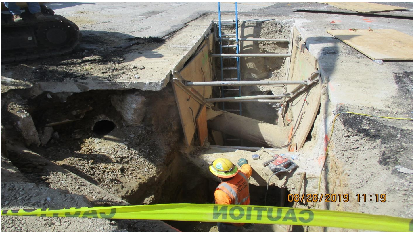
LA BREA BRIDGE- WSCC La Brea SD relocation.
