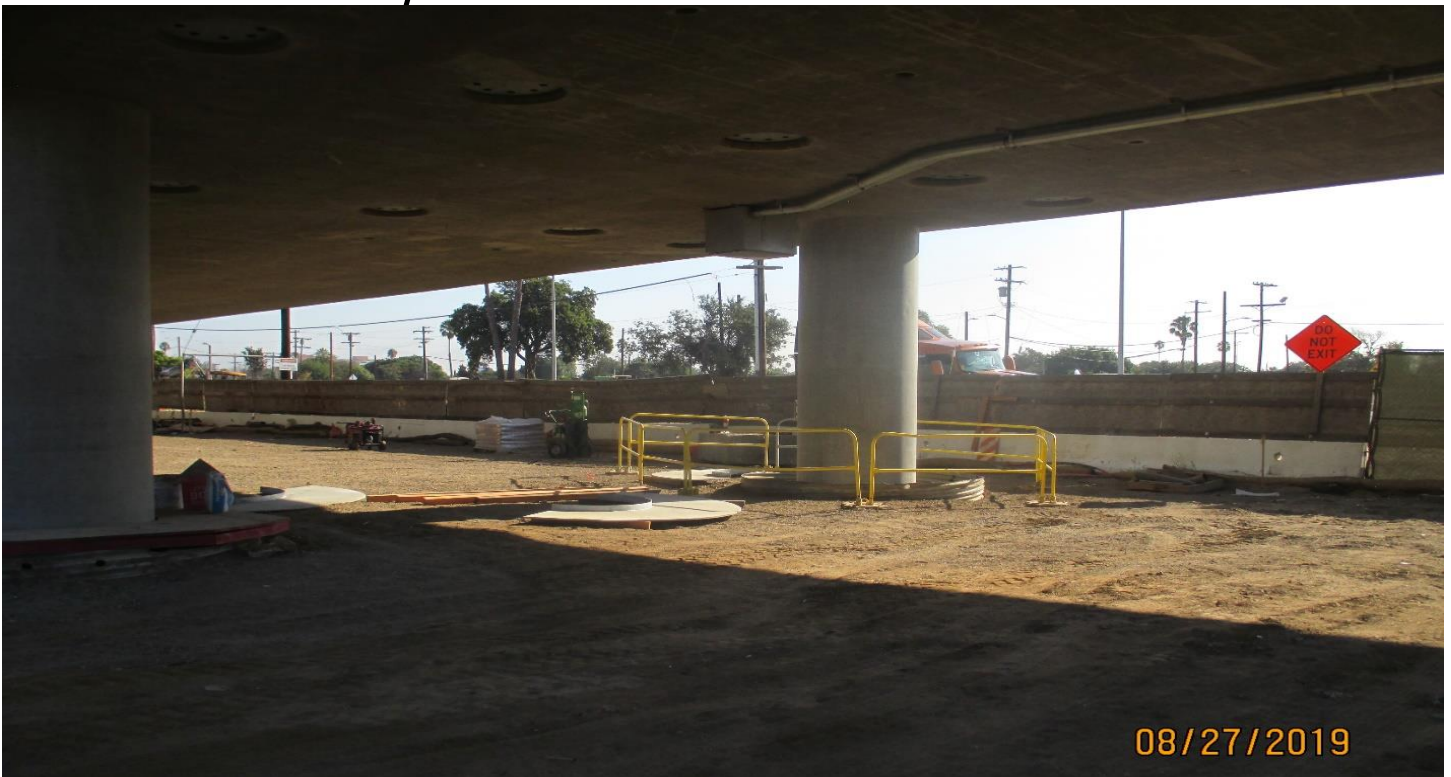
AVIATION/CENTURY- Installing the bent safety covers at the Aviation Station.
