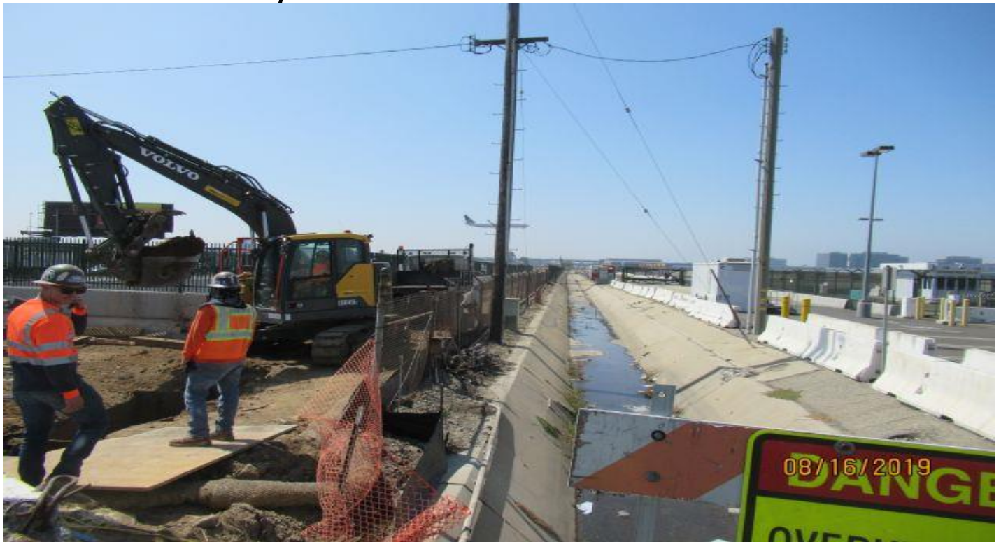
UG1- WA Rasis loading dump truck with native spoils at 104th street for UG1.
