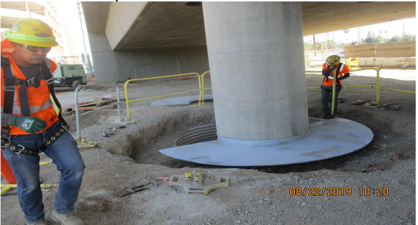
AVIATION/CENTURY- WSCC Placing CIDH insulator covers at Aviation bridge.
