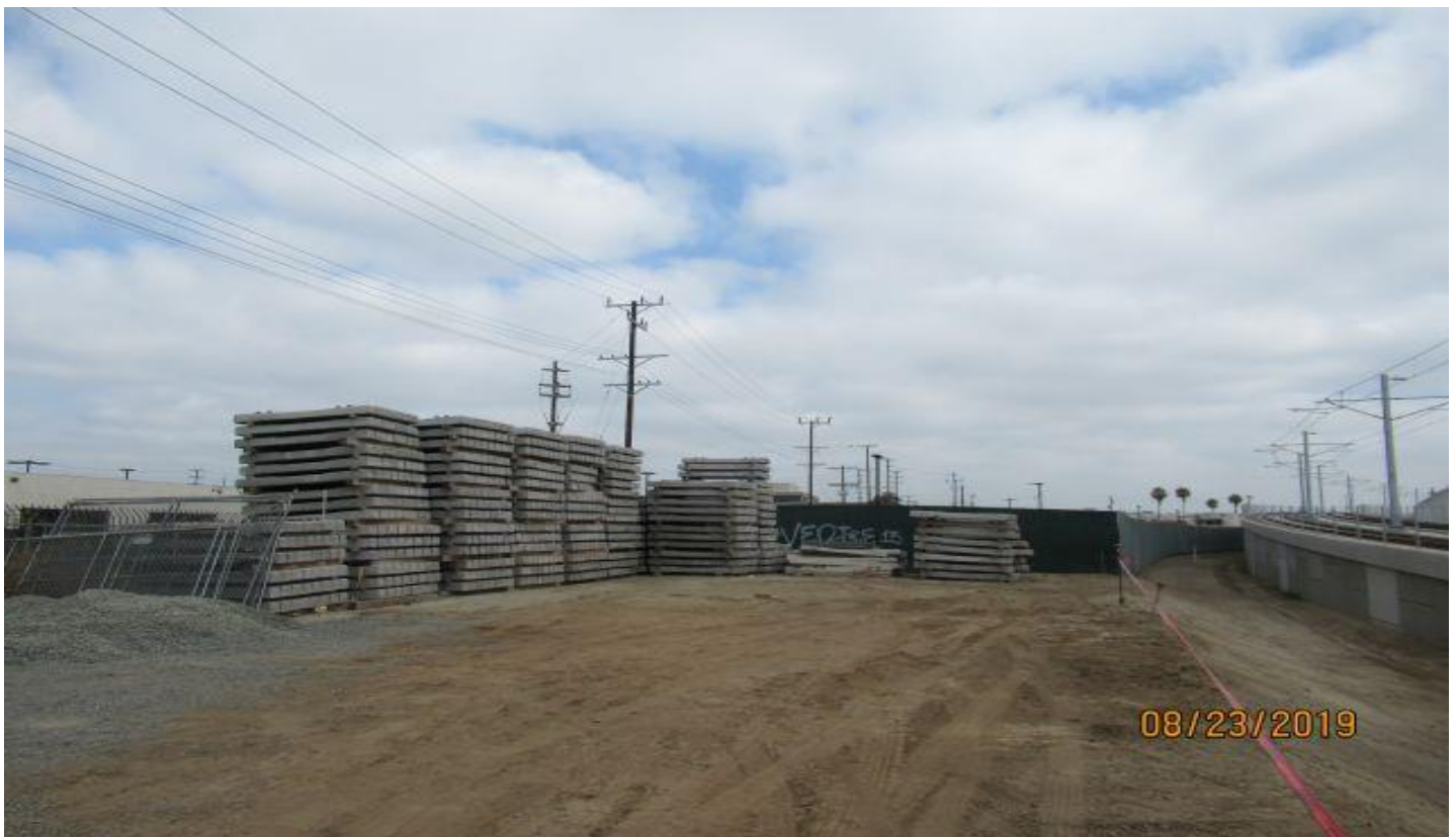
MANCHESTER BRIDGE- WSCC 8' common ties stacked near Manchester Bridge.
