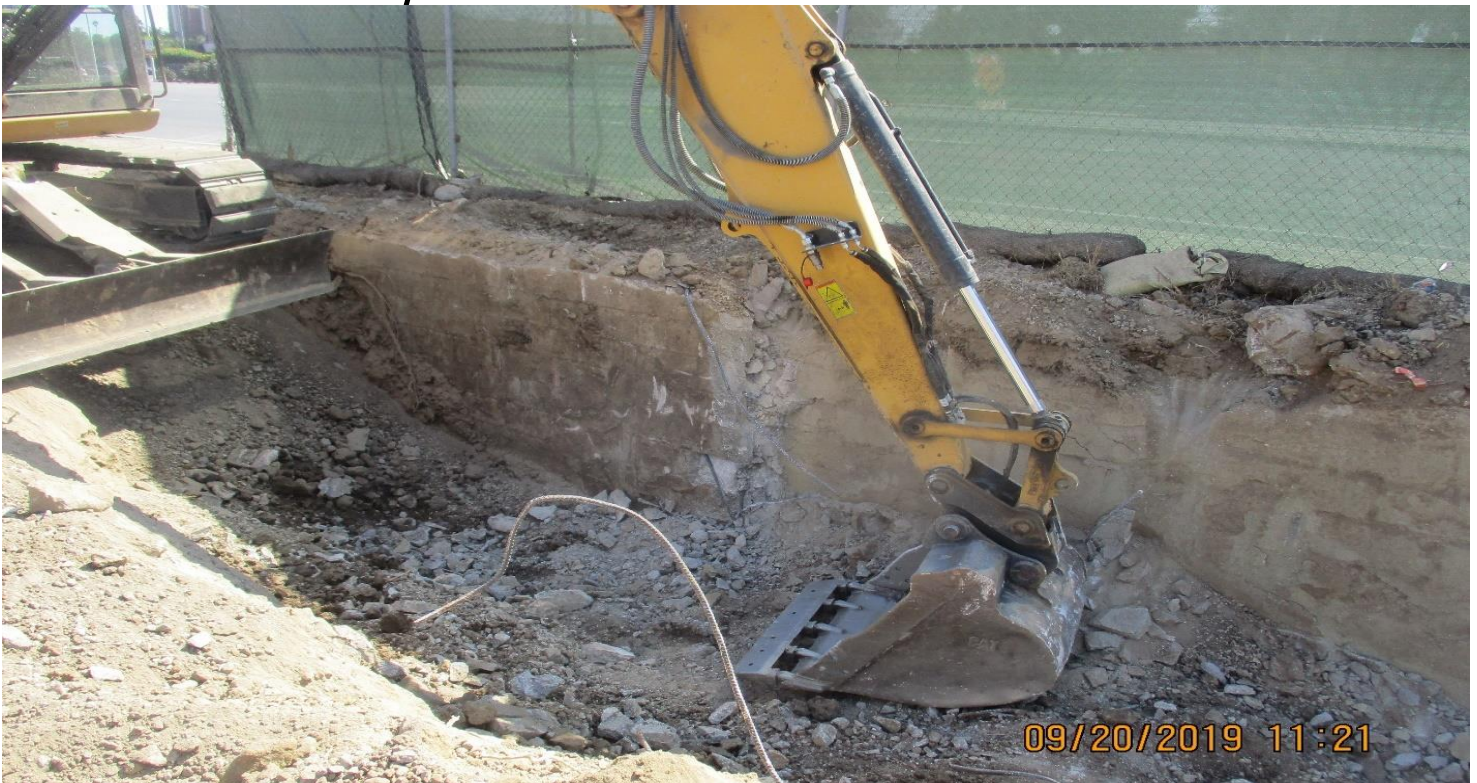
FLORENCE/LABREA STREET - WSCC Removing existing wall at La Brea parking lot.
