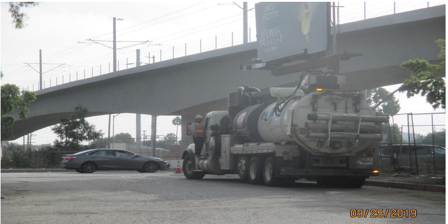
405 BRIDGE - Vacuum truck excavating for the 405-bridge abutment 1 COS protection.
