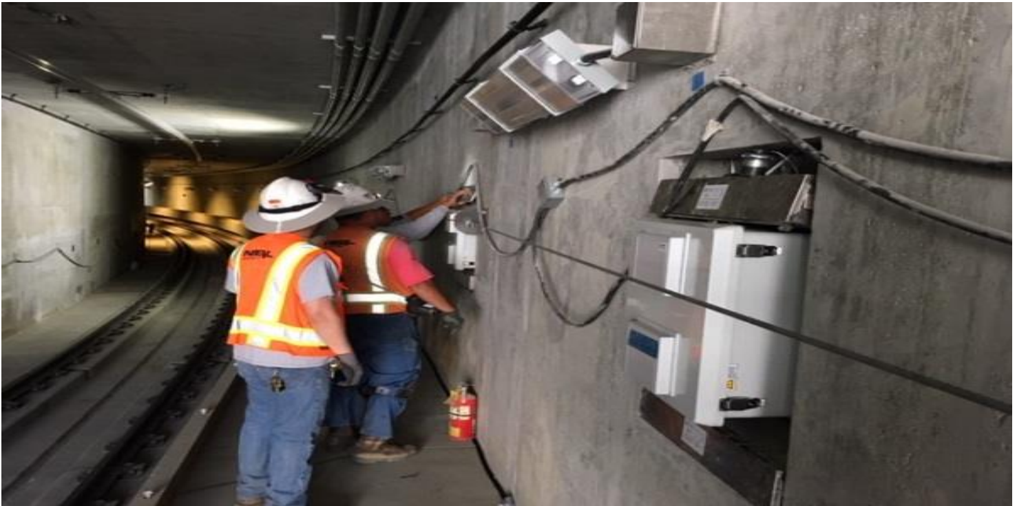
UG3- Installation of communications interface cabinet box at the southbound portal.
