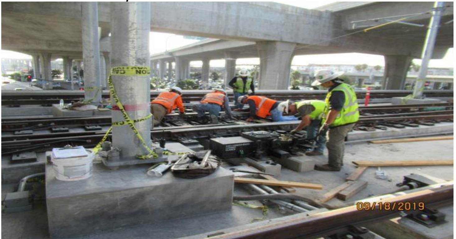
GREENLINE WYE- HCC & LKC performing adjustments on Movable Point Frog.
