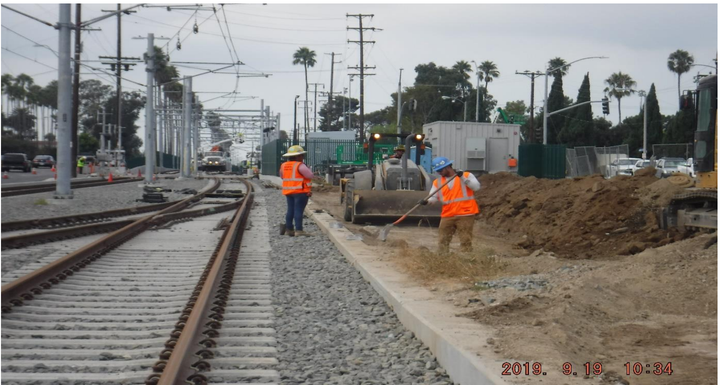
FLORENCE/WEST- Looking North- Grading work.
