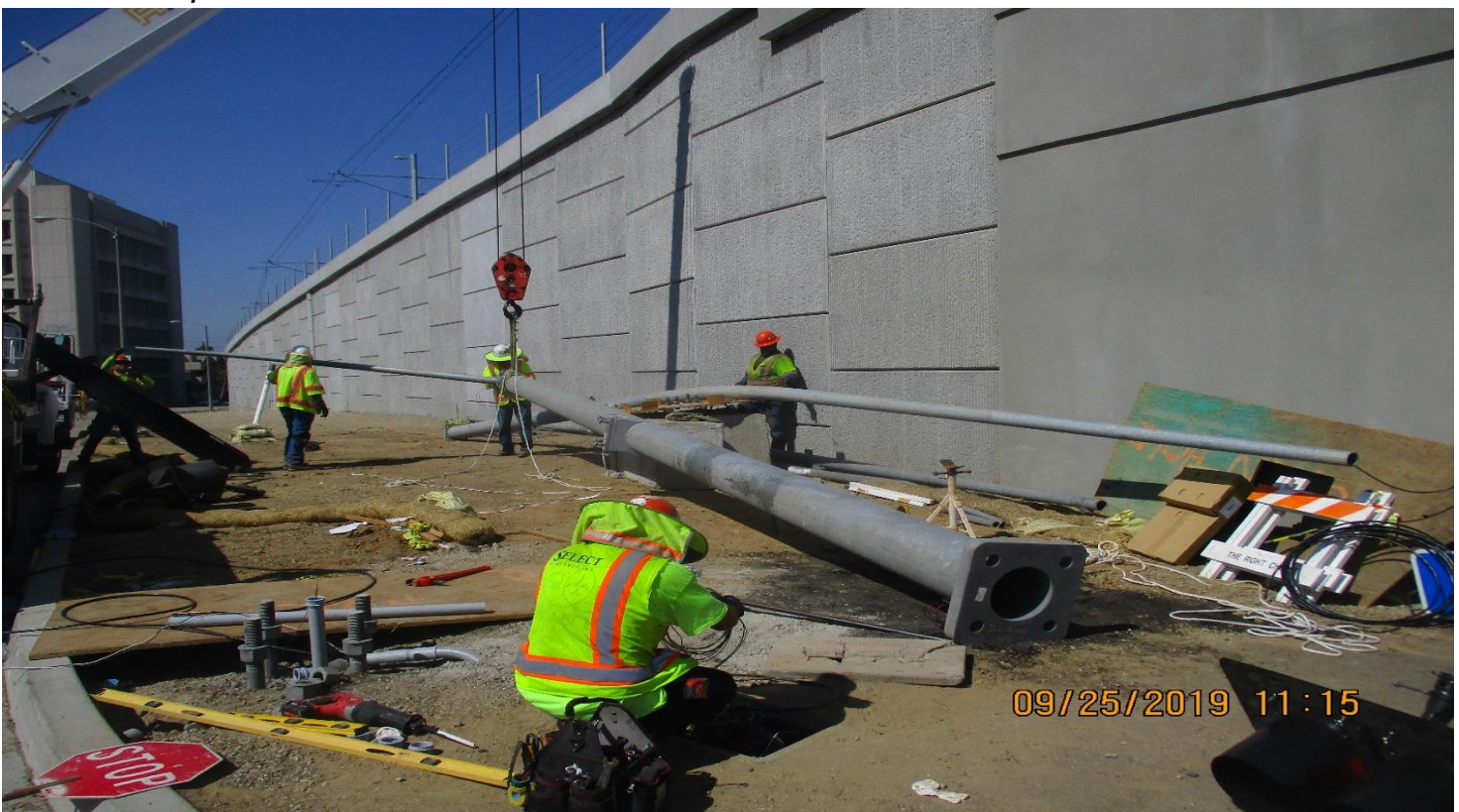
FLORENCE/LA BREA- Select Electric Stand TS and SL pole SEC of La Brea and Florence.
