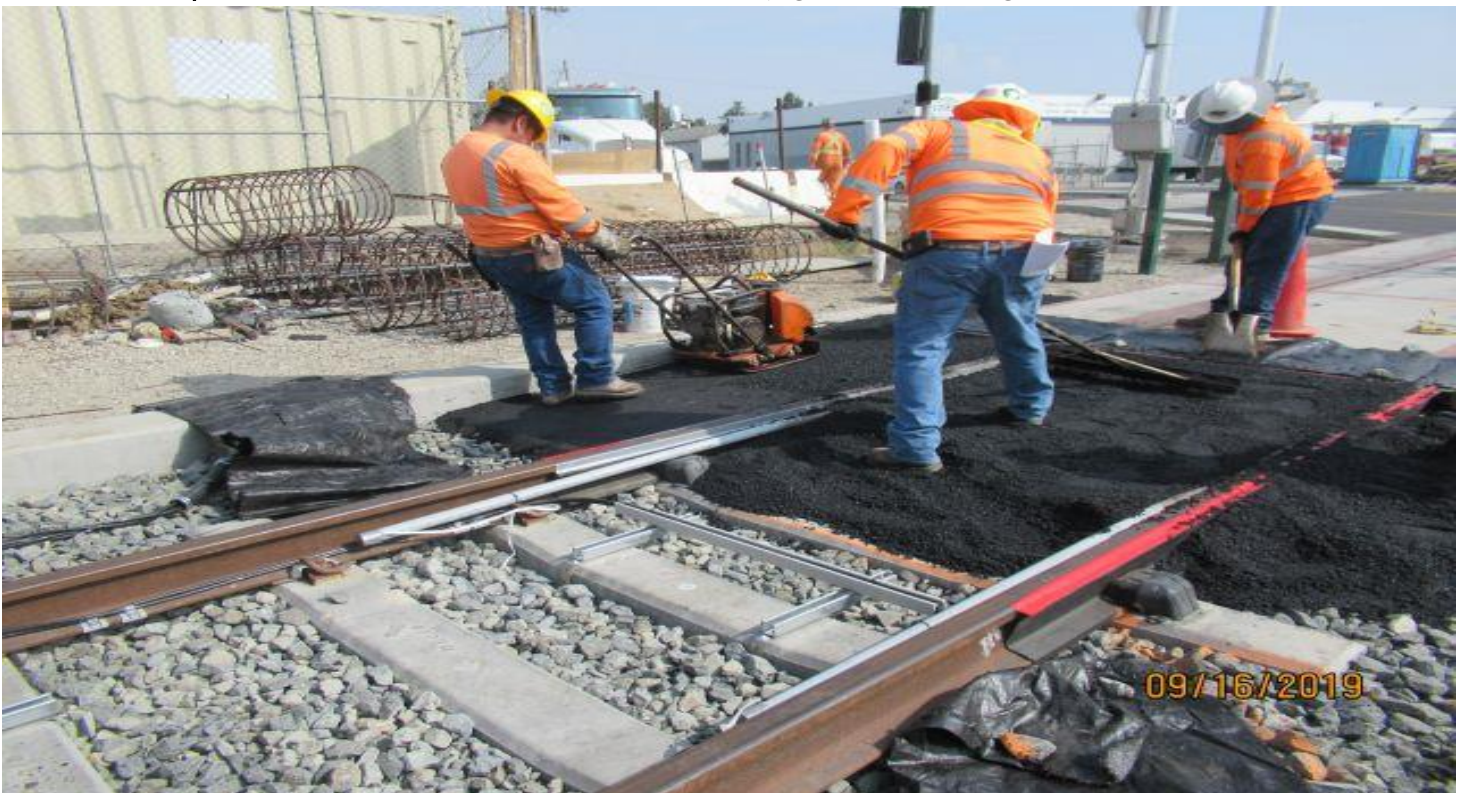
FLORENCE/HINDRY - WSCC compacting & Grading AC at Hindry Grade crossing STA 135+50.
