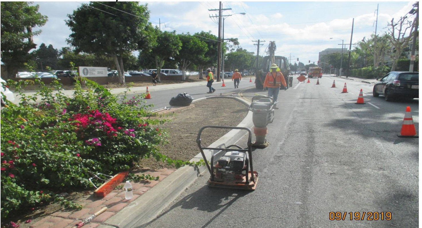
EUCALYPTUS STREET - Placing concrete for the median island on Eucalyptus.
