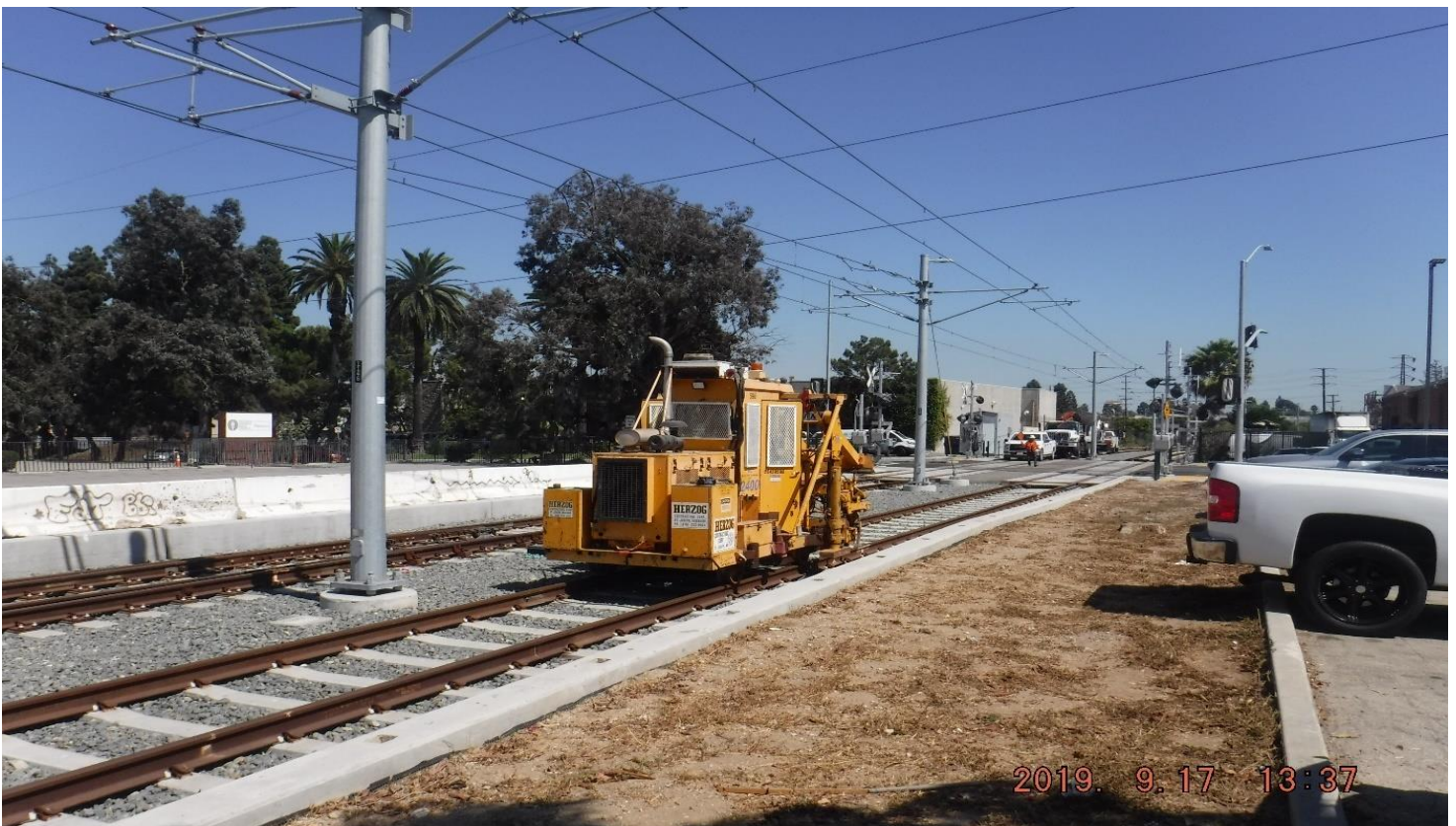
EUCALYPTUS STREET - Looking North- Moving hi-rail equipment.
