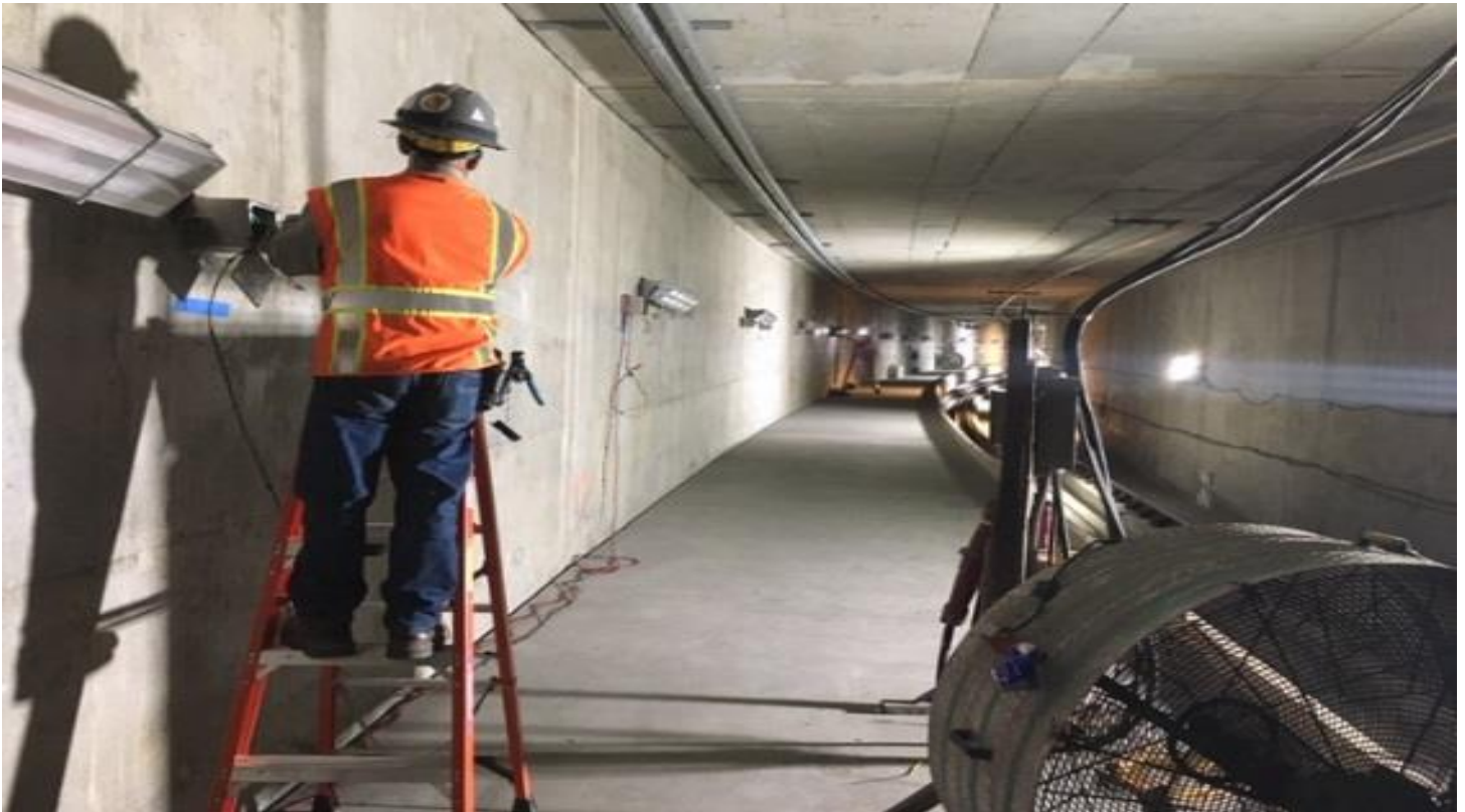
UG4- Continued lighting installation on both sides of the northbound tunnel.
