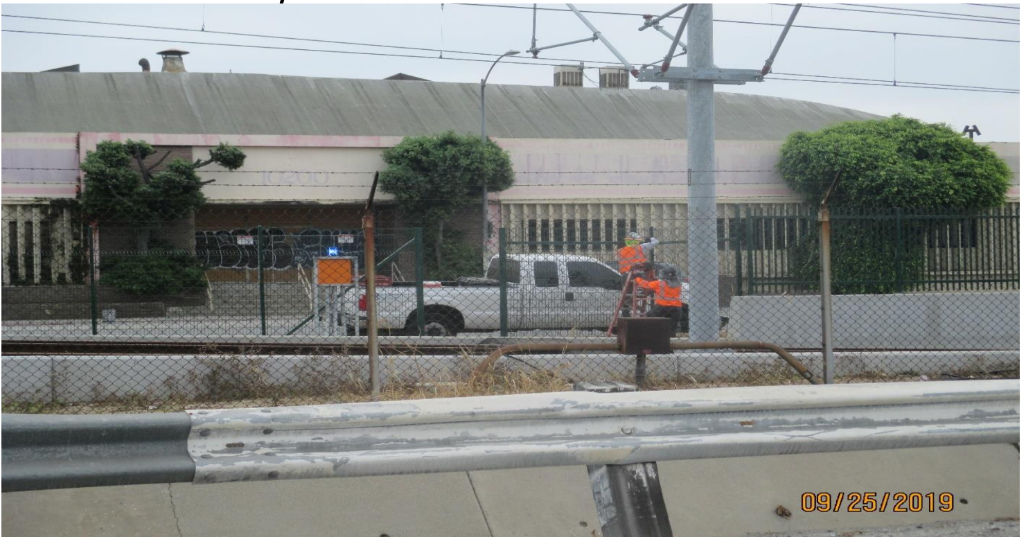
UG-1- Wire mesh gate installation at UG-1.
