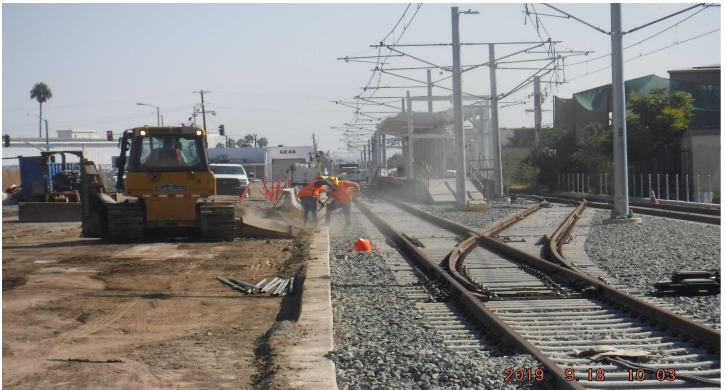
FLORENCE/WEST- Looking North- Grading work.
