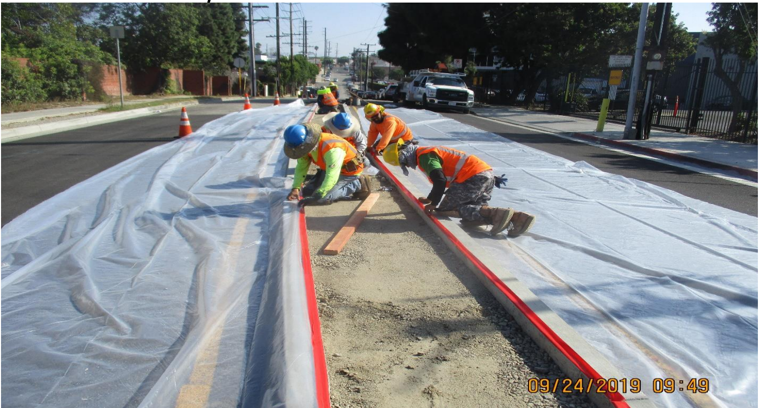
FLORENCE/IVY - WSCC Worked on SD lines at Locust and Florence.
