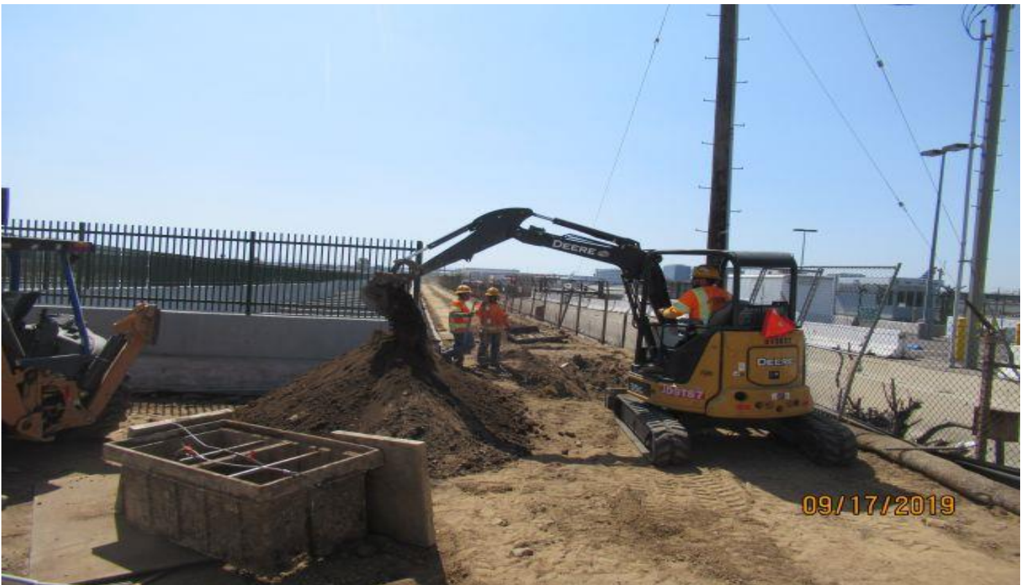
111 TH STREET- WA Rasic excavating for relocating Quest hand holds.
