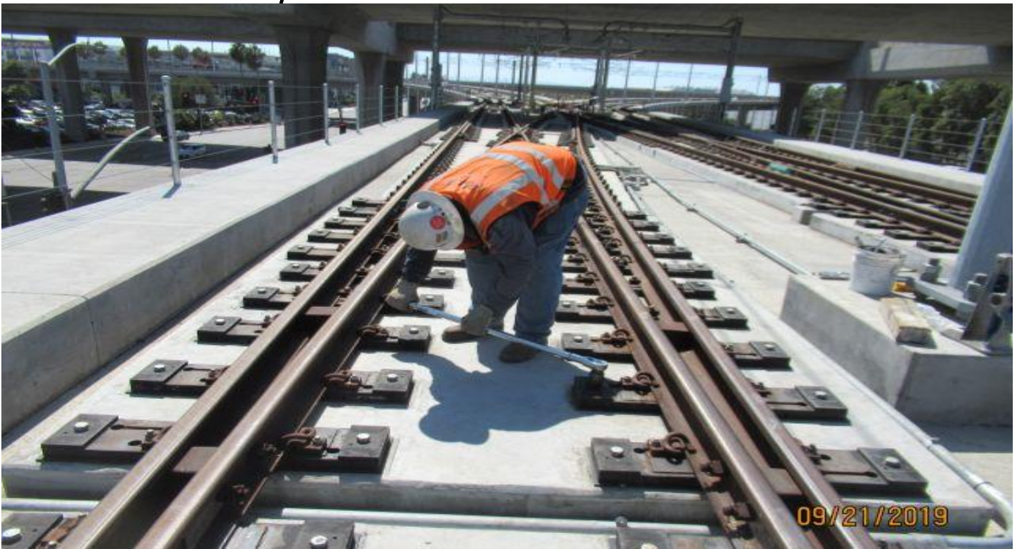
GREENLINE WYE- HCC retorquing fastener bolts on NB track.
