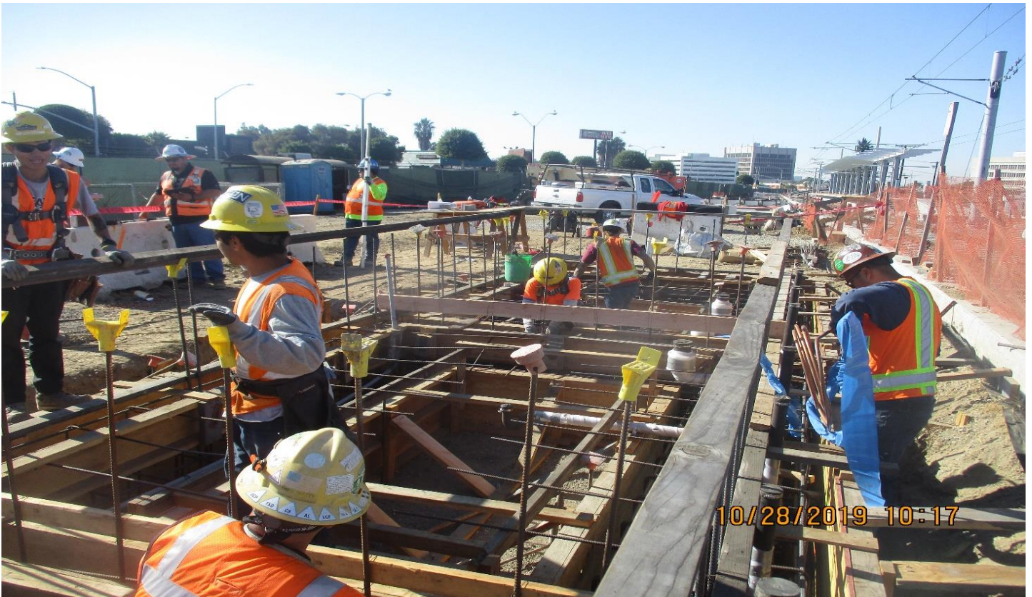
FLORENCE/LA BREA - WSSC Forming to place concrete foundation at restroom building.
