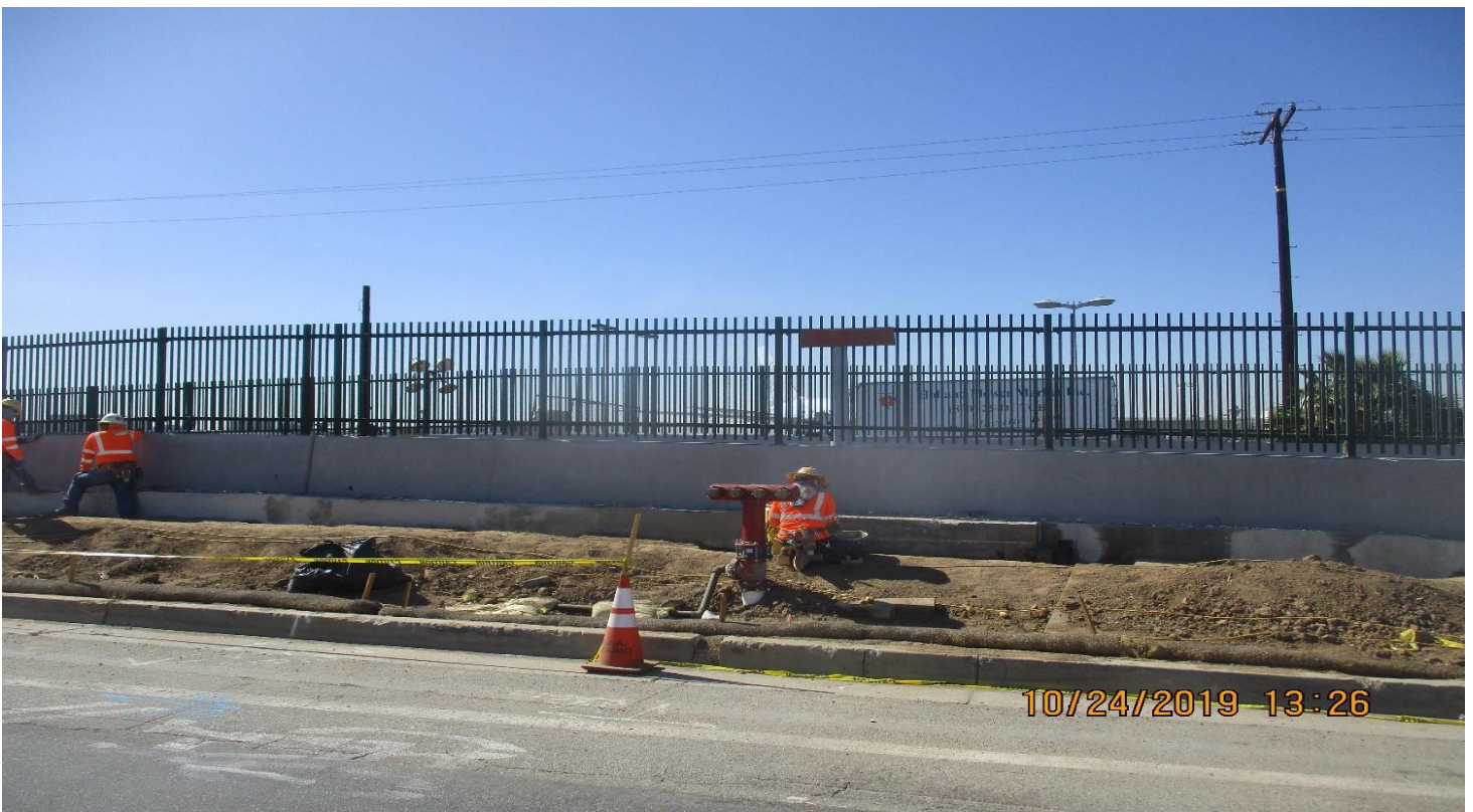
UG-1- WSCC Concrete finishing UG-1 wall south end of UG-1
