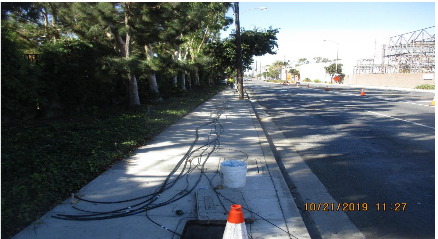
FLORENCE/IVY – Select Electric Pulling cable at Ivy intersection.
