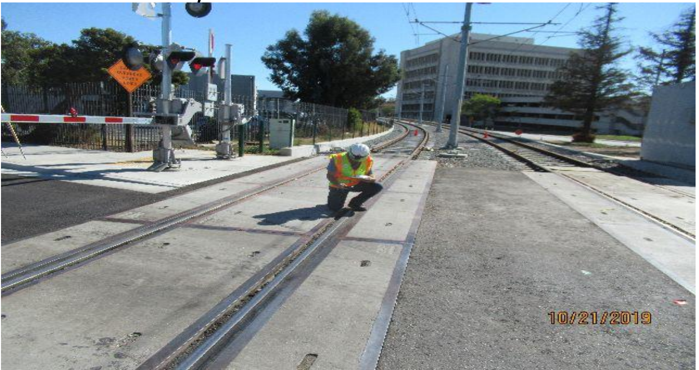
FLORENCE/IVY – Metro track inspector walking grade crossing for damaged rail conditions.
