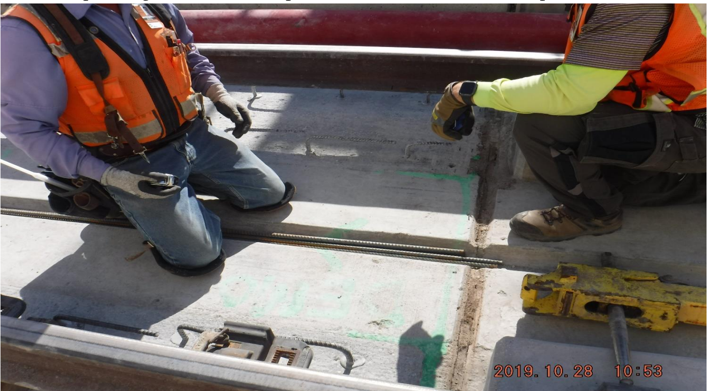
UG3- STA279+08_ Looking North_ Plinth demo_ Re-work_ QC_UG3_Victoria.
