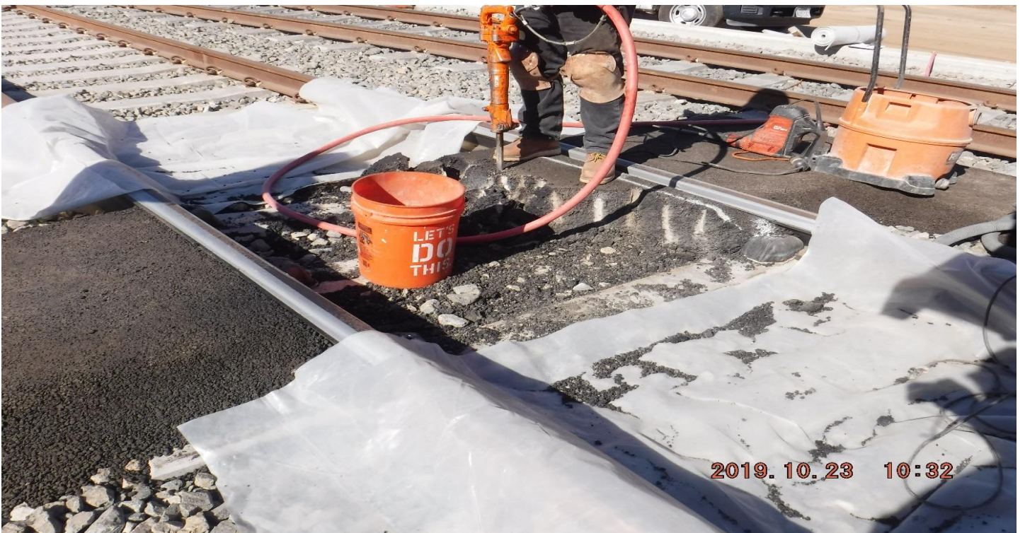
FLORENCE/WEST- STA261+63_ Looking South_ New AC walkway demo 4 system work.
