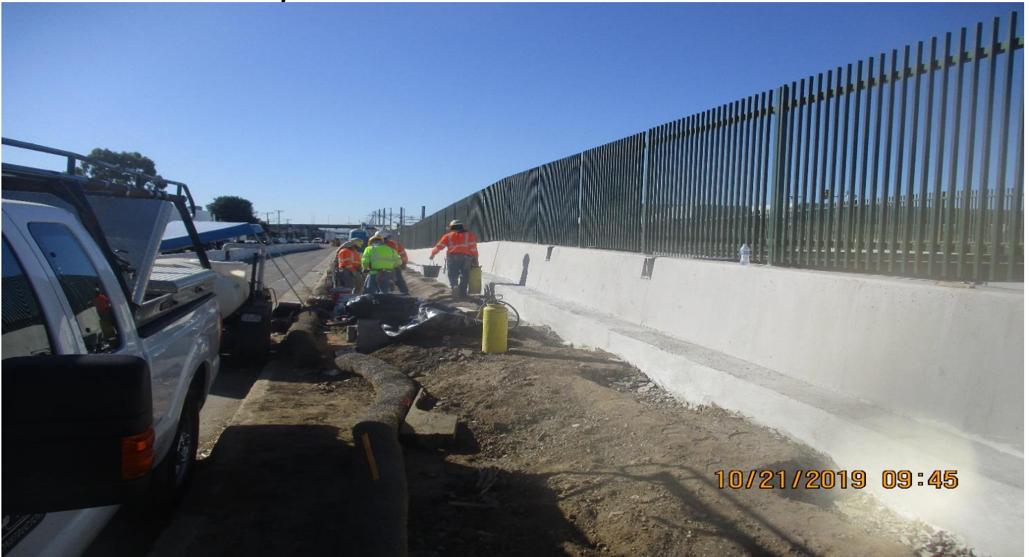
UG-1- WSCC Conc finisher UG-1 Wall.
