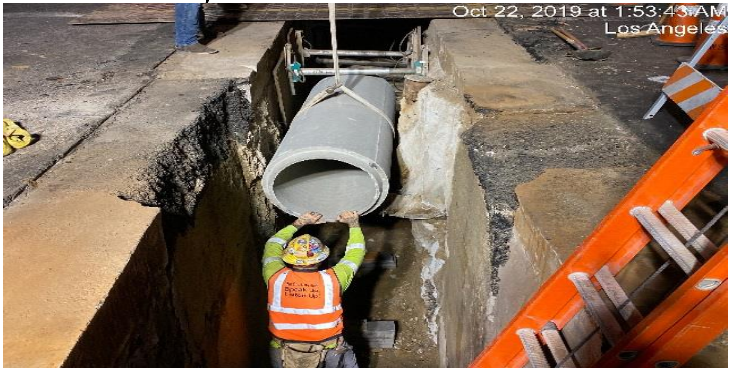
LEIMERT PARK STATION- Excavation at W – Line storm drain to install remaining concrete pipe on the intersection of 43rd St & Crenshaw Blvd.
