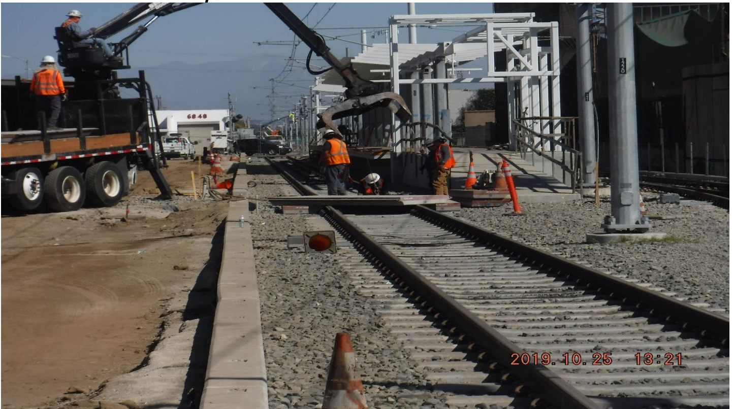
FLORENCE/WEST- STA262+74_ Looking North_ Install crossing panels 4 pedestrians.
