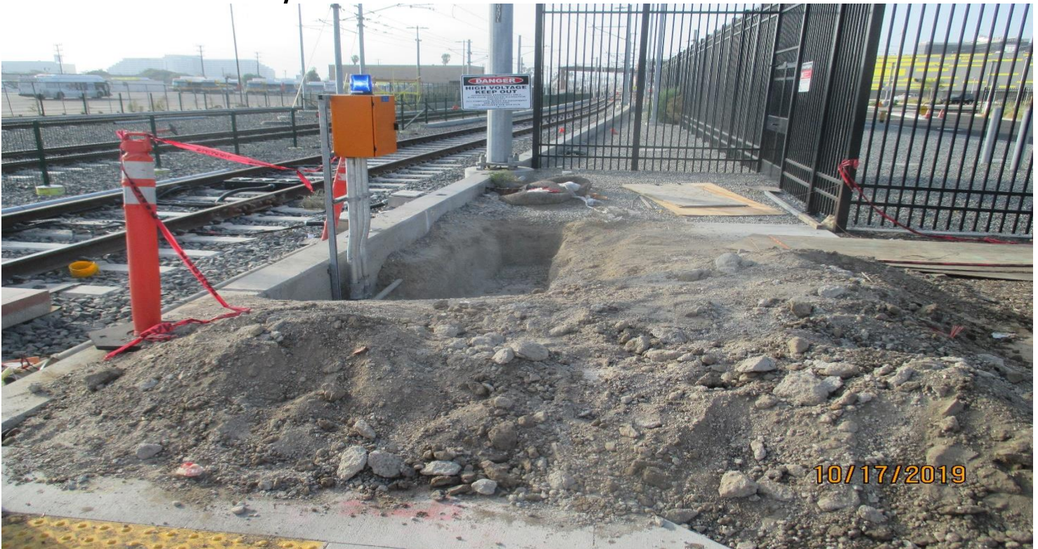
ARBOR VITAE – BLS Trip Station at Arbor vitae prior to backflying the conduits.
