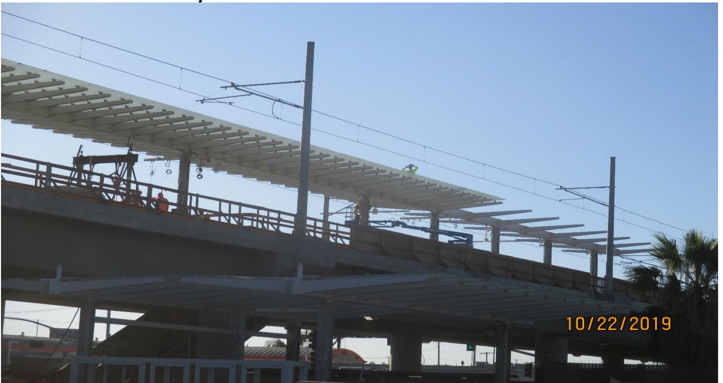
AVIATION STATION – Aviation Station platform canopy glass reinstatement.
