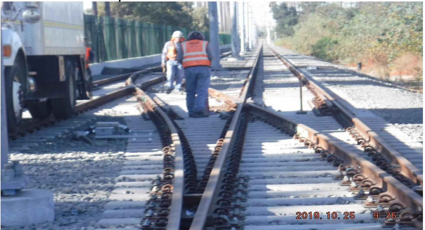
HIGH STREET- STA246+70_ Looking South_ Install tie plates frog 10Q2LHXO_rework.
