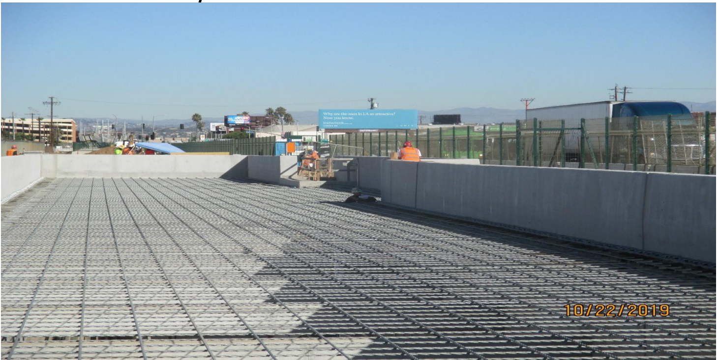
UG-1- Cable barrier installation at UG-1.
