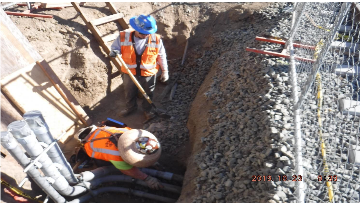
OAK STREET - STA161+10_ Looking North_ LT shoulder_ Excavation_ PUNCH LIST.
