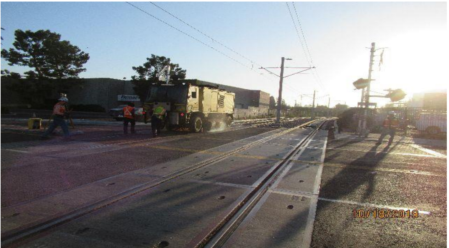
EUCALYPTUS STREET - Profile grinder inside Eucalyptus grade crossing SB #3 track STA 182+00.
