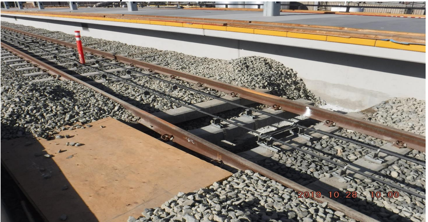
FLORENCE/LA BREA - STA210+00_ Looking South_ TK ballast disturbance for water line.
