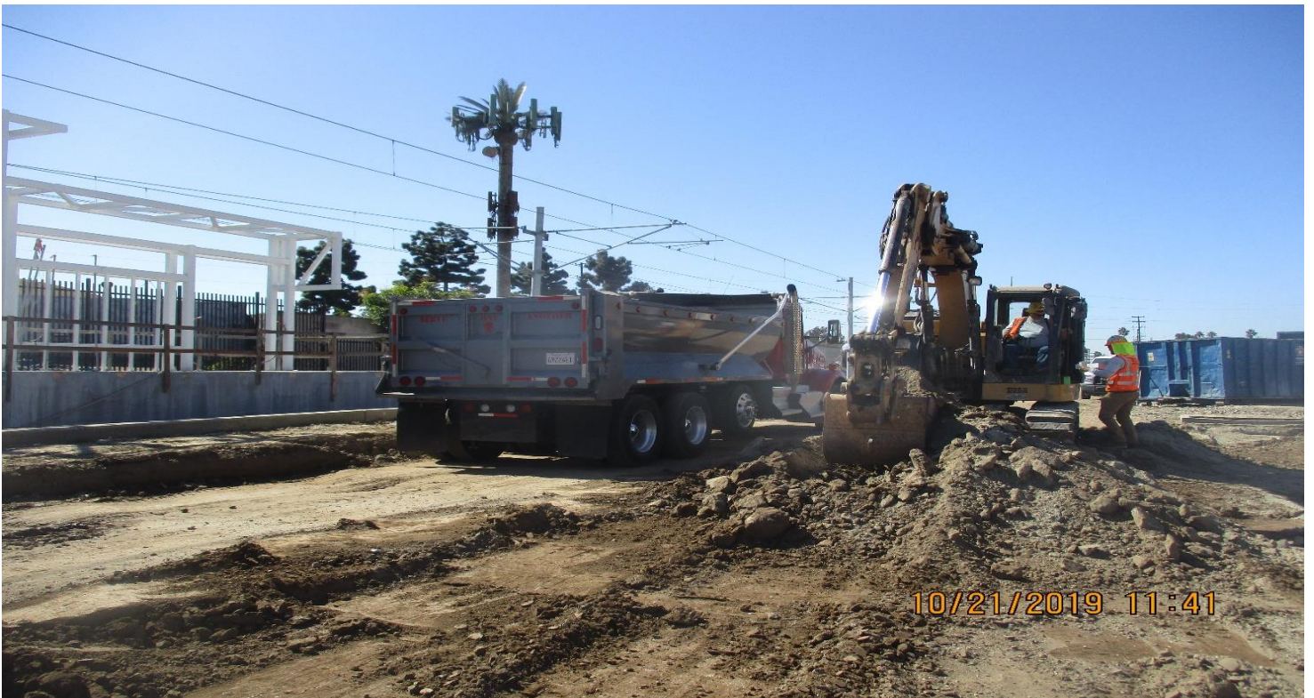
UG-1- WSCC Concrete finisher UG-1 Wall.
