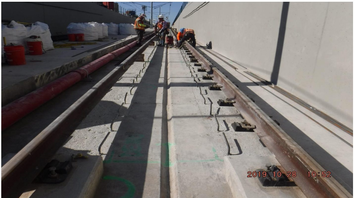
UG3- STA279+68_ Looking South_ Plinth demo_ Re-work_ UG3_ Victoria.
