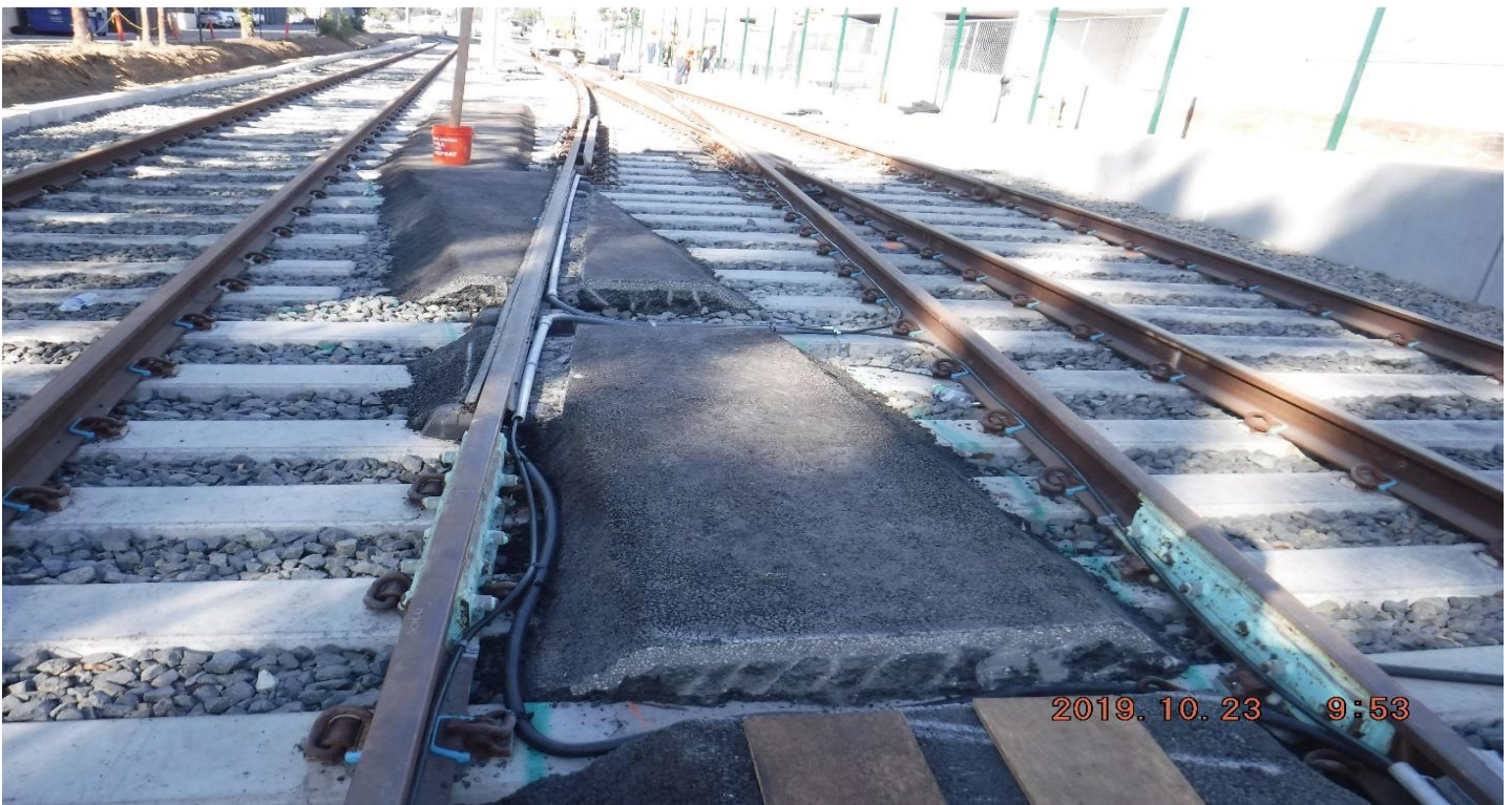
EUCALYPTUS STREET - STA171+30_ Looking South_ System work & AC walk demo.
