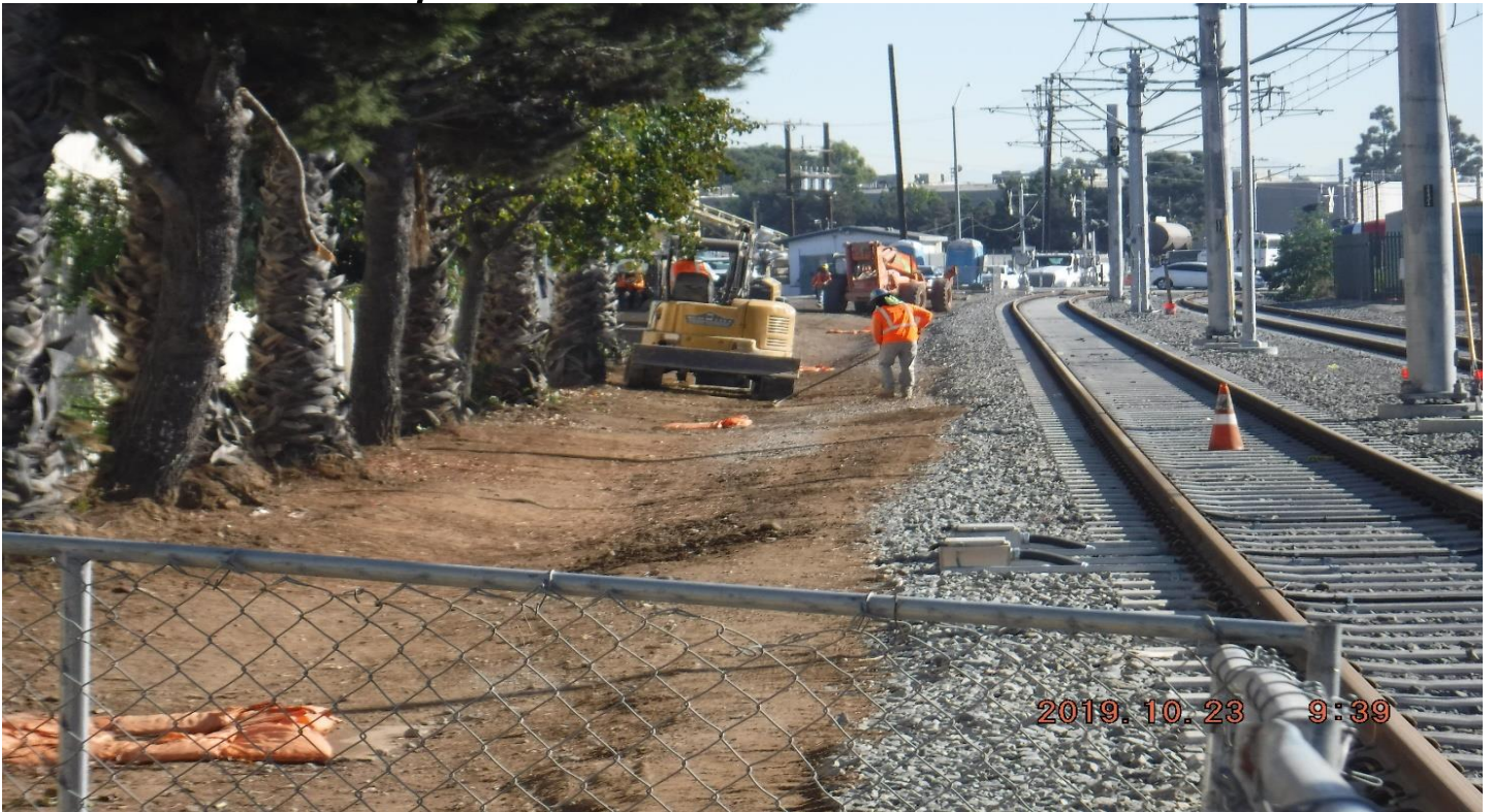
OAK STREET - STA161+20_ Looking North_ LT shoulder_ GR work.
