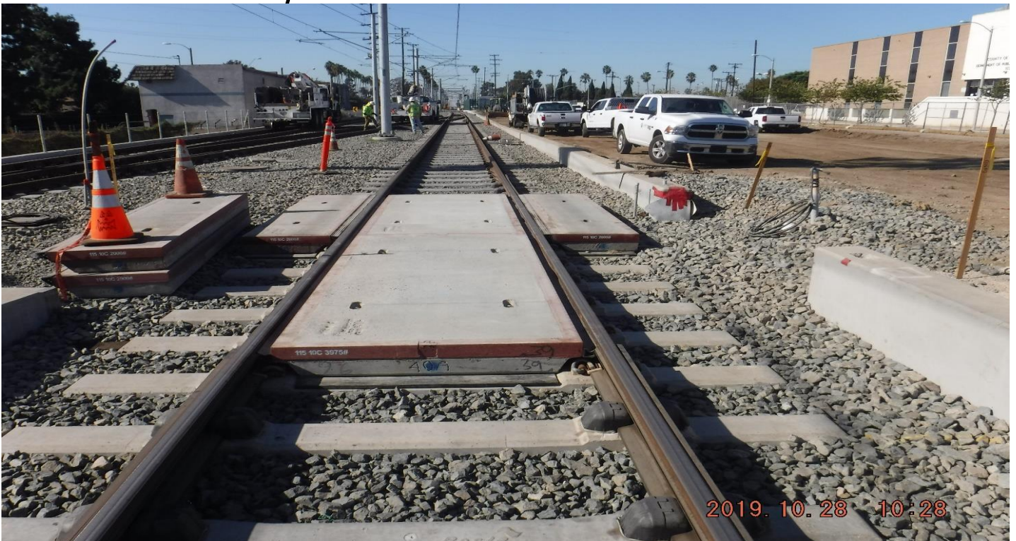
FLORENCE/WEST- STA262+74_ Looking South_ Status install crossing panels for pedestrians.
