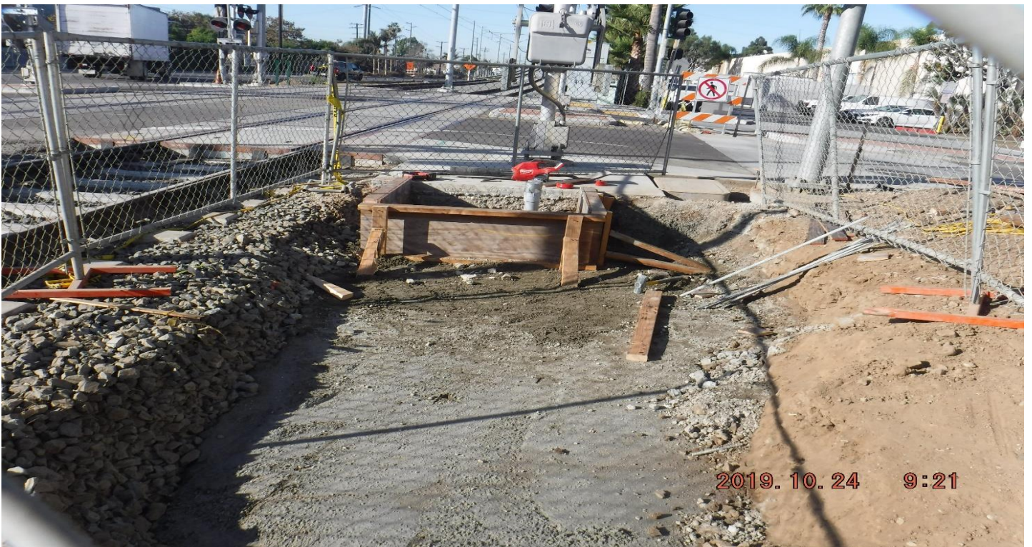
OAK STREET - STA161+20_ Looking South_ LT shoulder_ Excavation backfilled_ PUNCH LIST.
