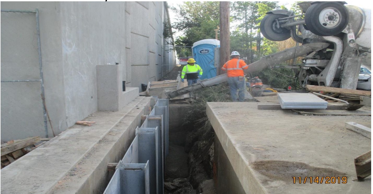
GUIDEWAY AT 405- Slurry backfill for the COS protection structure at abutment 1 of the 405 bridge.
