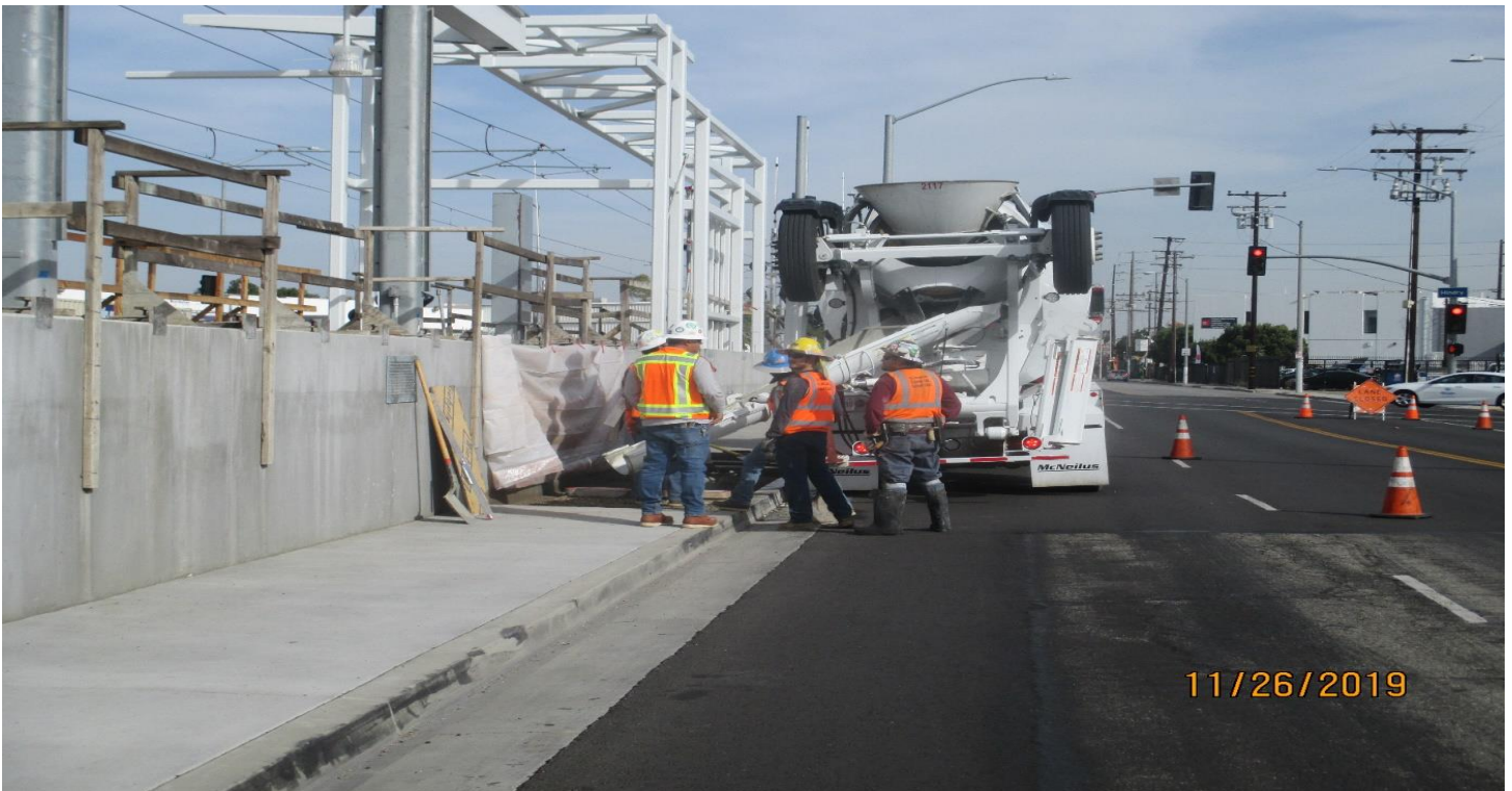
WESTCHESTER STATION – Placing concrete for some sidewalk panels on Florence at the Westchester Station.
