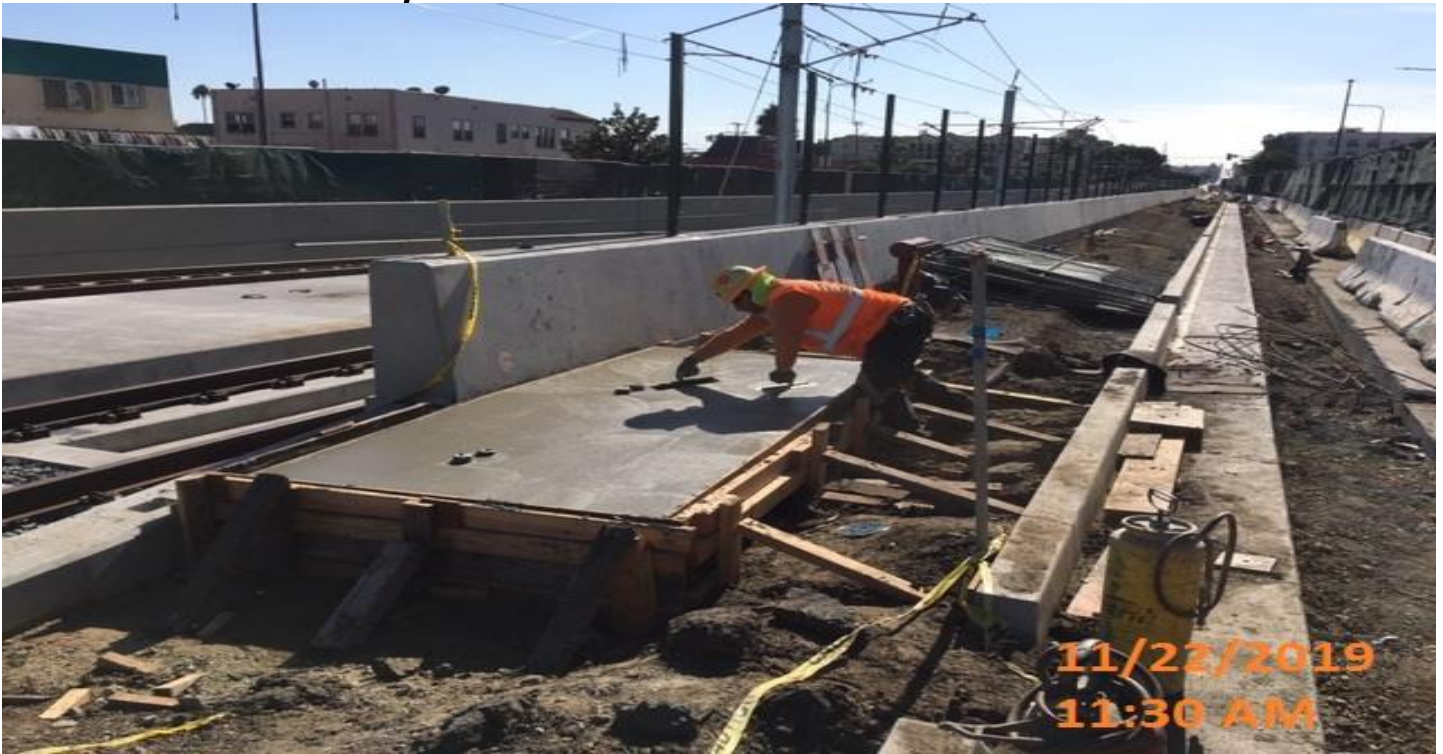
UG3- Smoothing surface to placed concrete at the north end portal.
