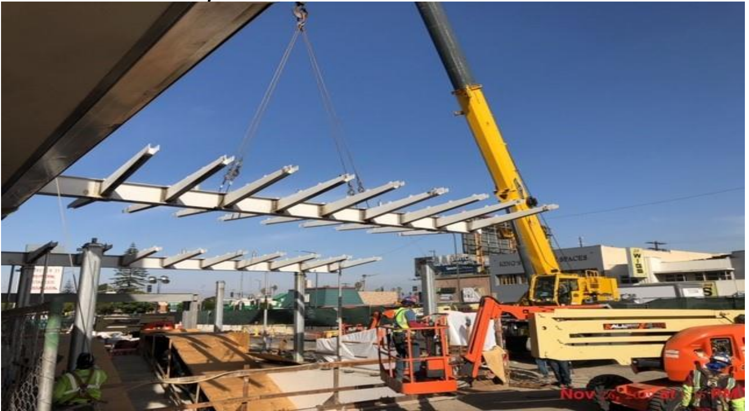
MARTIN LUTHER KING JR. STATION- Setting canopy section pieces over the main entrance of the portal at the plaza level.
