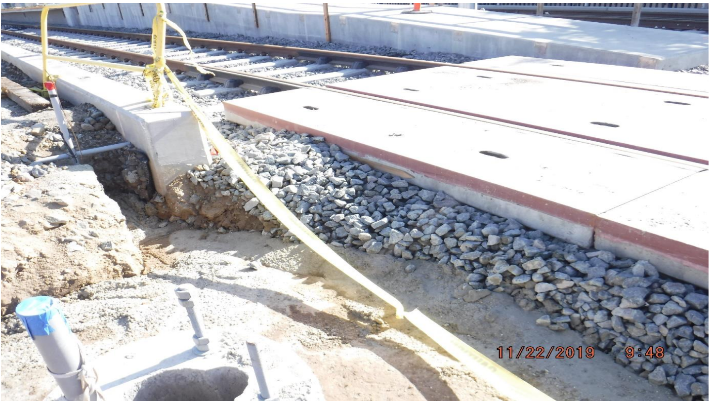
FLORENCE/WEST – STA262+68_ Looking North_ Disturbed track ballast.
