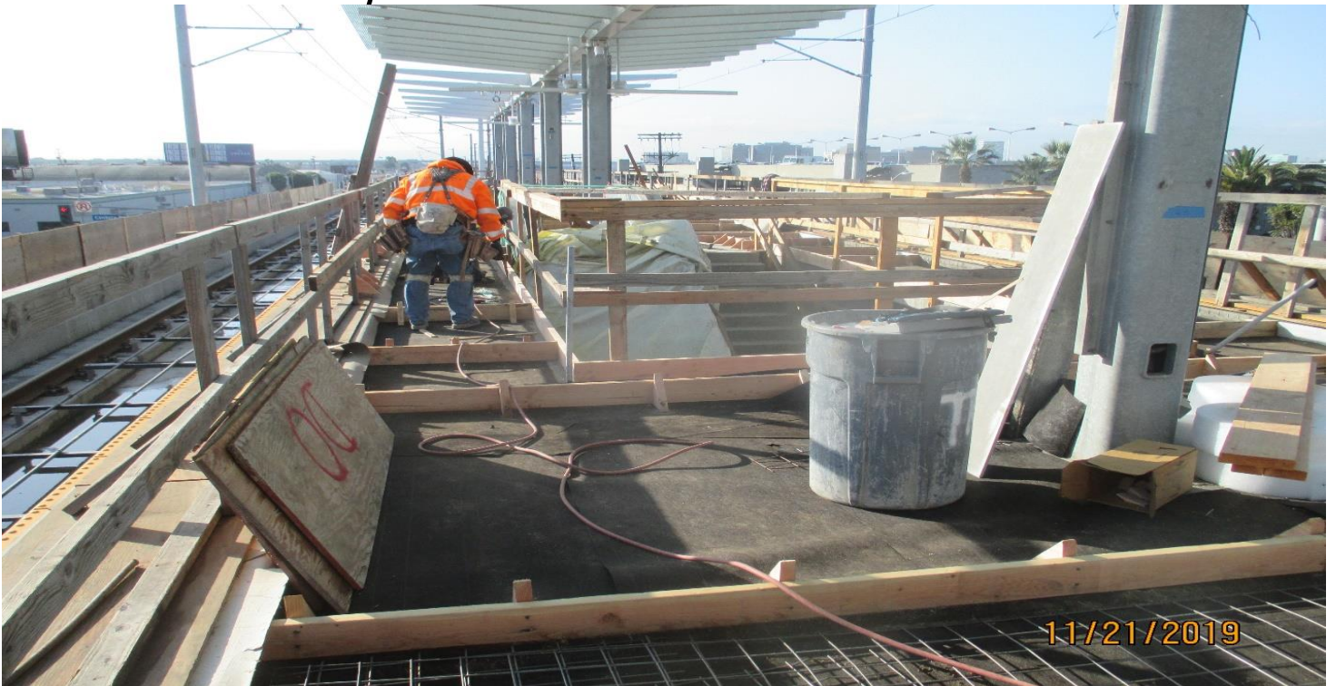
AVIATION STATION – Setting forms for the topping slab for the Aviation Station platform.
