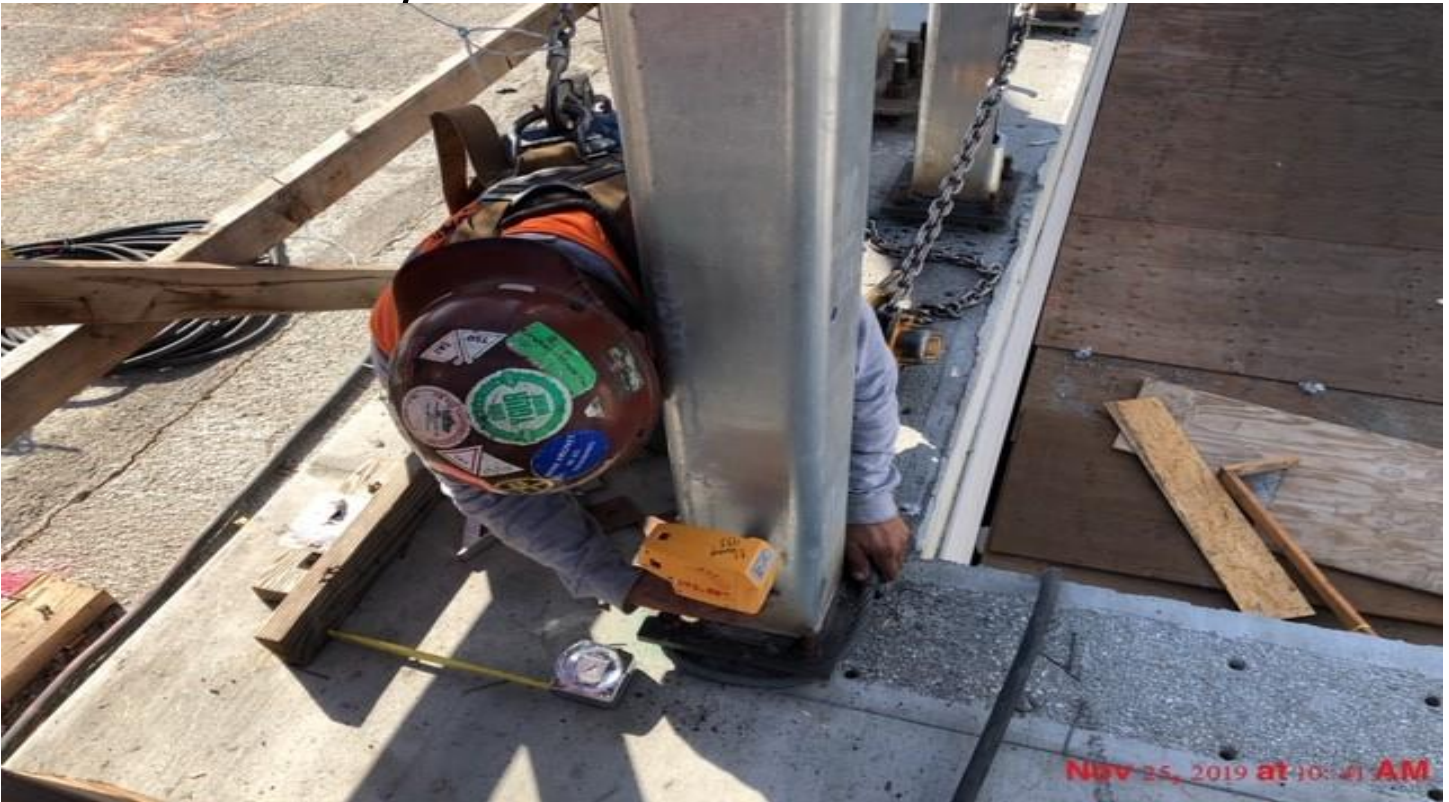
EXPOSITION/CRENSHAW STATION – Installation of windscreen frames for the main entrance portal at the plaza level.
