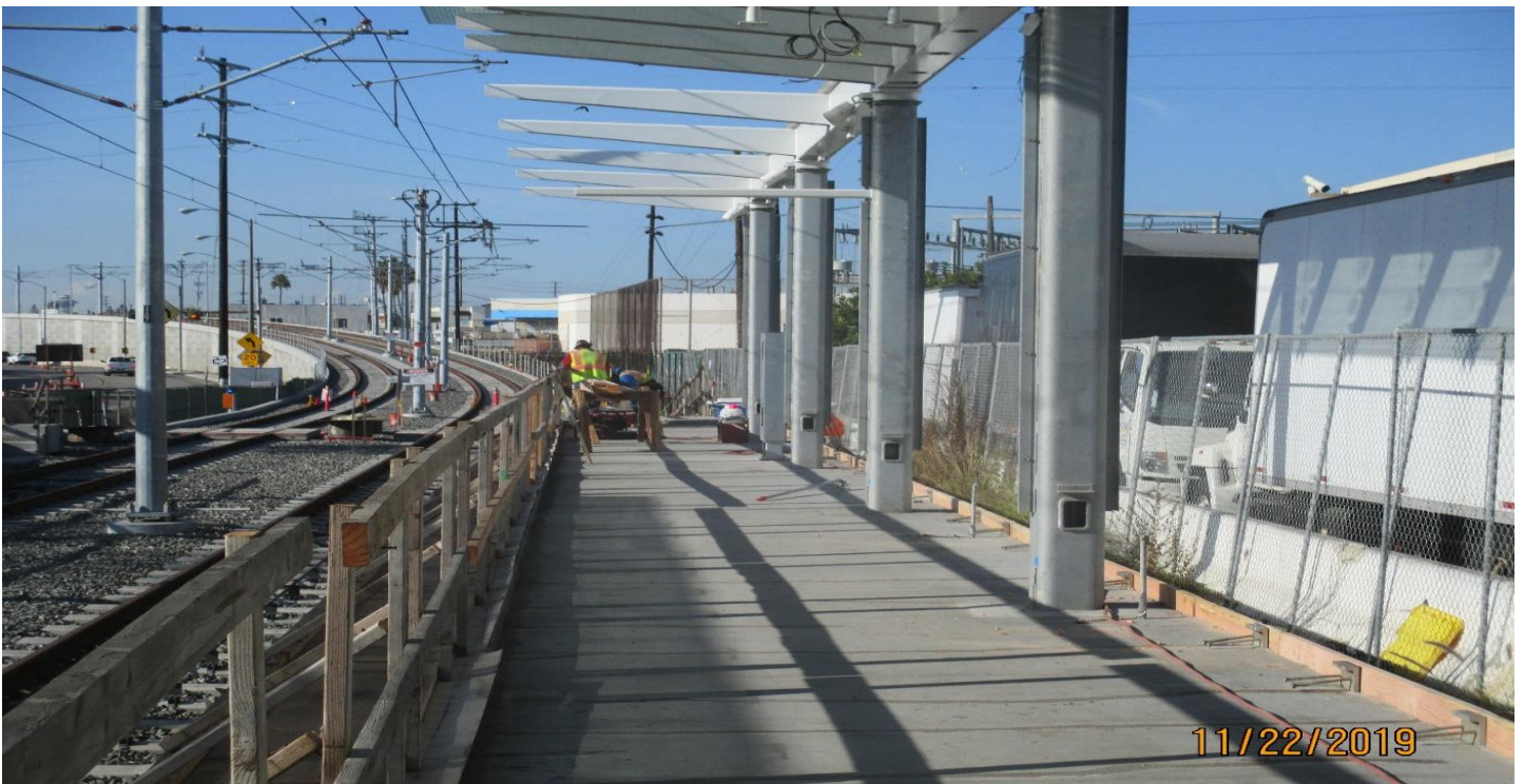
WESTCHESTER STATION – Setting forms for the Westchester Station SB platform topping slab.
