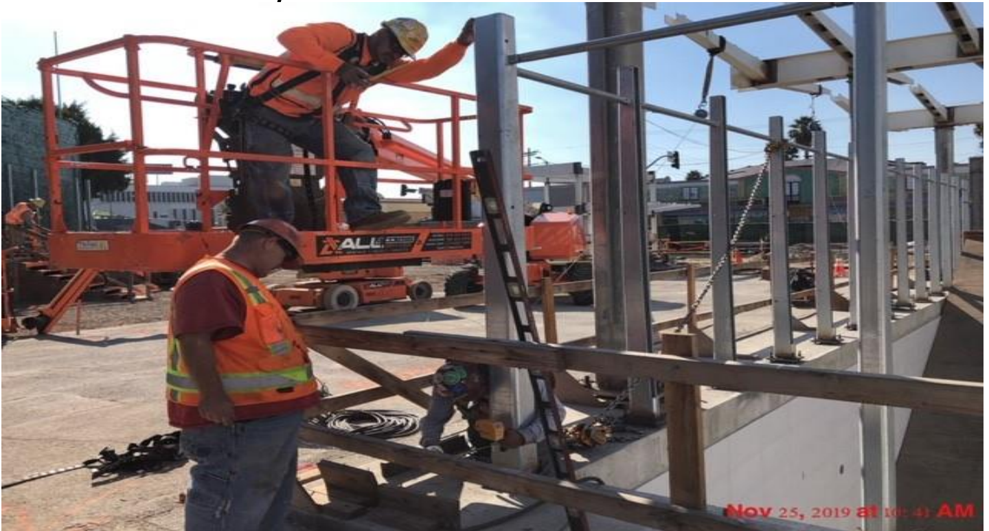
LEIMERT PARK STATION- Continued surveying of the wind screen base plate for the main entrance portal at the plaza level.
