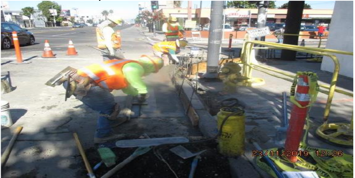
HYDE PARK- Curb and gutter placement on the southeast corner of Hyde Park Blvd & Crenshaw Blvd.
