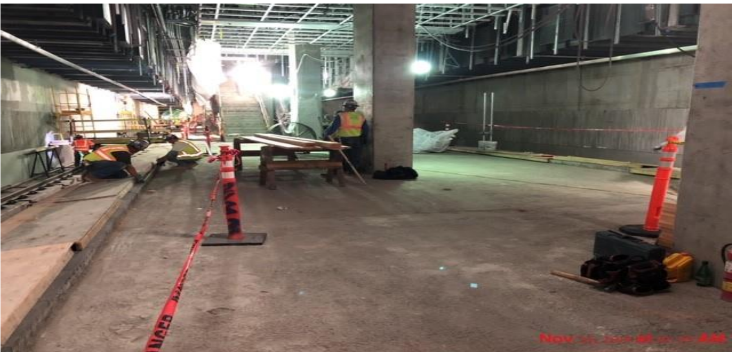
LEIMERT PARK STATION- Laying and forming for architectural topping slab at the platform level.
