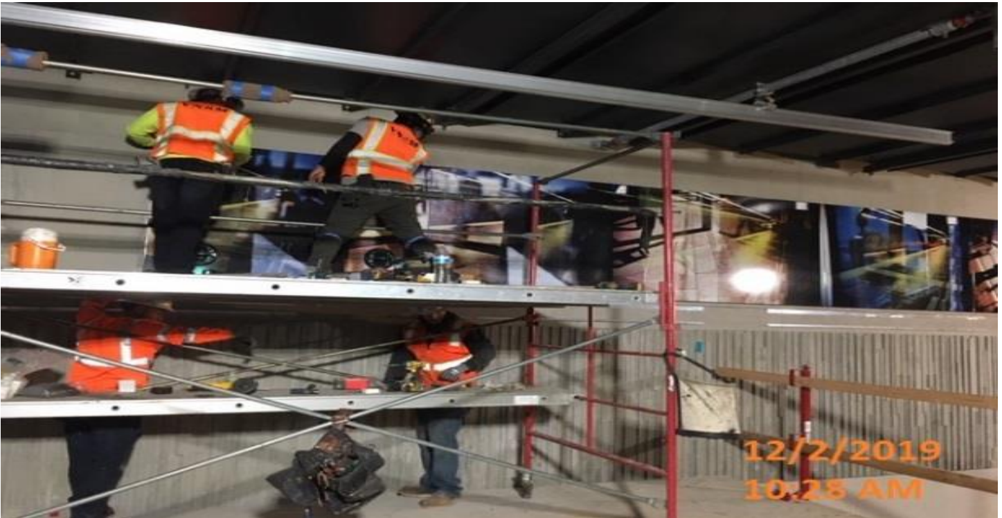
LEIMERT PARK STATION- Installation of porcelain enamel art panel on the southbound track of the platform level.
