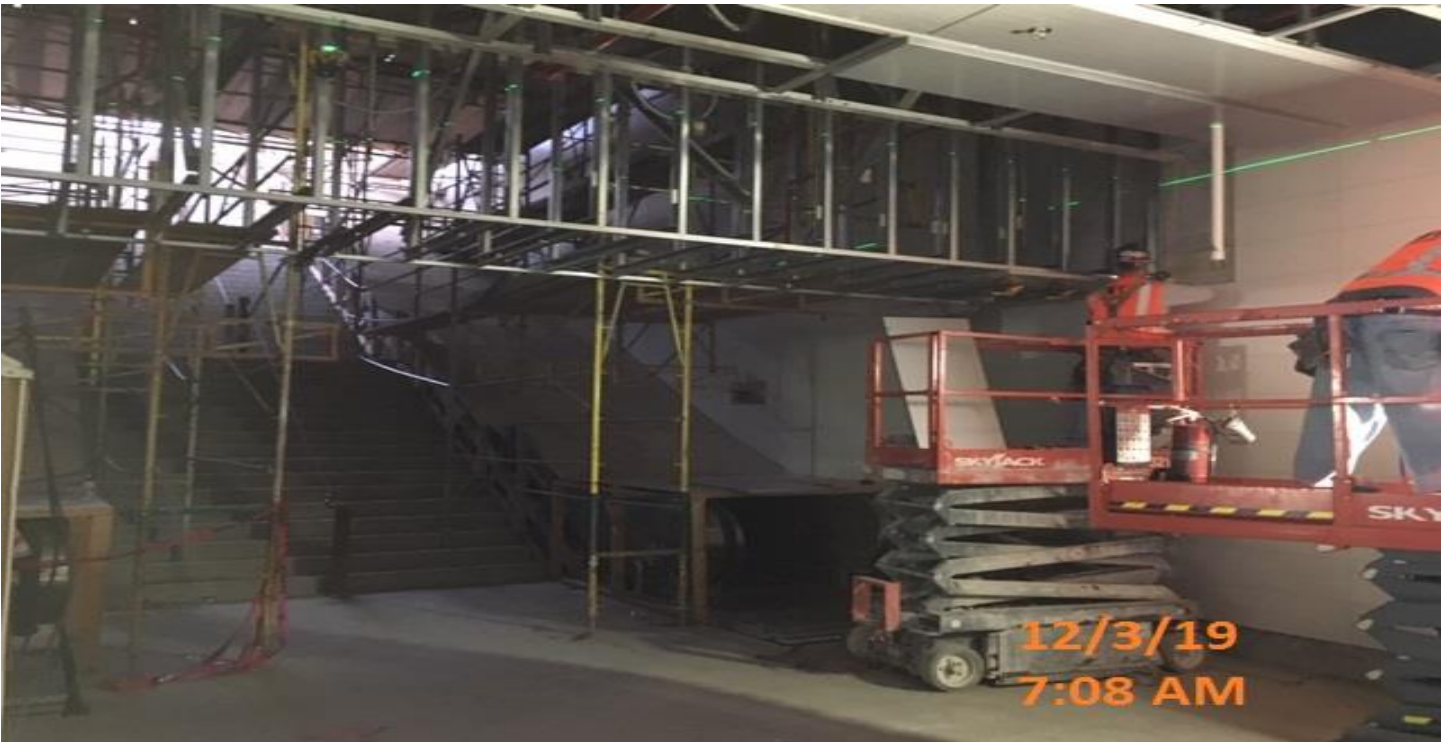
EXPOSITION/CRENSHAW STATION – Installation of bulkhead panels in the Pan Free Area of the concourse level.
