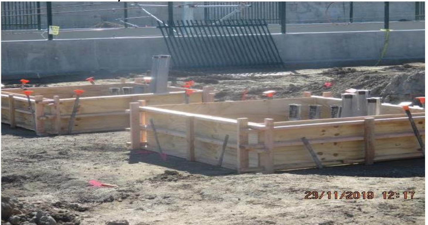
UG3- Building forms for DWP electrical slabs at Victoria Yard.
