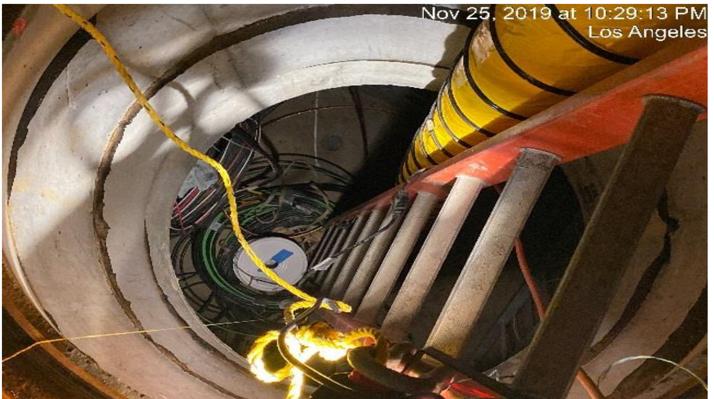
UG3- LKC ATC conducting continuity testing of wire for the ETS-38 in UG-3.
