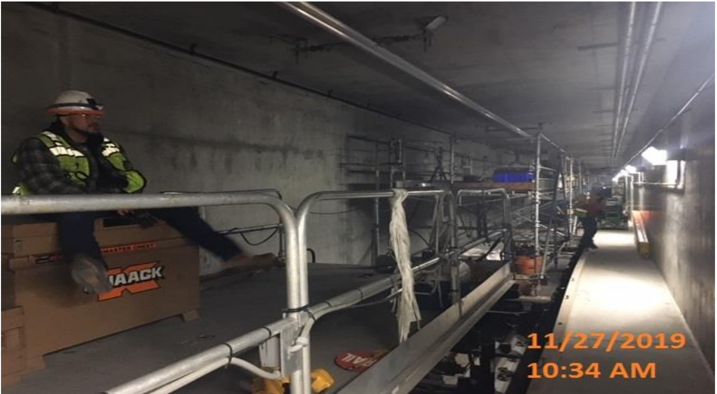
UG3- Continued installation of conductor rail for the overhead contact system on the southbound tunnel at Sta 378+00.
