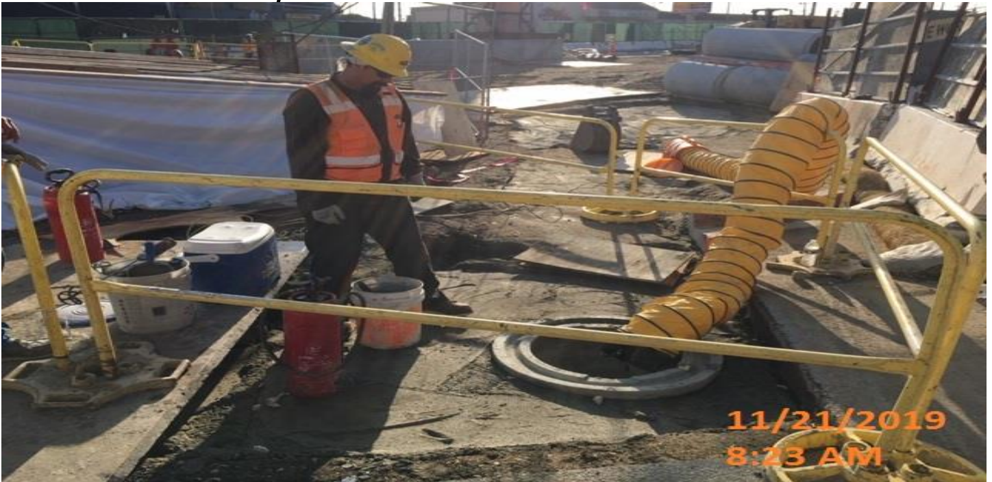
MARTIN LUTHER KING JR. STATION- Chipping inside Manhole #1 for A – Line storm drain at the topside.
