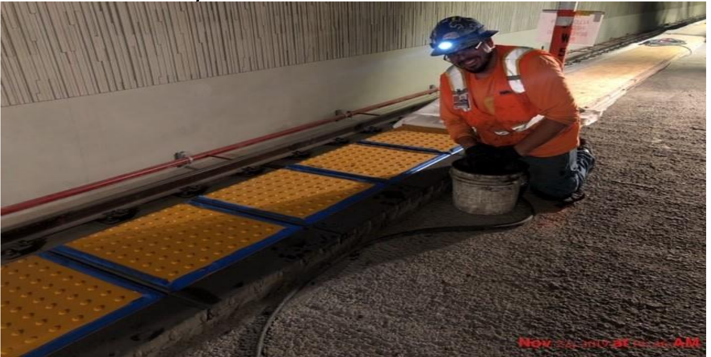
MARTIN LUTHER KING JR. STATION- Continued installation of ADA edge pavers on both sides of the platform level.
