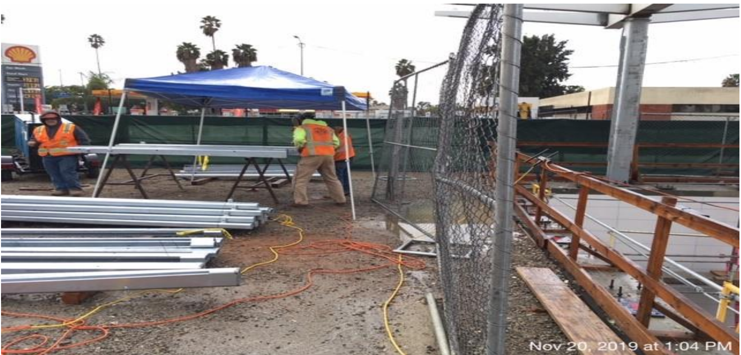
EXPOSITION/CRENSHAW STATION – Fabrication and installation of windscreen frames for the main entrance portal at the plaza level.
