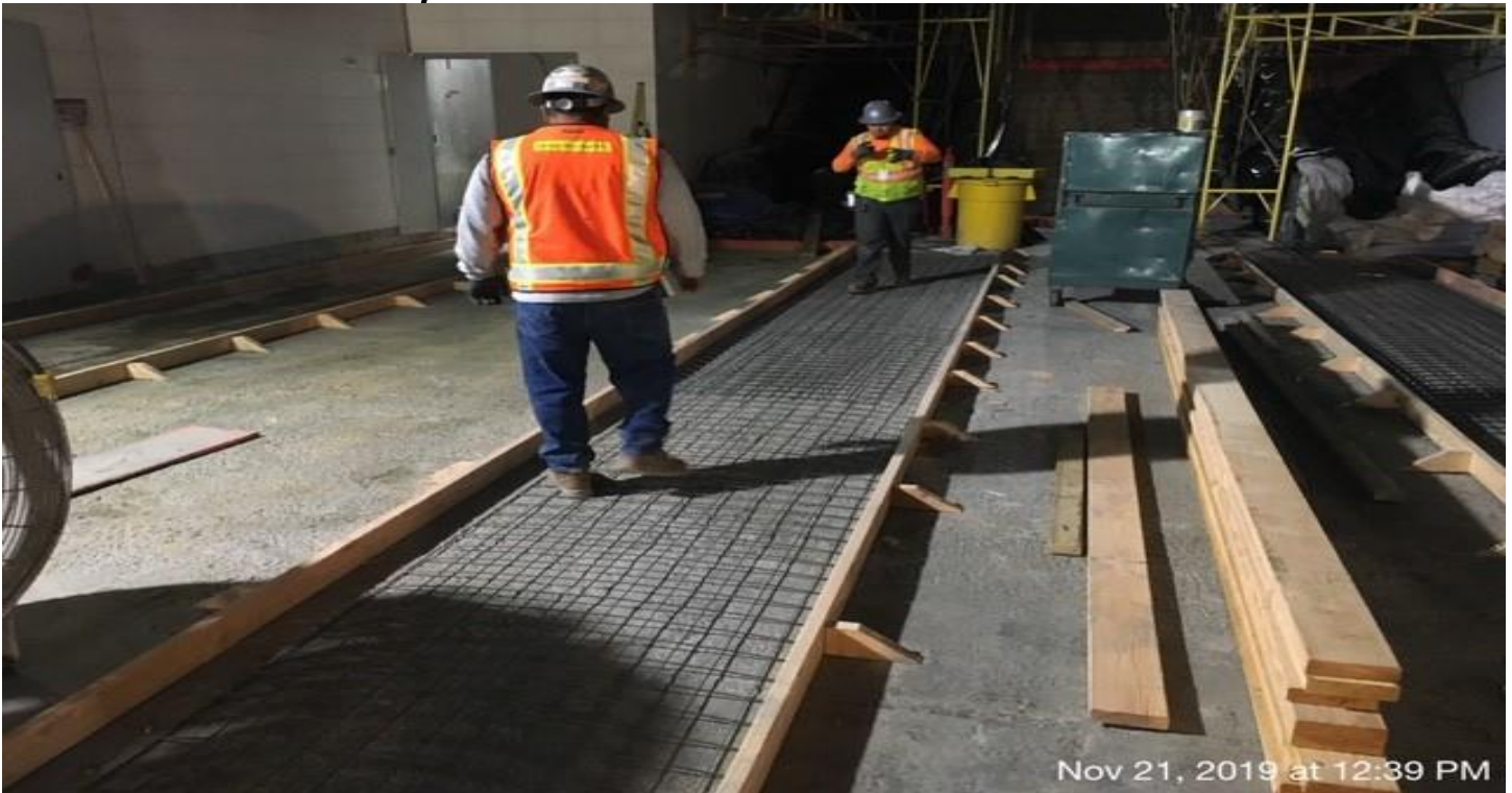
LEIMERT PARK STATION- Continued laying and forming second portion of architectural topping slab at the concourse level.
