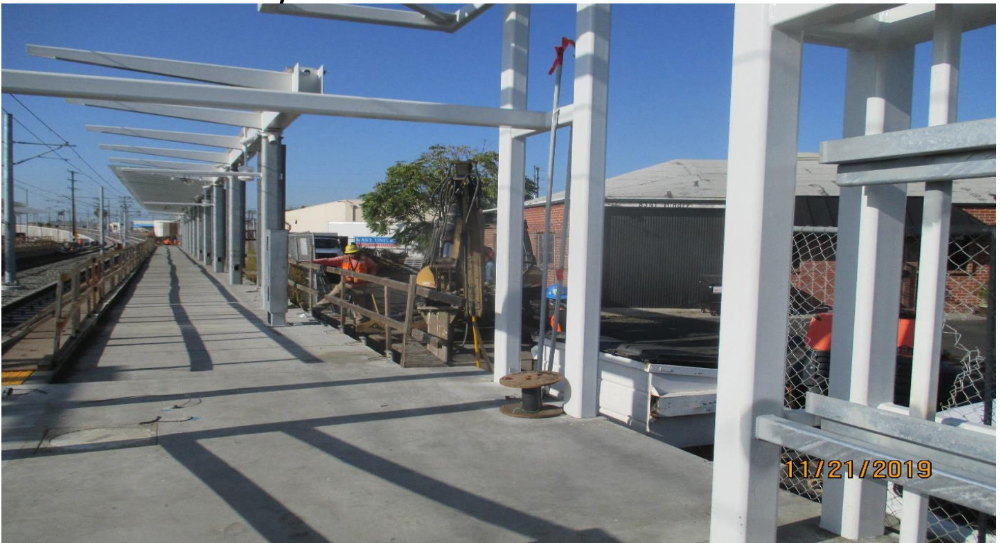
WESTCHESTER STATION – Demo of the parking lot to access the Westchester Station SB platform drain line.
