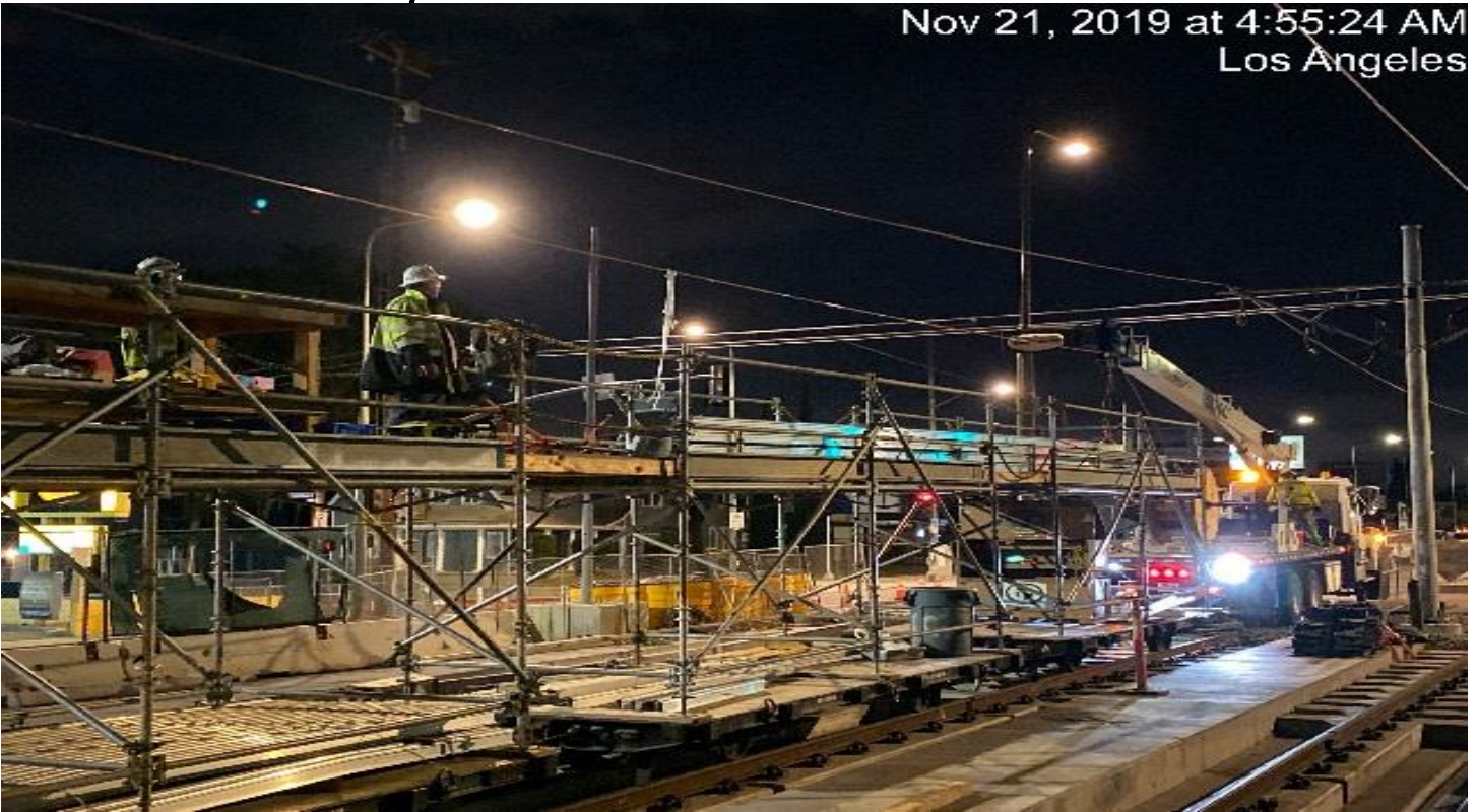
PARK MESA – Installation of overhead contact system wire from UG4 north portal to 48th St and Crenshaw Blvd.
