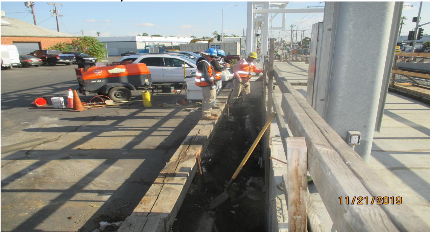
WESTCHESTER STATION – Demo to access the backside of the Westchester Station SB platform drain line..
