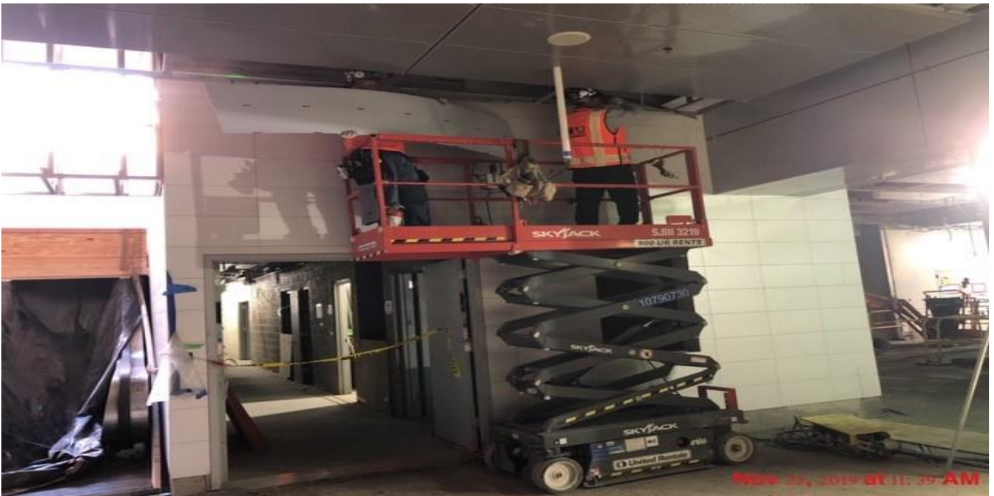
MARTIN LUTHER KING JR. STATION- Continued installation of device panels and ceiling at the concourse level.
