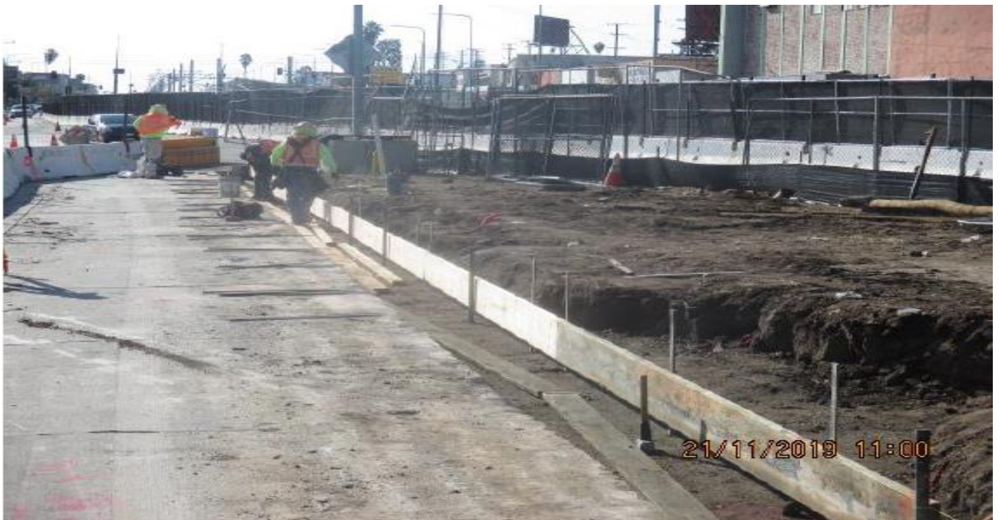
LEIMERT PARK STATION- Curb and gutter placement on northbound Leimert Blvd and Crenshaw Blvd.
