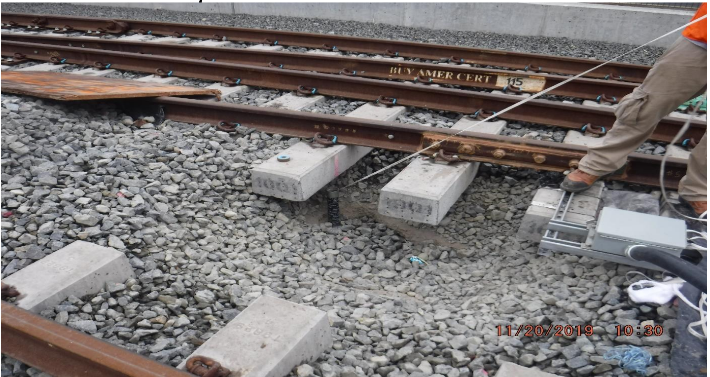
HIGH STREET - STA245+15_ Looking East_ Disturbed track ballast_ PUNCH LIST_S616.
