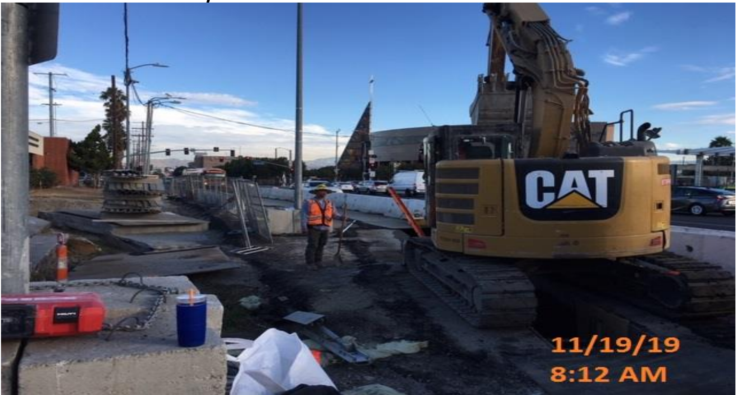
EXPOSITION/CRENSHAW STATION – Excavation for reinforced concrete pipe placement for W – Line storm drain on the northwest corner of Obama Blvd and Crenshaw Blvd.
