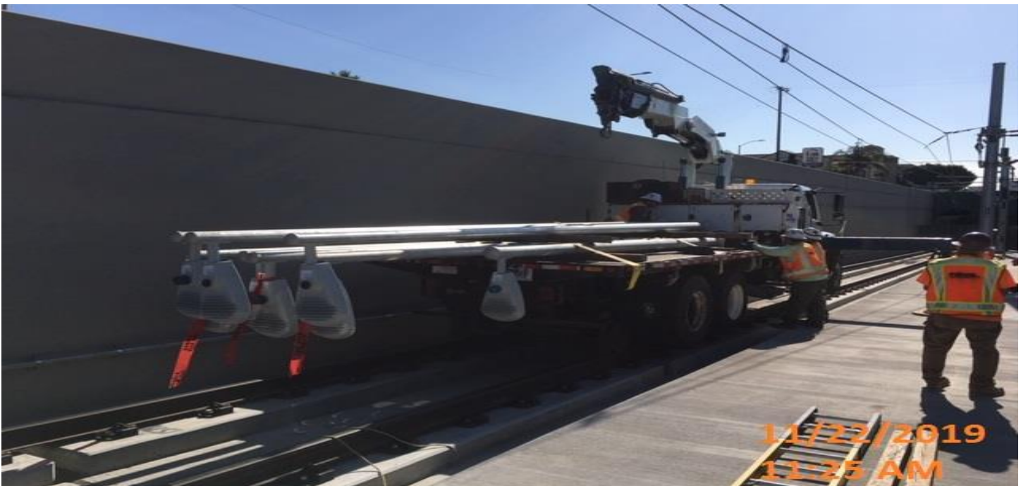
UG3- Installation of light posts on the center divider at the north end portal.
