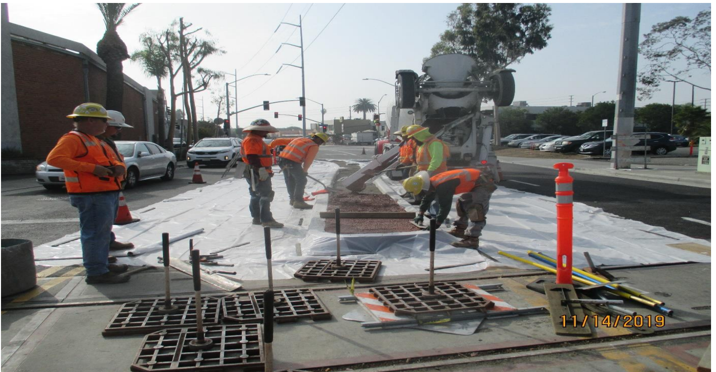
EUCALYPTUS STREET - Placing colored concrete for the median island at Eucalyptus.
