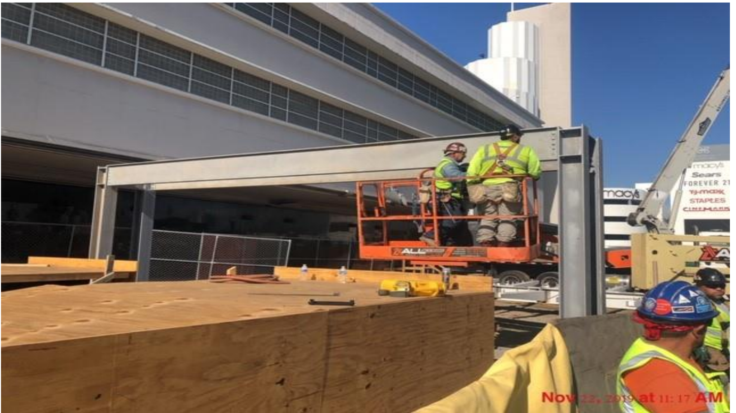
MARTIN LUTHER KING JR. STATION- Fitting up main entrance canopy portal frame at the plaza level.
