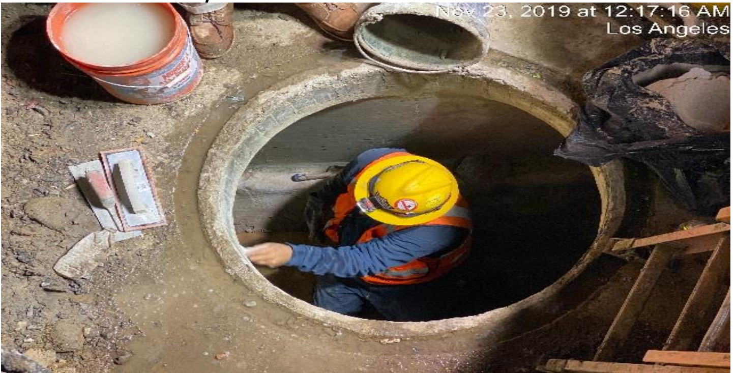
PARK MESA – Removing forms and sacking and patching new northern manhole for 1025 Line storm drain on the intersection of Slauson Ave & Crenshaw Blvd.
