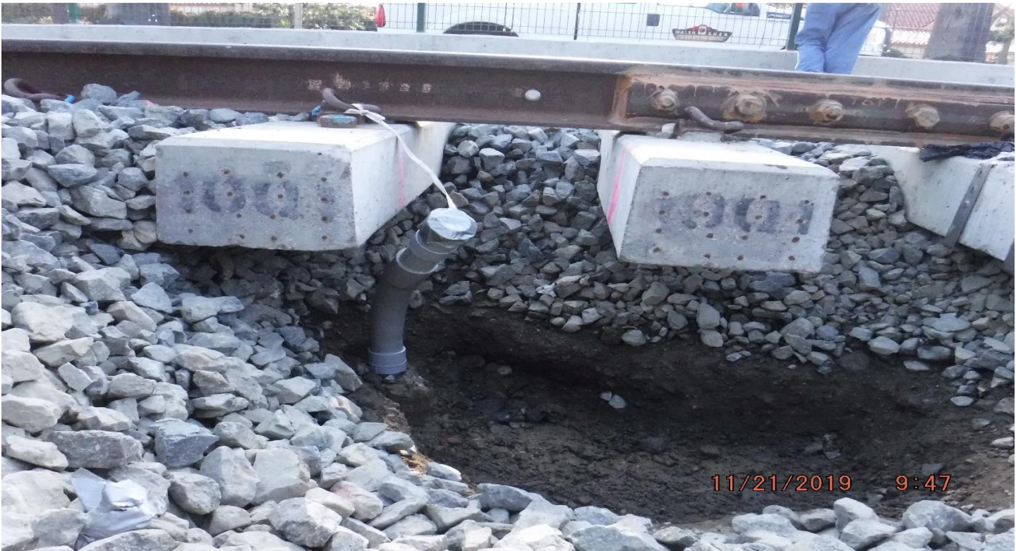
HIGH STREET - STA245+15_ Looking East_ Disturbed track ballast_ PUNCH LIST_S616.
