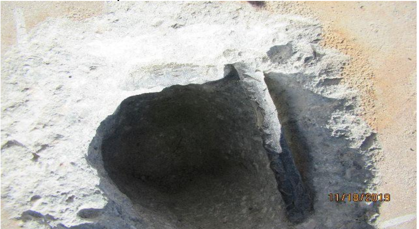
GUIDEWAY AT 405- Damaged strip rebar while coring insert on SB #3 track 405 fwy OP.
