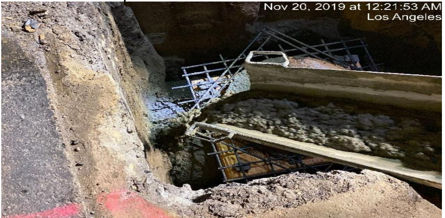
PARK MESA- Placing concrete on new manhole for 1025 – Line storm drain on the intersection of Slauson Ave & Crenshaw Blvd.
