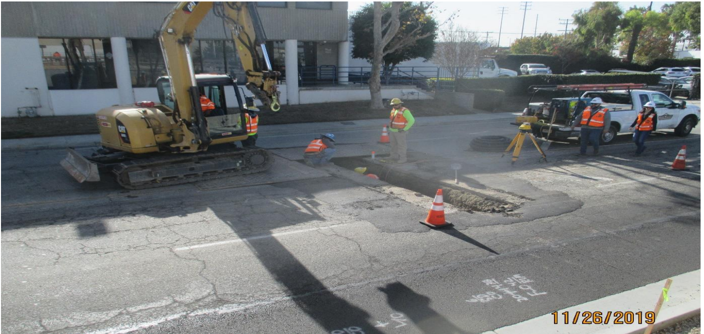
WESTCHESTER STATION – Excavating and placing a temporary 3 sump pump drain line at the Westchester Station on Florence.
