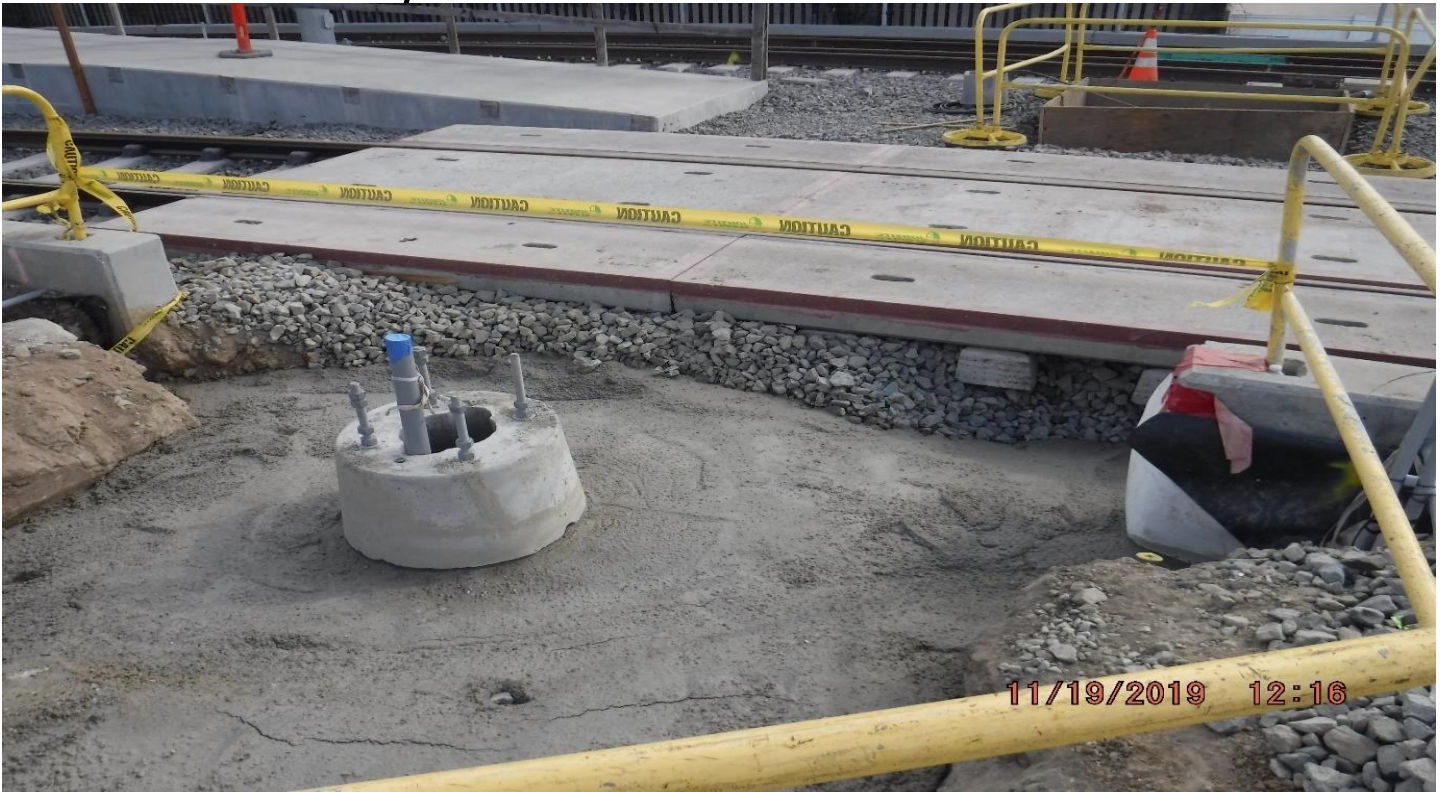
FLORENCE/WEST - STA262+74_ Looking East_ Disturbed track ballast_ Slurry pour.
