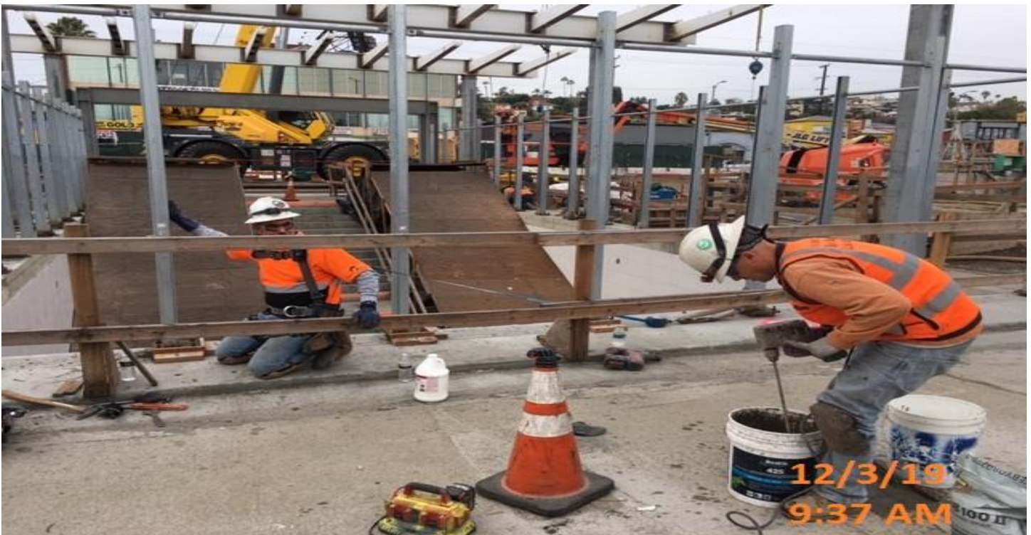
LEIMERT PARK STATION- Continued working on wind screen frames for the main entrance portal at the plaza level.
