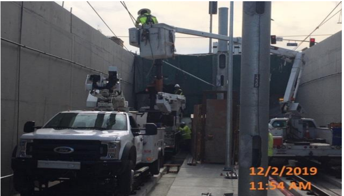
UG3- Continued installation of conductor rail for the overhead contact system on the northbound tunnel at Sta 311+20.
