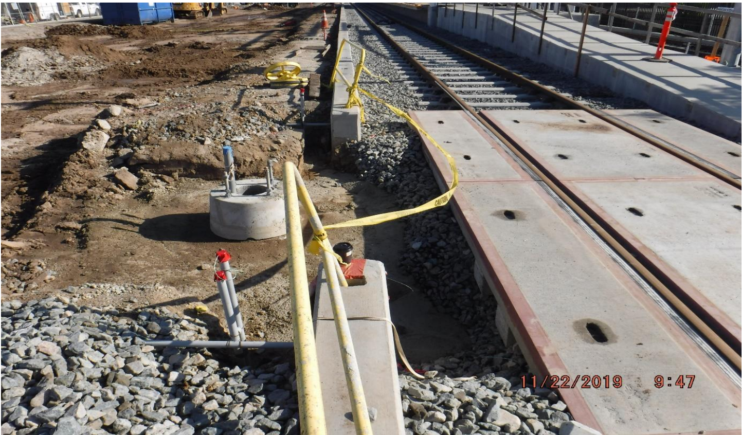
FLORENCE/WEST - STA262+74_ Looking North_ Disturbed track ballast.
