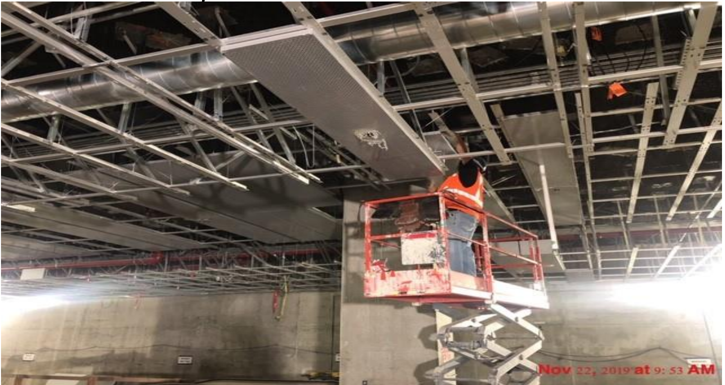
EXPOSITION/CRENSHAW STATION – Continued installation of device and field drop ceiling panels at the concourse level.
