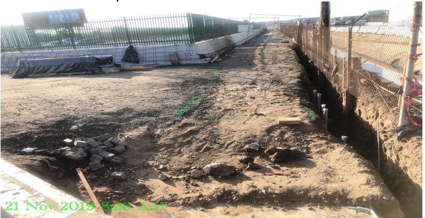
AVIATION STATION – Dyna Electric continue installation of DWP underground conduits at 104th street and Aviation Blvd.
