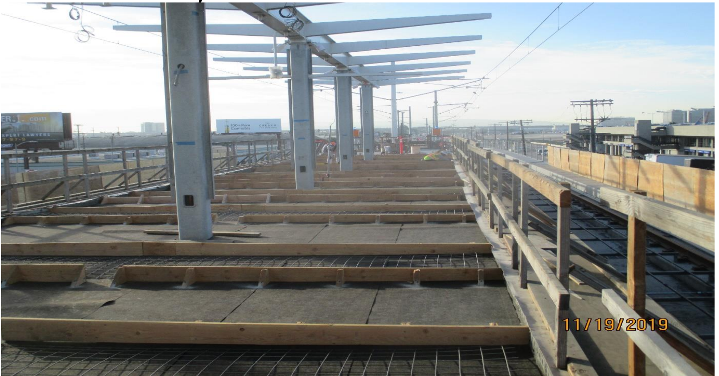
AVIATION STATION – Setting bond breaker paper, wire mesh and forms for the Aviation Station platform topping slab.
