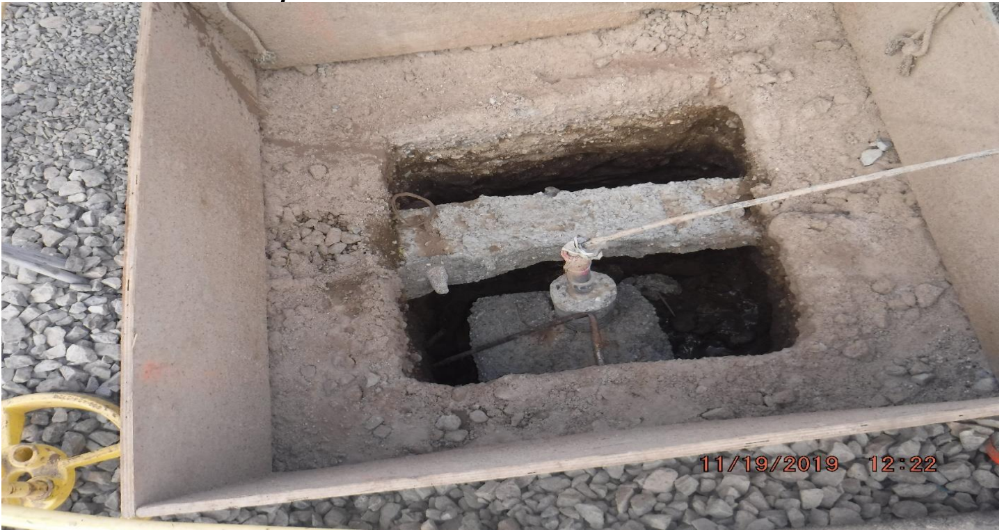
FLORENCE/WEST – STA262+74_ Looking Down_ Vacuum Excavation_ Disturbed track ballast.
