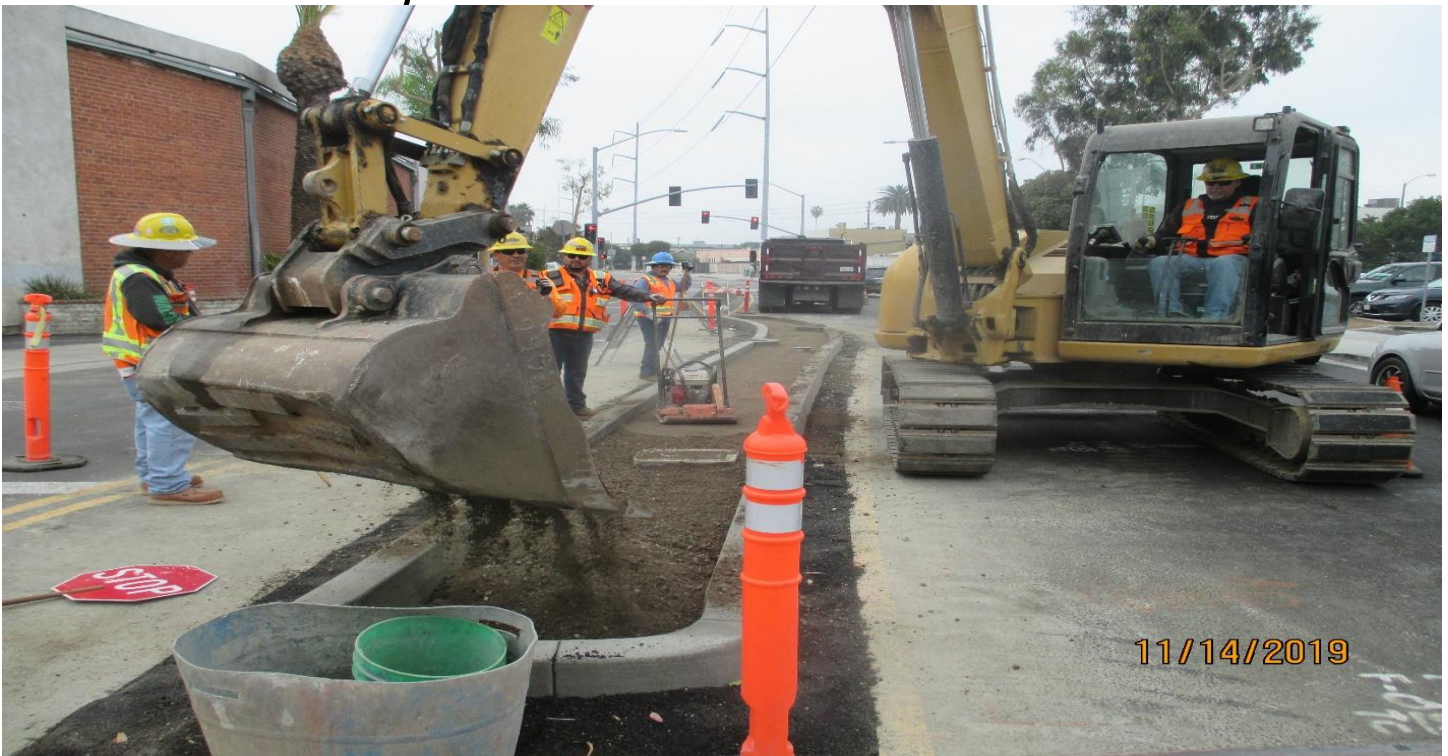
EUCALYPTUS STREET - Base placement and compaction for the median island on Eucalyptus.
