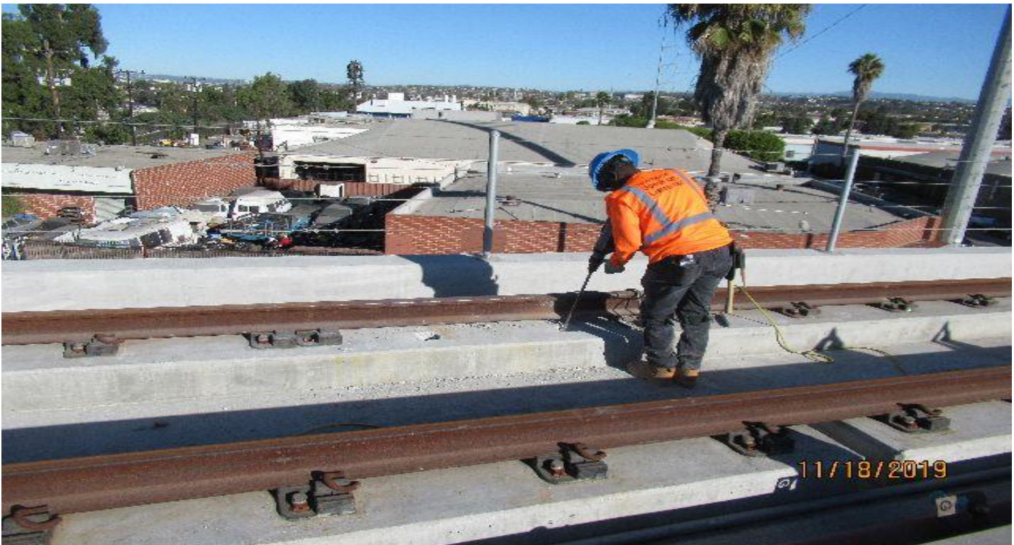
GUIDEWAY AT 405- WSCC chipping out concrete around insert hole on SB #3 track 405 fwy OP.
