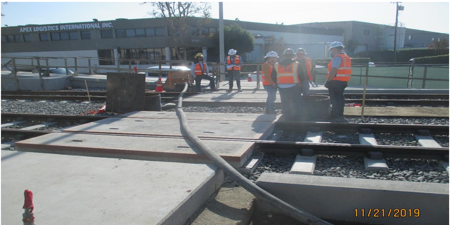
WESTCHESTER STATION – Slurry placement for light foundations #203, 205 & 206 at the Westchester Station.
