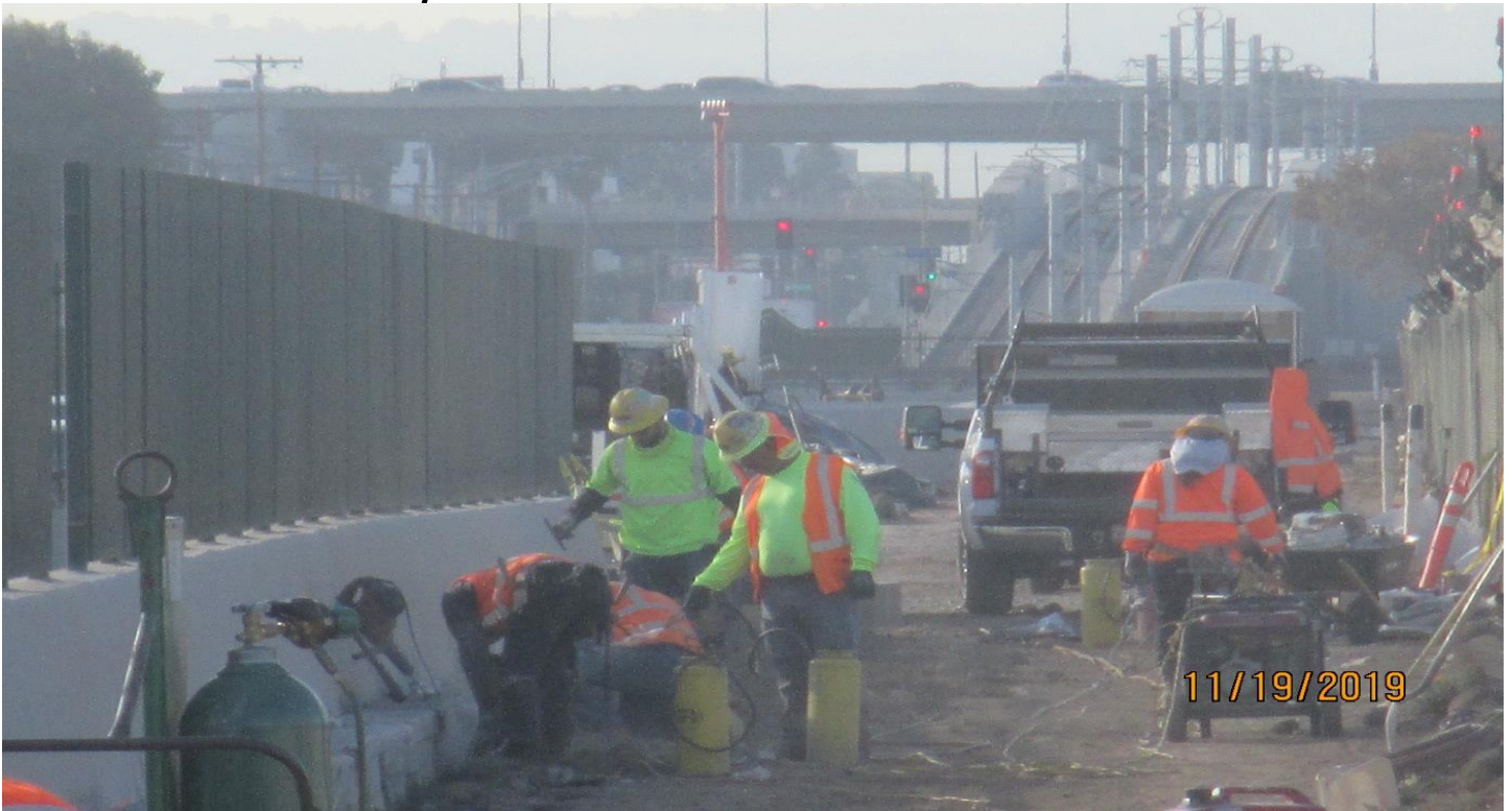
UG1- Concrete finish work after cutting out the imbedded flanges at UG-1.
