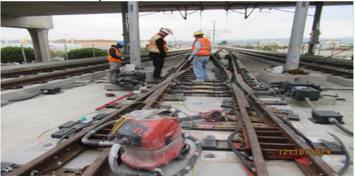
GREENLINE – Performing Cleanup of demoed DF inserts.
