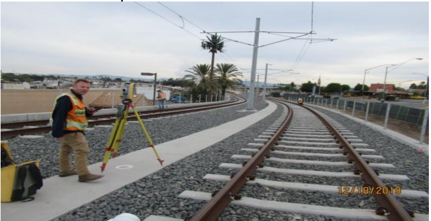
B1 GUIDEWAY - Surveying rail alignment and elevations on La Brea Bridge.
