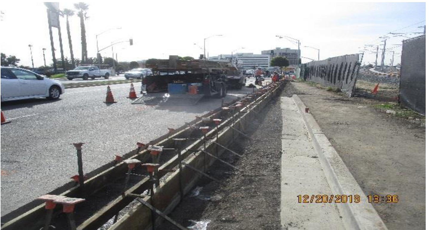
B1 GUIDEWAY - Form for curb & gutter on Florence at Market St.
