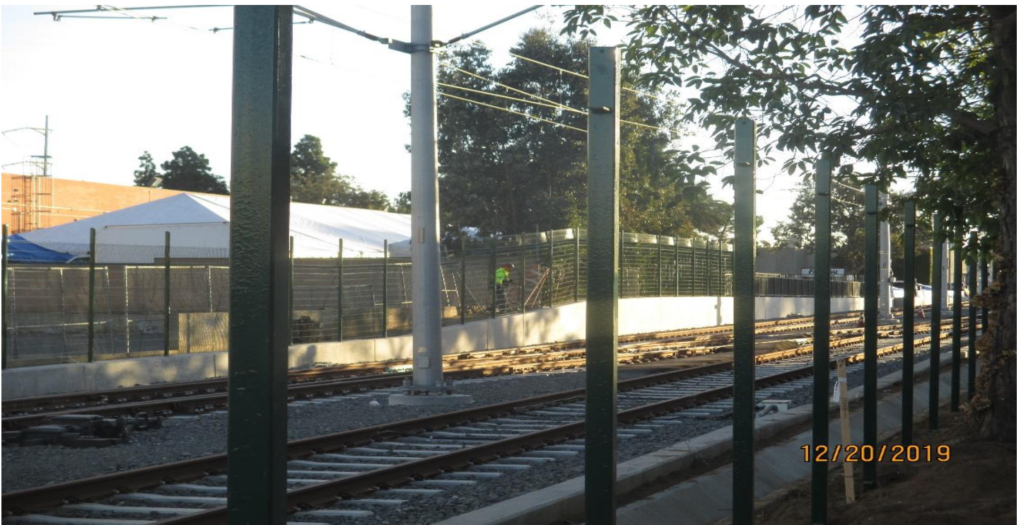
B1 GUIDEWAY – Setting wire mesh fence panels along SB B-1 Guideway.
