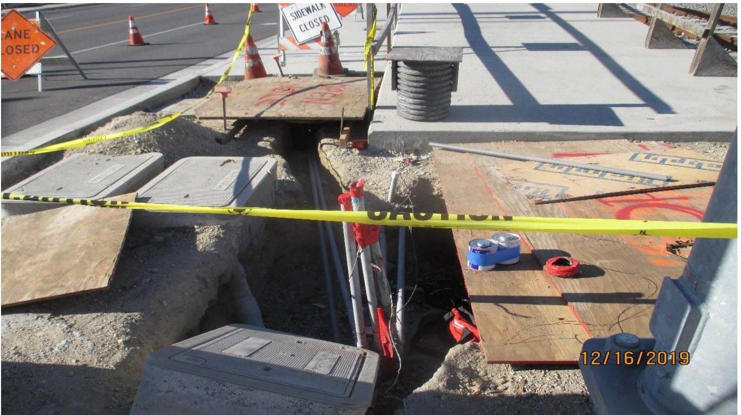
WESTCHESTER STATION – Setting conduit and foundation forms for light pole #214.
