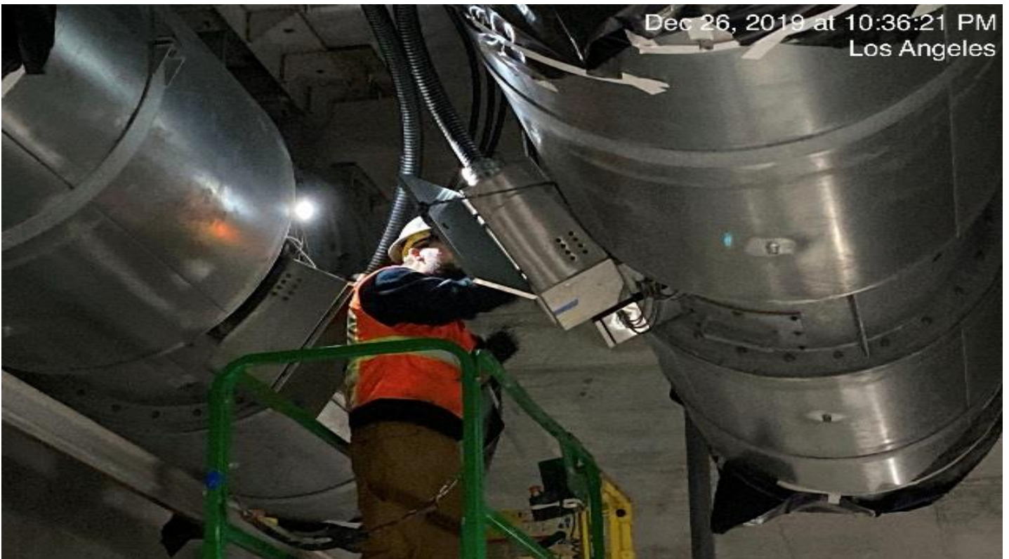
UG3- Continue wiring booster fans at the northbound tunnel at Sta 386+20.
