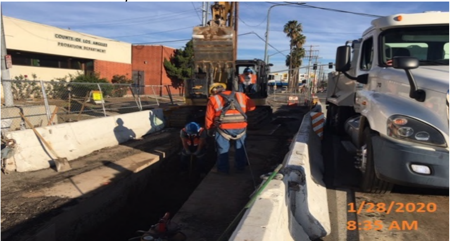
Expo Station - Excavating and shoring for Line W – storm drain near the northwest corner of Rodeo Blvd and Crenshaw Blvd.
