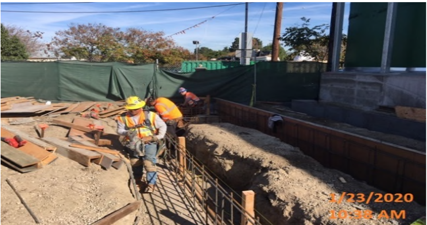
Leimert Park Station – Continued building sections of formwork for the north planter box footing at the plaza level.
