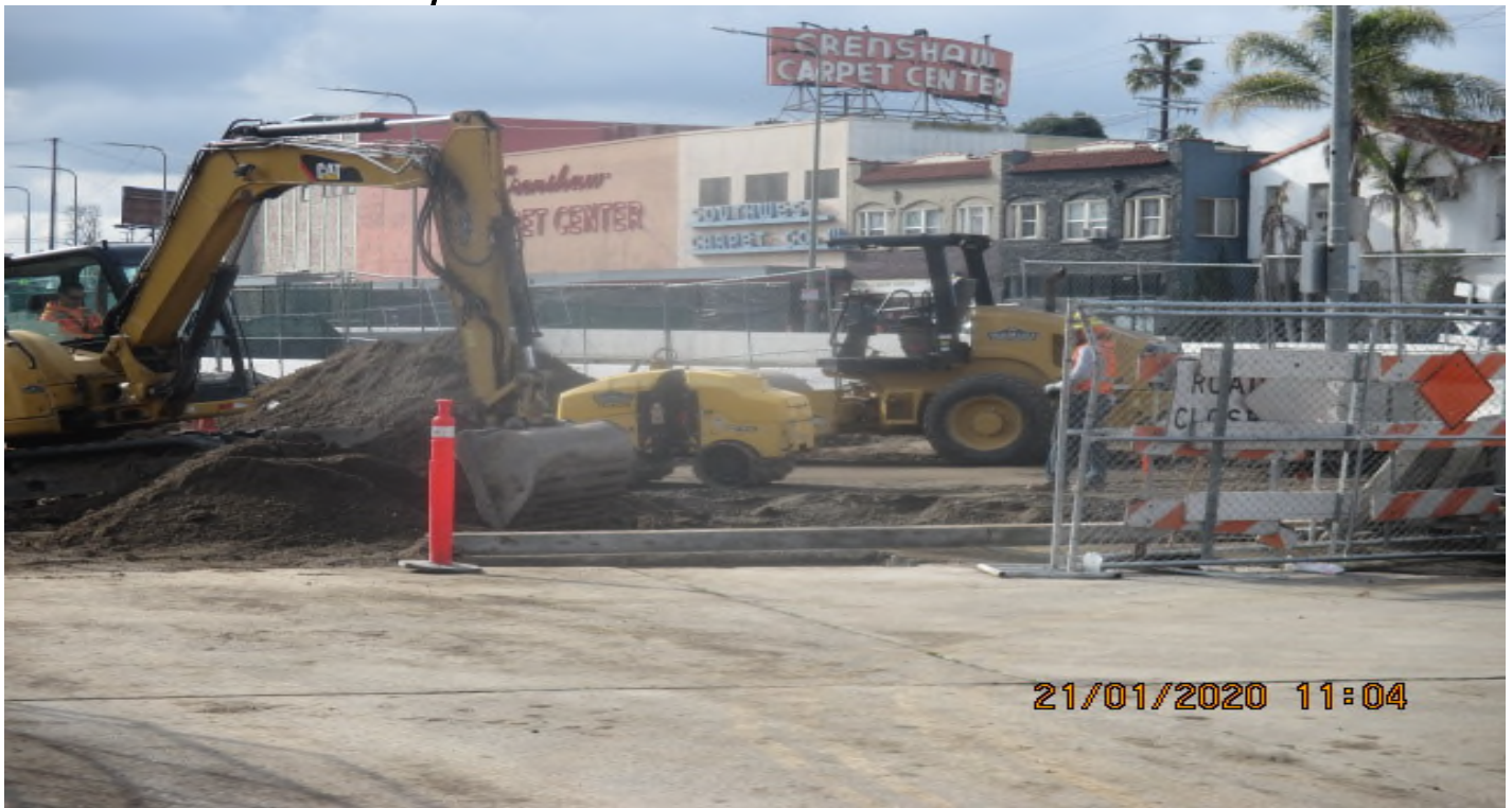
Leimert Park Station – Continued excavation/backfill and compacting median “Pork Chop” island between northbound Leimert Blvd and Crenshaw Blvd. 1/21/20
