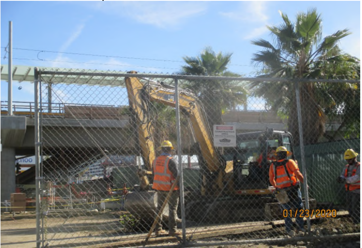
Aviation/Century – Demo and rough grading at the Aviation Station plaza area.
