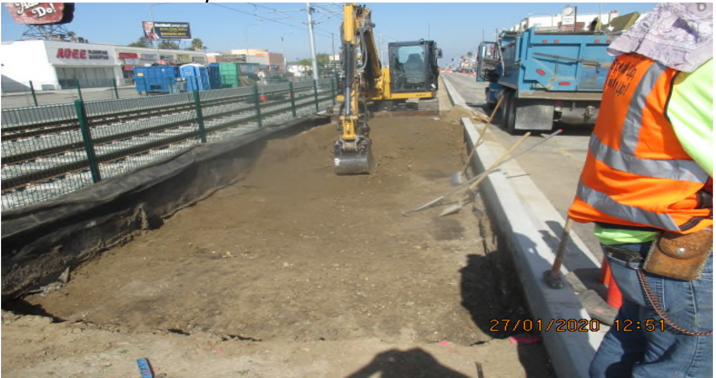
Park Mesa – Excavating northbound ballast wall for median embedded cobble installation on Crenshaw Blvd between 57th and 54th St. 1/27/20
