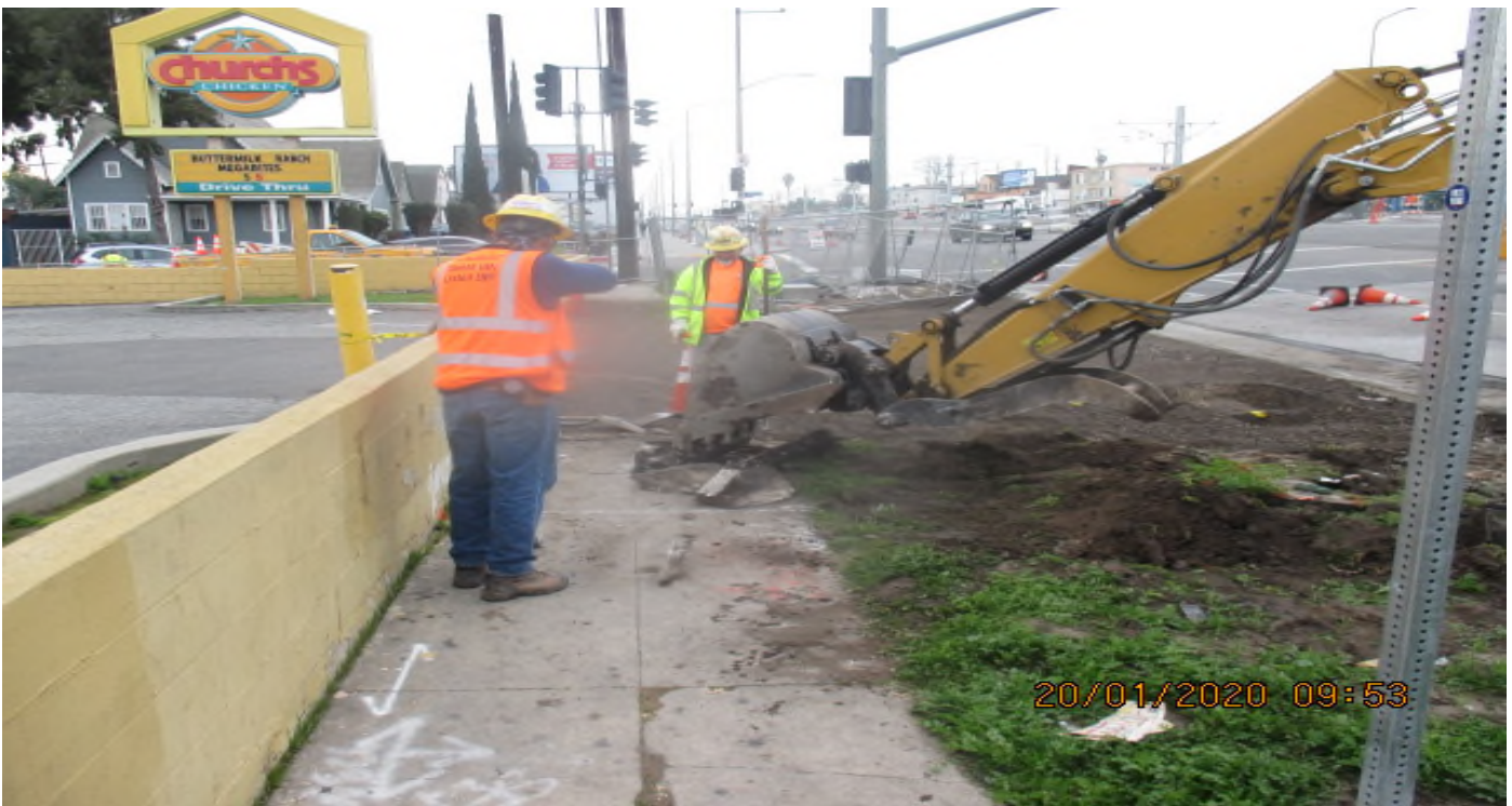
Park Mesa – Excavating northbound ballast wall for median embedded cobble installation on Crenshaw Blvd between 57th and 54th St. 1/27/20
