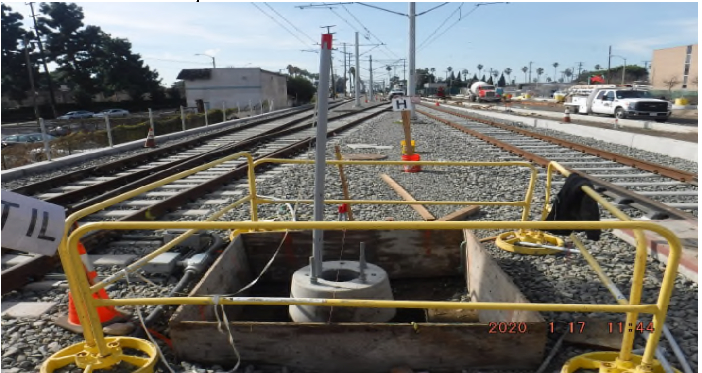
Florence/West – STA262+75_ Track structure disturbed to set Xing foundation between tracks_ West.
