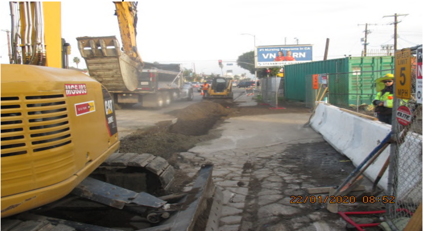
UG3 – Continued excavation and removal of existing northbound curb/gutter and abandoned rail lines near the southeast corner of 67th St and Crenshaw Blvd. 1/22/20
