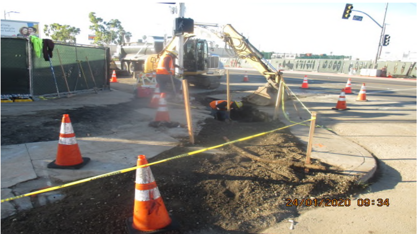
UG3 – Excavating for the installation of signal light conduits on the northeast corner of 67th St and Crenshaw Blvd. 1/23/20
