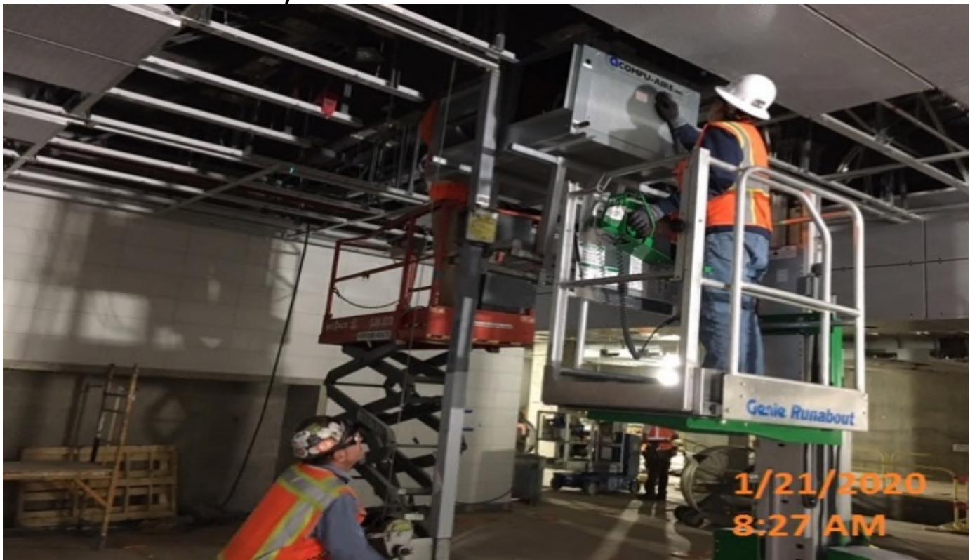
Expo Station - Hosting AC units into the ceiling of the Free Area C – 133 at the concourse level.
