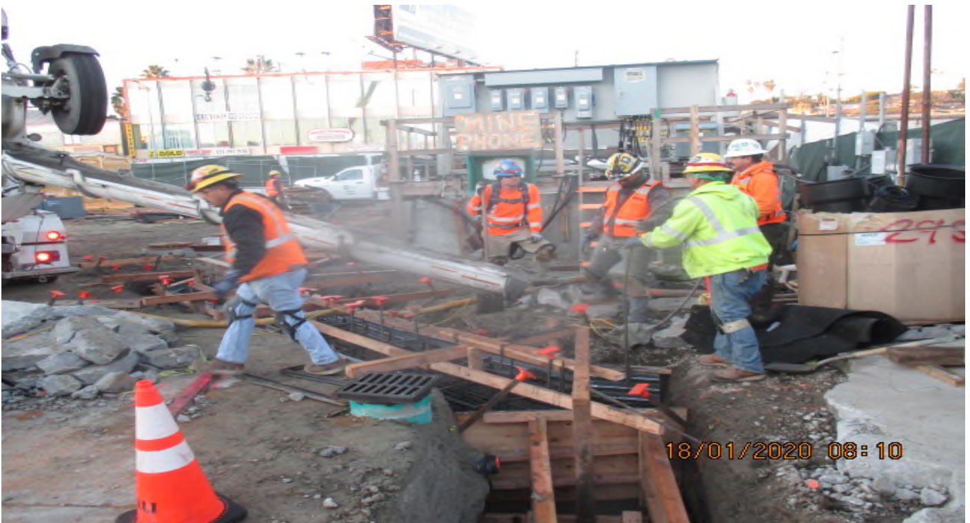
Leimert Park Station – Placing concrete on the east section of the south planter box footing at the plaza level. 1/18/20
