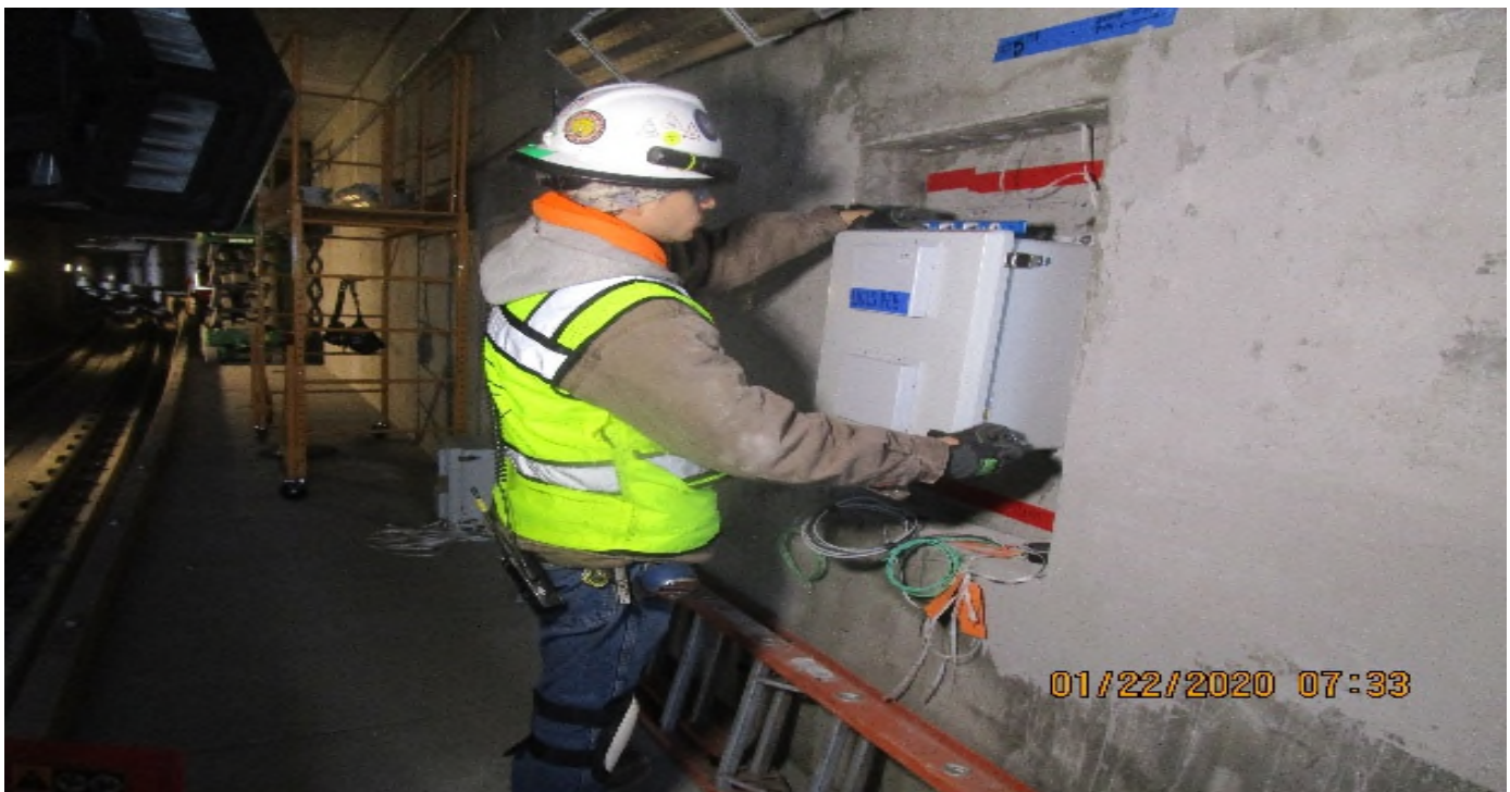
UG-4- Began wiring and running cable for the booster fans at the southbound tunnel at Sta 377+85.
