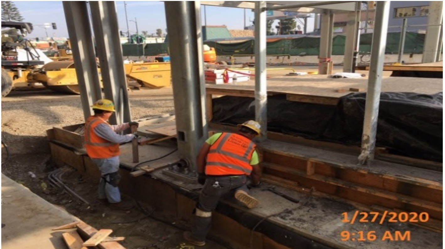
MLK Station - Concrete placement of the wind screen curbs on the main entrance canopy at the plaza level.
