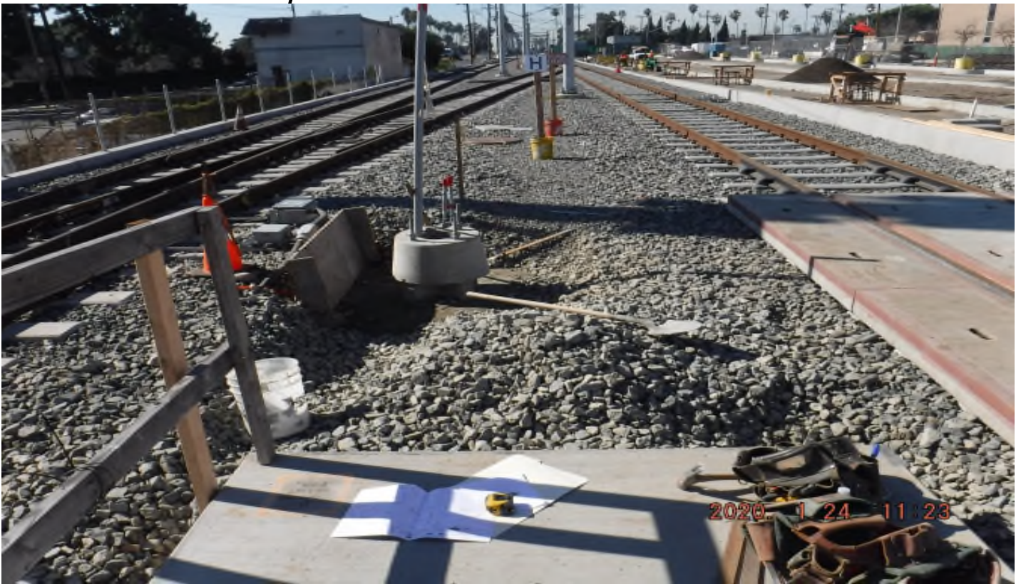
Florence/West – STA262+74_ Looking South_ Track ballast removal 4 pedestrian landing pad_ West.
