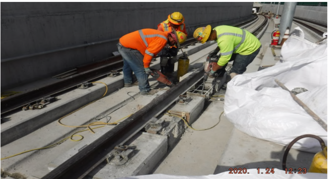
48 th Street - STA364+46_ Looking South_ Track structure disturbance in search of BLS conduits_ 48ST.
