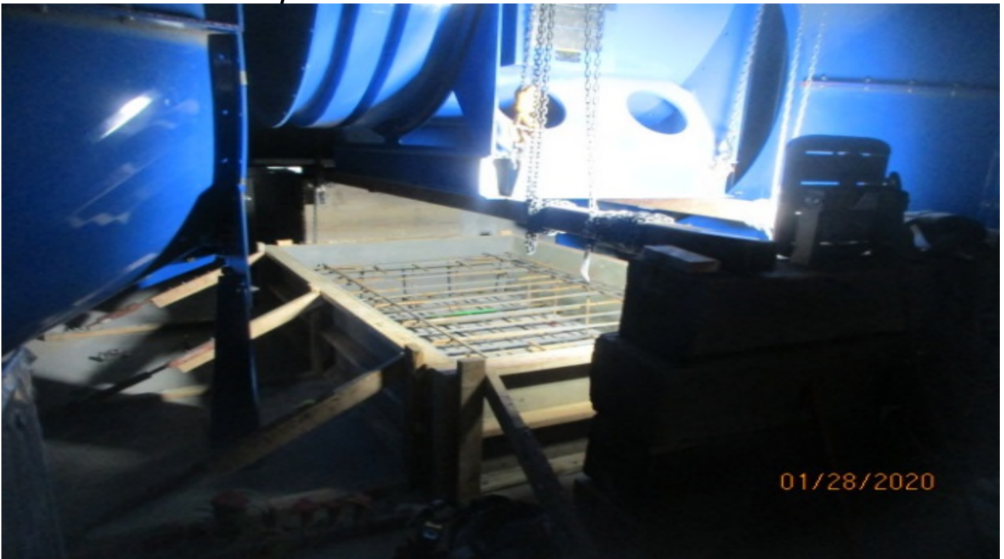
MLK Station - Began formwork and installing rebar to EVF-7-122 and EVF-322 equipment pads in the North Fan Room C – 142 of the concourse level.
