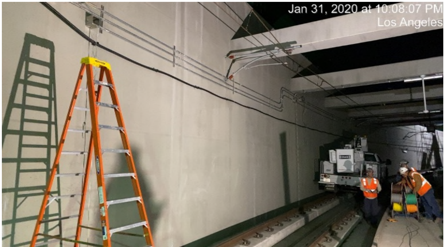
UG3 – Continue pulling wire for the emergency lighting at the south end portal entrance.
