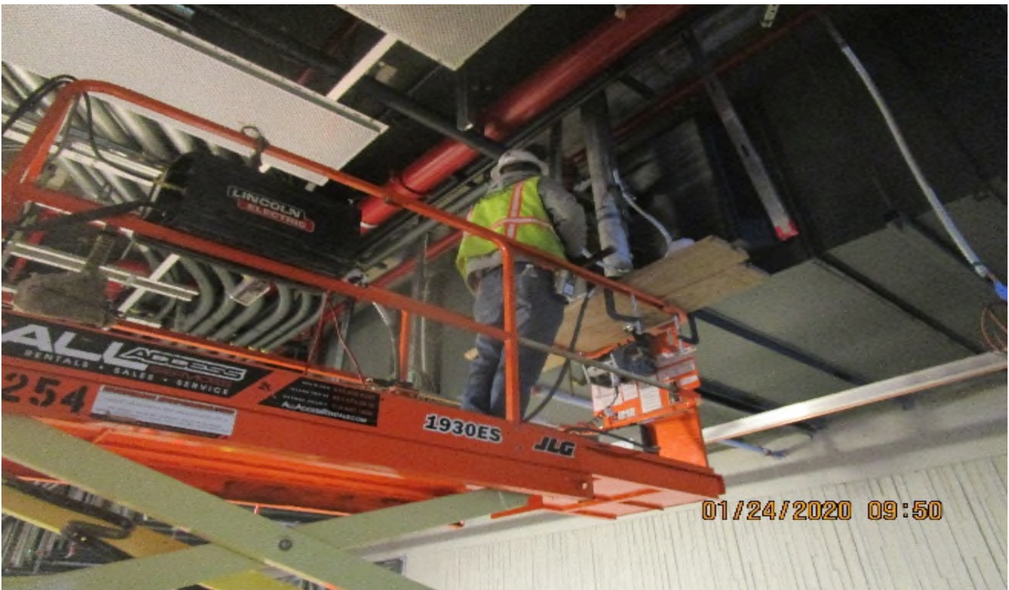
MLK Station - Continued rigging and installing 15" PVC into HDPE sleeve and hydraulic jack for Elevator hoist way/pit #3&4 at the platform level.
