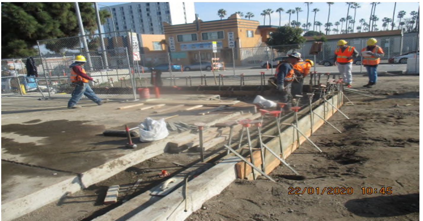
Leimert Park Station – Continued excavation/backfill and compacting median “Pork Chop” island between northbound Leimert Blvd and Crenshaw Blvd. 1/21/20
