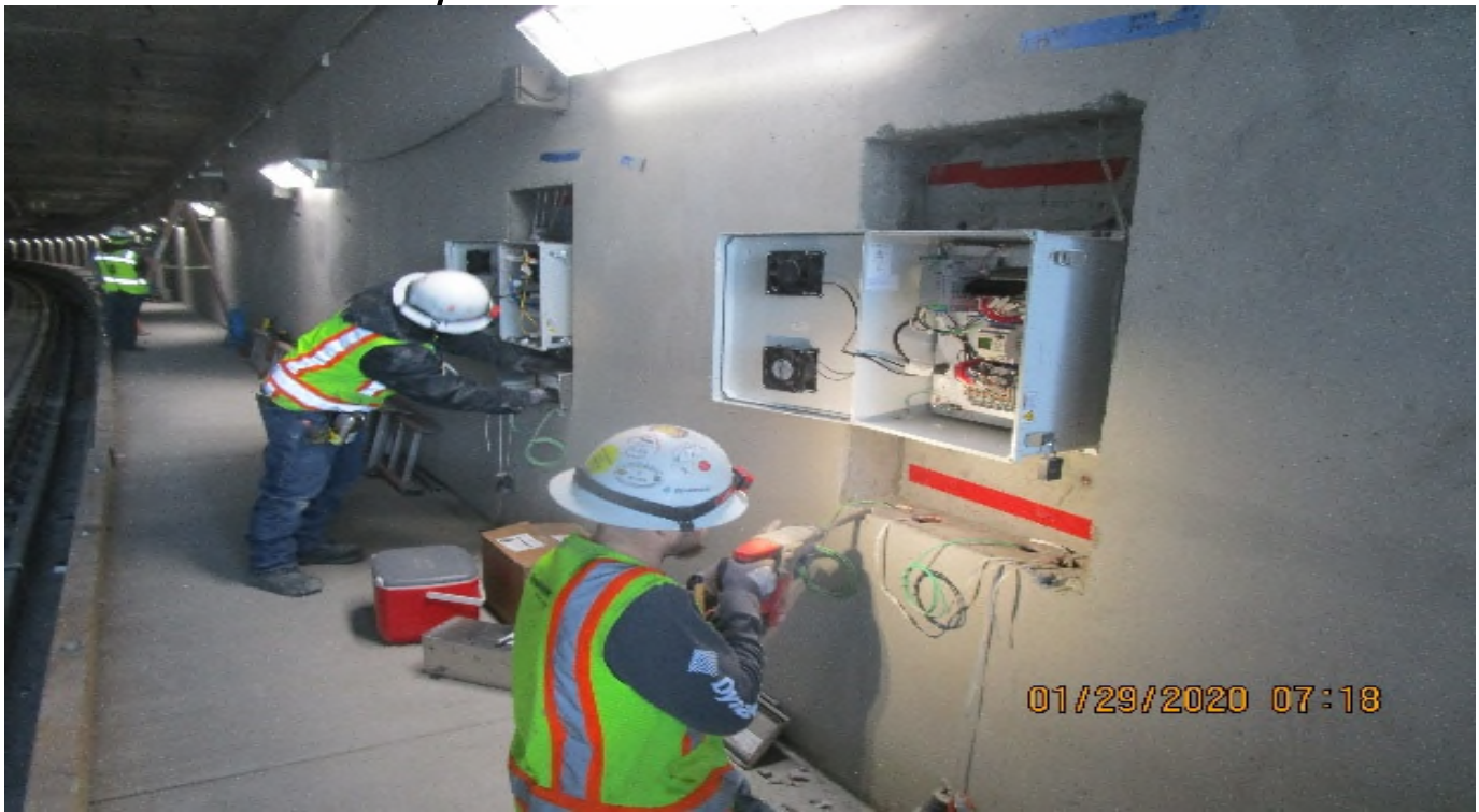
UG-4- Continue pulling ground wires and power to the IDS control cabinets in the southbound tunnel at Sta 371+25.
