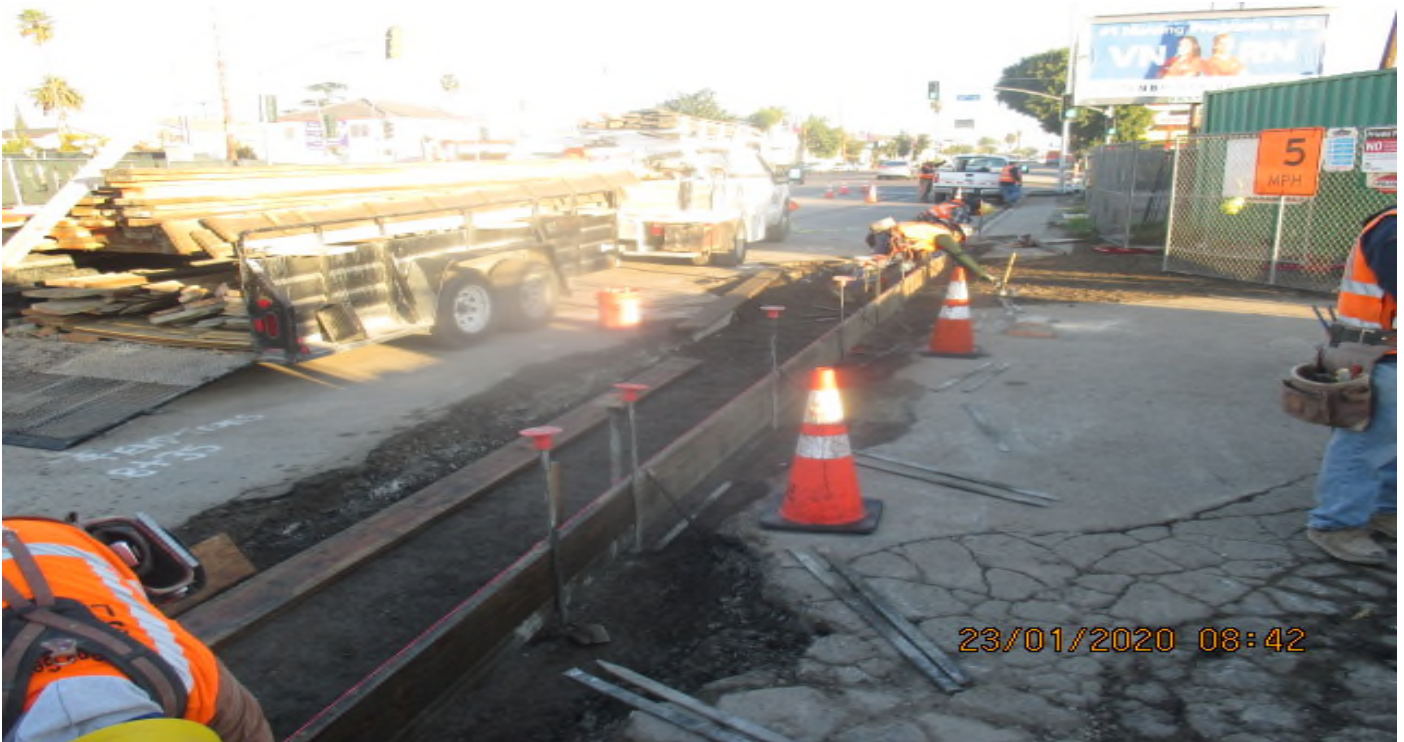
UG3 – Continued excavation and removal of existing northbound curb/gutter and abandoned rail lines near the southeast corner of 67th St and Crenshaw Blvd. 1/22/20
