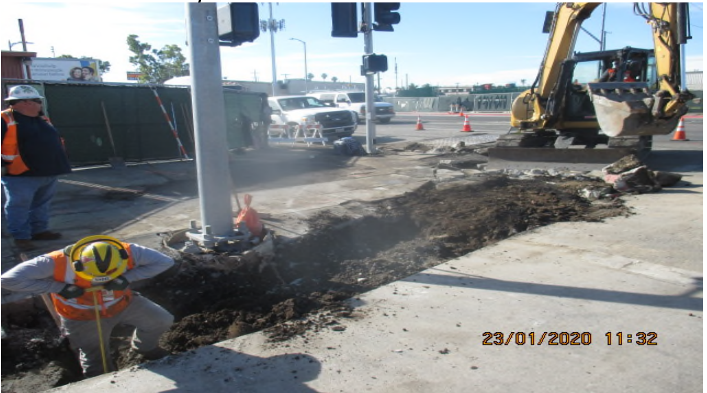
UG3 – Excavating for the installation of signal light conduits on the northeast corner of 67th St and Crenshaw Blvd. 1/23/20
