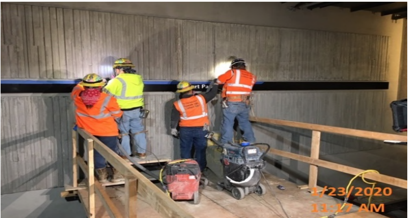
Leimert Park Station – Continue installing angle ceiling panels above the southbound track of the platform level.
