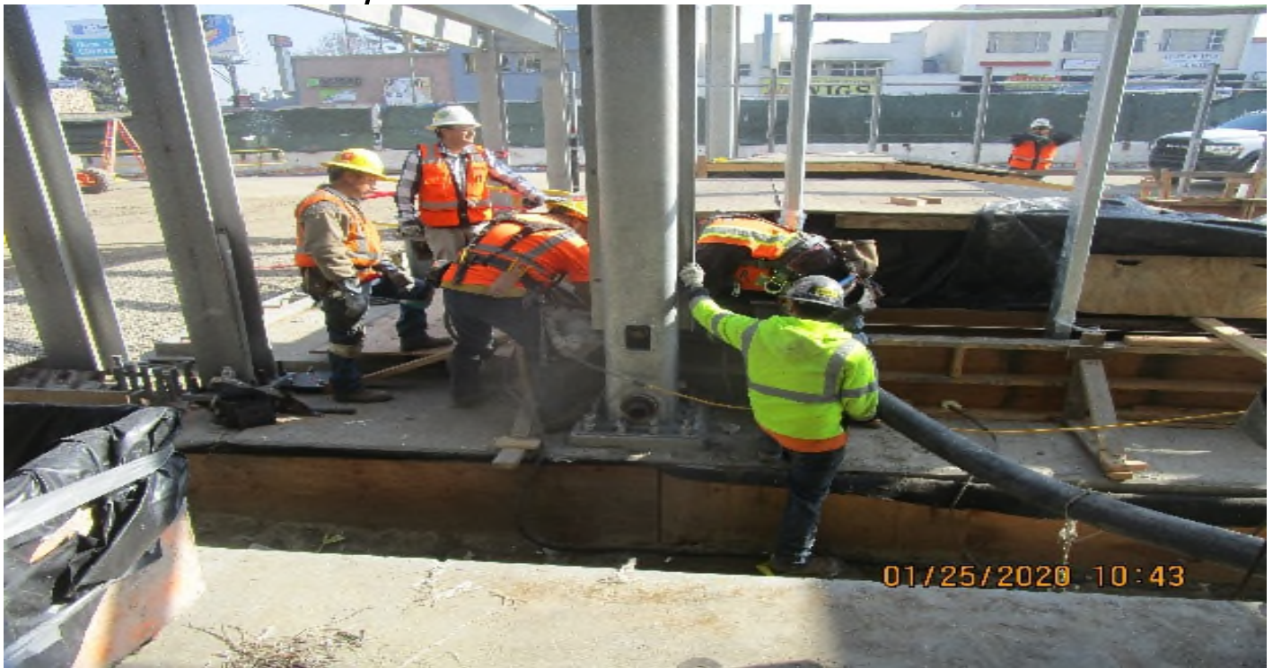
MLK Station - Concrete placement of the wind screen curbs on the main entrance canopy at the plaza level.
