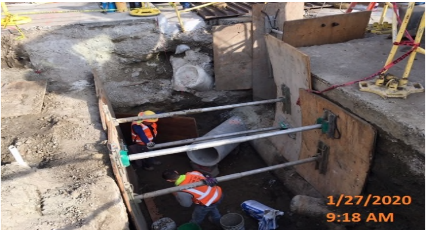
MLK Station - Capping and removing abandoned 10" oil pipe located on the southwest corner of Martin Luther King Blvd and Crenshaw Blvd.
