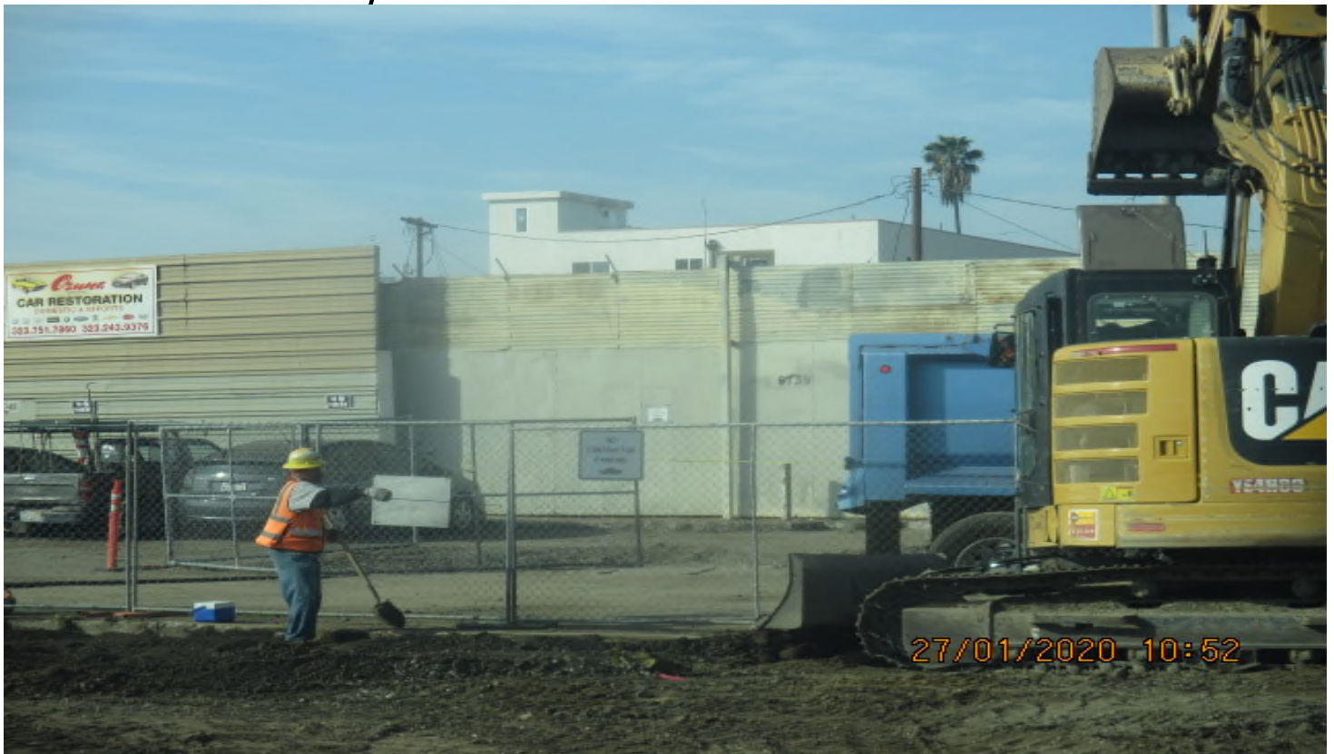
UG3 – Continued excavation and compaction for new curb/gutter at North Victoria Ave. 1/27/20
