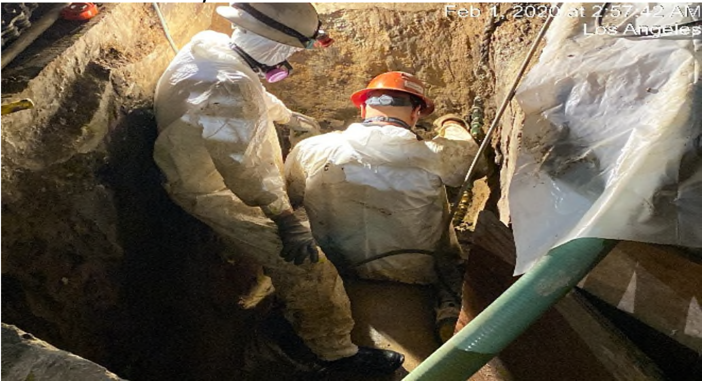
Park Mesa – Resumed LADWP main line tie-in on the intersection of 60th St & Crenshaw Blvd.
