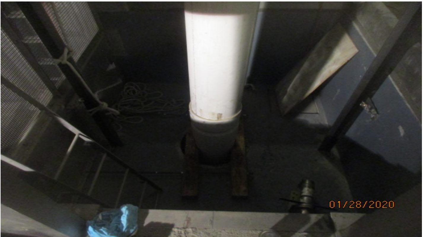
MLK Station - Prepping to install 15" PVC into HDPE sleeve within Elevator hoist way/pit #3&4 at the platform level.
