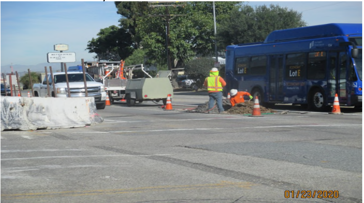
Aviation/Century – Potholing to locate utilities on Aviation at 111th.
