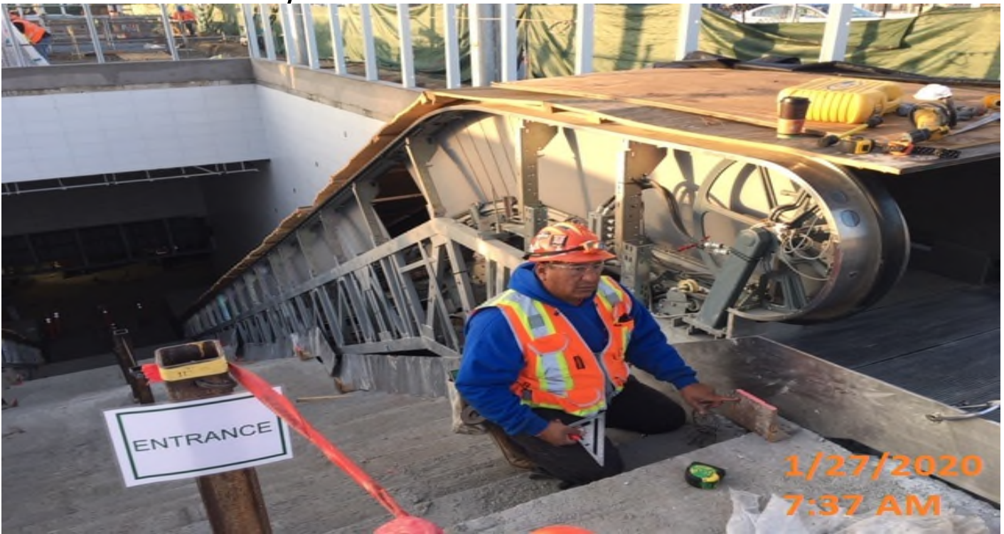
Expo Station - Setting and installing edge plates for Escalator 1&2 at the main staircase landing of the plaza level.
