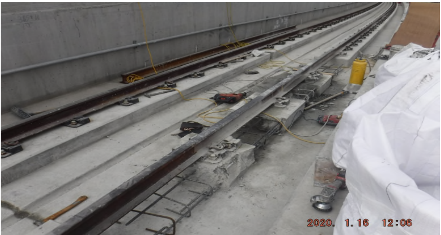
48 th Street - STA363+30_ Looking North_ Cleaning flangeway_48ST.
