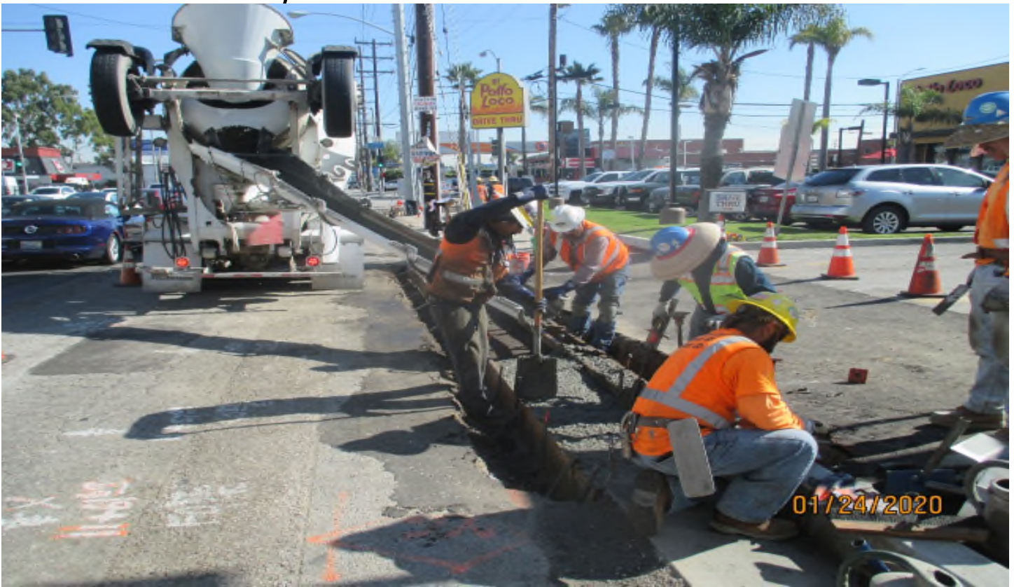
Manchester Bridge: – Placing gutter concrete at Manchester.
