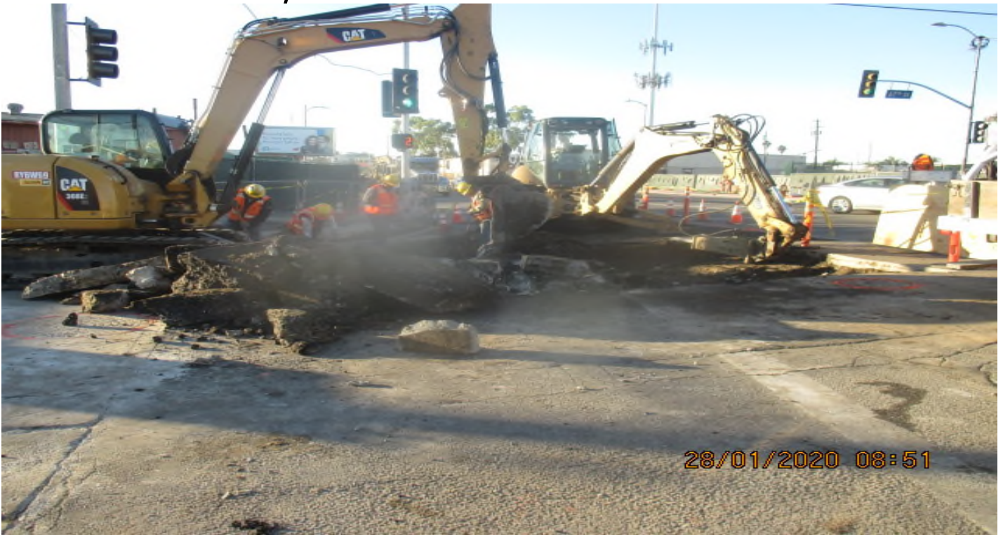
UG3 – Continued excavating and removing existing rail lines and roadway along the northbound lane of 67th St and Crenshaw Blvd. 1/28/20
