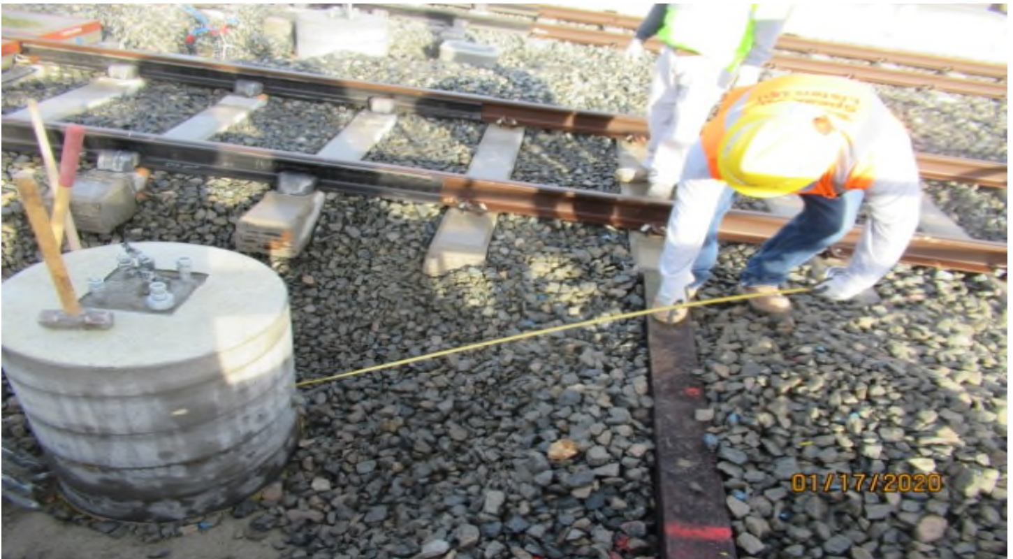
Florence/Hindry: – WSCC labor measuring crossing warning device foundation for pull box on SB track Hindry Ped.
