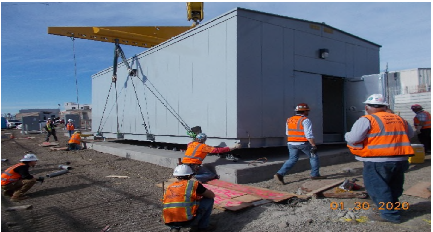
UG3 – Delivering the sub-station bungalow for the auxiliary power site at Victoria Yard adjacent to the south end portal.
