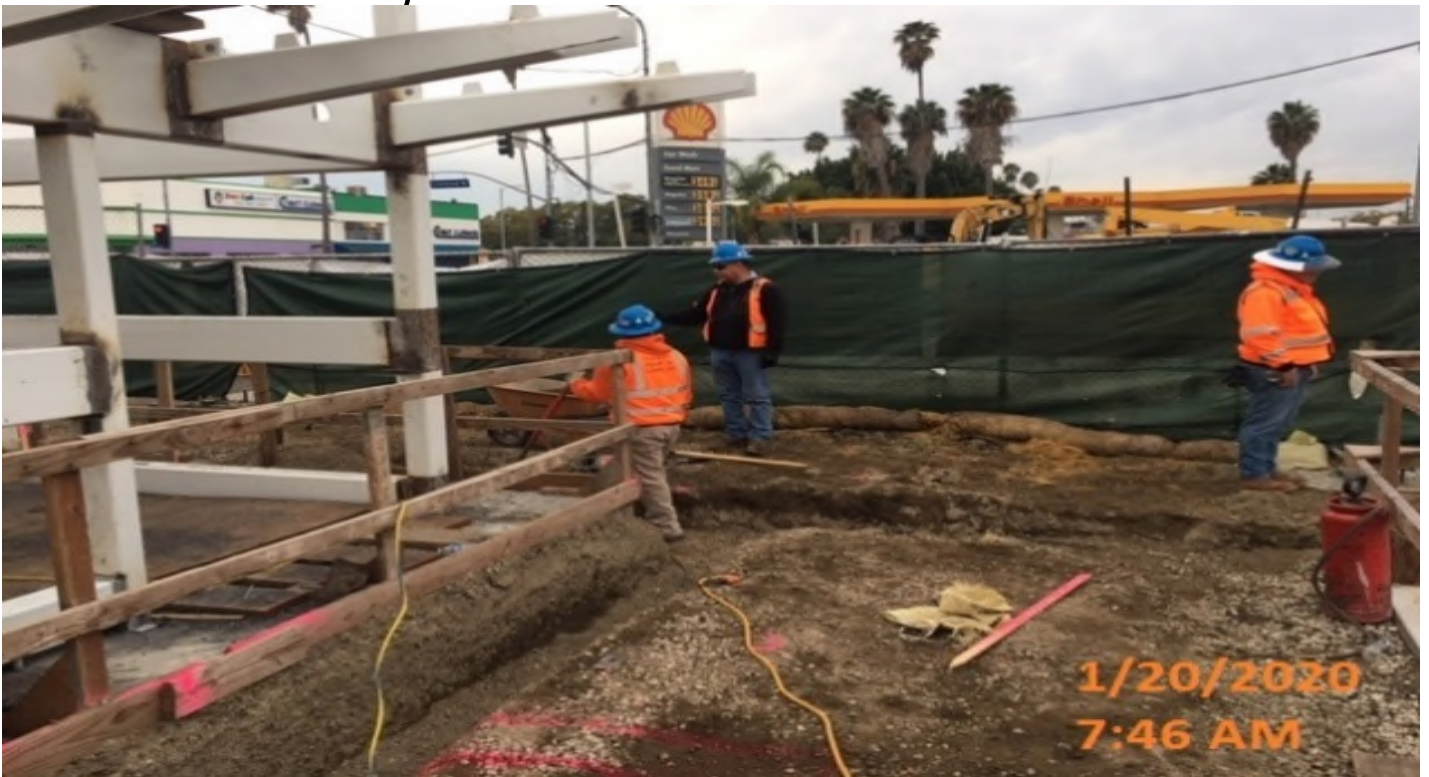
Expo Station - Continue excavating for drainage adjacent to structural Elevators 1&2 at the plaza level.
