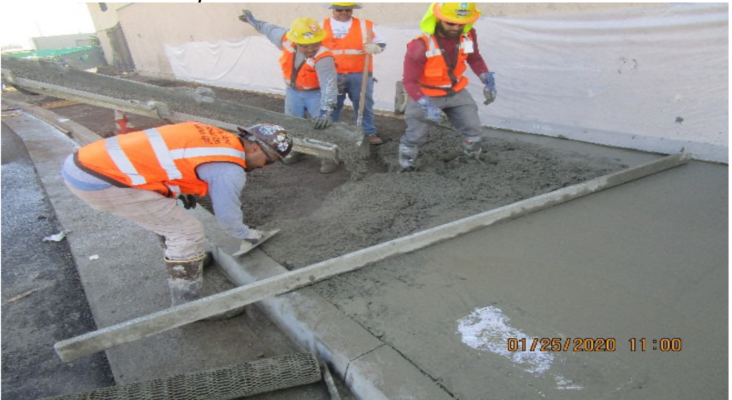
UG3 – Concrete placement of the eastbound sidewalk of “New Road.”
