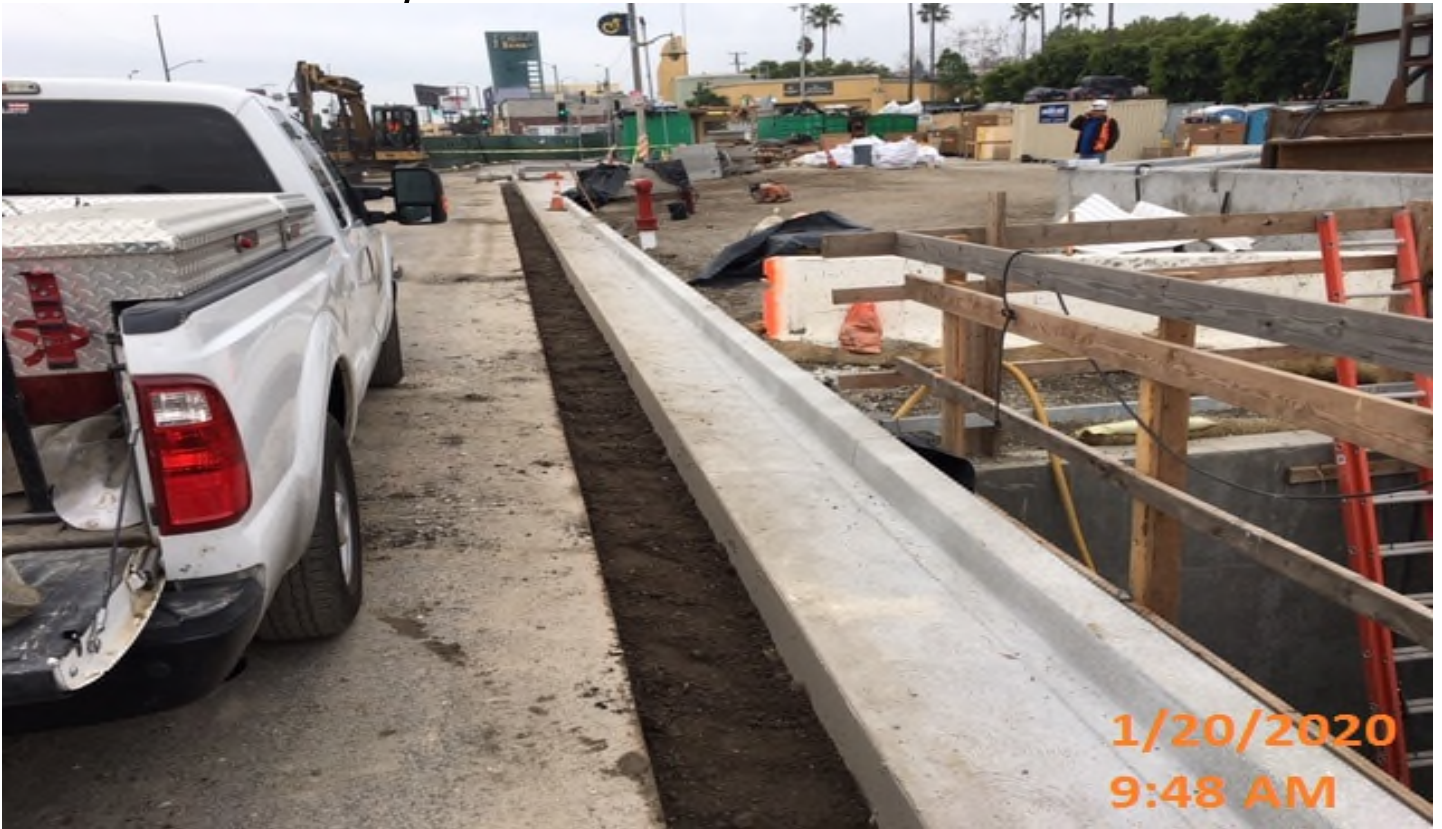
MLK Station - Grading gutter in preparation for paving from Sta 129+50 – 130+05 at the plaza level.
