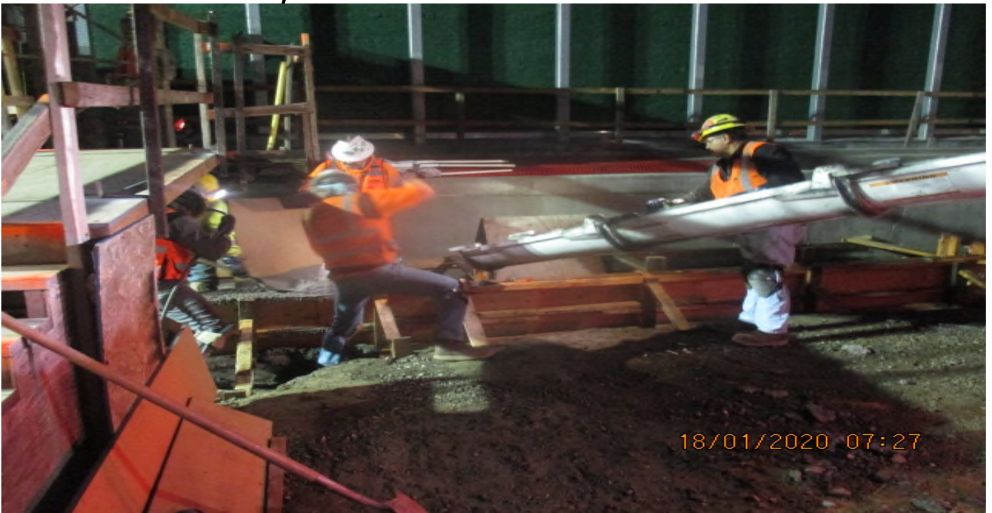
Leimert Park Station – Placing concrete on the east section of the south planter box footing at the plaza level. 1/18/20
