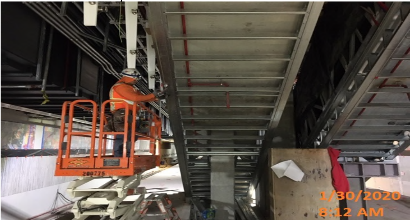
Expo Station - Installation of laminated cladding frame for the metal panels beneath staircase 1&2 and escalator 3&4 at the platform level.
