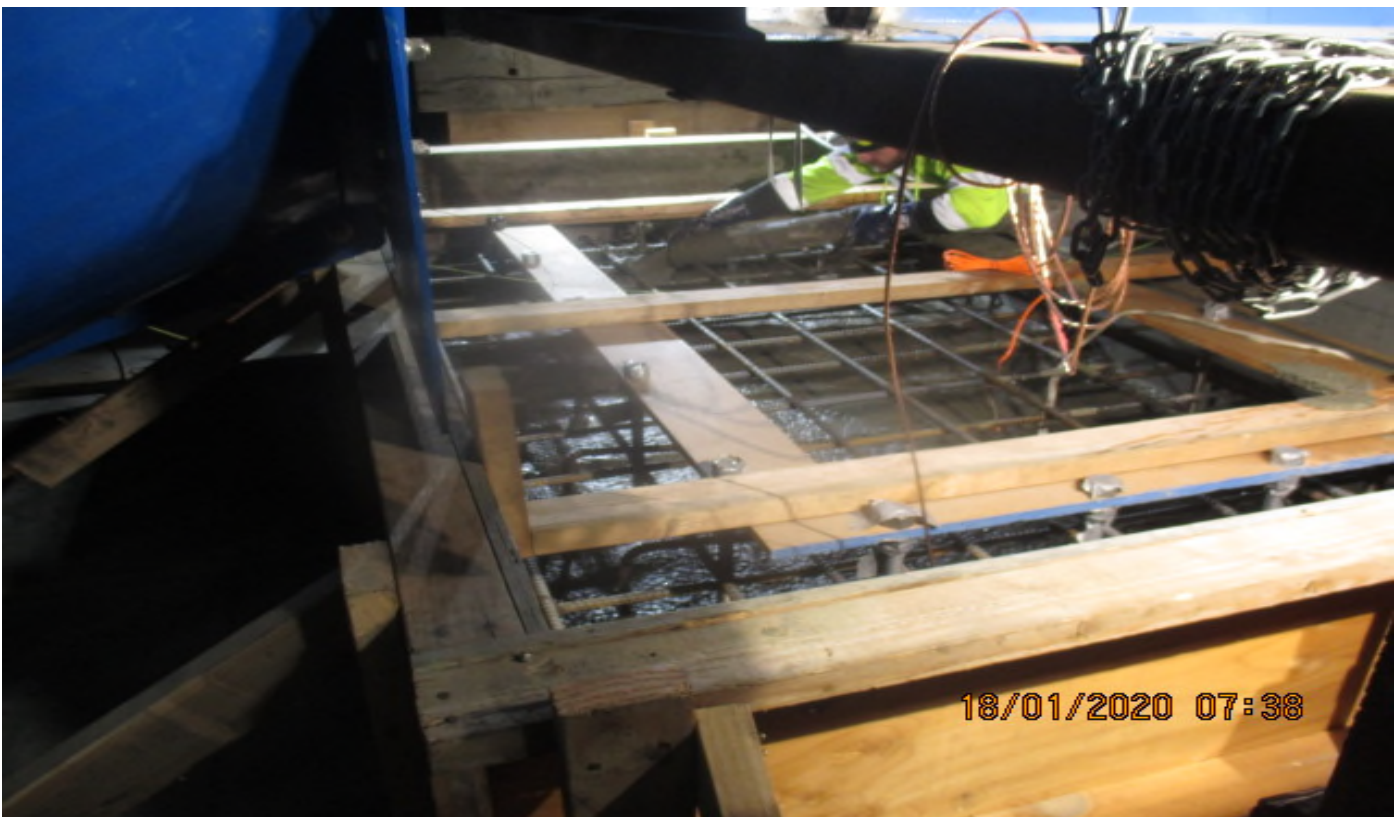
Leimert Park Station – Prepping steel framing edge in order to mount EMP box at the concourse level.
