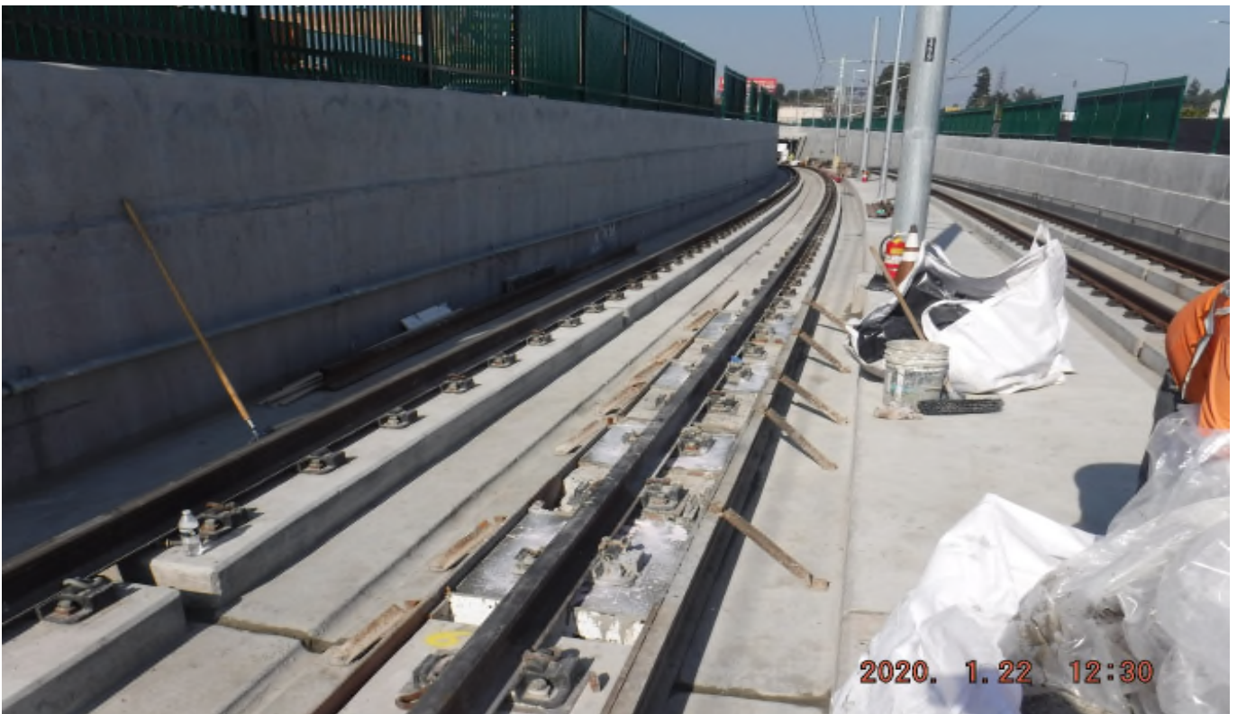
48 th Street - STA364+46_ Looking North_ Track structure disturbance in search of BLS conduits_ 48ST
