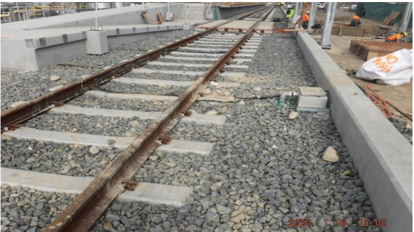
Florence/Brea – STA211+30_ Looking North_ Track structure disturbed_ PUNCH LIST_ La Brea.
