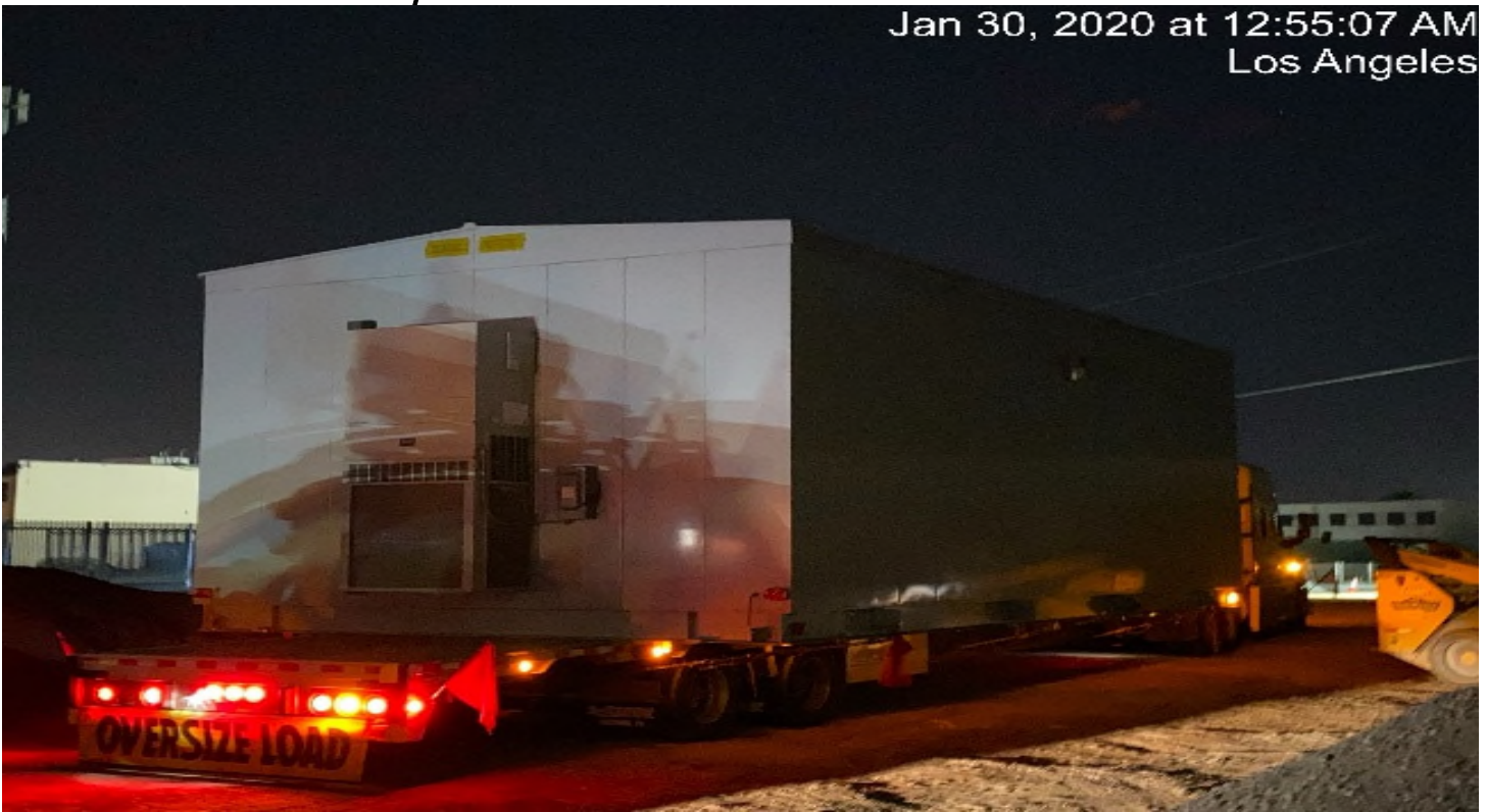
UG3 – Delivering the sub-station bungalow for the auxiliary power site at Victoria Yard adjacent to the south end portal.
