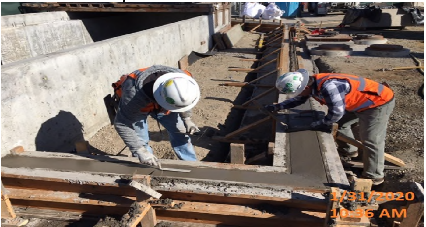
Leimert Park Station – Continued placing concrete and smoothing the surface for both north and south planter box sections at the plaza level.
