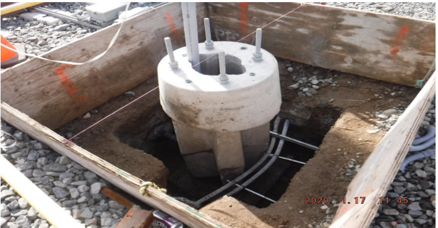
Florence/West – STA262+75_ Track structure disturbed to set Xing foundation between tracks_ West.
