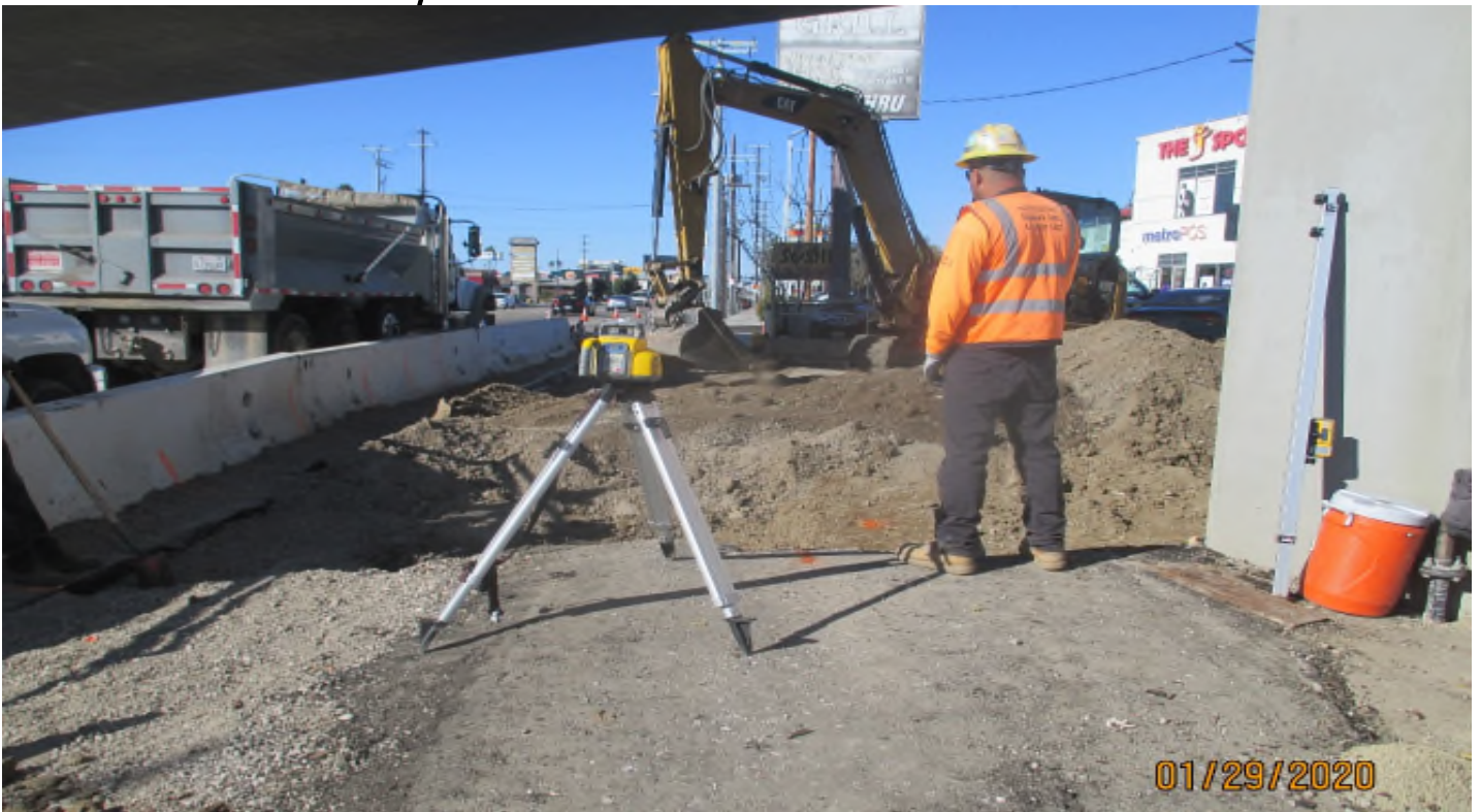
Manchester Bridge: – Sidewalk grading on Manchester.
