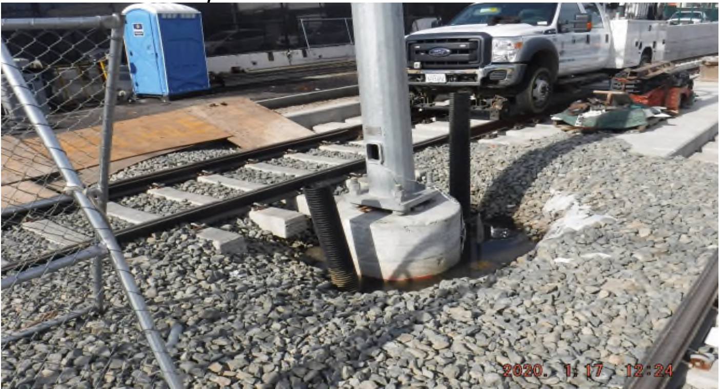
48 th Street - STA364+50_ Looking North_ Excavation full of water around OCS 1278 foundation_ 48ST
