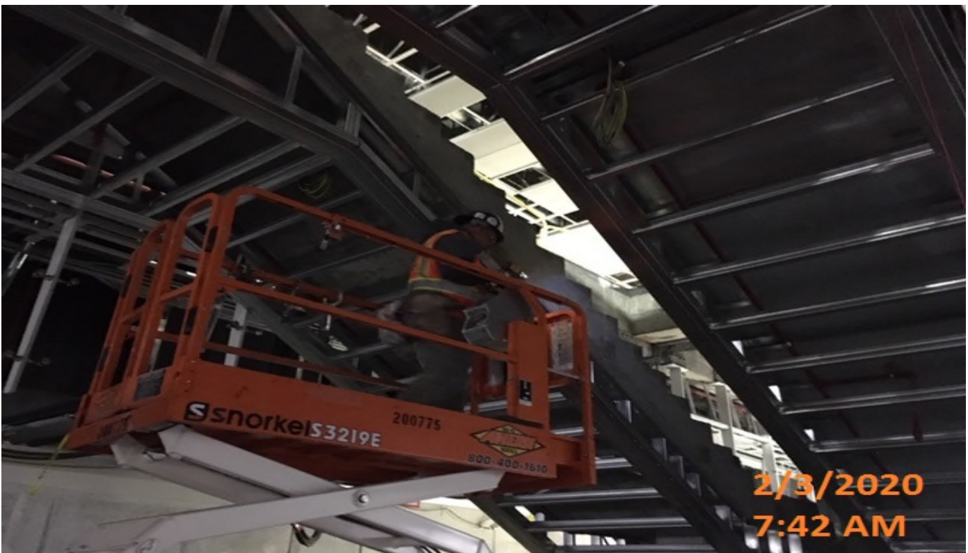
Expo Station - Installation of laminated cladding frame for the metal panels beneath staircase 1&2 and escalator 3&4 at the platform level.
