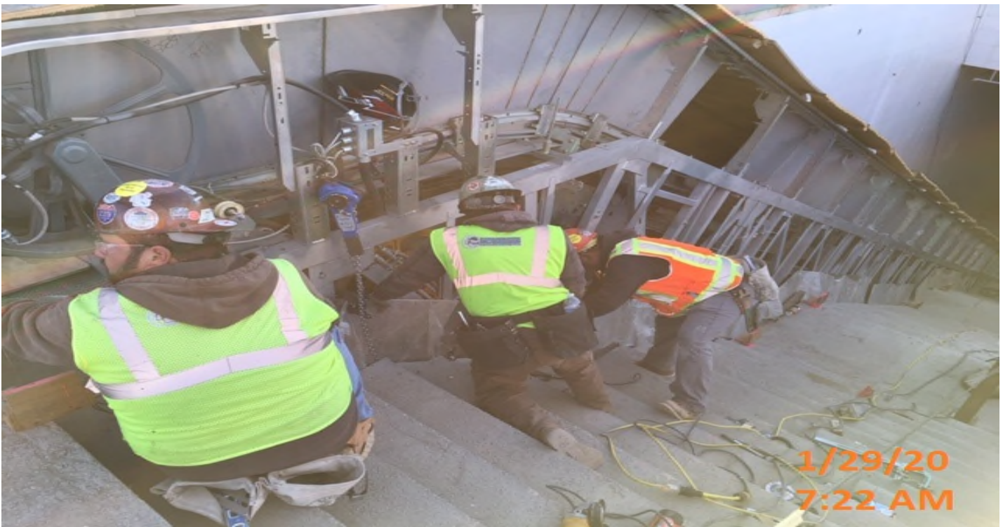
MLK Station - Continued installing edge plates for Escalator 1&2 at the main staircase landing of the plaza level.
