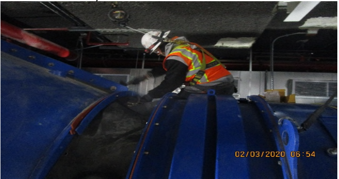
Leimert Park Station – Continue installing silicone gaskets and roughing in flex connectors to EVF-6-101 and EVF-6-301 in the South Fan Room C – 102 Fan Rooms of the concourse level.
