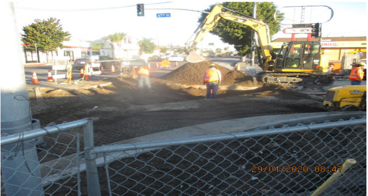
UG3 – Continued excavating and removing existing rail lines and roadway along the northbound lane of 67th St and Crenshaw Blvd. 1/28/20
