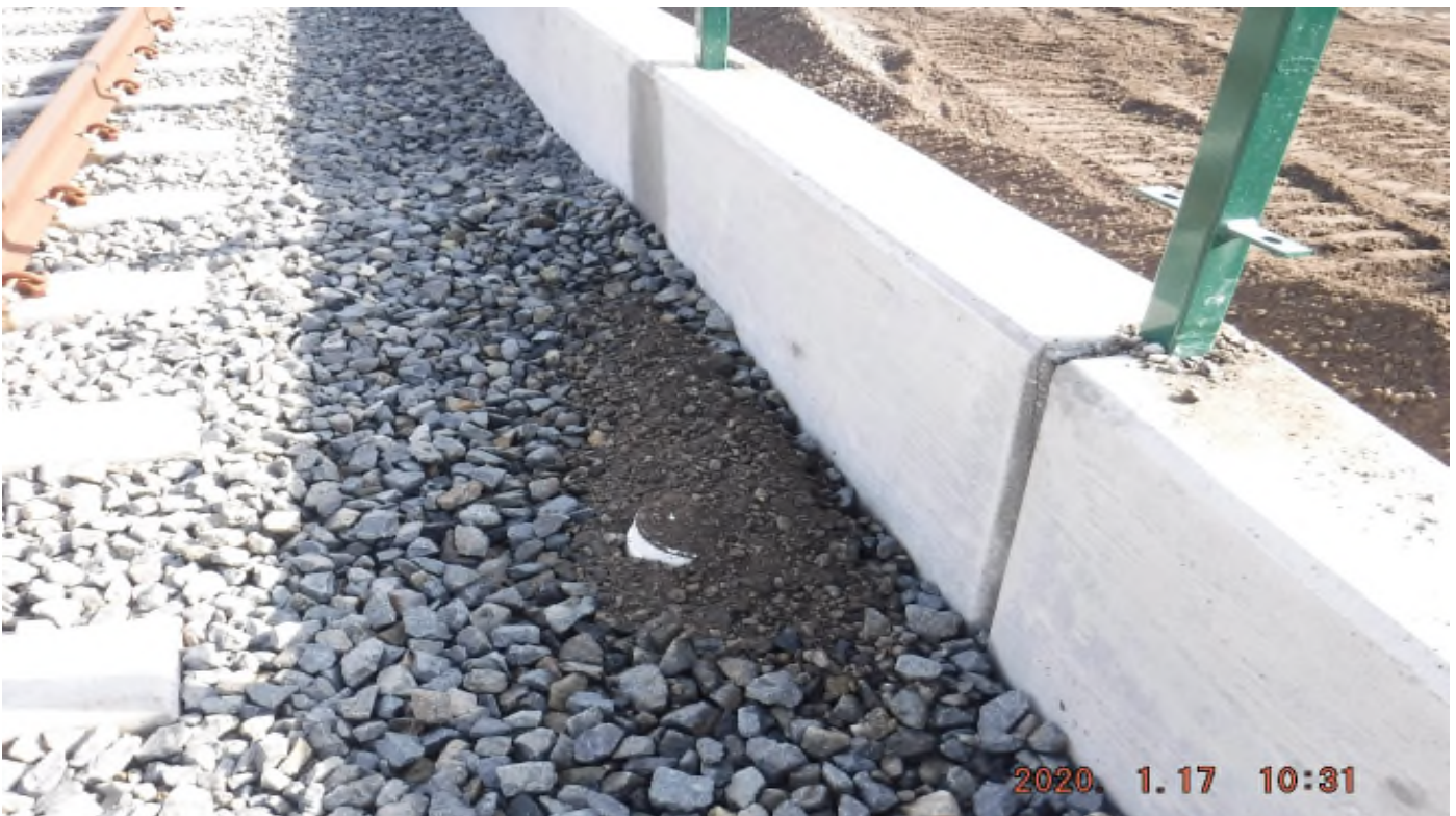
Florence/Brea – STA211+20_ Looking South_ Dirt spill over track ballast_ PUNCH LIST_ La Brea.
