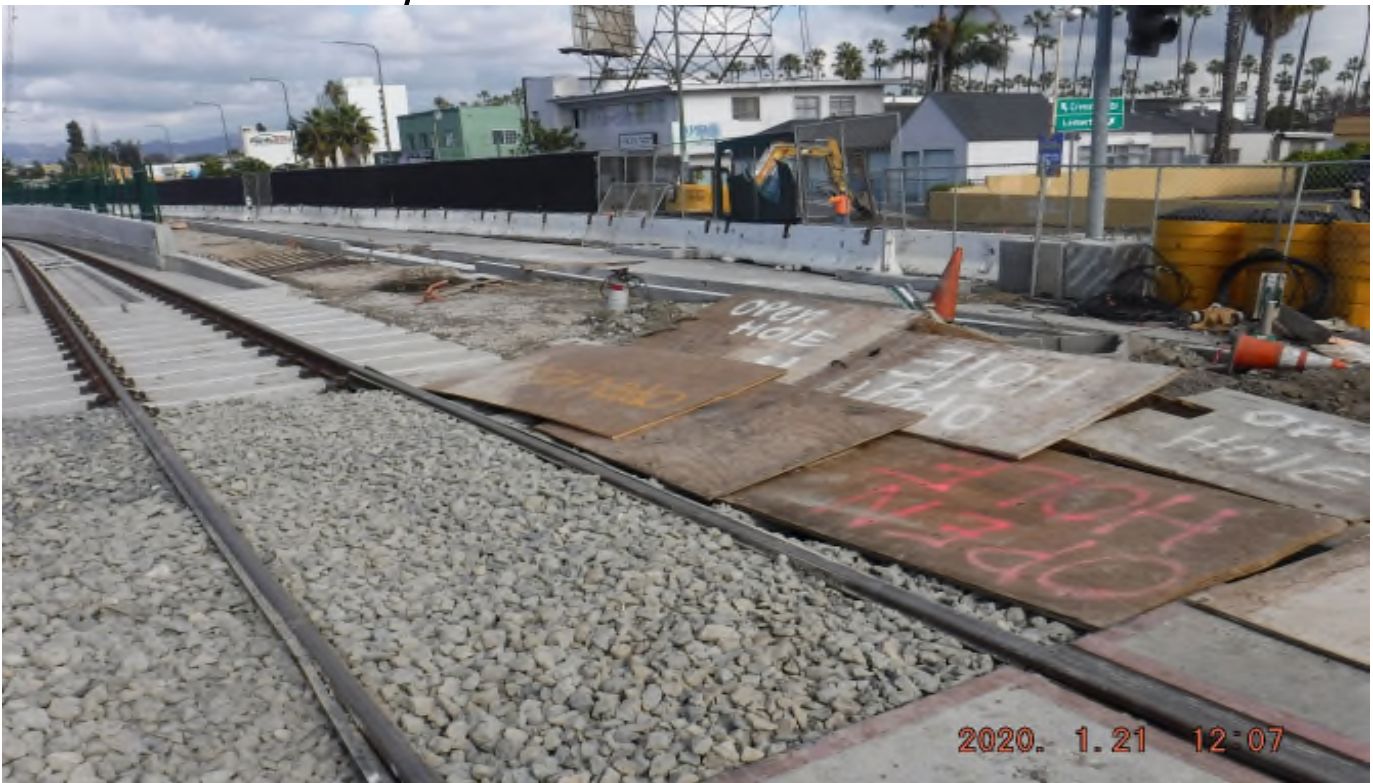
48 th Street - STA364+46_ Looking North_ Track structure disturbance in search of BLS conduits_ 48ST
