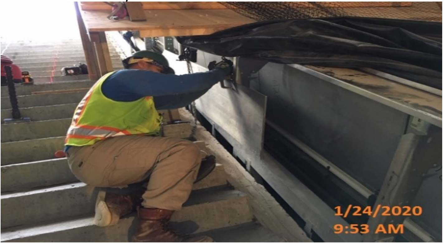
MLK Station - Continued installing edge plates for Escalator 1&2 at the main staircase landing of the plaza level.
