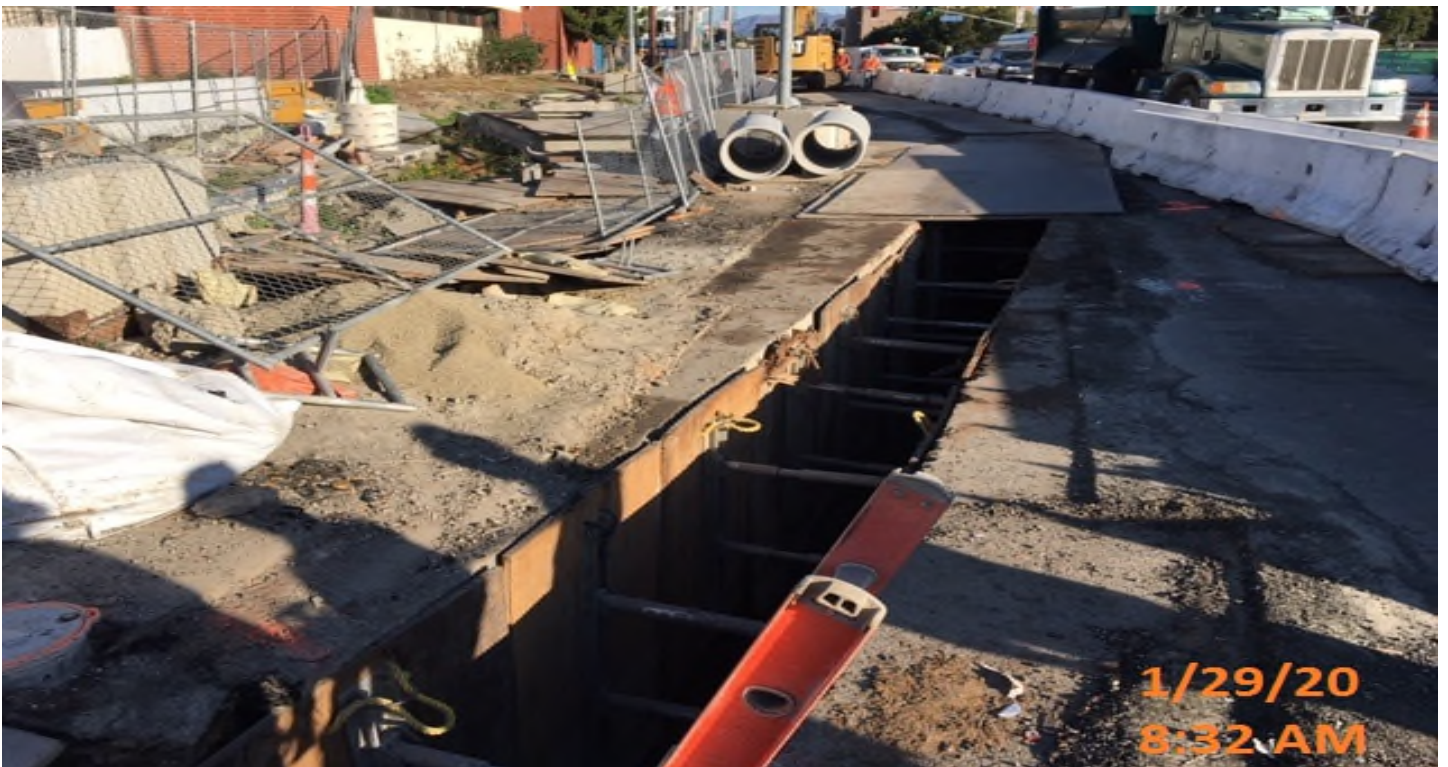
Expo Station - Excavating and shoring for Line W – storm drain near the northwest corner of Rodeo Blvd and Crenshaw Blvd.
