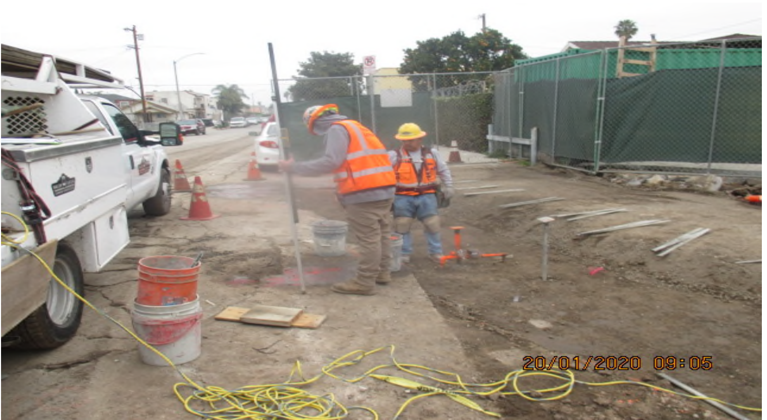
UG3 – Concrete placement of the eastbound sidewalk of “New Road.”
