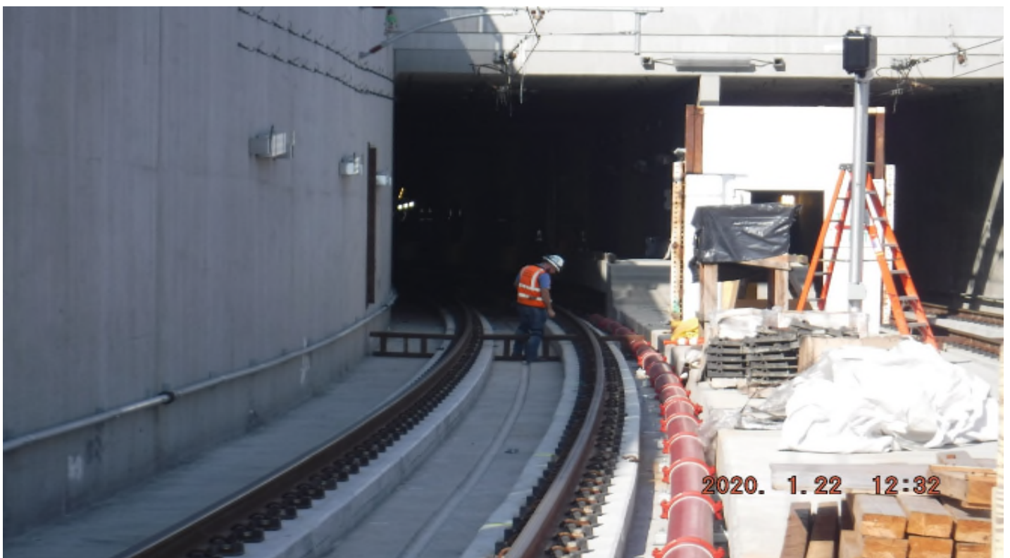
UG-4- Continue sack and patch and applying fog cure for walls along the northbound tunnels from Sta 372+00 – 377+26.
