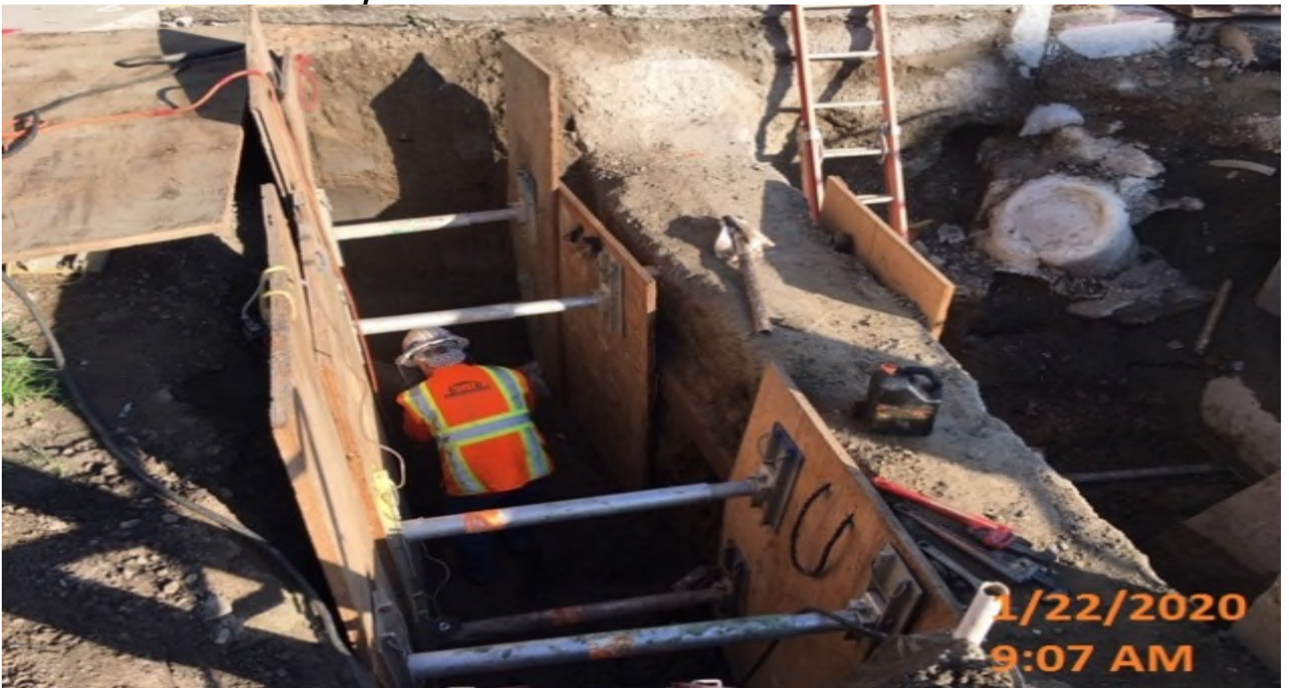
MLK Station - Capping and removing abandoned 10" oil pipe located on the southwest corner of Martin Luther King Blvd and Crenshaw Blvd.
