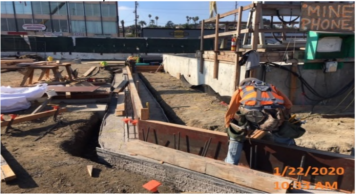
Leimert Park Station – Continued building sections of formwork for the north planter box footing at the plaza level.
