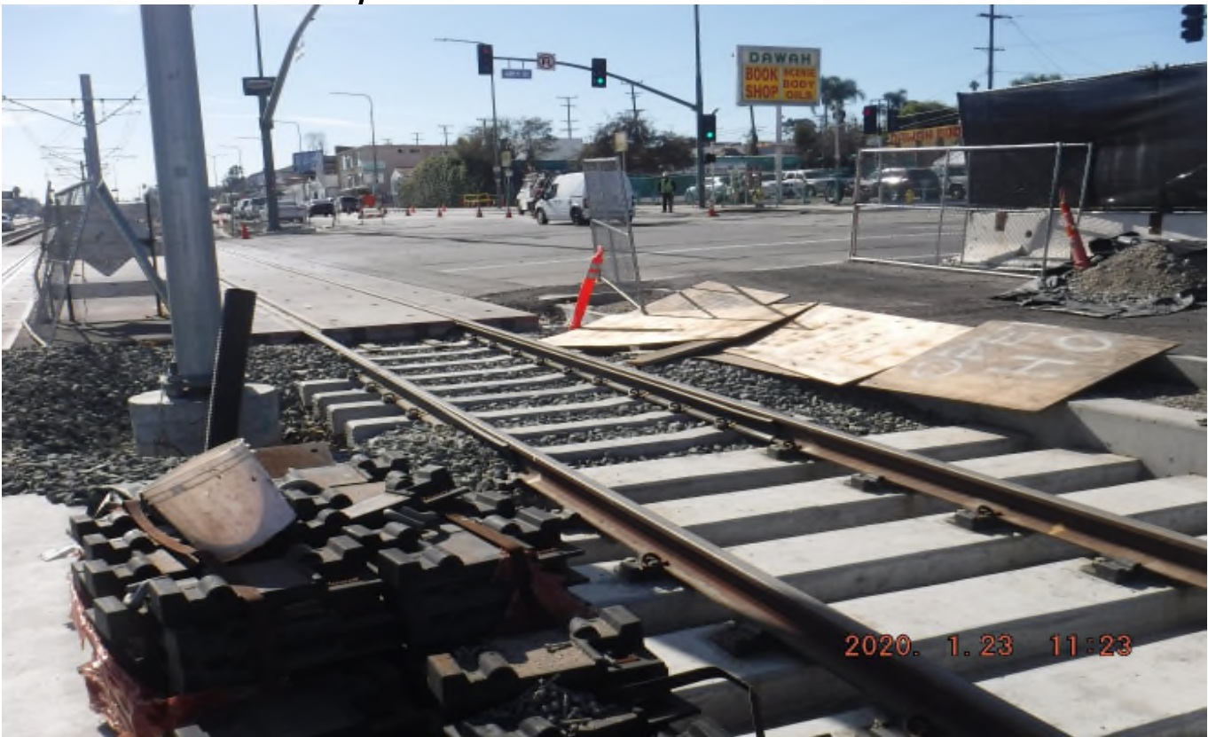
48 th Street - STA364+46_ Looking South_ Track structure disturbance in search of BLS conduits_ 48ST.
