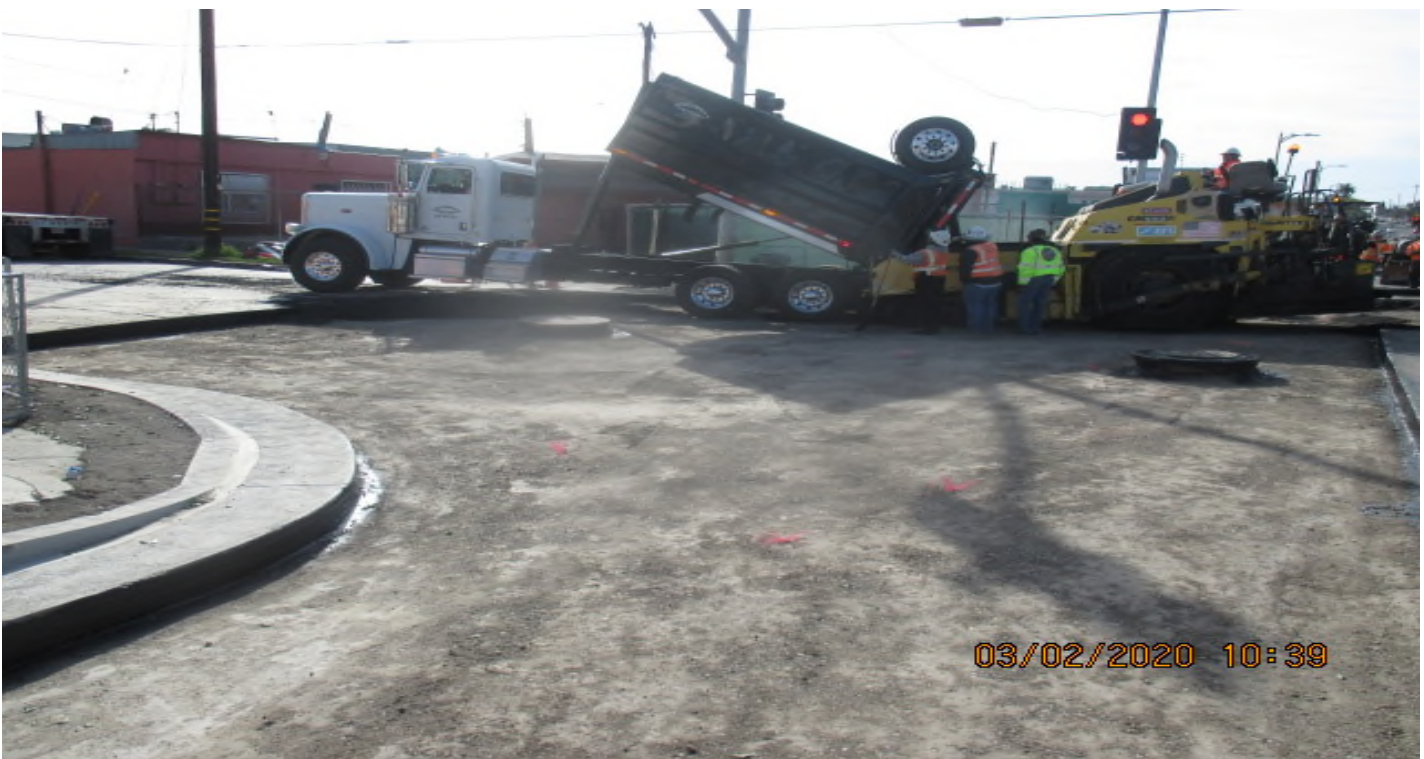
UG3 – Continued backfilling and compacting to final roadway grade in preparation for concrete placement on 67th St and Crenshaw Blvd. 2/1/20
