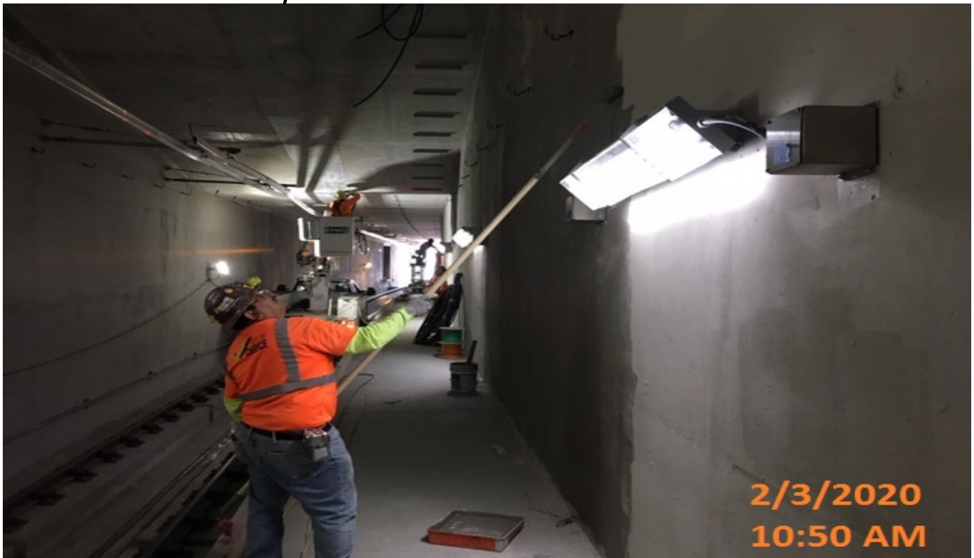
UG-4- Continue sack and patch and applying fog cure for walls along the northbound tunnels from Sta 372+00 – 377+26.
