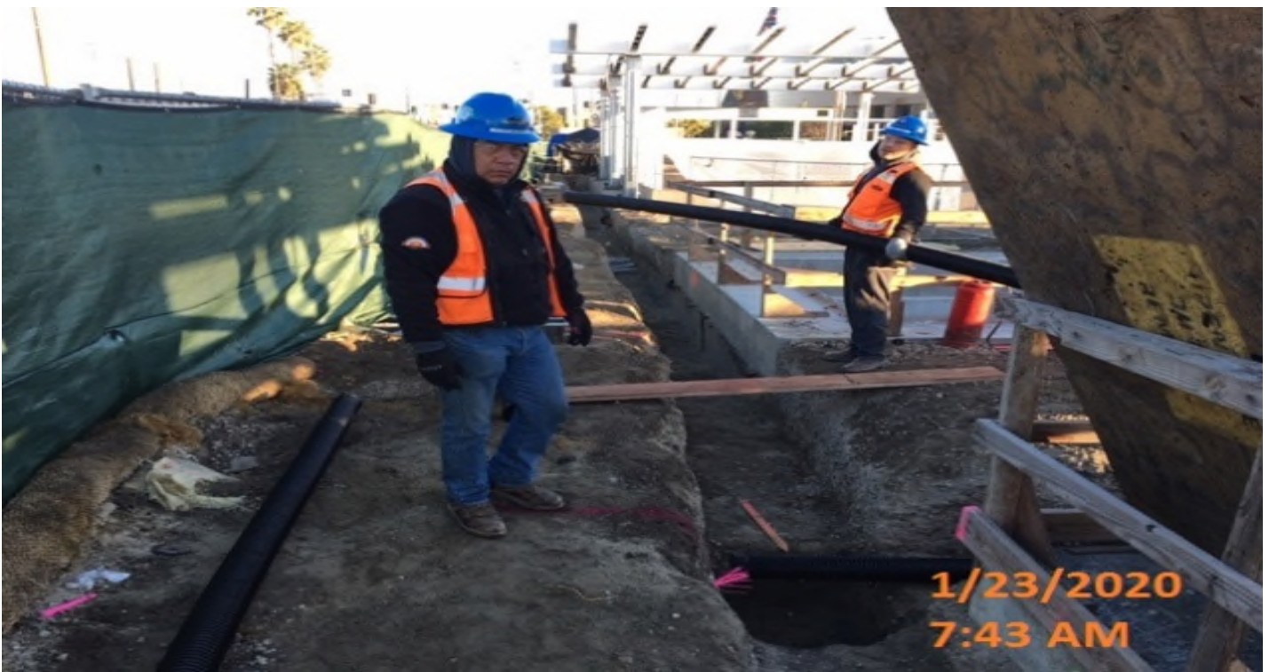
Expo Station - Continue excavating for drainage adjacent to structural Elevators 1&2 at the plaza level.
