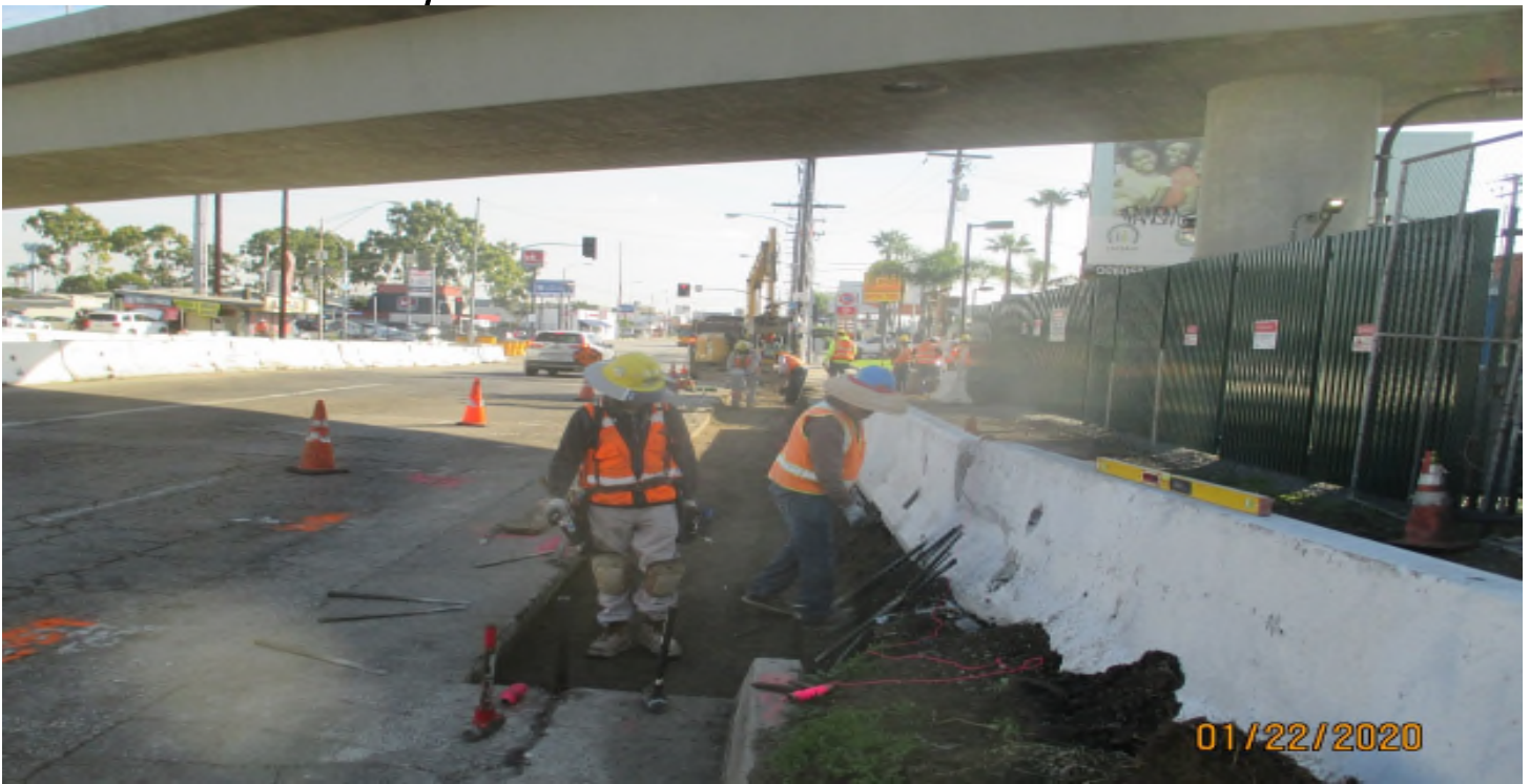
Manchester Bridge: – Curb and gutter grading and setting forms on the south side of Manchester.
