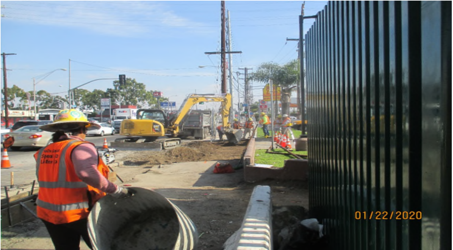
Manchester Bridge: – Curb and gutter grading and setting forms on the south side of Manchester.
