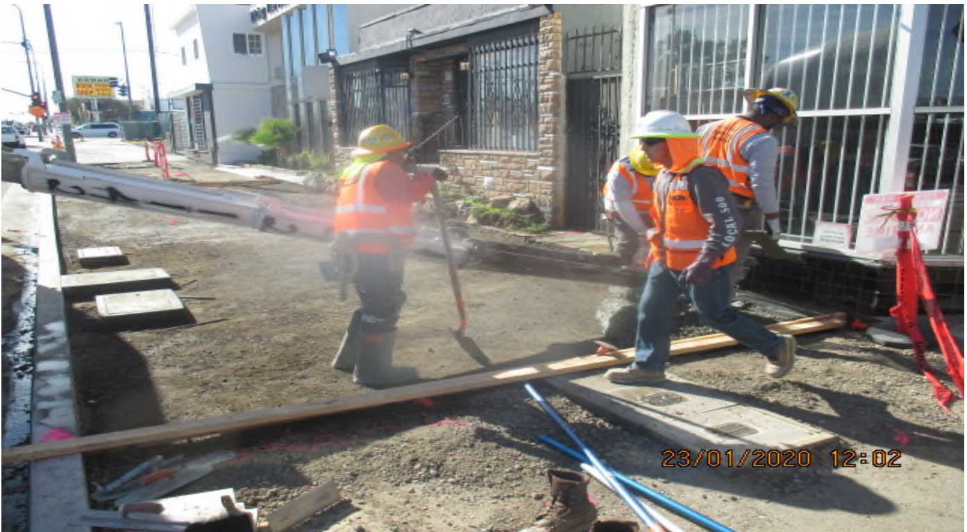
Park Mesa – Began formwork for meter/utility boxes on Crenshaw Blvd between Brynhurst Ave to 48th St. 1/22/20
