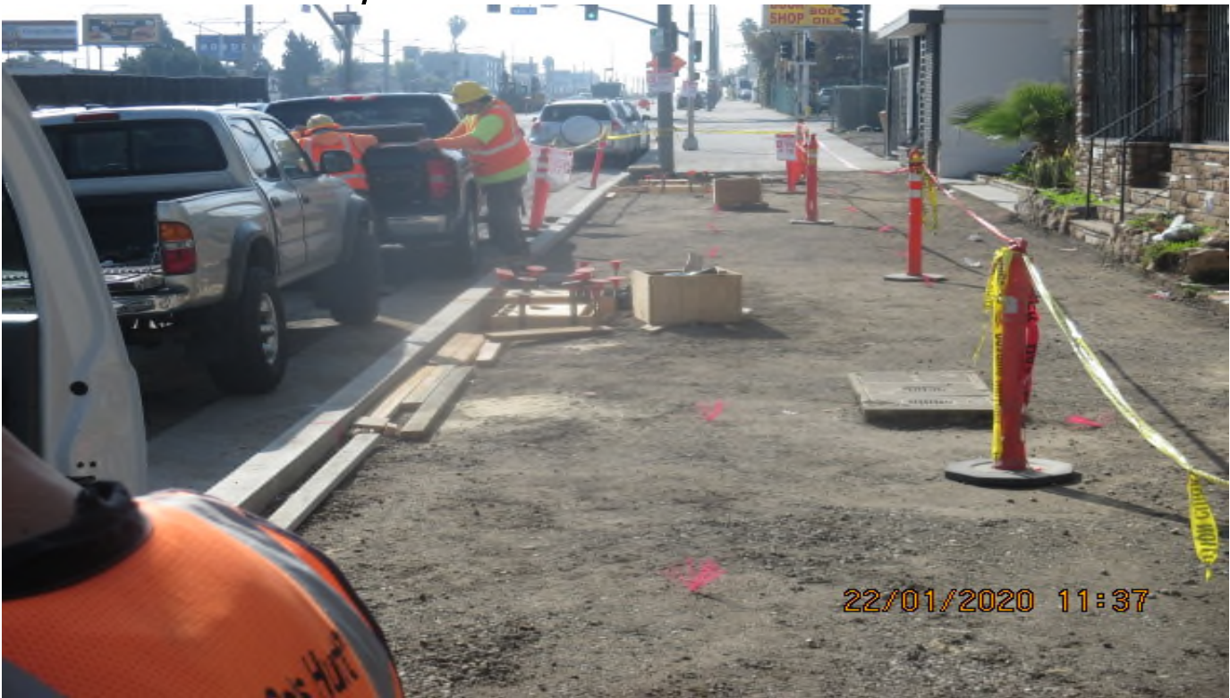
Park Mesa – Began formwork for meter/utility boxes on Crenshaw Blvd between Brynhurst Ave to 48th St. 1/22/20
