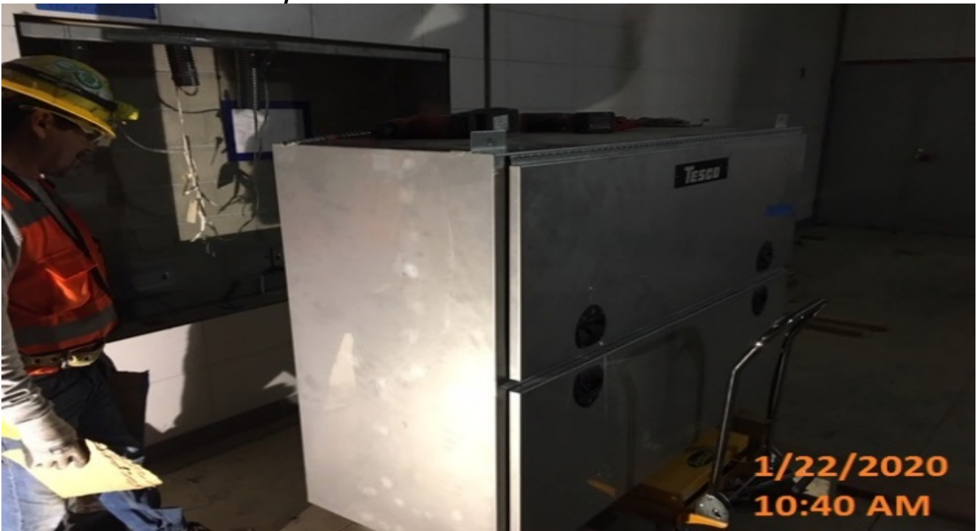
Leimert Park Station – Prepping steel framing edge in order to mount EMP box at the concourse level.
