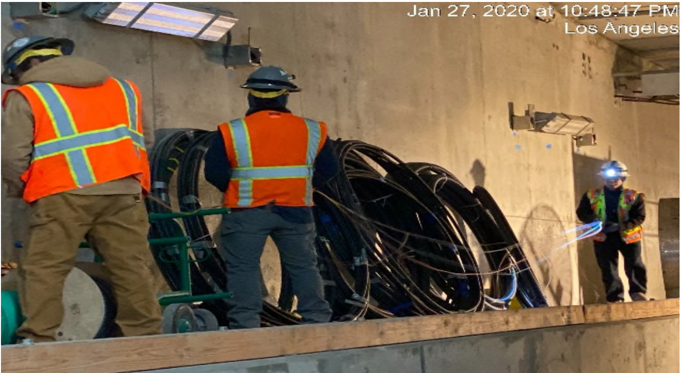
UG-4- Continue pulling wire for the emergency lighting along the northbound tunnel at Sta 375+50.
