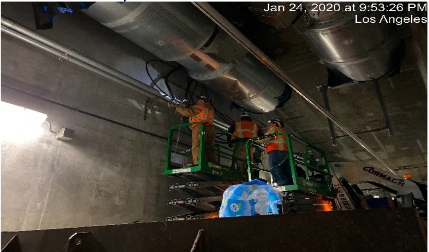
UG3 – Continue wiring and running cable for the booster fans at the northbound tunnel at Sta 307+25.
