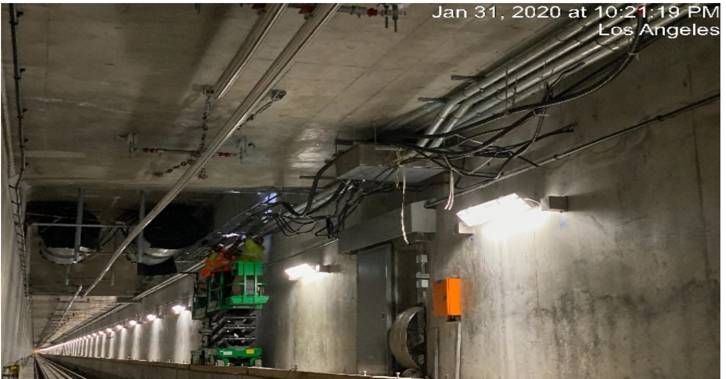
UG3 – Continue wiring and running cable for the booster fans at the northbound tunnel at Sta 307+25.
