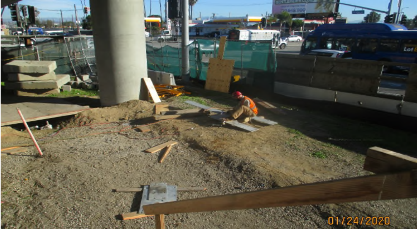
Aviation/Century – Potholing to locate utilities on Aviation at 111th.
