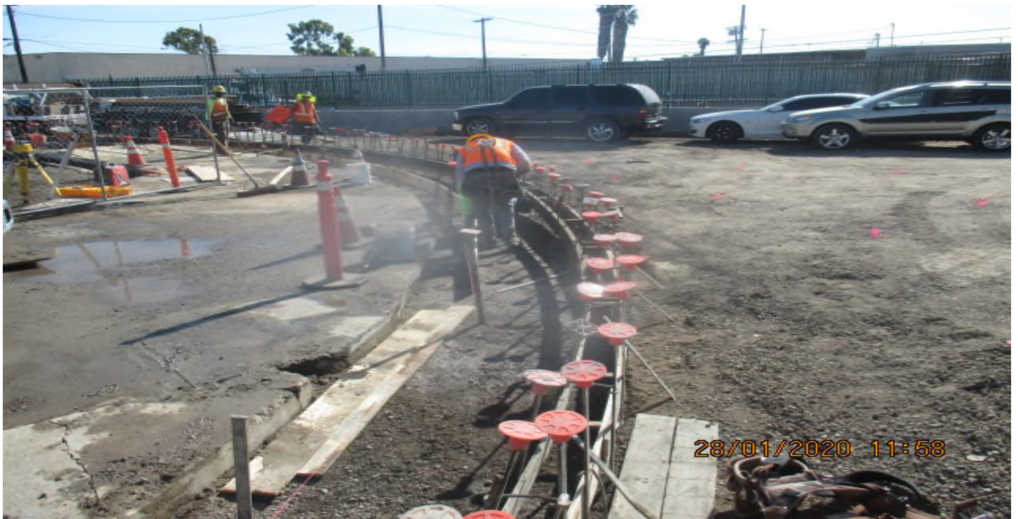
UG3 – Continued excavation and compaction for new curb/gutter at North Victoria Ave. 1/27/20
