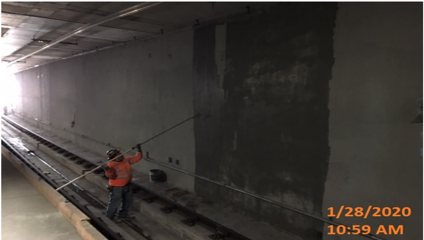
UG-4- Continue pulling ground wires and power to the IDS control cabinets in the southbound tunnel at Sta 371+25.
