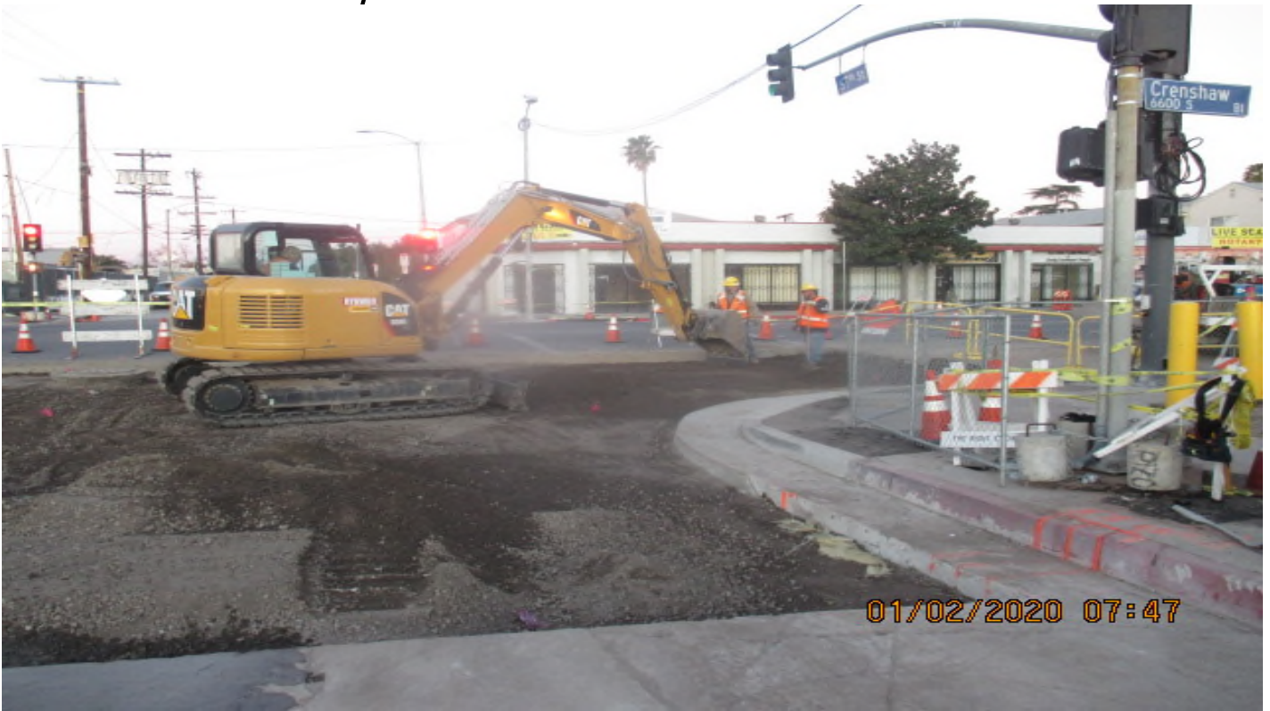
UG3 – Continued backfilling and compacting to final roadway grade in preparation for concrete placement on 67th St and Crenshaw Blvd. 2/1/20
