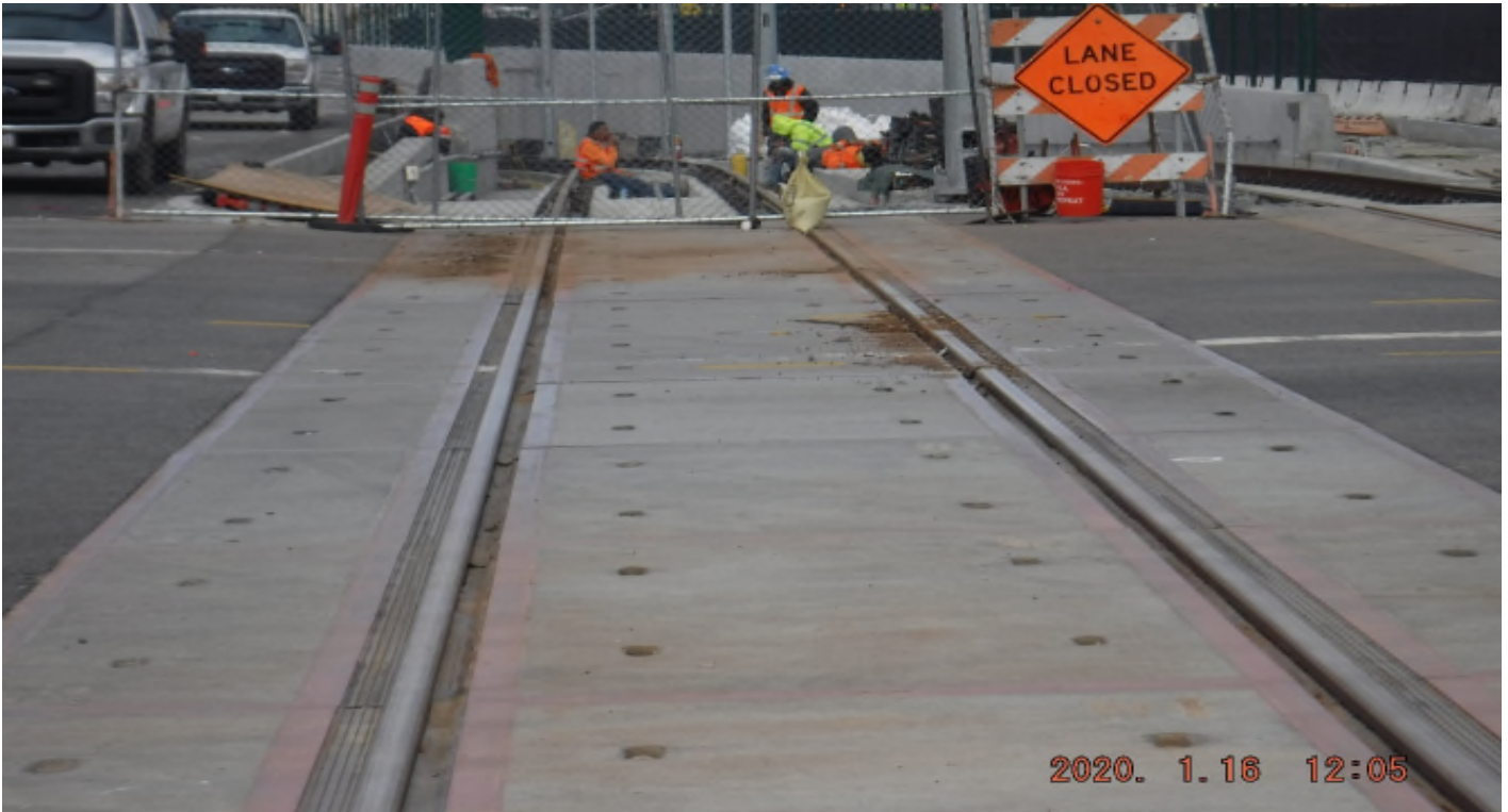
48 th Street - STA363+30_ Looking North_ Cleaning flangeway_48ST.
