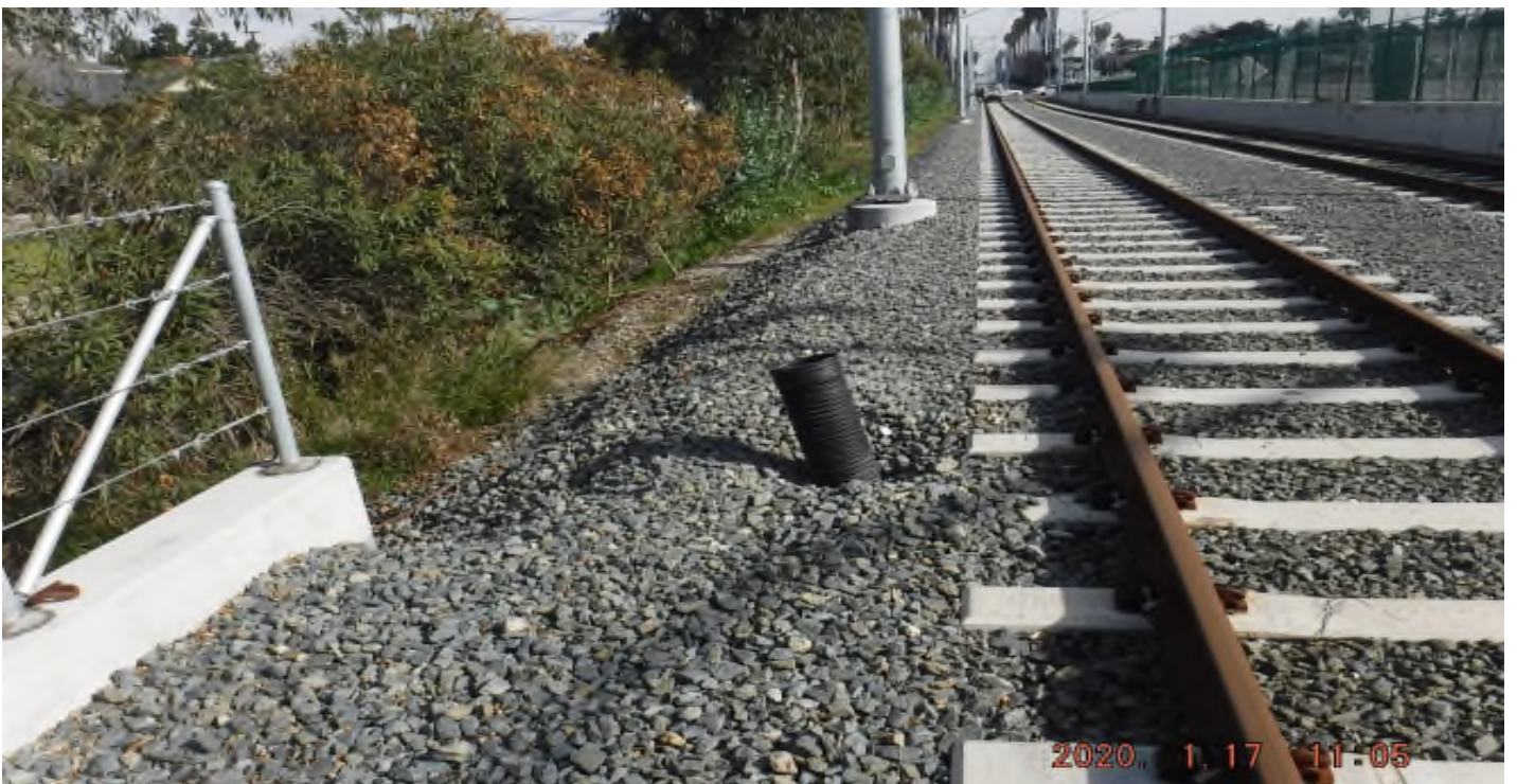
Florence/West – STA262+74_ Looking South_ Track ballast removal 4 pedestrian landing pad_ West.
