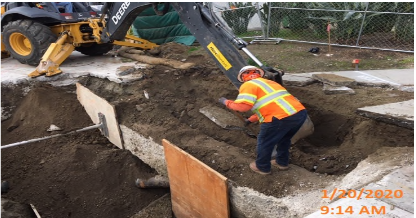
MLK Station - Grading gutter in preparation for paving from Sta 129+50 – 130+05 at the plaza level.
