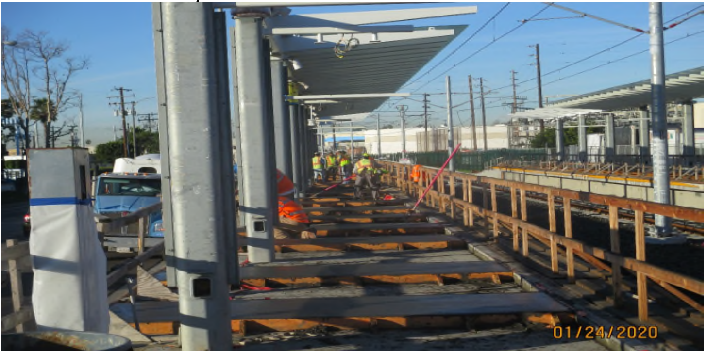
Florence/Hindry: – Sanding and prepping for paint at the Hindry Station.
