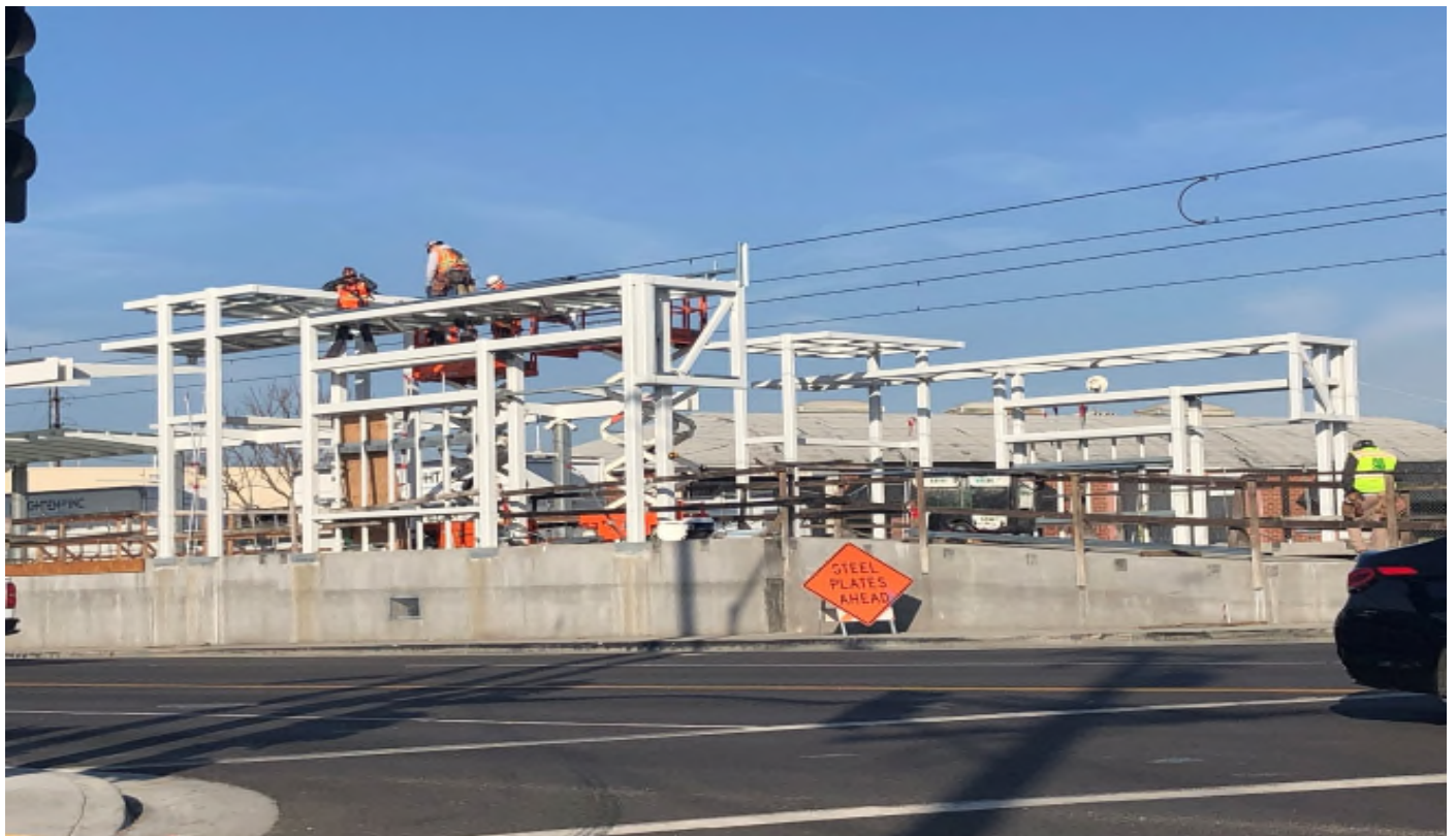
HINDRY AVE- Metal stub framing at the Hindry Station.
