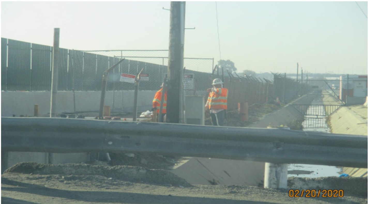
104 th STREET – Chain link fence repair at 104th street.
