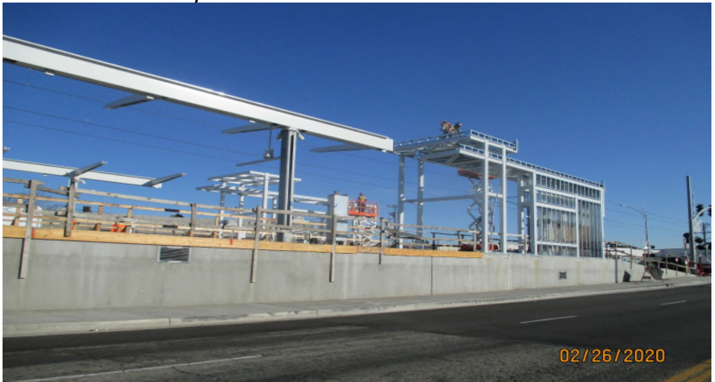
HINDRY AVE- Metal stud framing at the Hindry Station.
