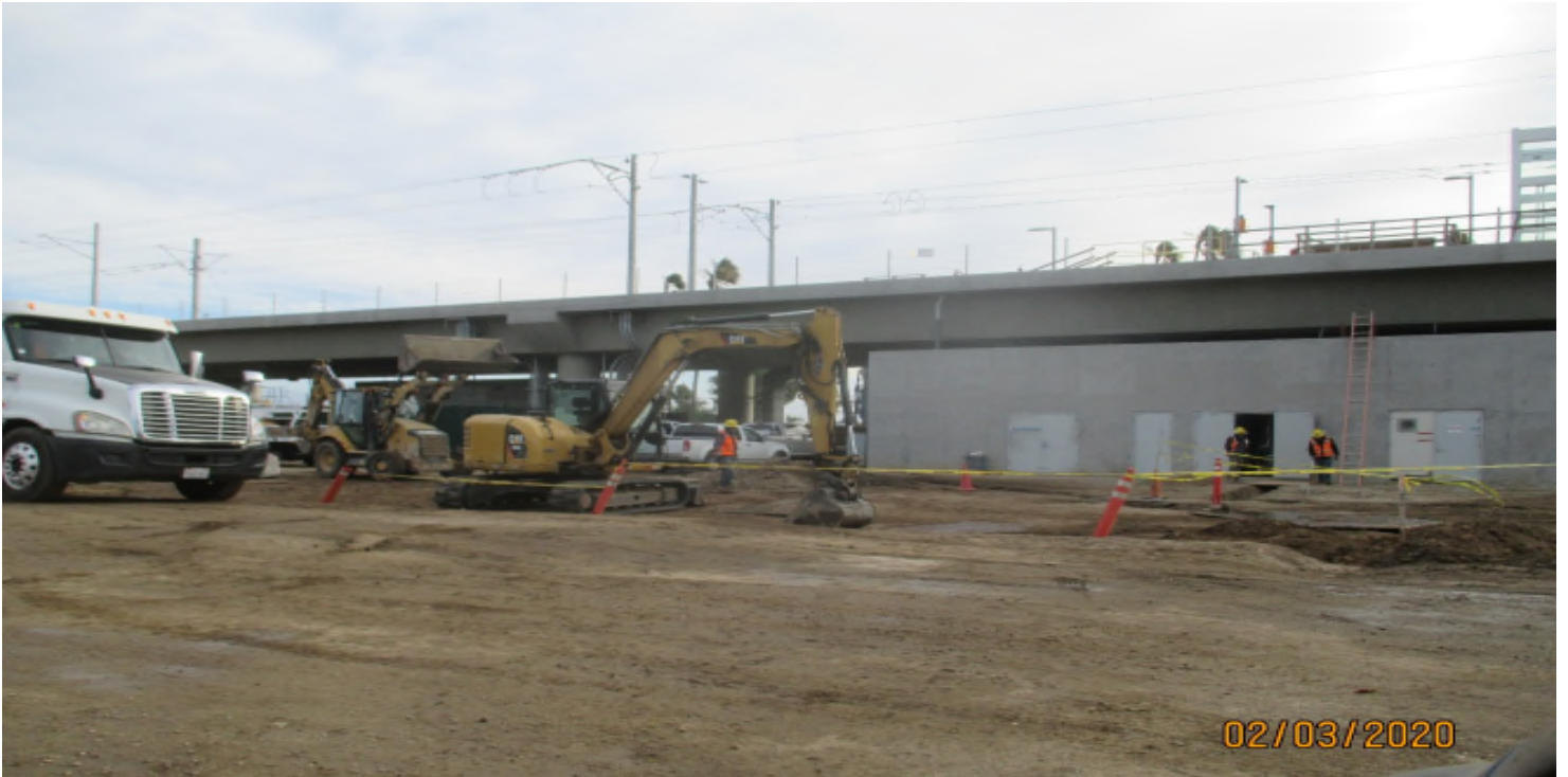
AVIATION/CENTURY- Grading and excavating at the Aviation Station plaza area.
