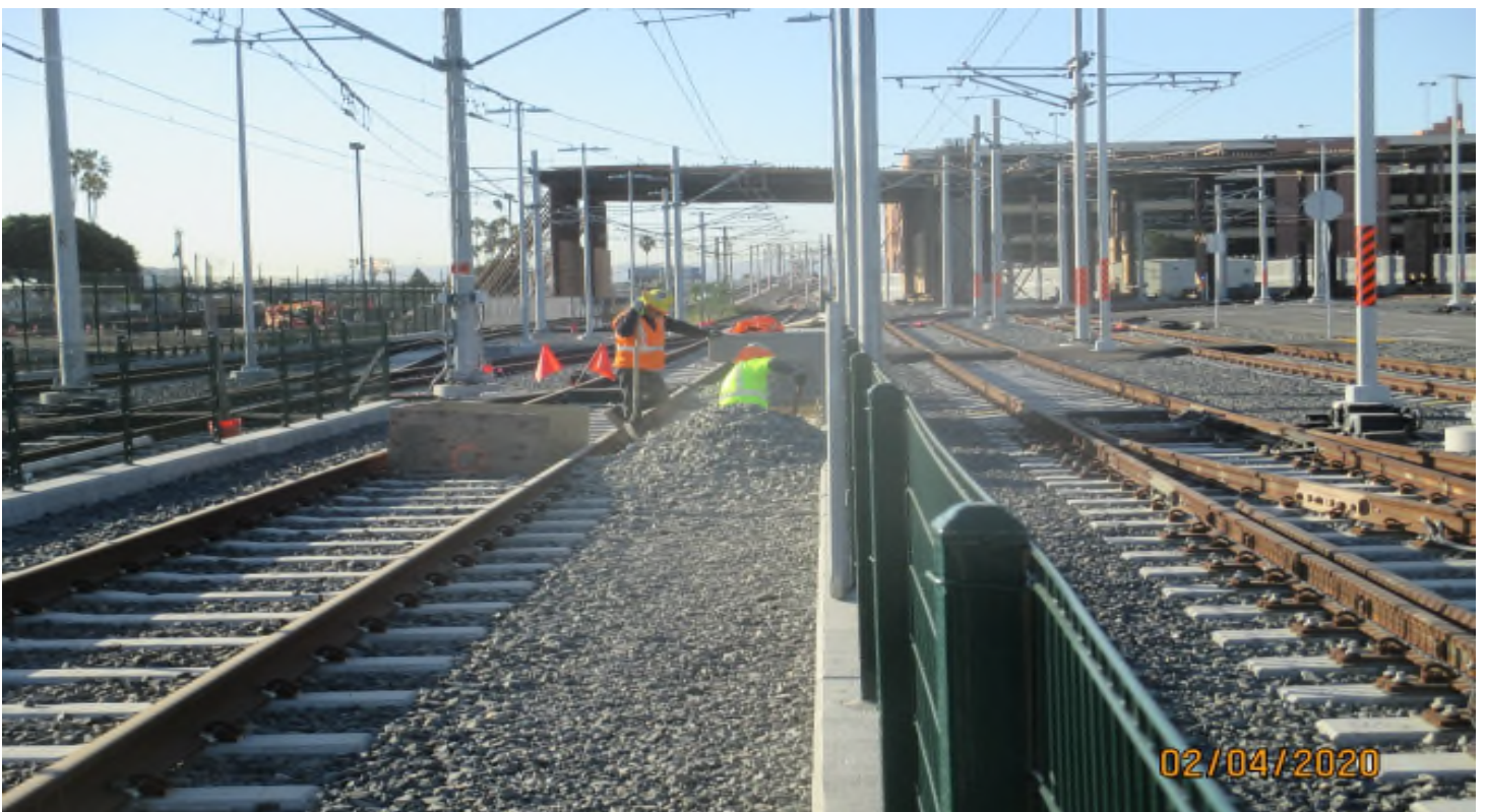
96 th STREET- Ballast removal to build the operator's platform stairs.
