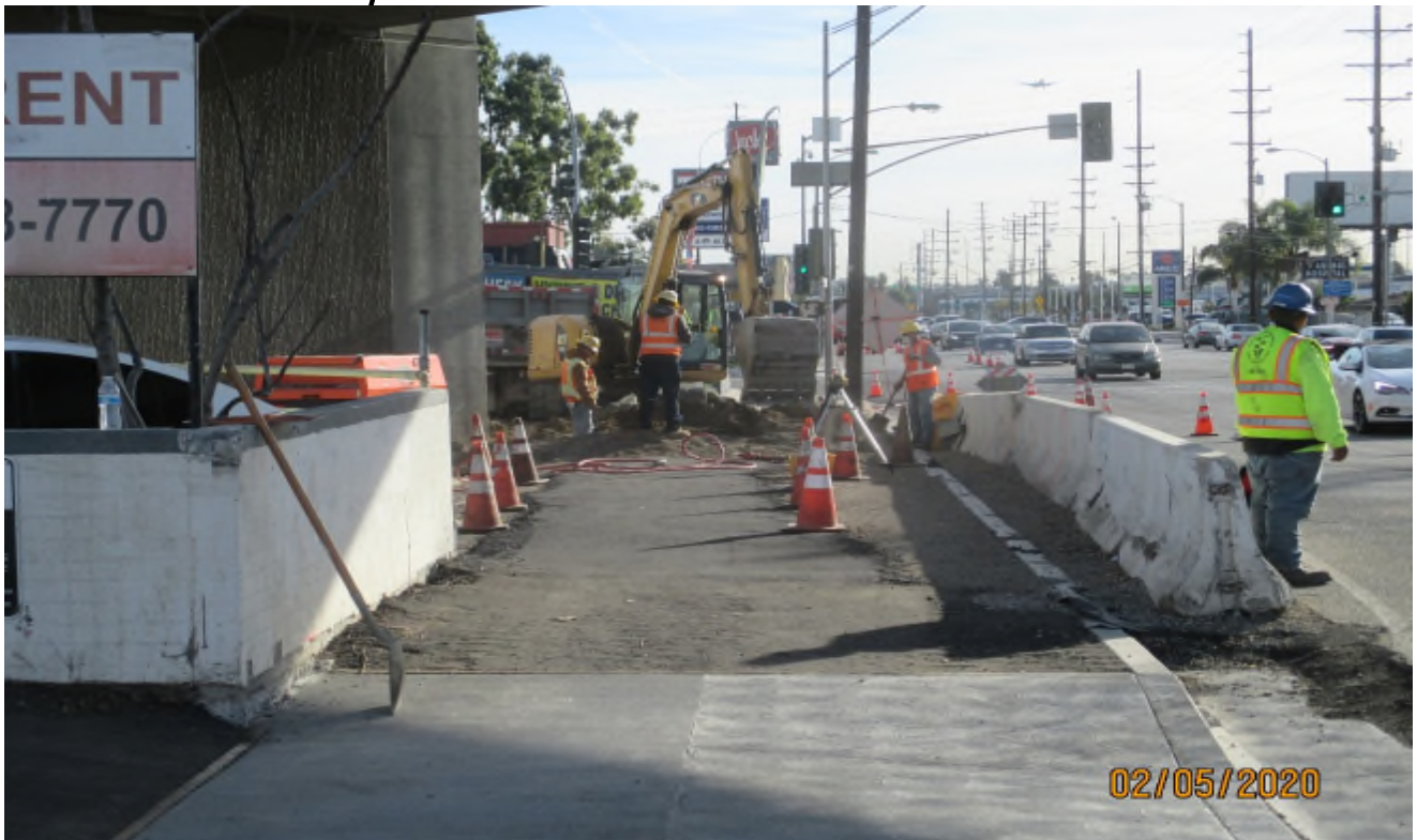
MANCHESTER AVE- Sidewalk subgrade grading at Manchester.
