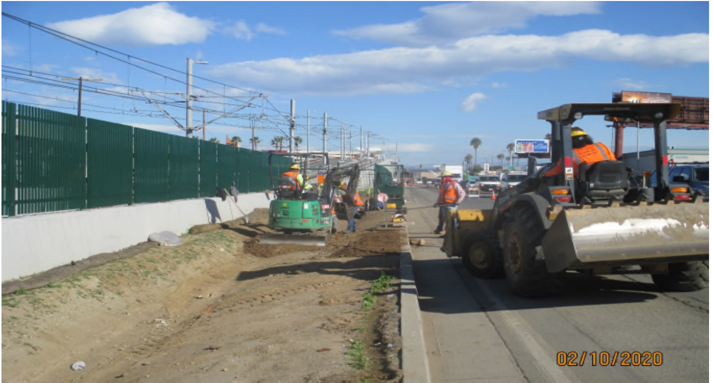
UG 1- Drainage swale grading at the north portal of UG-1.
