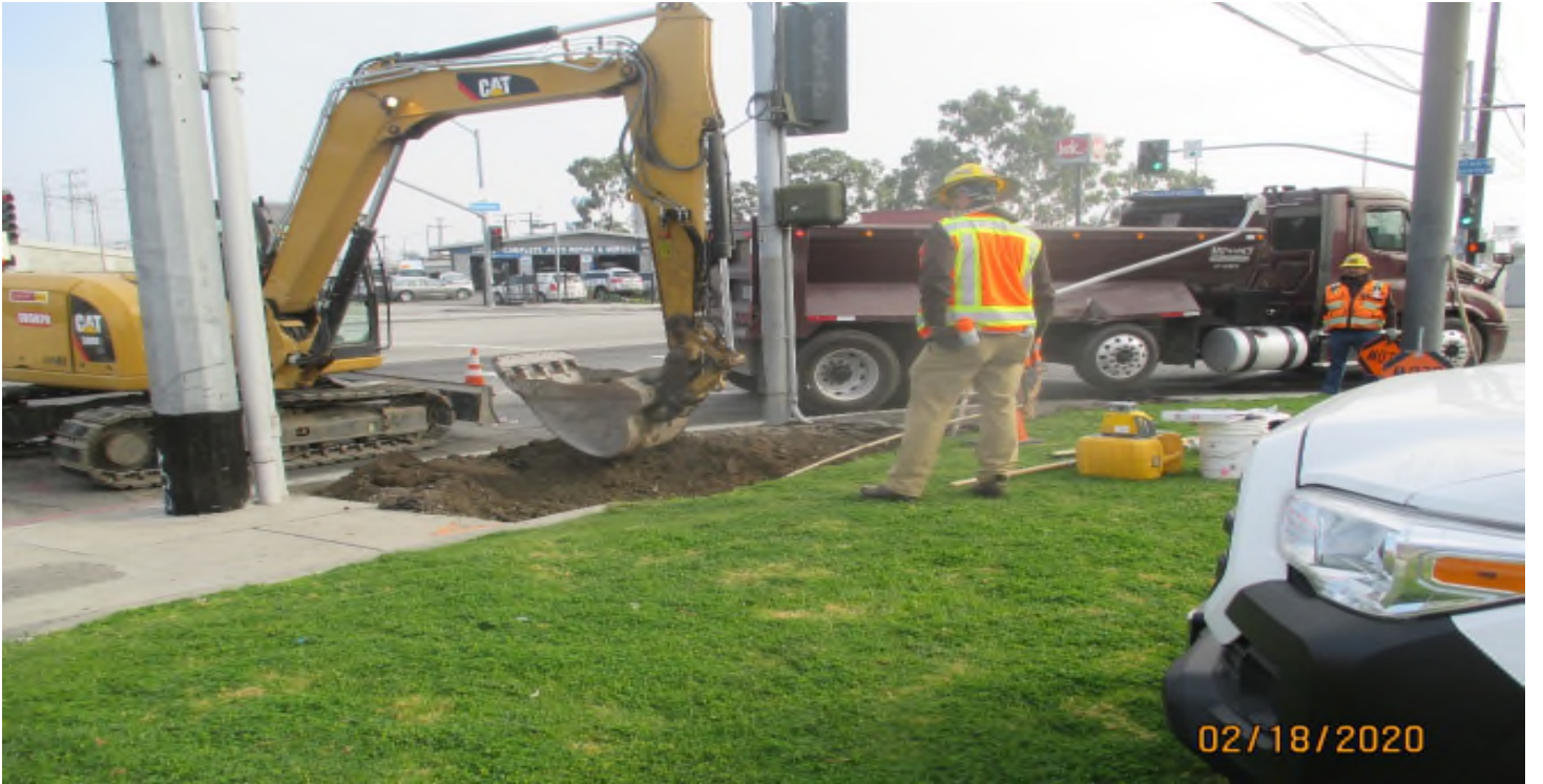
AVIATION/CENTURY- Sidewalk subgrade grading at Aviation and Manchester.
