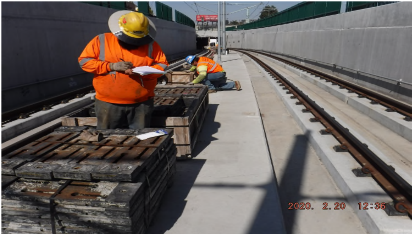
UG4 – STA367+50_ Looking North_ OTM inventory_UG4 south ramp_48ST
