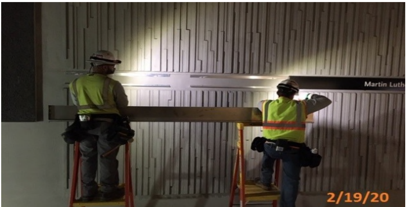
MLK STATION –Smithcraft installing hardware and signage.
