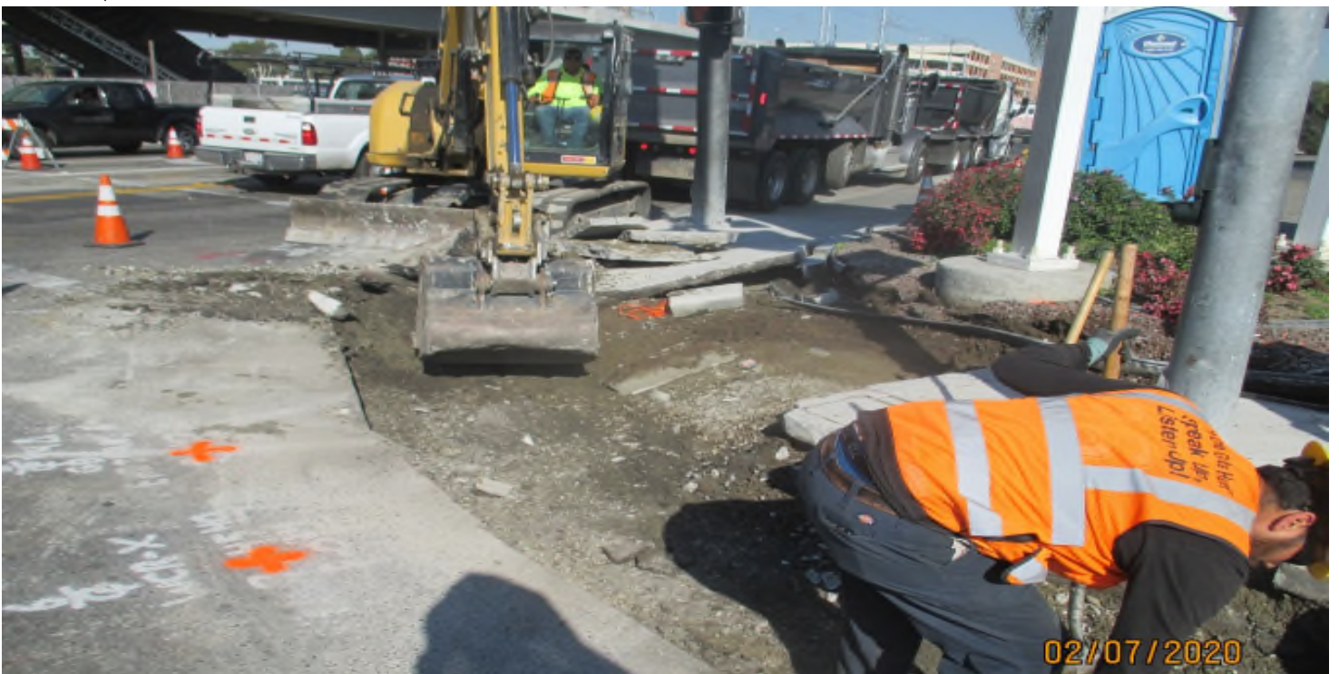
AVIATION/CENTURY- Curb & gutter demo on Aviation & Century.
