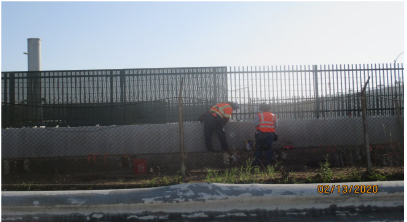
UG 1- Installing the screen panels at UG-1.
