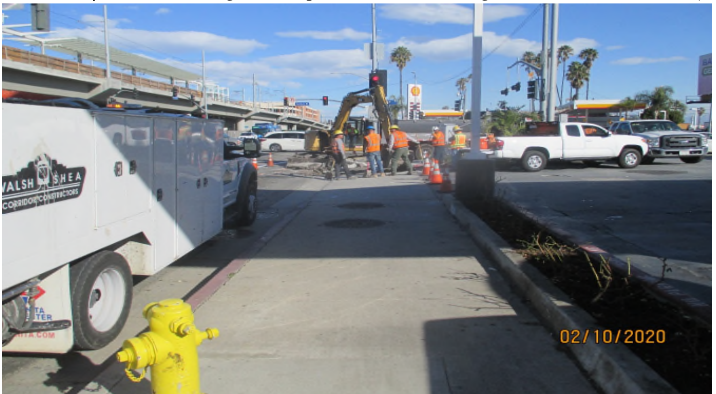
AVIATION/CENTURY- Curb & gutter demo on Aviation and Century.
