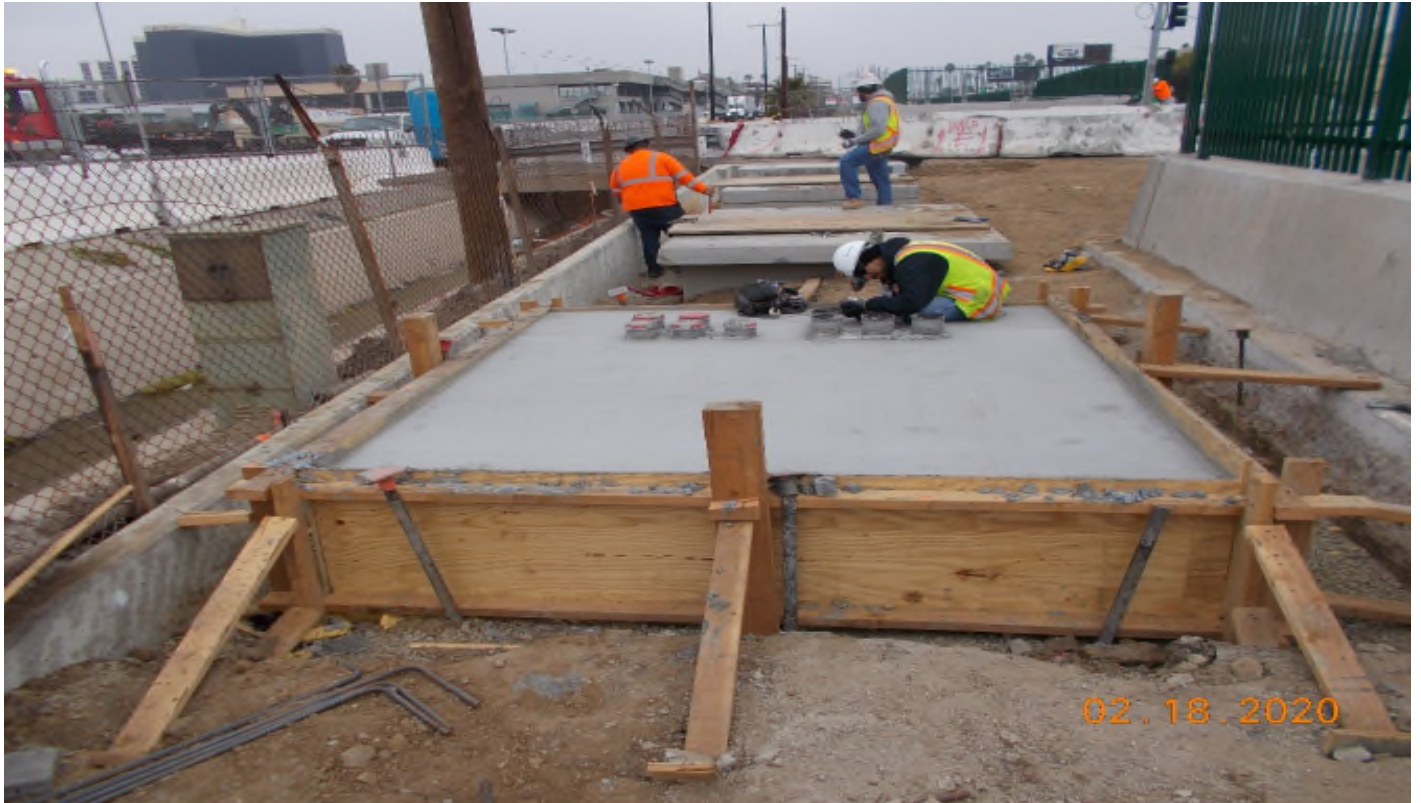
104 th STREET – The DWP meter section was poured.
