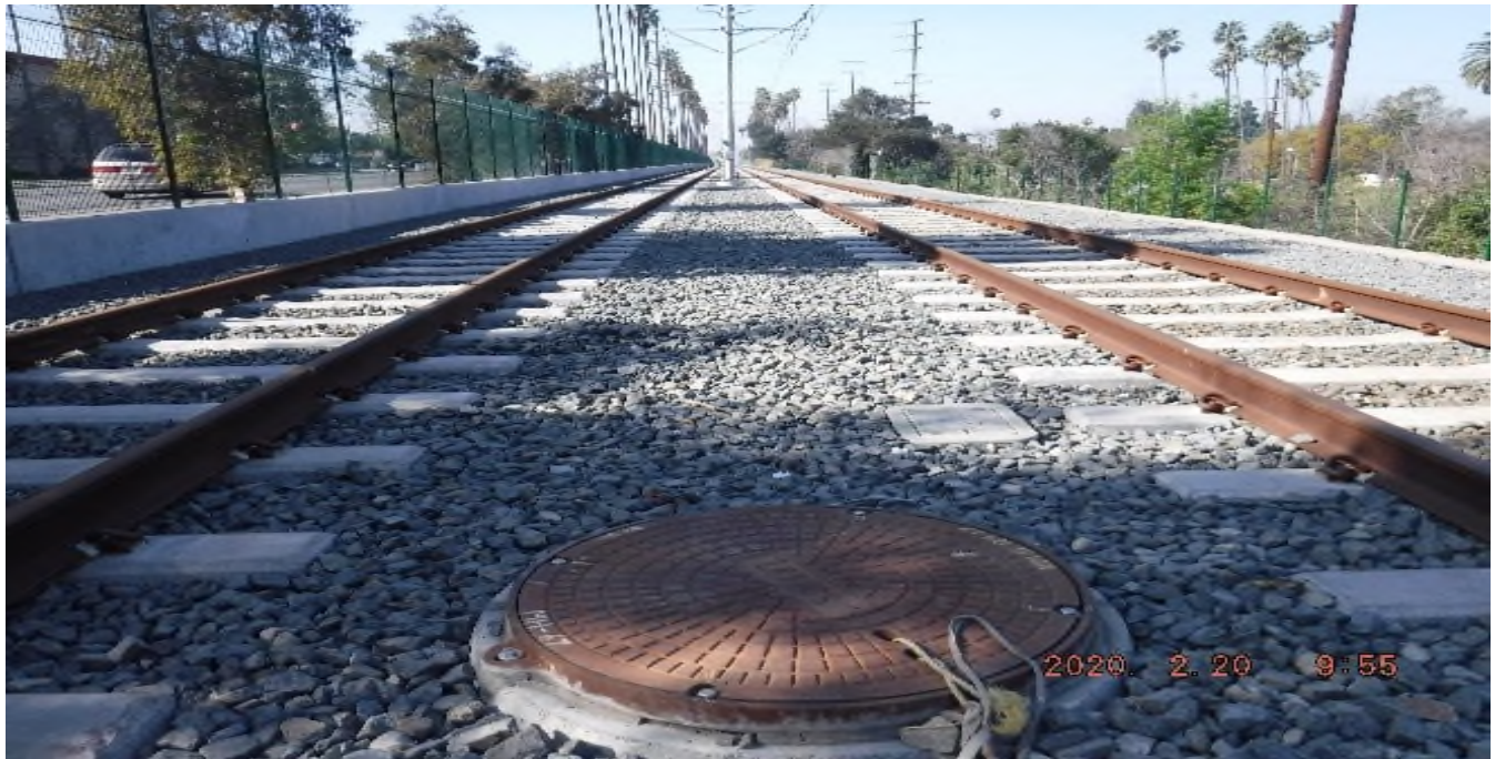
HIGH STREET- STA 241+40 NB looking south – MH#67 rim elevation vs. TOT; no track work (Centinela – High)
