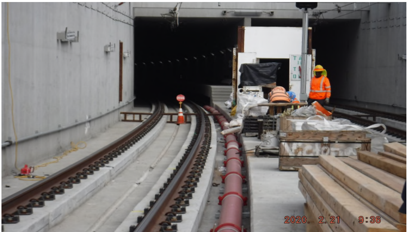
UG4 – STA370+00_ Looking North_ OTM inventory_ UG4 south ramp_48ST
