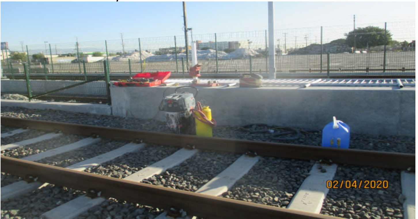
96 th STREET- Drilling handrail post holes at 96th Street Station.
