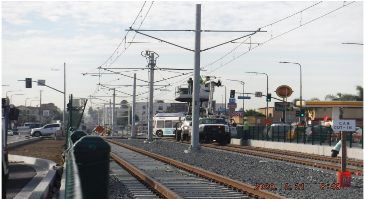
SLAUSON STA – STA262+75_ Looking South_ OCS work_ Slauson-57ST
