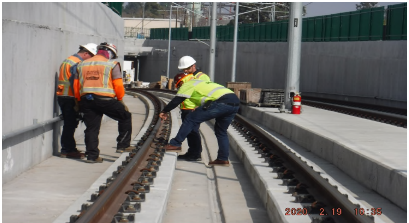
UG4 – STA366+00_ Looking North_ WSCC QC field meeting_ NCR-A-111_UG4_48ST
