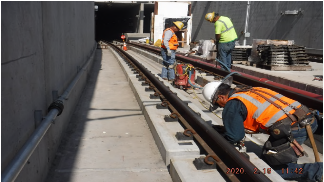
UG4 – STA369+62_ lookN_ Protecting drilled holes_ Drilling RT plinth_ NCR-A-111_UG4_48ST
