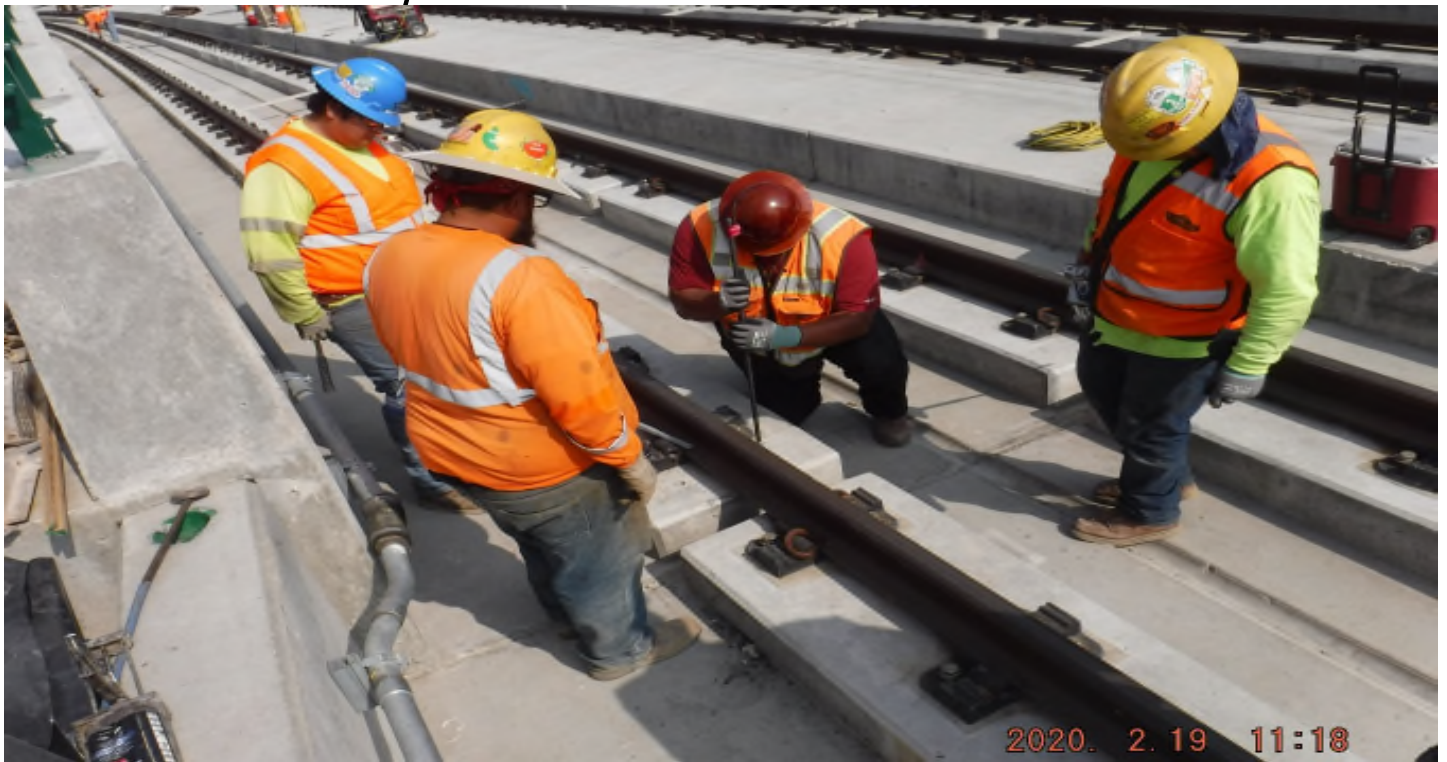
UG4 – STA365+12_ Looking North_ LT plinth dowel epoxy_NCR-A-111_UG4_48ST
