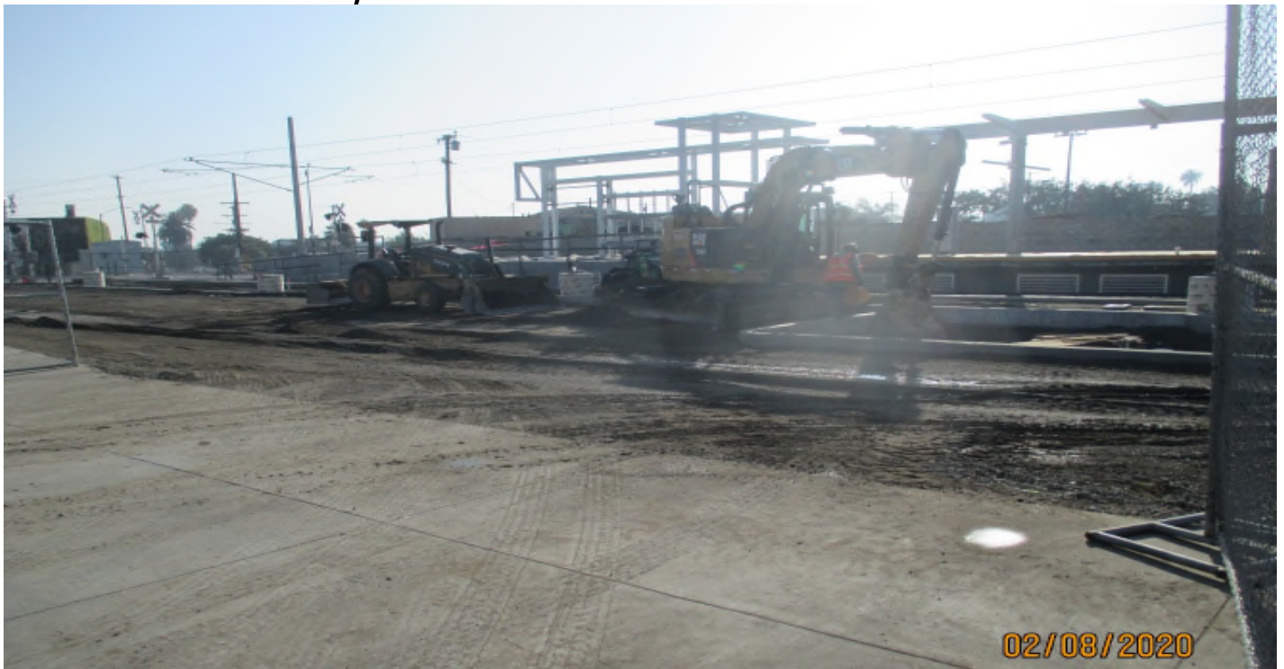
WEST STATION- Base grading for the West Station park & ride.
