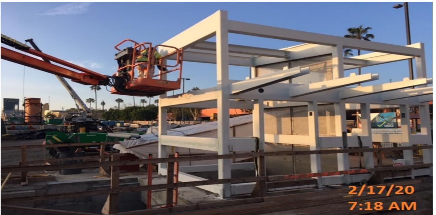
MLK STATION – Continued painting Elevator structures 1&2 at the plaza level.
