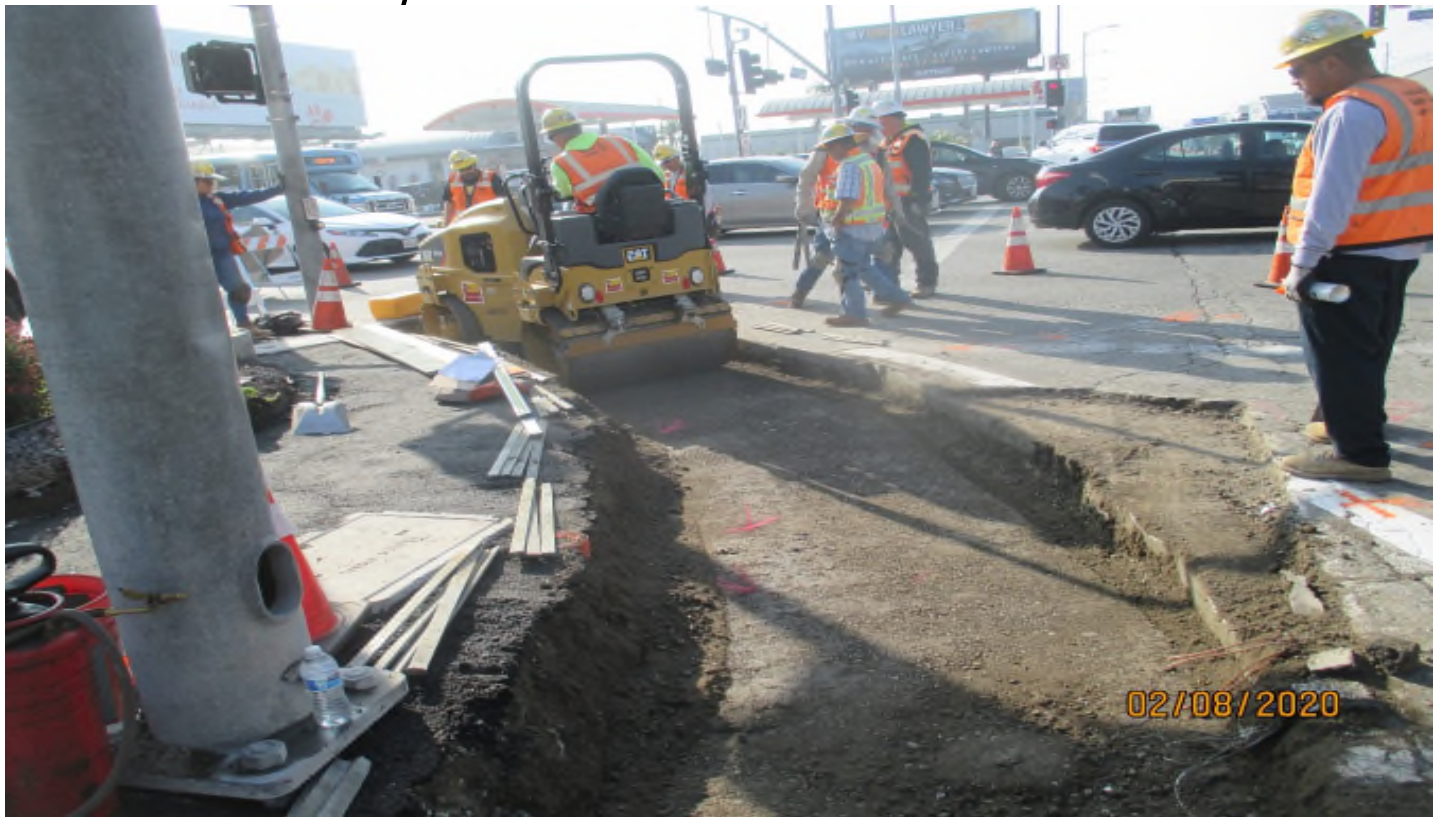
AVIATION/CENTURY- Subgrade compaction for the curb & gutter on Aviation & Century.
