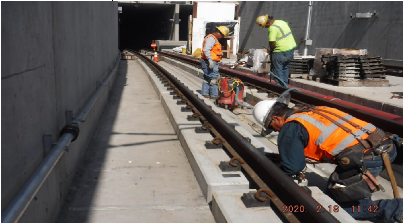
UG4 – STA369+62_ lookN_ Protecting drilled holes_ Drilling RT plinth_ NCR-A-111_UG4_48ST
