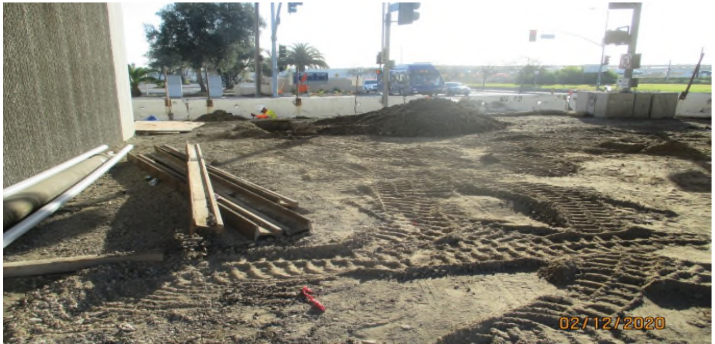
111 STREET – Electrical trench excavation at 111th Street.
