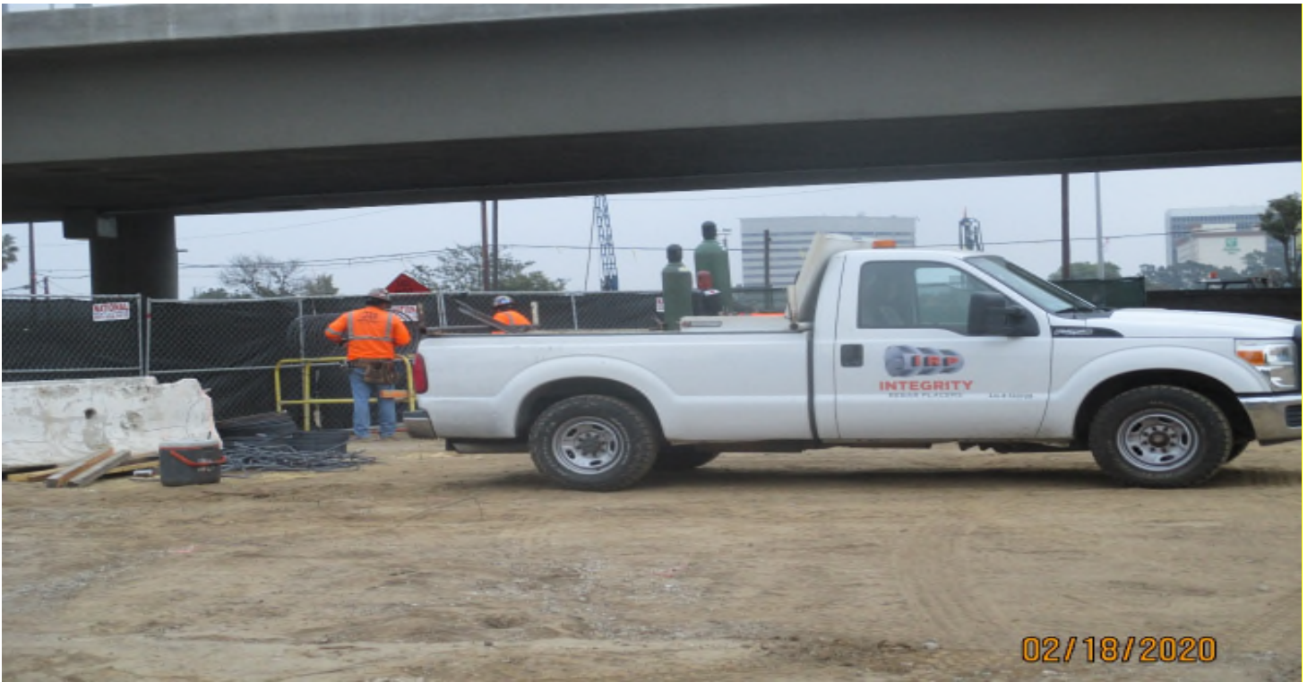
AVIATION/CENTURY- Integrity is building rebar cages at the Aviation Station.
