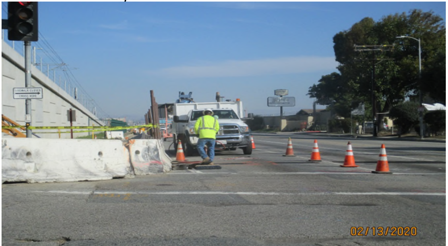
111 STREET – Signal conduit installation on Aviation at 111th.
