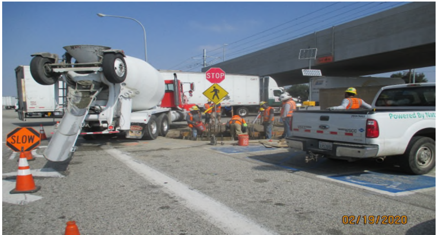
111 STREET – Placing concrete for the new curb and gutter on 111th.
