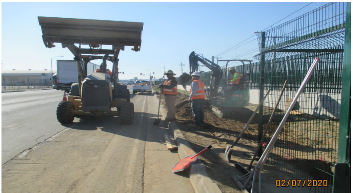
UG 1- Drainage swale grading at UG-1.
