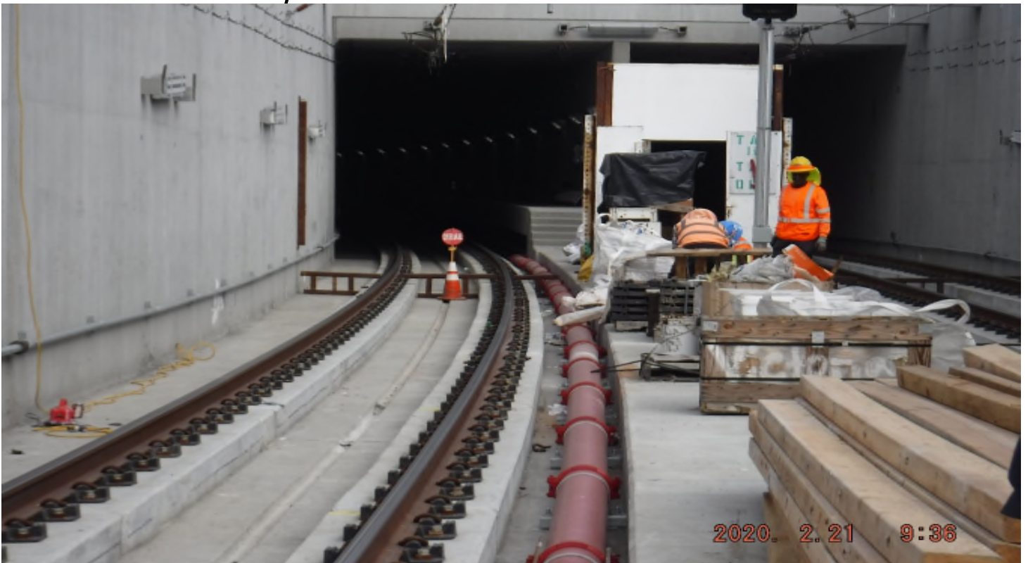
UG4 – STA370+00_ Looking North_ OTM inventory_ UG4 south ramp_48ST
