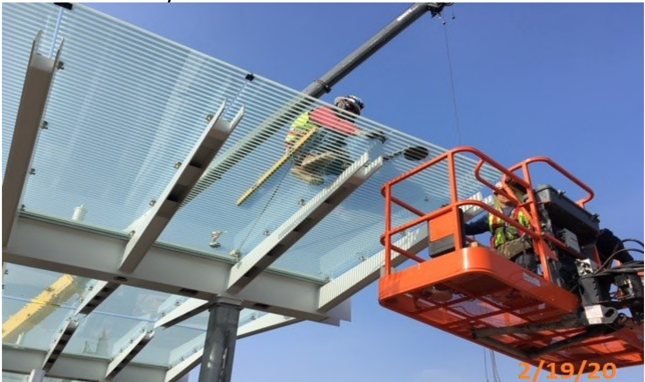
VERNON STA – Giroux Glass aligning canopy glass
