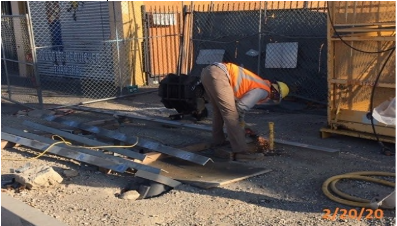
VERNON STA –Ironworkers fabricating trim edge.
