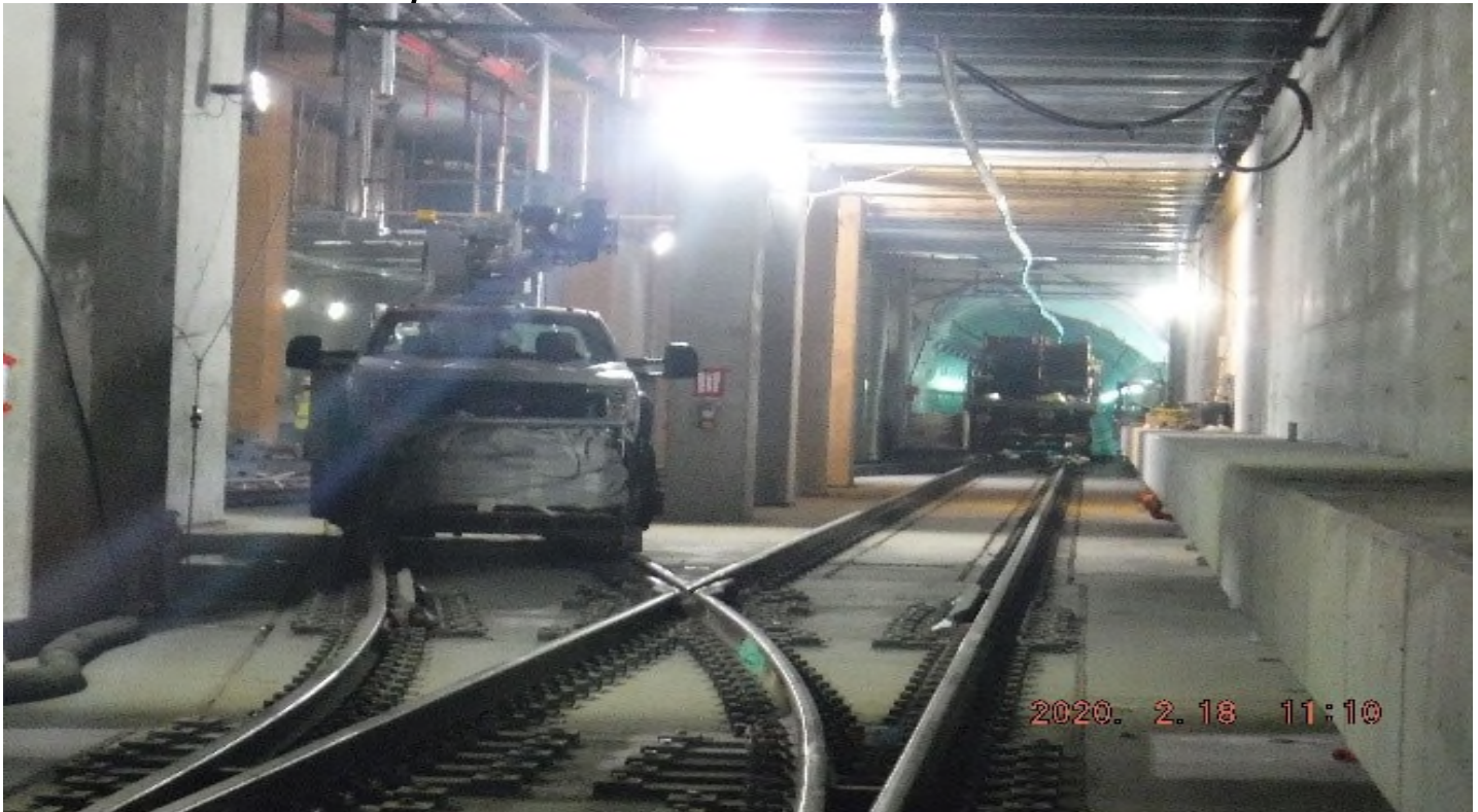
EXPO STATION- STA 444+50 TK#3 SB looking south – OCS work XING 5 – UG4.
