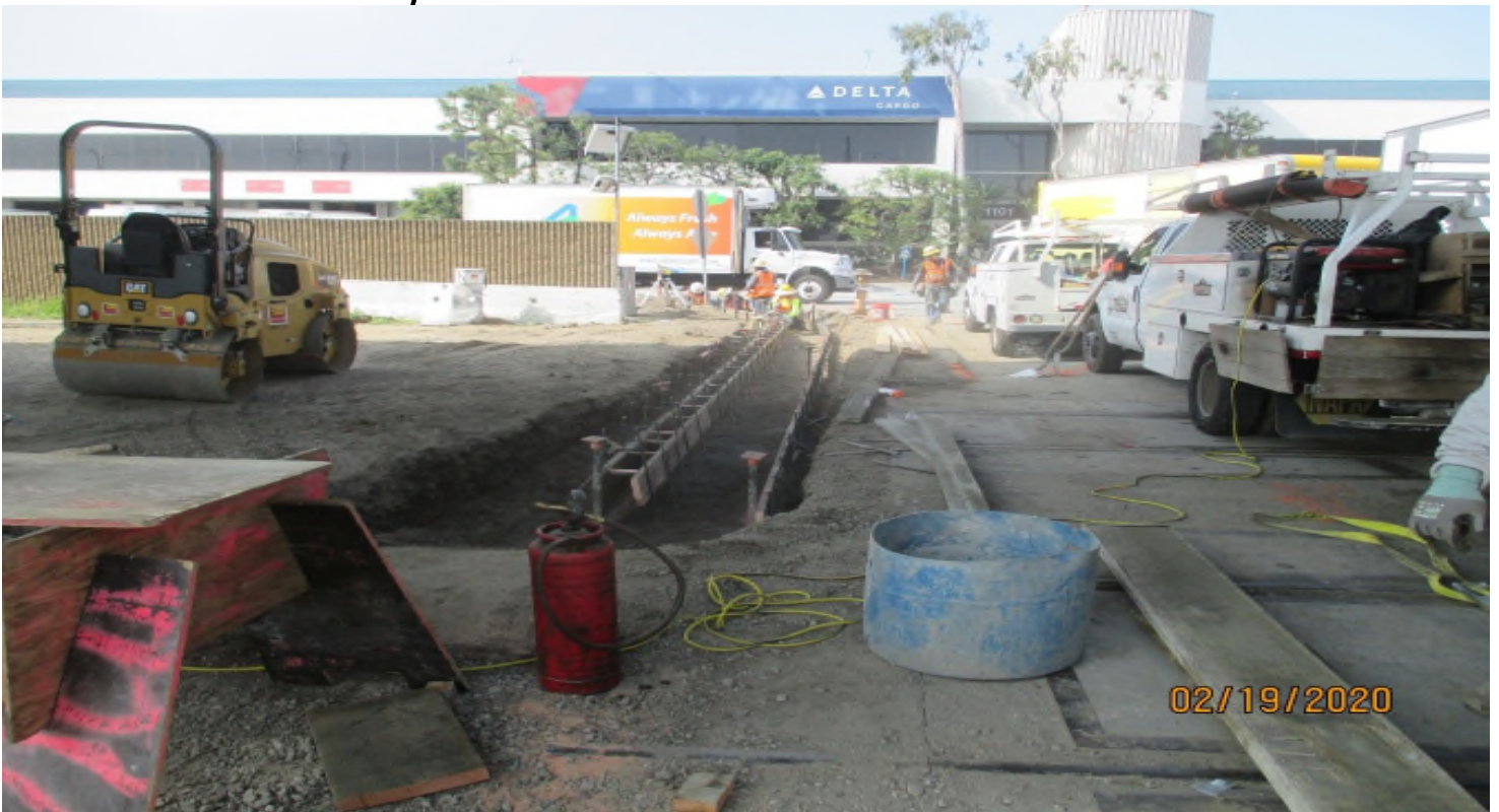
111 STREET – Forming the curb & gutter on 111th street. Facing west.
