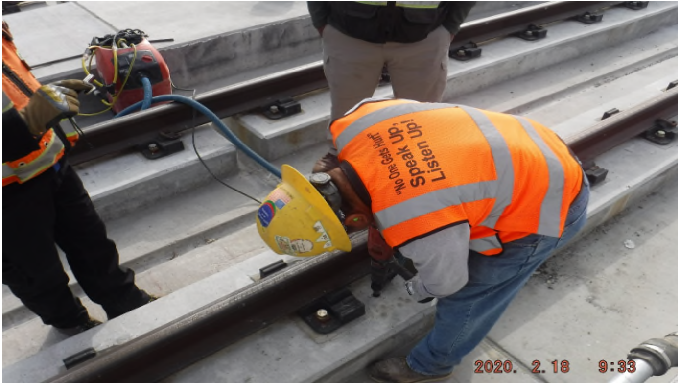
UG4 – STA365+12_ Looking East_ LT plinth drilling_ NCR-A-111_UG4_48ST
