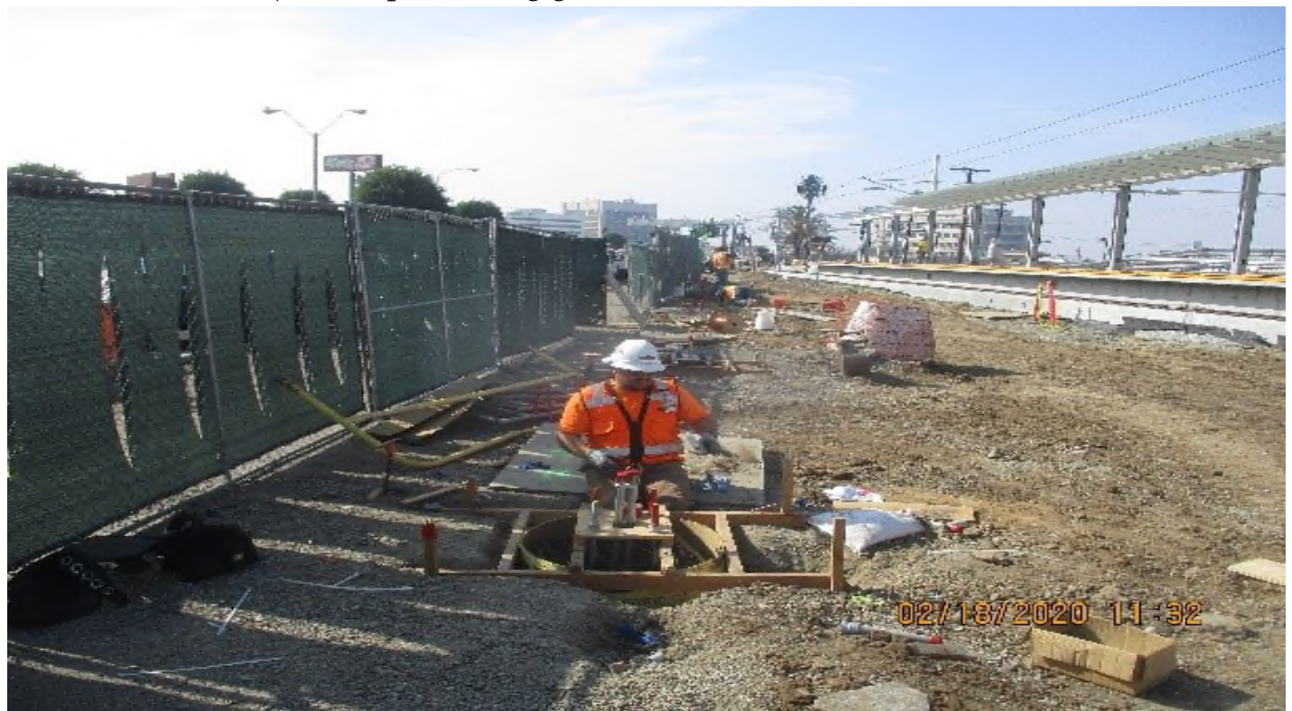
LA BREA – WSCC Preparing light foundations at La Brea.
