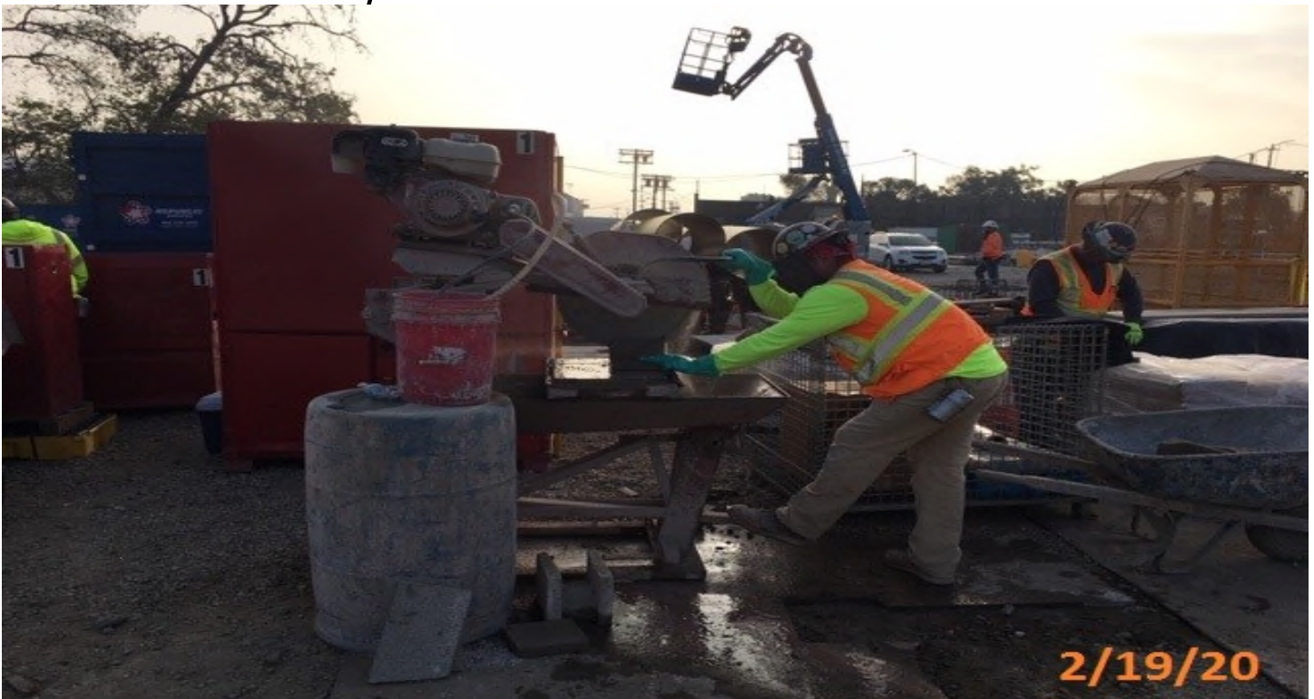
EXPO STATION- Masonry Concepts making cuts to cinder.
