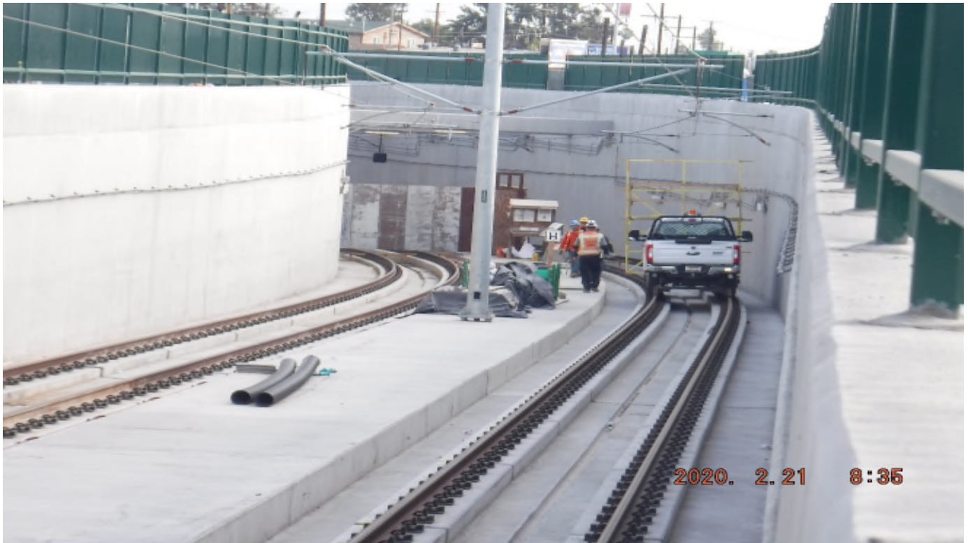
UG3 – STA277+50_ Looking North_ Check VDC clearance_ UG3_ Victoria
