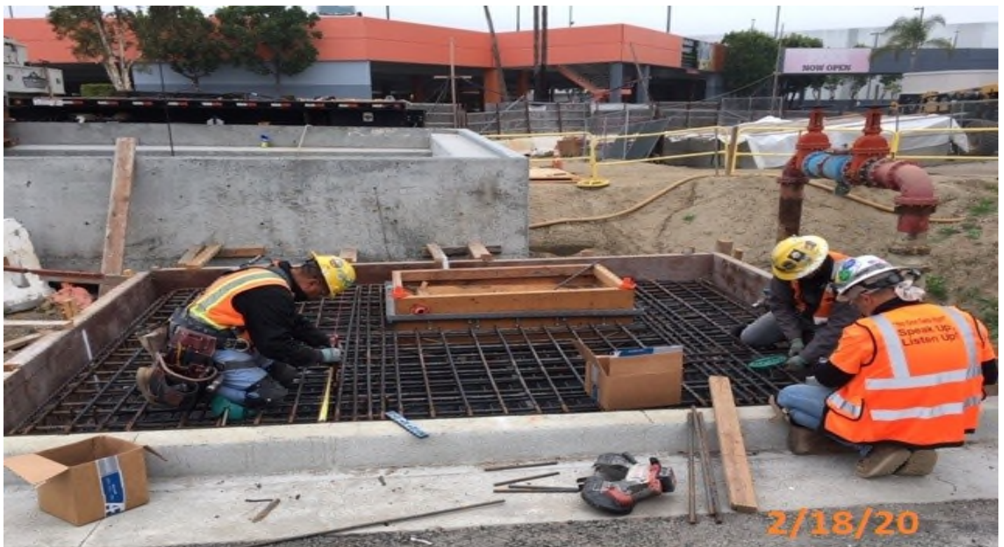
MLK STATION – WSSC installing anchors for concrete valve pit top slab.
