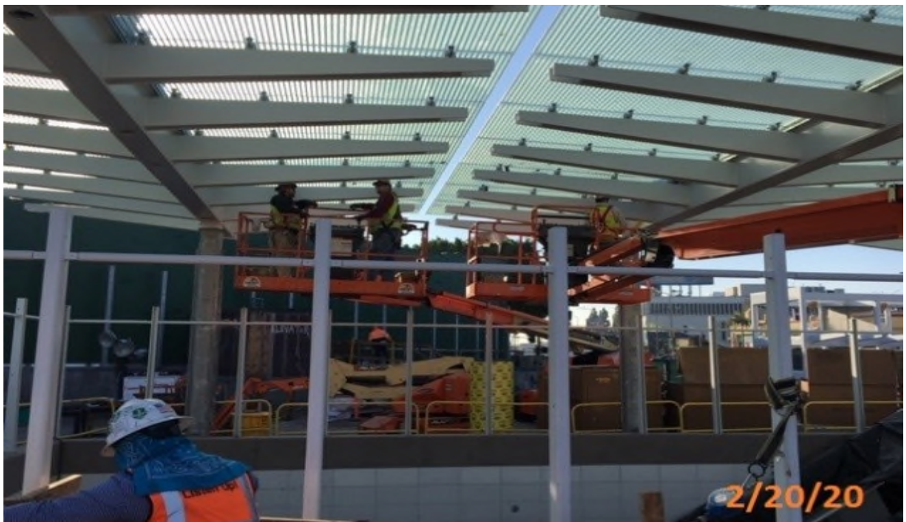
VERNON STA – Giroux Glass aligning and spacing canopy glass panels.
