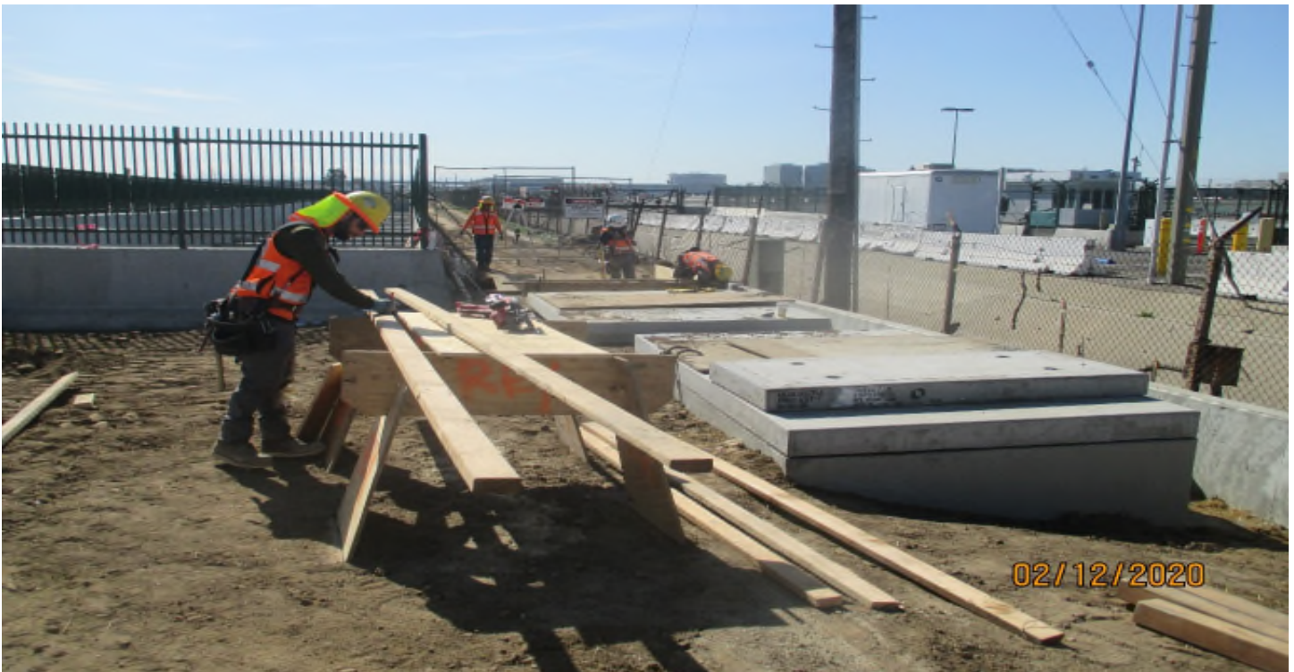
104 th STREET – Forming the DWP meter pad at 104th Street.
