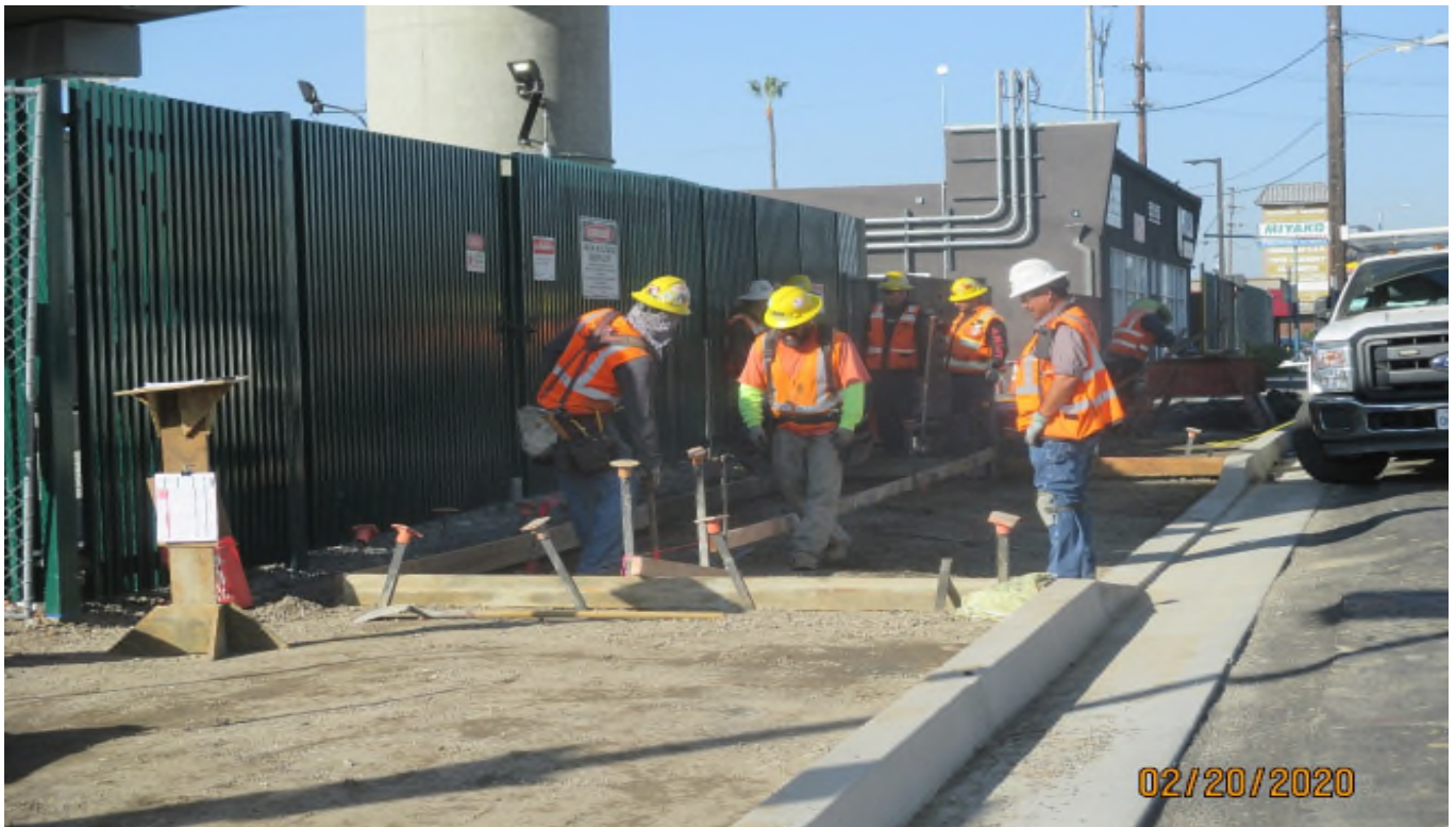
MANCHESTER AVE- Forming the TPSS #3 drive approach on Manchester.
