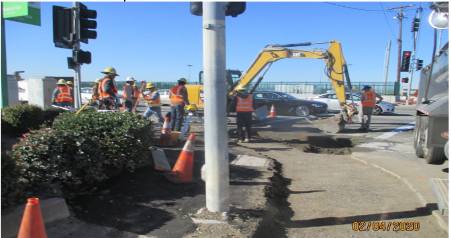
111 STREET – Curb & gutter subgrade compaction at 111th street.
