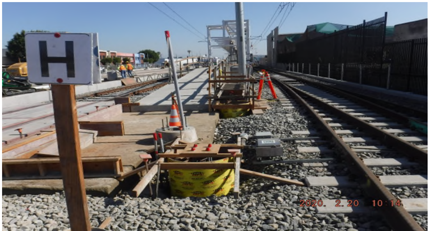
WEST STATION- STA262+75_ lookN_ Status landing pad & light pole foundations_PUNCH LIST
