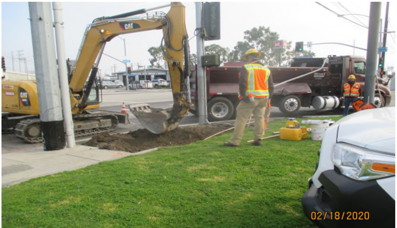
MANCHESTER AVE- Sidewalk subgrade grading at Aviation and Manchester.
