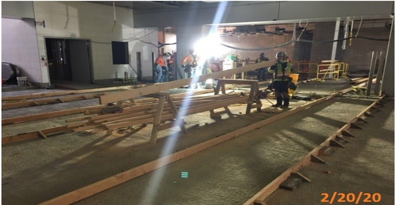
MLK STATION – Dean Visosky at concourse building formwork .
