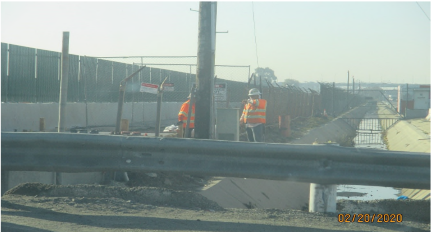
UG 1- Chain link fence repair at 104th street. Facing south.
