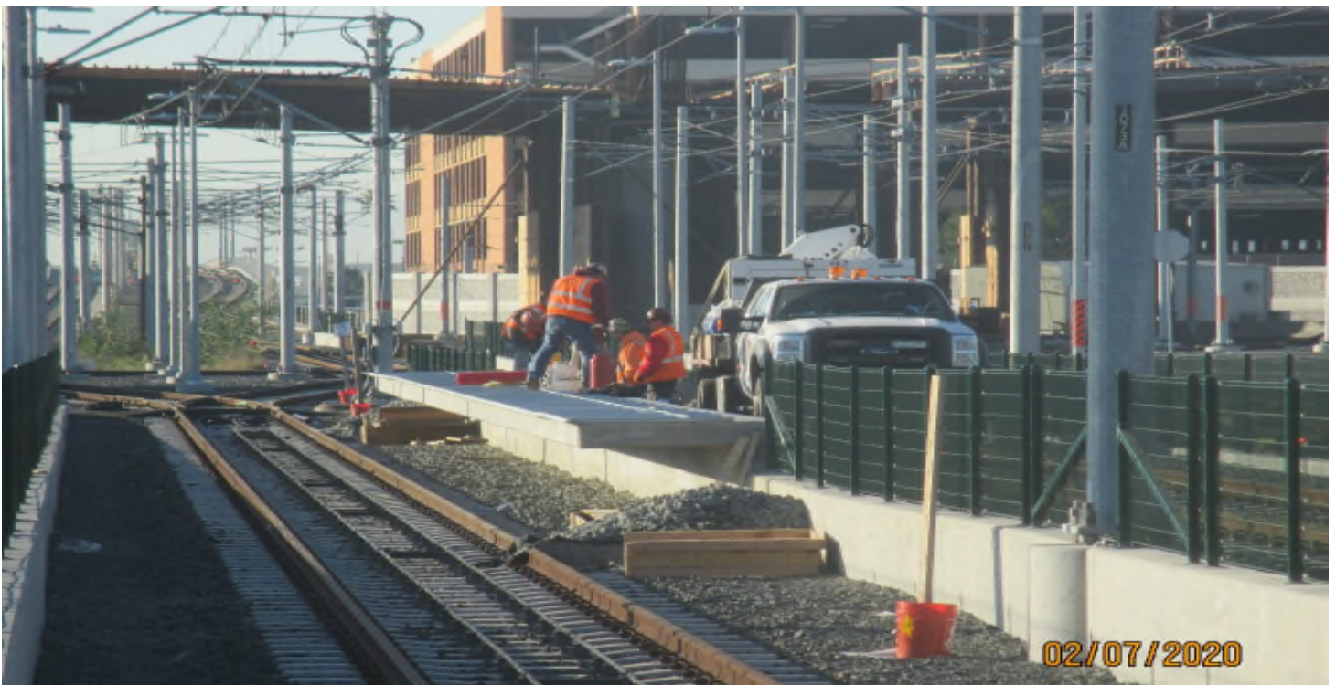
96 th STREET- 96th Street Station operator's platform handrail installation.
