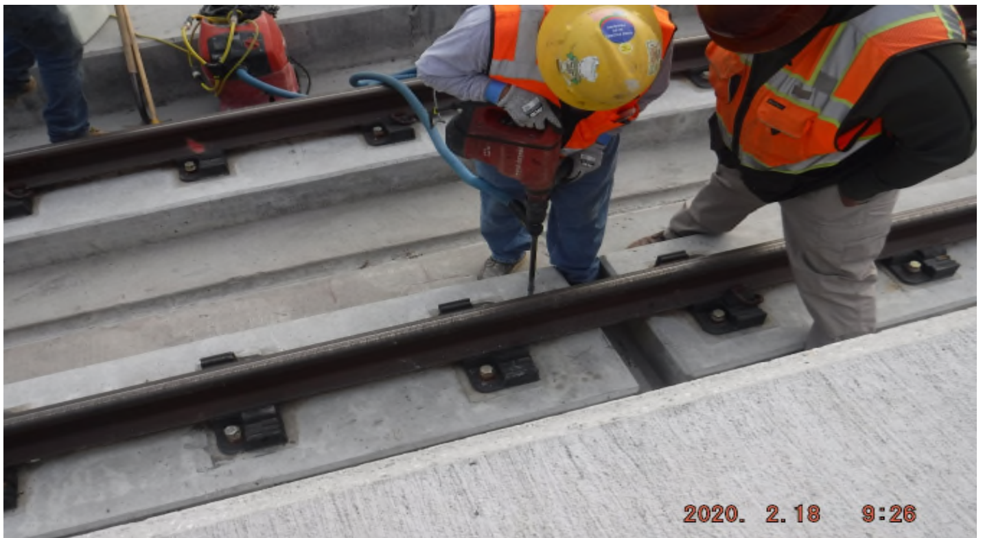
UG4 – STA365+12_ Looking East_ LT plinth drilling_ NCR-A-111_UG4_48ST
