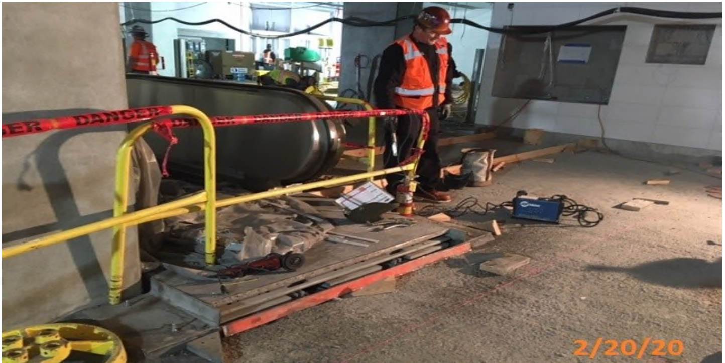
MLK STATION – WSSC Ironworkers aligning bent plate .
