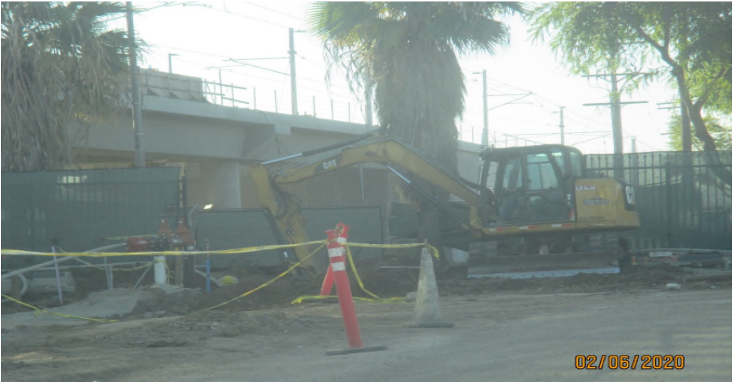
AVIATION/CENTURY- Fire line excavation at the Aviation Station.
