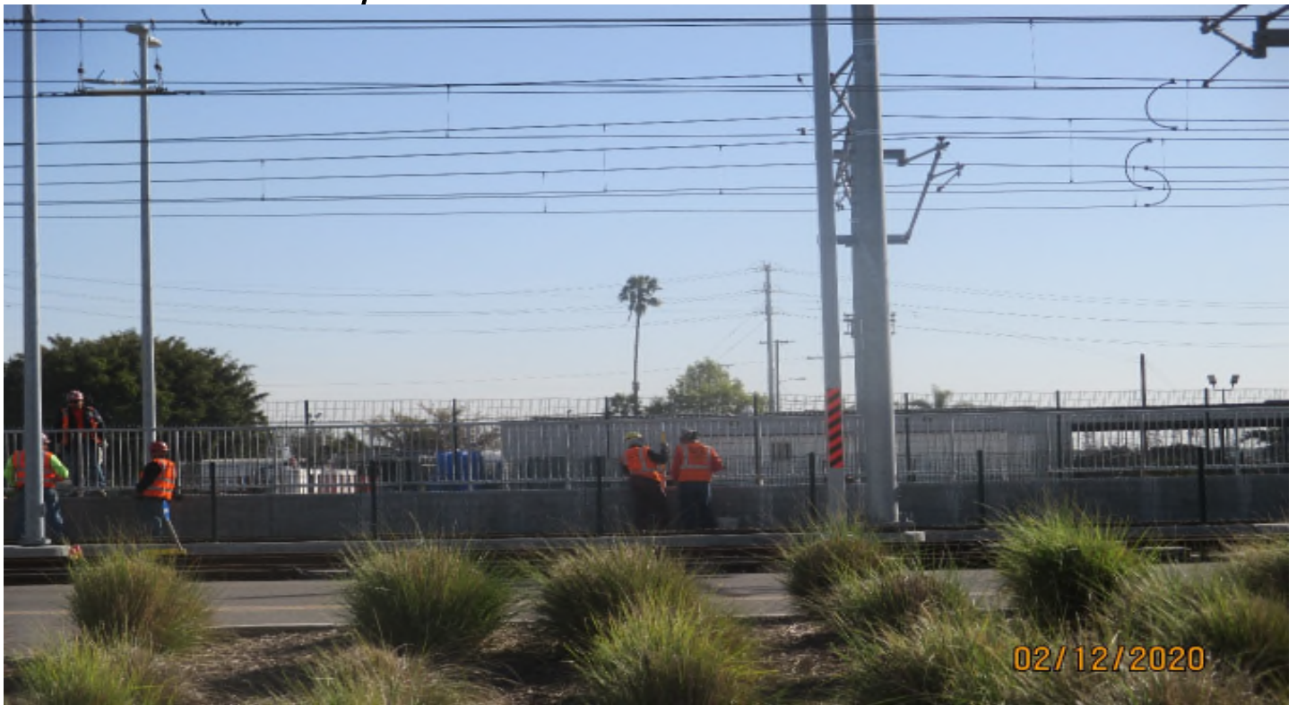
96 th STREET- Grouting the handrails at the 96th Street Station.
