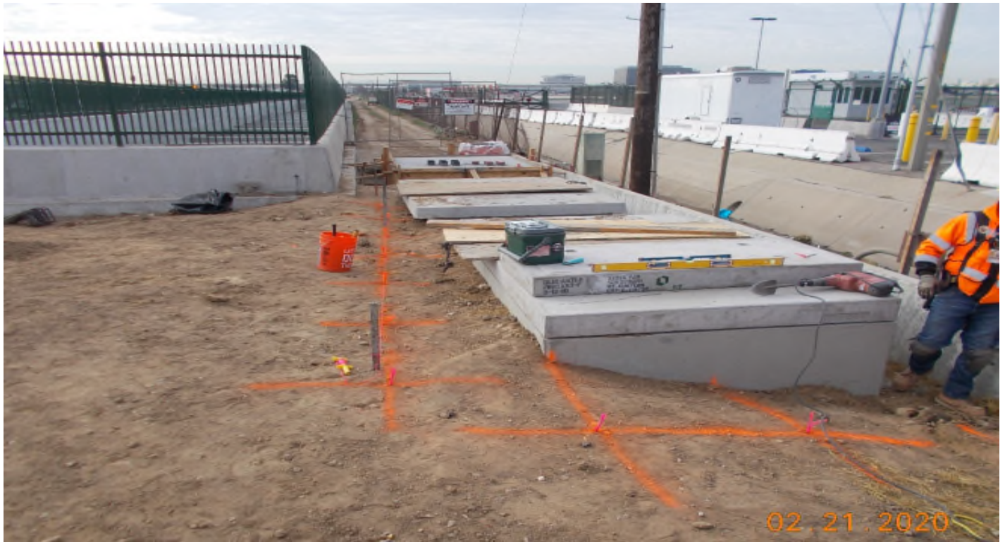
104th STREET – WSCC was digging to install bollards around utilities.
