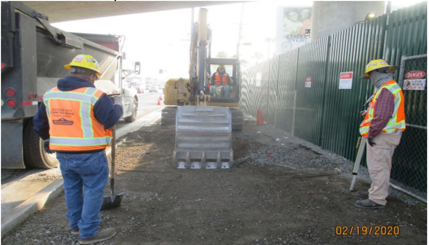
MANCHESTER AVE- Cutting sidewalk subgrade on Manchester.
