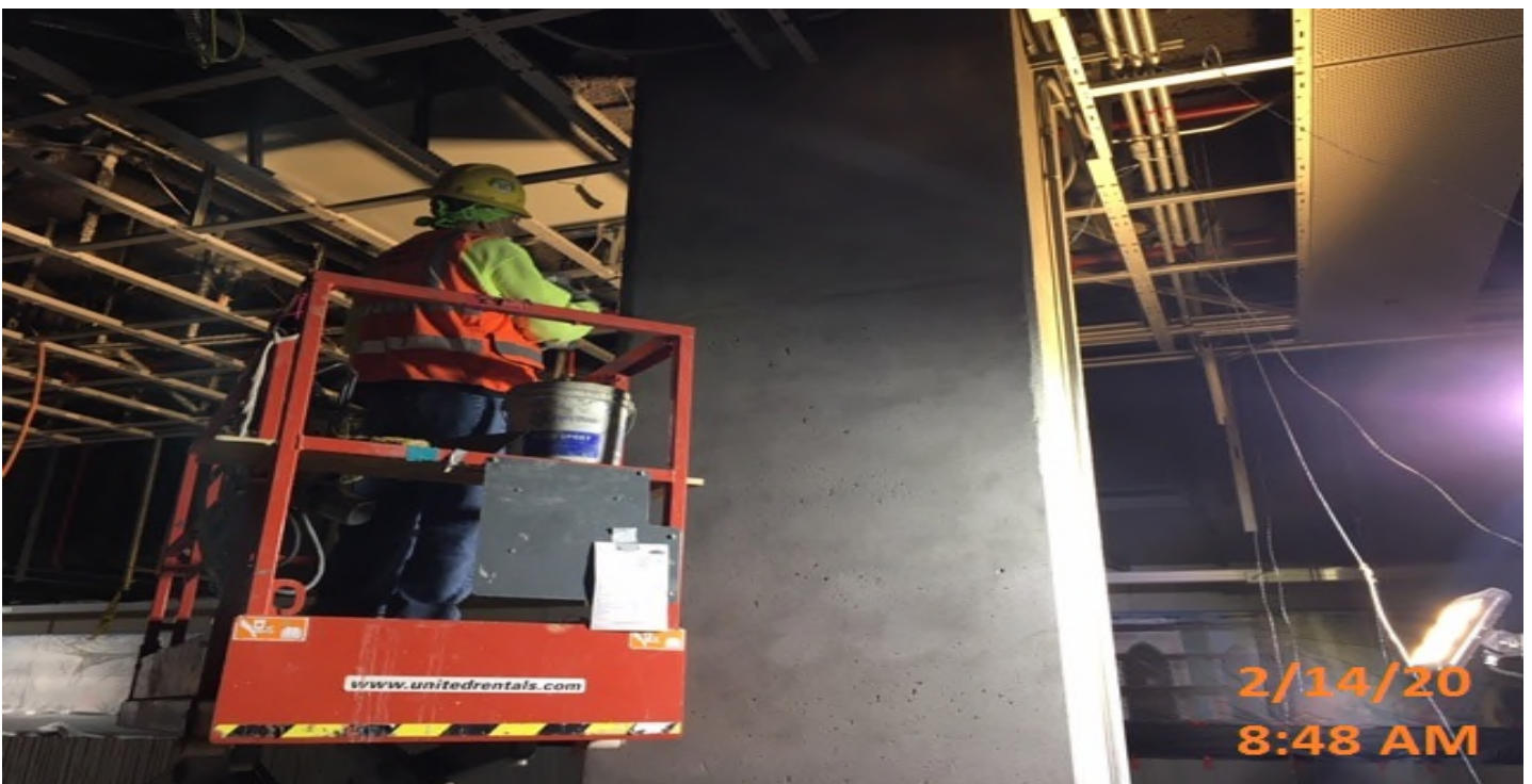
EXPO STATION – Grinding and smoothing columns at the platform level.
