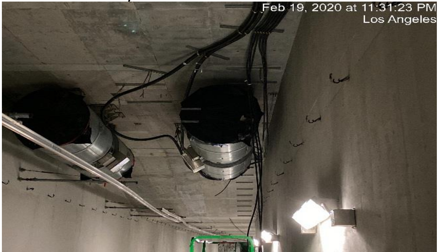
UG4 – Continue wiring and running cable for the booster fans in the northbound tunnel at Sta 374+25.
