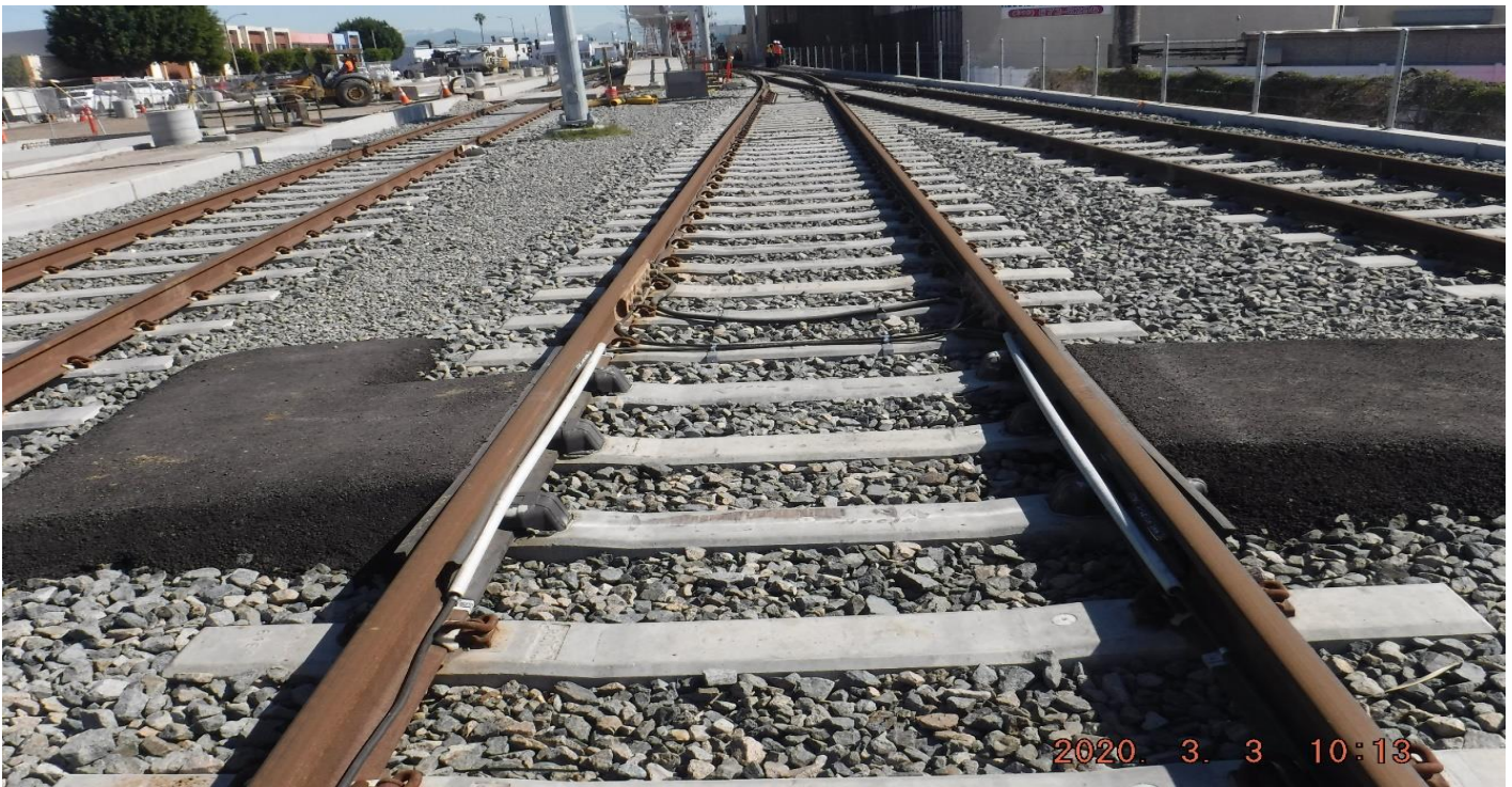
WEST Blvd- STA261+63_ Looking North_ AC Xwalk placing pending_ West.
