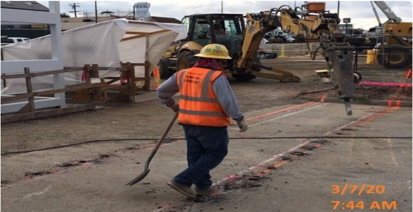
MLK STATION - Excavating/demolishing for planter wall footings at the plaza level.
