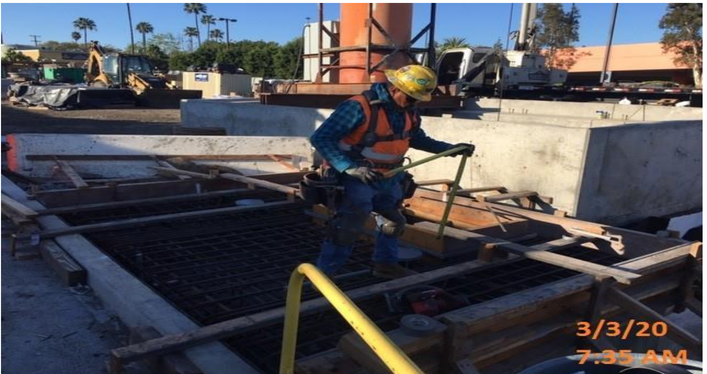
MLK STATION – WSCC crew setting rod embeds for concrete slab.
