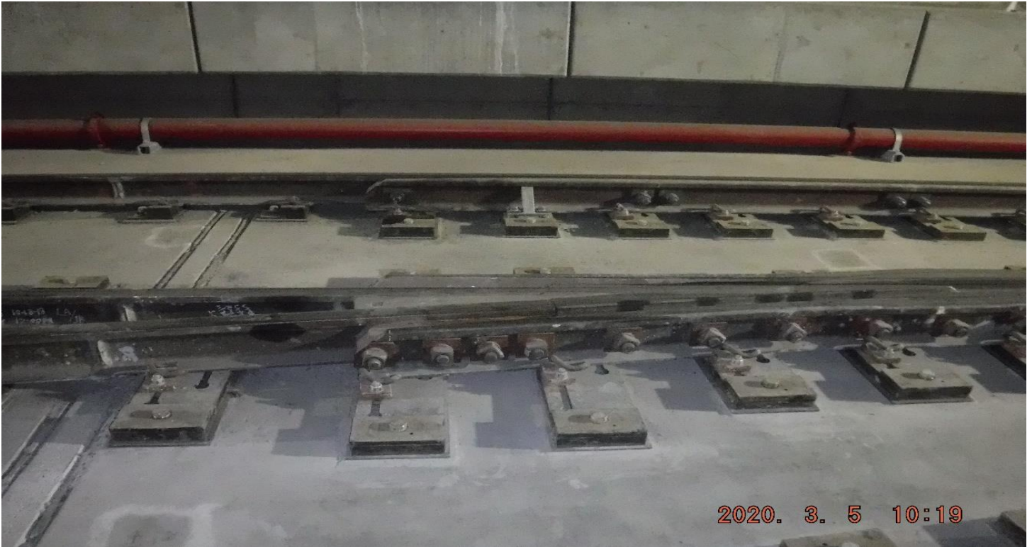
UG4 – STA443+70_TK3_ Looking West_ Installed guard rail brace_ 8W2_ UG4_ Expo.
