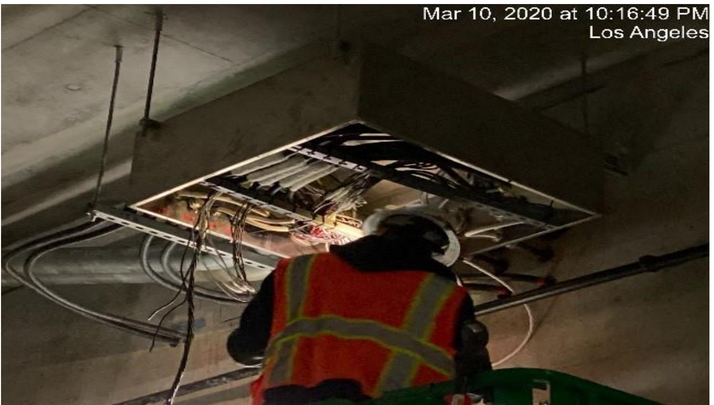
UG3 – DCD splicing wires in junction box southbound UG-3.
