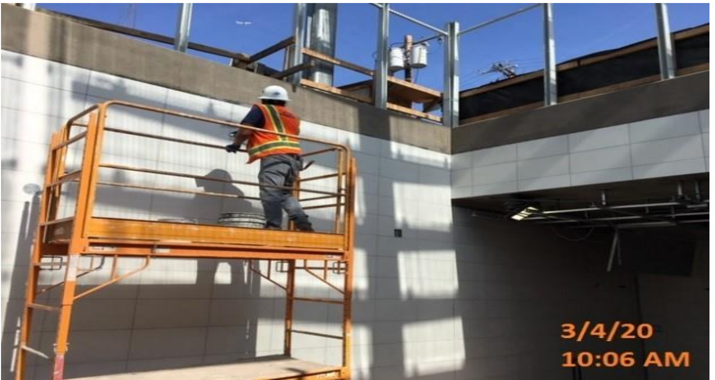
Crenshaw/Vernon – VERNON – Premier Tile & Marble installing misc.
