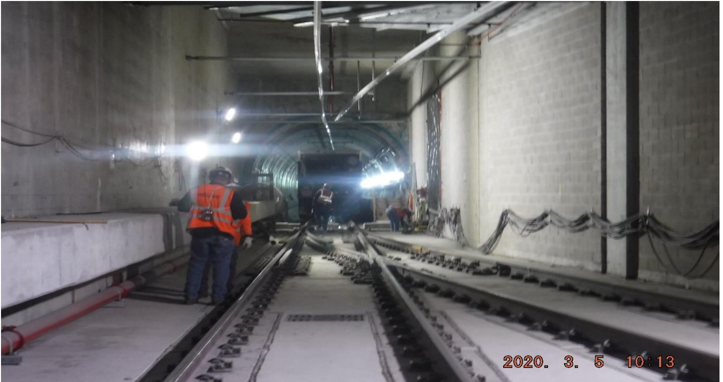
UG4 – STA442+00_ Looking South_ TK geometry adjustment_8W1_ UG4_ Expo.
