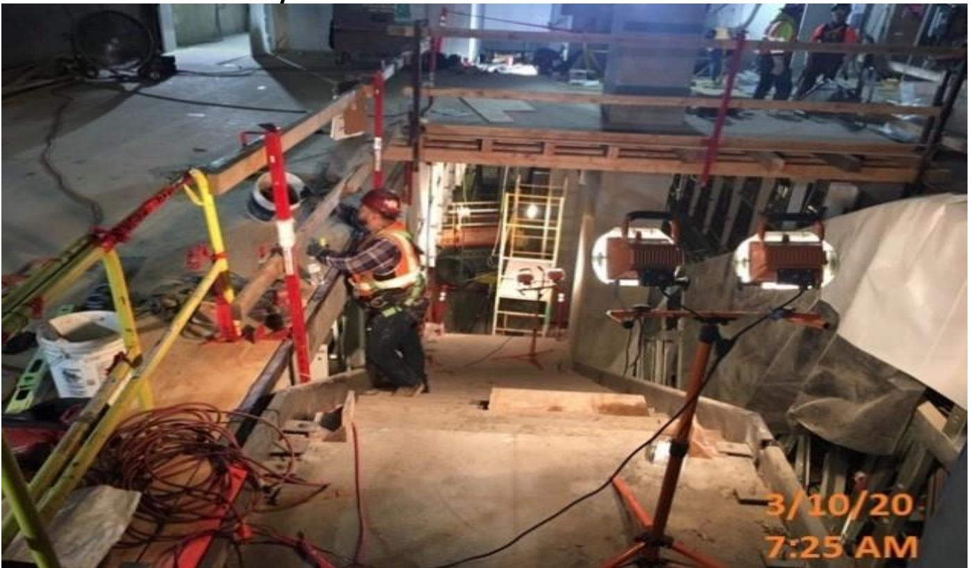
MLK STATION – Carrera Marble laying out granite risers for stair #3.
