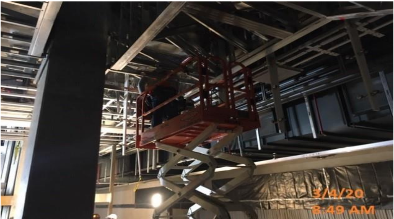
MLK STATION – KHS&S installing steel stud track beneath stairs.
