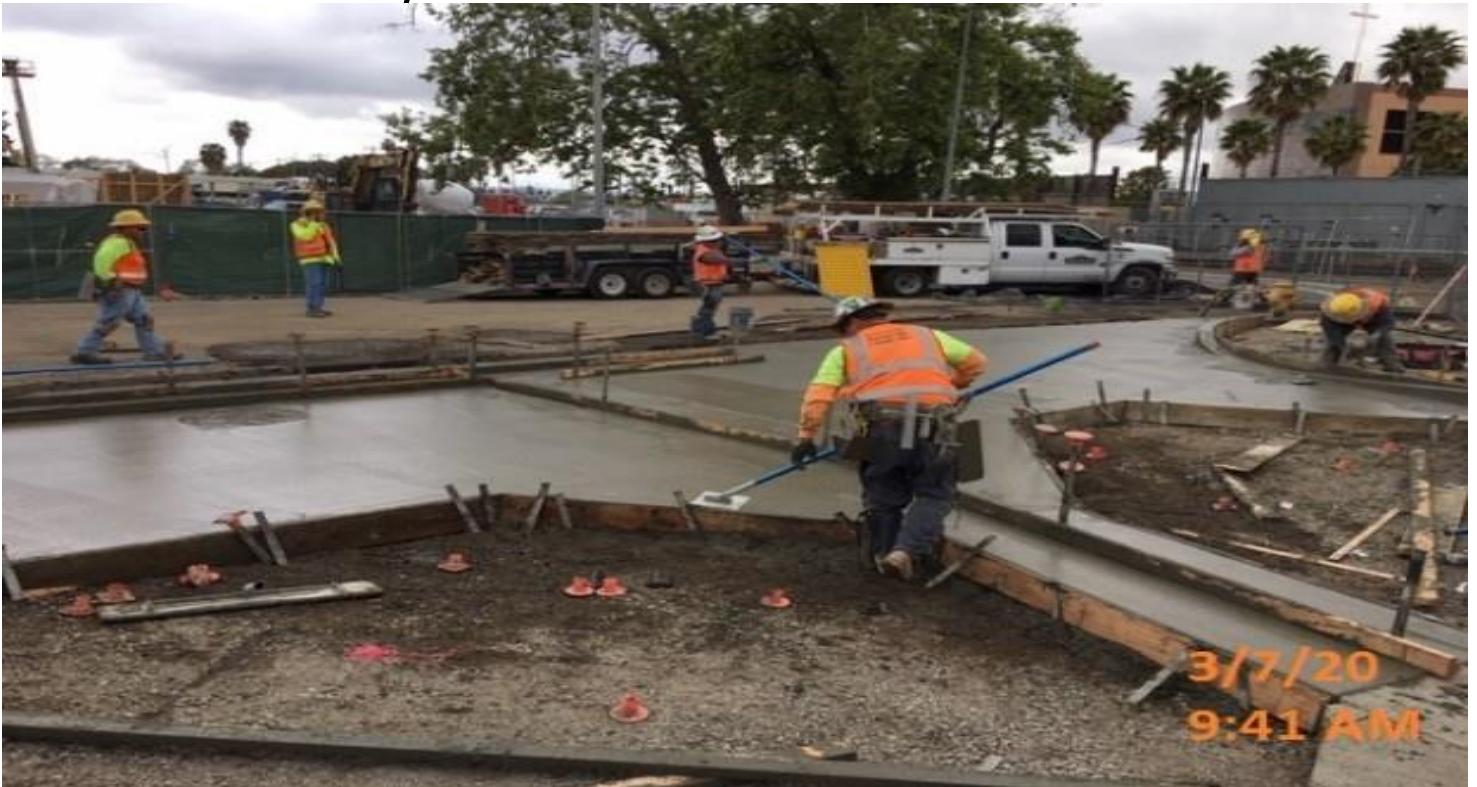
EXPO STATION- EXPO Civil- WSCC placing concrete for cross gutter.
