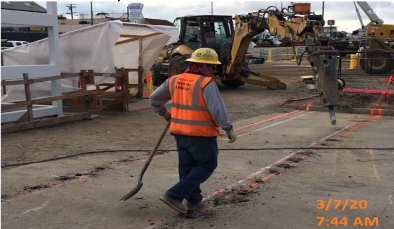
MLK STATION – WSCC crew demoing AC for planter.
