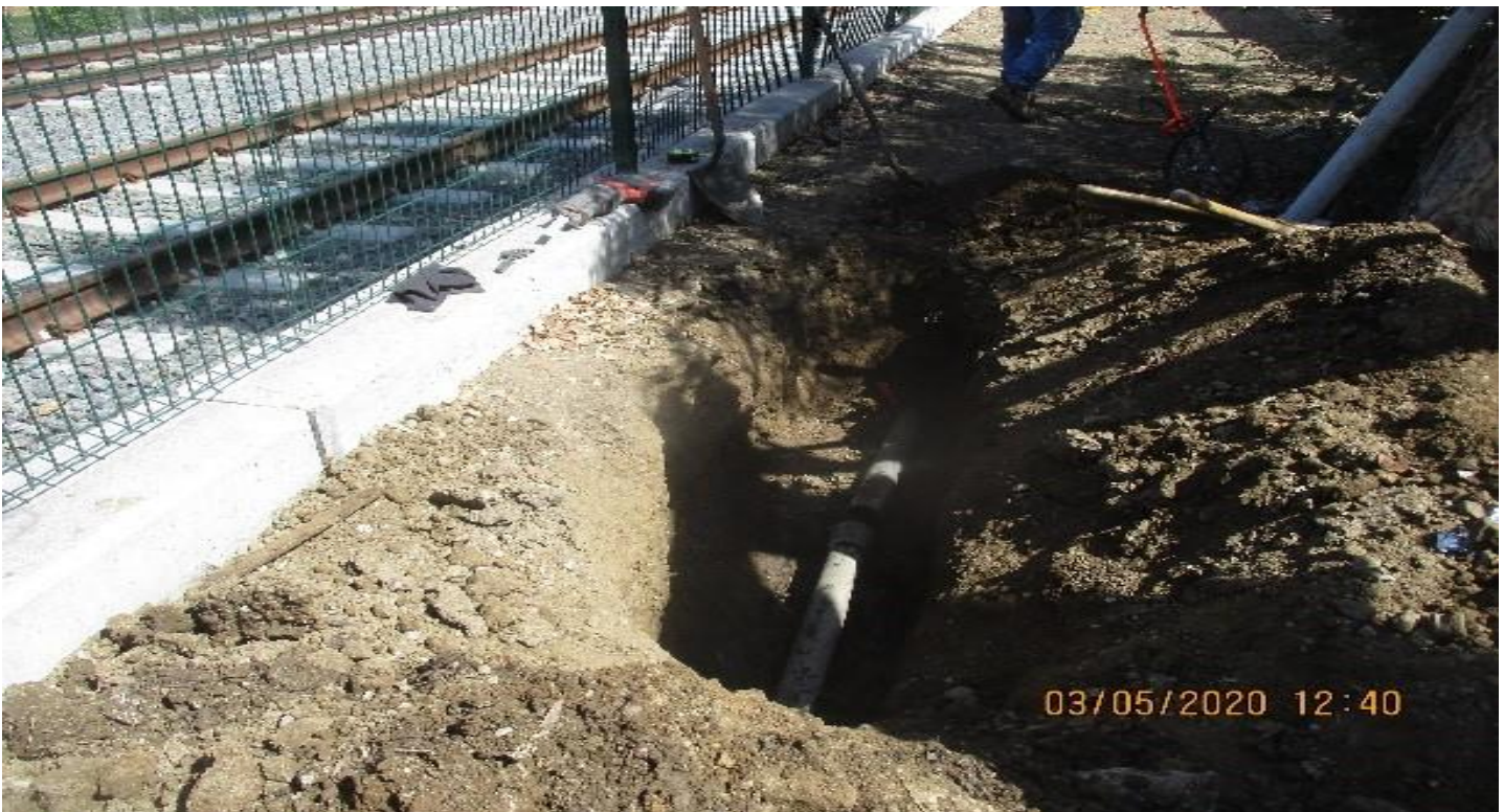
Florence/Ivy - Select Electric Repair damaged conduit between High and Prairie.
