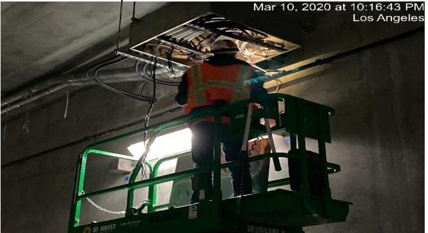
UG3 – DCD splicing wires in junction box southbound UG-3.
