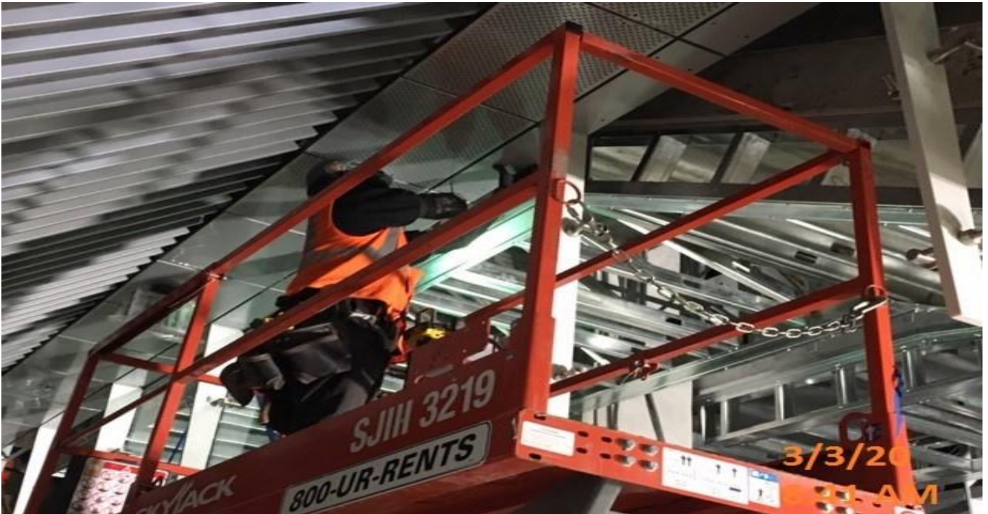
Crenshaw/Vernon – VERNON – PCI swapping out bolts on down stand.
