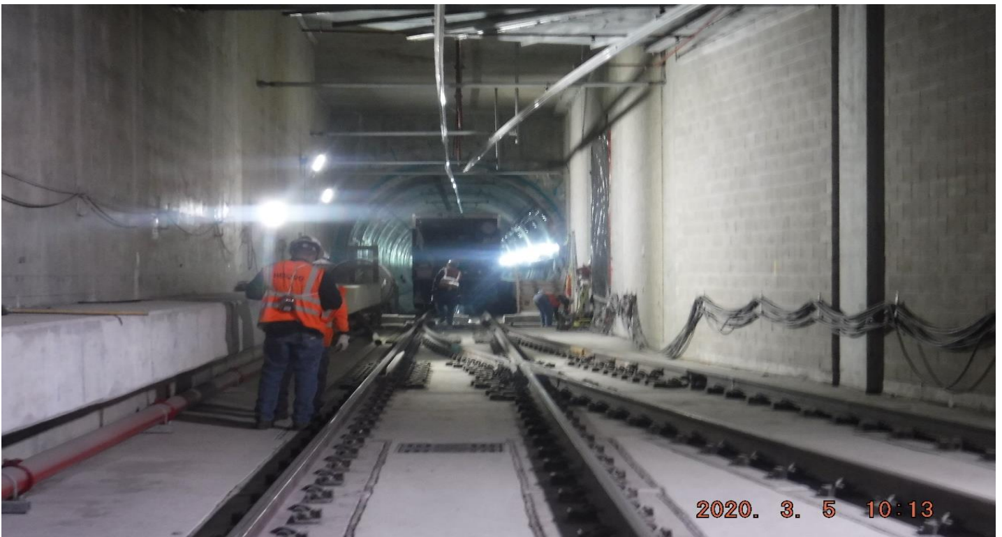
UG-4- STA442+00_ Looking South_ TK geometry adjustment_8W1_ UG4_ Expo
