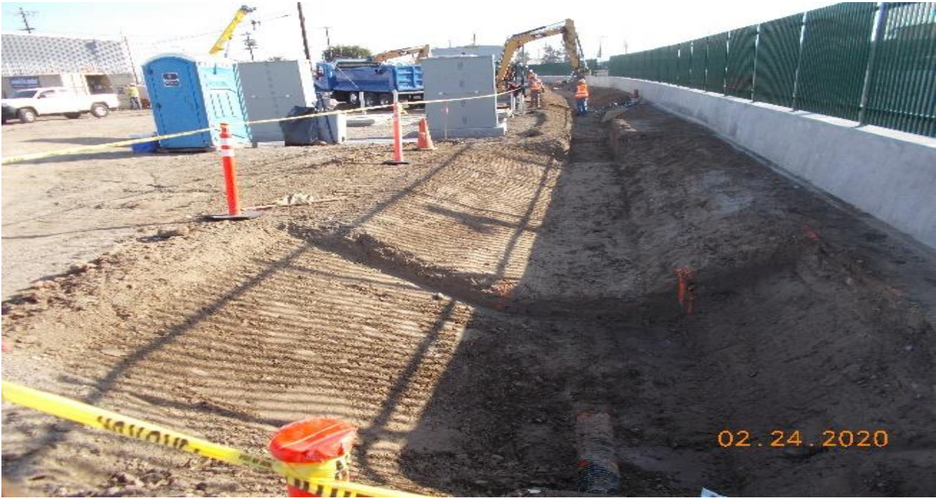
UG3 – Continue excavation for culvert drainage along the southbound barrier wall from Sta 279+20 – 282+93.
