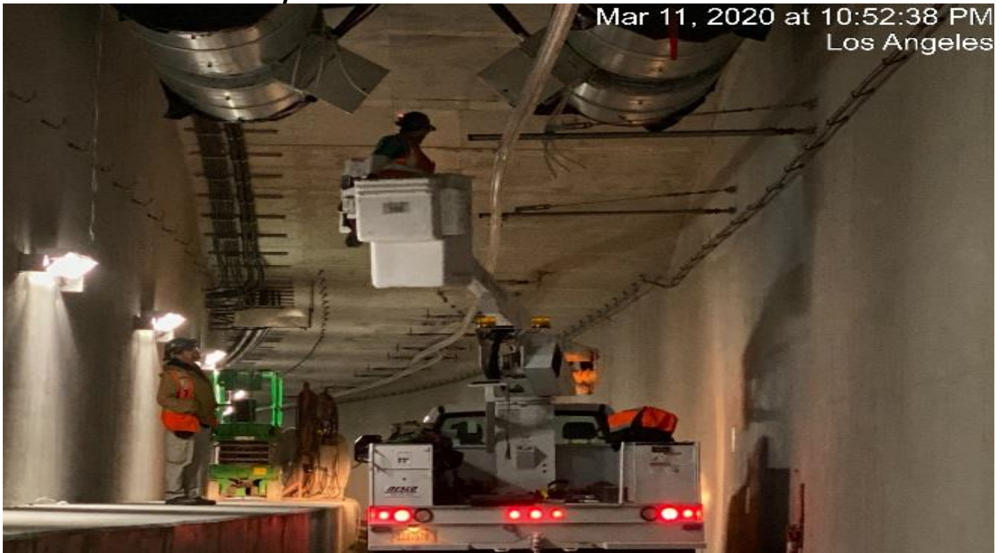
UG-4- – Continue wiring and running cable for the booster fans in the northbound tunnel at Sta 378+75.
