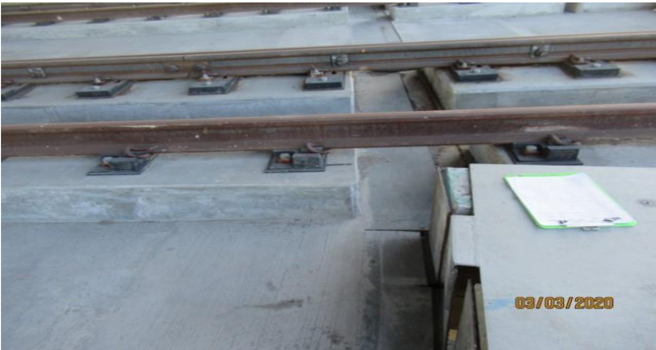
GUIDEWAY - Taper gauge under fastener plate east leg of wye.
