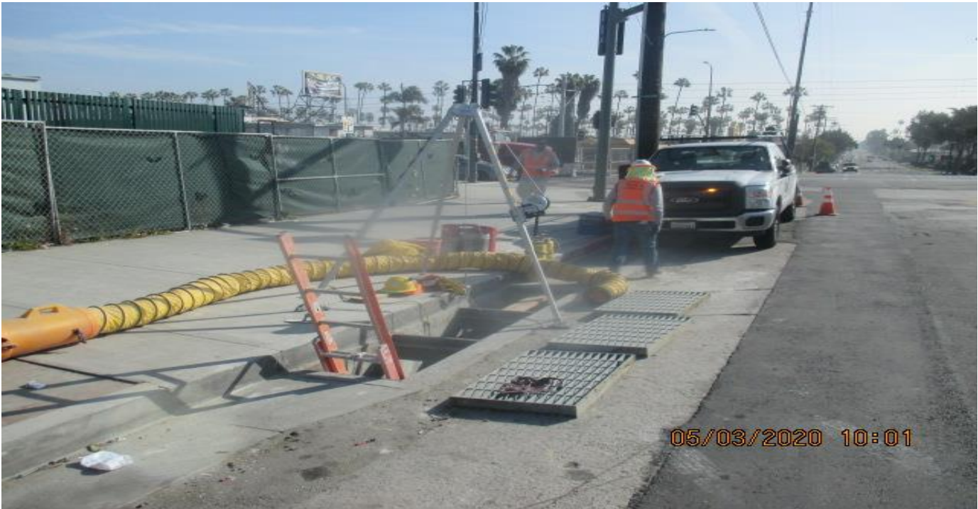
Park Mesa – Continued sack and patch of Catch Basin #37 on the northwest corner of 48th St and Crenshaw Blvd. 3/5/20
