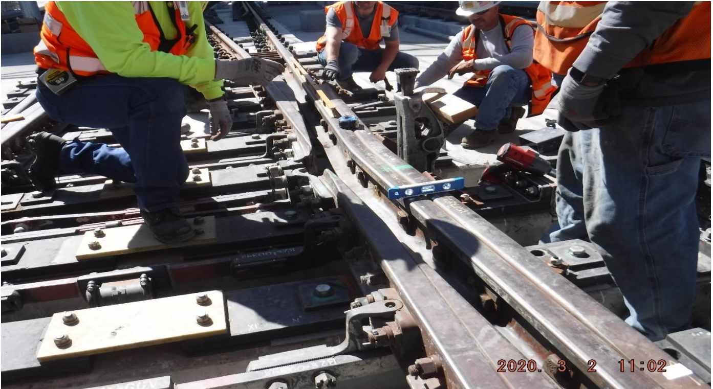
Imperial Hwy - STA14+00_ Looking South_ XING3_ Set components_ Imperial
