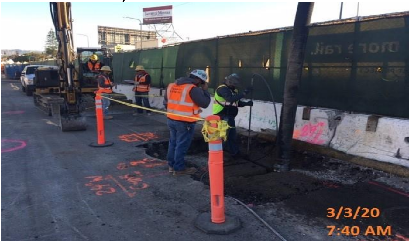
MLK STATION – WSCC crew and Norcal potholing in new area.
