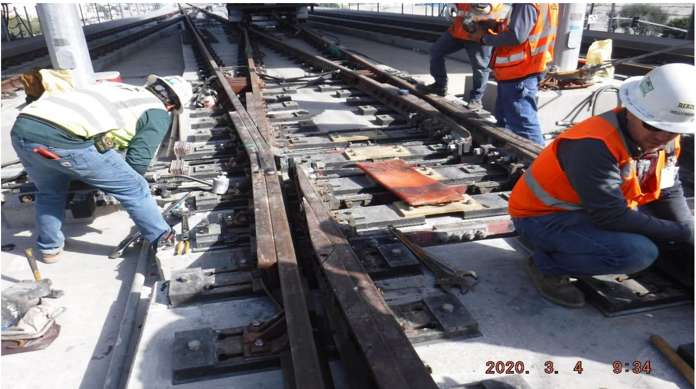
Imperial Hwy - STA14+00_ Looking North_ XING3_ Set-up switch rods_ Imperial.
