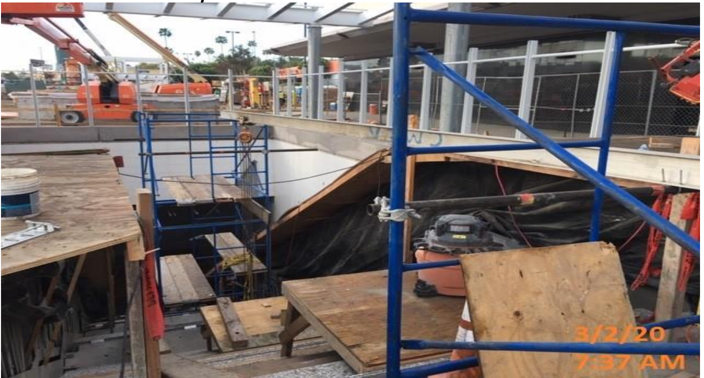
Crenshaw/Vernon – VERNON – WSCC crew marking gridlines at plaza level.
