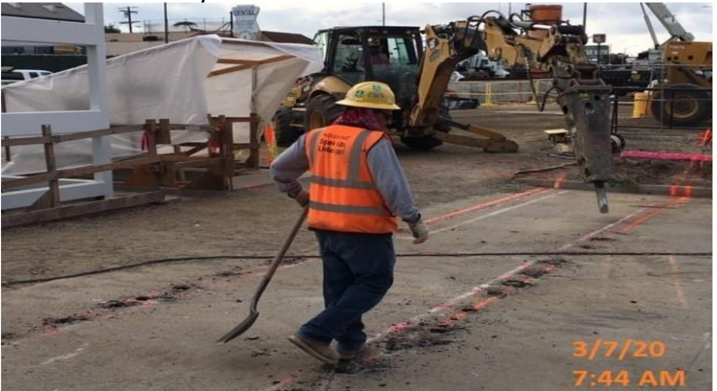
MLK STATION – WSCC crew demoing AC for planter.
