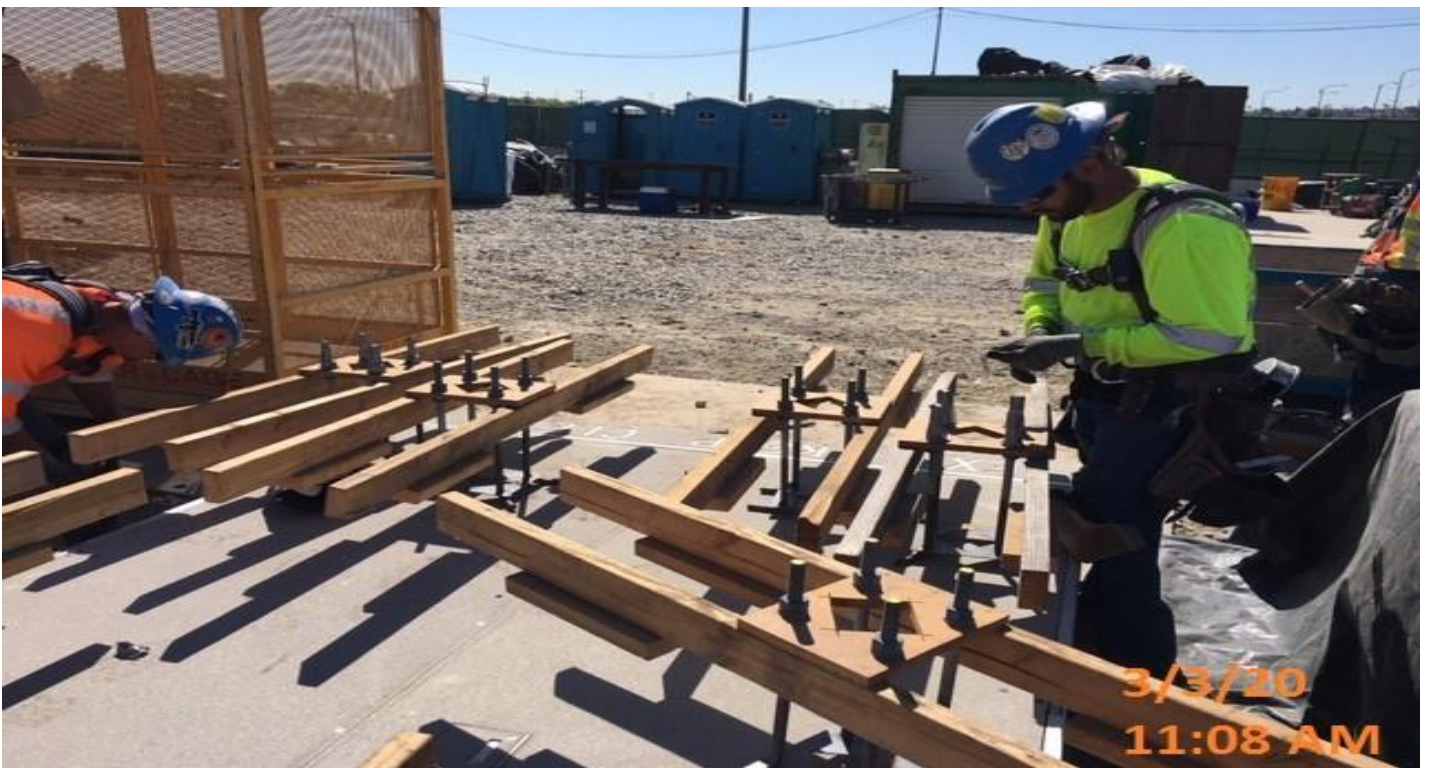
EXPO STATION- WSCC crew setting bolt templates for sono tubes.
