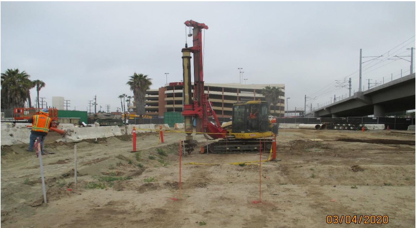
AVIATION/CENTURY- Drilling light pole foundations at the Aviation Station plaza area.
