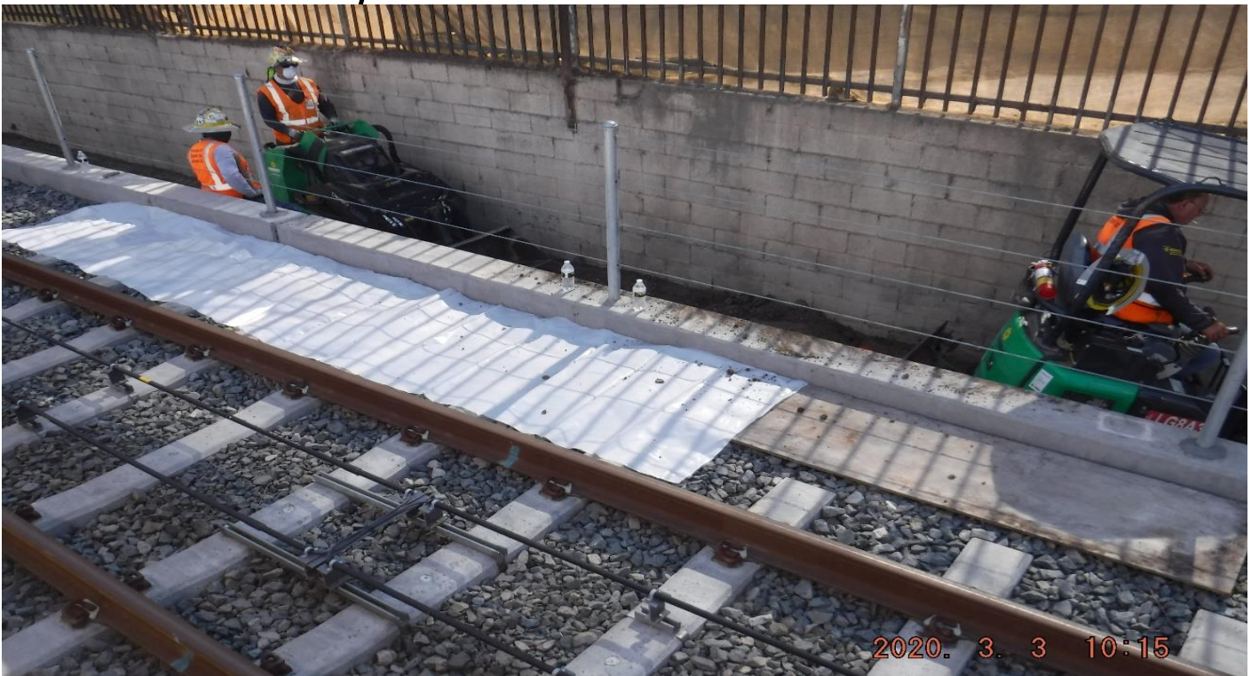
WEST Blvd - STA264+00_ Looking North_ Grading work behind ballast wall_ West.
