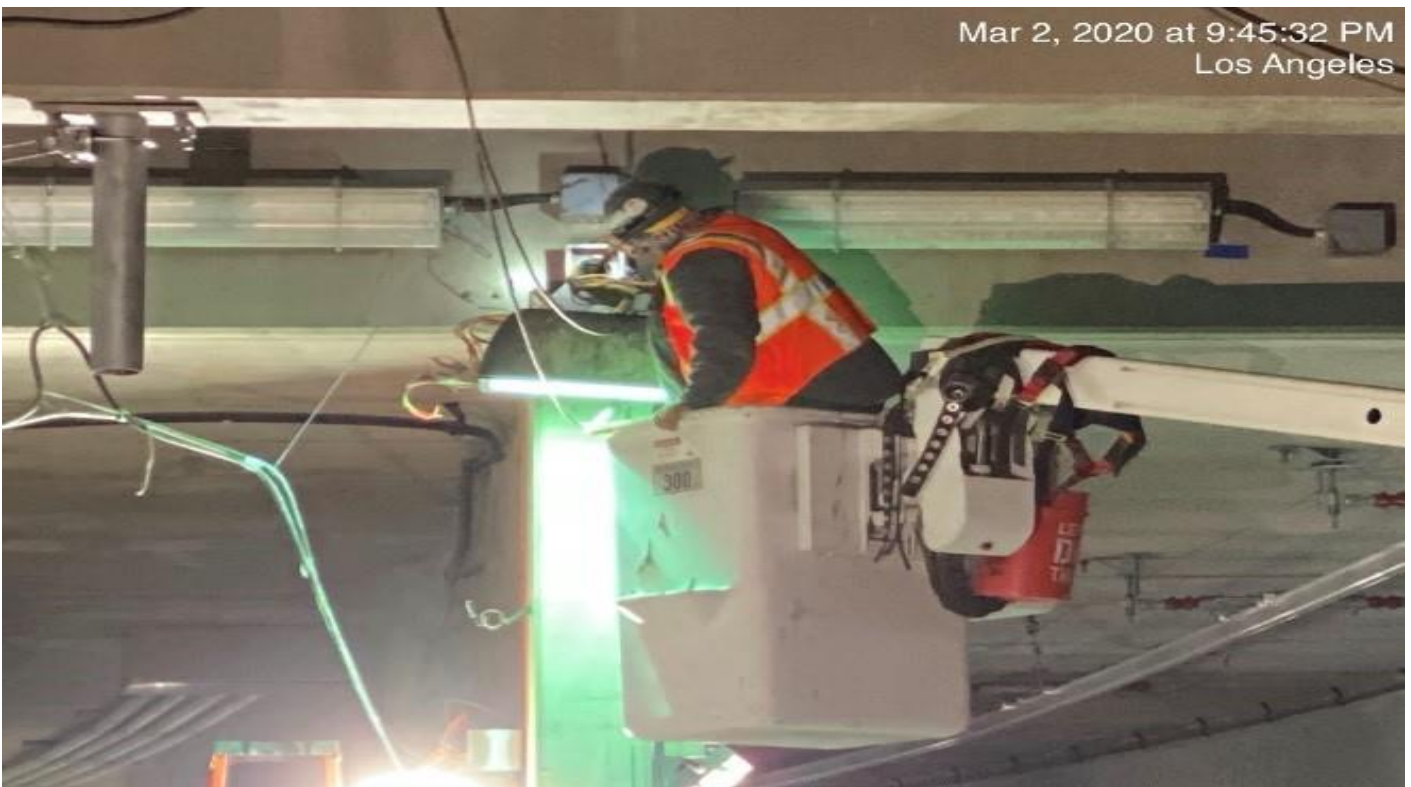
UG3 – DCD pulling wires for security lighting at UG-3.
