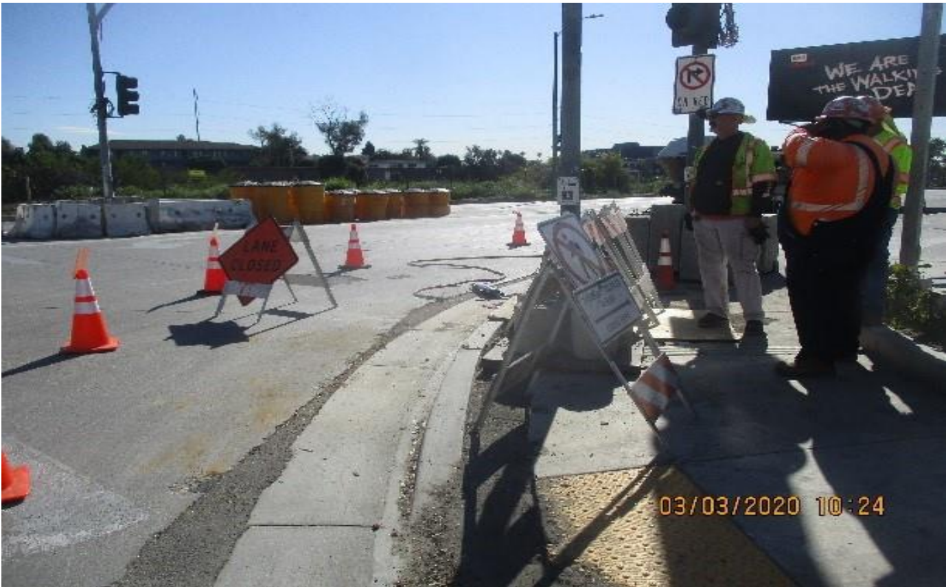
La Cienega/Florence - Select Electric Removing foundations at La Cienega and Florence.
