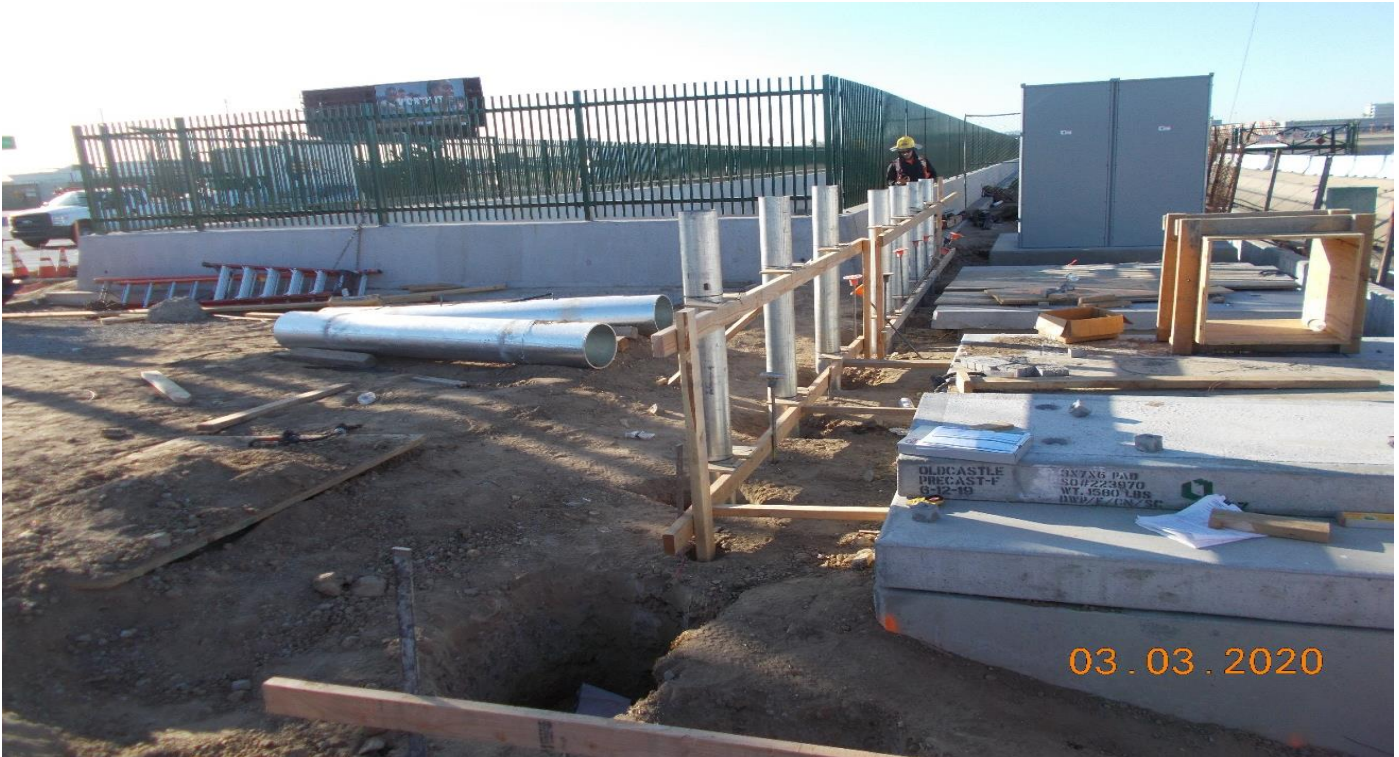
104th STREET – 104th St - WSCC was installing DWP bollards.
