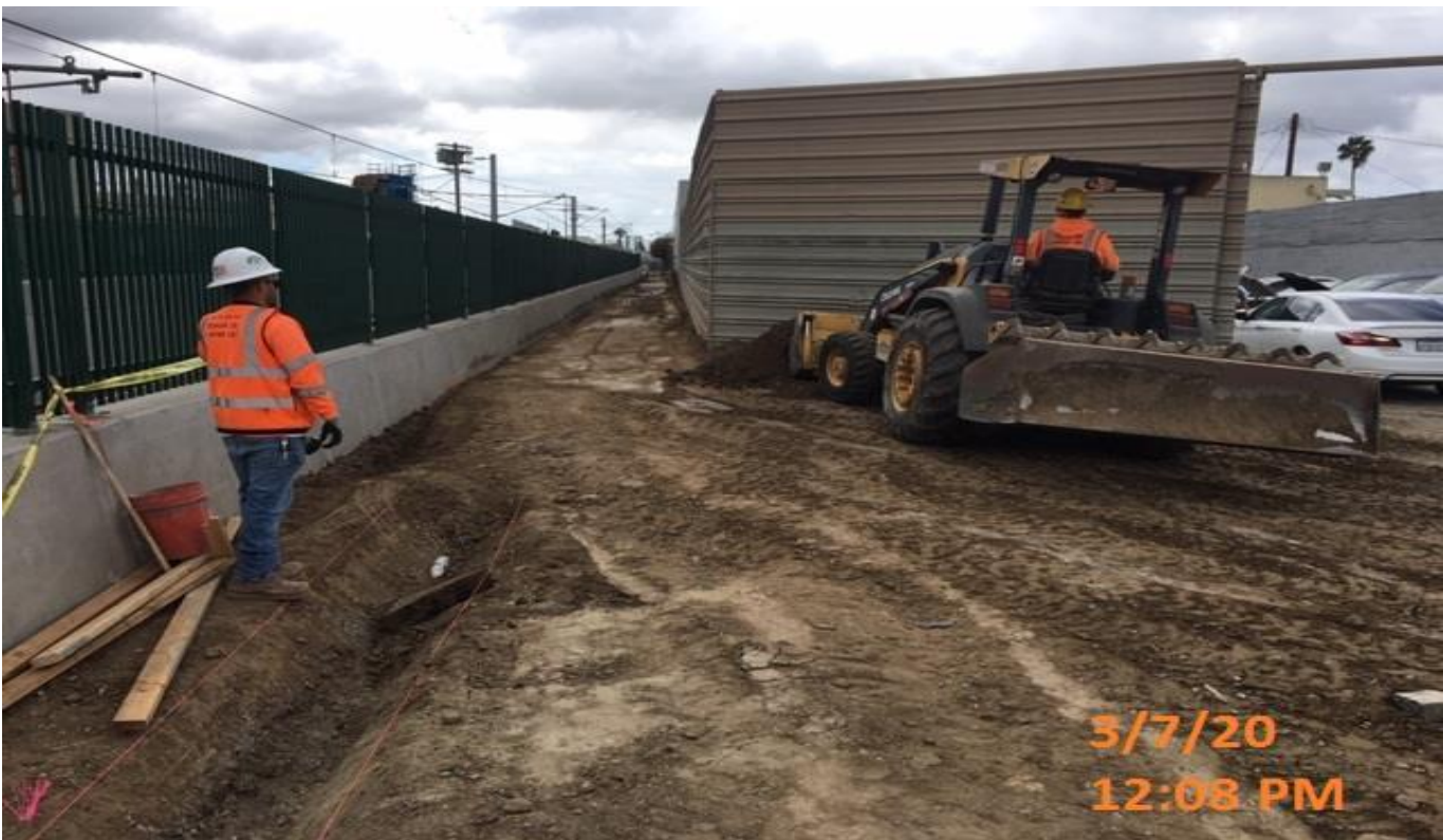
UG3 – Continued excavating the culvert drainage along the southbound barrier in preparation for concrete placement. 3/6/20
