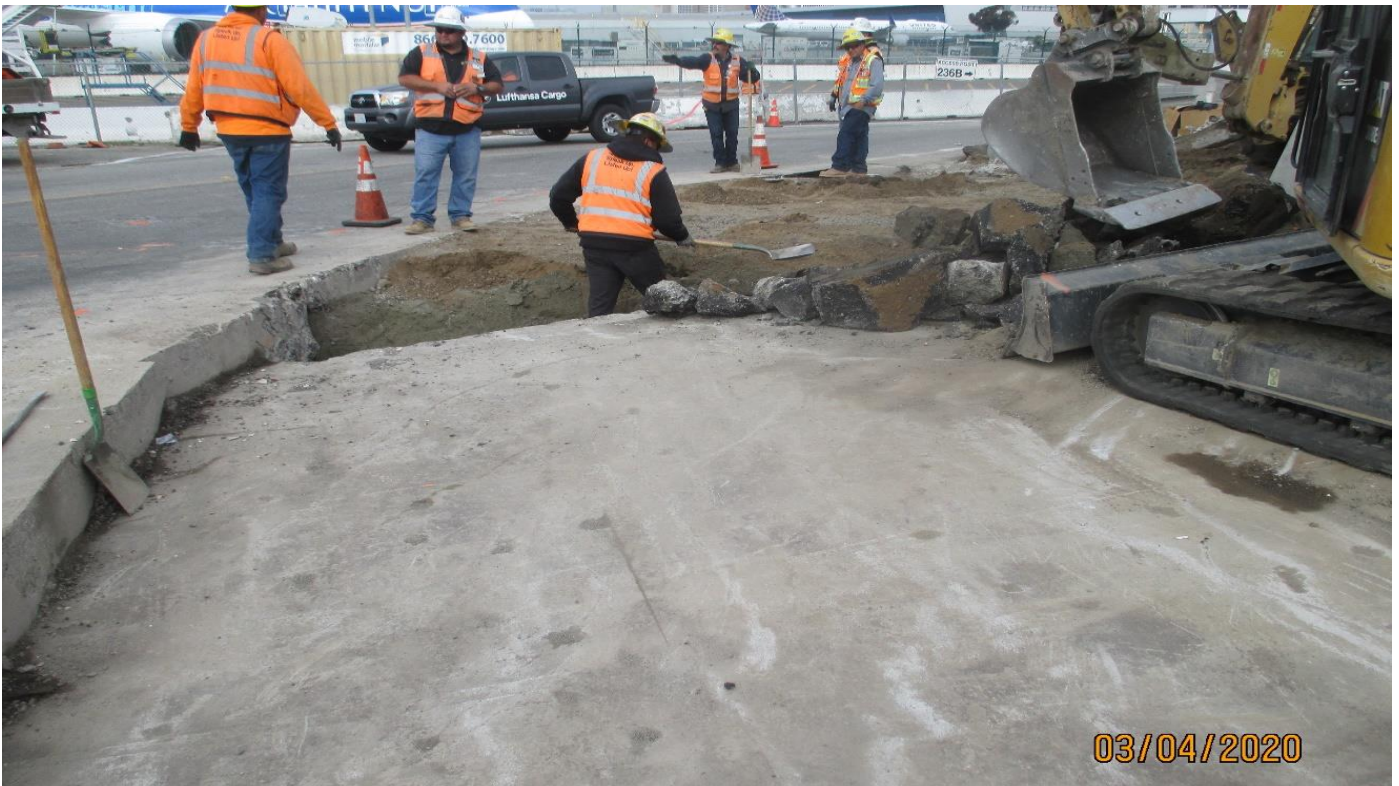
104th STREET – Curb & gutter removals at 104th street.
