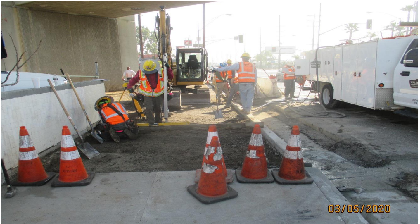
MANCHESTER AVE- Sidewalk grading at Manchester.
