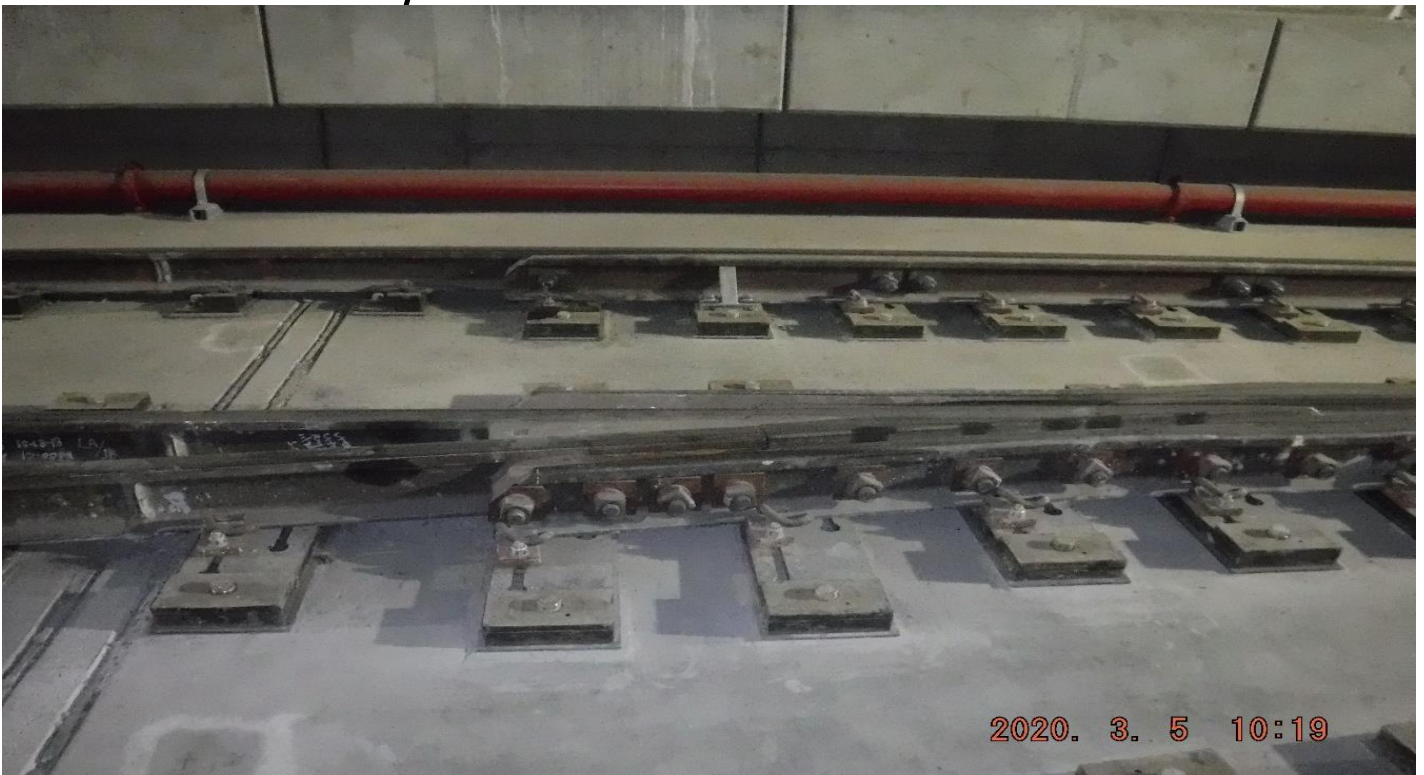
UG-4- STA443+70_TK3_ Looking West_ Installed guard rail brace_ 8W2_ UG4_ Expo.
