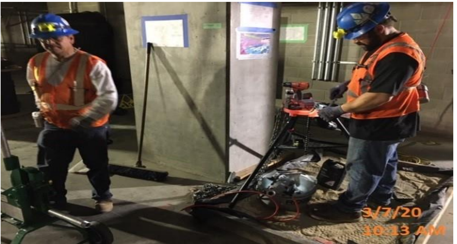
EXPO STATION- WSCC electricians installing FA conduit.
