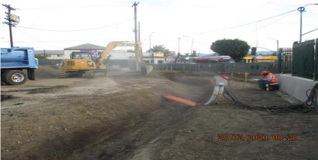
UG3 – Continue excavation for culvert drainage along the southbound barrier wall from Sta 279+20 – 282+93.
