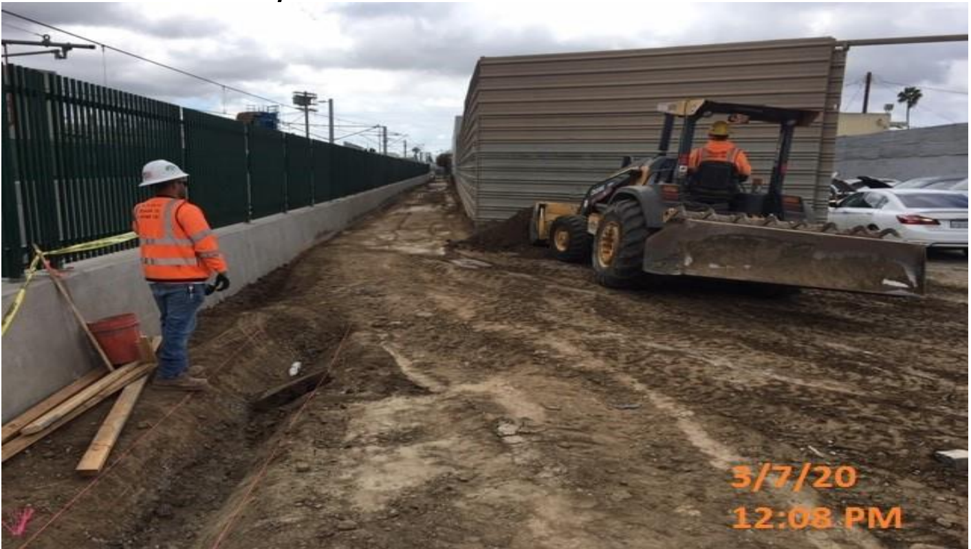
UG3 – UG3.Victoria Yard– WSCC crew backfilling guideway.
