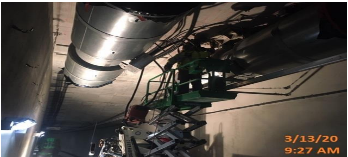
UG-4- – Installing seismic cables for the tunnel booster fans on the northbound tunnel at Sta 374+32.
