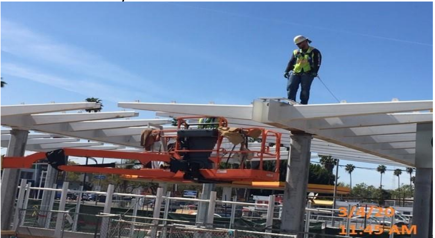
EXPO STATION- McMahon installing cat walk grating above main.
