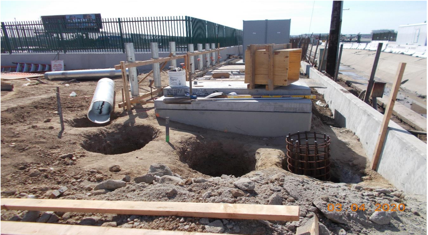
104 th STREET – WSCC had dug large footings for large DWP bollards.
