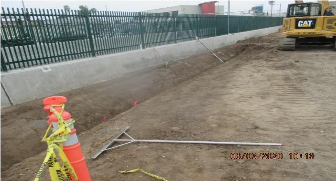
UG3 – Continued excavating the culvert drainage along the southbound barrier in preparation for concrete placement. 3/6/20
