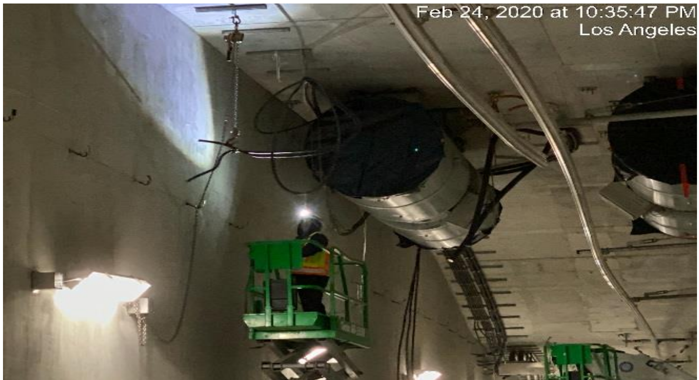
UG4 – Continue wiring and running cable for the booster fans in the northbound tunnel at Sta 374+25.
