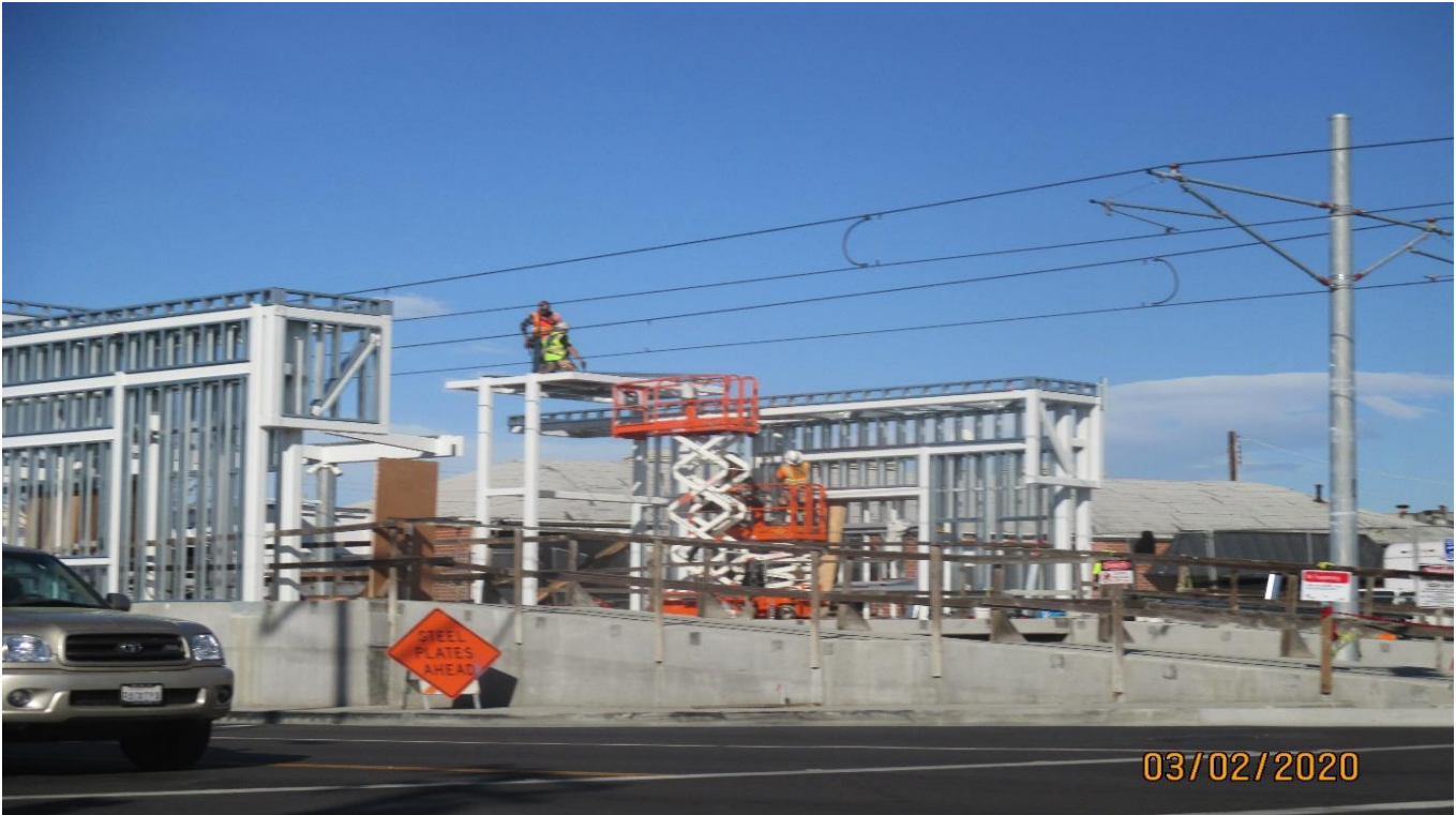
HINDRY AVE- Metal stud framing at the Hindry Station.
