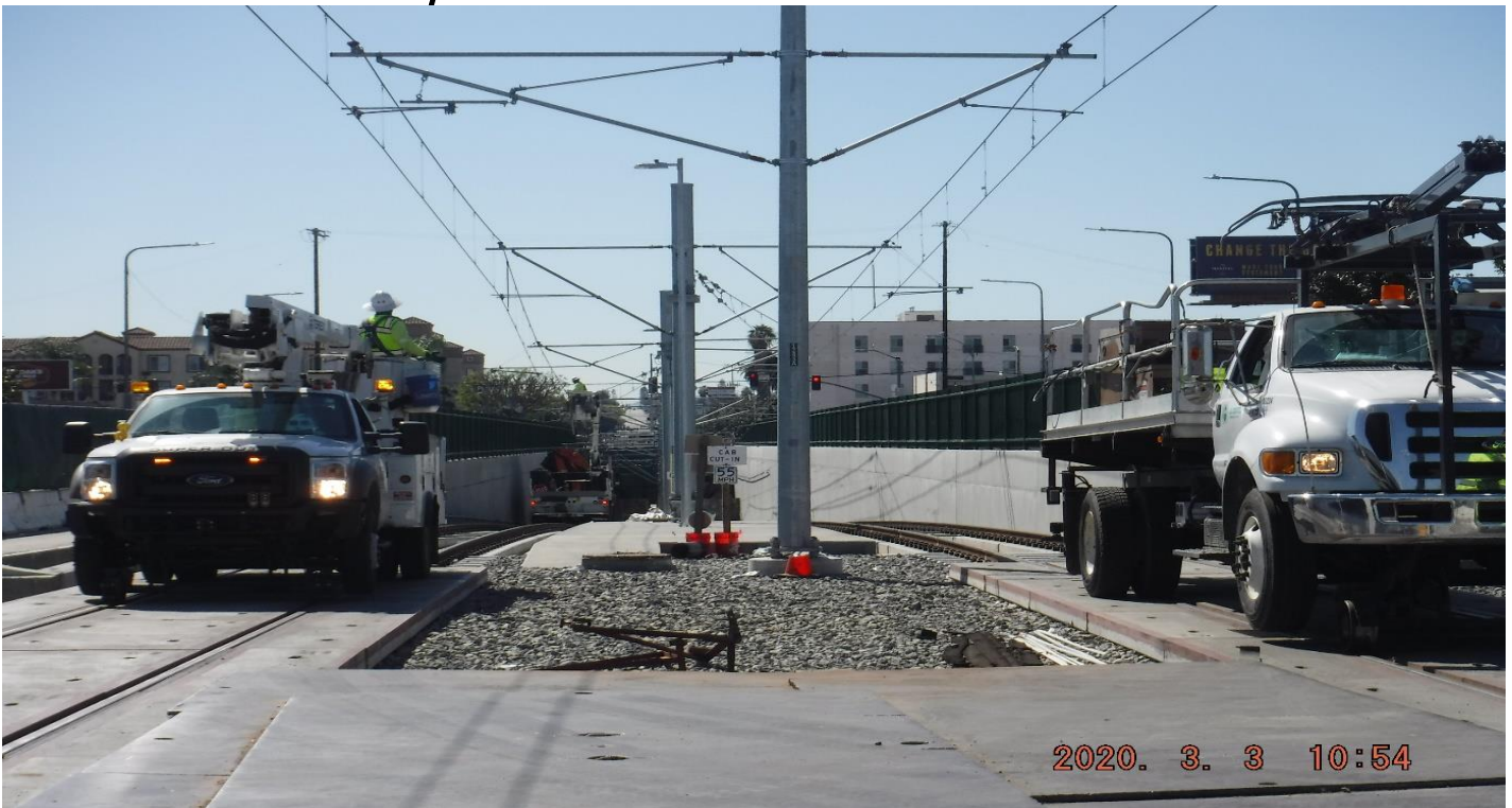
UG3 – STA317+00_ Looking South_ OCS work north ramp UG3_ 59ST.
