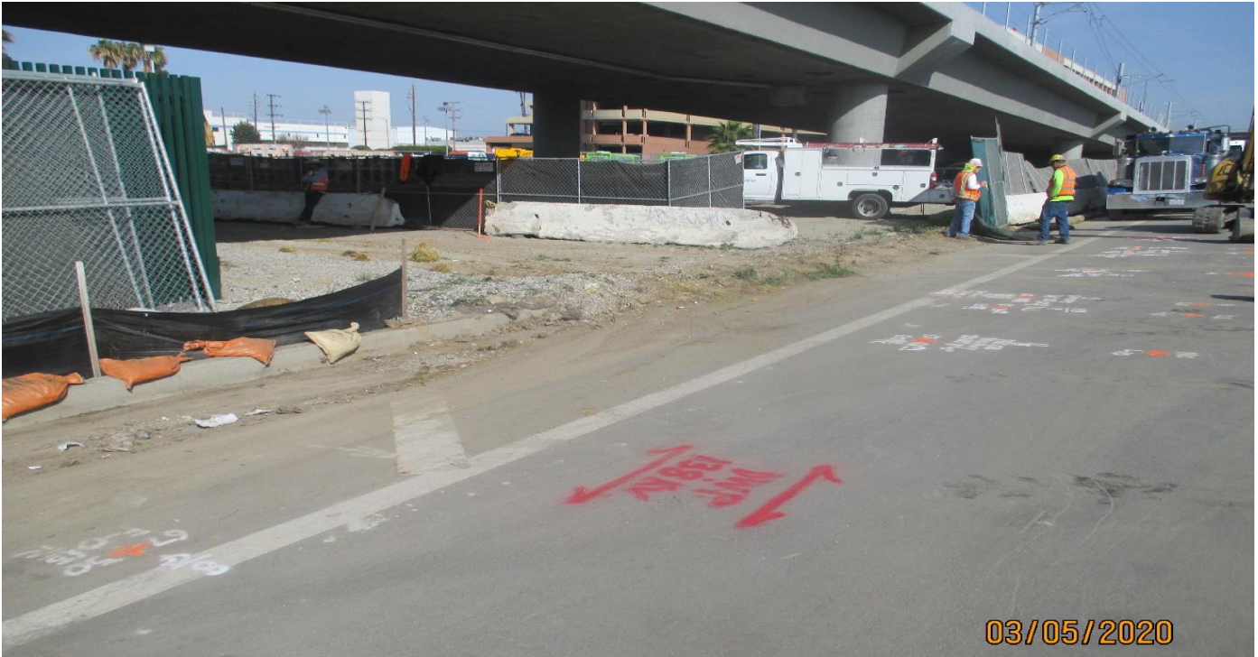
AVIATION/CENTURY- Grading for the Aviation Station plaza and parking lot.
