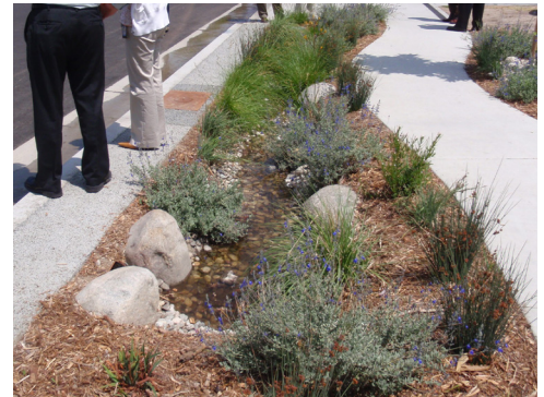
Bioswales help mitigate stormwater run-off while infiltrating and removing silt and pollution from run-off water.
