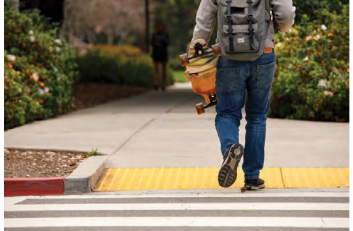
Sidewalks with tactile striping and banked corners help pedestrians with a range of abilities.
