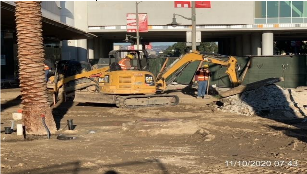
MLK STATION – Grading/compacting the far northwest area of the plaza.
