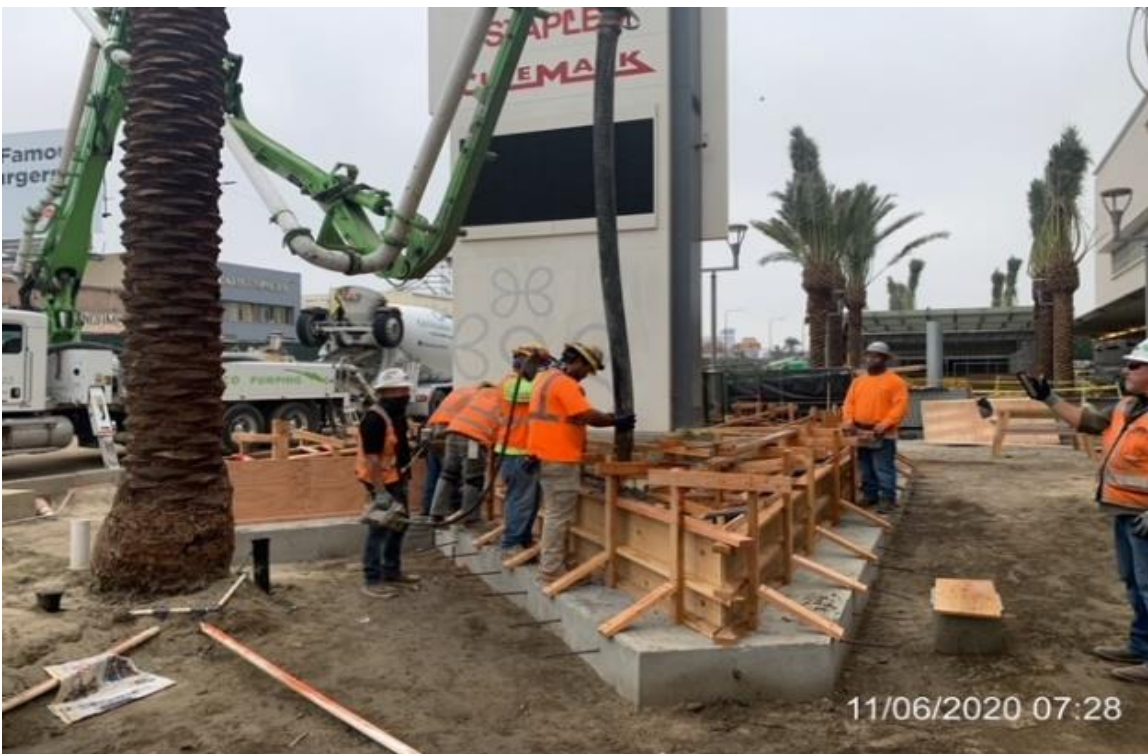
MLK STATION – WSCC crew placing concrete for north planter wall.
