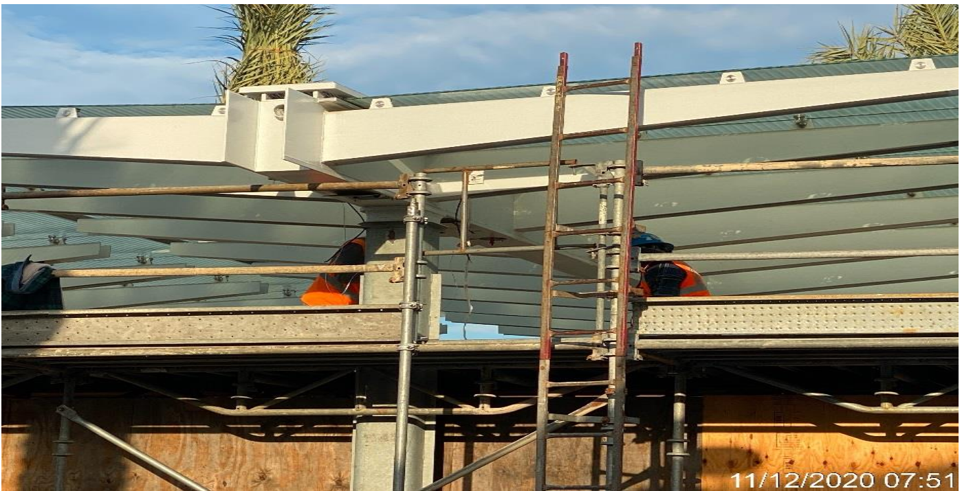
LEIMERT PARK STATION – Continue installing BOCA light fixtures to the main entrance canopy outriggers at the plaza.
