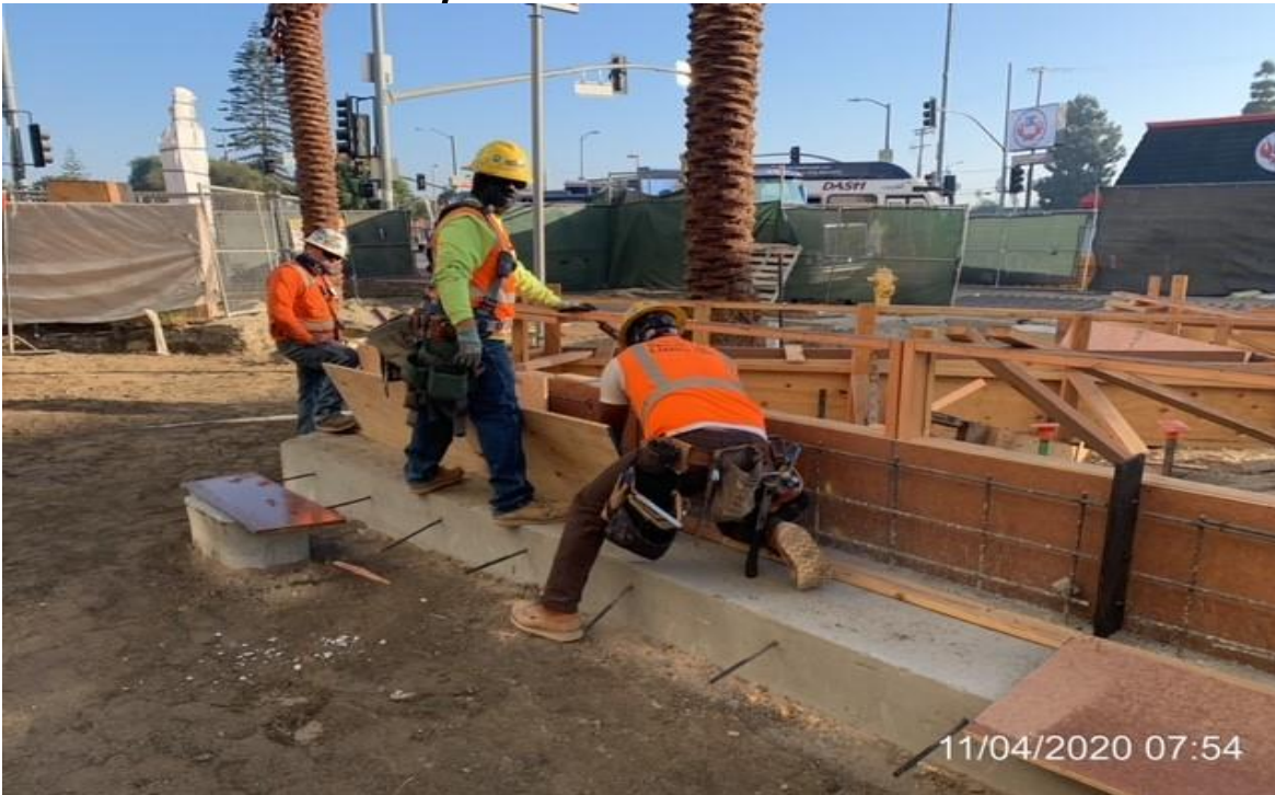
MLK STATION – WSCC carpenters building formwork for north planter wall.
