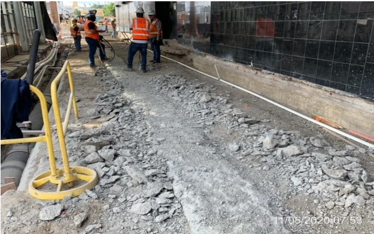
MLK STATION – WSCC crew chipping concrete encasement.
