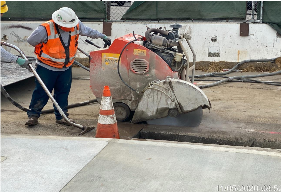
Leimert Park – WSCC saw cutting asphalt for removal at Vernon
