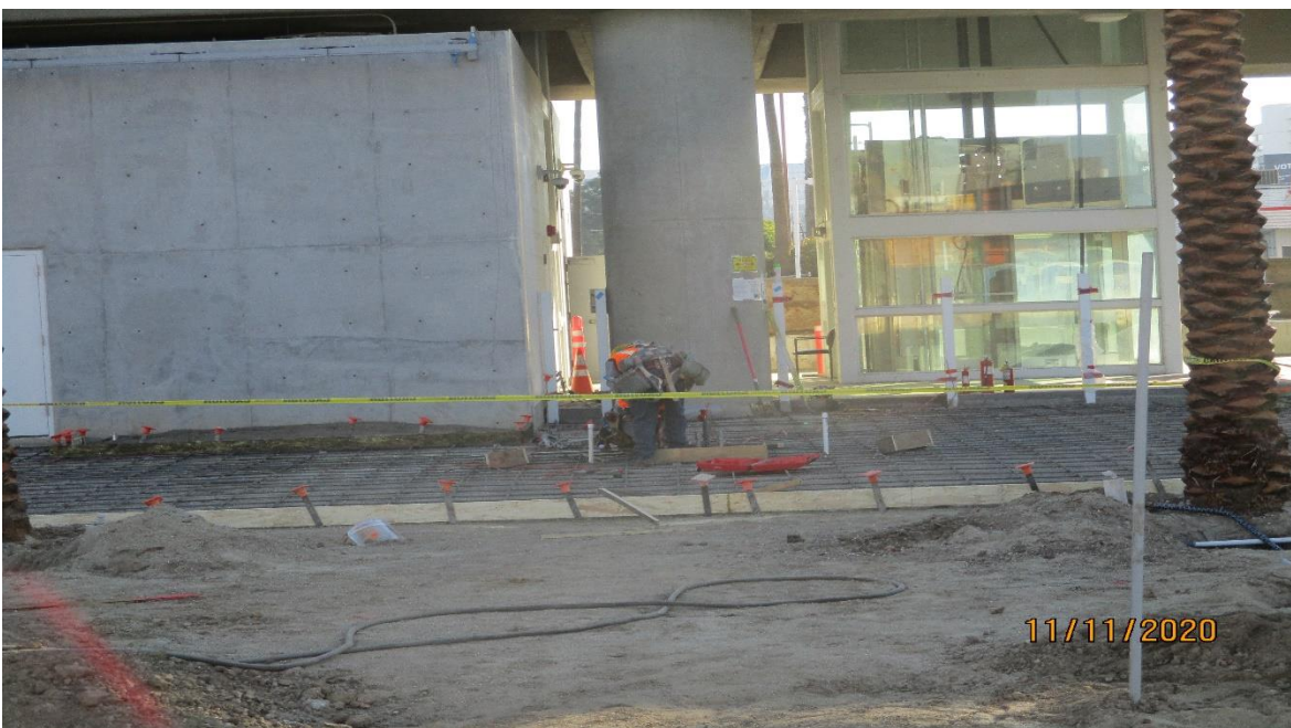
AVIATION/CENTURY- Building light pole foundation blockouts at the Aviation Station plaza.
