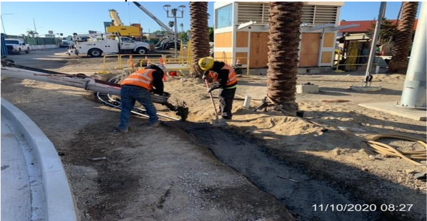
MLK STATION – Encased landscape conduit with concrete at the plaza.
