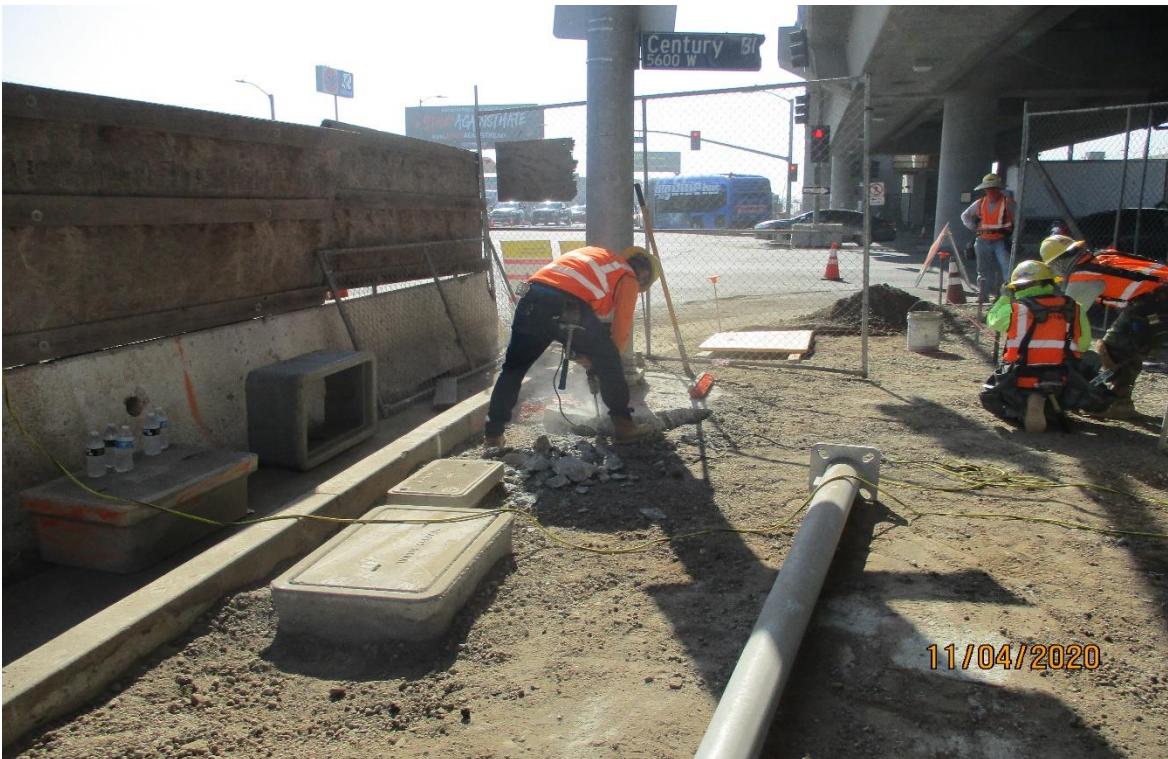
AVIATION/CENTURY- Layout for the ADA ramp on the NW corner of Aviation and Century.
