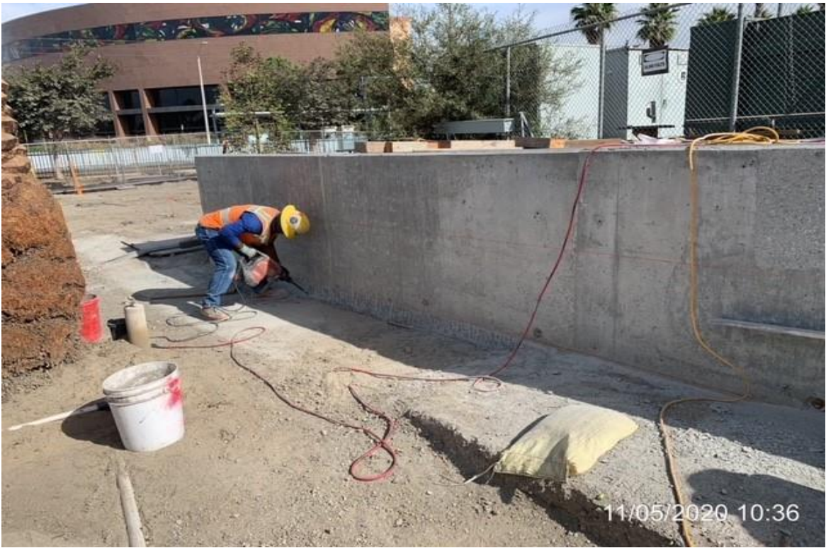
EXPO STATION – WSCC crew chipping footing of air exhaust shaft north.
