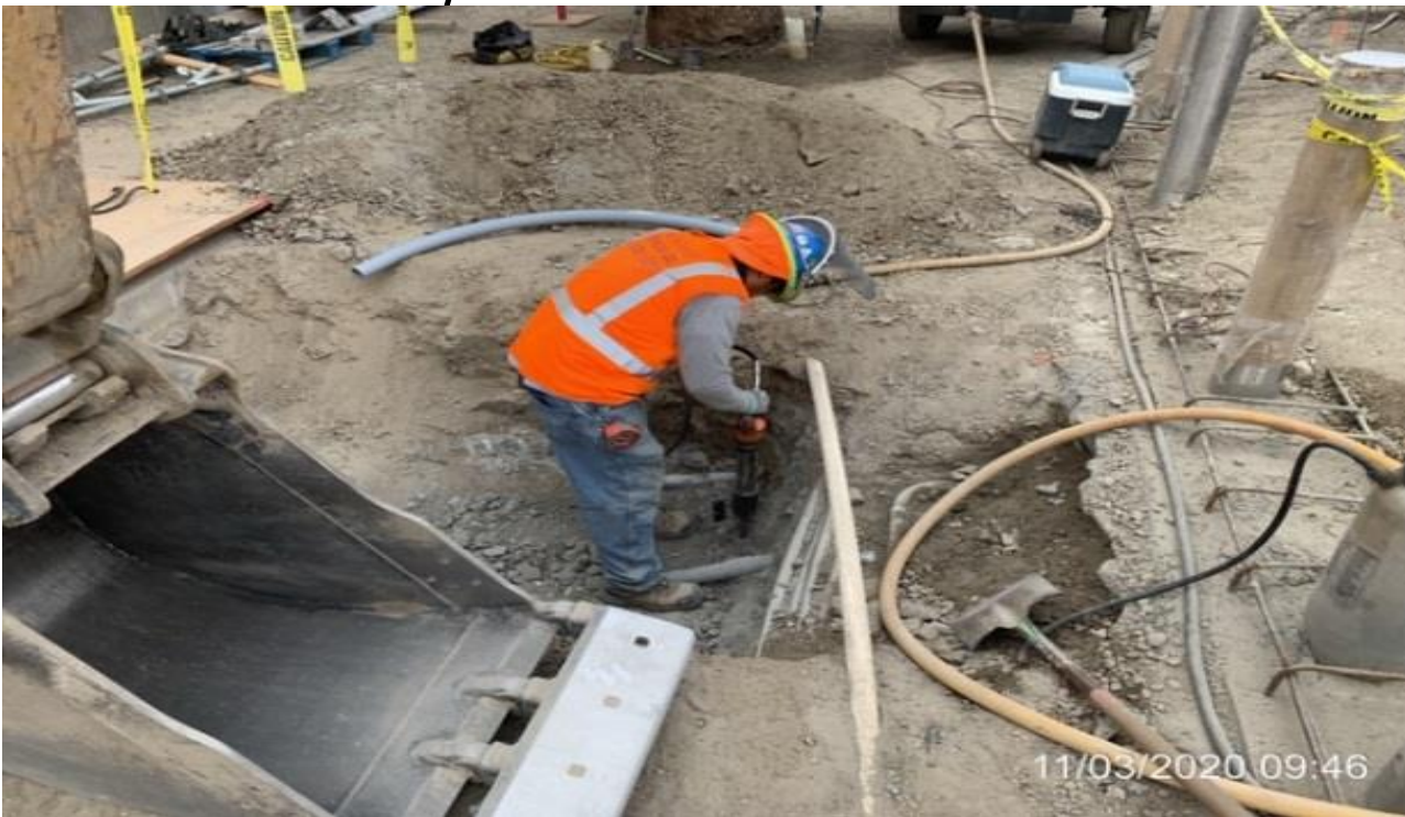
EXPO STATION – WSCC crew chipping for electrical conduit replacement.
