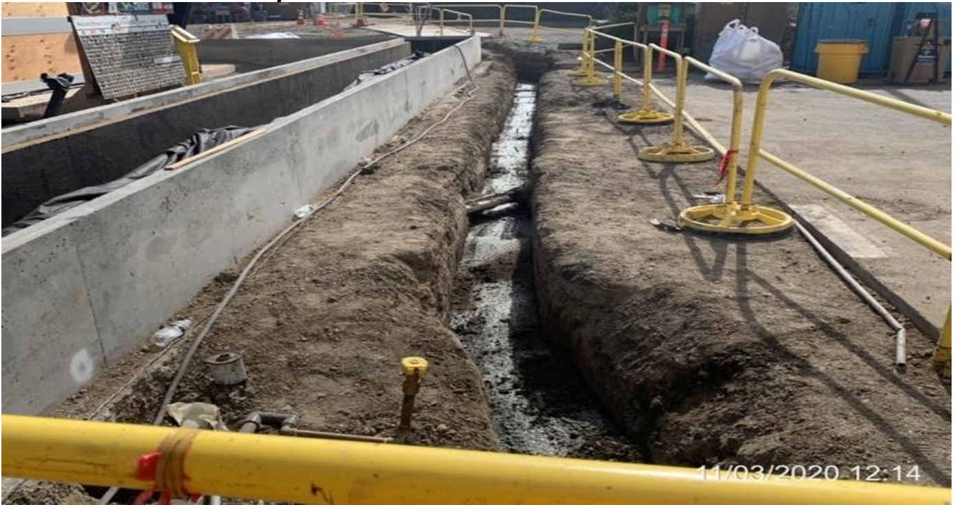
MLK STATION – Encased irrigation conduit with concrete at the plaza.
