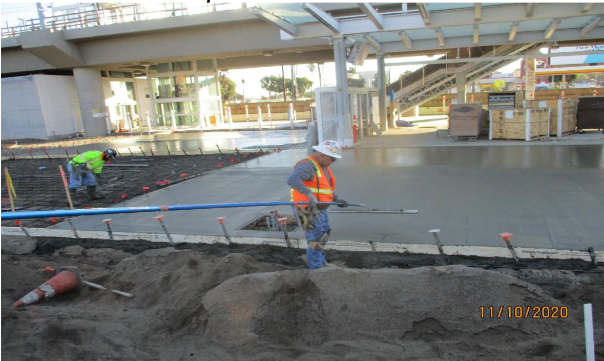
AVIATION/CENTURY- Finishing the concrete placed for the Aviation Station plaza hardscape.
