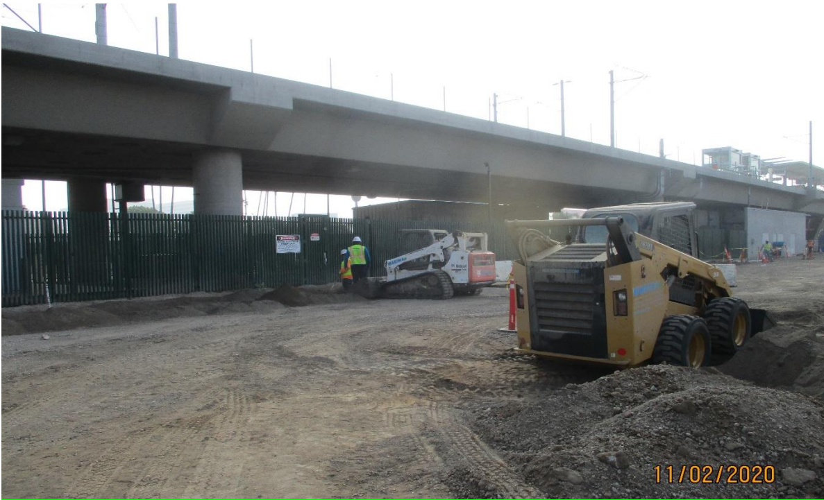
AVIATION/CENTURY - Placing amended soil for the planters at Aviation Station.
