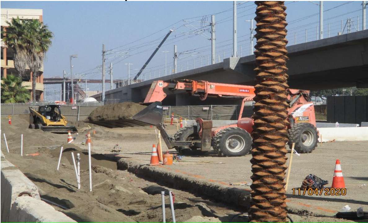
AVIATION/CENTURY- Placing amended soil at the Aviation Station plaza area.
