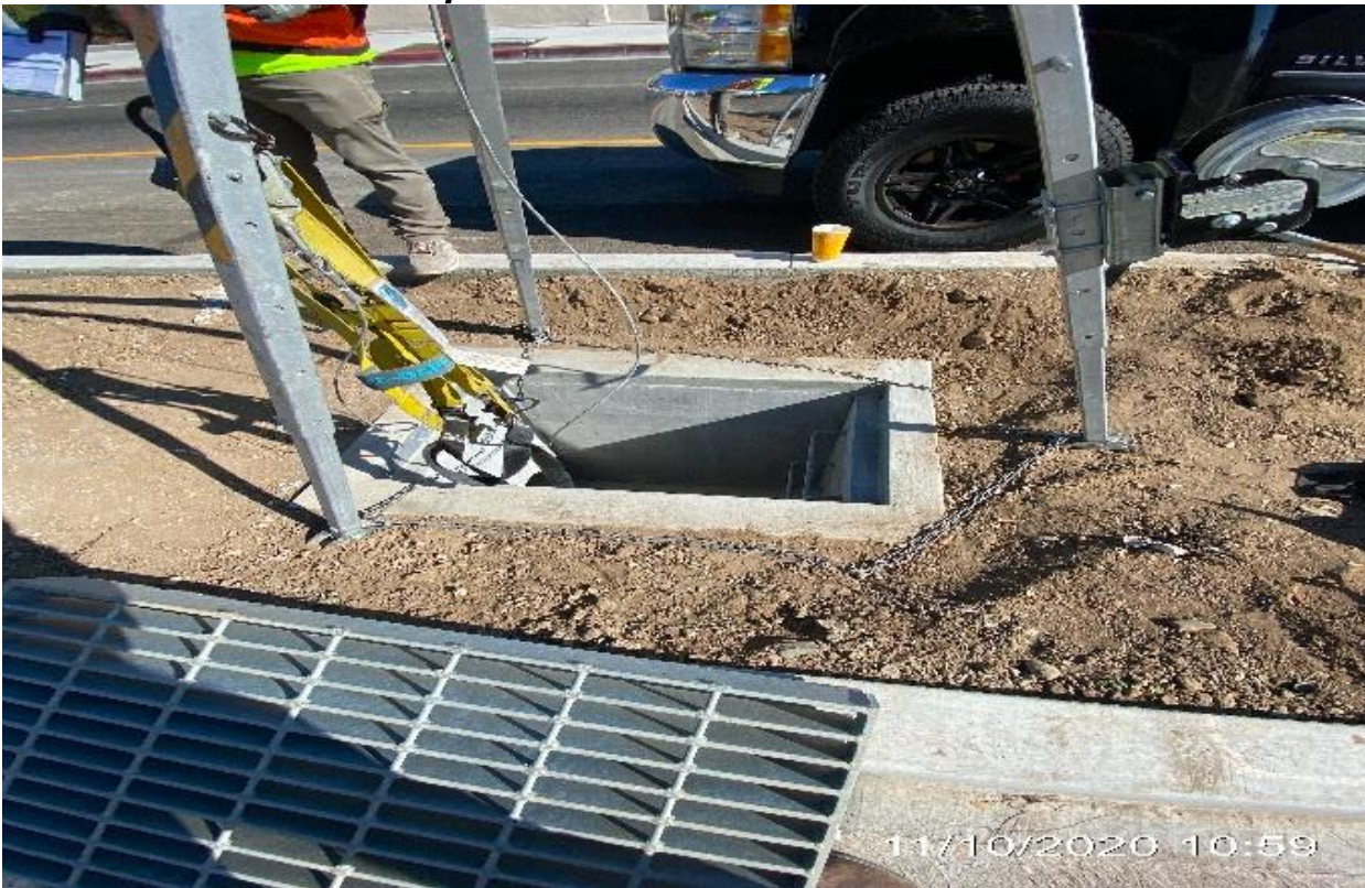
LEIMERT PARK STATION – Sacking and patching CB#10 and #11 on SB/NB Crenshaw Blvd and Brynhurst Ave.
