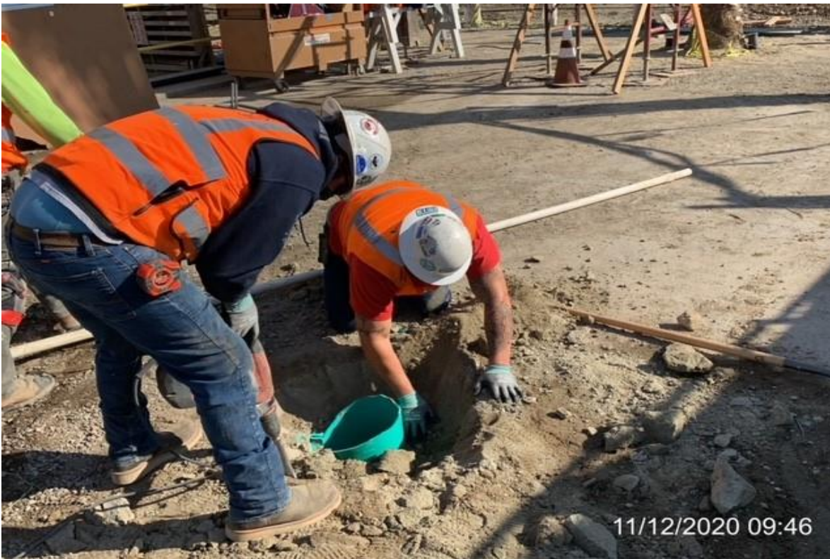
EXPO STATION – WSCC crew removing and replacing damaged 12' PVC drain.
