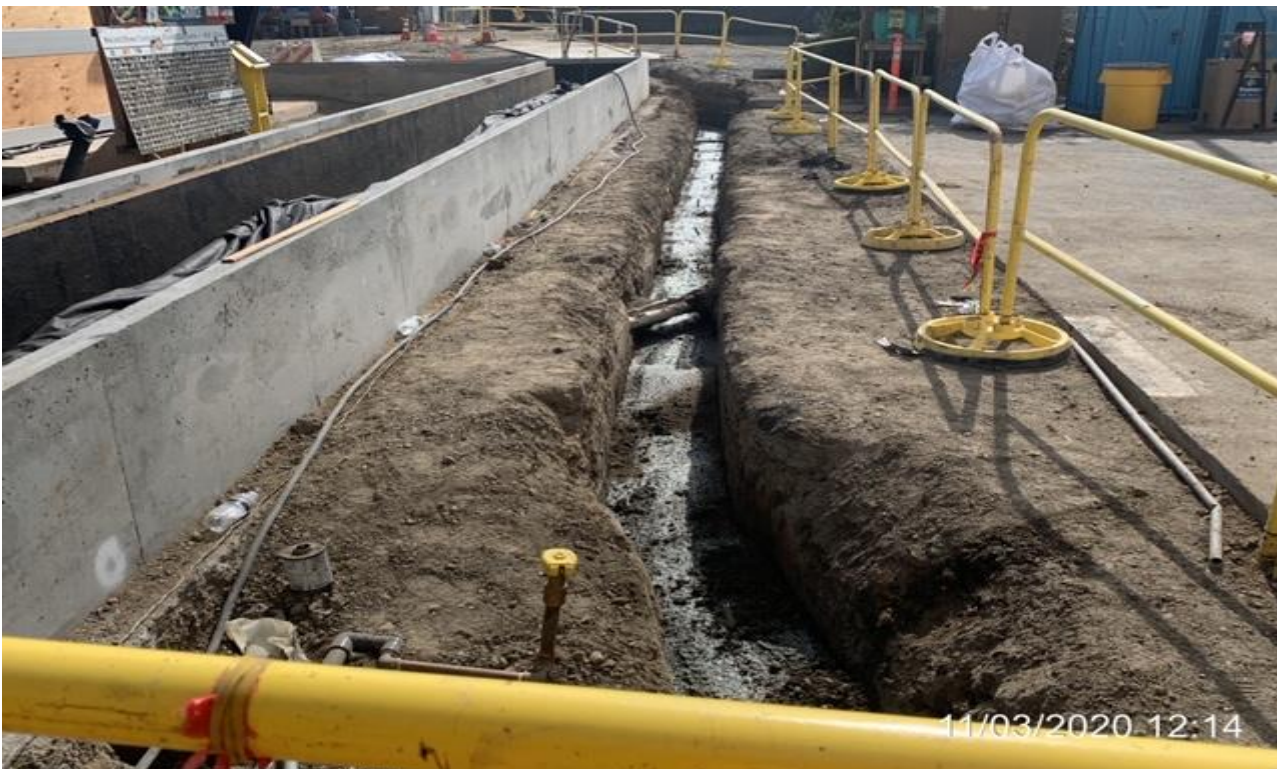
MLK STATION – WSCC crew placed concrete encasement for irrigation electrical conduit.
