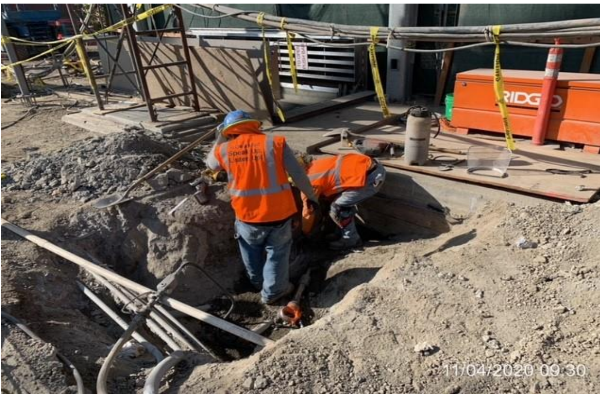
EXPO STATION – WSCC crew chipping encasement to add pull box..
