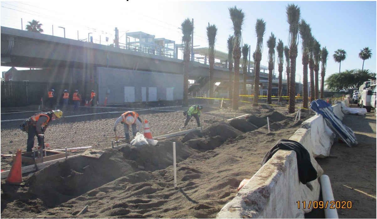
AVIATION/CENTURY- Setting forms for the Aviation Station hardscape.
