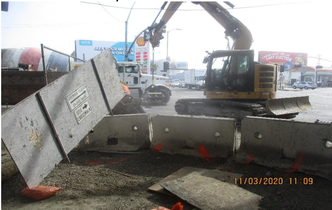
AVIATION/CENTURY- WSCC remove Krail at Aviation and Century Blvd.
