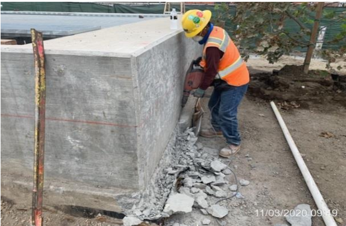
EXPO STATION – WSCC chipping footing of north emergency ventilation shaft.
