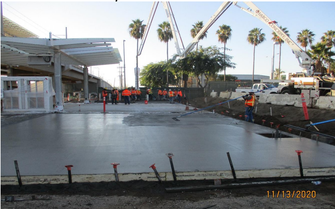
AVIATION/CENTURY- Placing concrete for the Aviation Station plaza.
