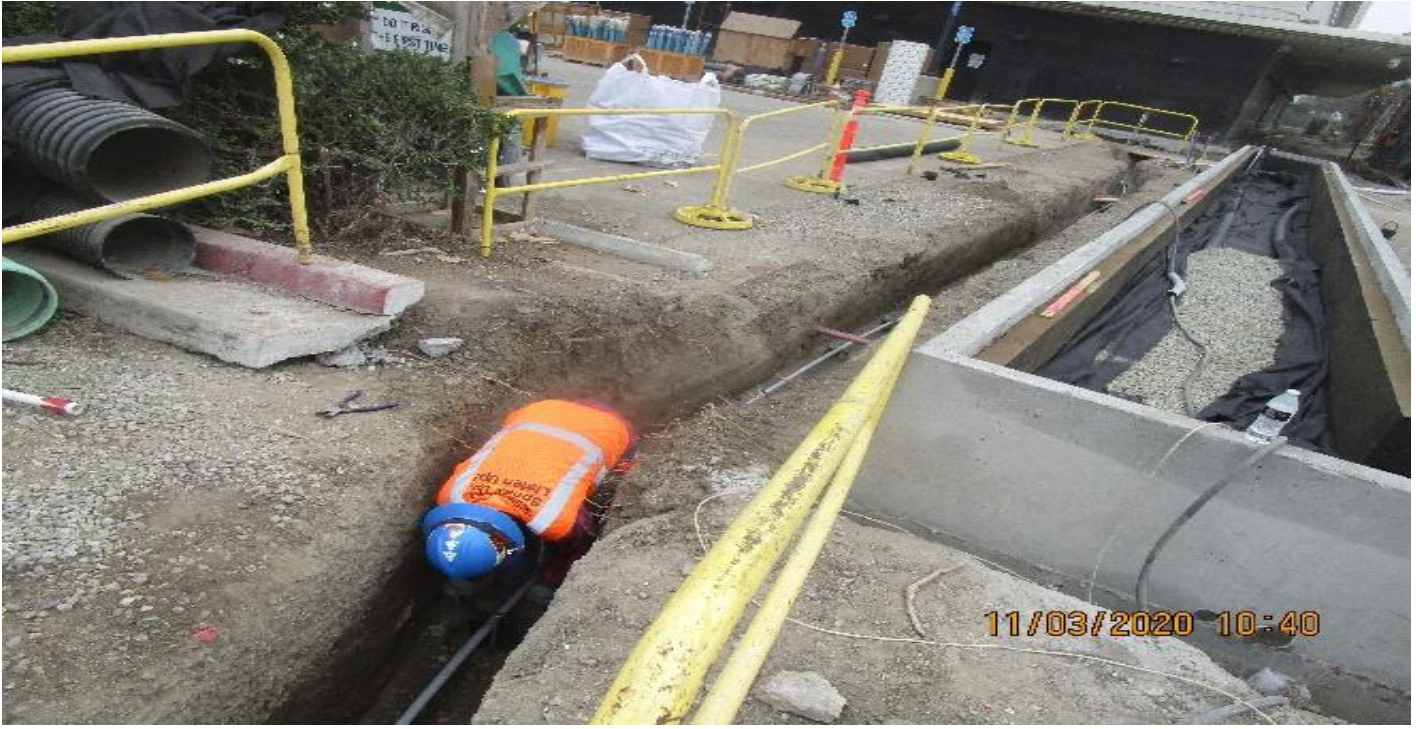
MLK STATION – Placing underground landscape conduit for irrigation at the plaza.
