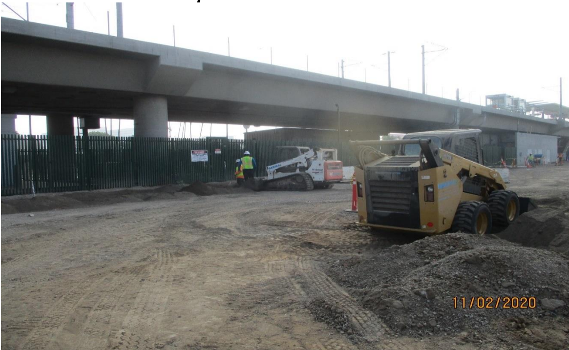
AVIATION/CENTURY- Placing and spreading the amended soil at the aviation Station. Facing SE.
