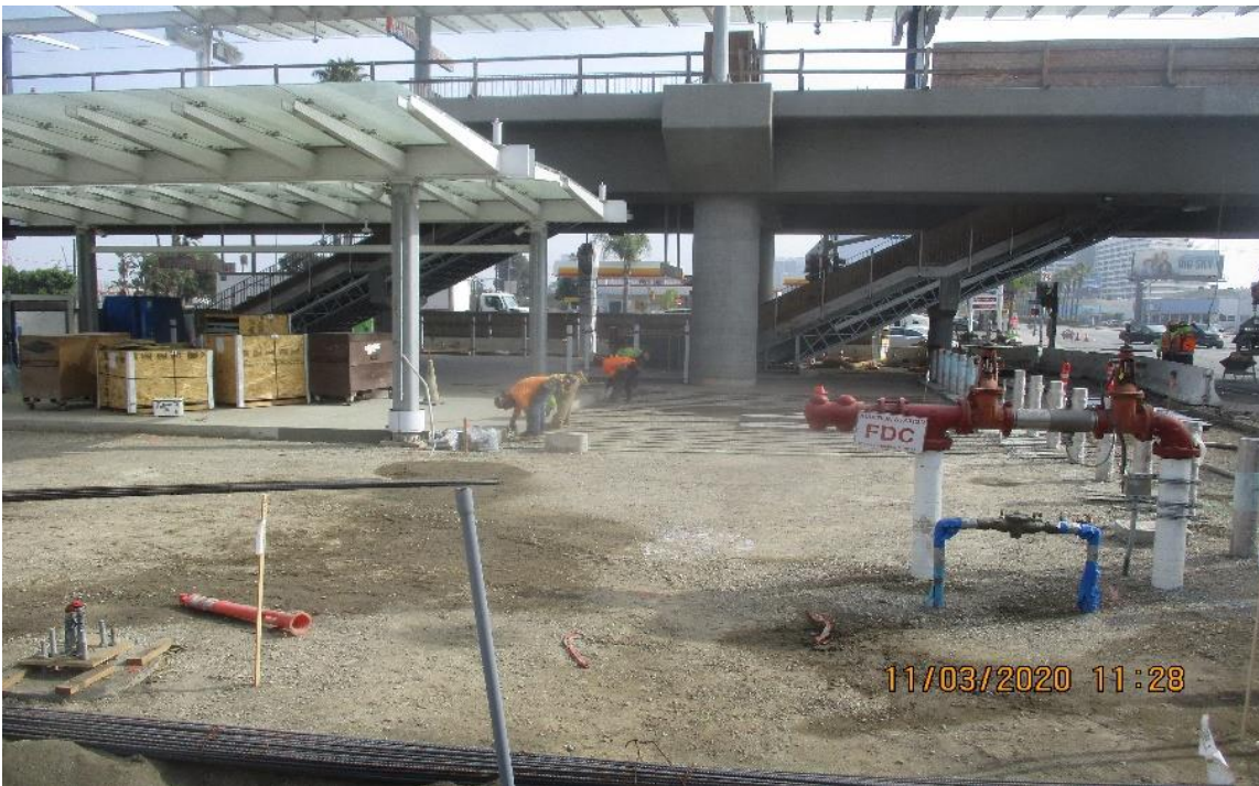
AVIATION/CENTURY- WSCC Placed rebar for Aviation Sta plaza floor.
