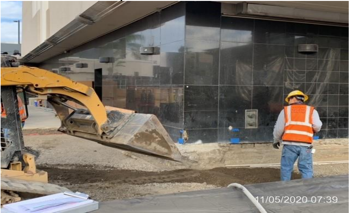
MLK STATION – WSCC crew backfilling and compacting.
