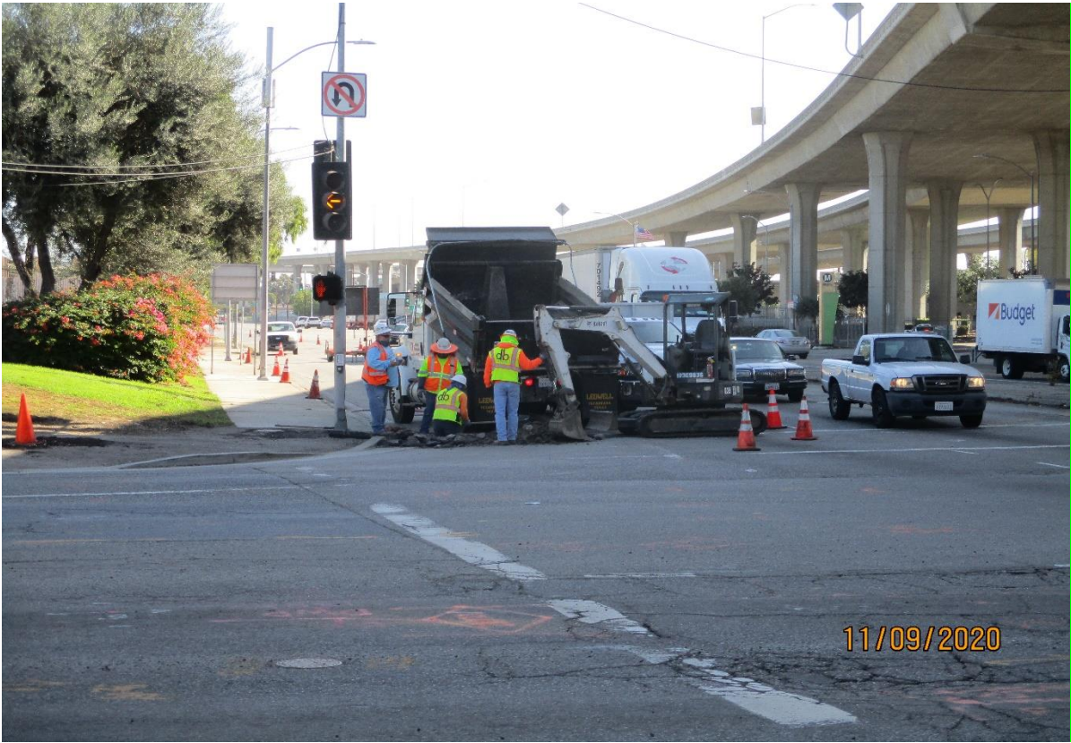
AVIATION/CENTURY- Excavating for traffic signal run 16 on Imperial at Aviation.
