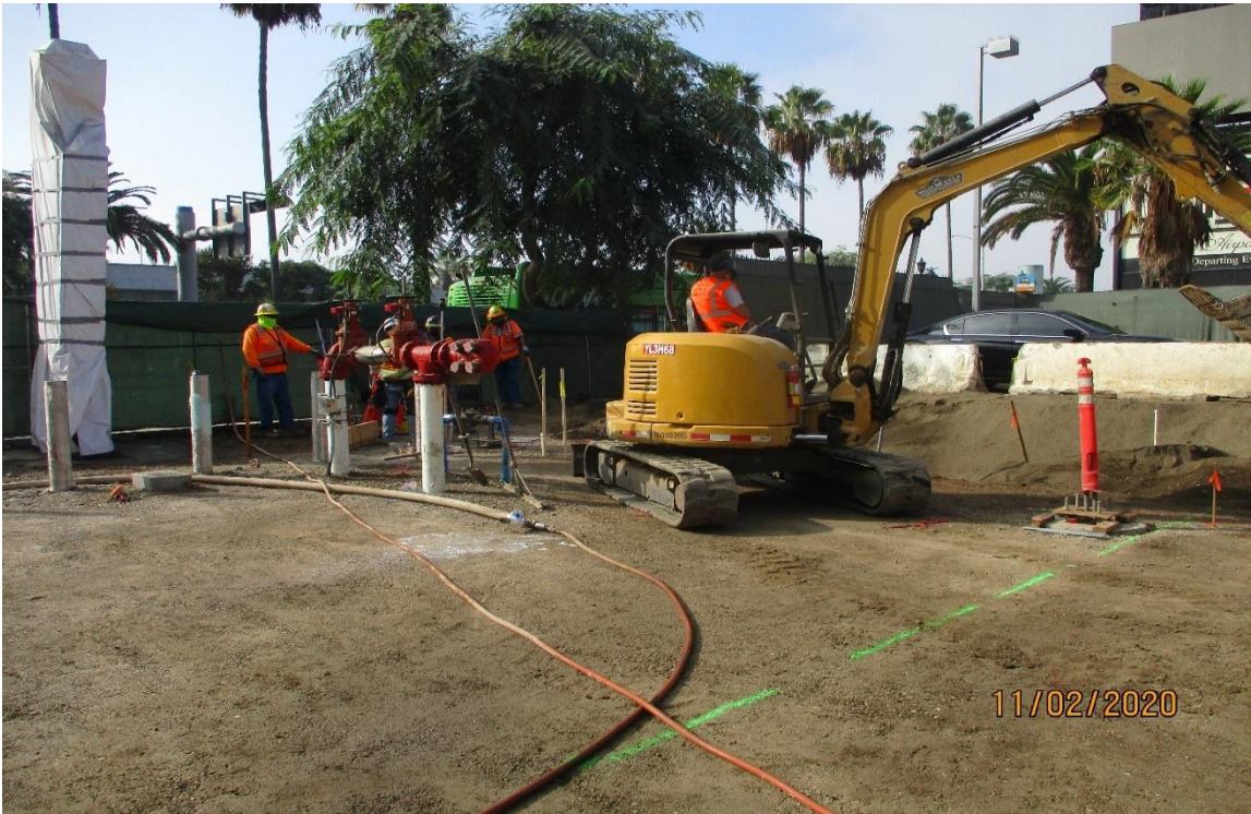
AVIATION/CENTURY- Grading for the hardscape at the Aviation Station.
