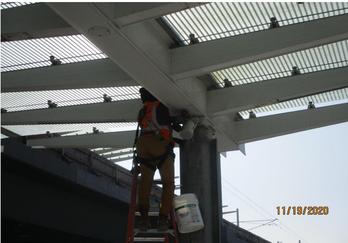
AVIATION/CENTURY- Cover plate installation at the Aviation Station ticket kiosk.
