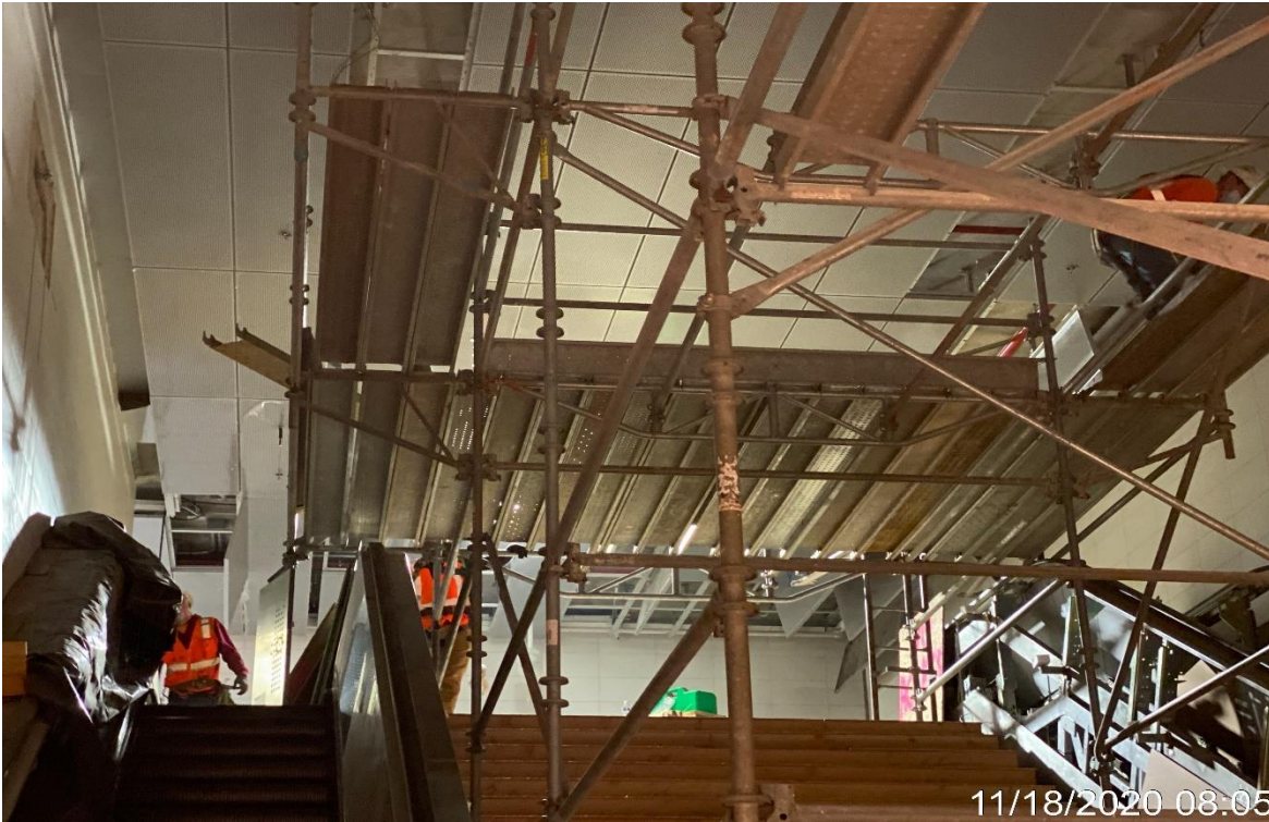
UG3 – Brand Safeway assembling scaffolding at Vernon.
