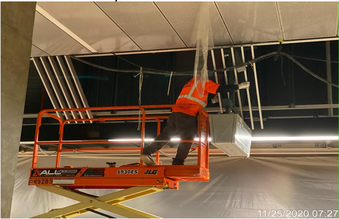
UG3 – PCI installing diagonal ceiling panels at Vernon
