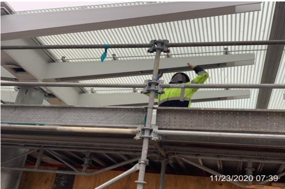
UG3 – VERNON – VNSM applying caulking to canopy Boca lighting
