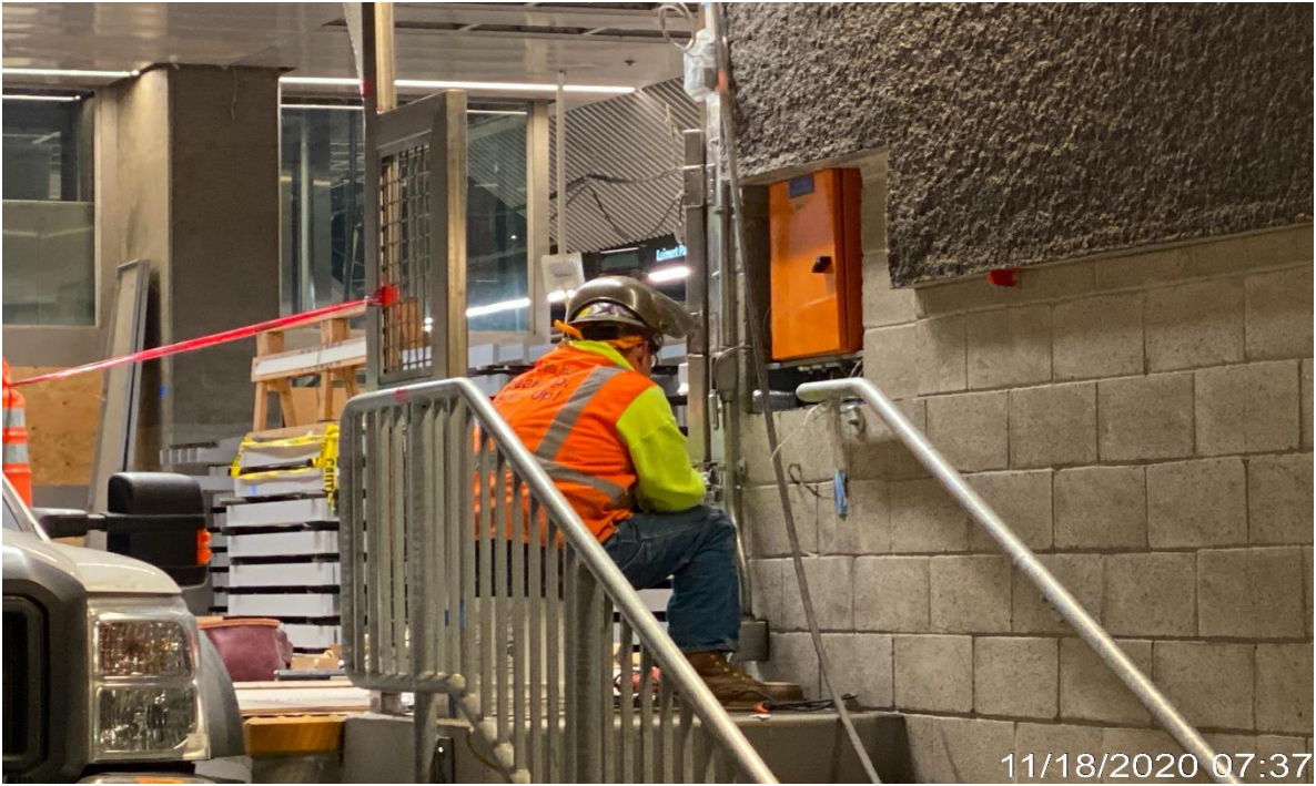
UG3 – WSCC welding hinges for end gates at Vernon.
