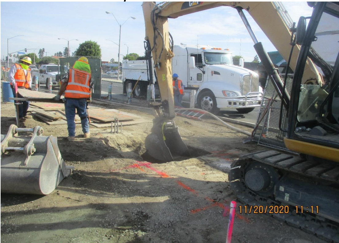
La Brea – WSCC Excavate and relocate holes at La Brea Plaza.
