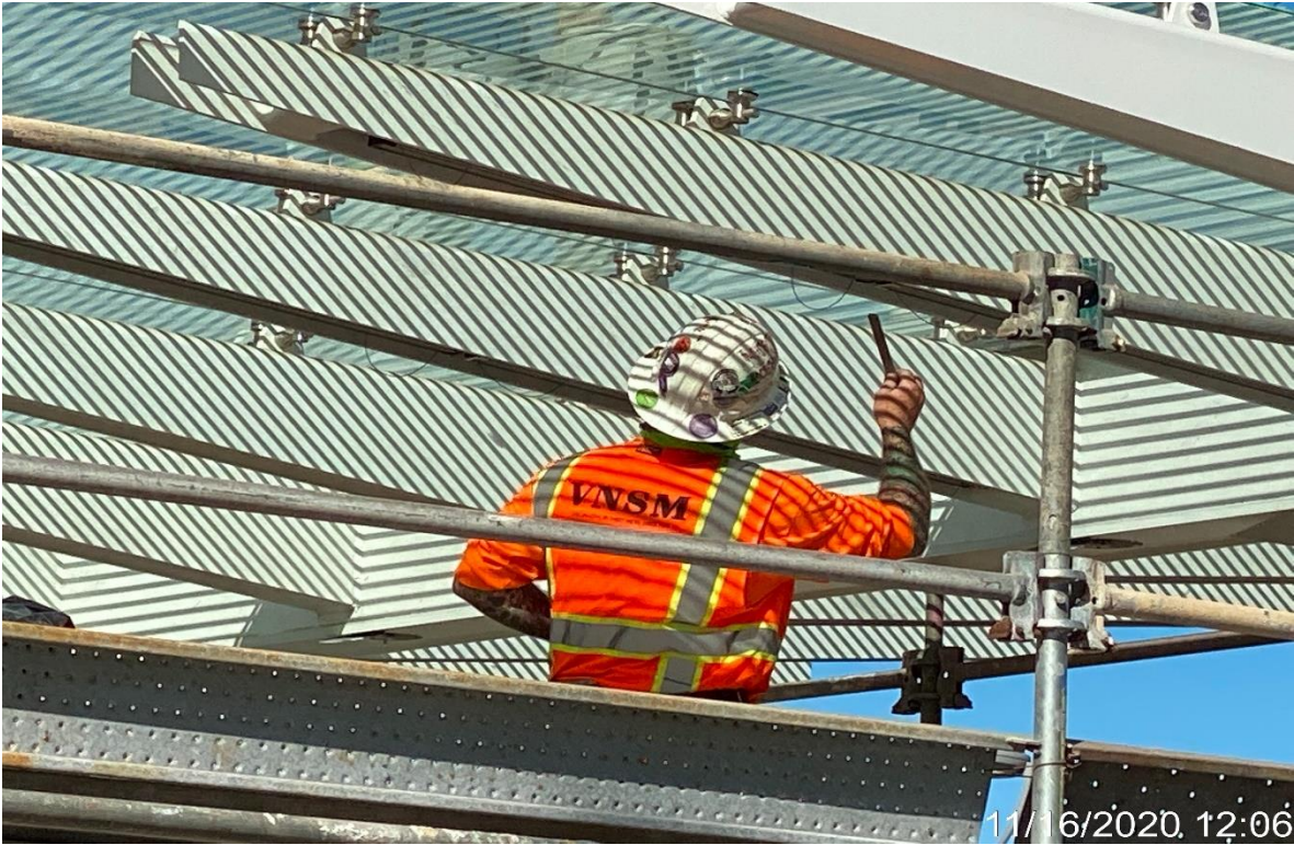
UG3 – VNSM installing Boca lighting brackets at Vernon.
