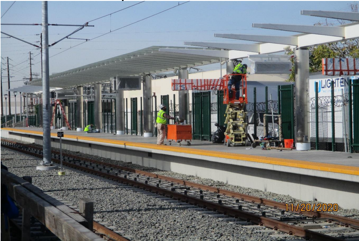
Hindry – Thermoplastic striping at the Hindry Station NB platform.
