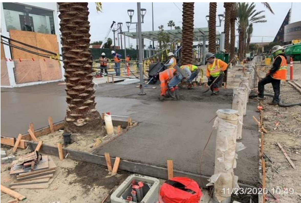
EXPO STATION – Dean Visosky placing 3 shades of grey concrete slab.
