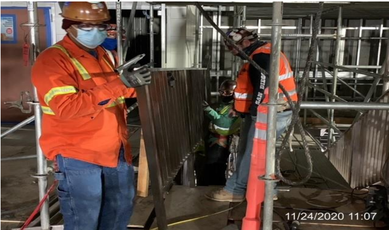
EXPO STATION – Installing guardrails for Staircase 2 from concourse to platform.
