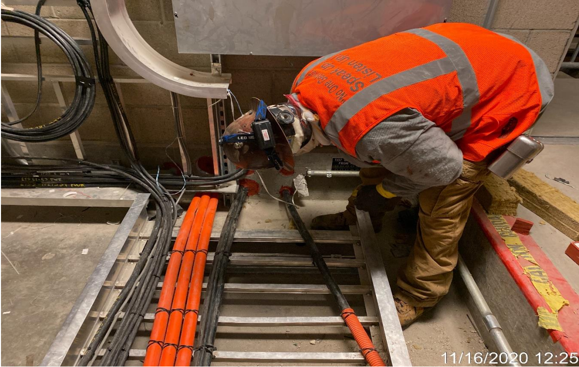
UG3 – Bielski applying firestop at Vernon cable room south.
