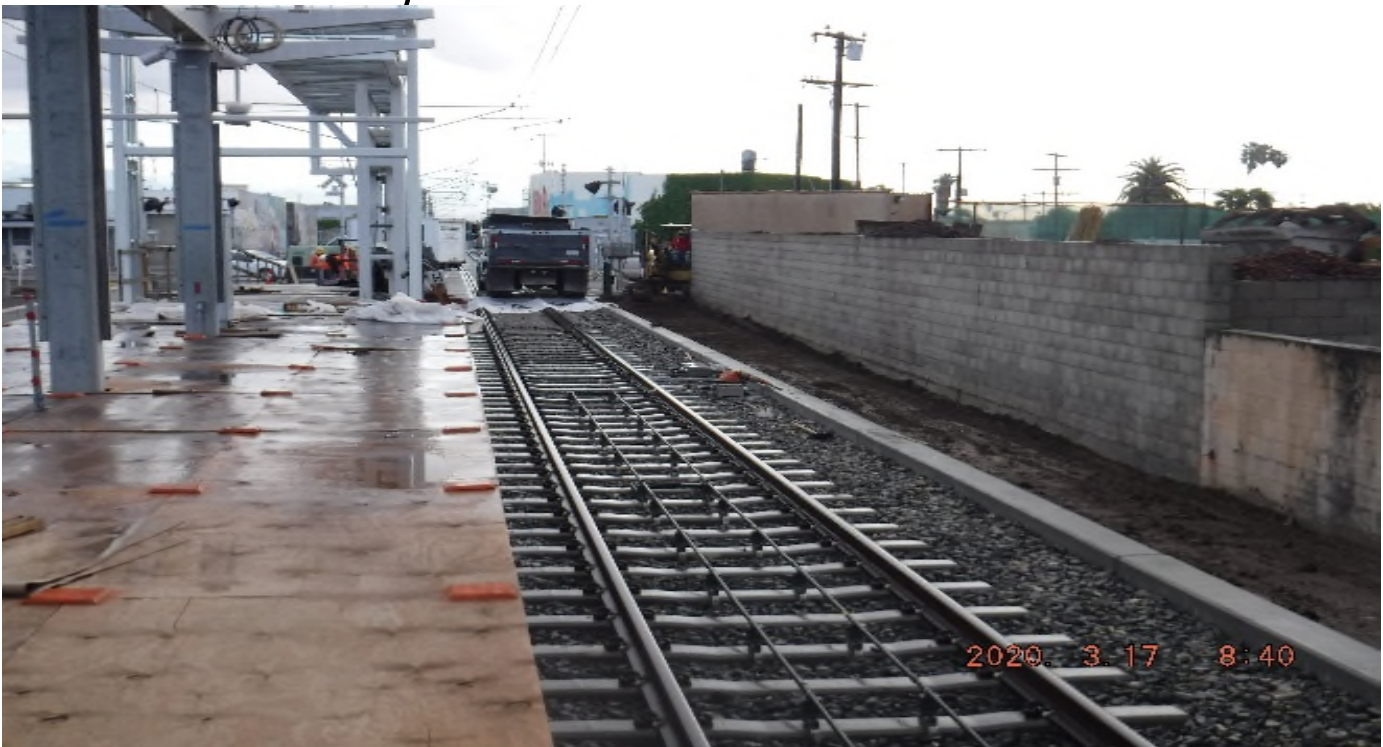
Florence/West – STA 265+00 TK#4.NB looking north – grading work outside ballast wall.
