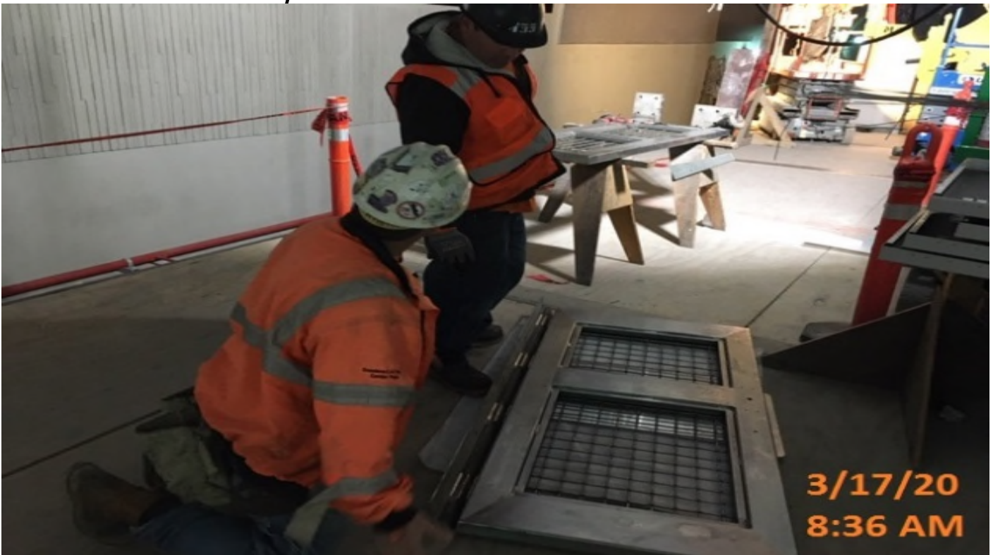
Crenshaw/Vernon - WSCC crew installing mock-up gates at platform level
