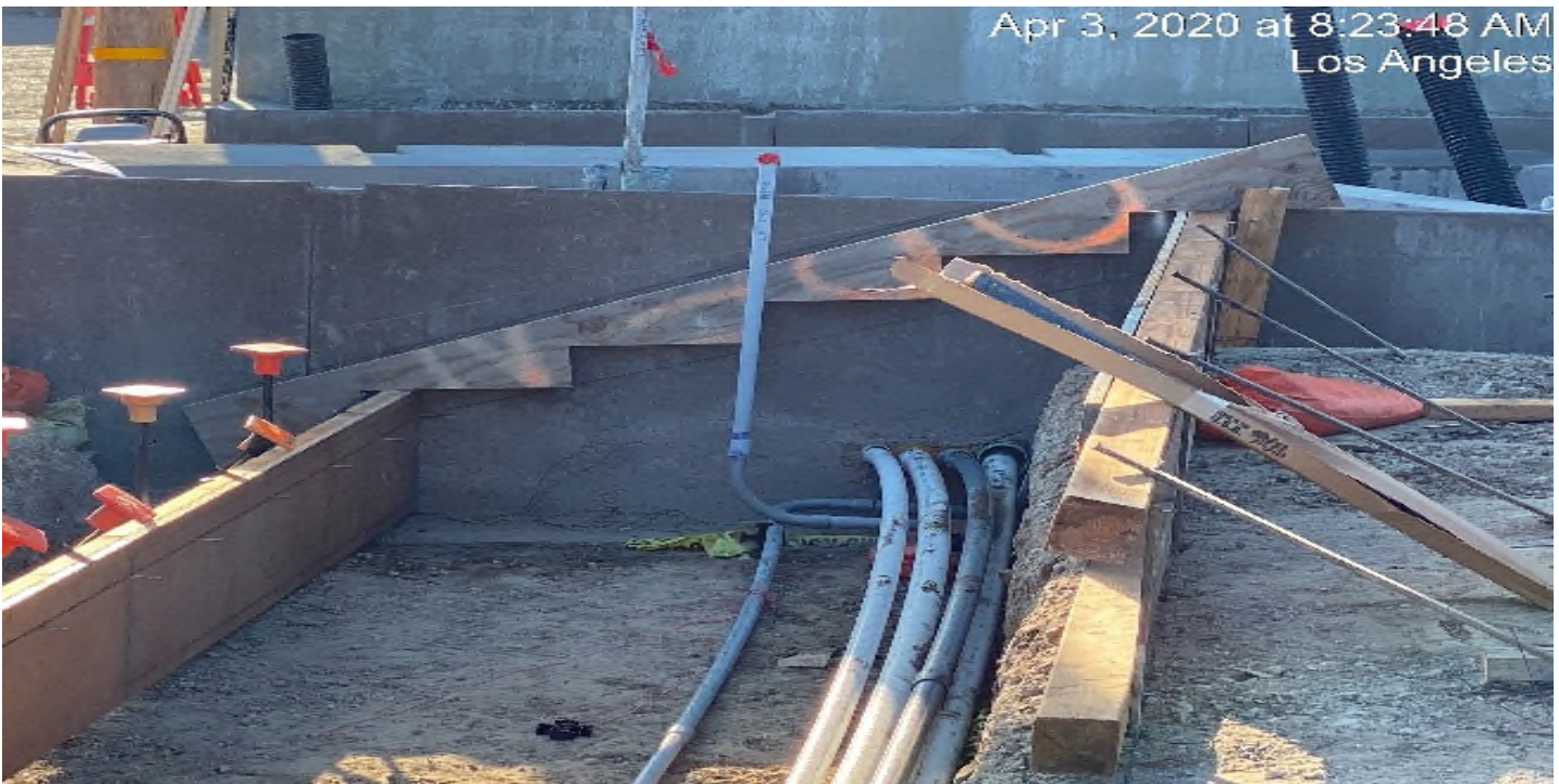
Crenshaw/Vernon - WSCC placing forms for stair risers at Vernon.
