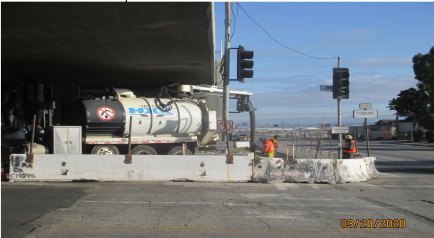
111 th Street – Potholing for utilities at 111thstreet.
