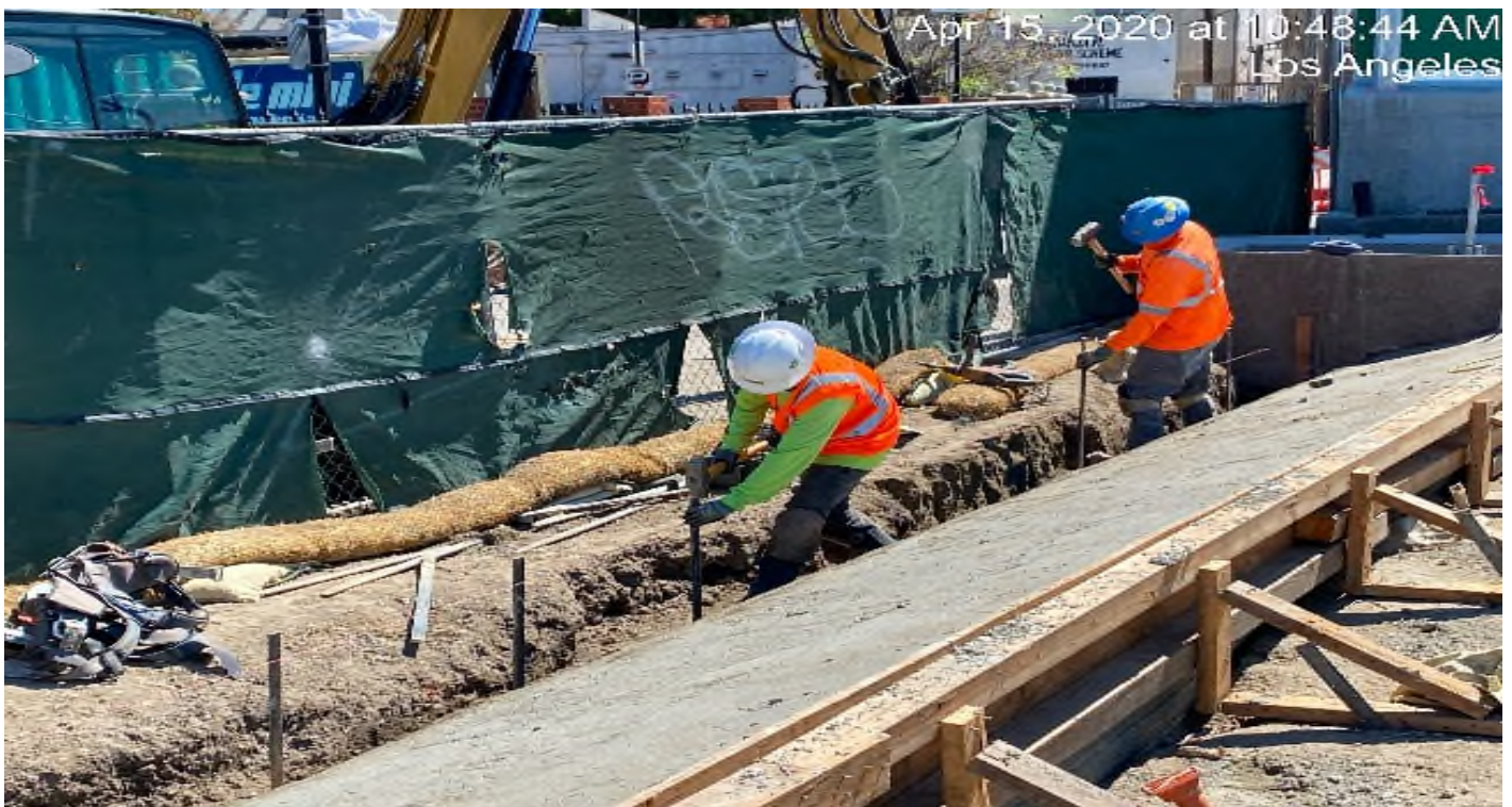
Crenshaw/Vernon - WSCC placing string line for formwork at Vernon.
