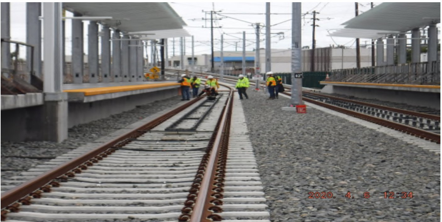
Florence/Hindry – STA 135+60 TK#4-NB looking south – checking rail grinding profile Hindry Station.
