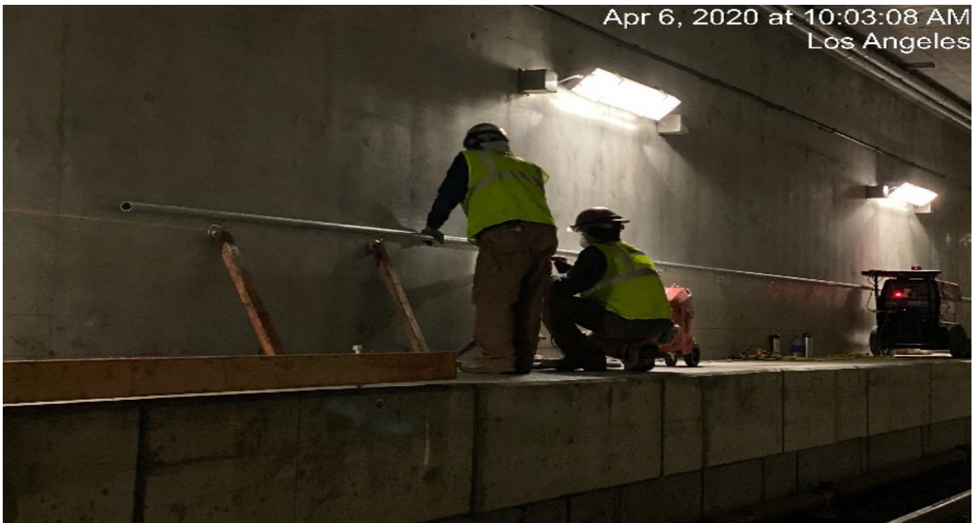
UG3 – MC Mahon installing handrail SB UG-3.
