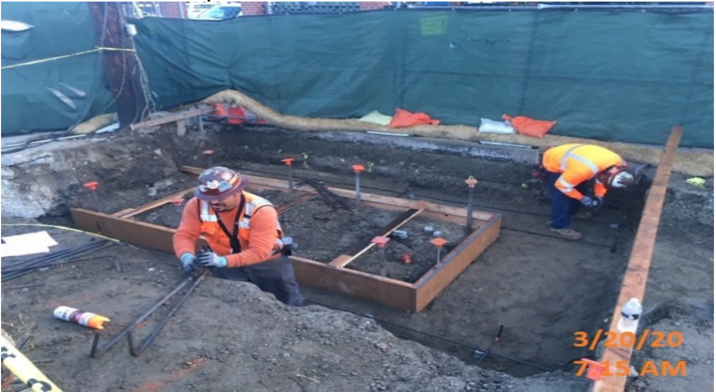
Crenshaw/Vernon - IRP installing rebar for planter wall and footings.
