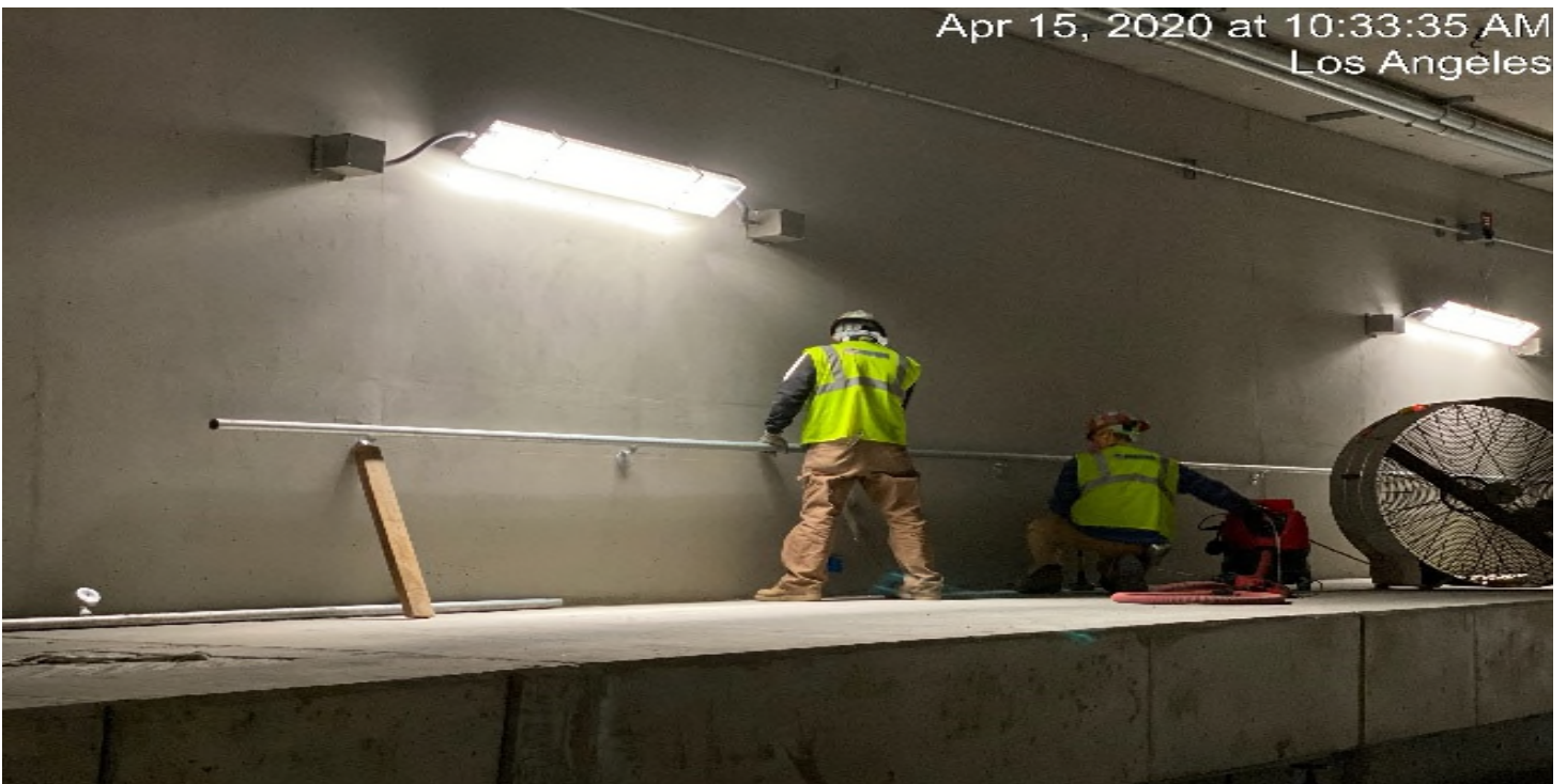
UG4 – McMahon layout for hand rail at UG-4.
