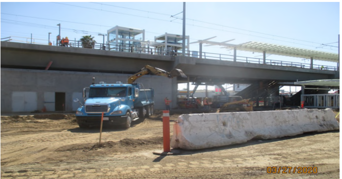
Aviation/Century – Subgrade grading and removals at the Aviation Station plaza area
