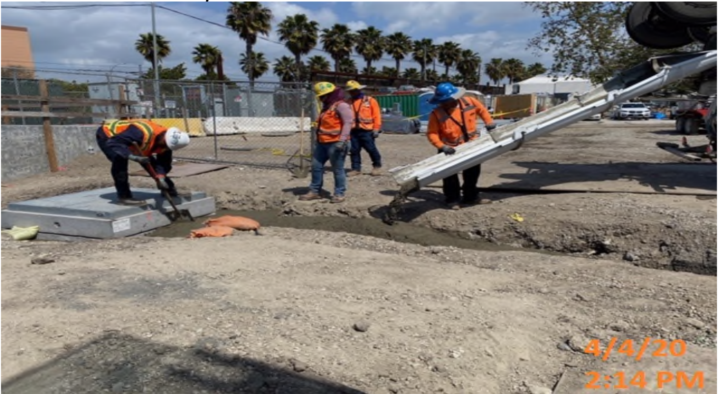
Crenshaw/Expo - EXPO – WSCC crew placing slurry backfill around electrical vault.
