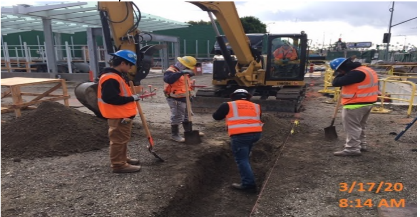
Crenshaw/Vernon - WSCC continue excavating trench for bollards.
