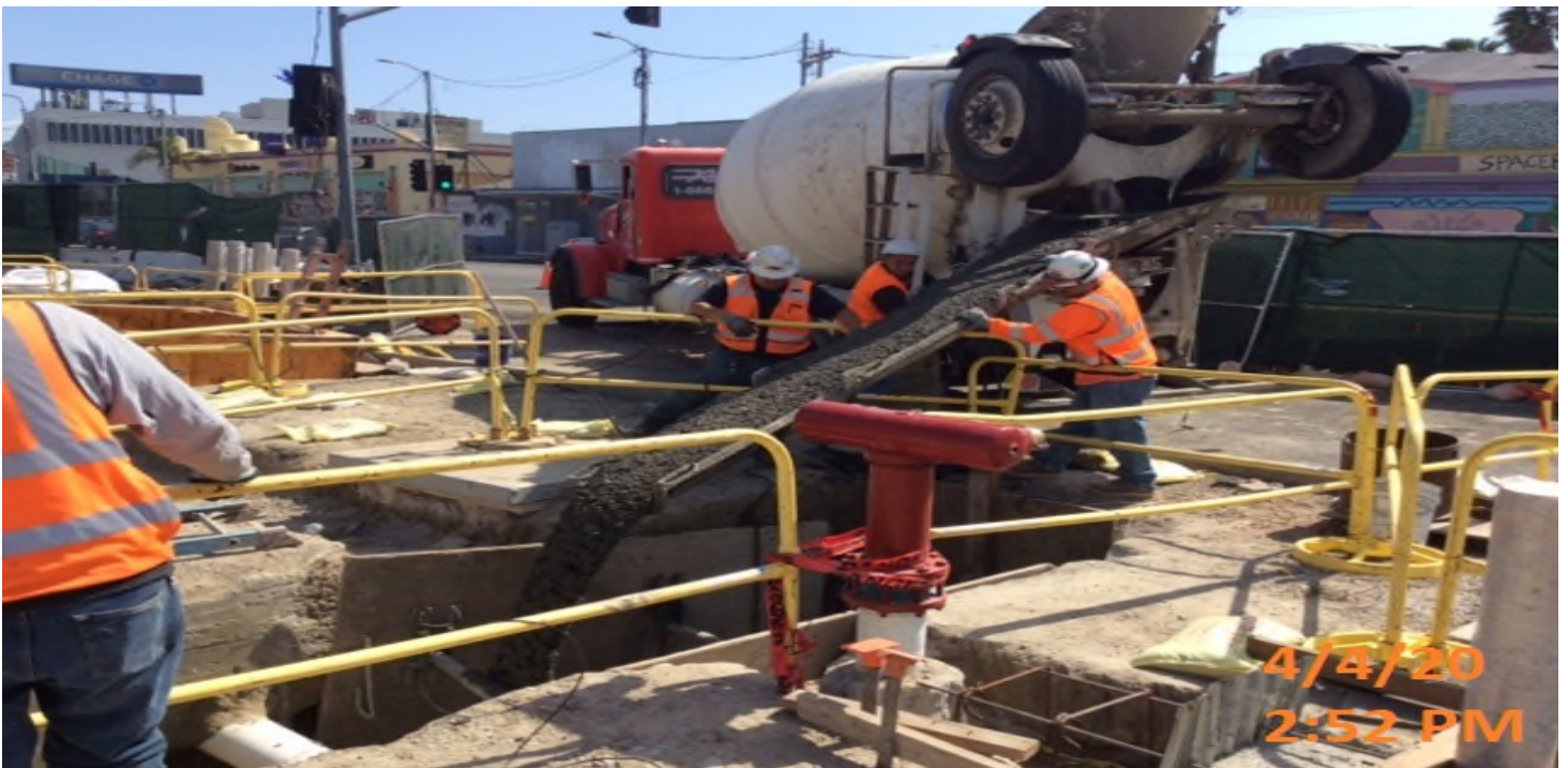
Crenshaw/Vernon - VERNON – WSCC crew placing 4” protective concrete slab over HCR membrane.
