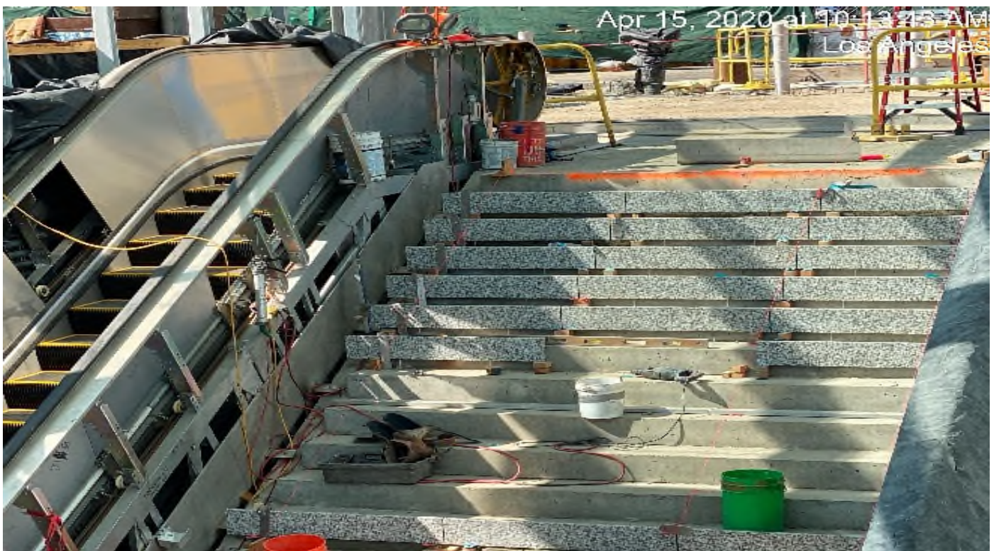
Crenshaw/Vernon - Carrera placing stair treads at Vernon.
