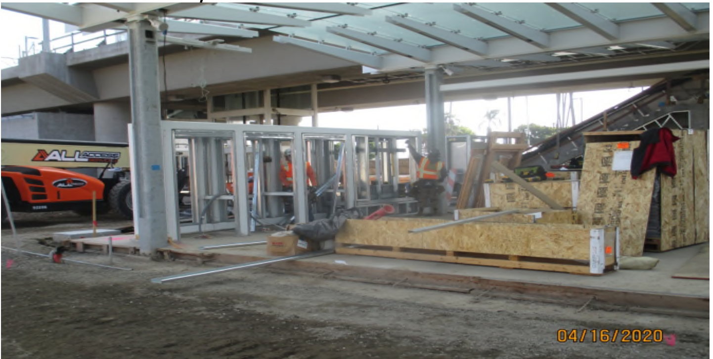
Aviation/Century – Metal stud framing at the Aviation Station ticket kiosk.
