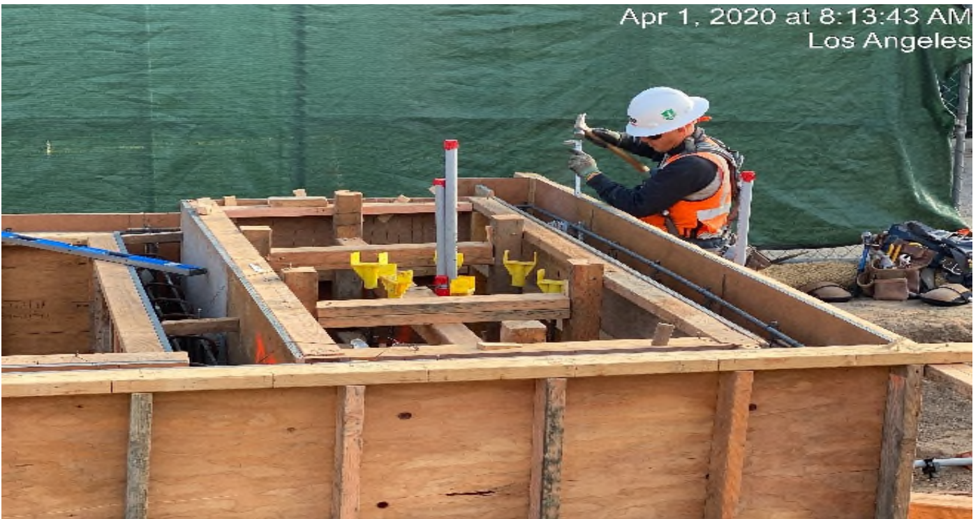
Crenshaw/Vernon - WSCC placing forms for planter box at Vernon.
