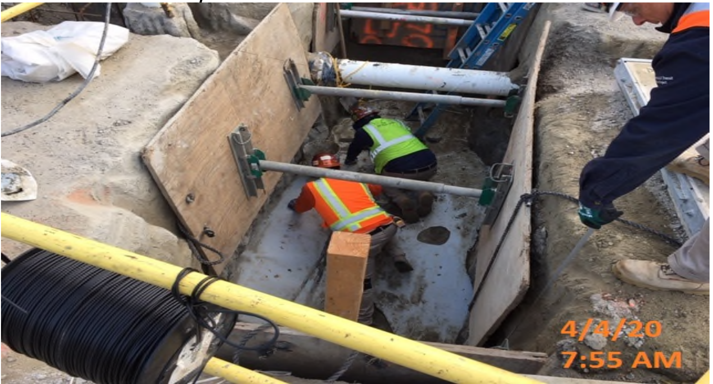
Crenshaw/Vernon - VERNON – ECA performing HCR membrane repair.
