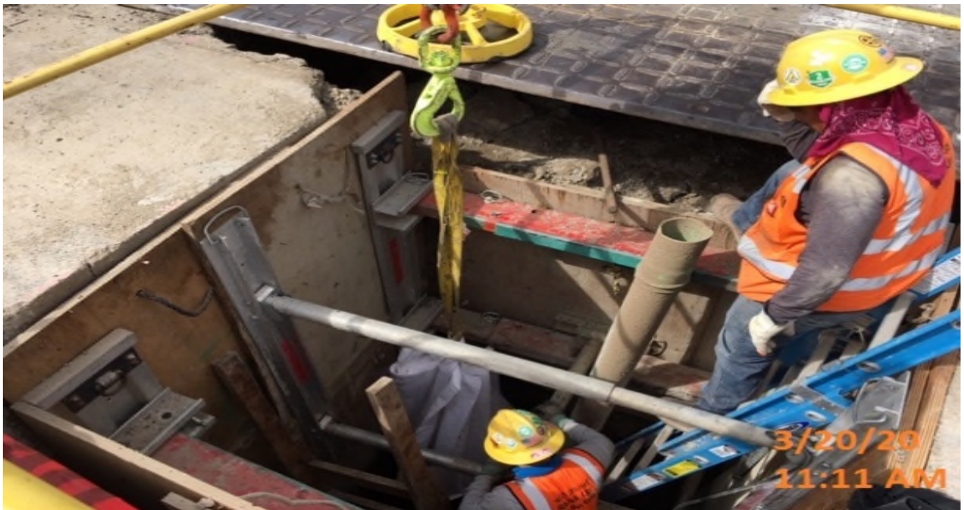
Crenshaw/MLK - WSCC crew continue exploratory excavation into station leak.
