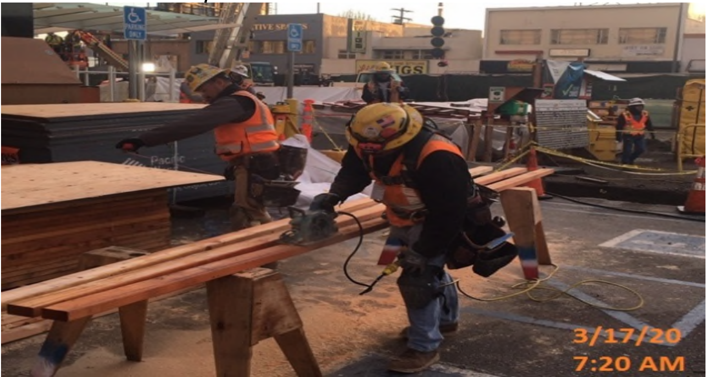
Crenshaw/MLK - WSCC crew building formwork for planter wall.
