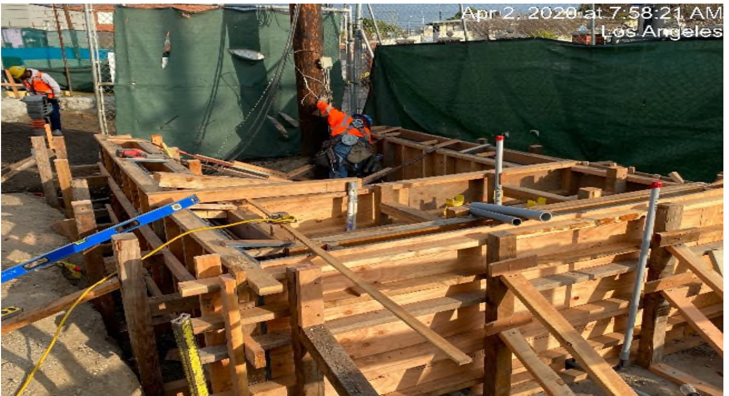
Crenshaw/Vernon - WSCC placing forms for planter box at Vernon.
