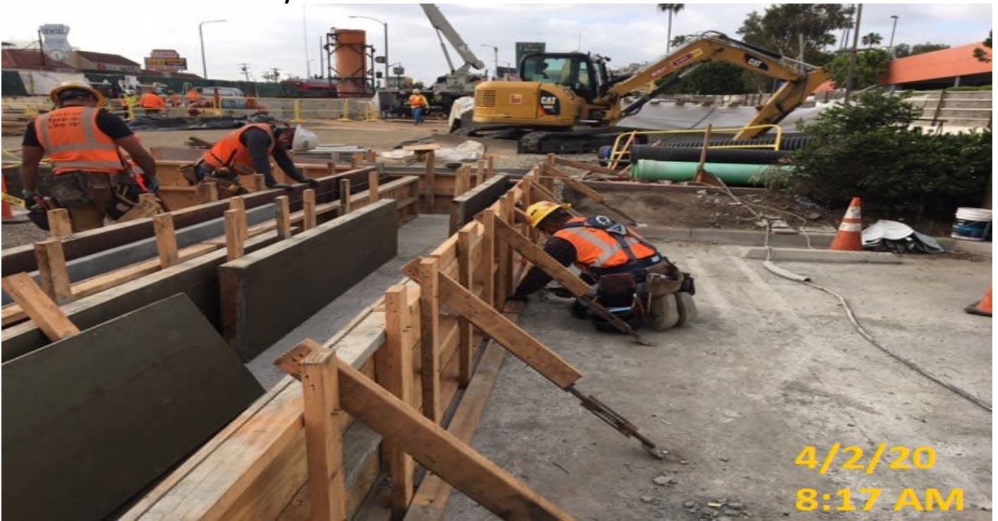
Crenshaw/MLK - MLK – WSCC crew building formwork for west planter wall.
