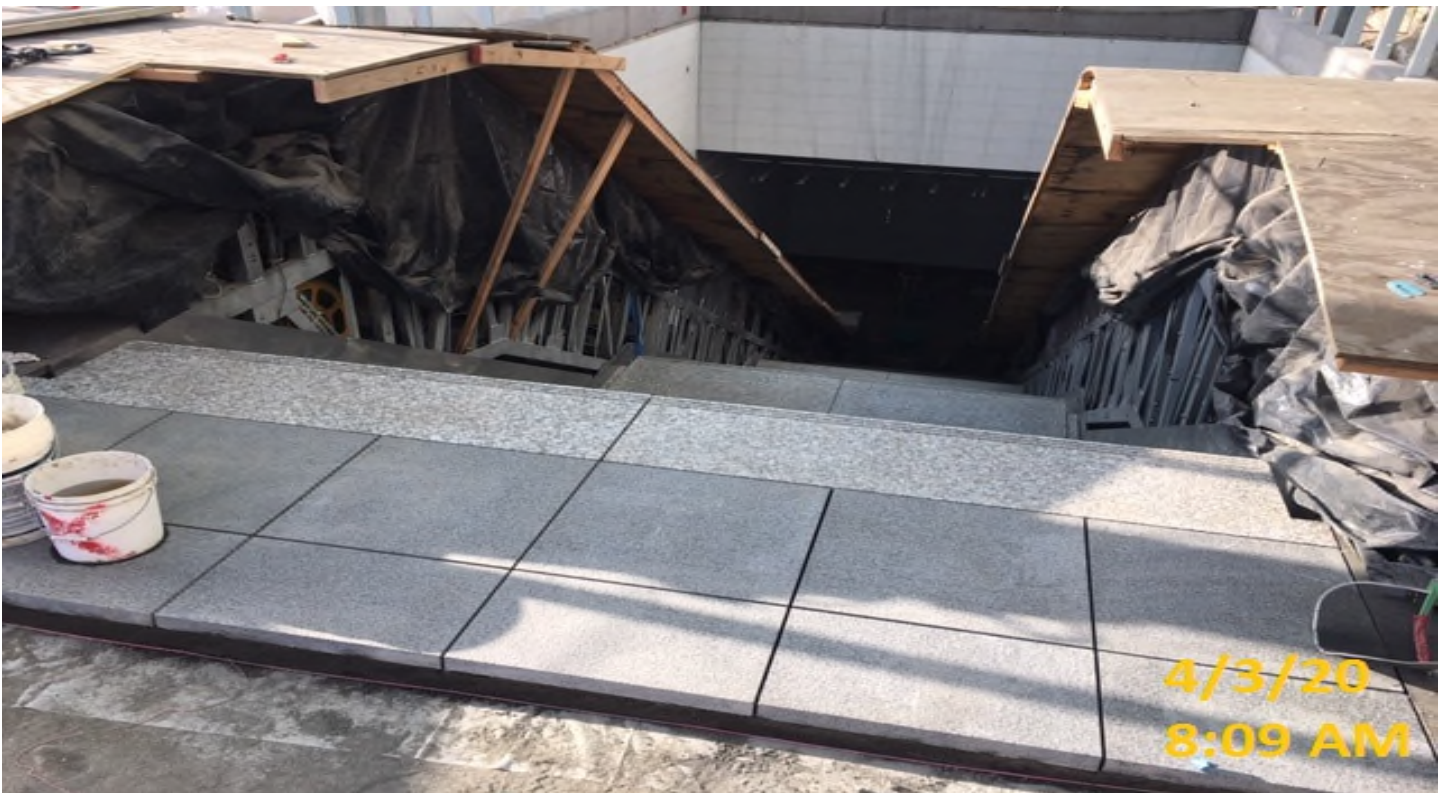
Crenshaw/MLK - MLK – Carrera Marble completing sections of landing at main entrance.
