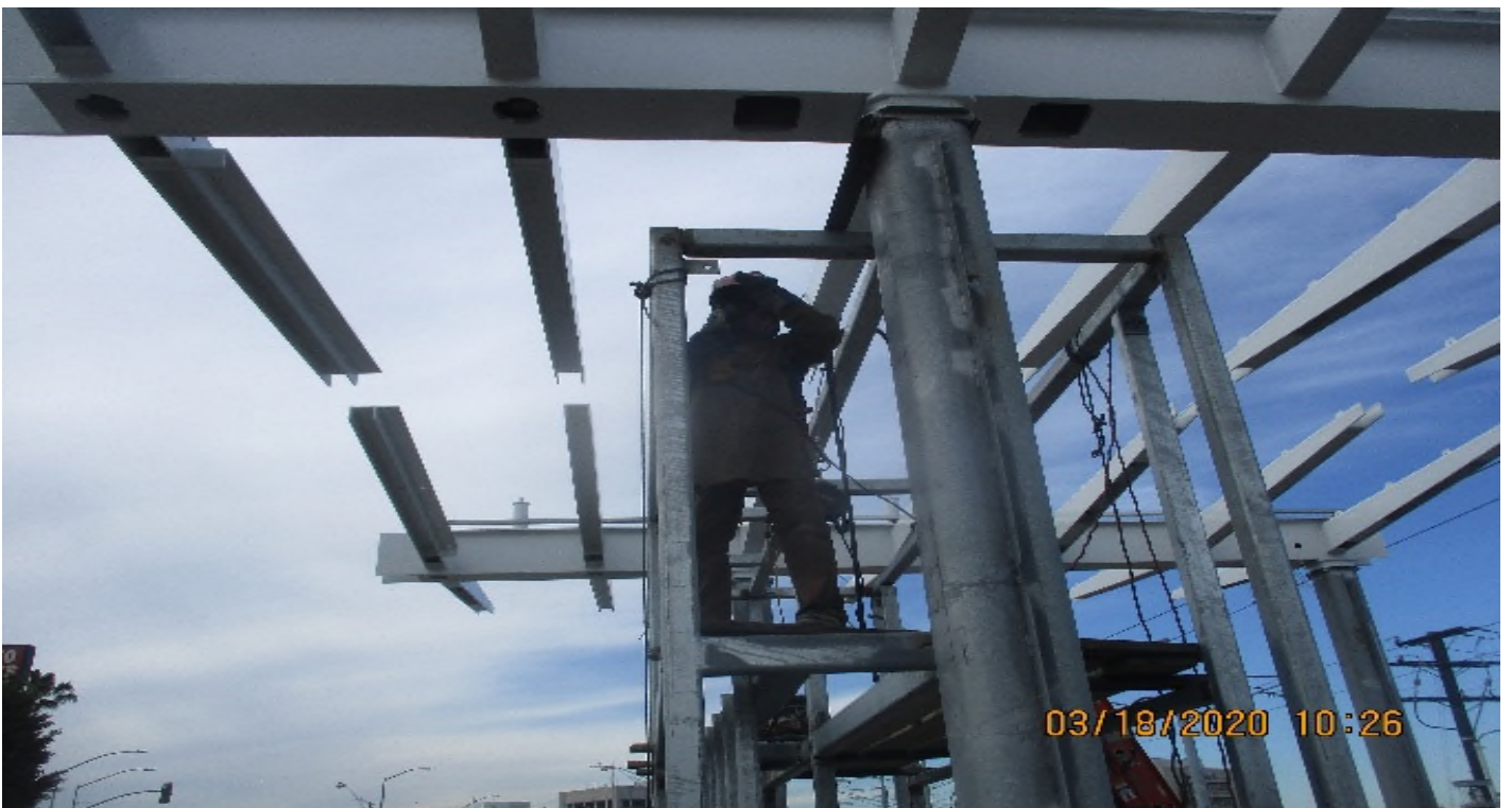
Florence/Brea – McMahon Weld beams at S-ticket pavilion at La Brea.
