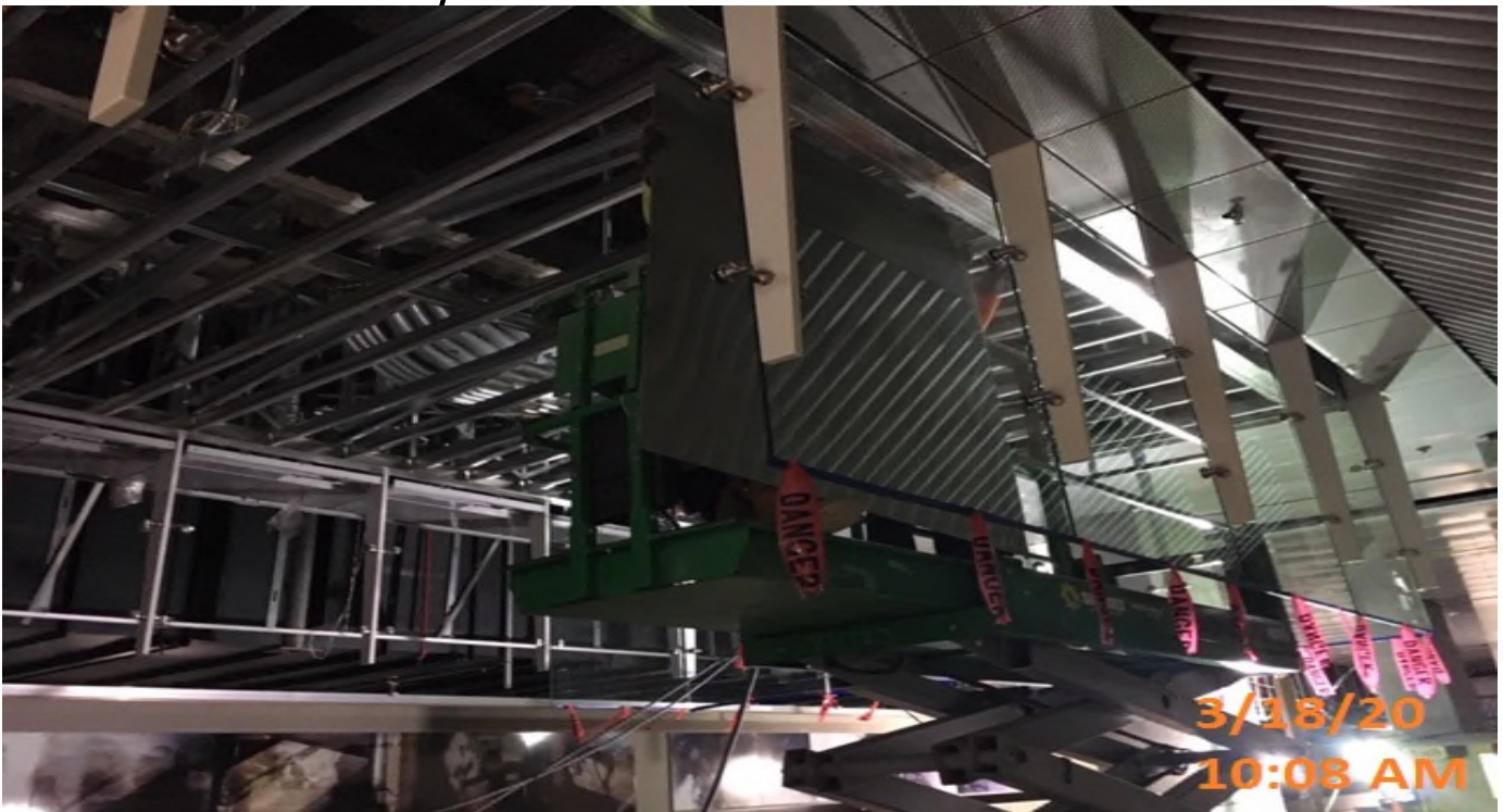
Crenshaw/Vernon - VNSM crew installing stainless steel panels adjacent to down stands.
