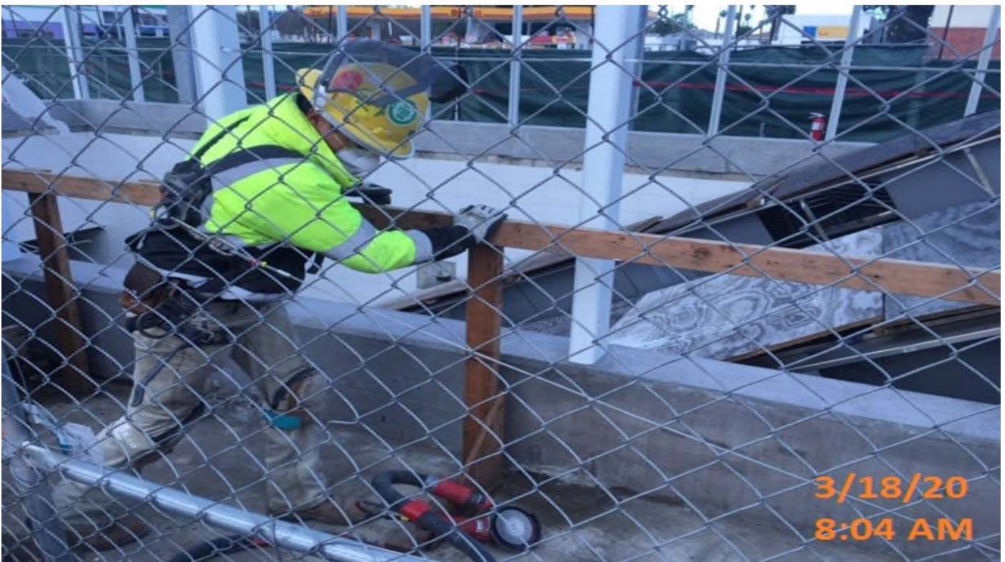
Crenshaw/Expo - WSCC crew at main entrance surface finishing wind screen curb.
