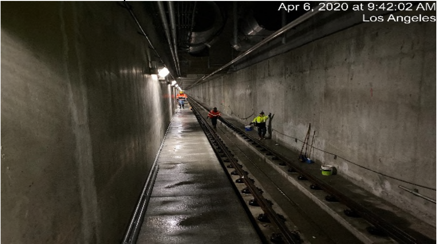
UG3 – WSCC washing floors at UG-3.
