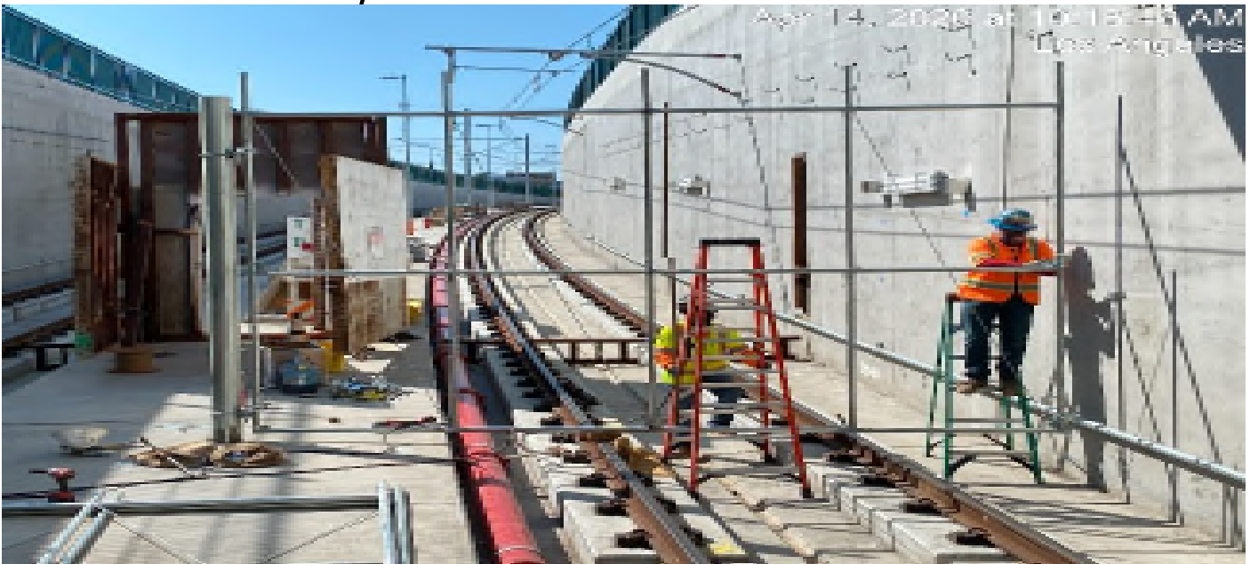
UG4 – Installing gates at the south end portal entrance.
