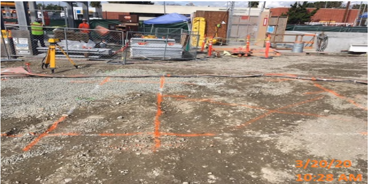
Crenshaw/Expo - WSCC setting gridlines for excavation and placement of electrical vaults.
