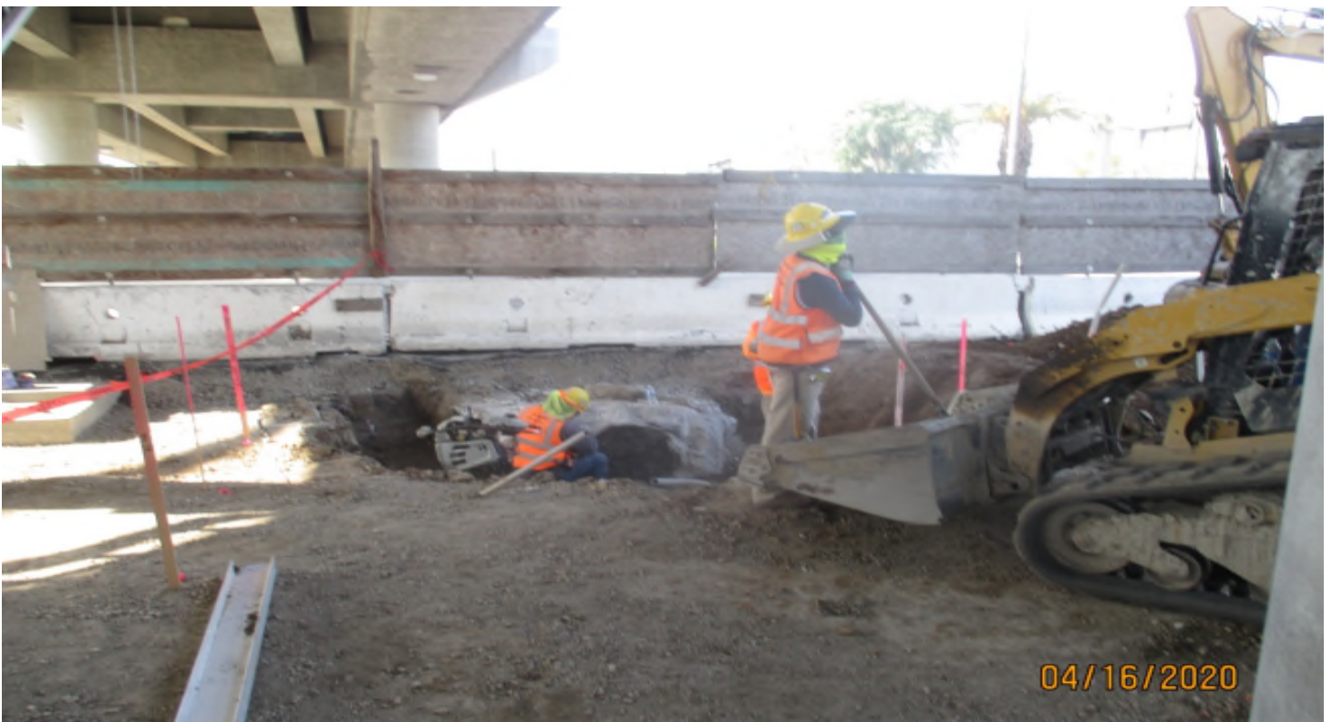
Aviation/Century – Abandoning a storm drain line at aviation Station.
