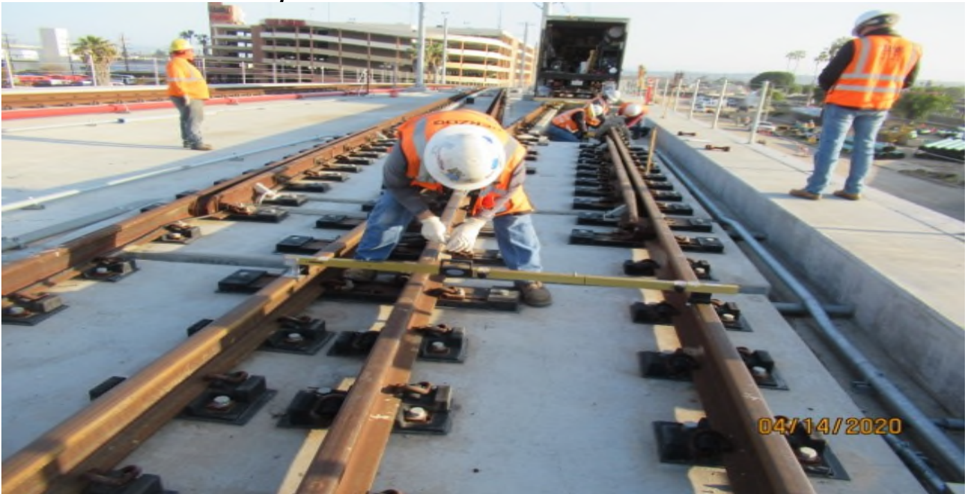
Aviation/Century – HCC installing Shim plates on 10K1LH XO on Century-Aviation bridge NB #4 track STA 70+50 (looking north) Rework
