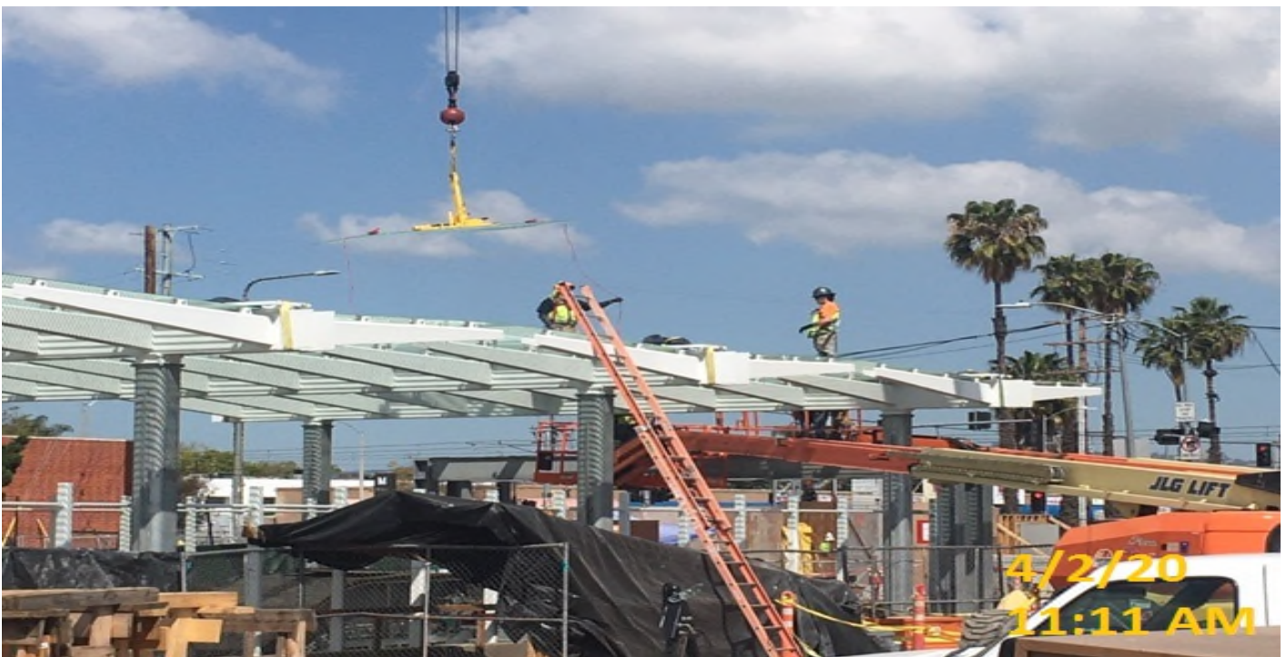
Crenshaw/Expo - EXPO – Giroux Glass installing glass panels at main entrance canopy.
