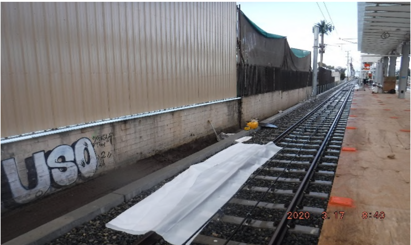
Florence/West – STA 265+00 TK#4.NB looking north – grading work outside ballast wall.
