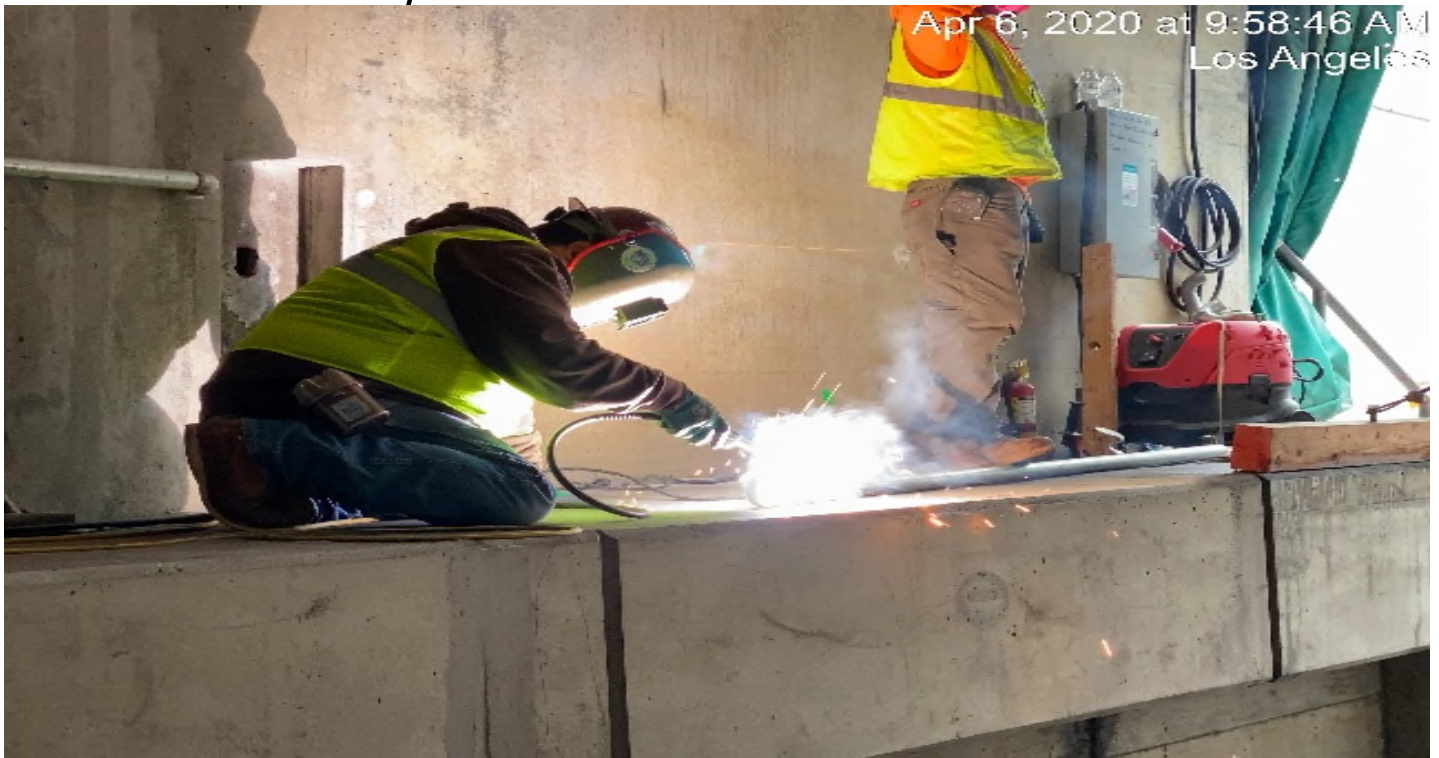
UG3 – MC Mahon welding handrail NB UG-3.
