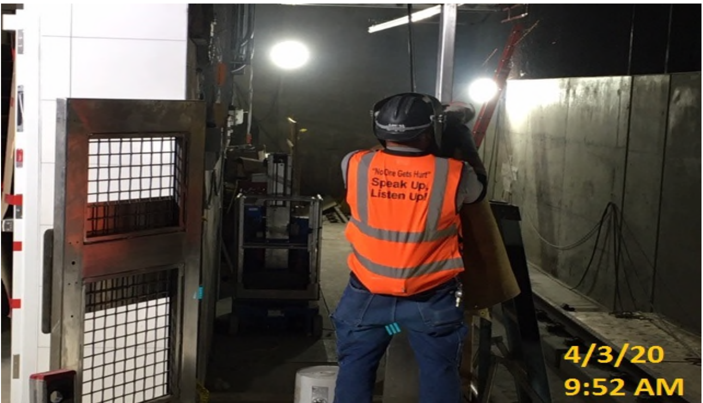
Crenshaw/Expo - EXPO – WSCC ironworkers grinding platform end gates.
