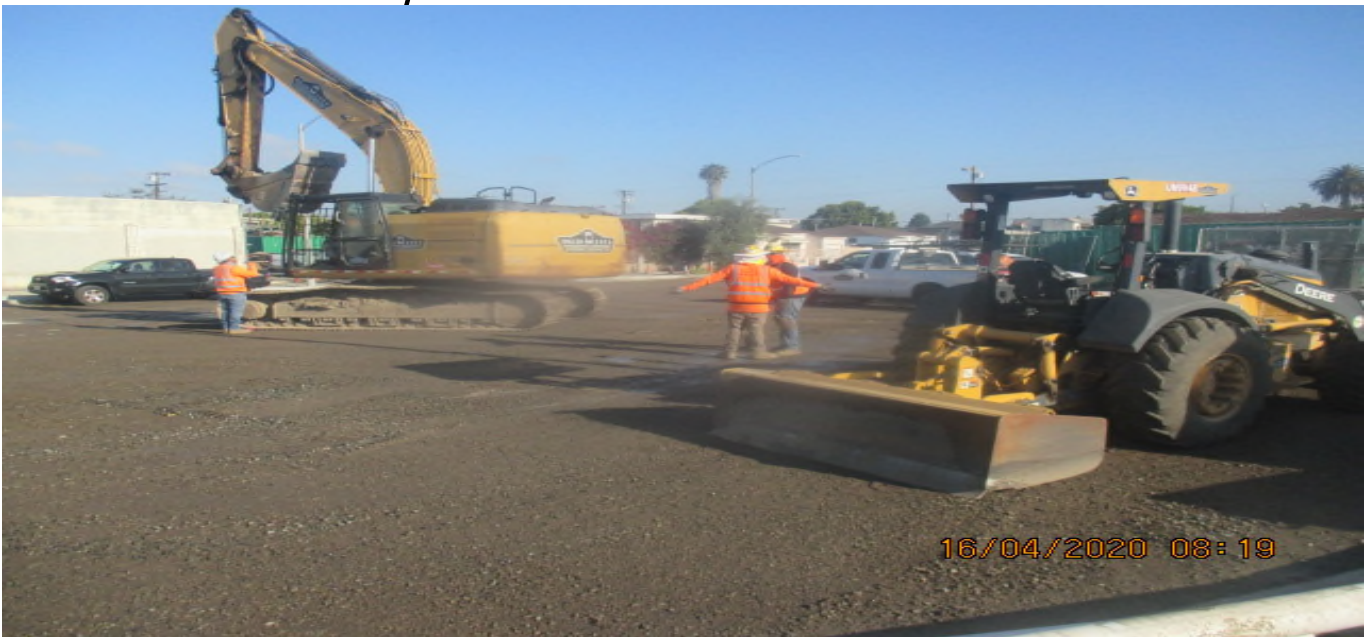
UG3 – Finalizing grading/compaction for the new Cul-de-sac at North Victoria Ave. 4/16/20
