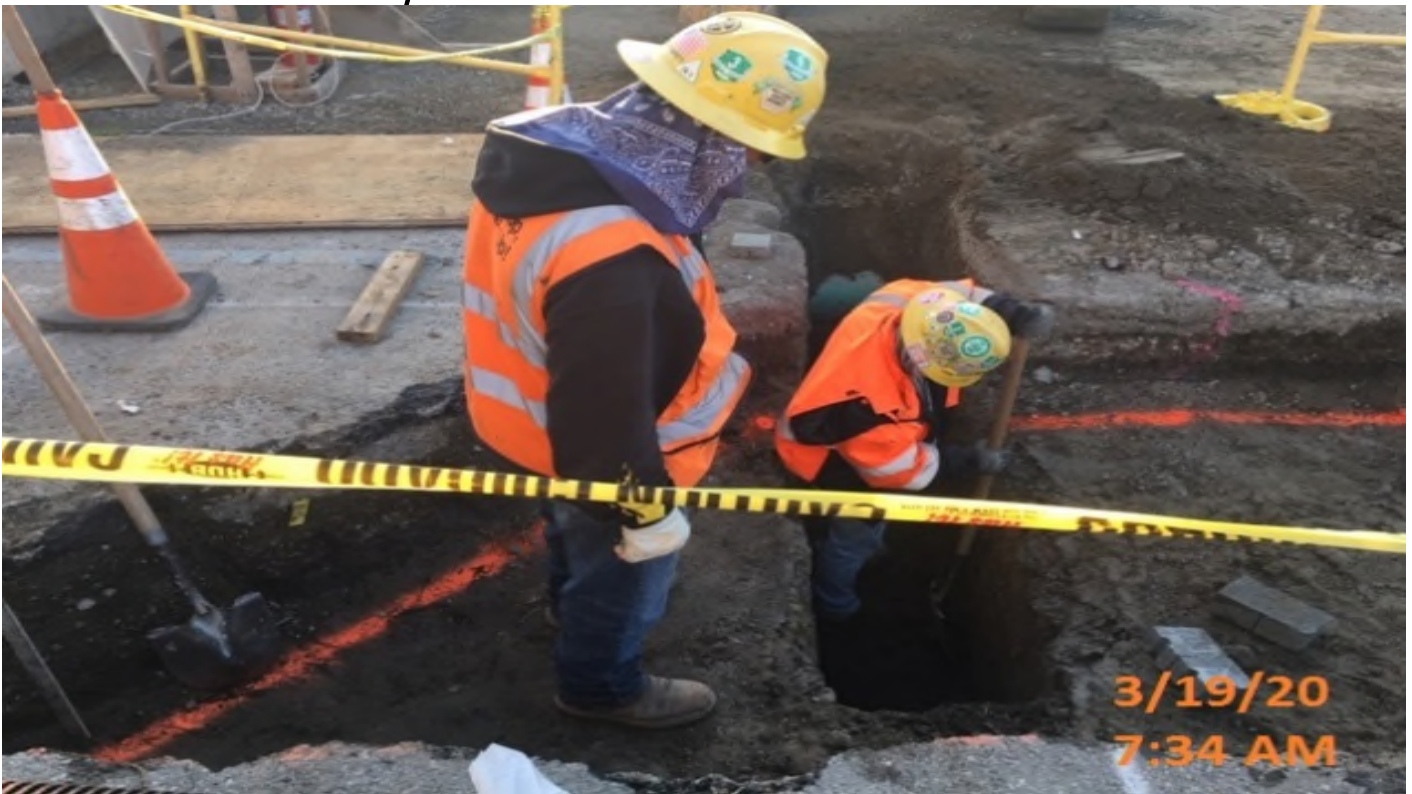
Crenshaw/MLK - WSCC crew hand excavating and setting drainage for planters.
