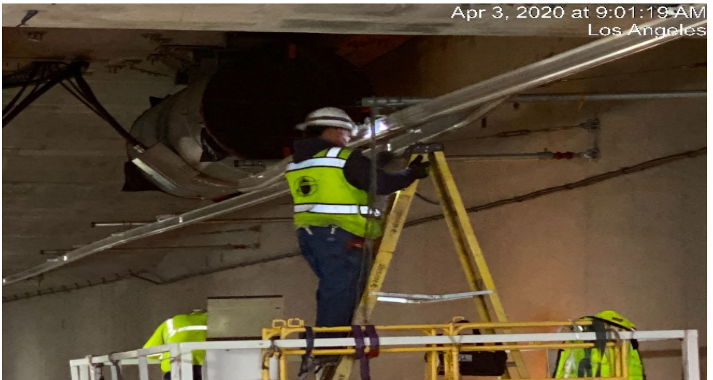
UG4 – LK Comstock adjusting OCS rail at UG-4.
