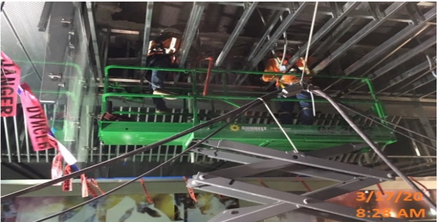
Crenshaw/Vernon - VNSM crew installing stainless steel clad panels.
