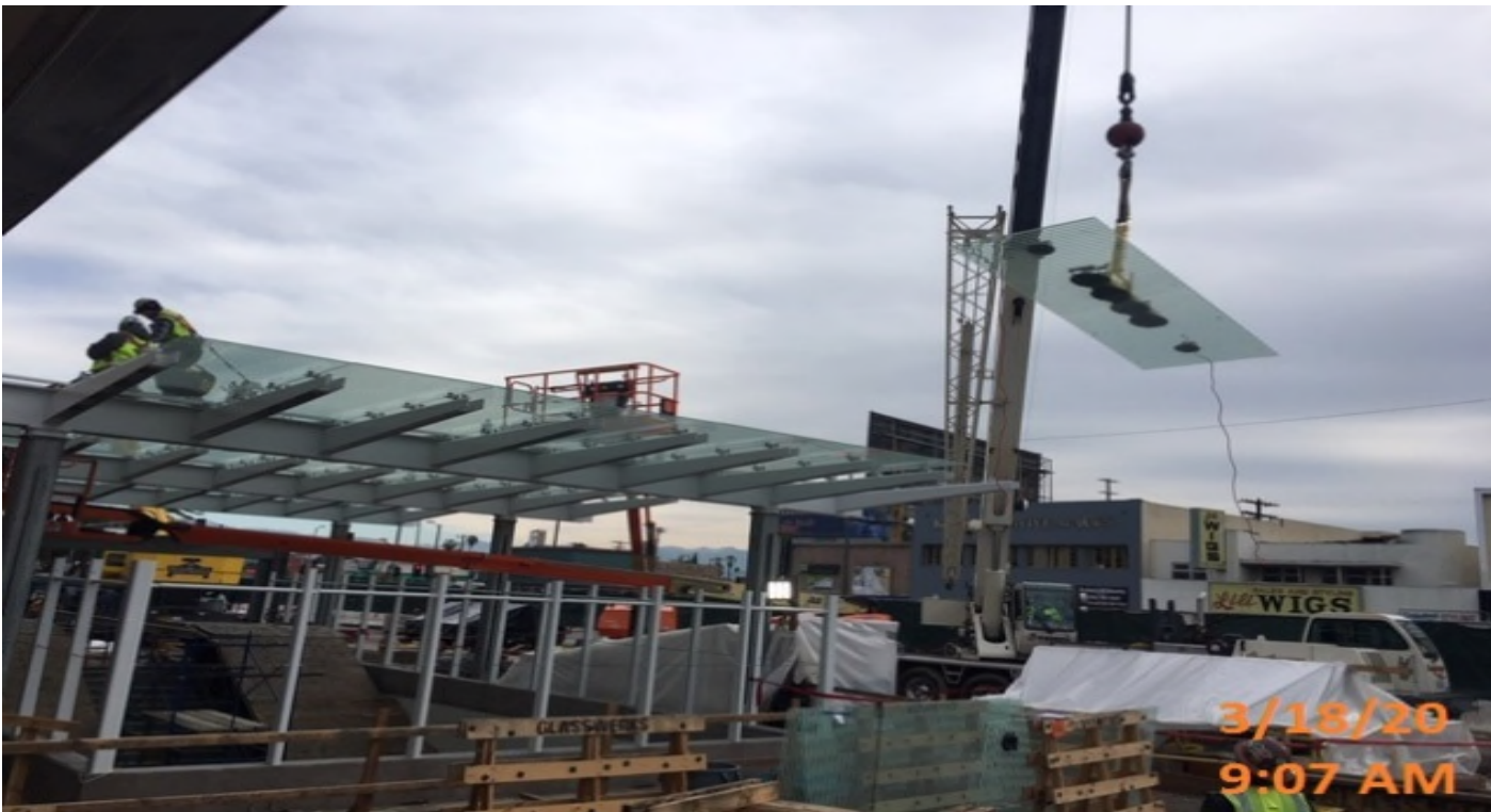
Crenshaw/MLK - Giroux Glass installing canopy glass panels at main entrance.
