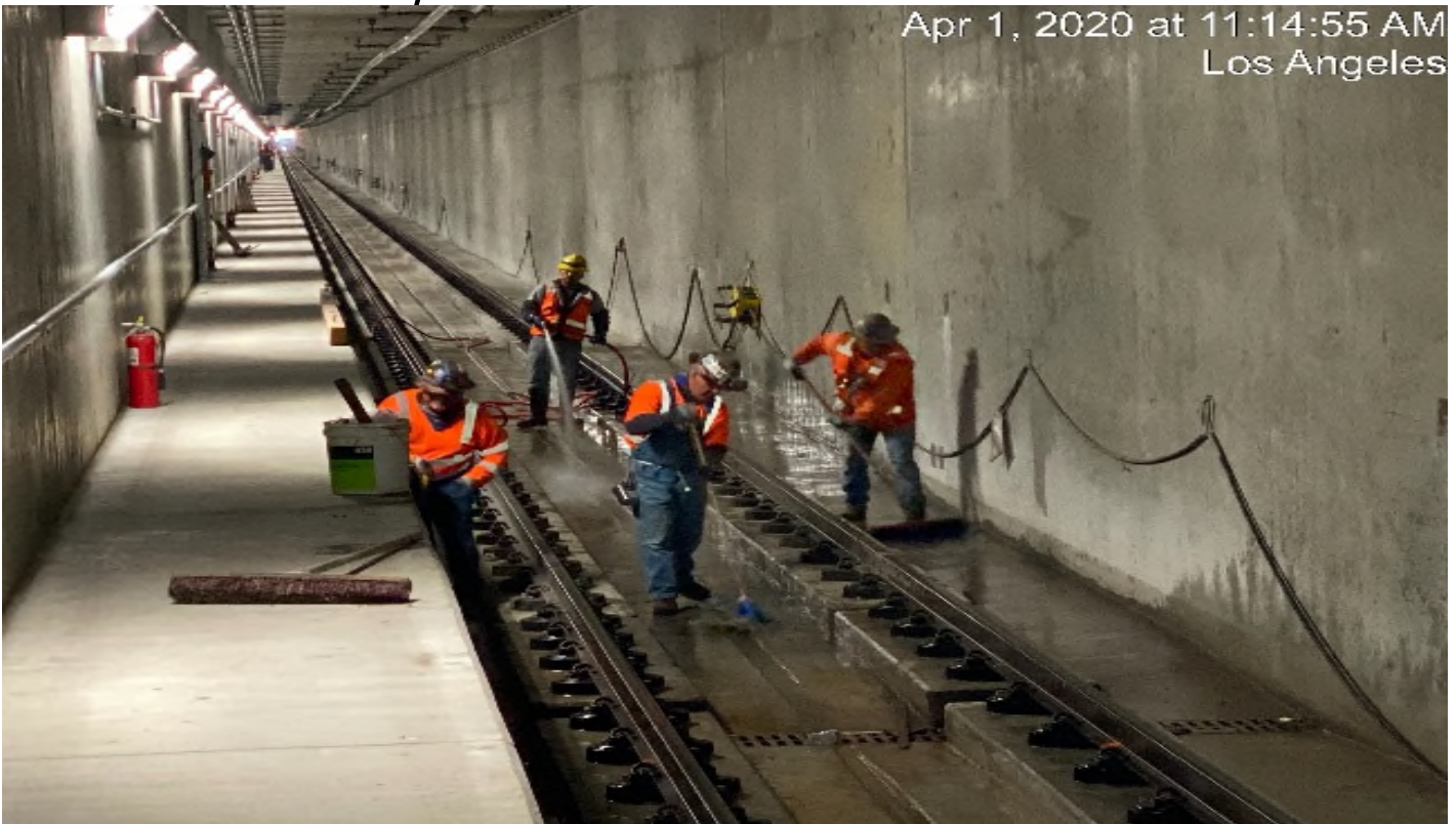
UG3 – WSCC scrubbing floors at UG-3.
