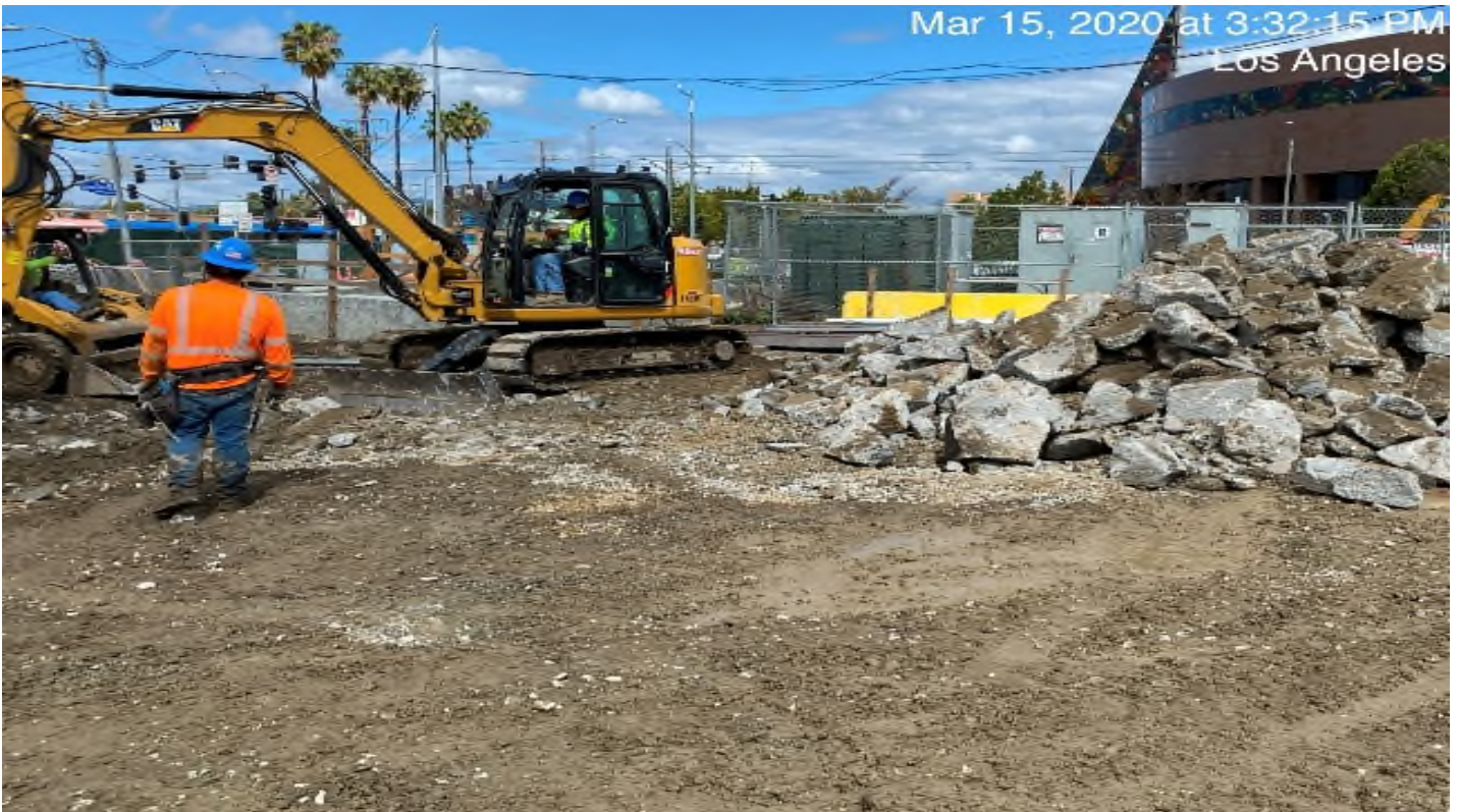
Crenshaw/Expo - WSCC excavating concrete slab at Expo yard.
