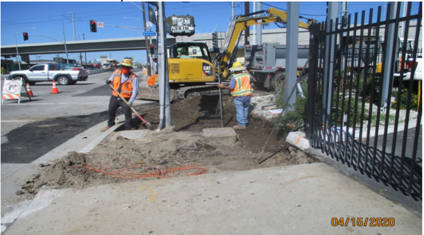
Manchester Bridge – Grading for the proposed new ADA ramp at Manchester.
