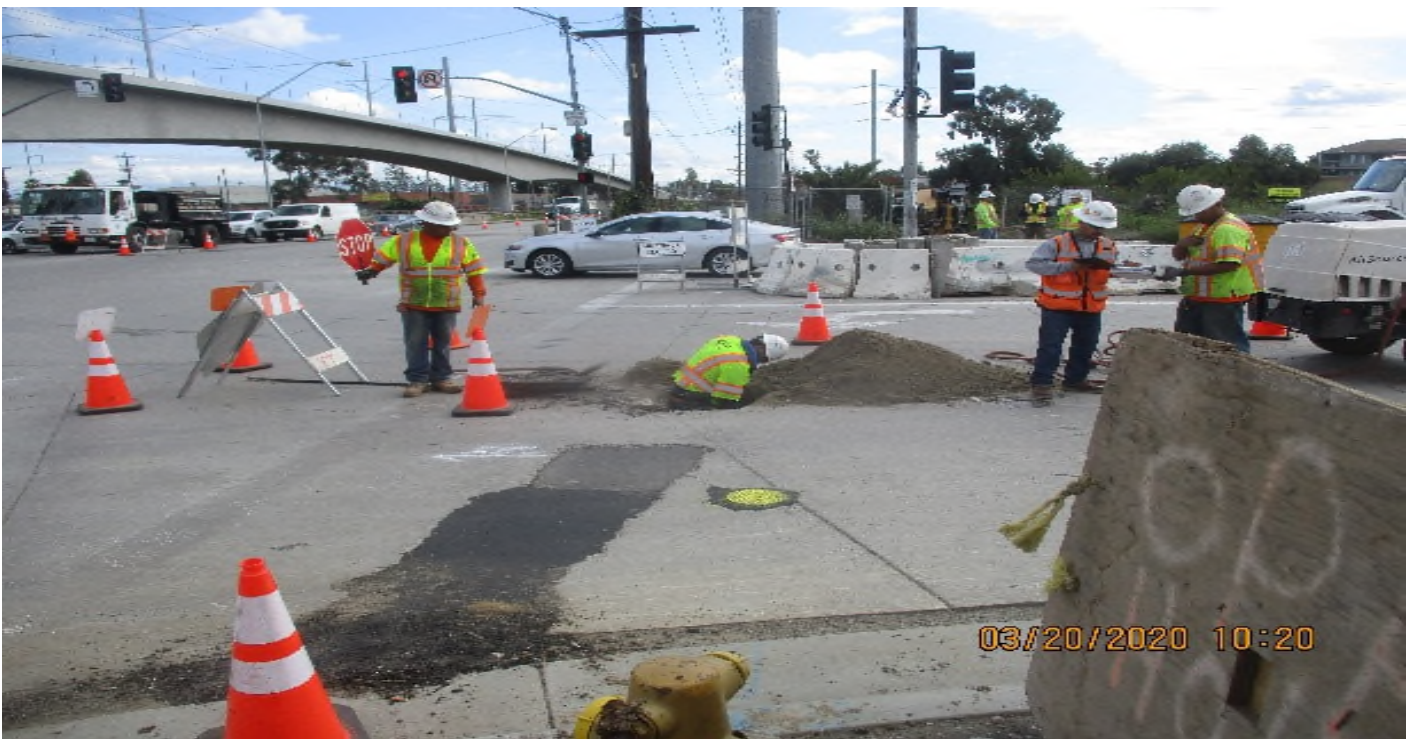
Aviation/Century – VT Electric Re directional bore conduit across Aviation.
