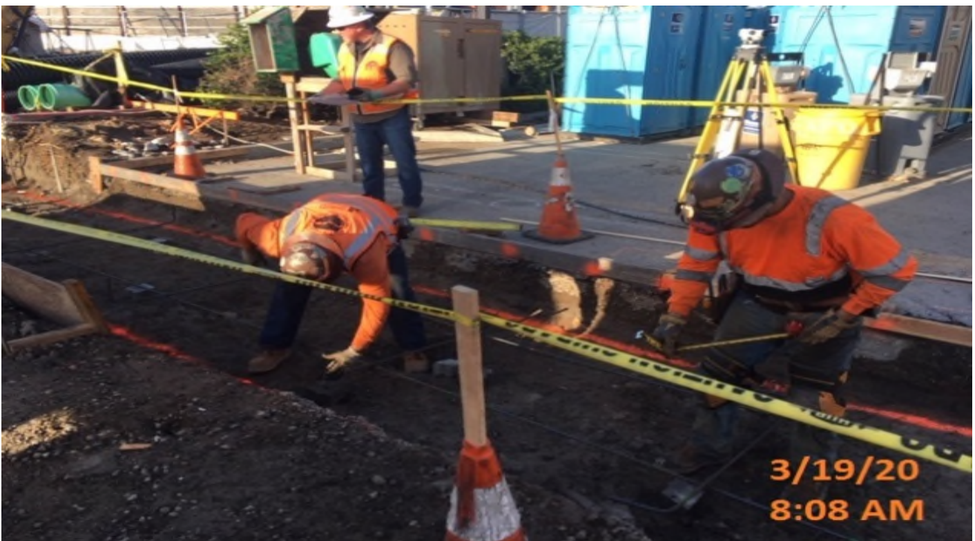
Crenshaw/MLK - IRP placing rebar for planter wall and footings
