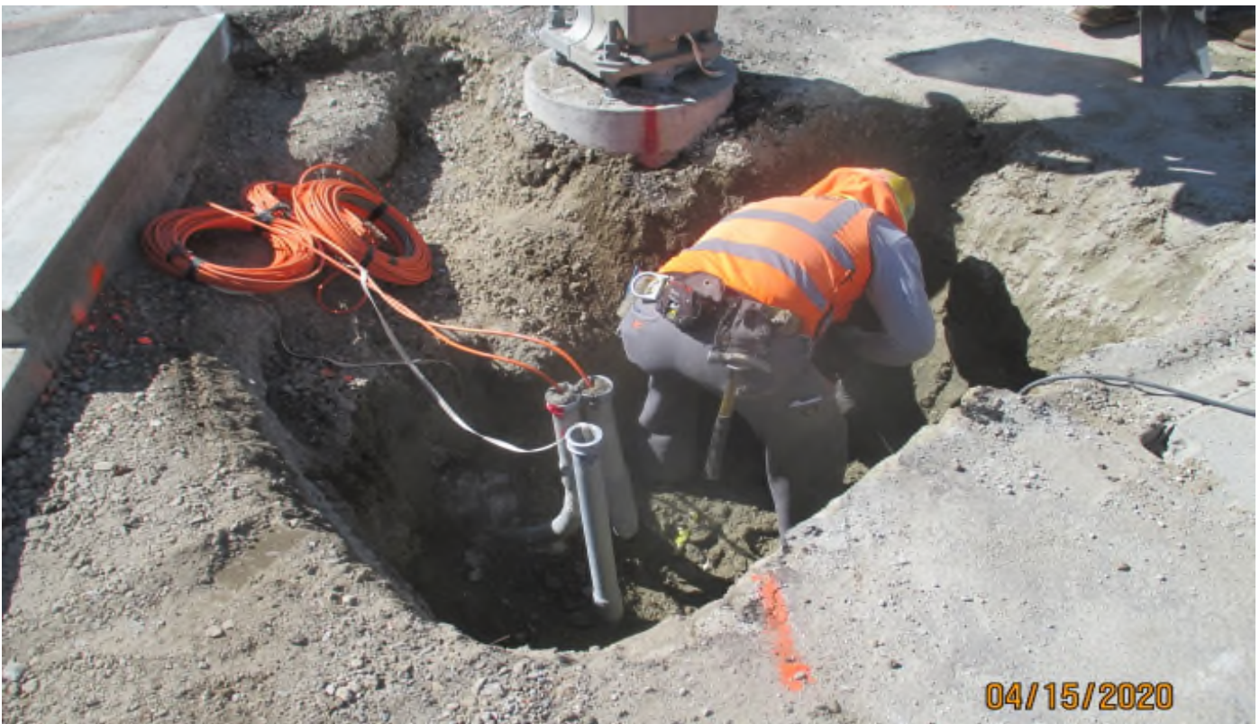
Florence/Hindry – Excavating to relocate a pull box at the Hindry crossing.
