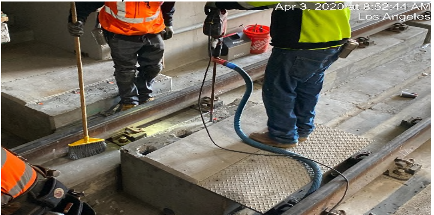
UG4 – WSCC adjusting diamond plates UG-4 sump walkway.
