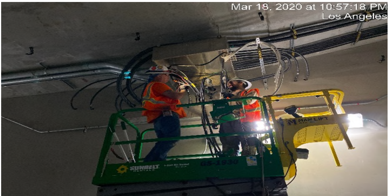
UG-4- DCD splicing wires in junction box southbound UG-4.
