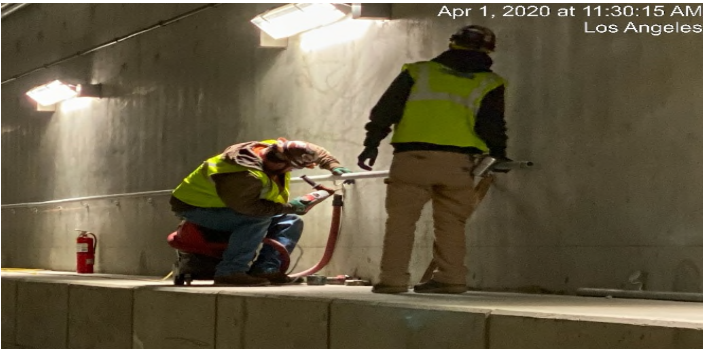
UG3 – McMahon installing hand rail at UG-3
