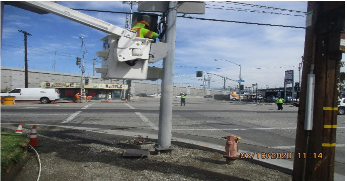
Manchester Bridge – Select Electric Shut down Intersection at Manchester.
