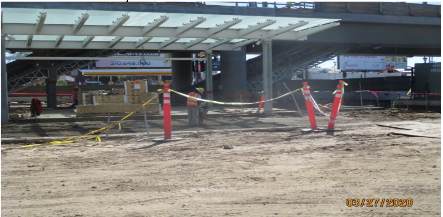
Aviation/Century – Subgrade compaction at the Aviation Station plaza area
