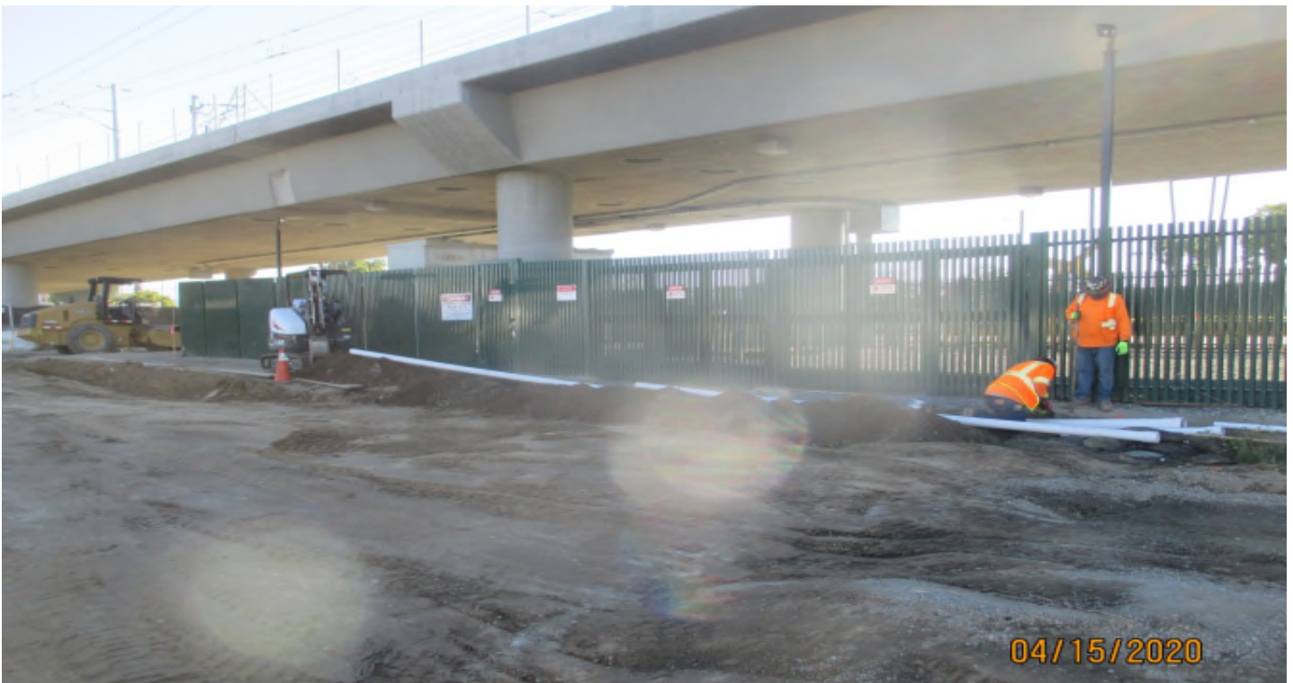
Aviation/Century – Irrigation pipe installation at the Aviation Station yard.
