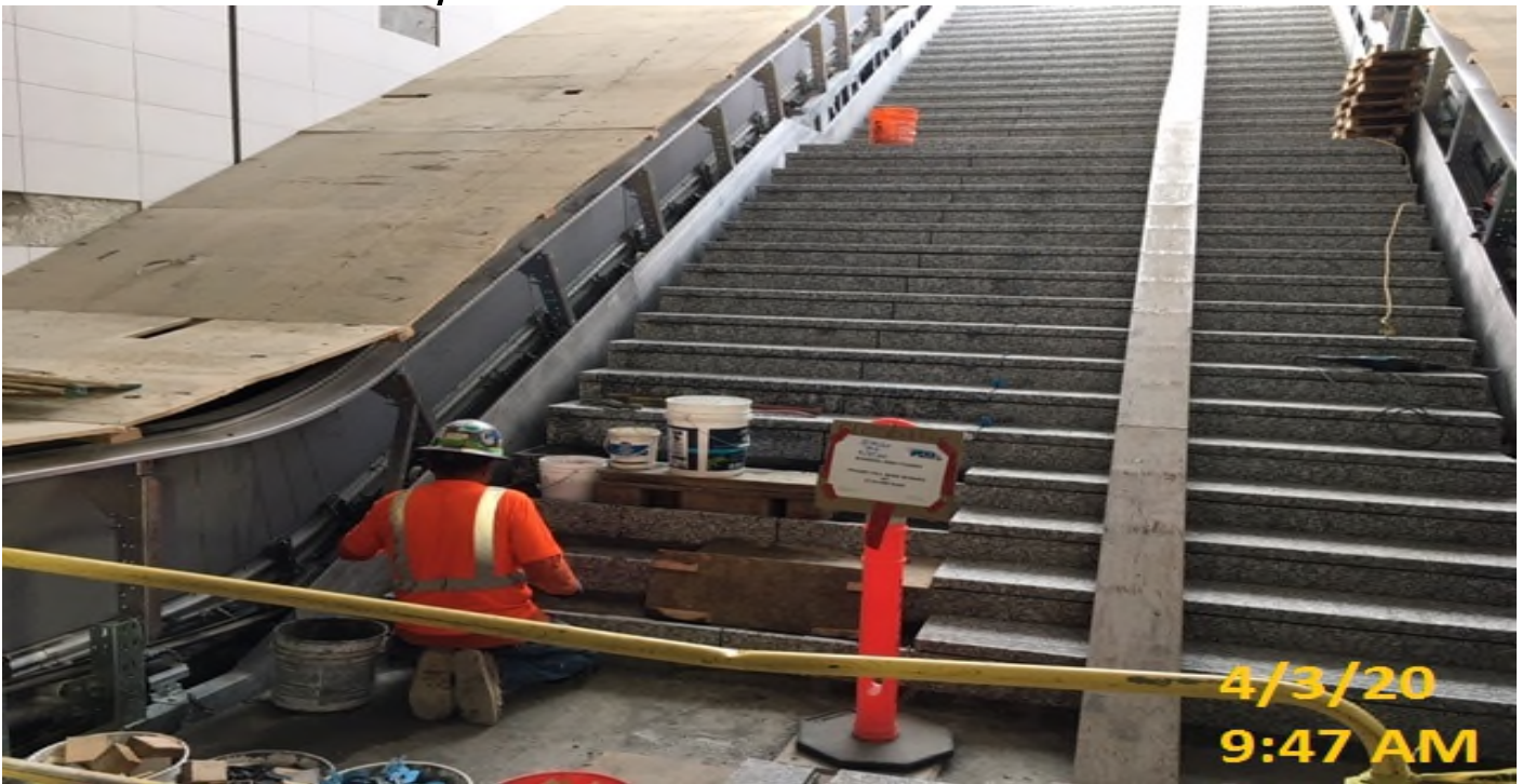
Crenshaw/Expo - EXPO – Carrera Marble continue installing treads at main staircase.
