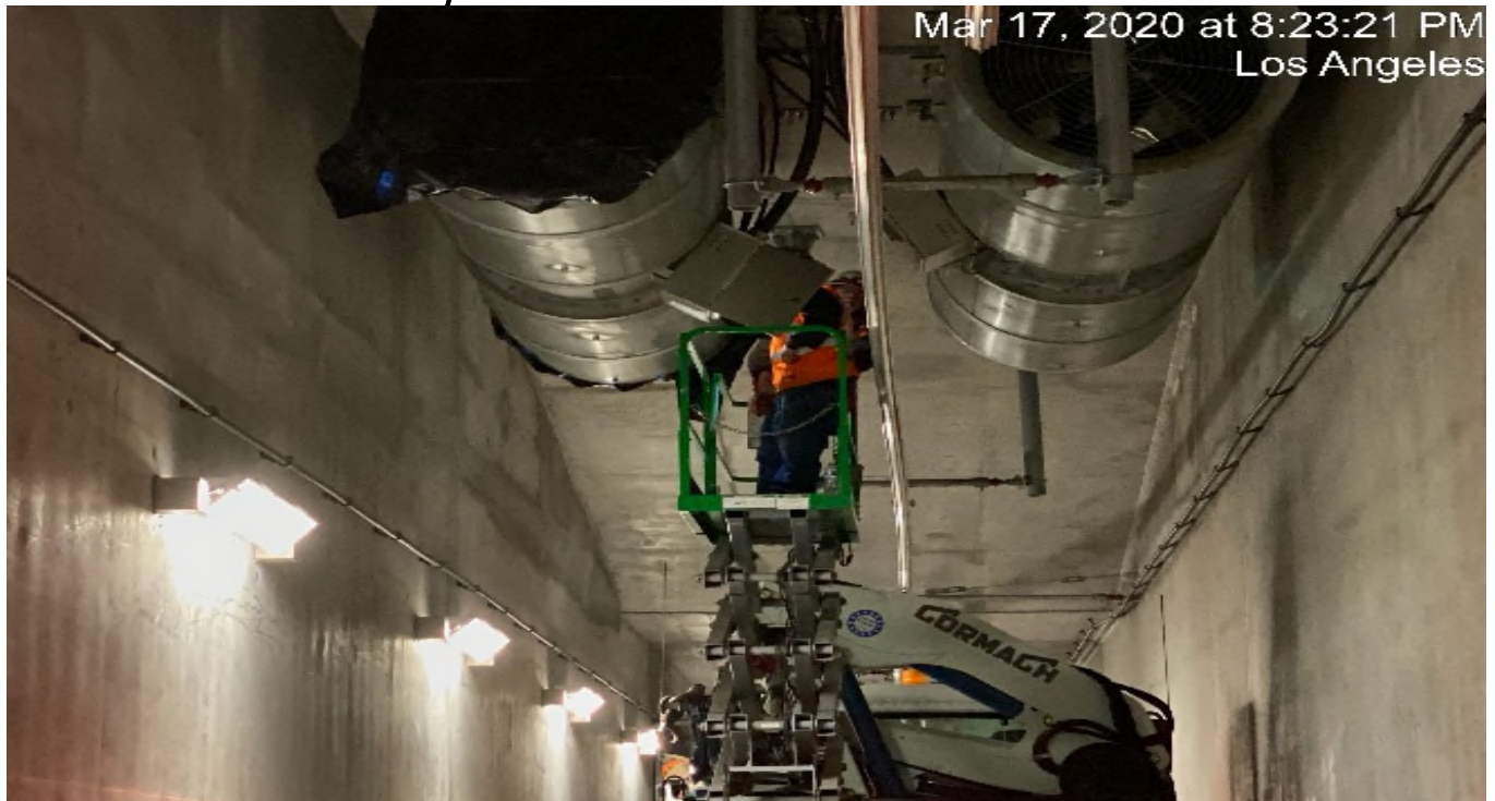
UG3 – DCD wiring up booster fans southbound UG-3.
