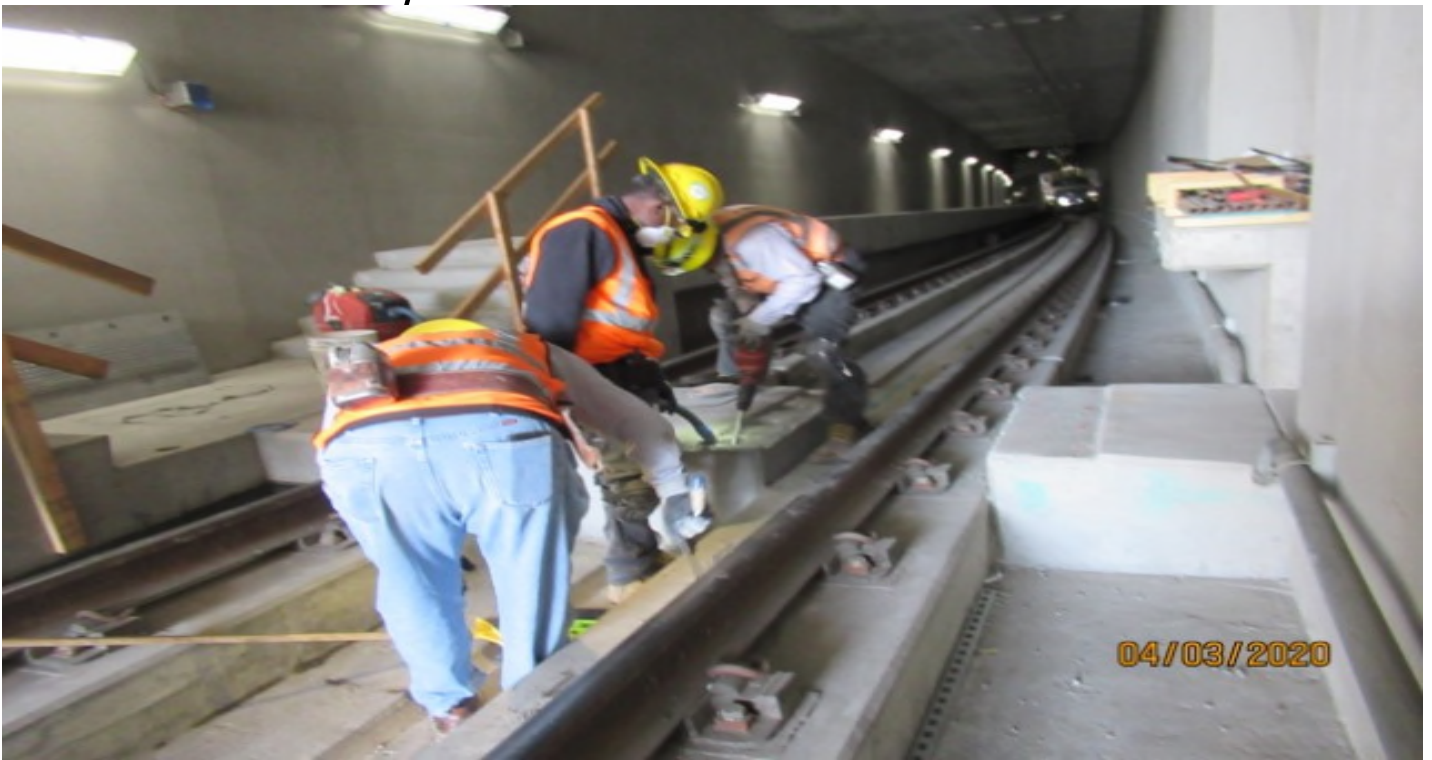
UG4 – WSCC in UG4 NB #4 track STA 371+64, repair work on emergency walkway foundations.
