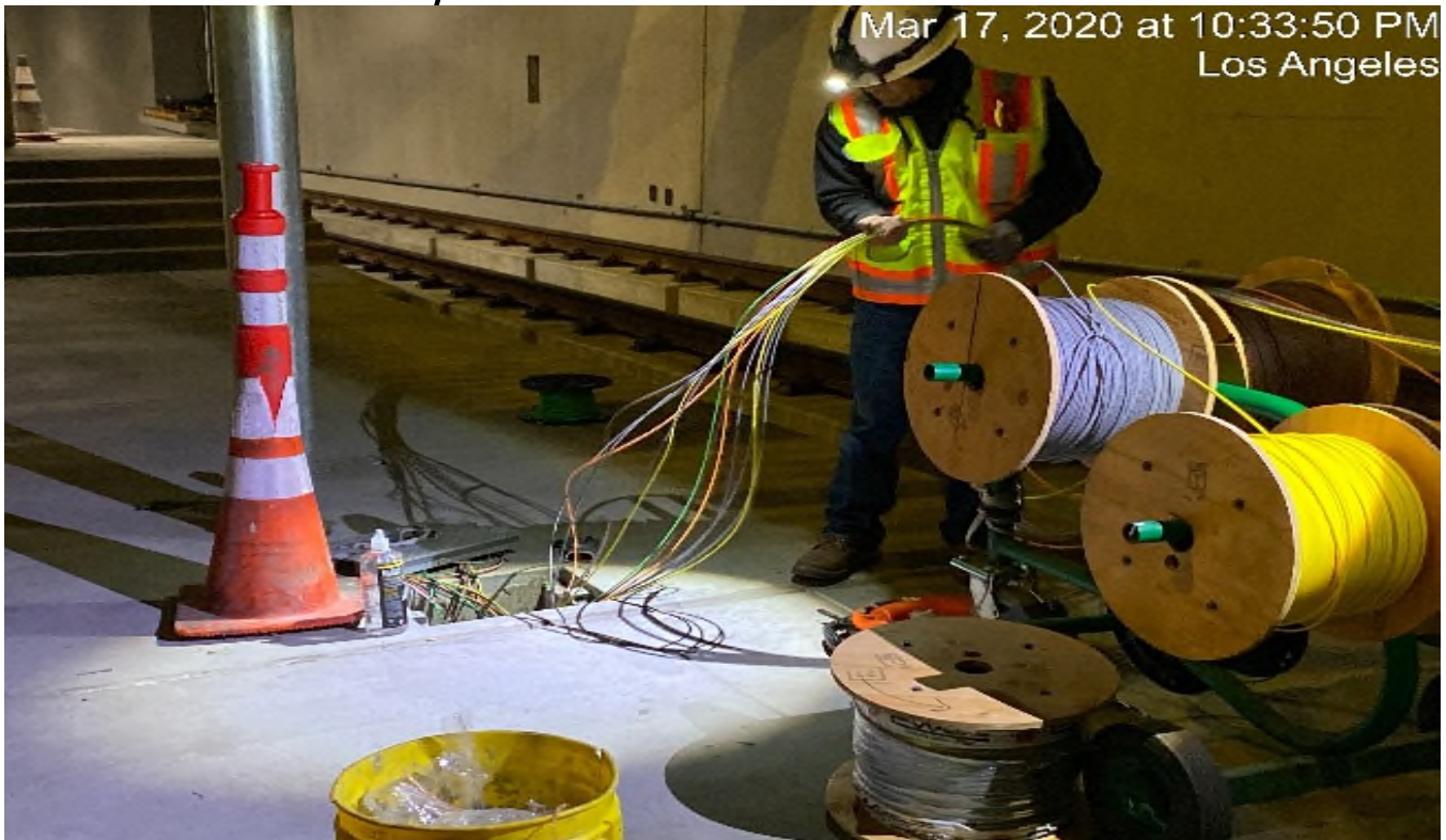
UG-4- DCD wiring up UG lighting southbound UG-4.
