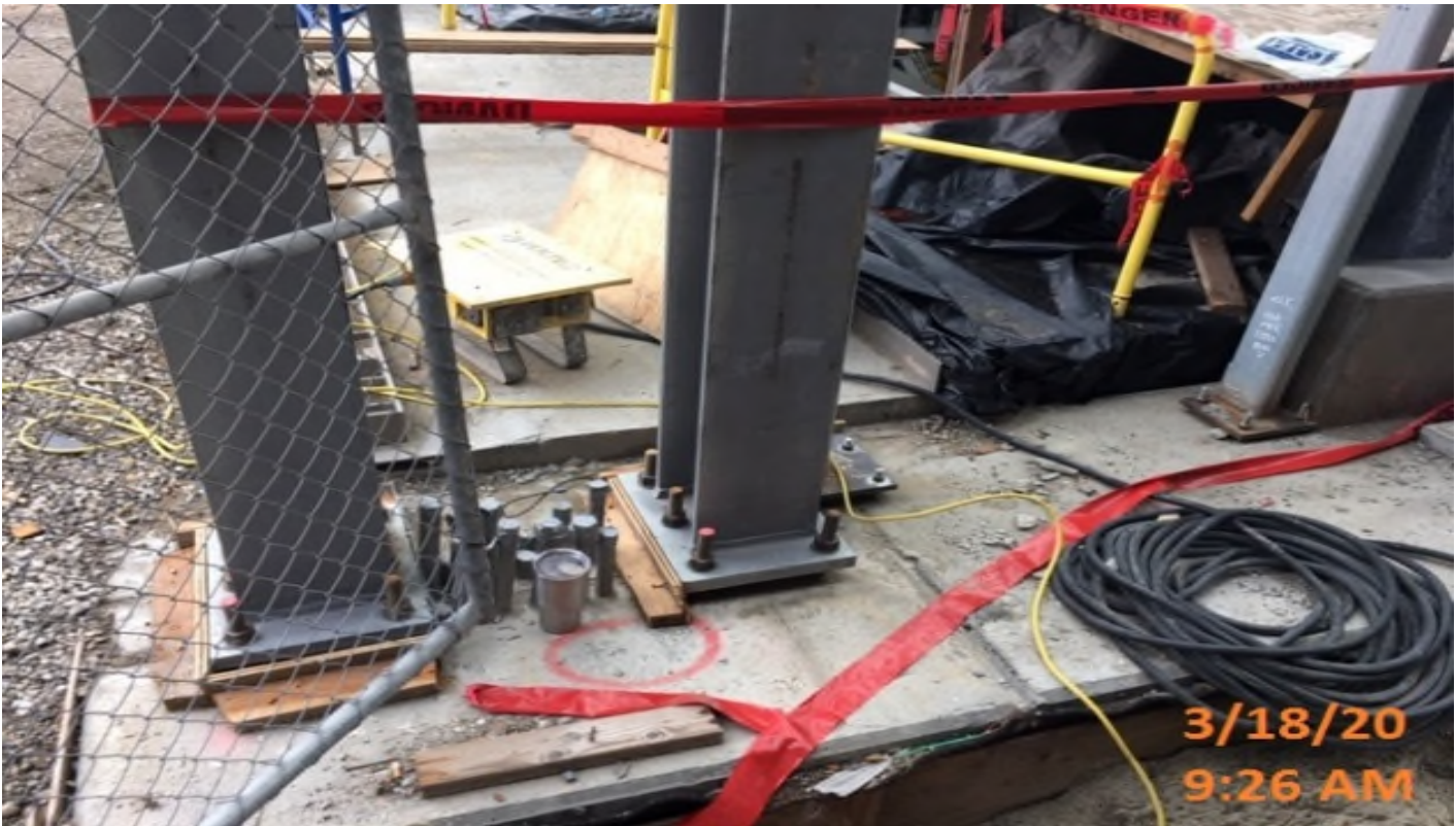
Crenshaw/MLK - WSCC crew building forms for main entrance canopy base plates.
