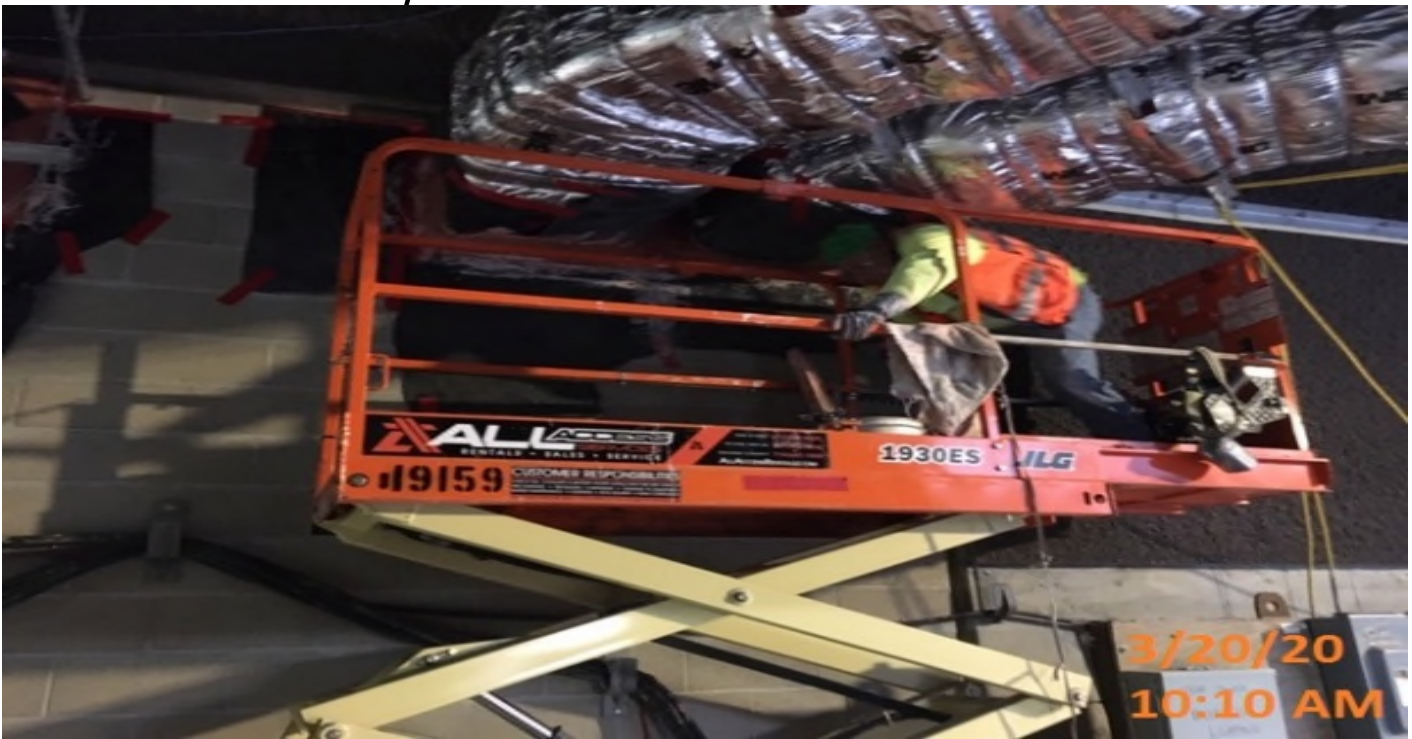
Crenshaw/Expo - WSCC finishers applying fire mortar around ductwork.
