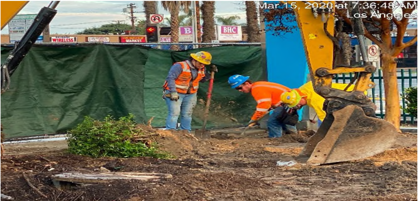
Crenshaw/Expo - WSCC excavating Neil Electric fiber optics Expo yard
