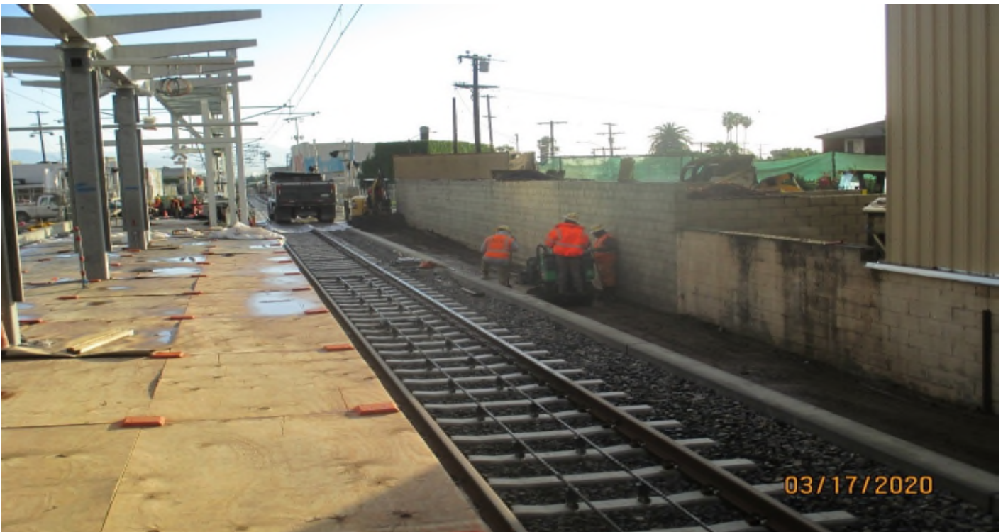
Florence/West – Drainage swale grading along the West Station platform. Facing east.
