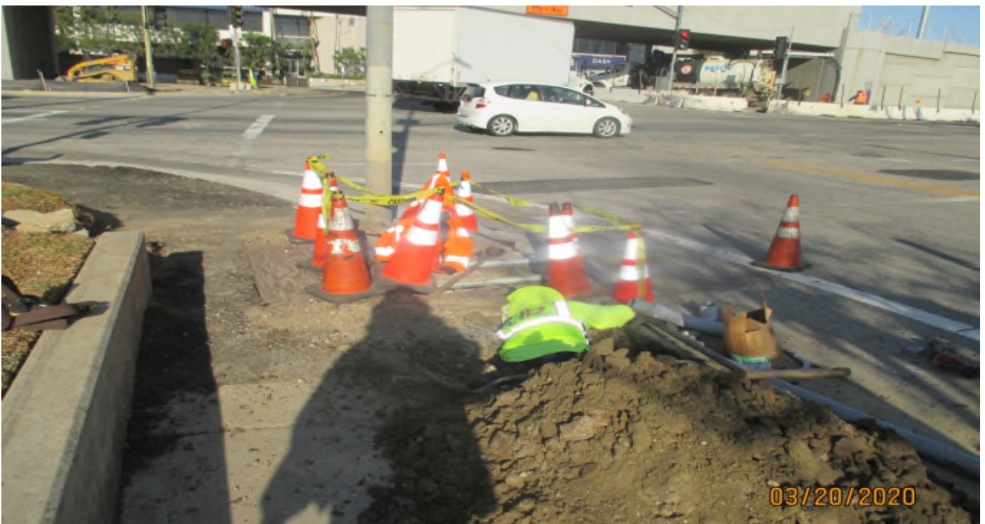
111 th Street – Terminating traffic signal connections on 111th street.
