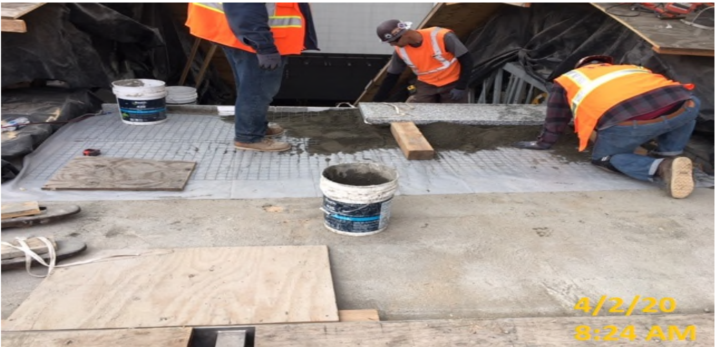
Crenshaw/MLK - MLK – WSCC crew building formwork for west planter wall.
