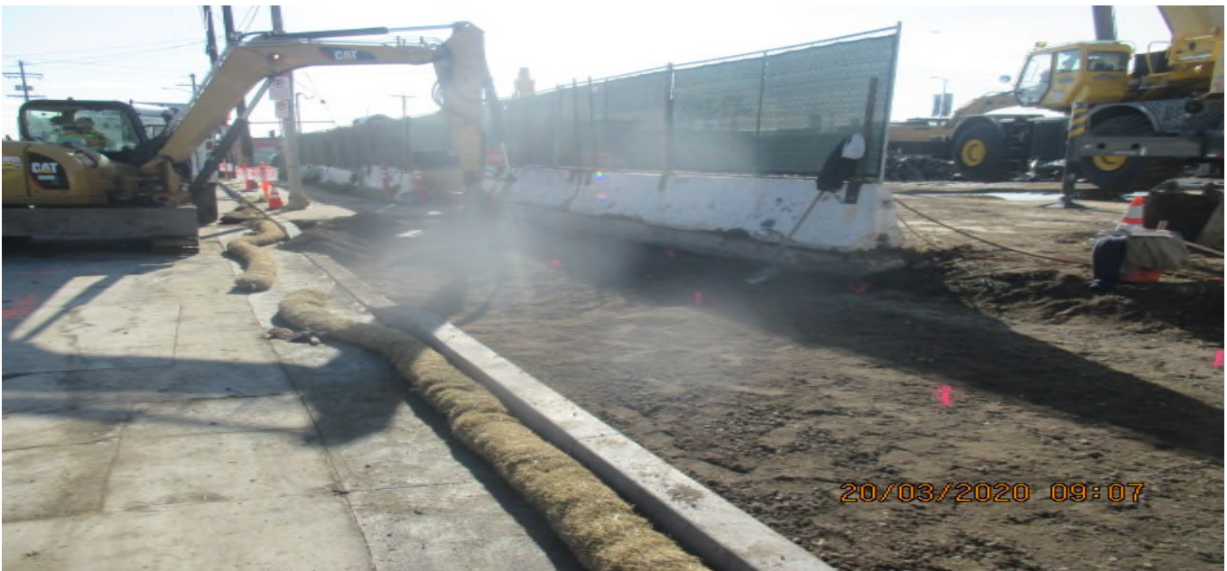
UG3 – Continue excavation for the new sidewalk/driveway installation on the southwest corner of 67th St and Crenshaw Blvd. 3/20/20
