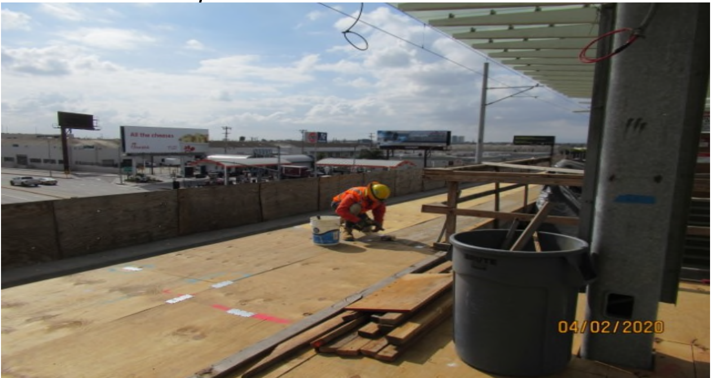
Aviation/Century – WSCC repairing protective plywood on platform at Century-Aviation station (looking southeast)
