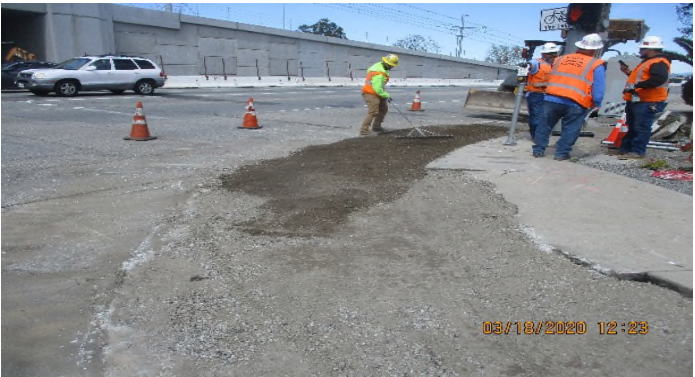
Aviation/Century – WSCC Make C&G removals at 111th and Aviation.
