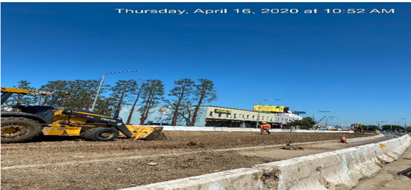
LEIMERT PARK STATION – Continue backfilling/grading the center median
