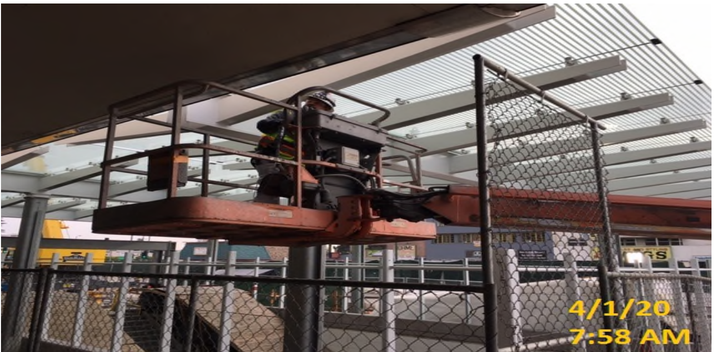
Crenshaw/MLK - MLK – Mariscal Painting applying primer touch-ups to main entrance canopy.
