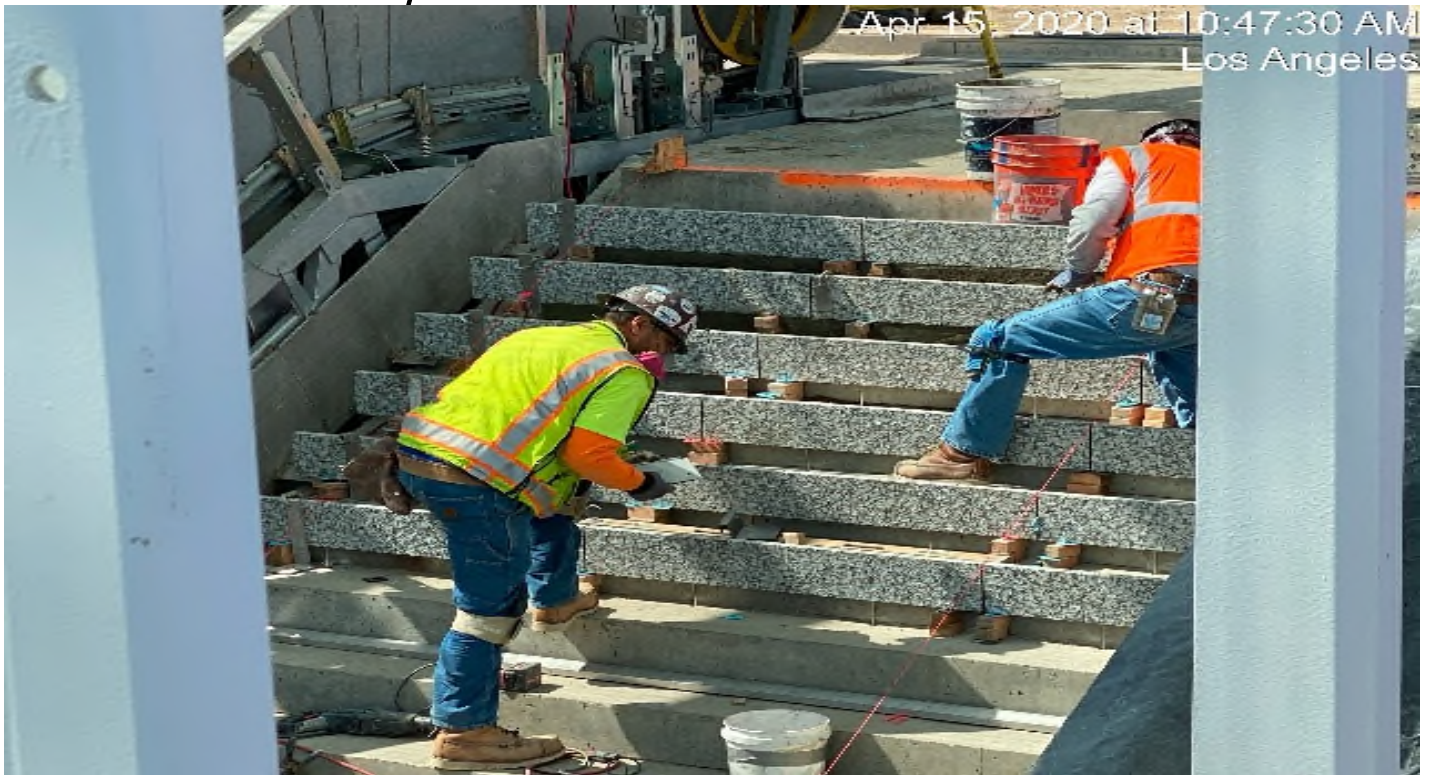
Crenshaw/Vernon - Carrera placing stair treads at Vernon.
