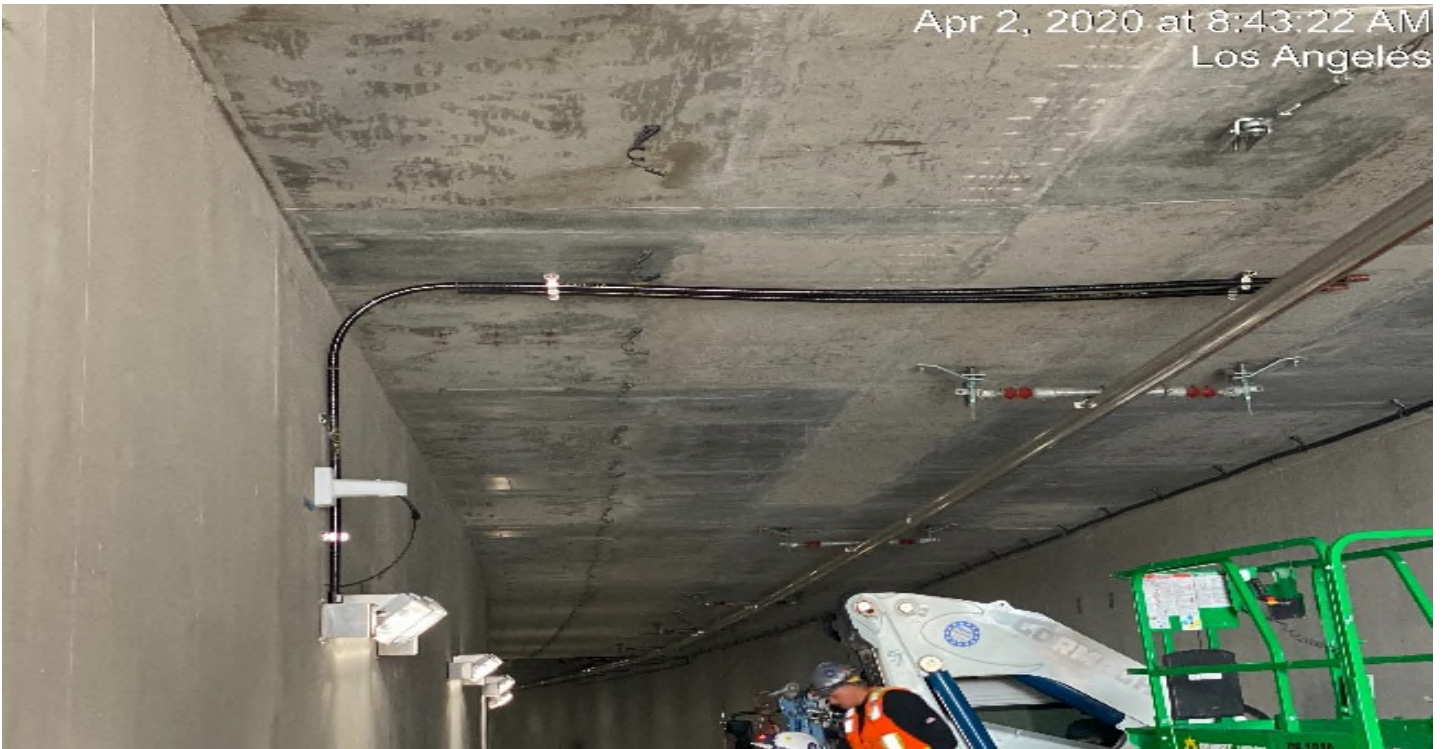
UG3 – DCD installing phenolic conduit at UG-3.
