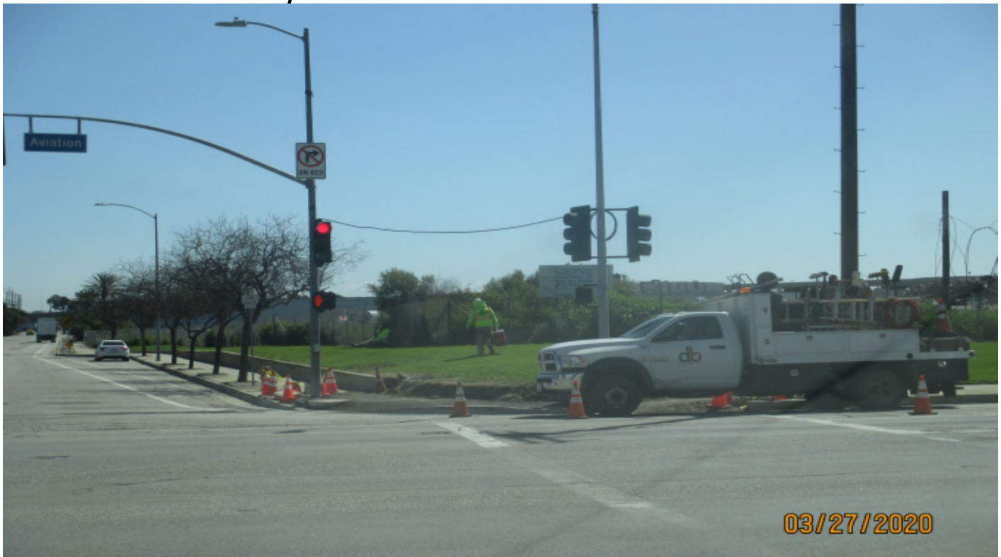
111 th Street – Traffic signal work at 111th street.
