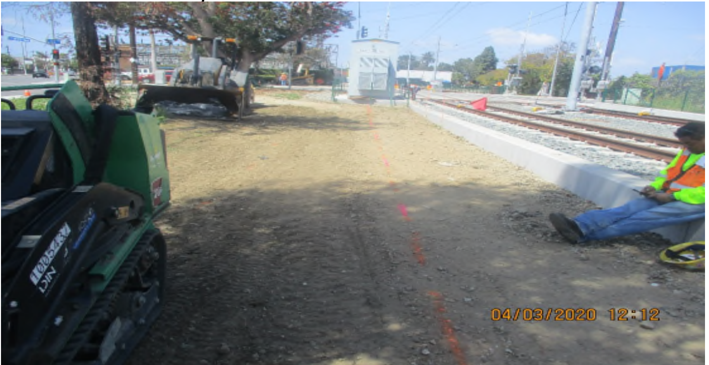
Florence/Brea – WSCC Start new swale from Fir St east toward La Brea.
