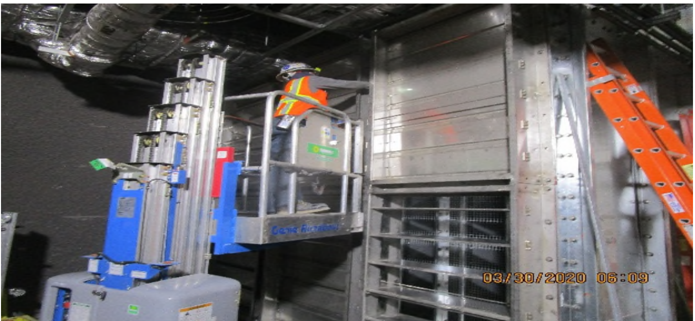
LEIMERT PARK STATION – Continue tunnel fan damper section installation for the sound attenuator for EVF-6-102 in the North Fan Room C – 142 of the concourse level.
