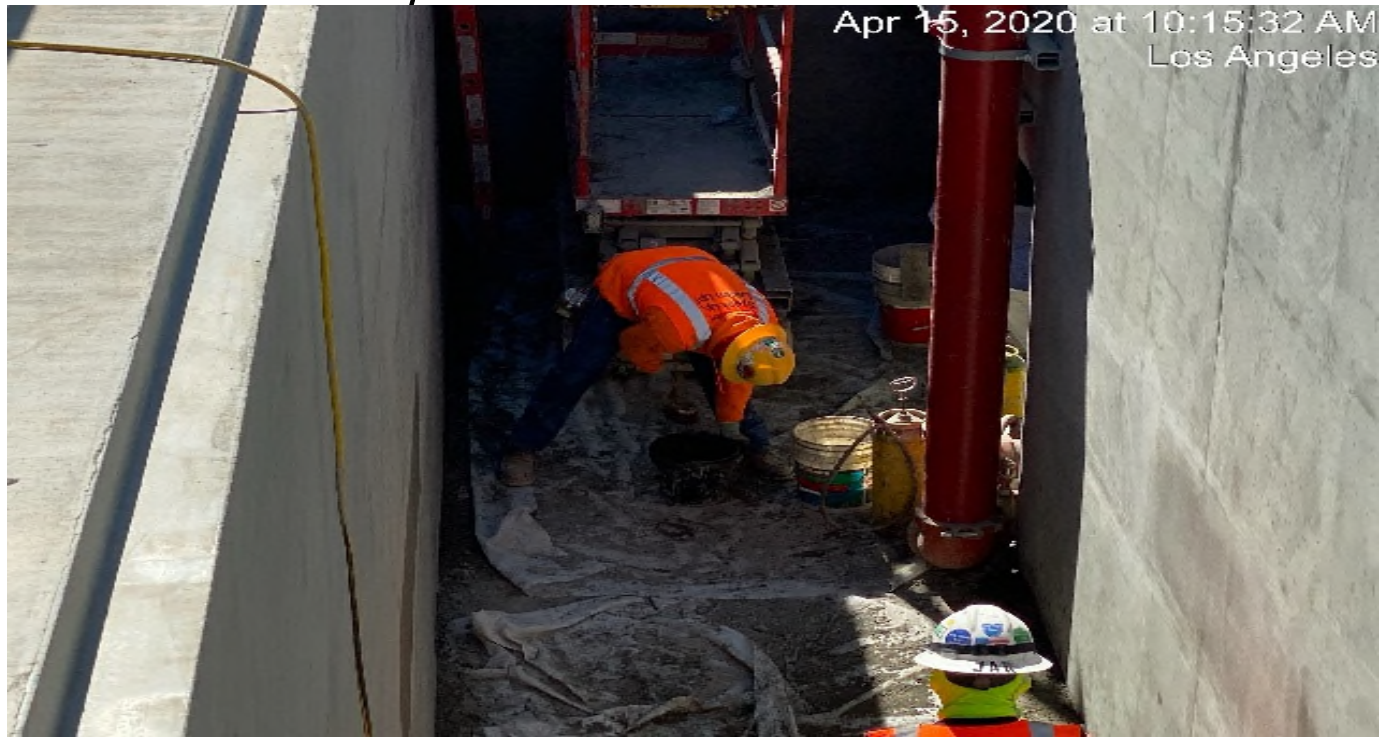
Crenshaw/Vernon - WSCC sacking and patching plenum walls at Vernon.
