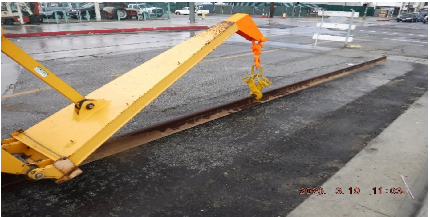
Crenshaw/Vernon - STA 363+00 TK#3 – new 22.7' rail plug delivered on site for T&M work Vernon Station
