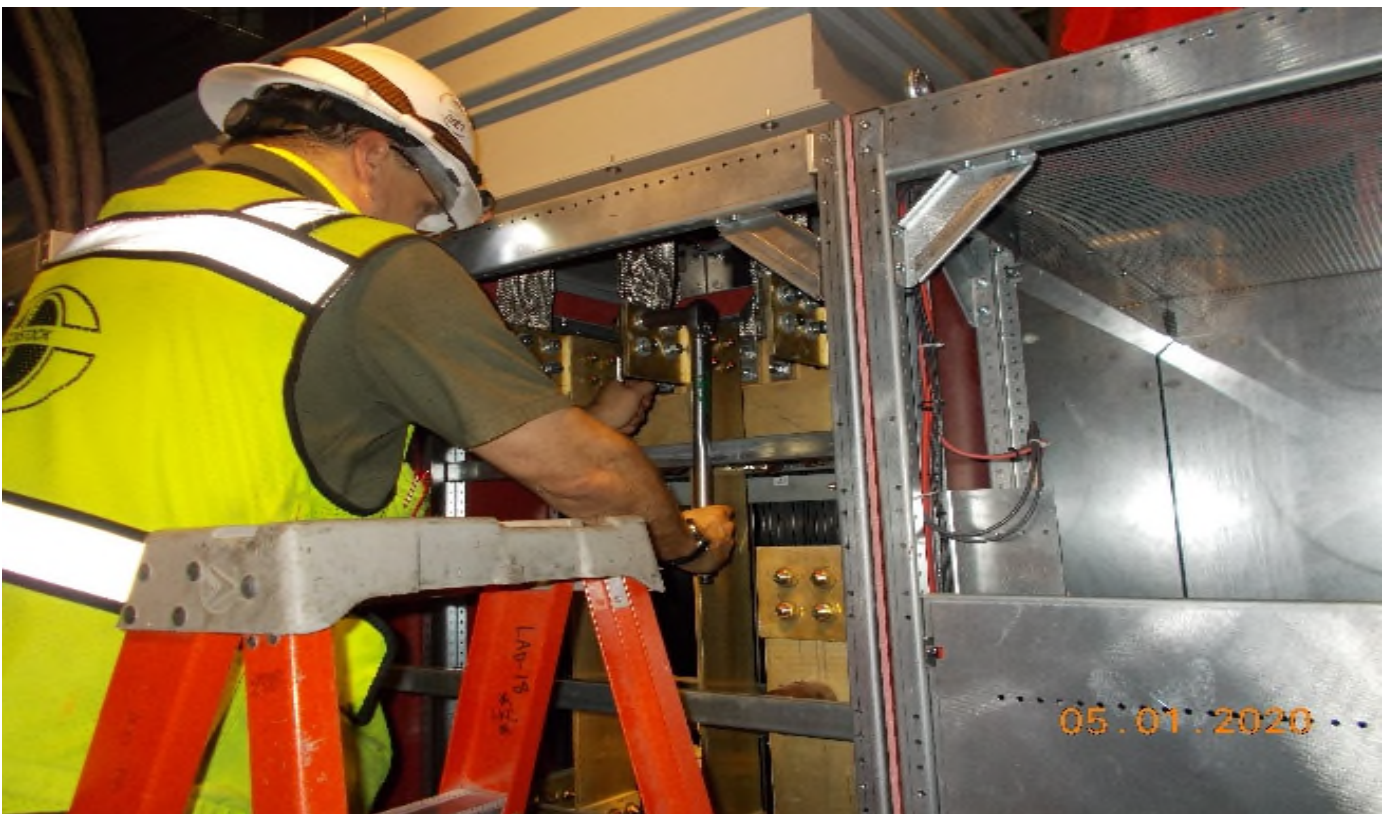
Crenshaw/Expo - LKC torquing the flex-bus between the rectifier and bus duct.
