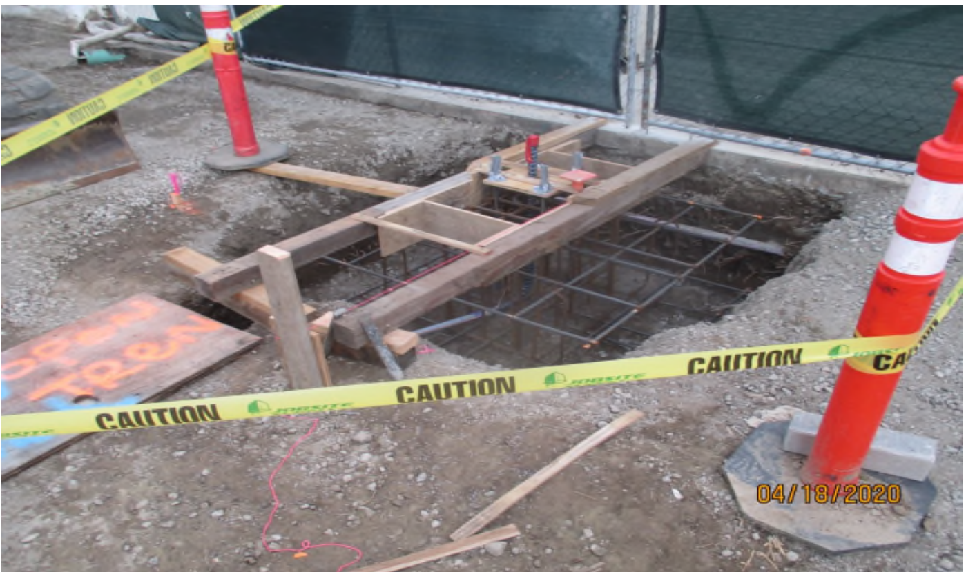
Aviation/Century – Irrigation pipe installation at the Aviation Station yard.
