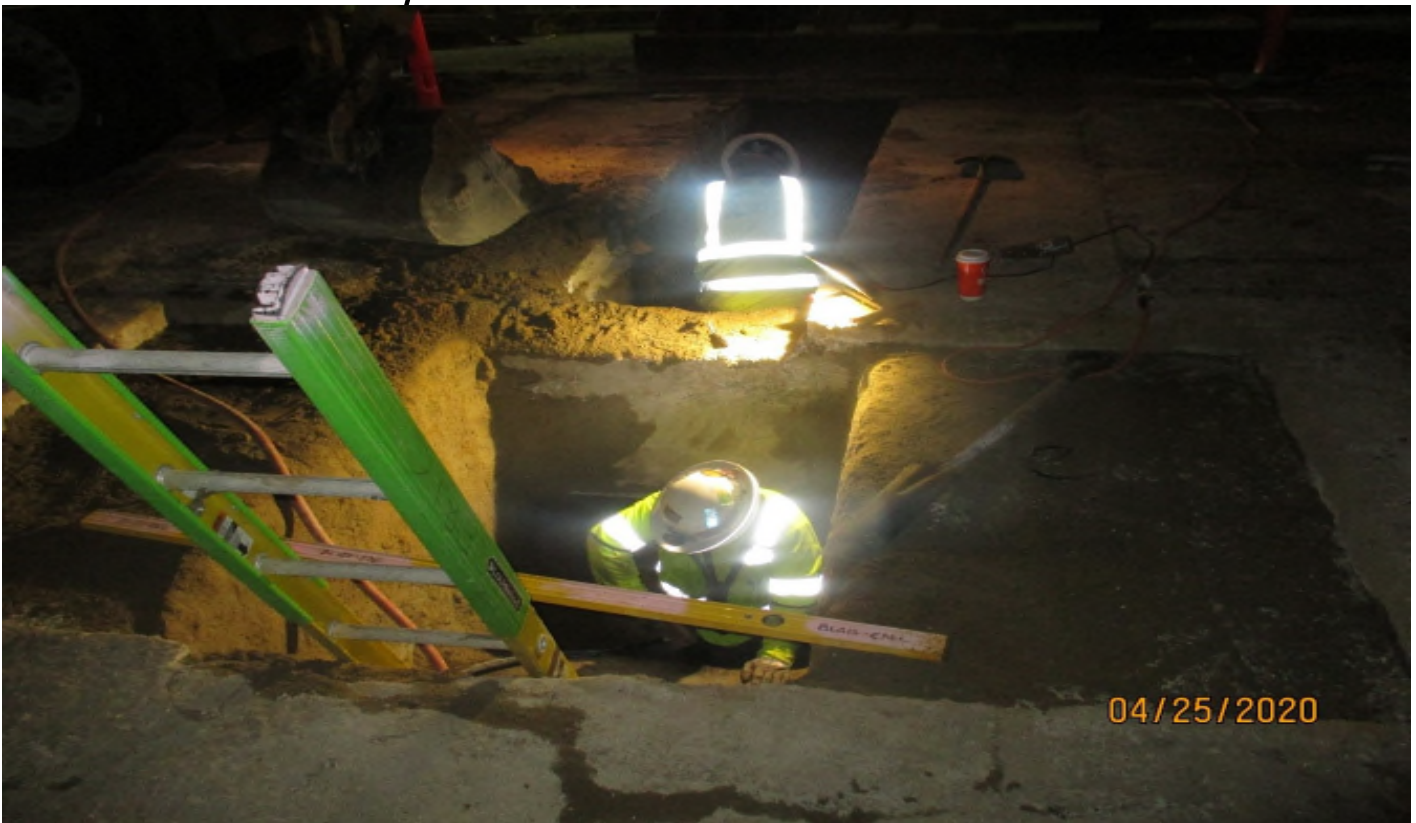
UG1- Fire line excavation at the south portal of UG-1.
