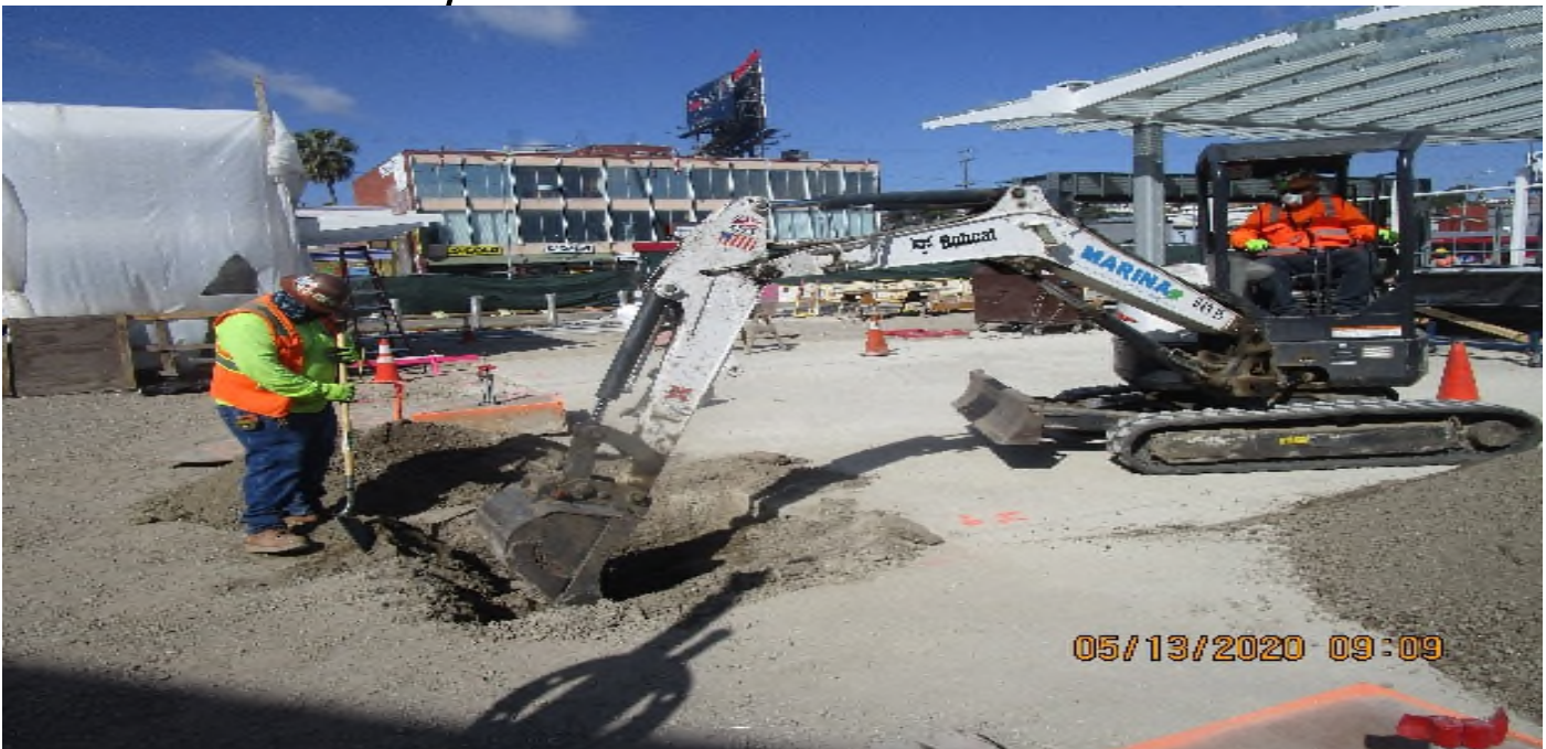
LEIMERT PARK STATION – Excavating for palm tree installation at the plaza.
