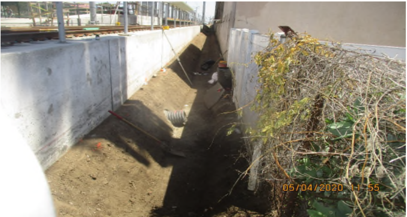
Florence/West – WSCC Cut and make grade For swale at West Station.
