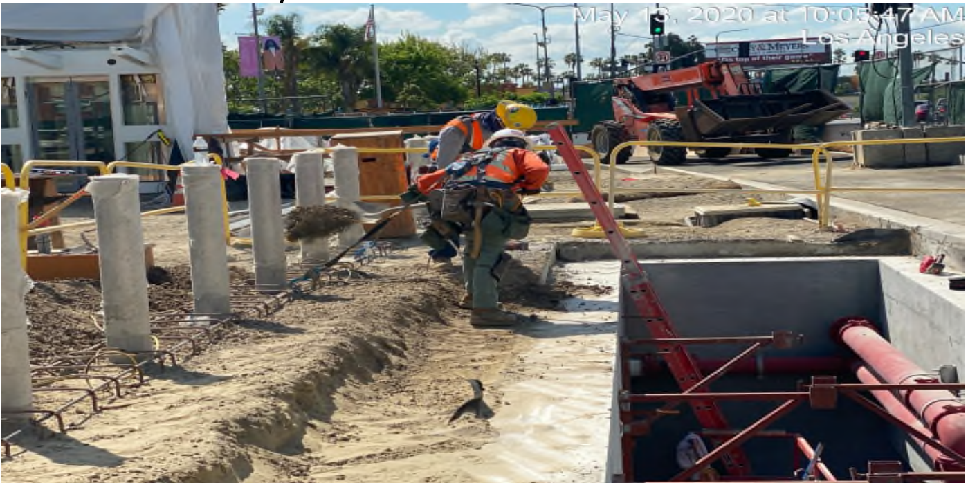
Crenshaw/Vernon - WSCC cleaning up around the plenum at Vernon.
