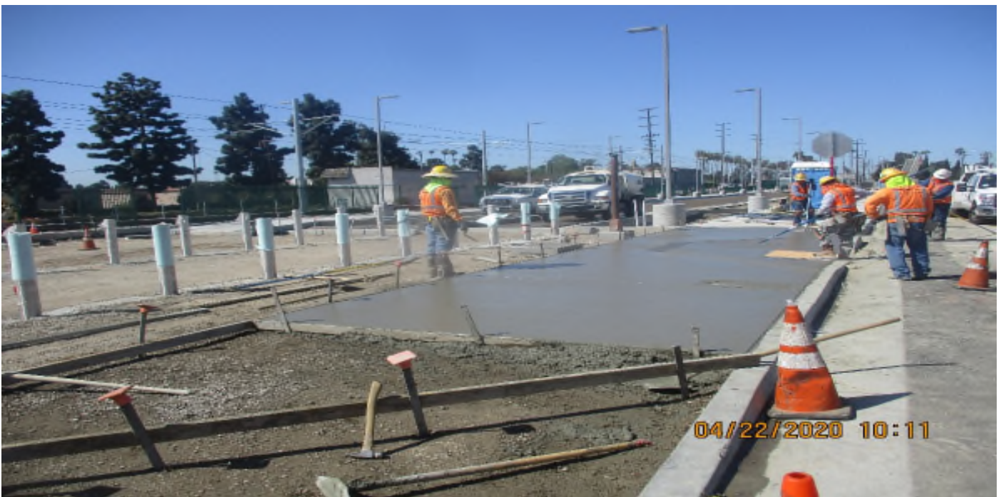
Florence/West – Placing SWK concrete at West Station parking lot.
