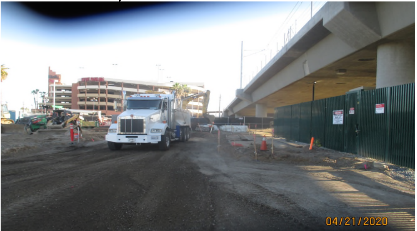
Aviation/Century – Grading at the Aviation station.
