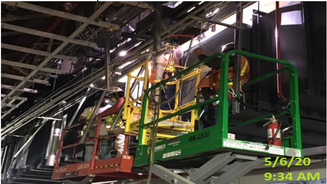
Crenshaw/Expo - WSCC ironworkers welding support post for platform edge lighting
