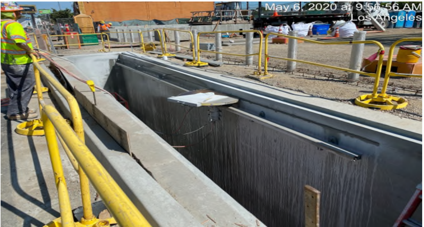
Crenshaw/Vernon - Penhall cutting top of plenum at Vernon.
