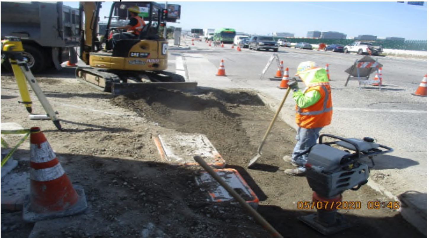
AVIATION/CENTURY - WSCC Making grade for C&G at 104th and Aviation.
