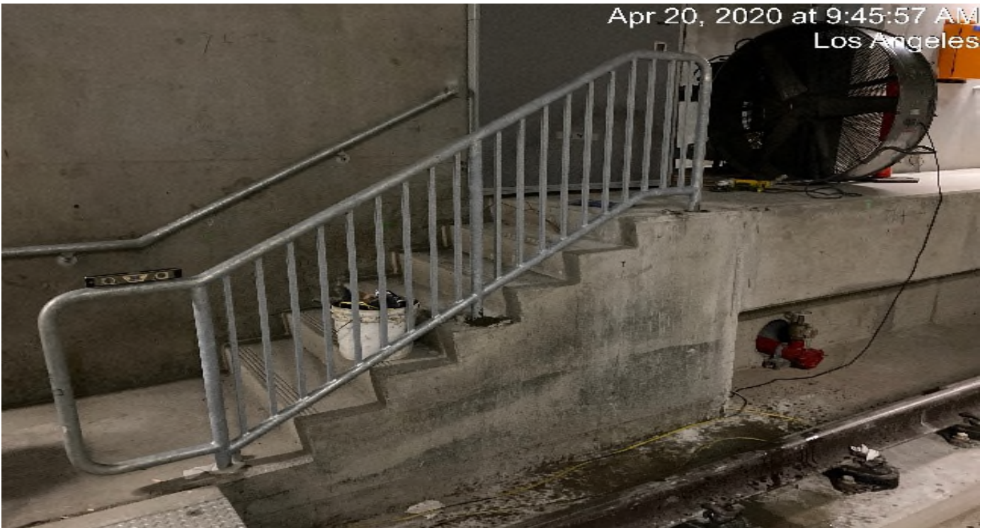
UG3 – Continue grading and excavating for the culvert drainage along the southbound barrier wall in preparation for concrete placement. 3/27/20
