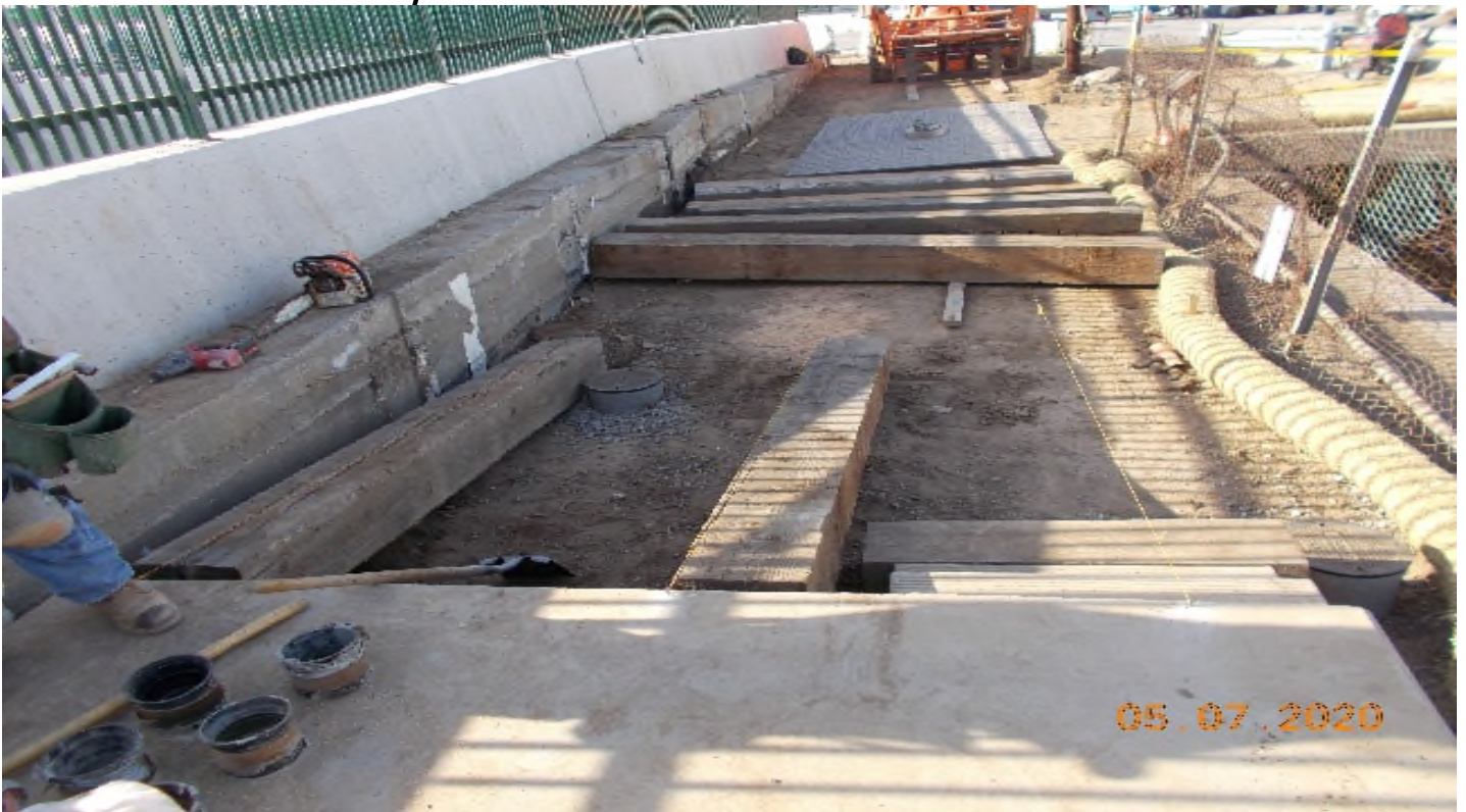
104 th Street - South view of WSCC building a ramp. 104 th
