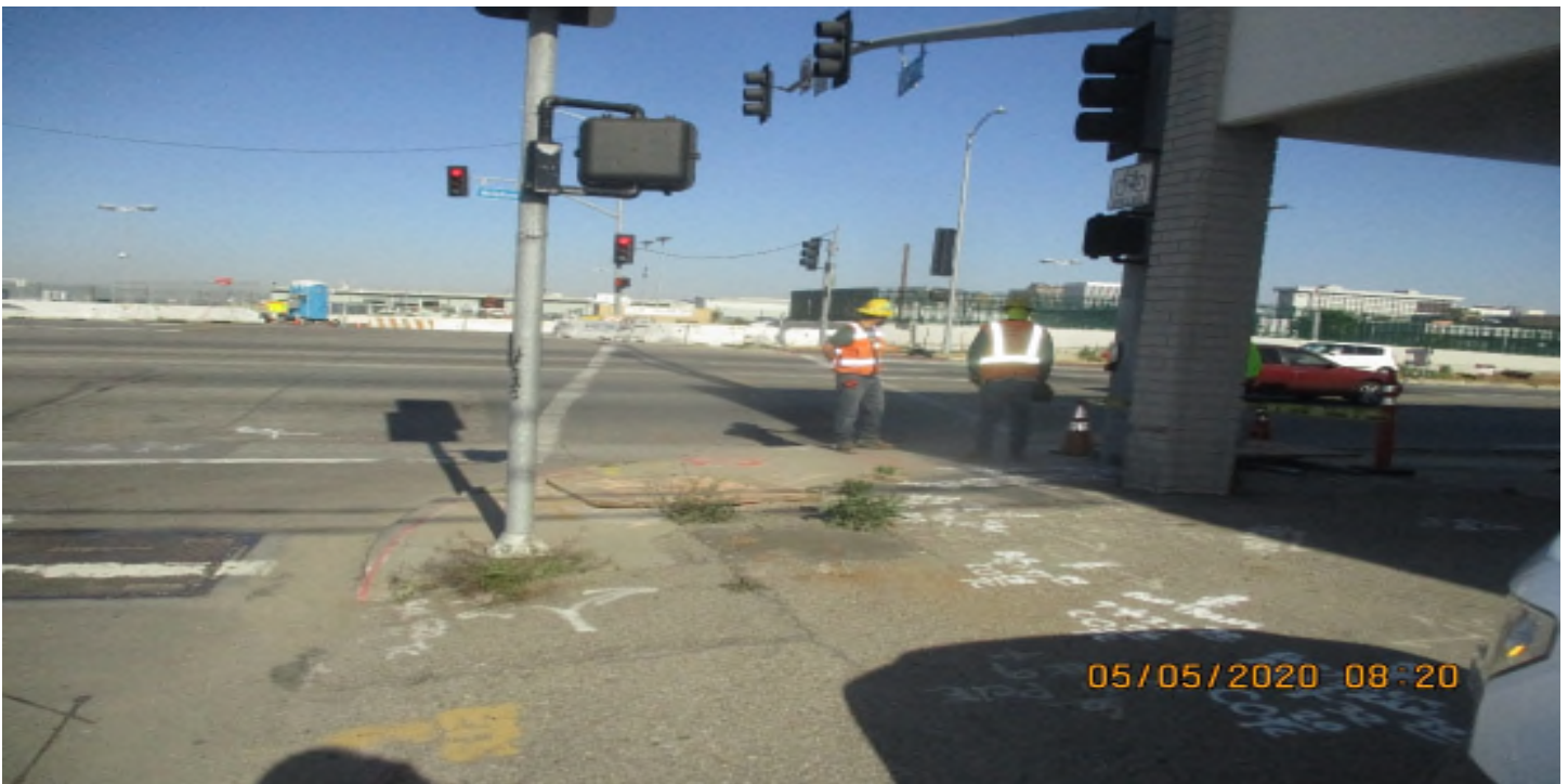
AVIATION/CENTURY - WSCC Start removals at Aviation and 104th St.
