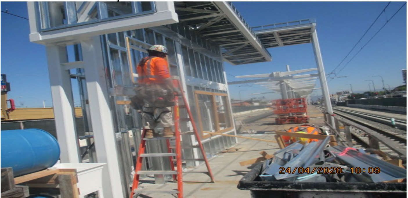
Hyde Park Station – Installing overhead lighting on the south end pavilion. 4/24/20
