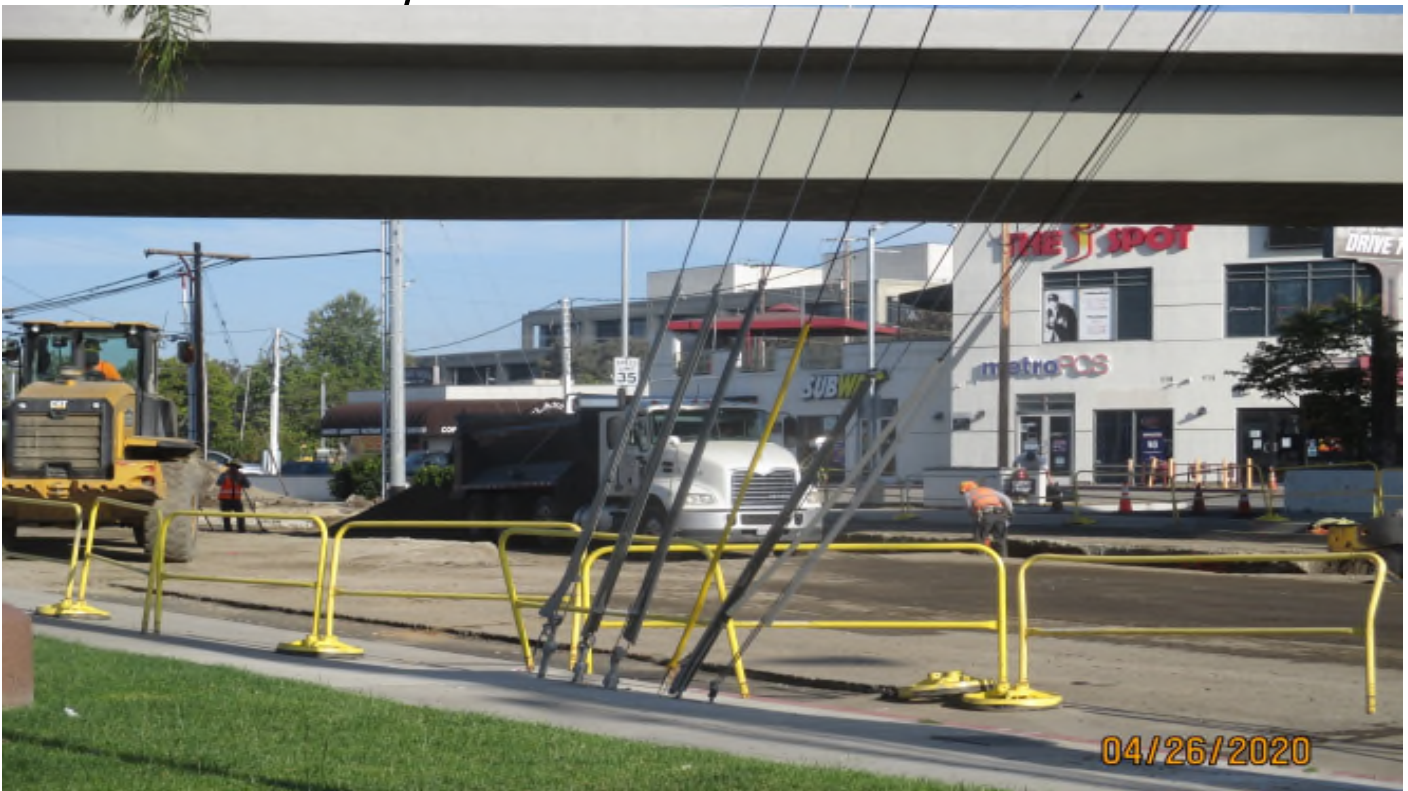
Manchester Bridge – Placing base on Manchester.
