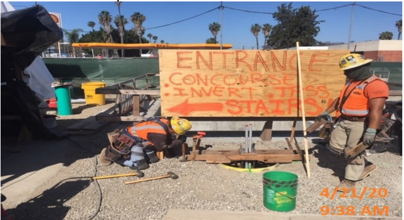
Crenshaw/Expo - EXPO – WSCC carpenters resetting bolt templates for plaza luminaires
