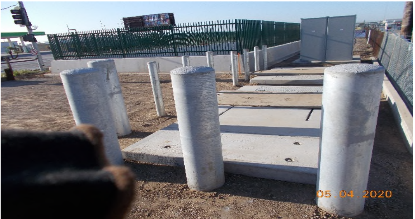
104 th Street - View of Dyna Electric preparing compressor work. 104 th
