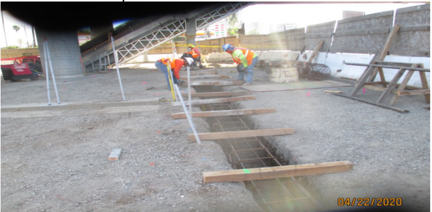
Aviation/Century – Setting rebar for the bollards at Aviation Station.
