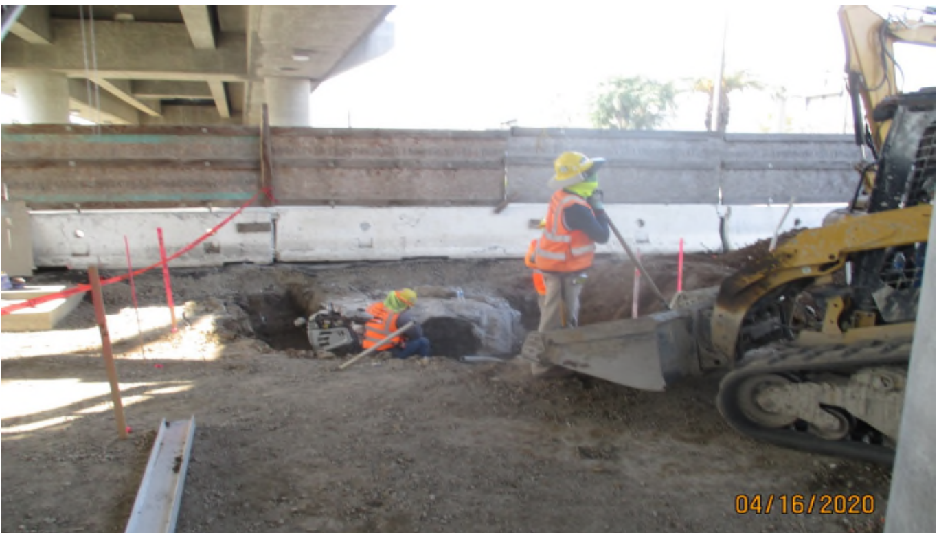
Aviation/Century – Abandoning a storm drain line at aviation Station.
