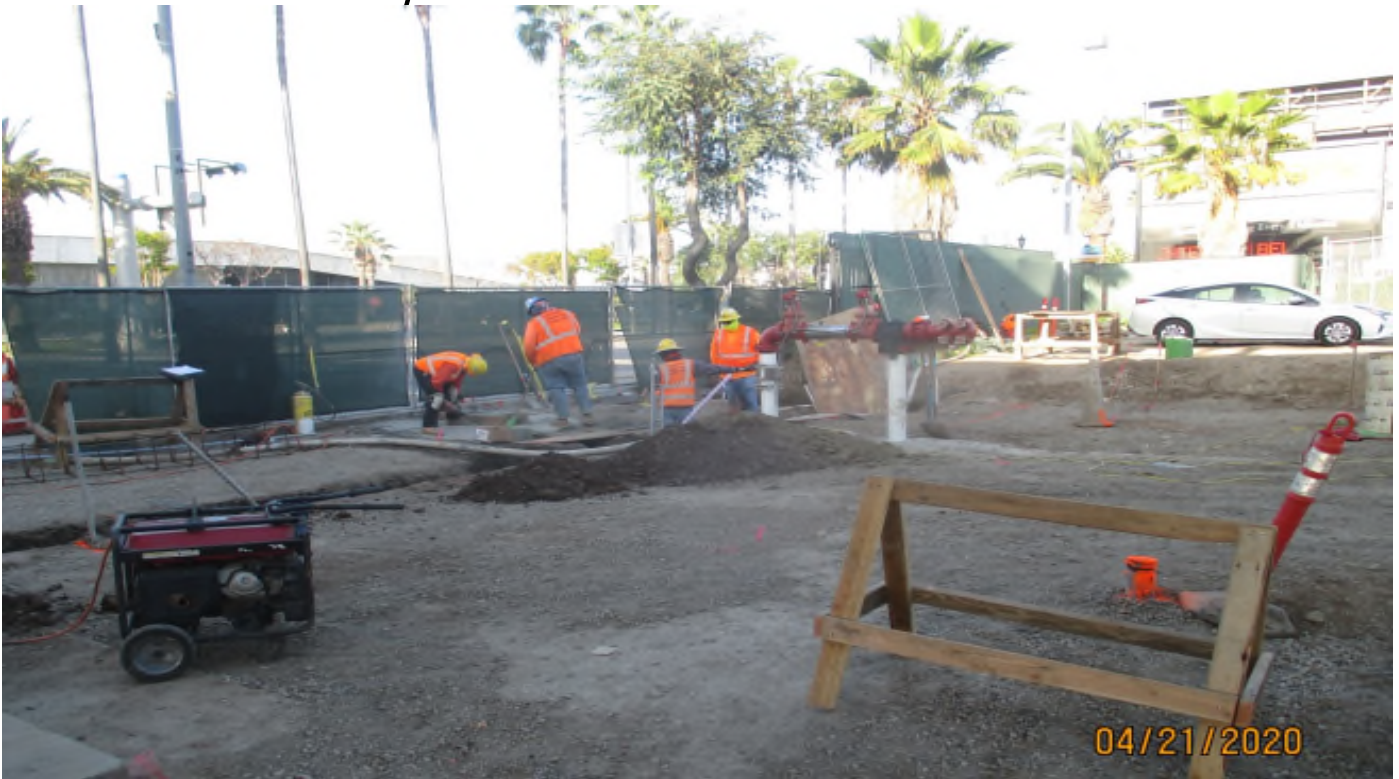
Aviation/Century – Metal stud framing at the Aviation Station ticket kiosk.
