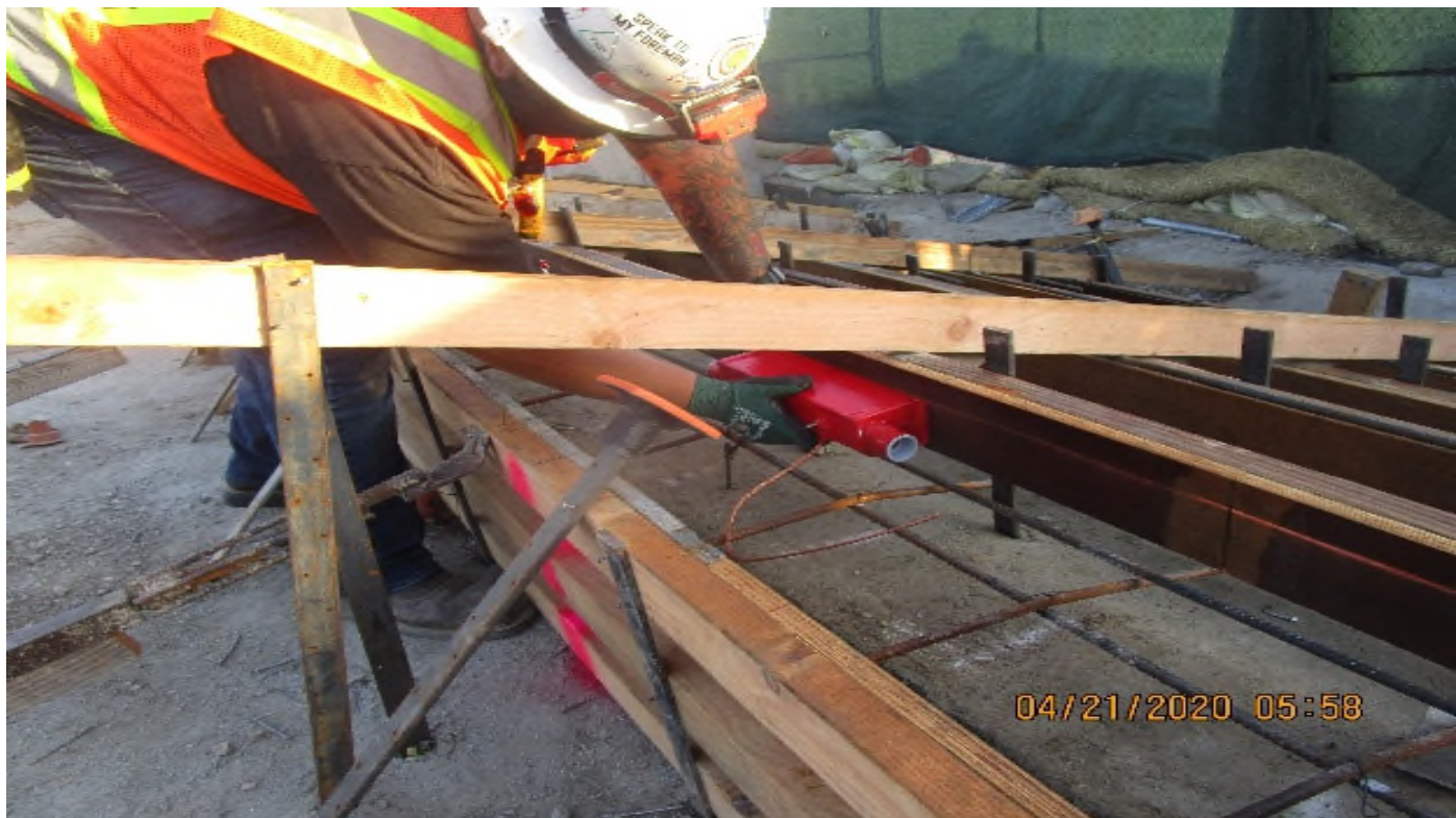
Crenshaw/Vernon - WSCC placing forms for the map case at Vernon.
