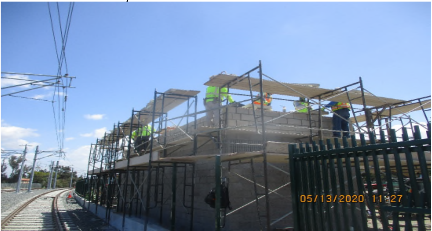
Florence/Brea - Masonry Concepts Place veneer walls at La Brea bathrooms.
