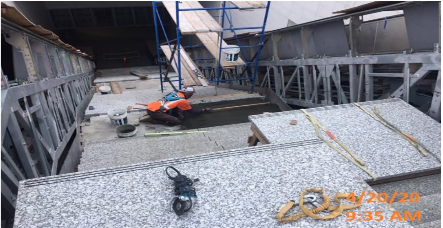
Crenshaw/Expo - EXPO – Carrera Marble installing landing sections at main staircase.
