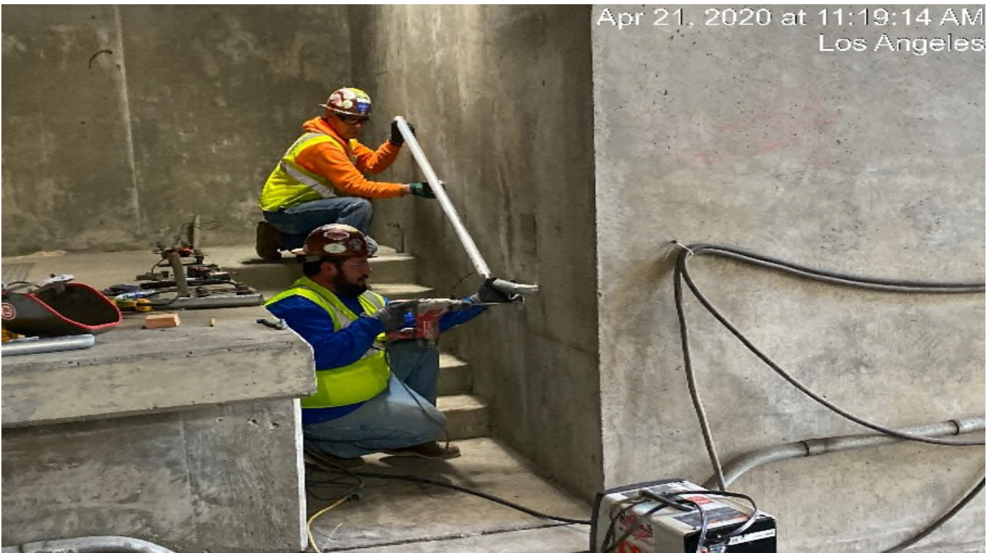
UG3 – McMahon installing handrail at UG-3.
