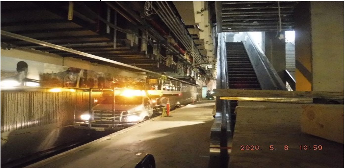
MLK - STA 402+00 TK#3/SB looking north – system work UG4 MLK Station.
