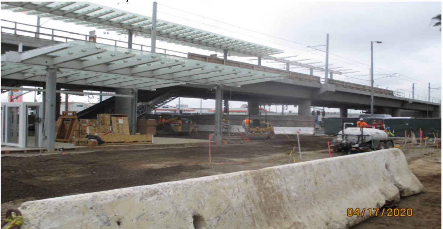
Aviation/Century – Base grading at the Aviation Station.
