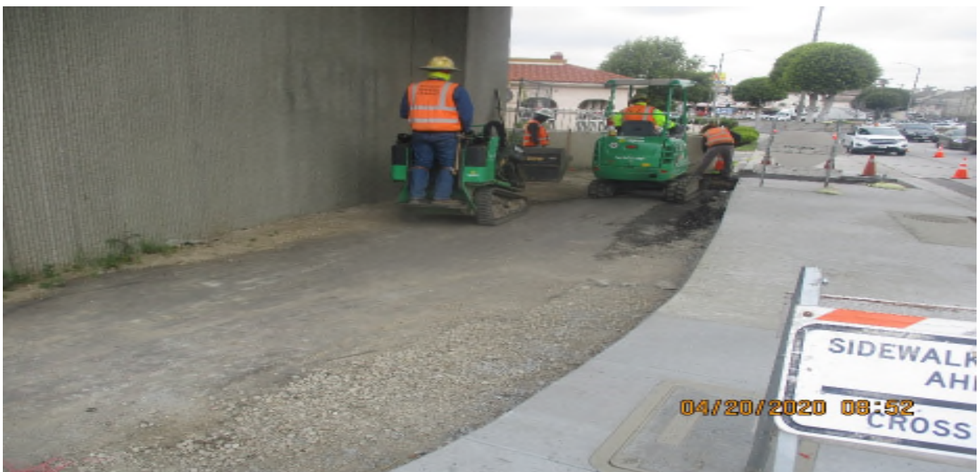
Florence/Brea - WSCC Grading behind SWK at La Brea and Florence S/E corner.
