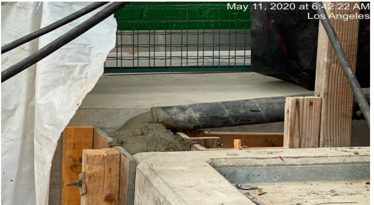
Crenshaw/Vernon - Placing concrete for planter end wall at Vernon
