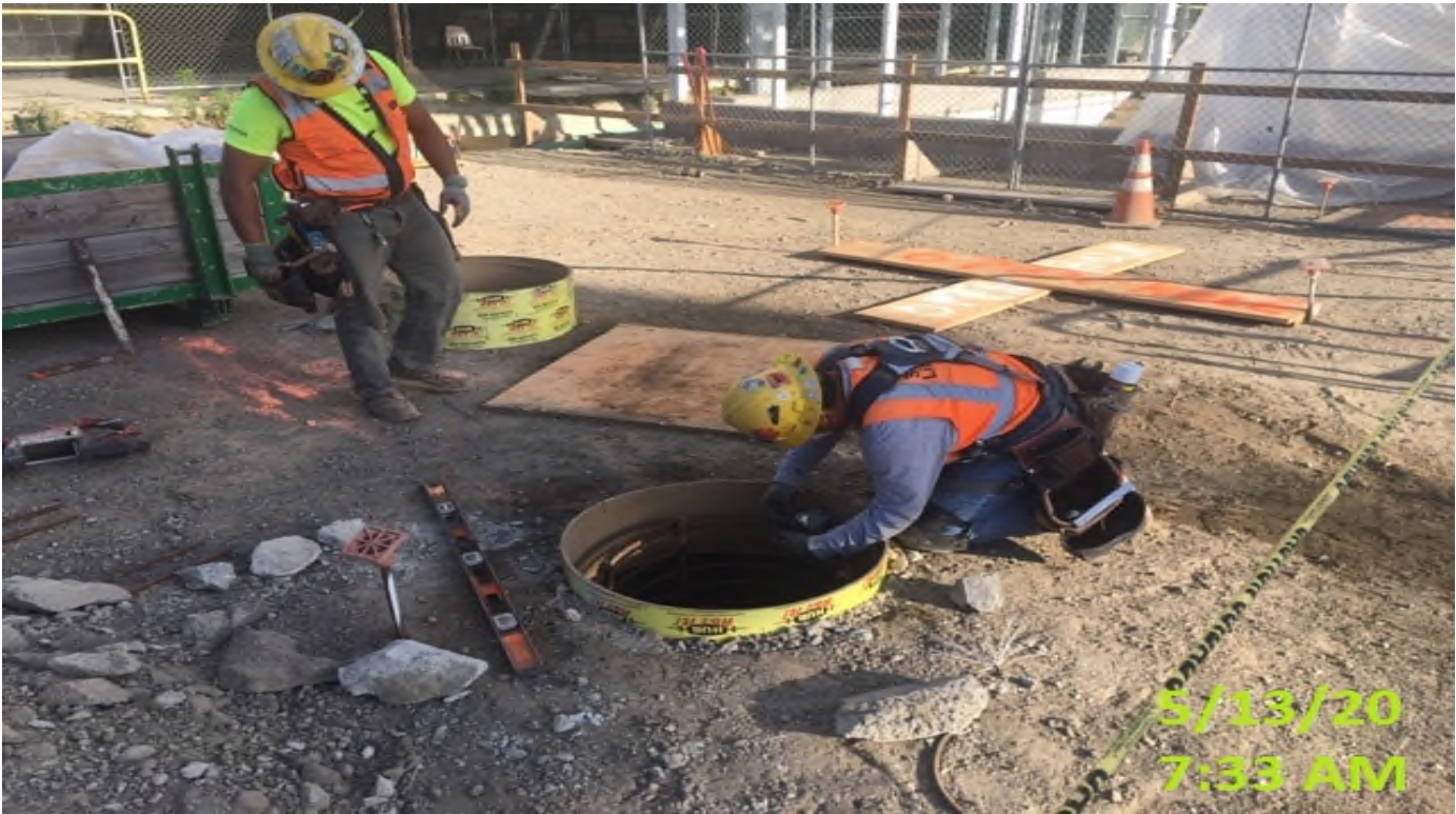
MLK – WSCC carpenters setting rebar cages in sono tubes for plaza lighting footings
