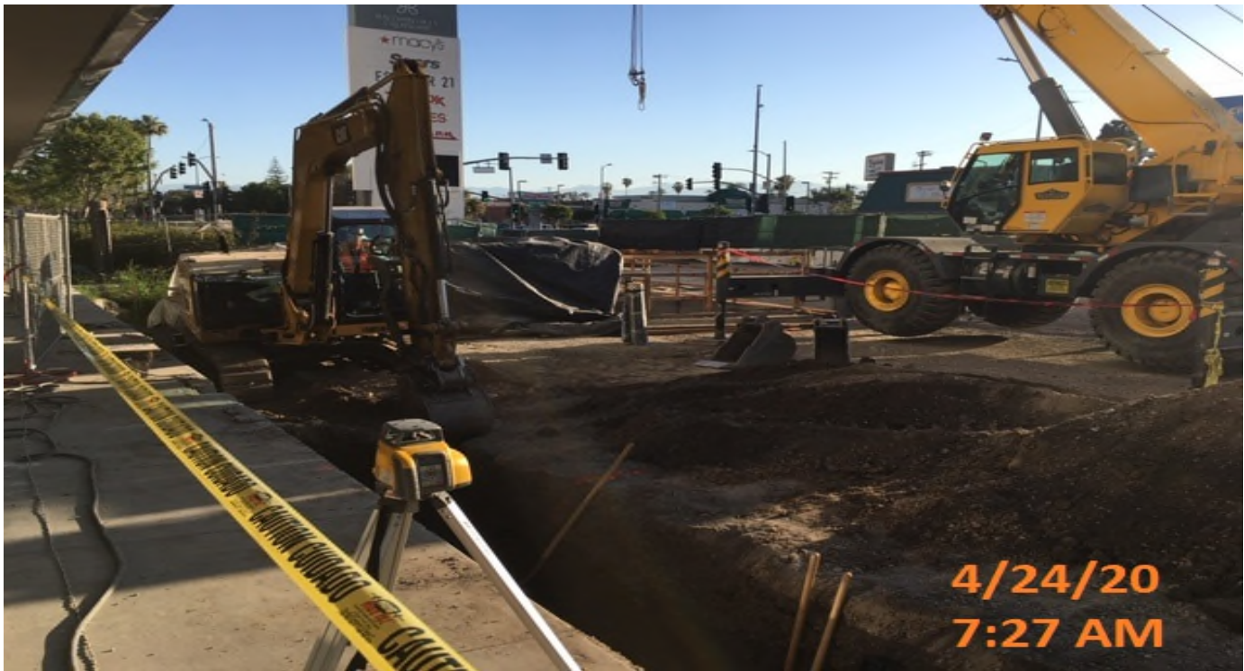
MLK STATION – Continue excavating for new 12” HDPE drainage pipe adjacent to the main entrance canopy structure at the plaza level.
