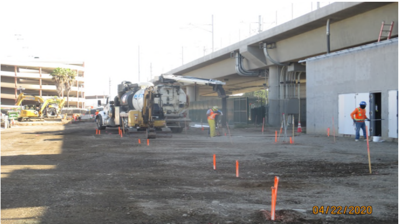
Aviation/Century – Base grading at the Aviation Station.
