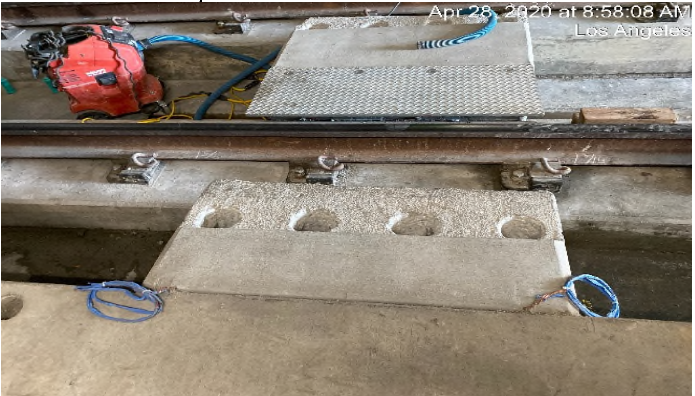
UG-4- WSCC re-drilling walk way plates at NB UG-4.
