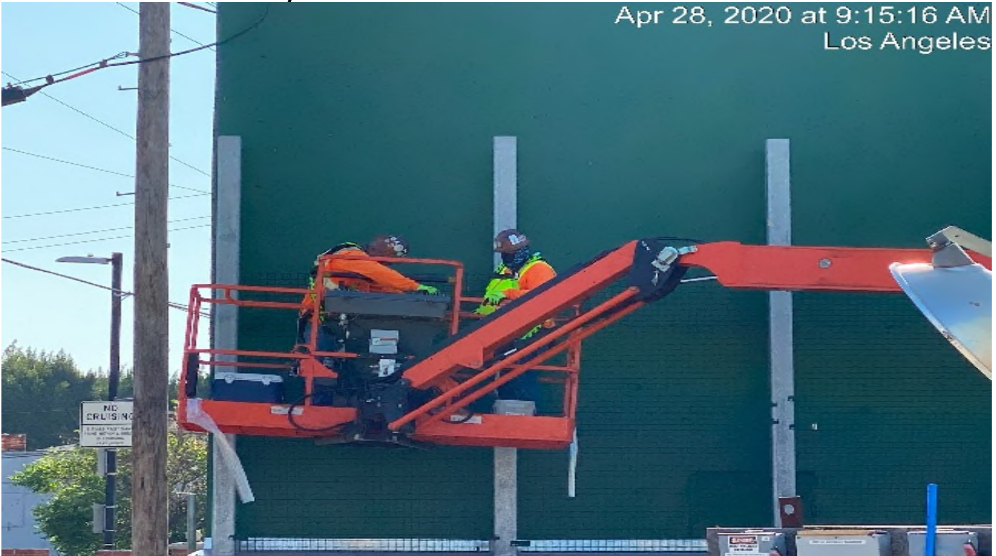
Crenshaw/Vernon - Marina landscape installing lattice at Vernon
