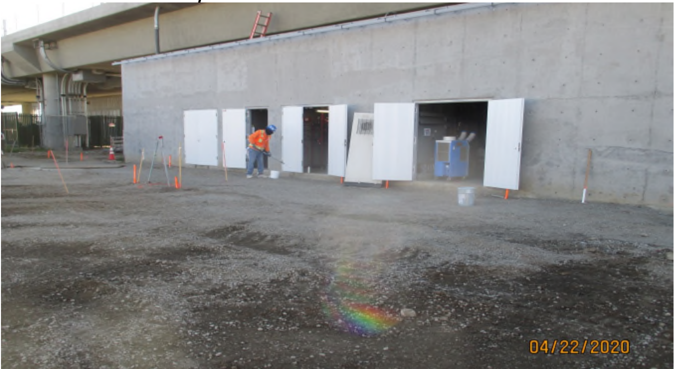
Aviation/Century – Painting the service building doors at the Aviation Station.
