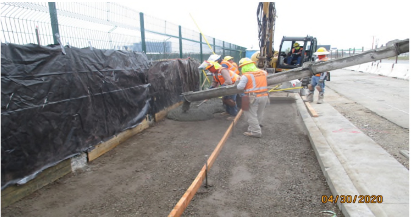
UG1 Placing concrete for a driveway at UG-1.
