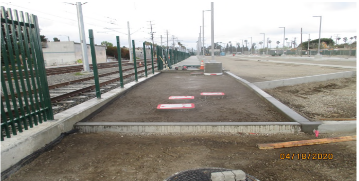
Florence/West – Sidewalk subgrade at West Station prior to concrete placement.
