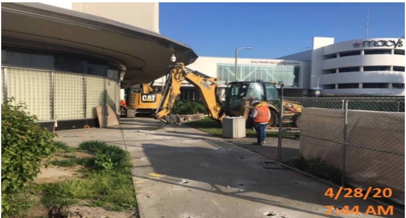
Crenshaw/MLK - MLK – WSCC crew excavating and demoing walkways and sidewalks
