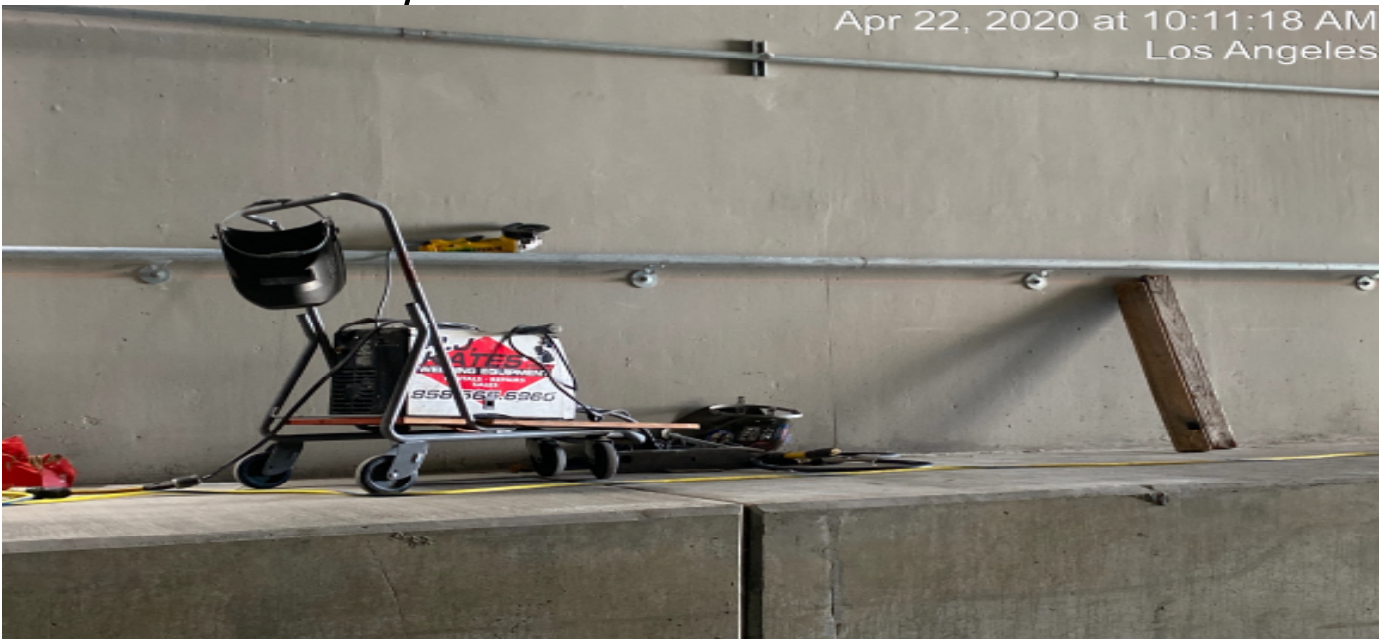
UG3 – Continue handrail installation at the north end stairs at Sta 311+00.
