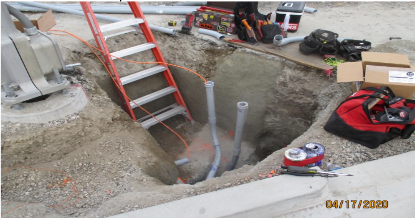
Florence/Hindry – Traffic signal pull box and conduit relocation at Hindry.
