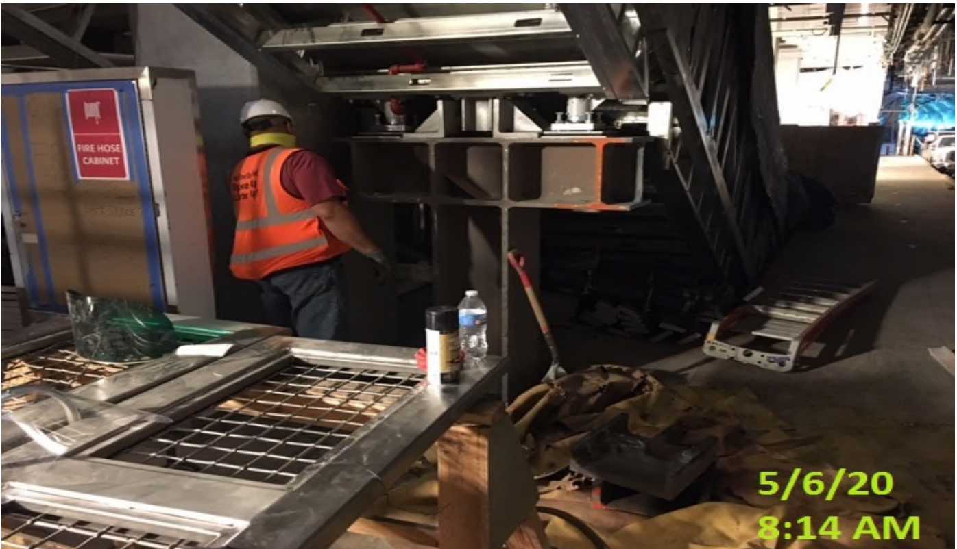
MLK Station - MLK – Ironworkers cutting escalator support column at platform.
