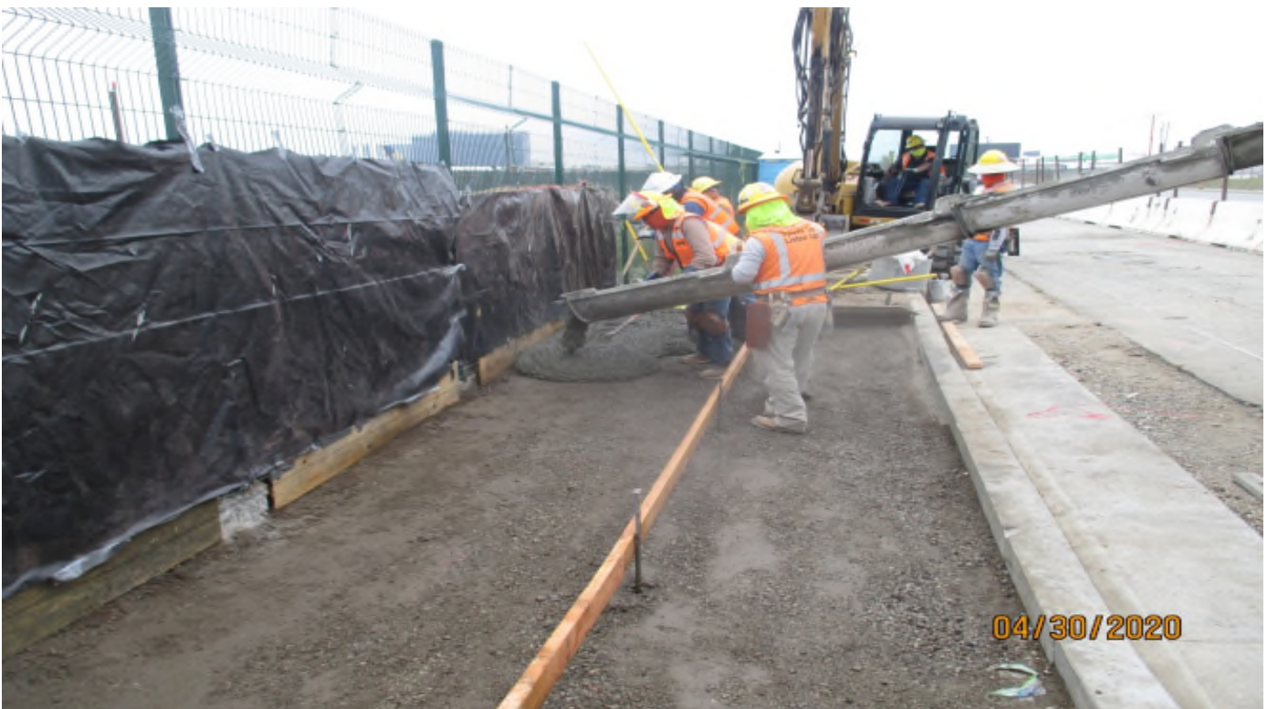
UG1 – Placing concrete for a driveway at UG-1.
