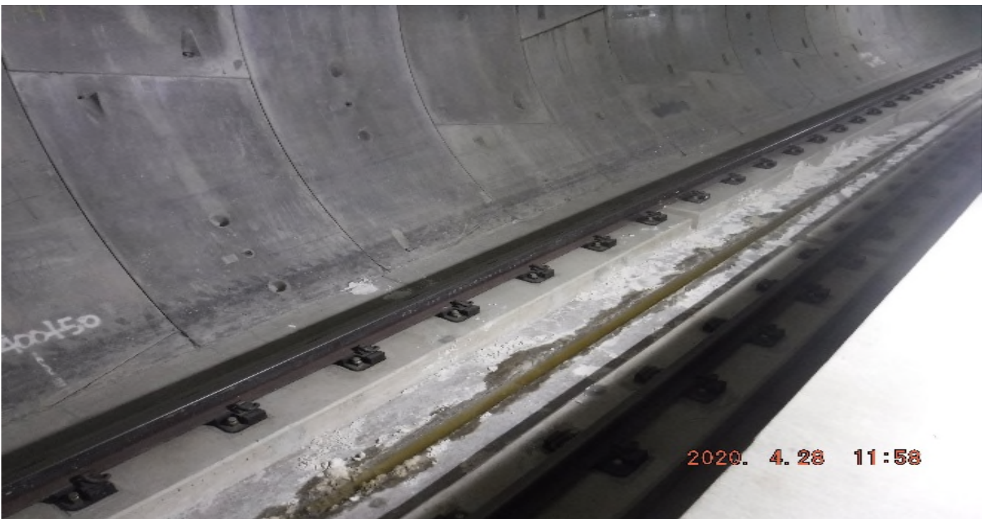
UG-4- STA 400+50 TK#4/NB looking south – minerals on UG4 invert between Vernon & MLK.
