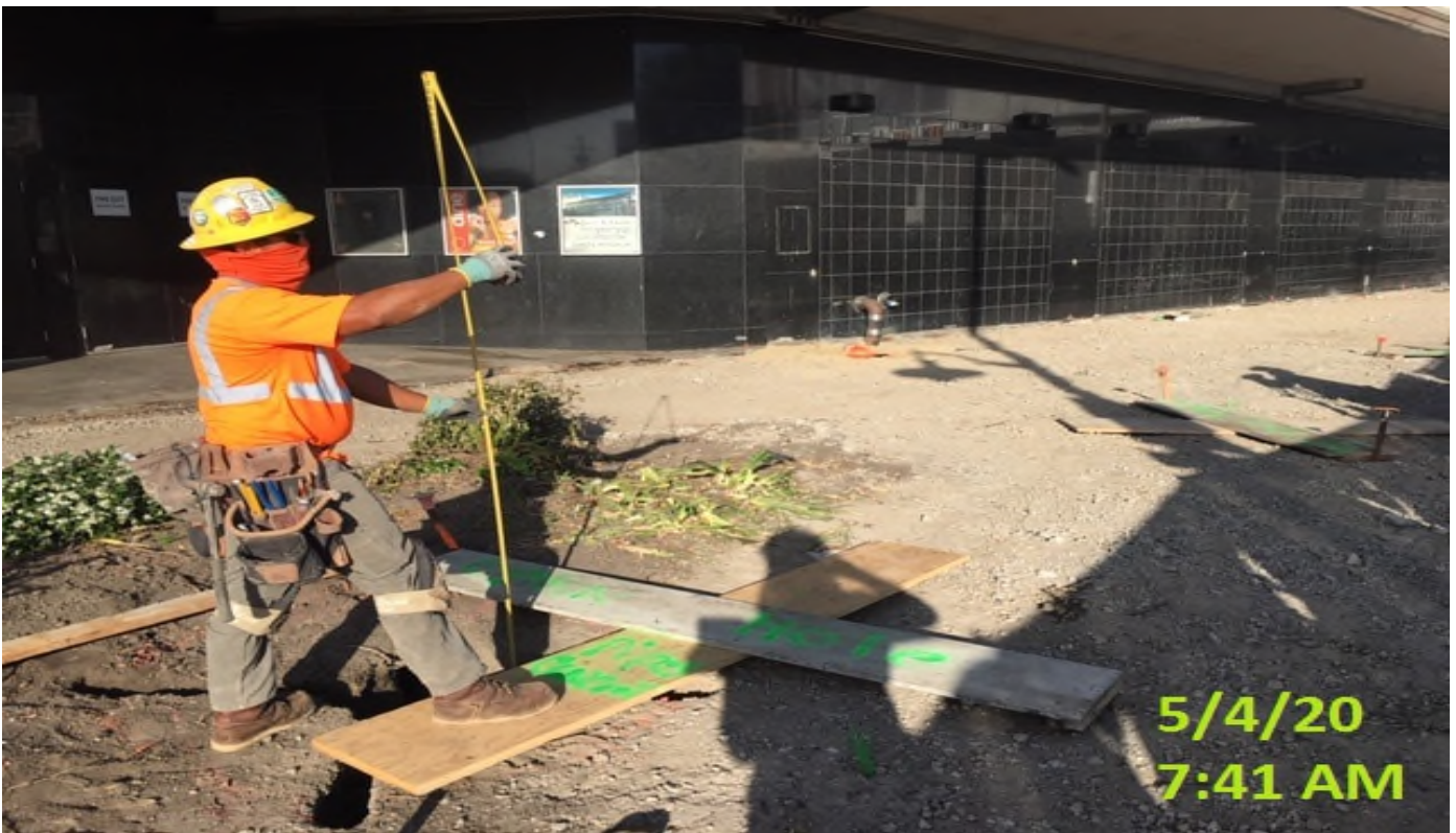
Crenshaw/Expo - EXPO – WSCC crew drilling and measuring for tree wells
