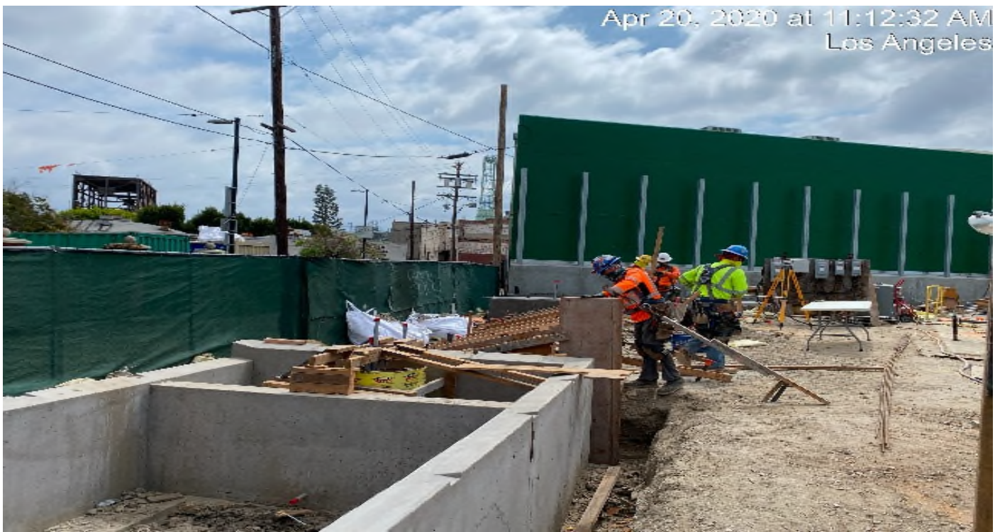
Crenshaw/Vernon - WSCC placing forms for the planter section at Vernon.
