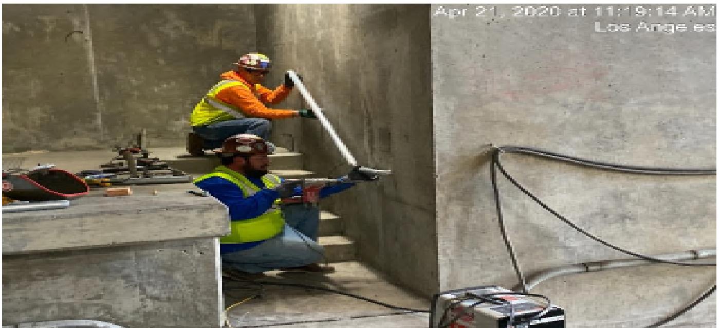
UG3 – Continue handrail installation at the north end stairs at Sta 311+00.
