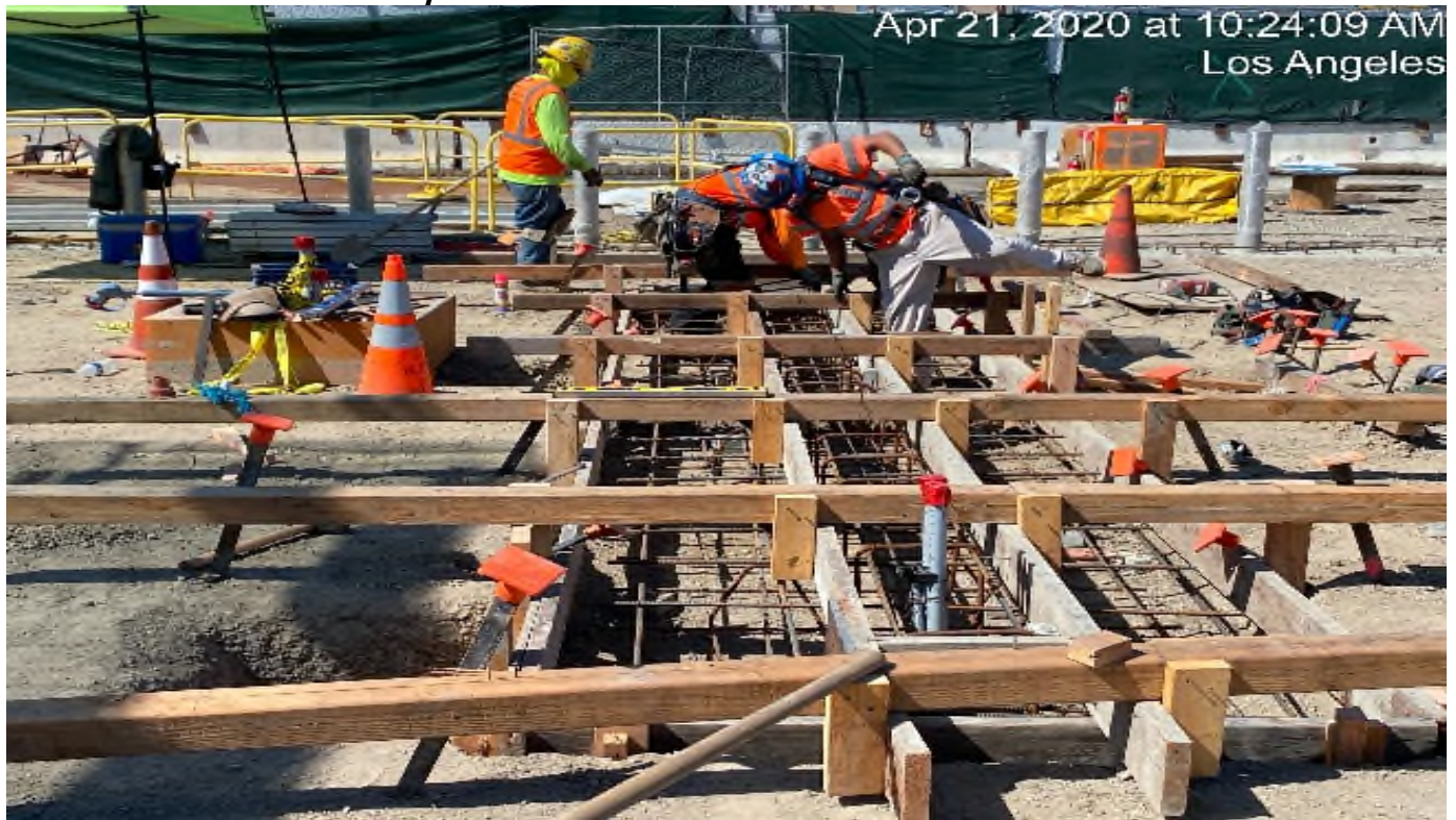
Crenshaw/Vernon - WSCC placing forms for the map case at Vernon..
