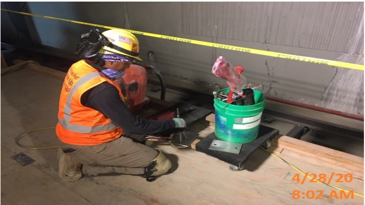
Crenshaw/MLK - MLK – WSCC Ironworkers installing header for platform end gates.
