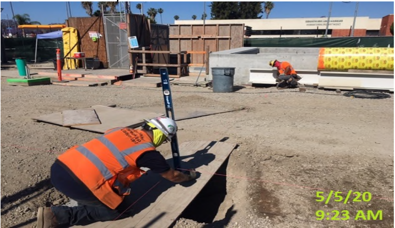
Crenshaw/Expo - EXPO – WSCC crew layout and adjusting measurements for plaza lighting.
