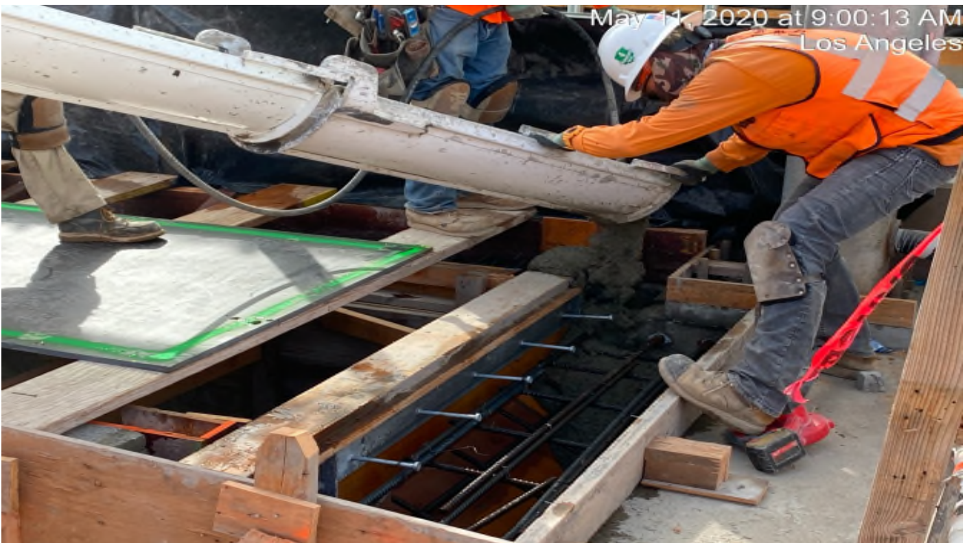
Crenshaw/Vernon - WSCC placing concrete for Bilco hatch at Vernon.
