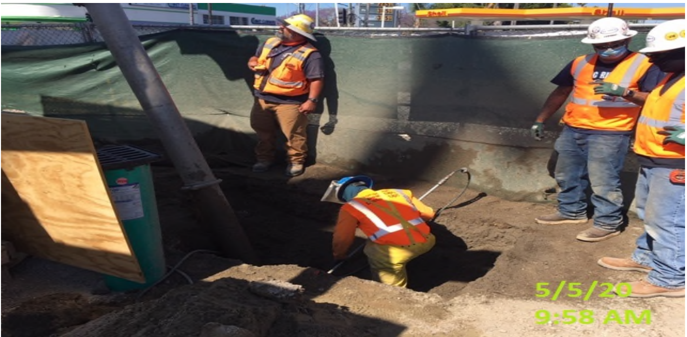
Crenshaw/Expo - EXPO – JF Shea potholing for conduit bank for Neal.
