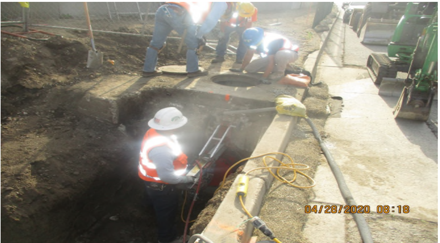
Florence/La Brea – WSCC Core hole in CB west of La Brea on W/B Florence.
