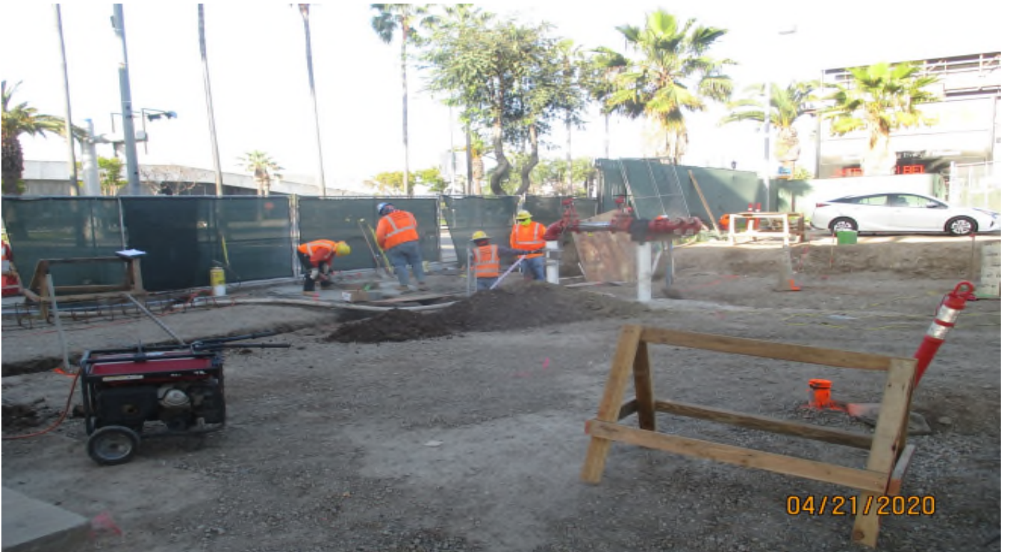
Aviation/Century – Stripping light pole foundation forms at Aviation Station.
