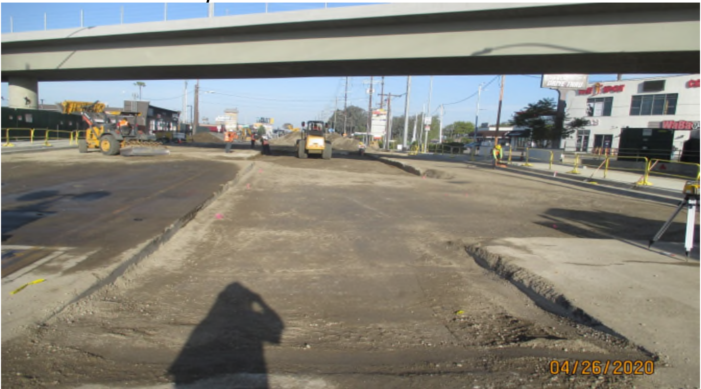
MANCHESTER STREET- Start of base placement this morning at Manchester.
