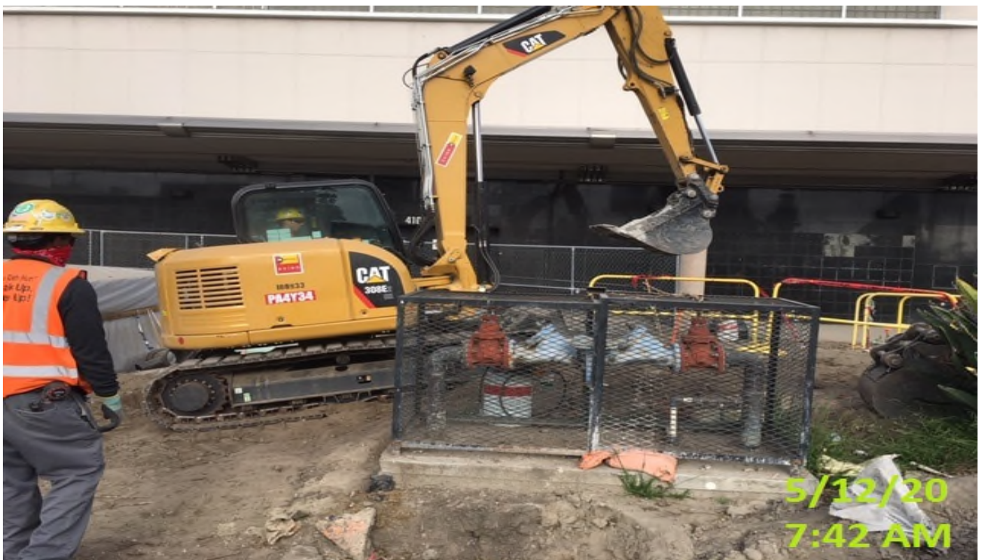
MLK – WSCC excavating to continue laying 12" HDPE drain line
