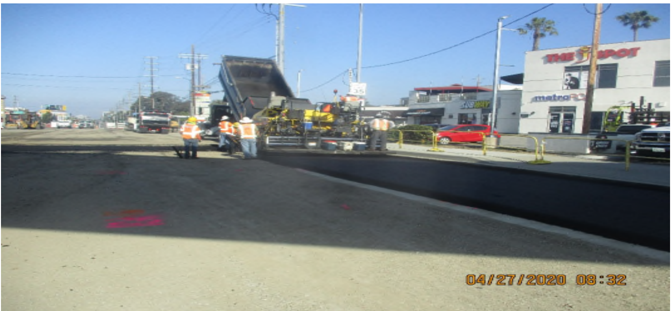
Manchester Bridge – WSCC Sully Miller Paving 8” of AC at Manchester crossing.
