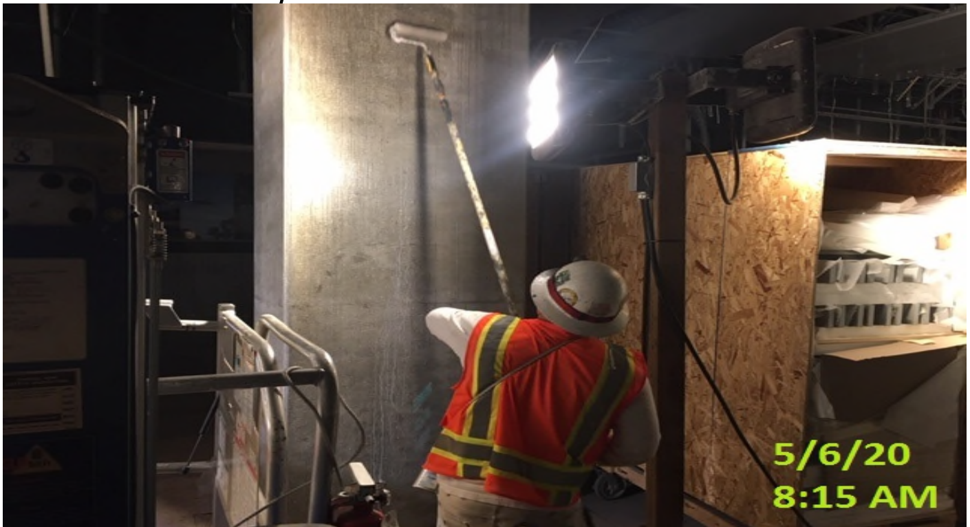
MLK – Mariscal Painting applying sealer to columns prior to anti-graffiti finish
