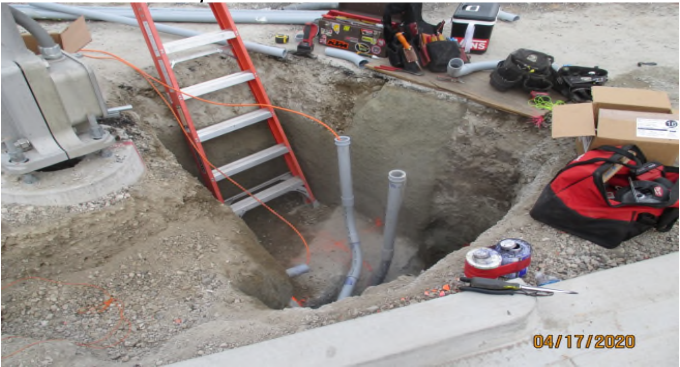
HINDRY STATION- Traffic signal pull box and conduit relocation at Hindry.
