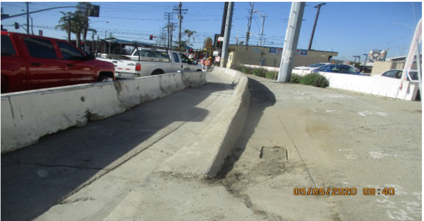
Manchester Bridge - WSCC Make Krail removals at Manchester and Florence.
