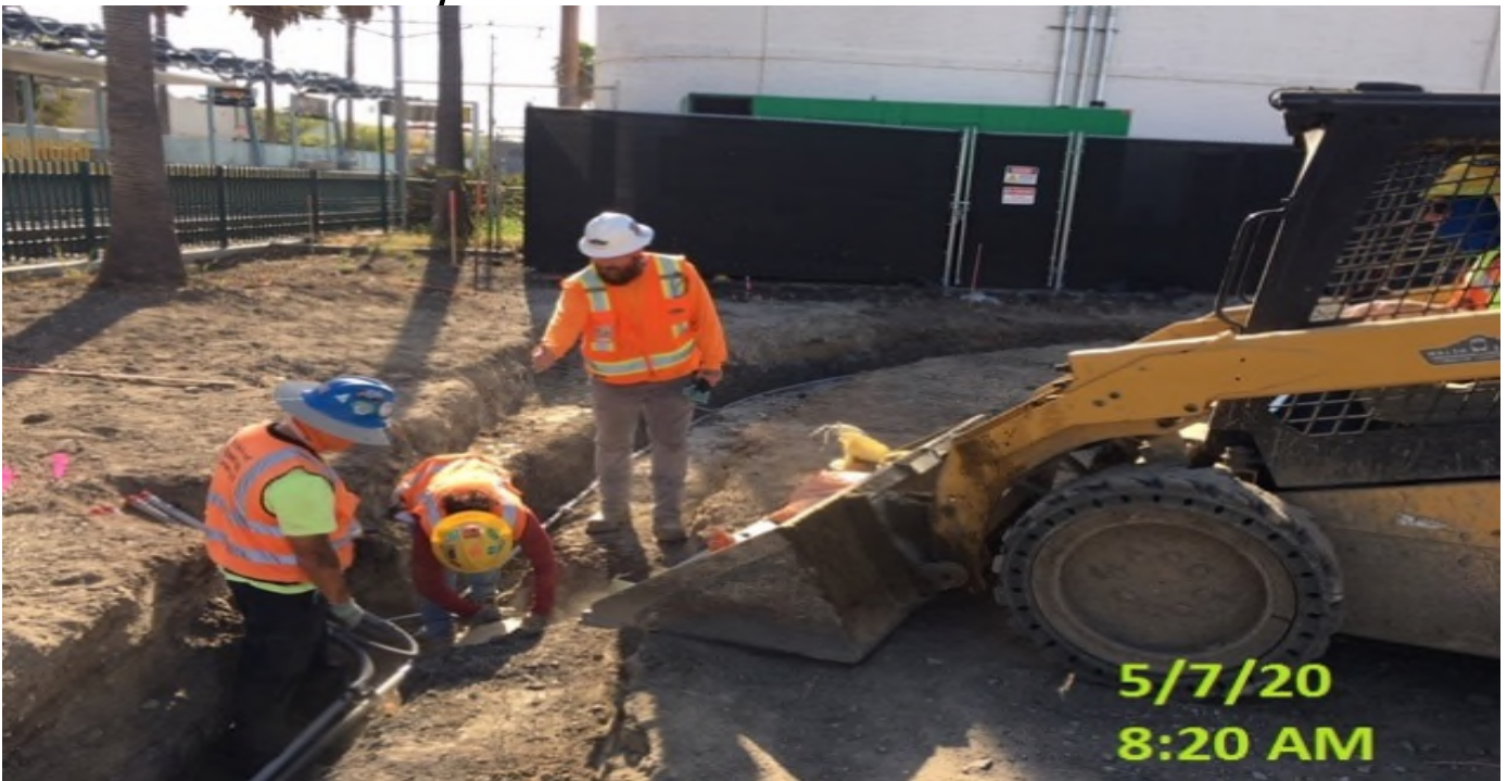
EXPO – WSCC crew bulk heading trench and prepping for concrete placement.
