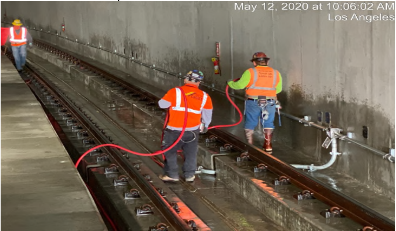
UG4 - WSCC pressure washing concrete at UG-4.
