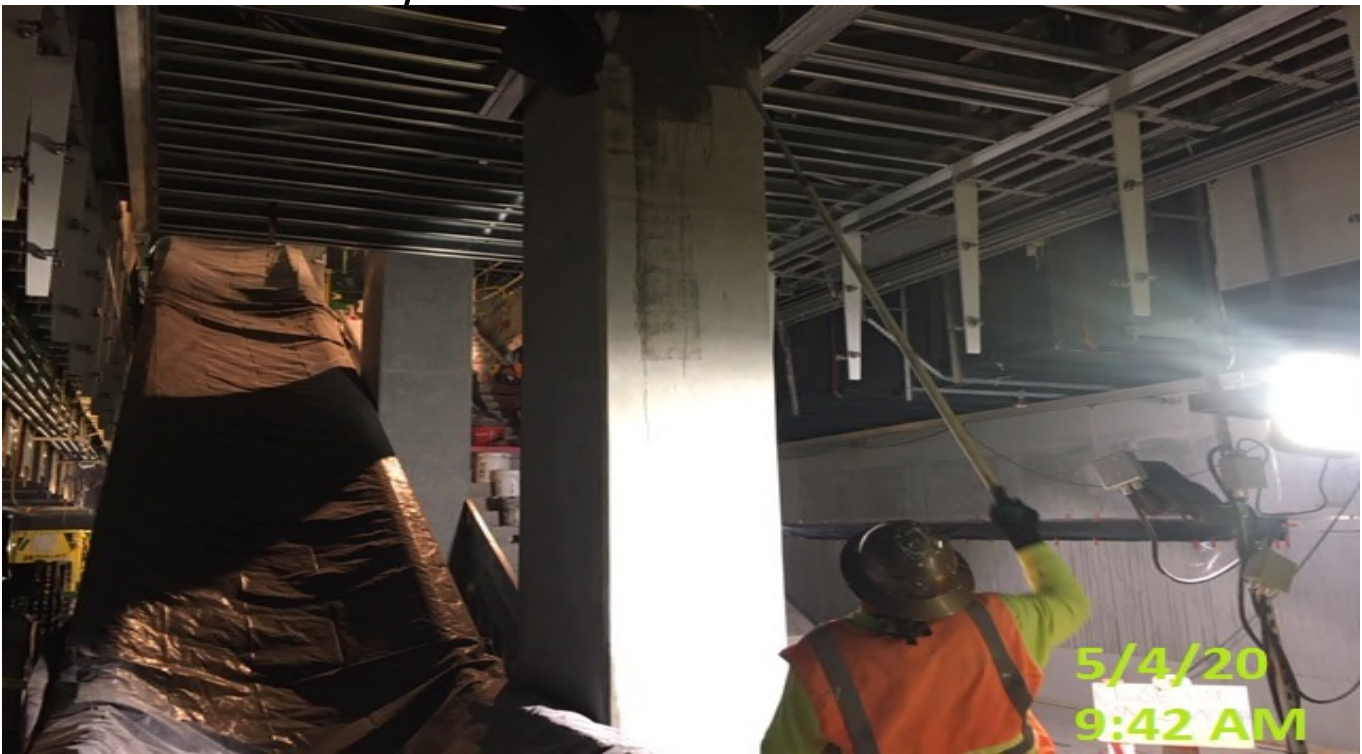
Crenshaw/Expo - EXPO – Mariscal Painting applying prep anti-graffiti finish to columns.
