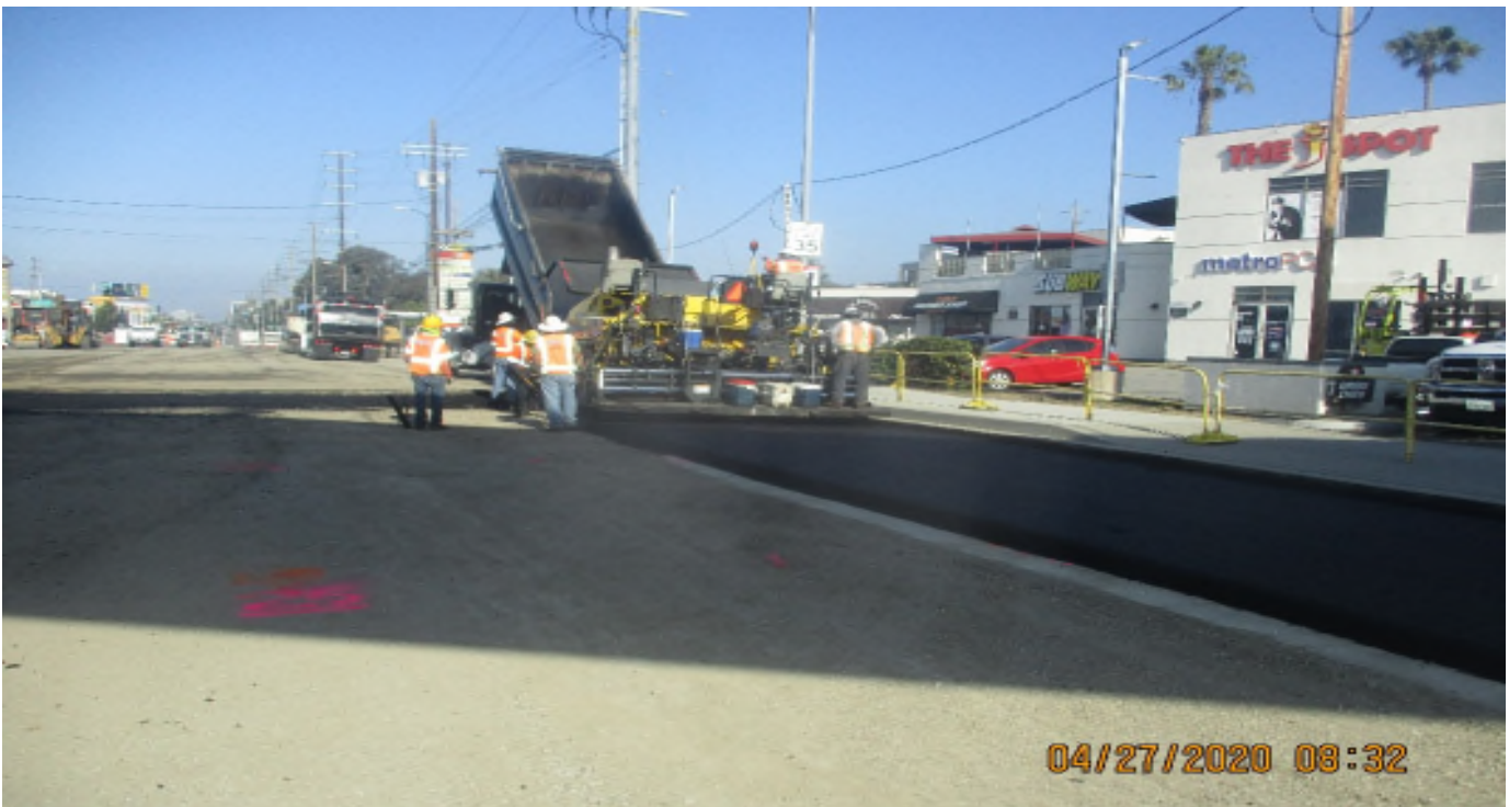
MANCHESTER STREET- WSCC Sully Miller Paving 8" of AC at Manchester crossing.
