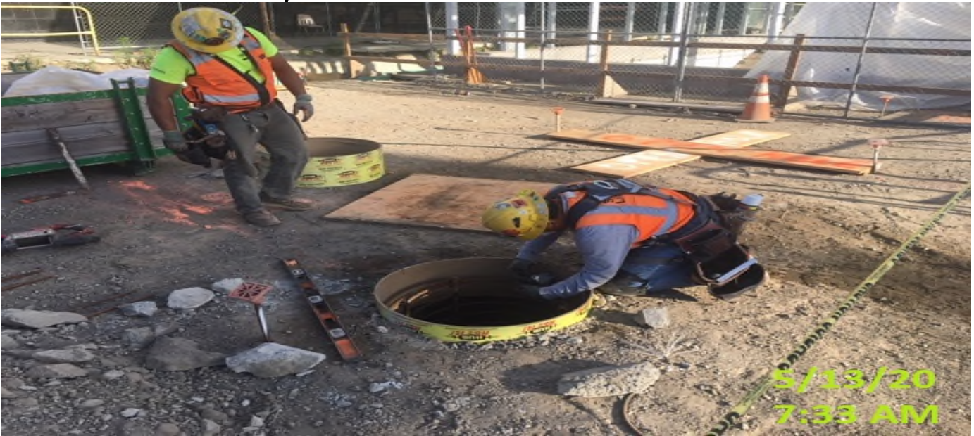
MLK STATION – Setting rebar into sonotube formwork for pedestrian light pole foundations throughout the plaza level.
