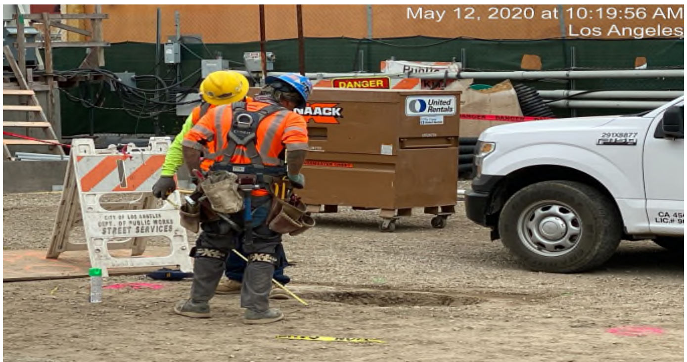
Crenshaw/Vernon - WSCC laying out tree locations at Vernon.
