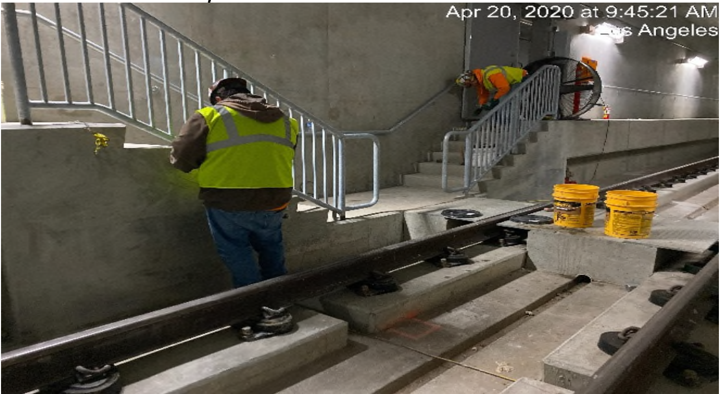
UG3 – McMahon installing handrail at UG-3.
