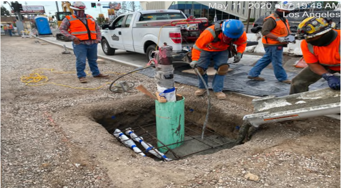
Crenshaw/Vernon - Placing concrete for vent stack at Vernon.
