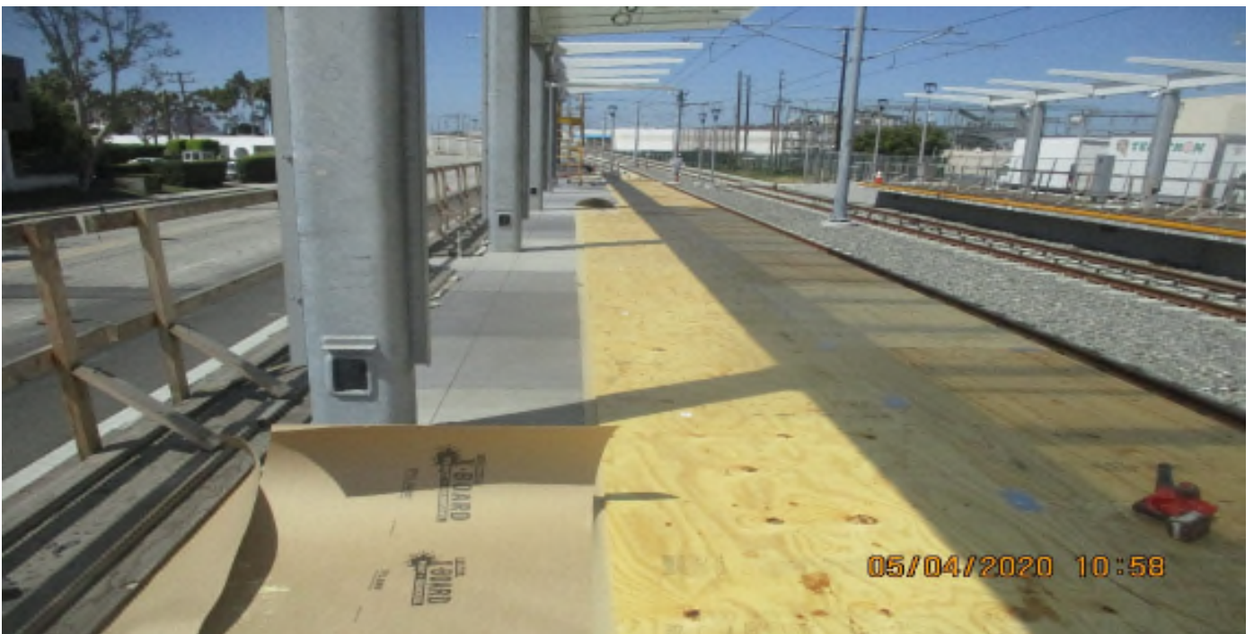
HINDRY STATION- WSCC Place protective ply wood on Hindry platform.
