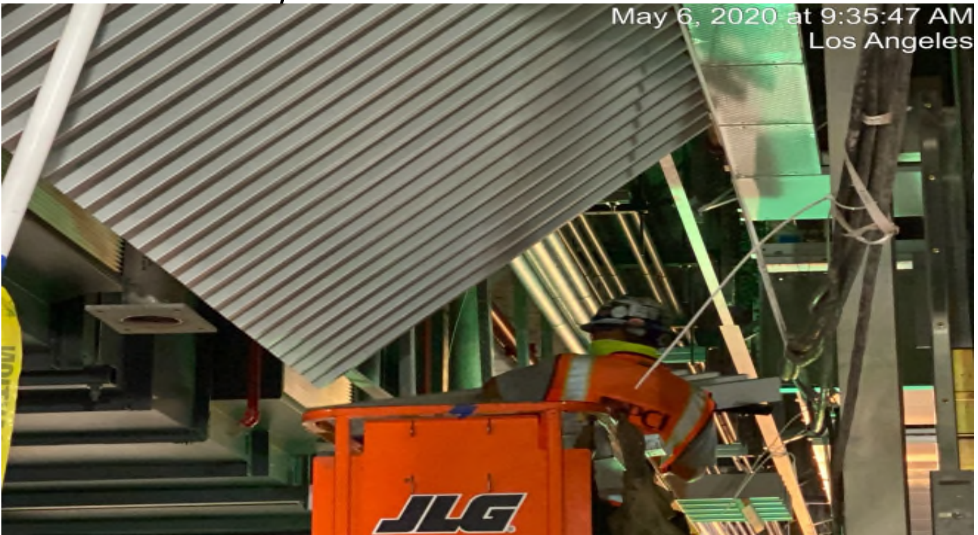
Crenshaw/Vernon - PCI Re-installing bar panels at Vernon.
