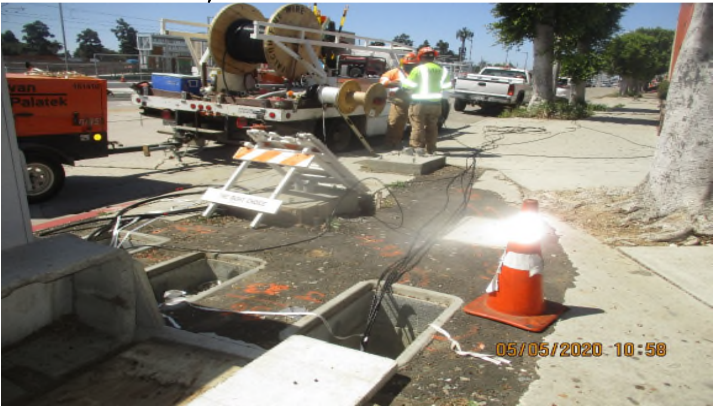
Florence/West – Select Electric Pull cable for all of Redondo/West intersection.
