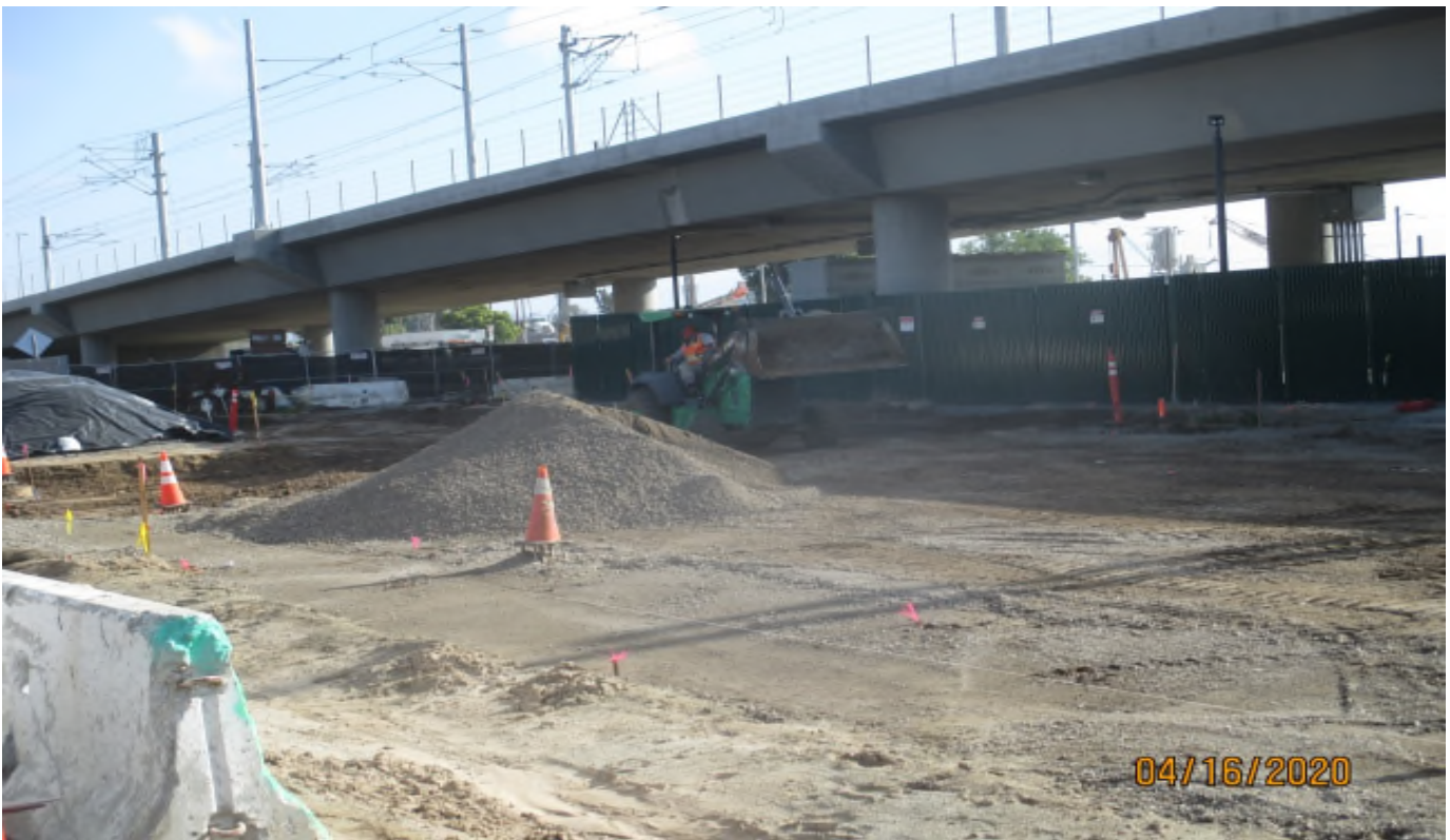
Aviation/Century – Grading the subgrade at Aviation Station.
