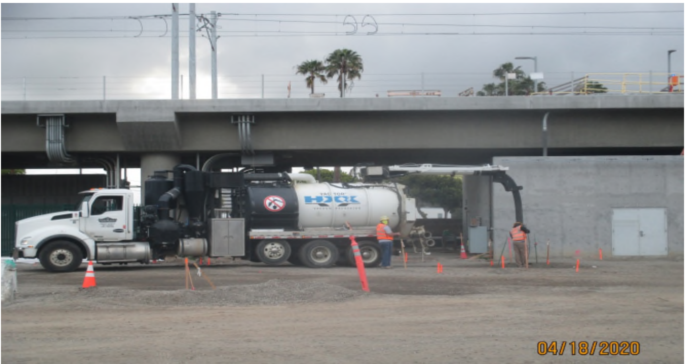
Aviation/Century – Vacuum truck excavating light pole foundations at Aviation Station.
