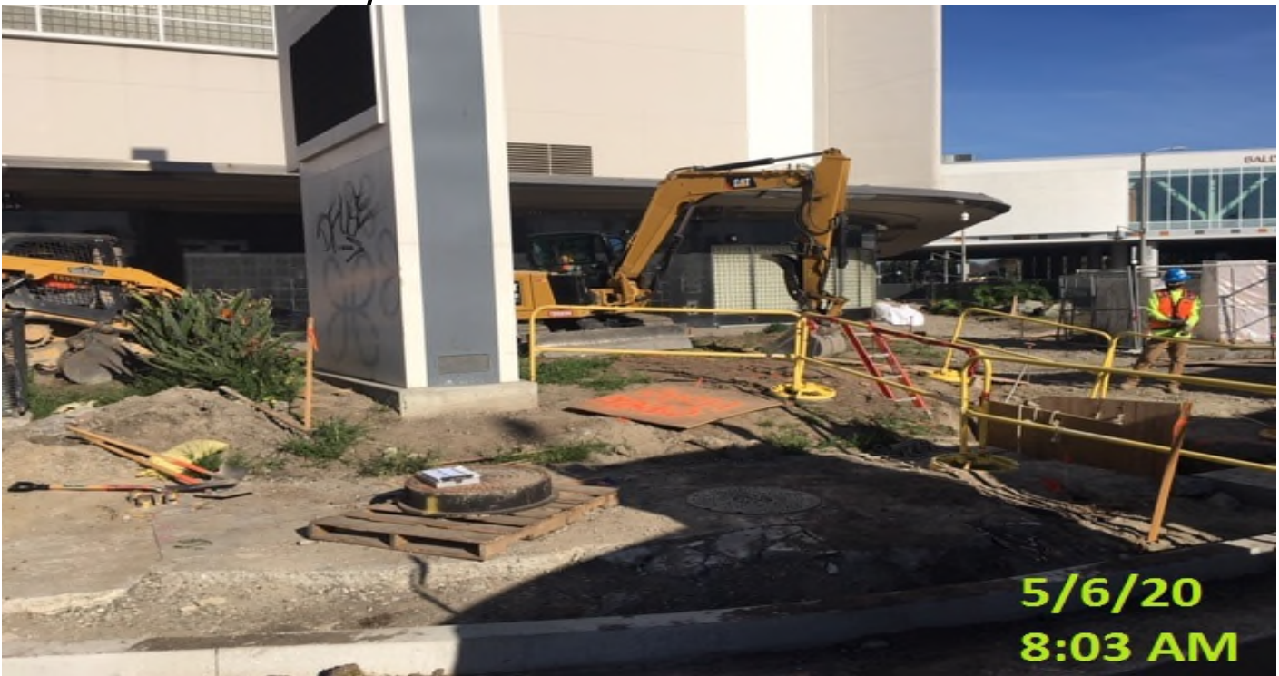
MLK Station - MLK – WSCC crew trenching for HDPE 12” drain pipe.
