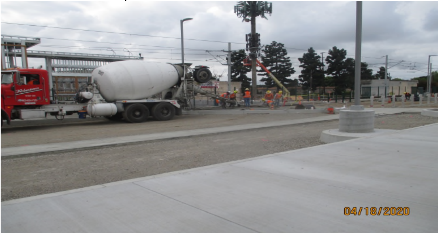
Florence/West – Placing concrete for the sidewalk at West Station.
