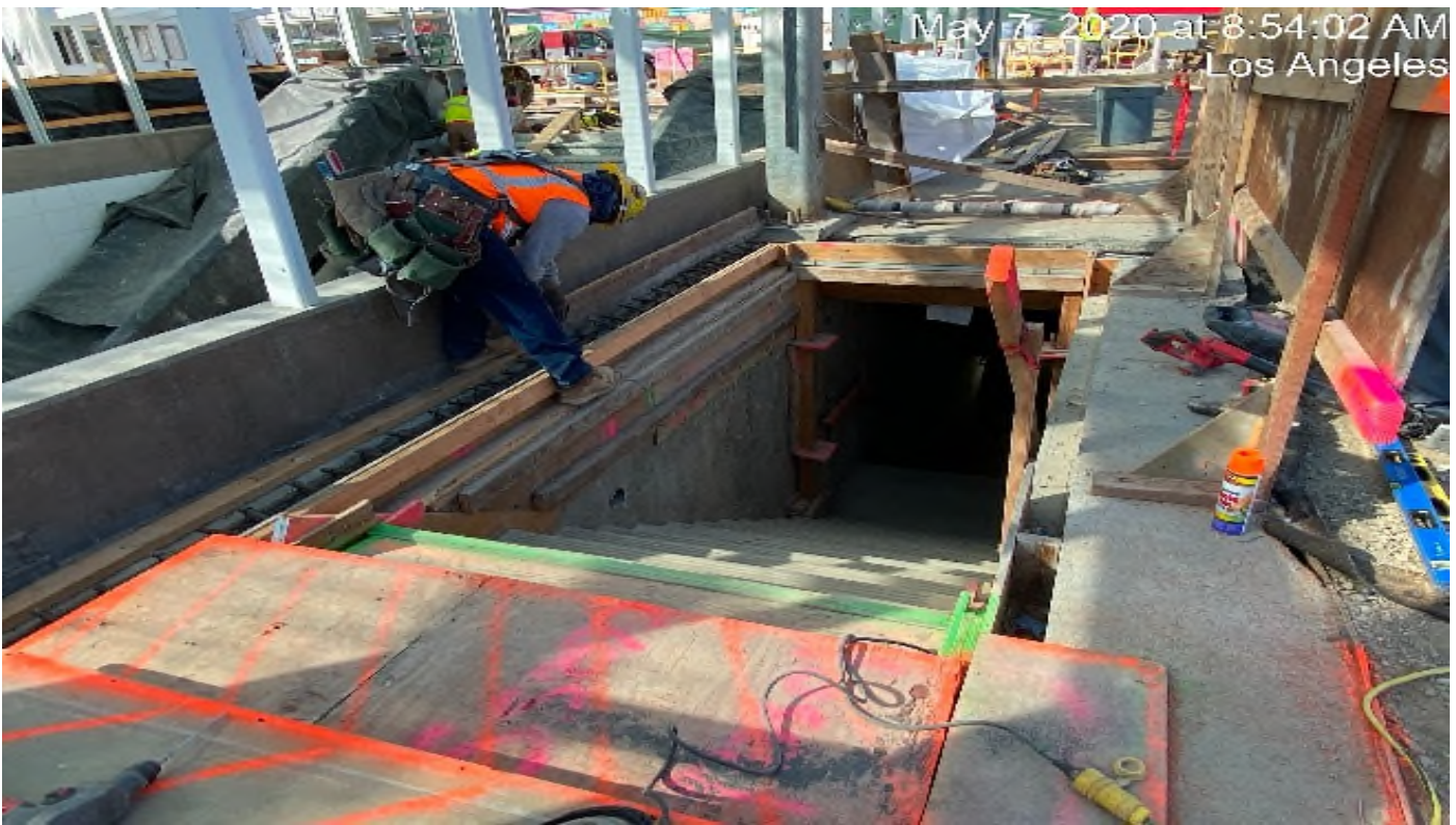
Crenshaw/Vernon - WSCC drilling for emergency hatch at Vernon.
