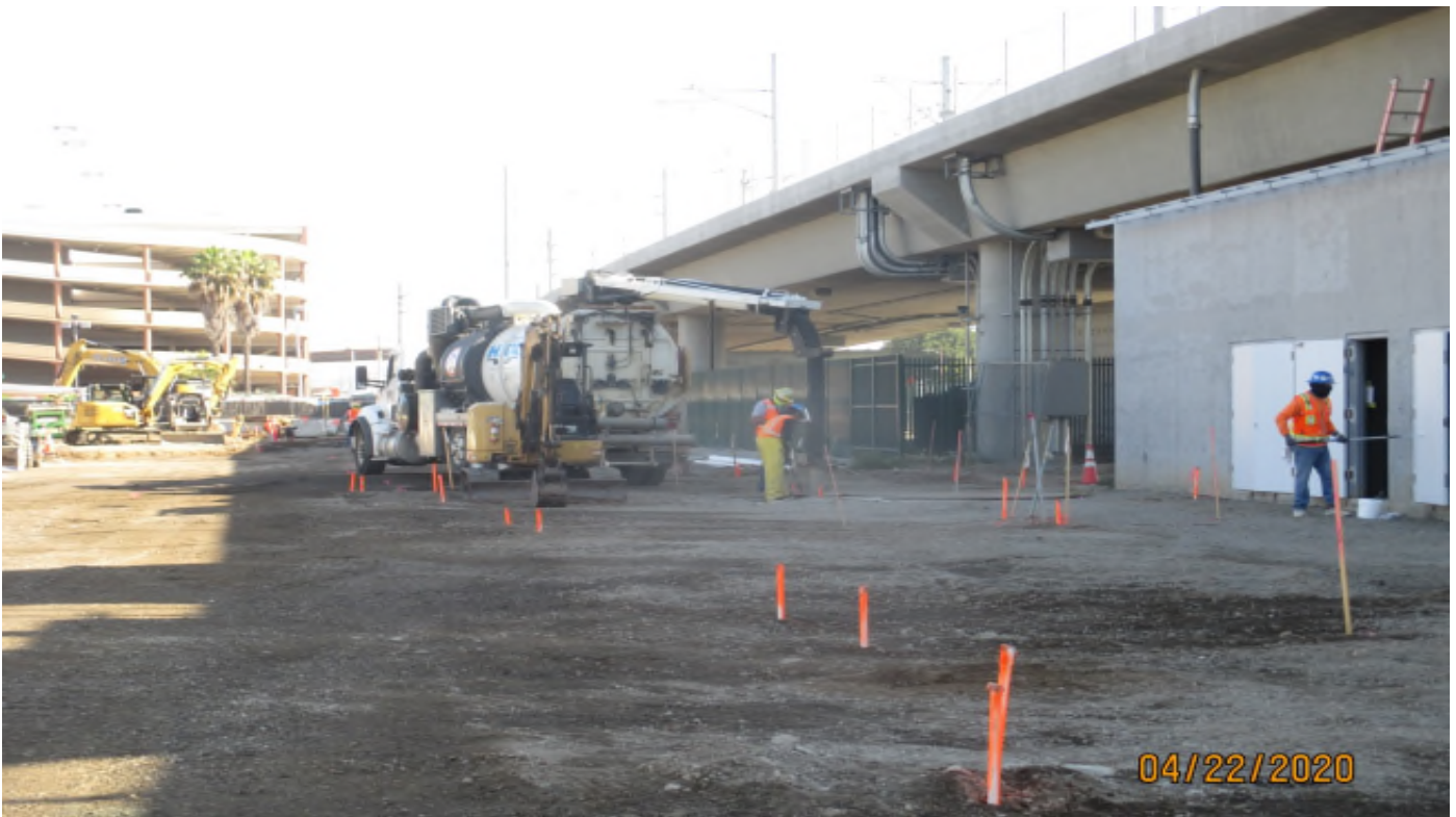
Aviation/Century – Base grading at the Aviation Station.
