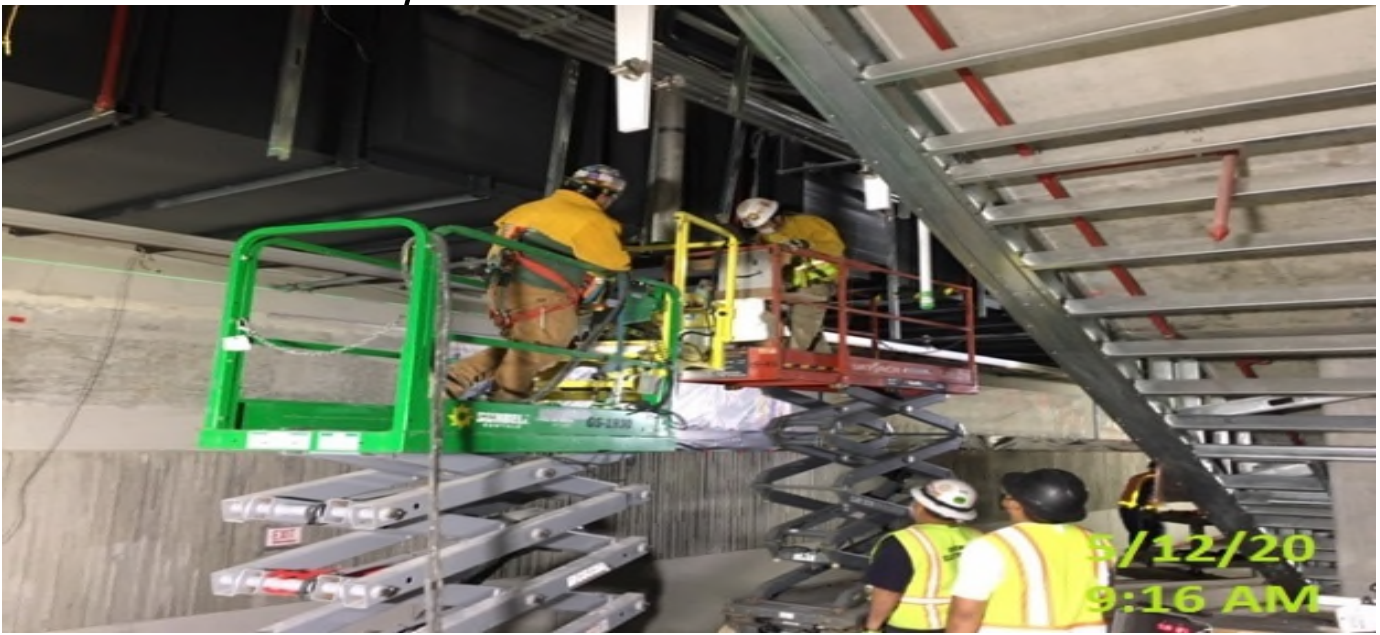
EXPO STATION – Continue welding supports posts for the platform edge lighting.
