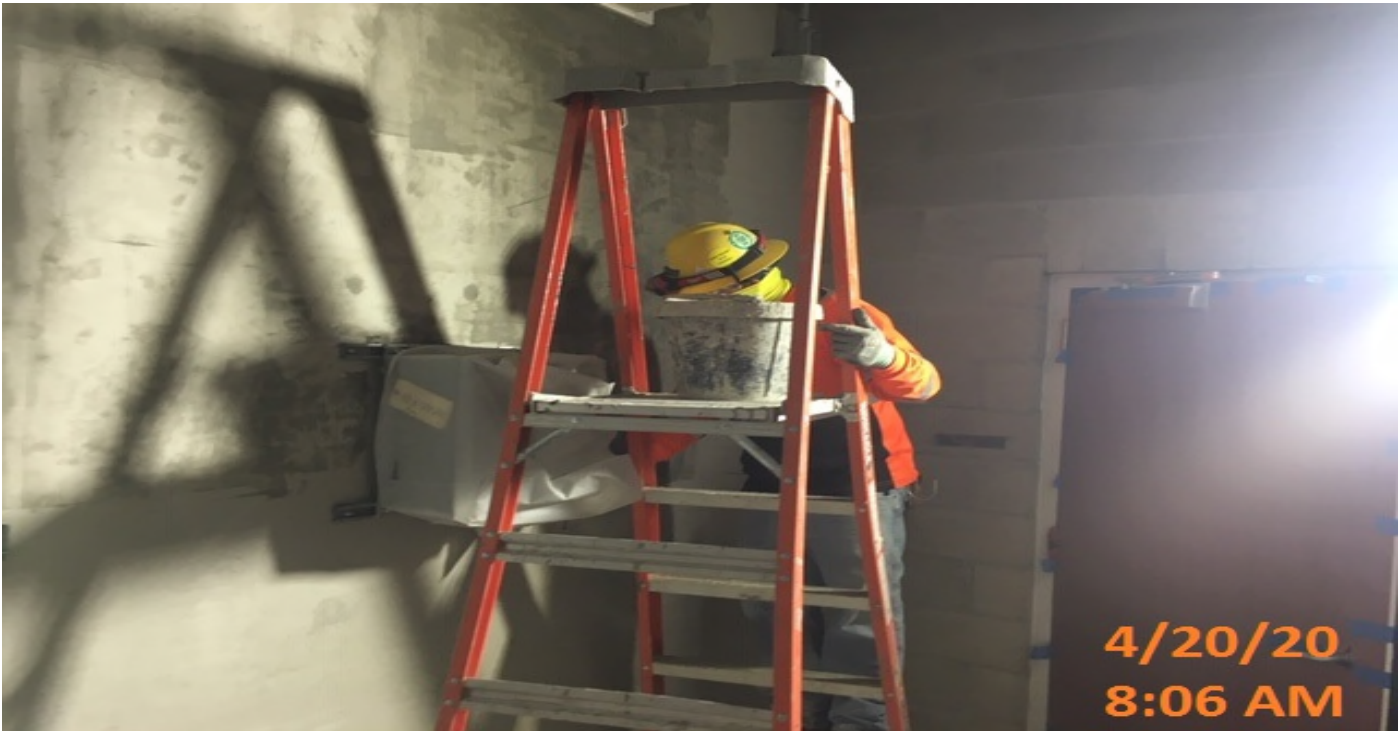
Crenshaw/MLK - MLK – WSCC crew excavating for new 12” drain pipe.
