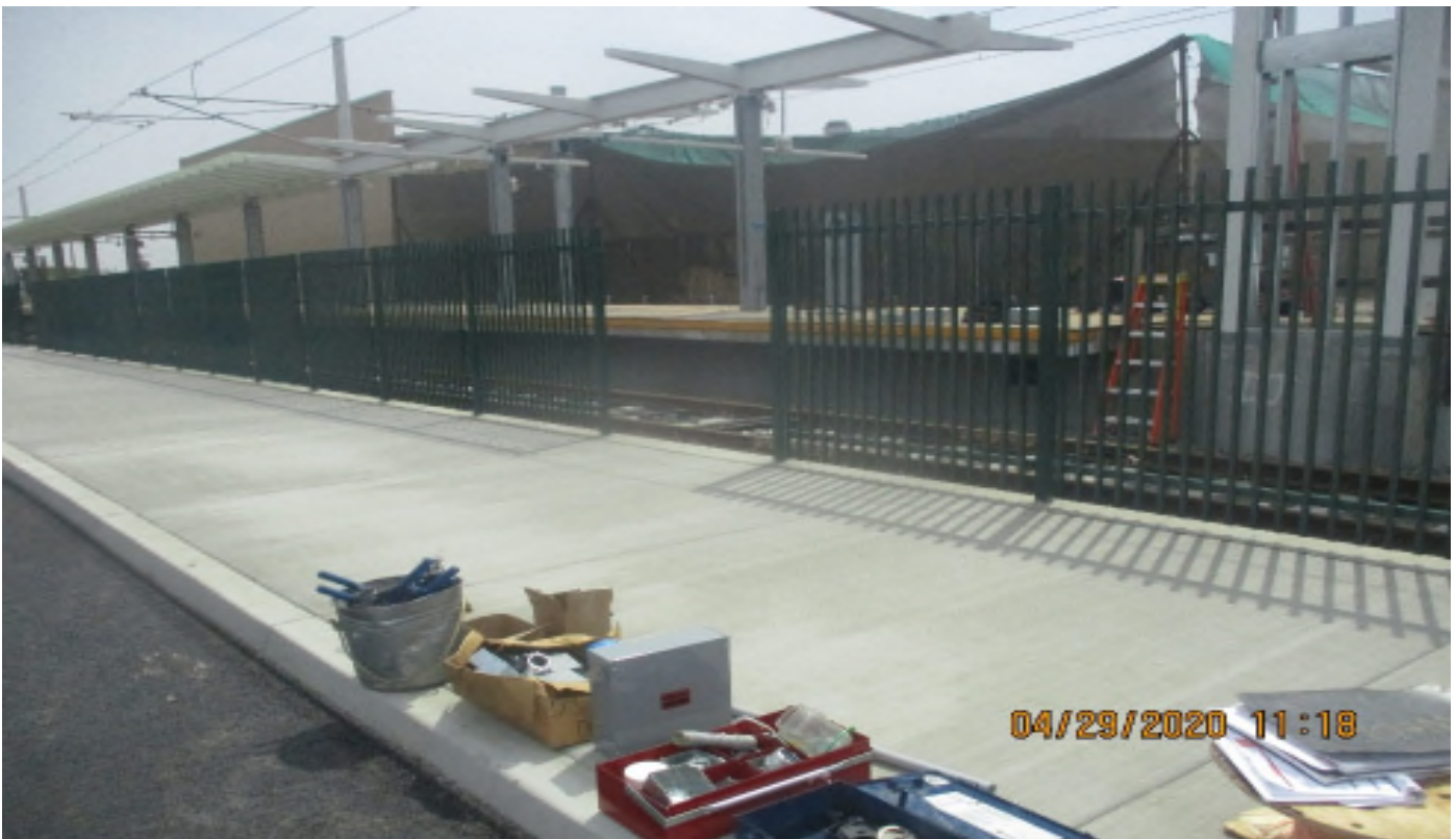
Florence/West – ACE fence place fence panels at West St Station.
