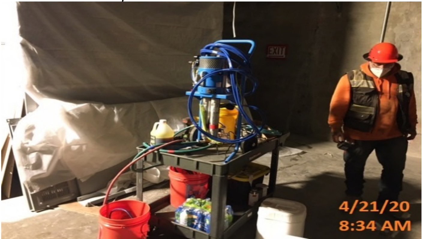
Crenshaw/MLK - MLK – MLK – Keller injecting new resin material into grout boxes.
