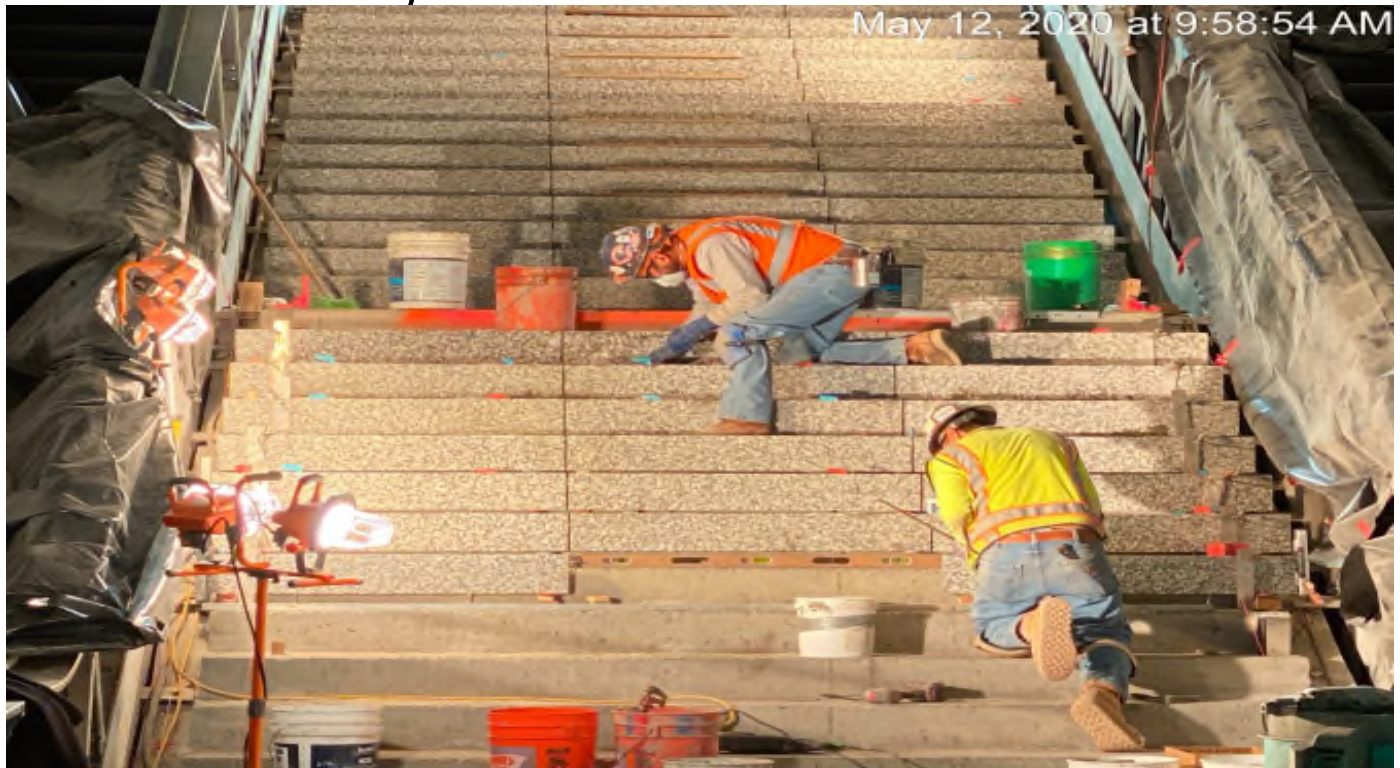
Crenshaw/Vernon - Carrera installing stair treads and risers at Vernon.
