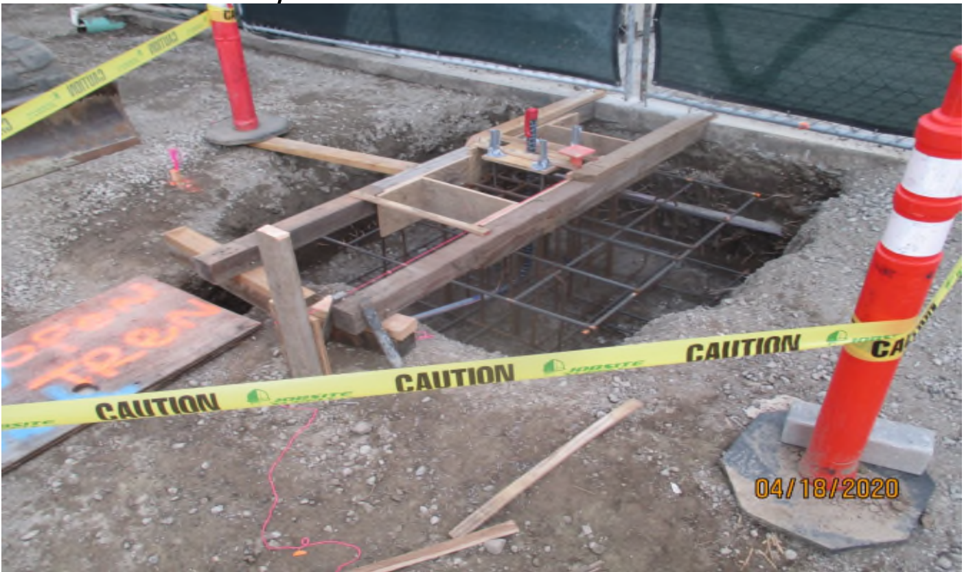
Aviation/Century – Formed light pole foundation at Aviation Station.
