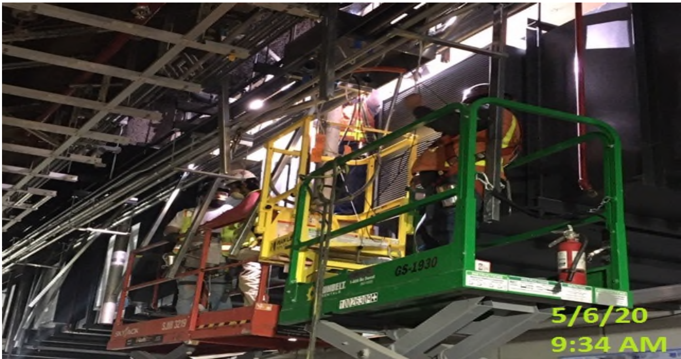
EXPO STATION – Resume welding for the platform edge lighting support posts.
