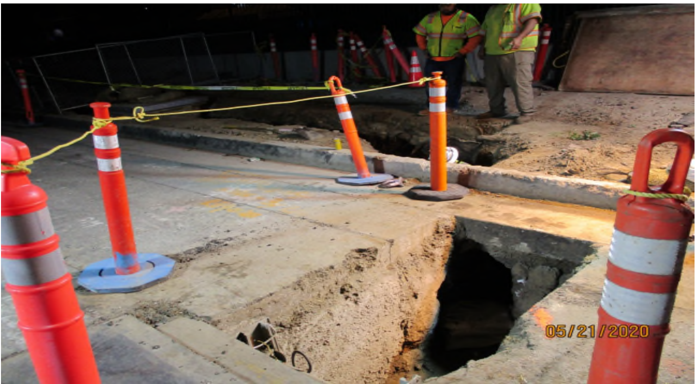
111 th Street – Fire line trench turn at 111th street.
