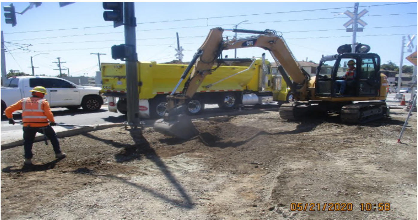
Florence/West – STA 265+00 TK#4/NB looking north – grading work outside ballast wall.
