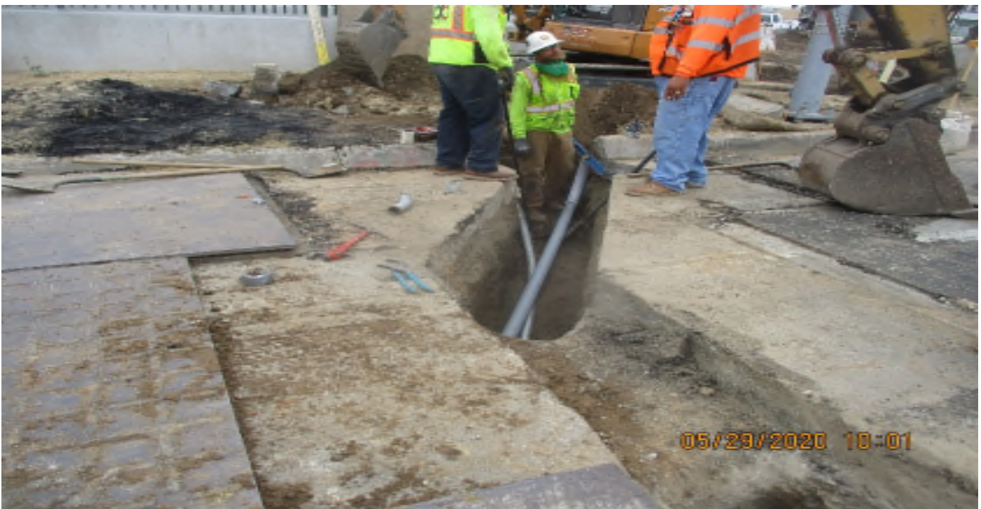
Aviation/Century – DB Electric place conduit across Aviation at 104th.
