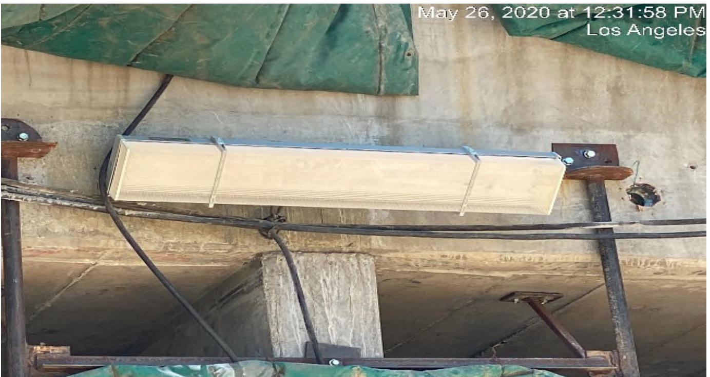
UG3 – Installing outdoor lighting at the south end portal entrance.
