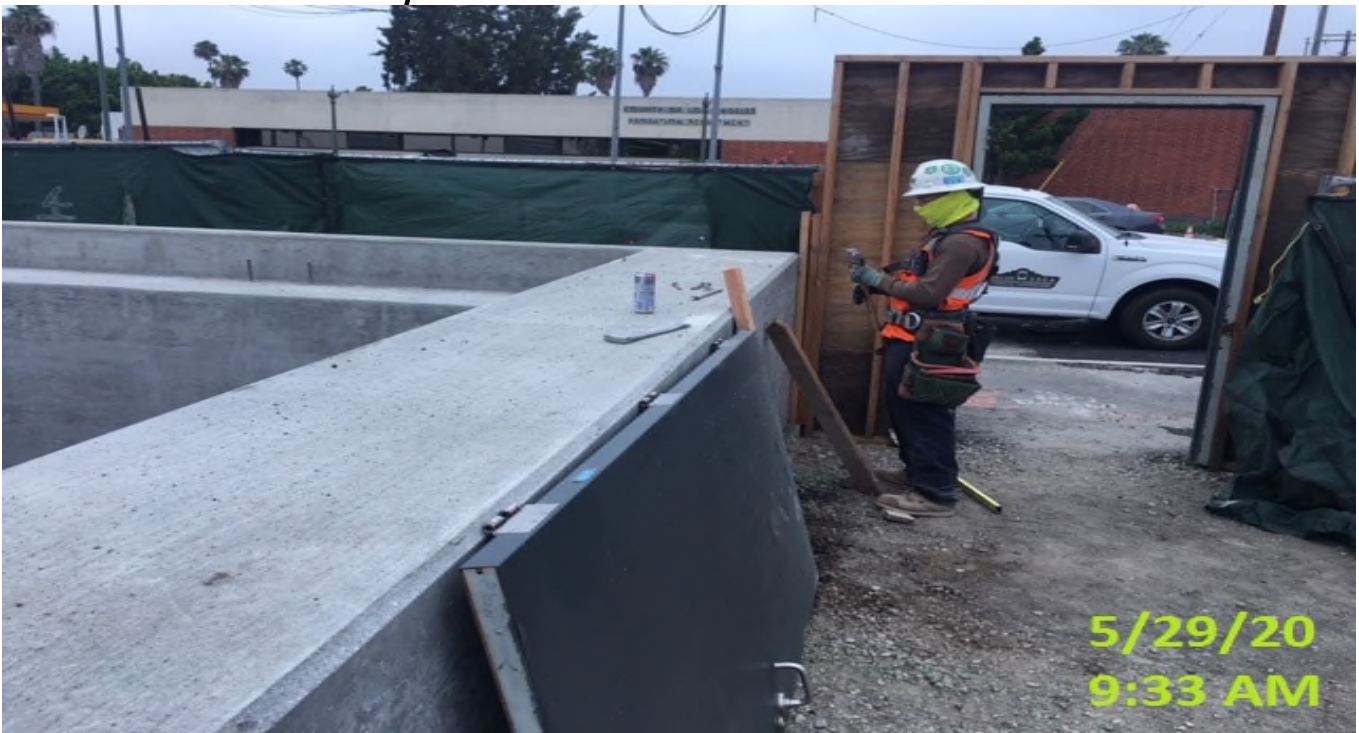
Crenshaw/Expo - WSCC carpenters relocating new temporary entrance for station
