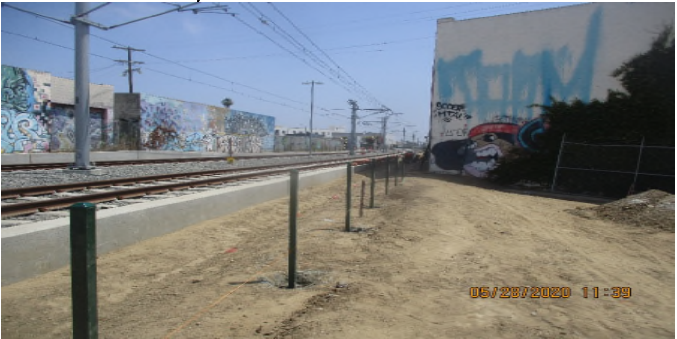
Florence/West – ACE Fence Place fence posts at East Bound Florence W-High
