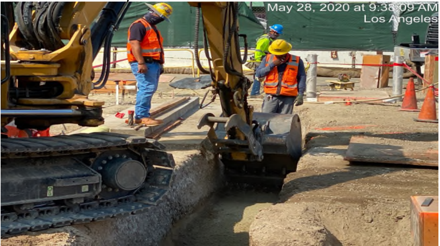
Crenshaw/Vernon - WSCC excavating for electrical trenches at Vernon.
