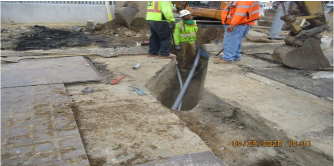
Aviation/Century – DB Electric place conduit across Aviation at 104th.
