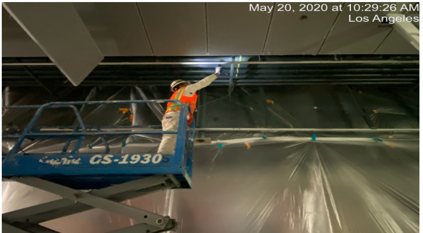
Crenshaw/Vernon - Mariscal painting conduit at Vernon.
