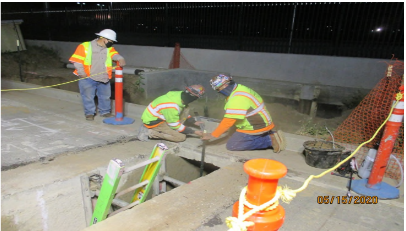
104 th Street - Fire line trench layout at 104th street.
