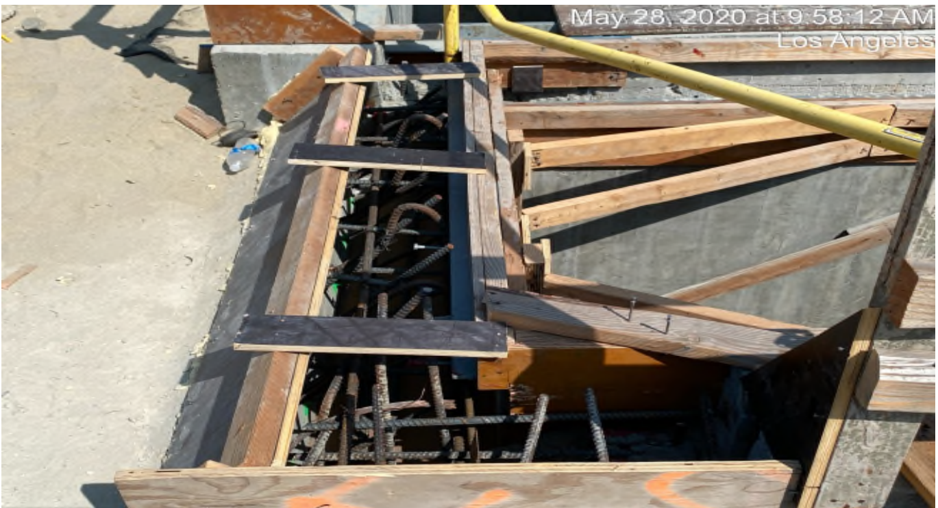
Crenshaw/Vernon - WSCC drilling and doweling the stairs at Vernon.
