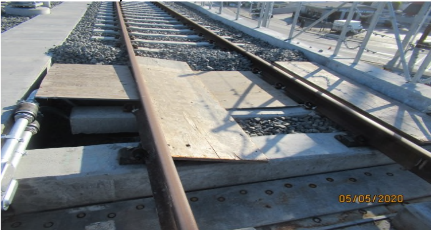
Manchester Bridge - Manchester Bridge NB #4 track STA 121+45 no condition changes for disturbed ballast . on Metro's Punch list, item #250 in Segment A.
