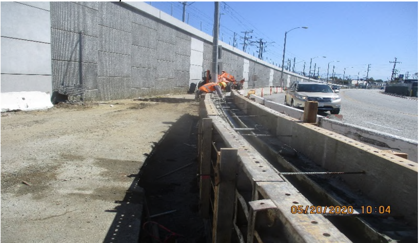
Manchester Bridge – WSCC Placed concrete for Krail at Manchester and Florence
