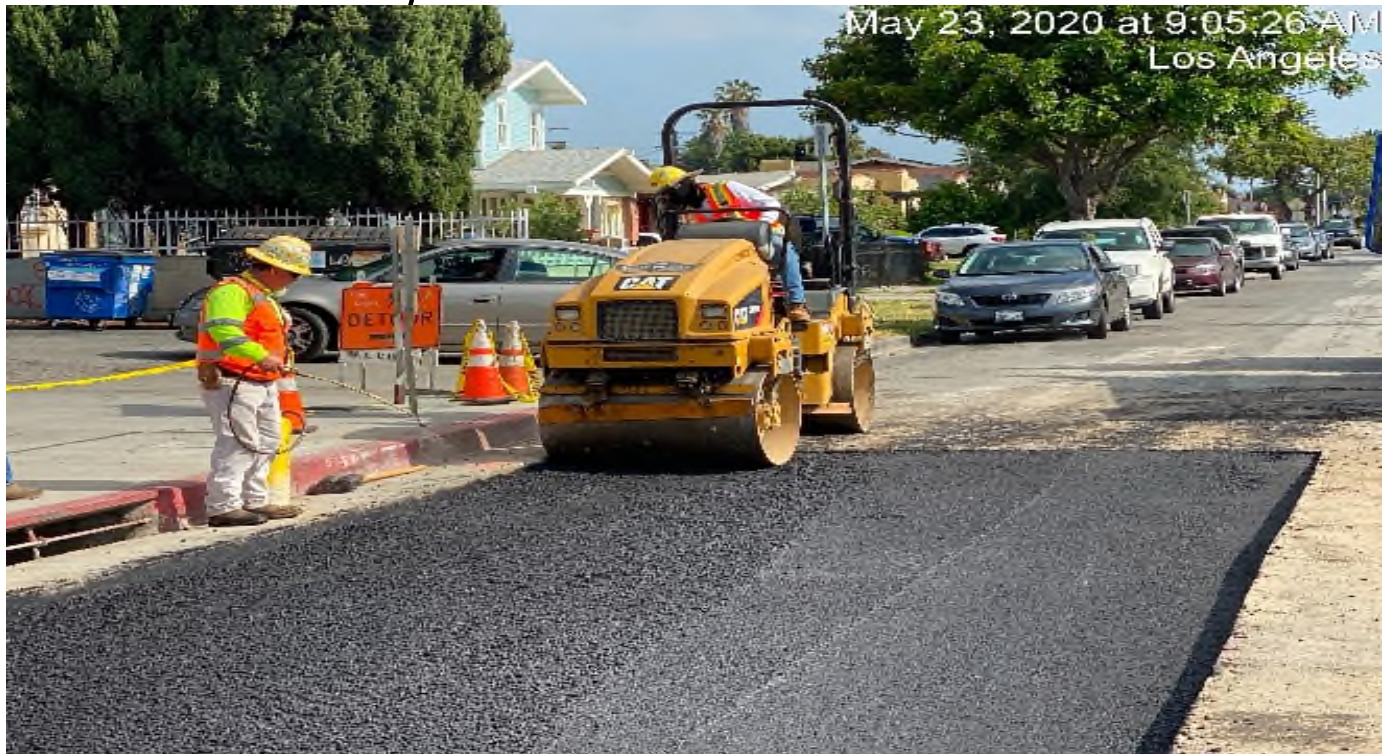
Crenshaw / Slauson – WSCC paving at Slauson and Victoria.
