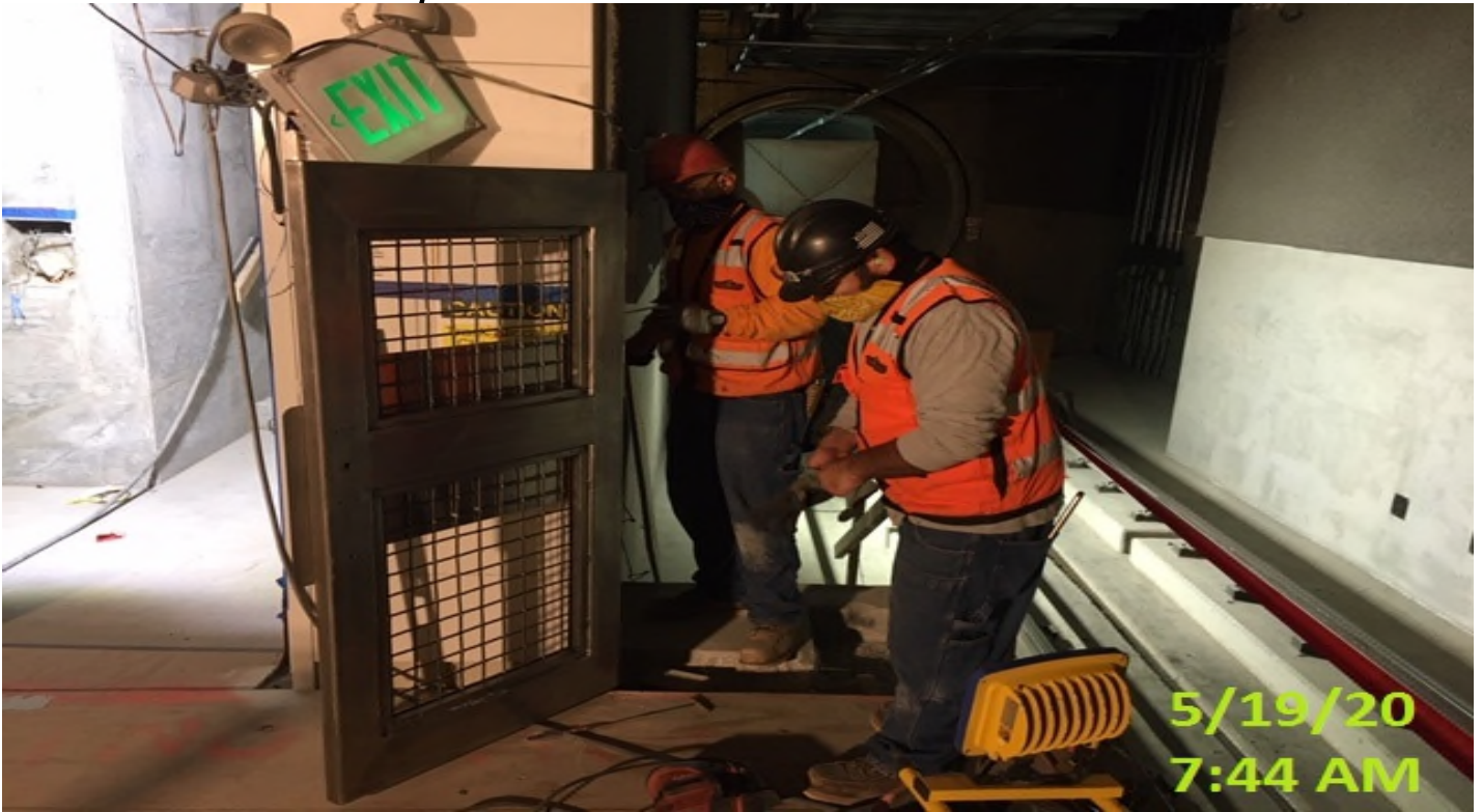
Crenshaw/MLK - MLK – Ironworkers installing side panel for platform end gates.
