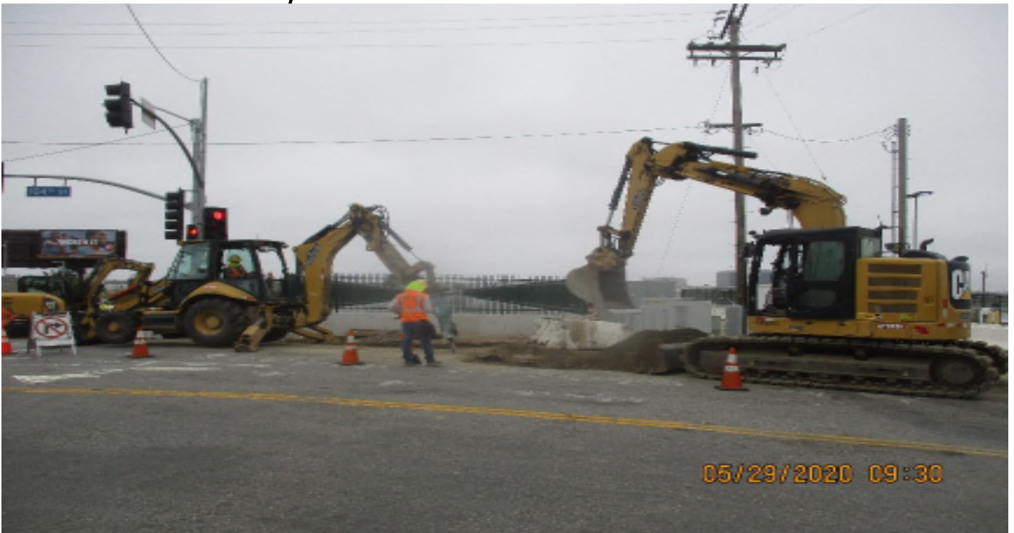
104 th Street - WSCC Making grade and removals at 104th for C&G.
