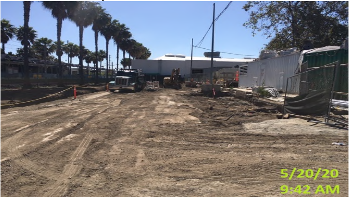
Crenshaw/Expo - WSCC crew grading to subgrade for top soil placement.
