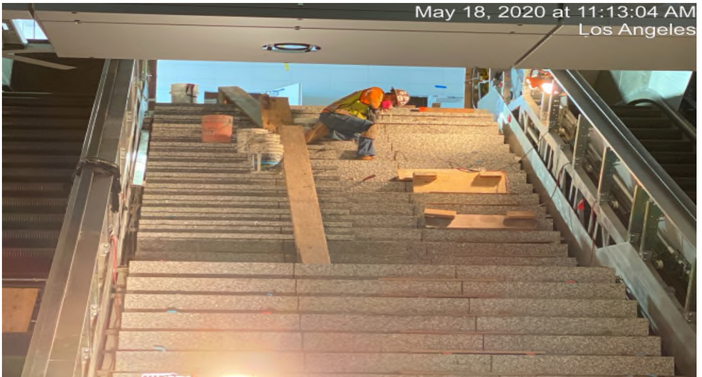
Crenshaw/Vernon - Carrera installing treads for the stairs at Vernon.
