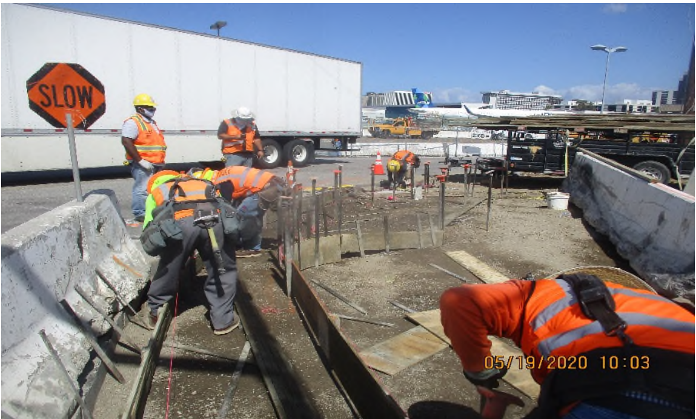
104 th Street - WSCC Place concrete C&G at 104th at crossing.
