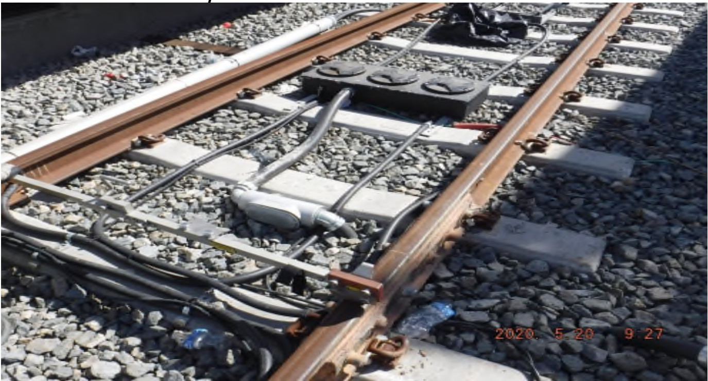
Florence/West – STA 263+66 TK#4/NB looking north – rail grind validation progress (West Station)
