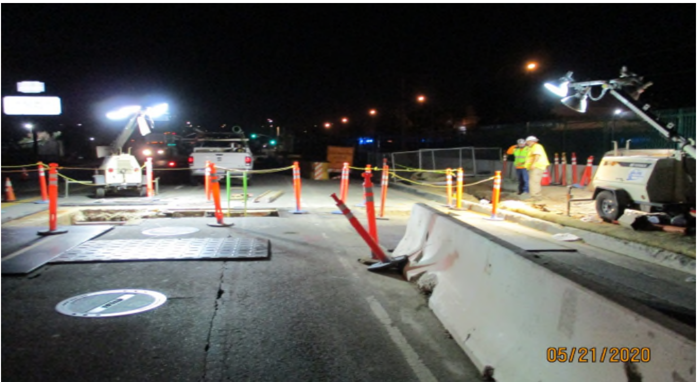
111 th Street – Fire line trench at 111th street.
