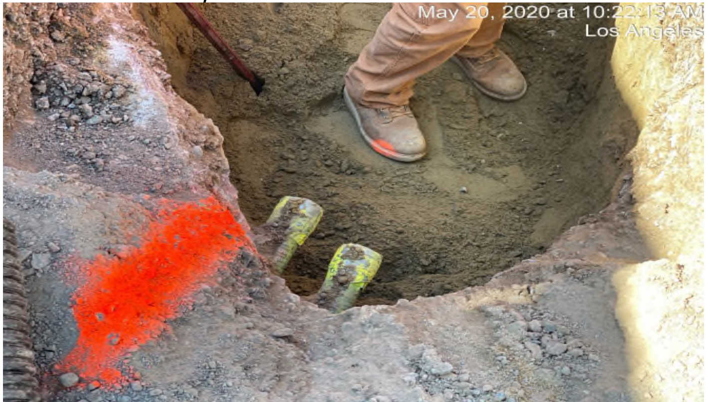
Crenshaw/Vernon - WSCC excavating for Select Electric at Vernon.
