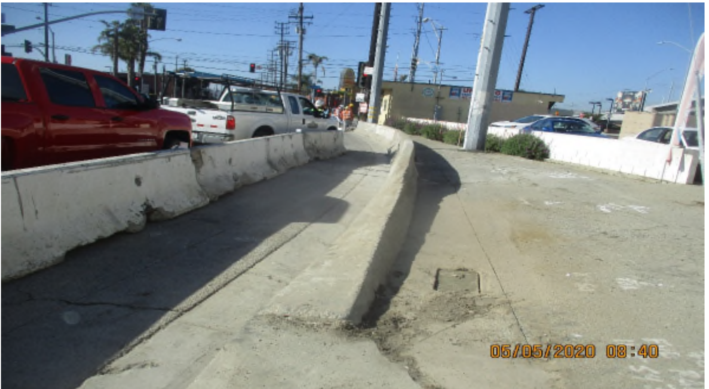
Manchester Bridge - WSCC Make Krail removals at Manchester and Florence.
