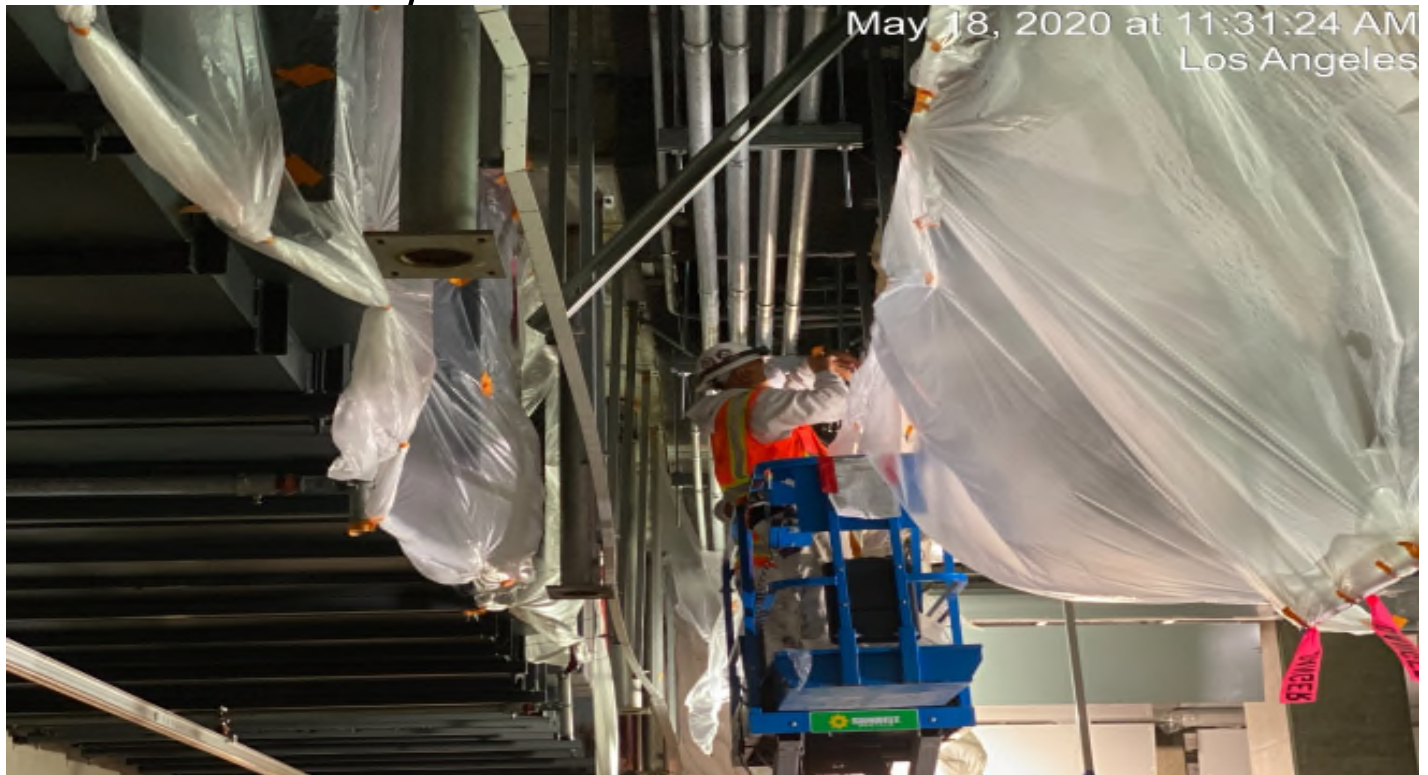
Crenshaw/Vernon - Mariscal prepping to paint conduit at Vernon..
