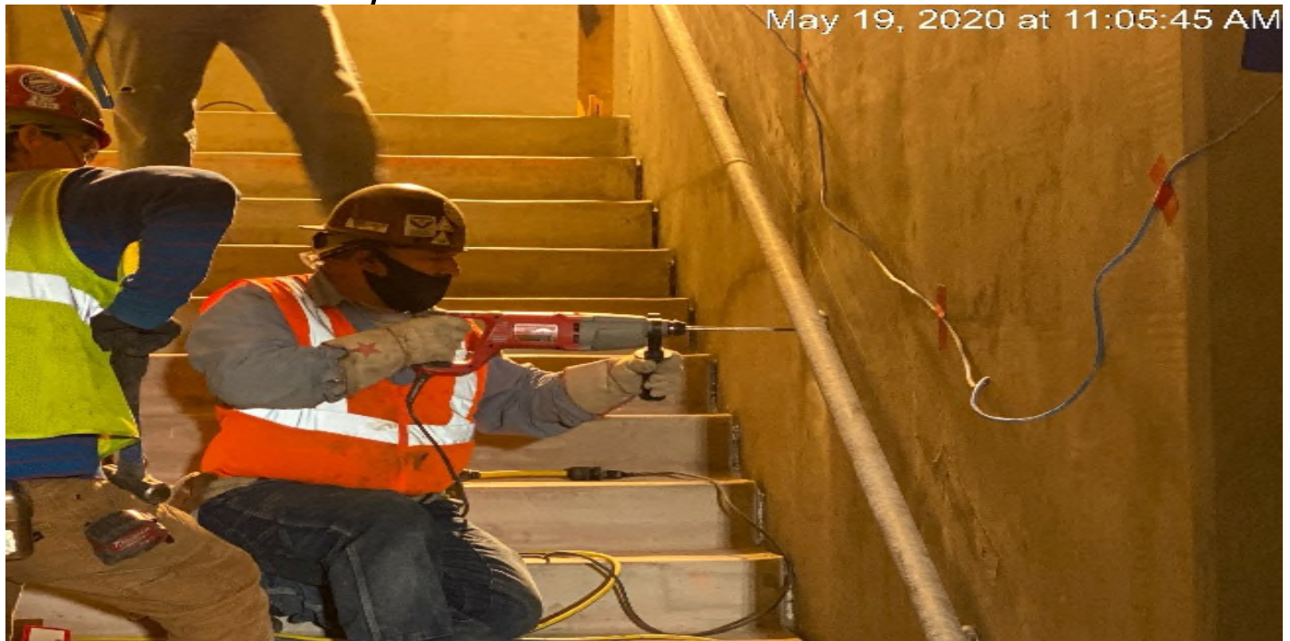
LEIMERT PARK STATION – Continue embedded and ramp lighting fixture installation for the planter stair risers on the northwest section of the plaza level.
