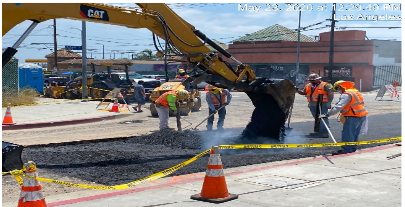
Crenshaw / Slauson – WSCC paving at Slauson and Victoria.
