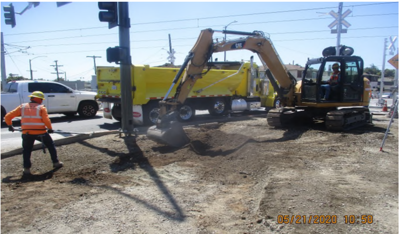
Florence/West – STA 265+00 TK#4/NB looking north – grading work outside ballast wall.
