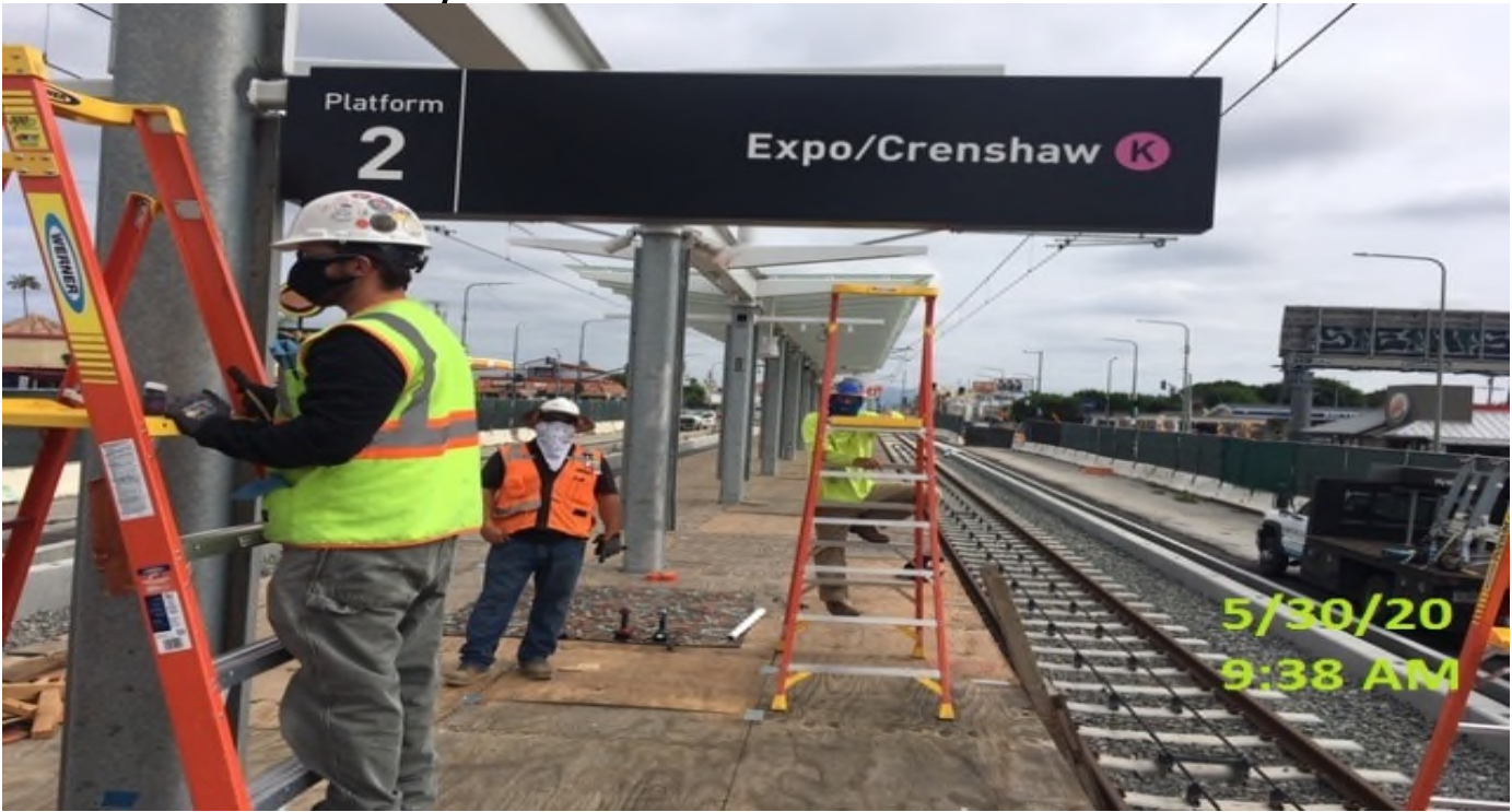
Hyde Park Station – Continue signage installation at the platform level.
