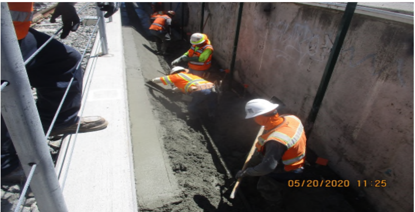
Florence/West – Griffith Co Placed concrete for West Station swale.
