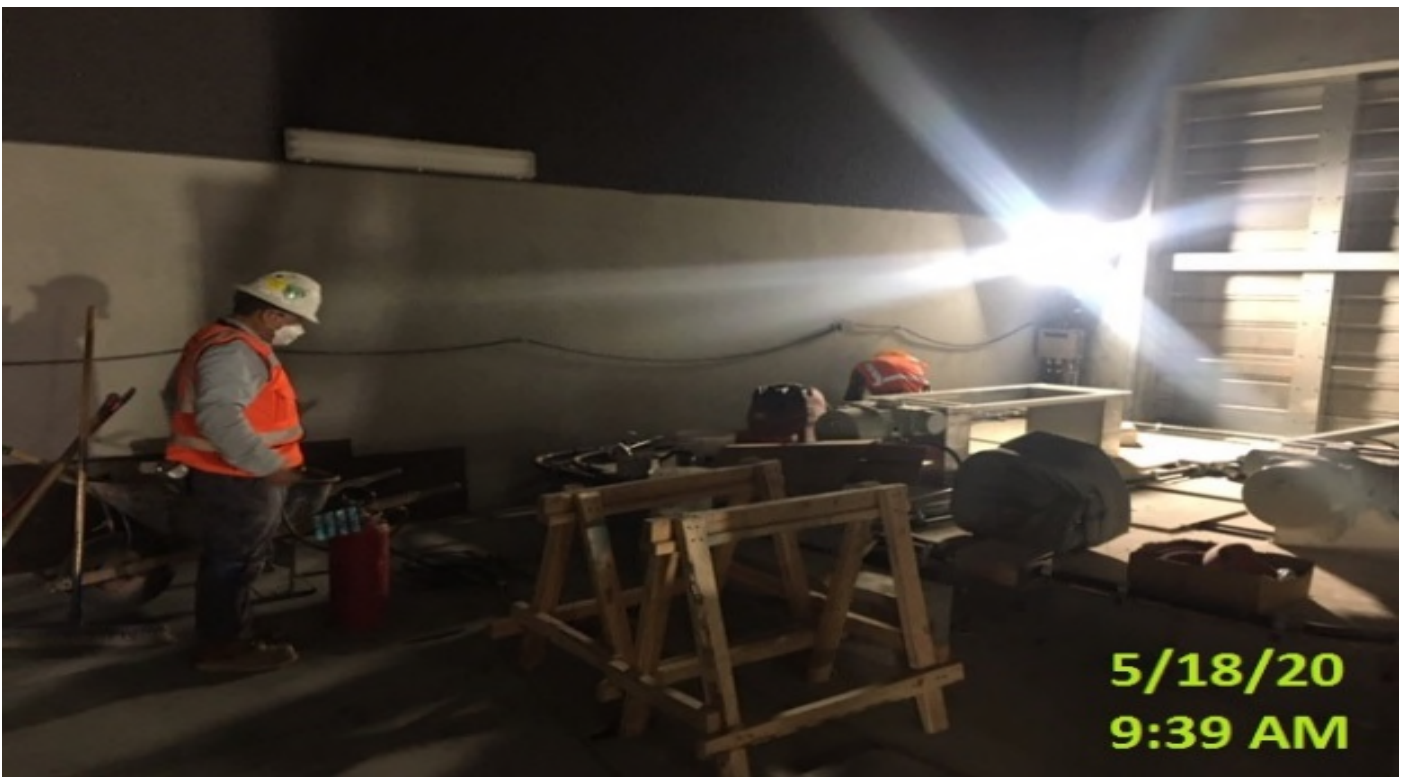
Crenshaw/Expo - WSCC finishers patching and resurfacing walls at north EVF room.
