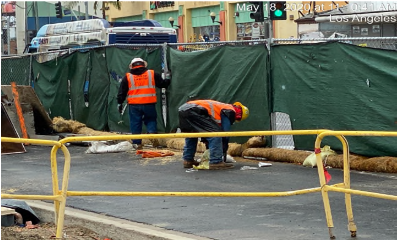
Crenshaw/Vernon - WSCC putting SWPP in place at Vernon.
