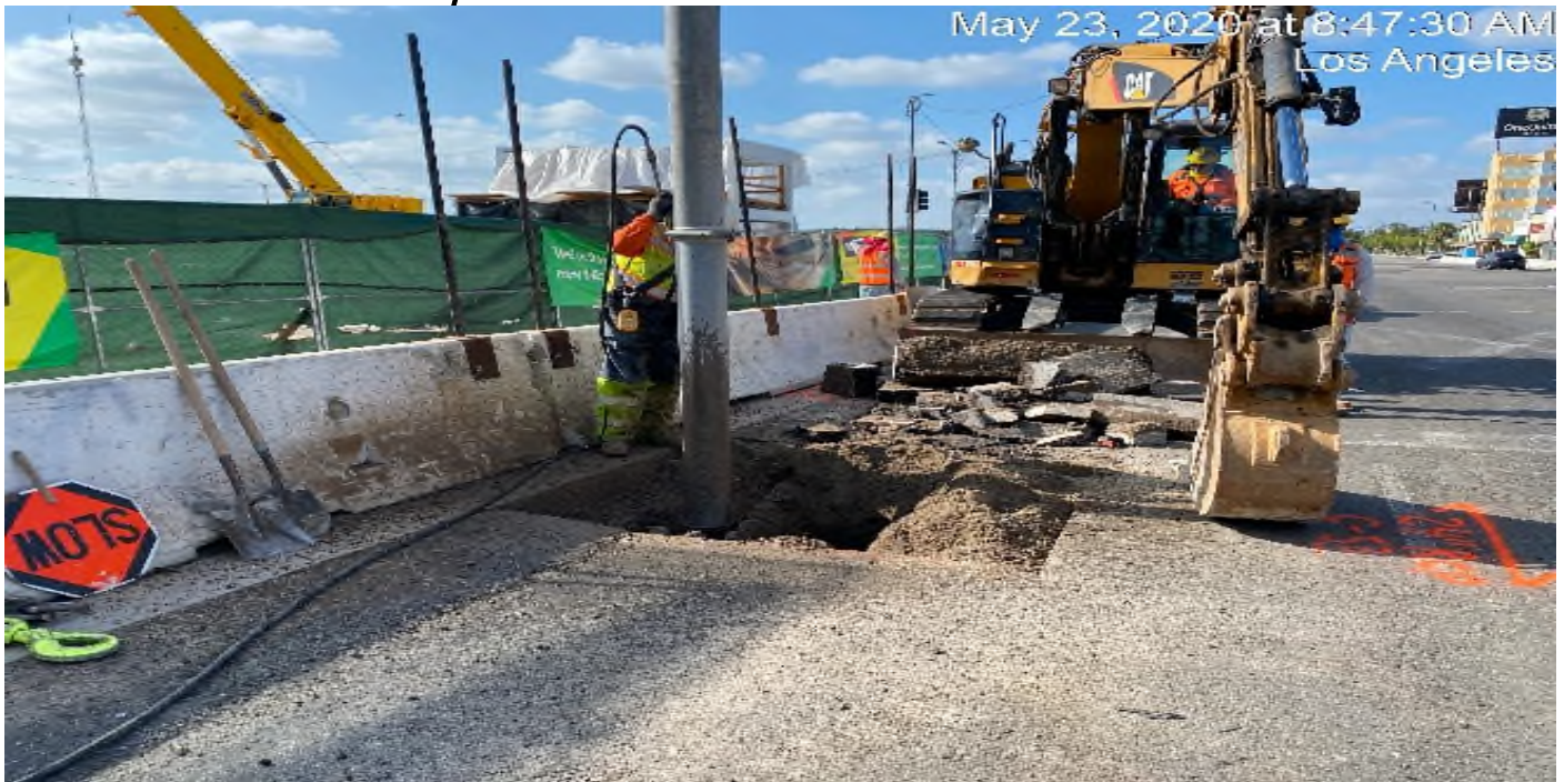
Crenshaw/Expo - WSCC potholing for Pan Pacific at Expo.
