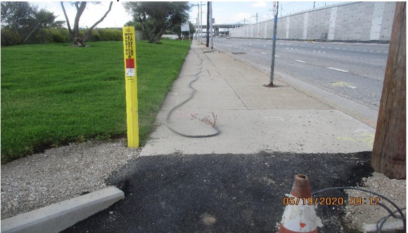
Aviation/Century – DB Electric Removed loop cable at N/B Aviation at 111Th St.
