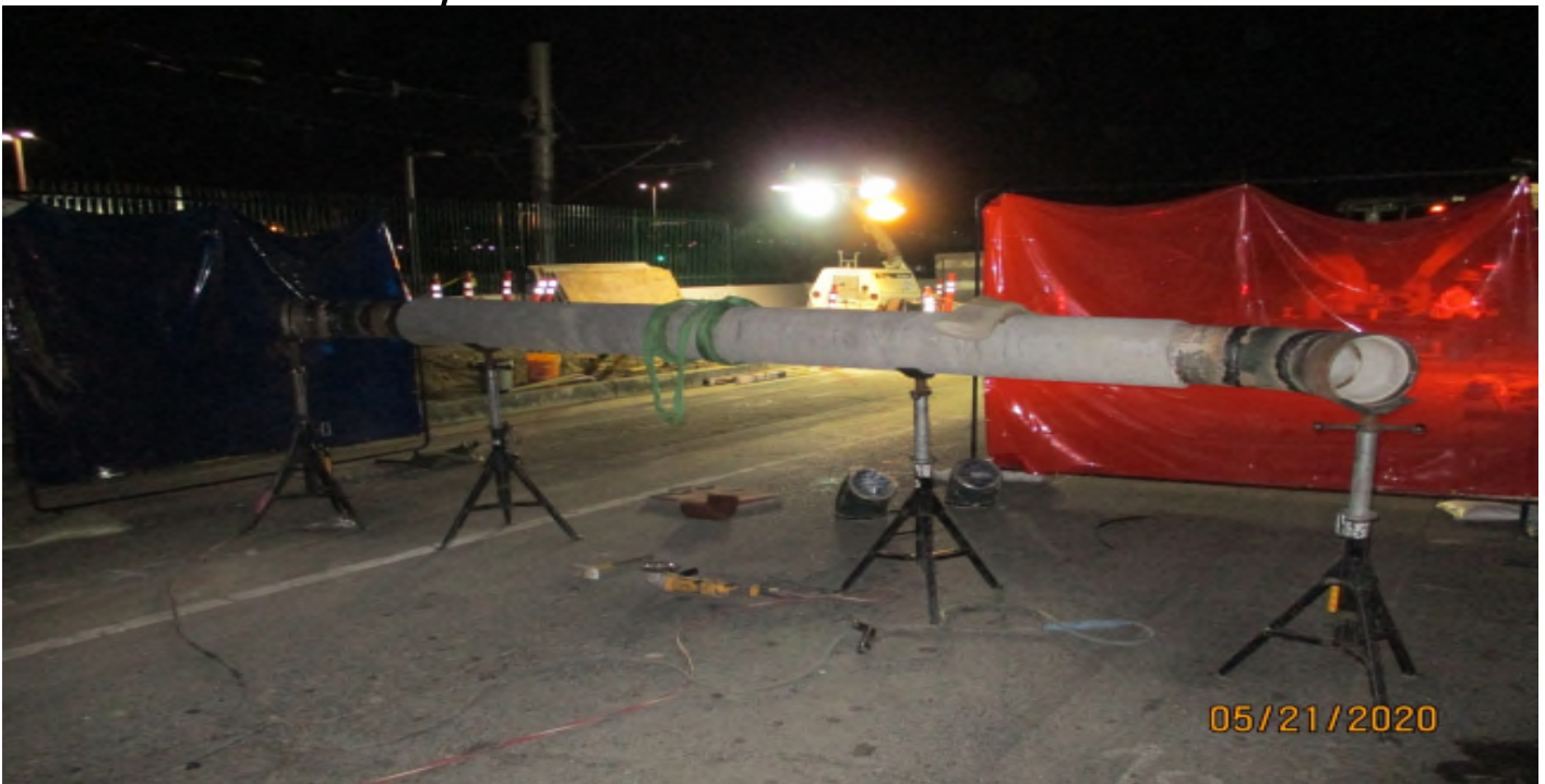
111 th Street – Welding fire line pipe at 111th street.
