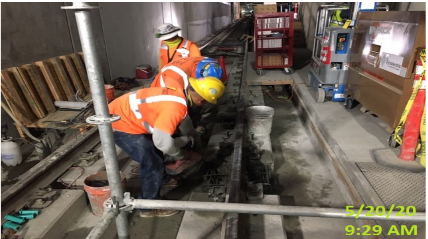
Crenshaw/Expo - EXPO – WSCC demoing plinth blocks at N. end platform.
