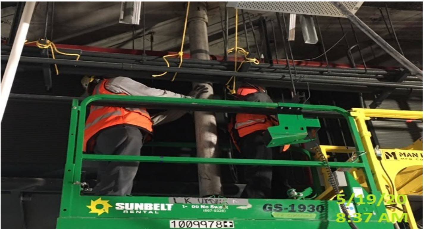
Crenshaw/MLK - MLK – WSSC crew strength testing support poles for edge lighting.
