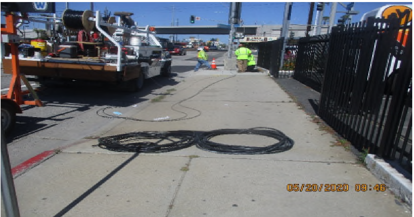
Manchester Bridge – Select Electric pulling loops cable at Manchester intersection
