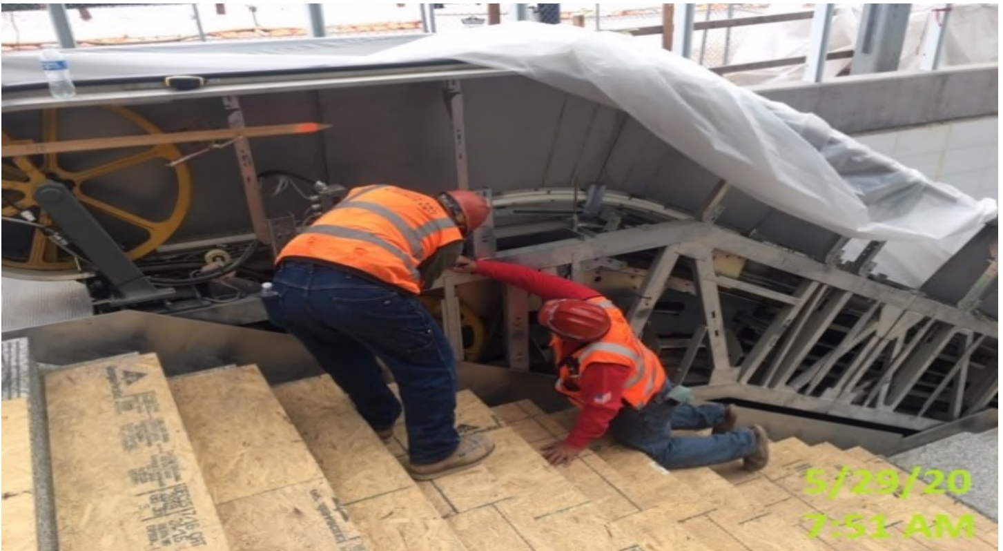
Crenshaw/MLK - MLK – WSCC ironworkers measuring layout for handrail on main staircase.
