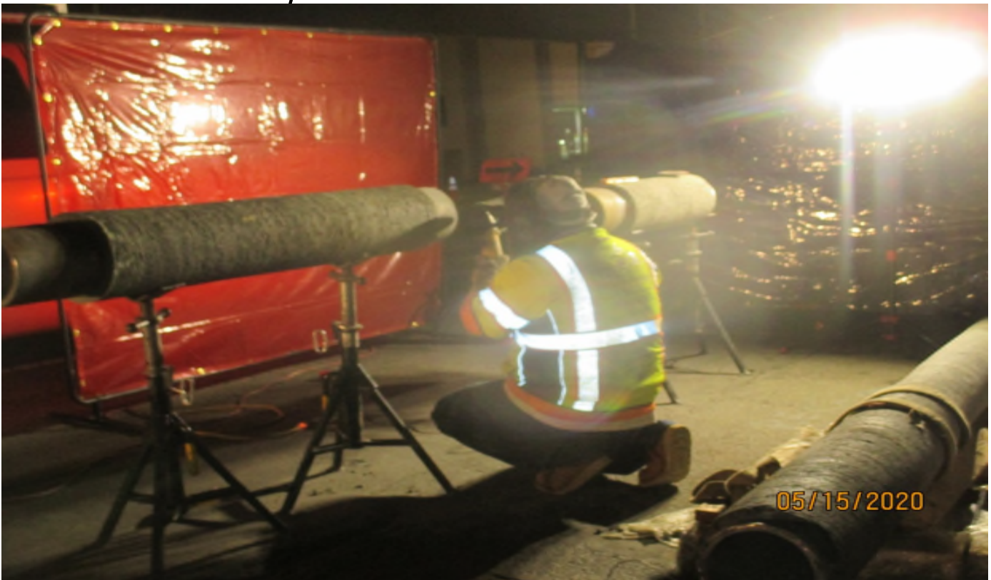
104 th Street - Welding the fire line pipe at 104th street.
