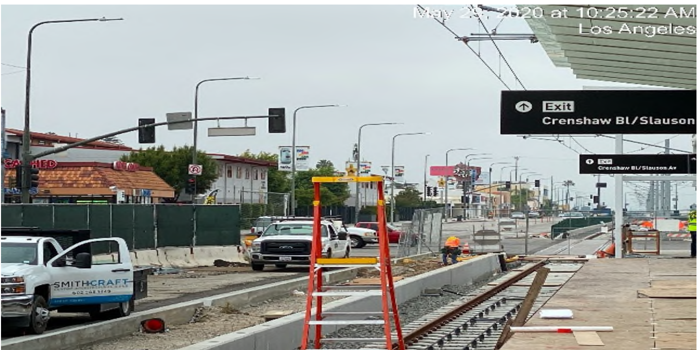
Hyde Park Station – Began signage installation at the platform level.
