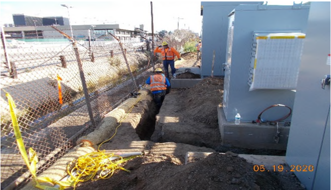
104 th Street - North view of WSCC digging trench. 104 th
