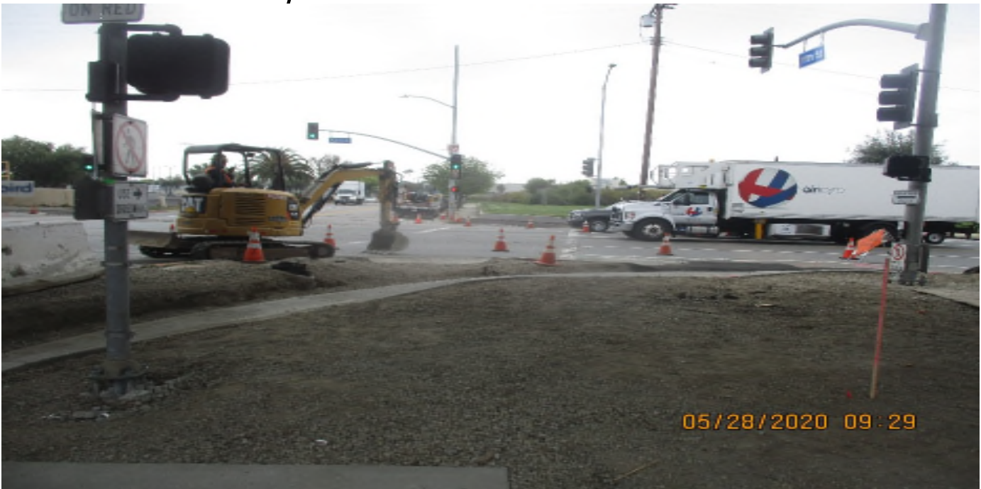
104 th Street - WSCC Making grade and removals at 104th for C&G.
