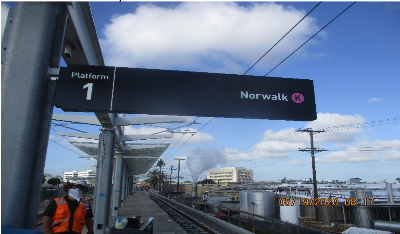
Florence/Brea - Smith Craft Placing Overhead signs at La Brea Station.
