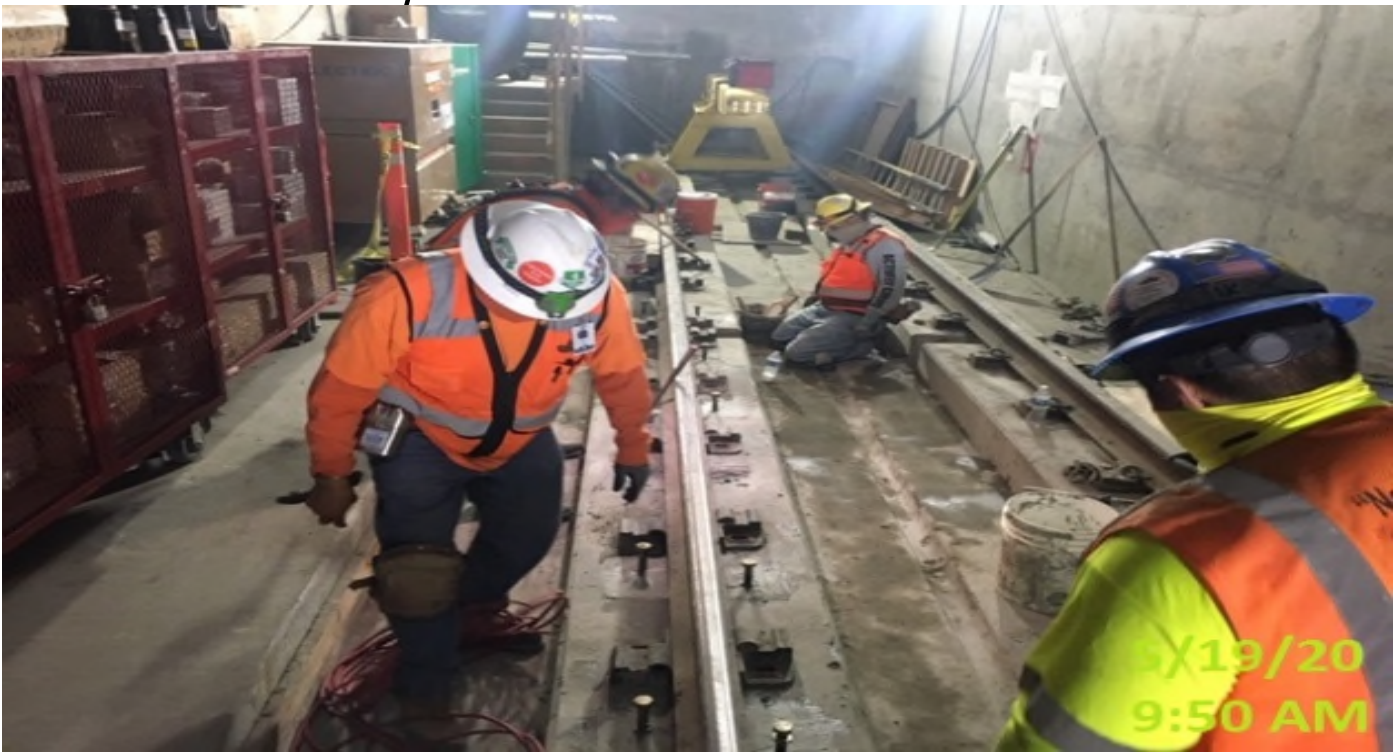
Crenshaw/Expo - WSCC installing rail fasteners and demoing plinth block.
