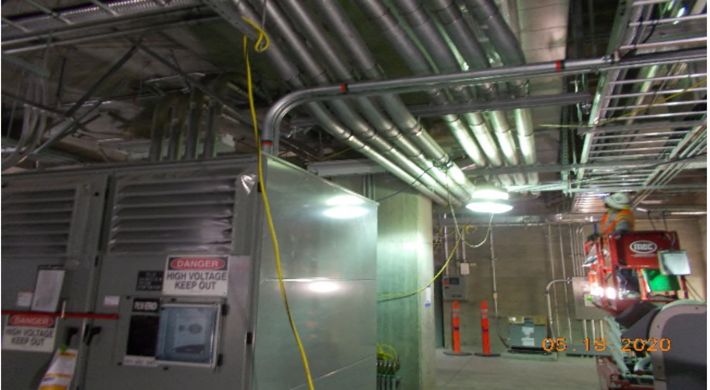
Crenshaw/Vernon - 2" conduits from PX to tray for interconnects.
