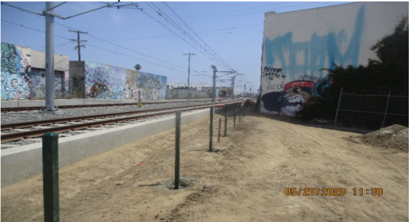
Florence/West – ACE Fence Place fence posts at East Bound Florence W-High
