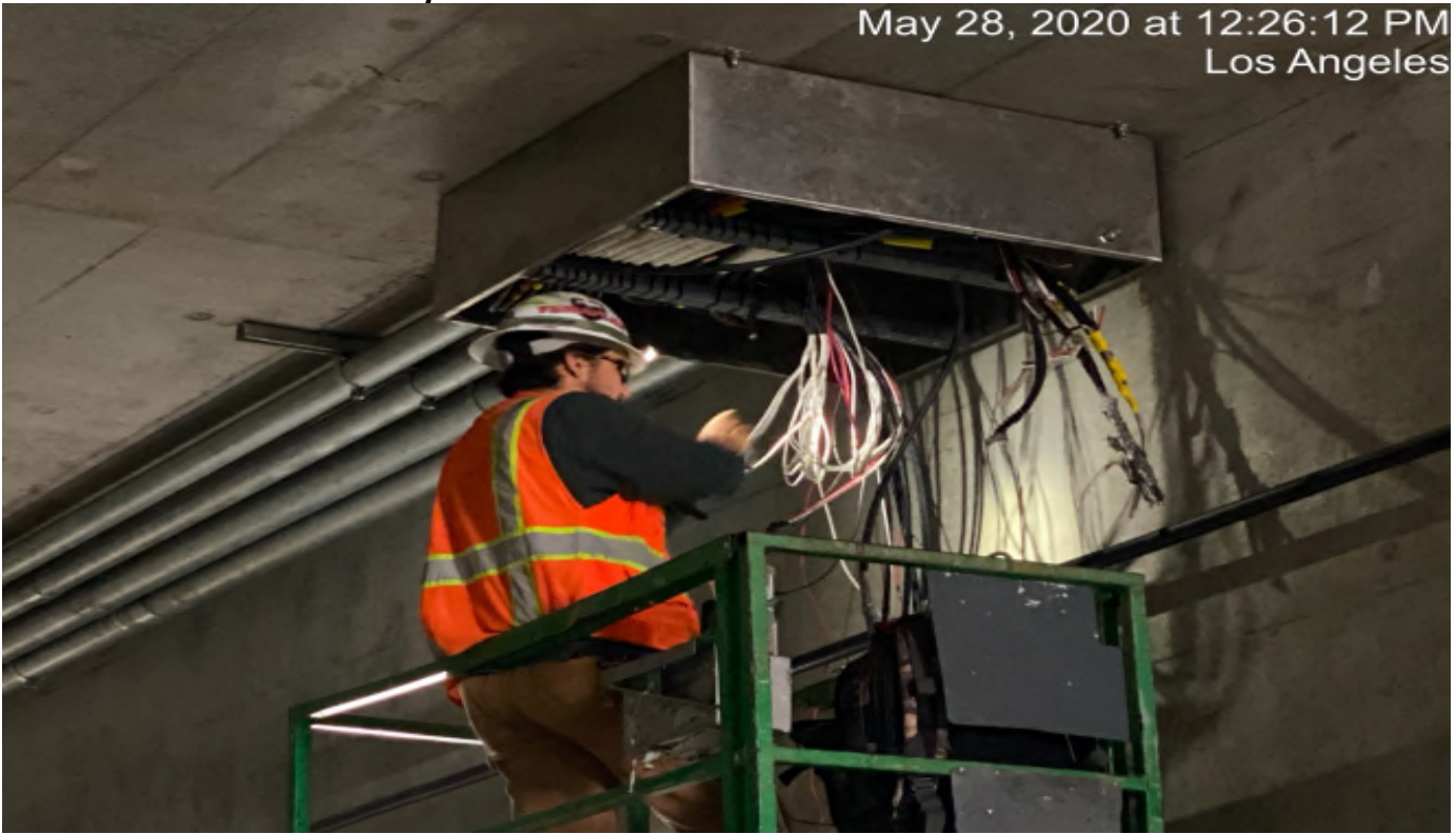
Crenshaw/Vernon - DCD splicing cables at Vernon northbound UG-3.
