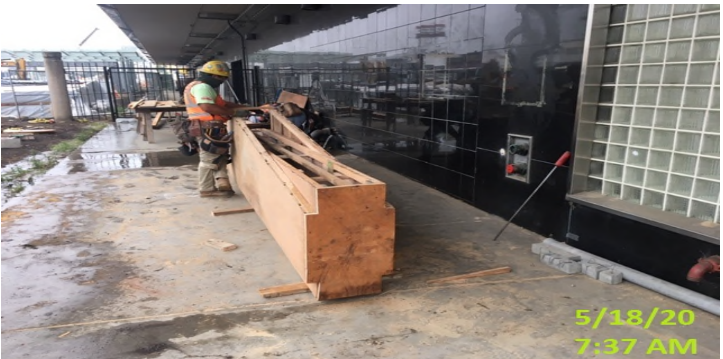
Crenshaw/MLK - MLK – WSCC carpenters building mock-up pylon signage.
