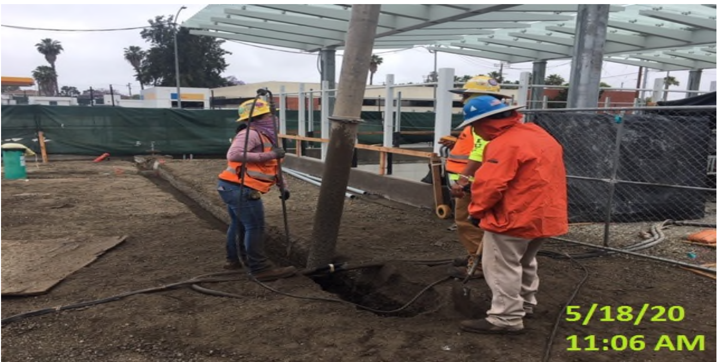
Crenshaw/Expo - WSCC crew at main entrance surface finishing wind screen curb
