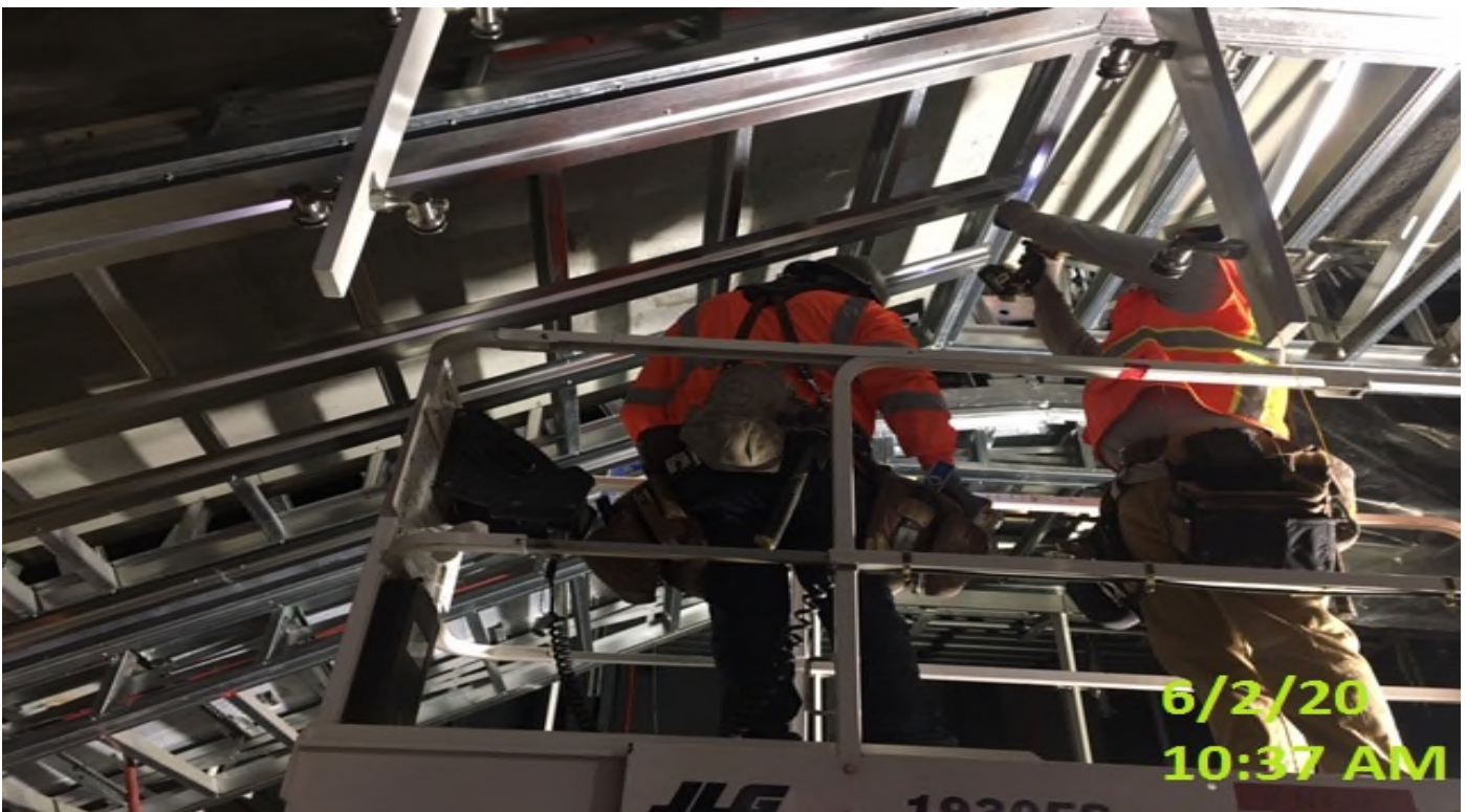
EXPO STATION- VNSM installing hat channel braces underneath stairway #2.
