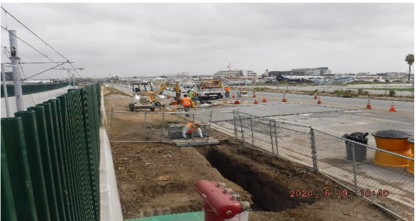
AVIATION/CENTURY- STA 33+00 looking north Aviation Blvd. fresh PCC road surface – BLOIS
