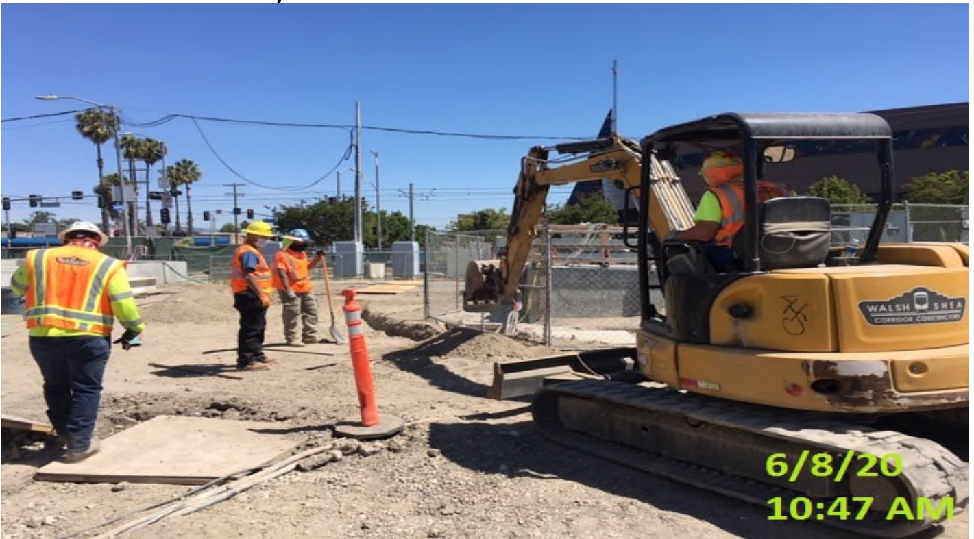
EXPO STATION- WSCC crew excavating for conduit and irrigation trench.
