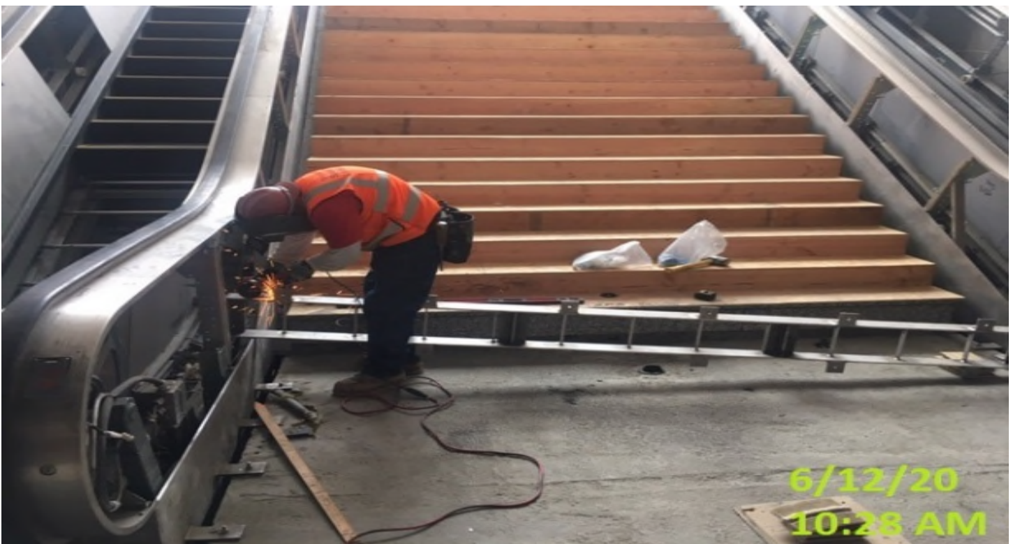
EXPO STATION- WSCC ironworkers installing trench drain at main staircase landing.
