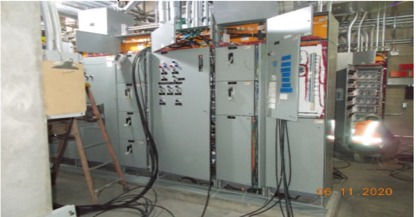
EXPO STATION- View of MCC1N and interconnects being routed.
