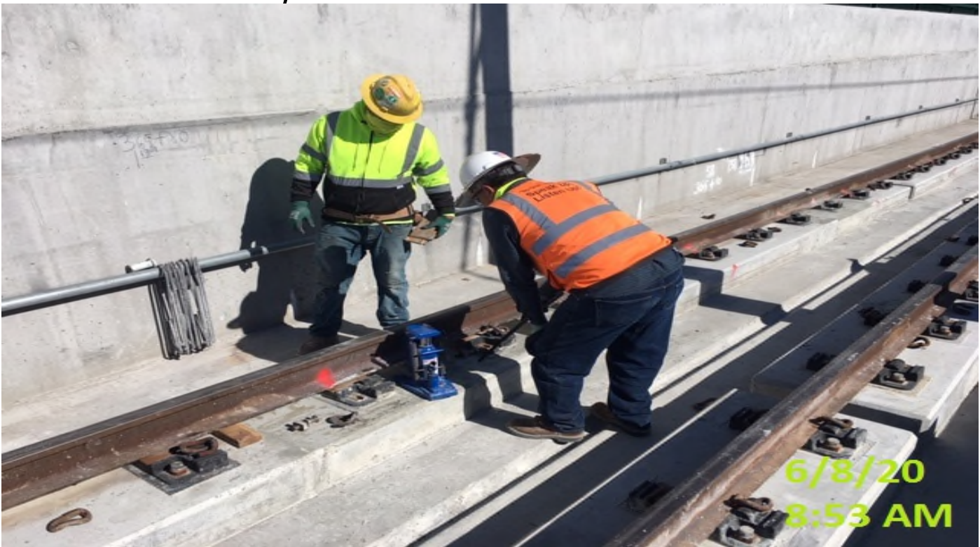
UG4 – WSCC crew removing rail fasteners.
