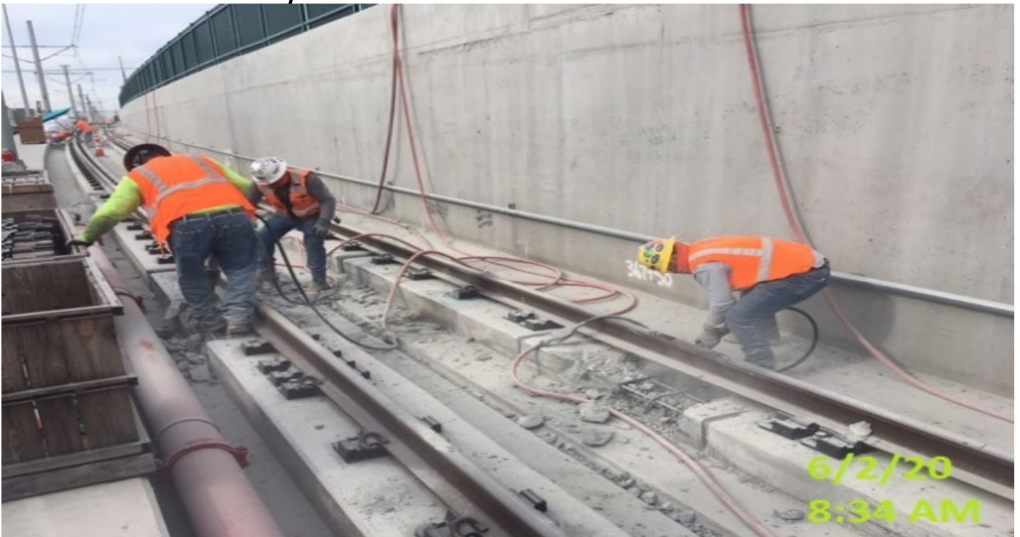
UG4 – Crew demoing sections of plinths blocks.
