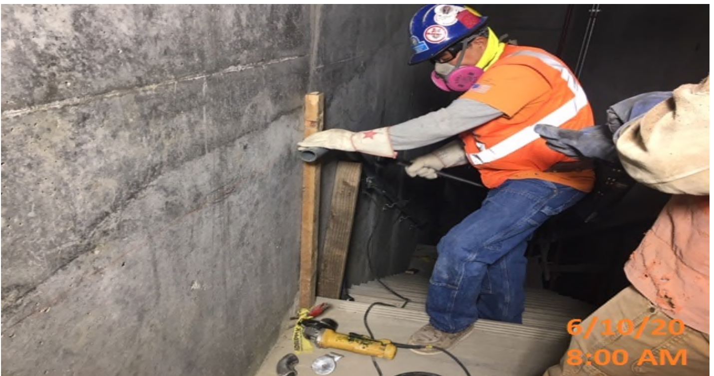
MLK STATION- McMahon Steel installing handrail at emergency exit north stair #2.
