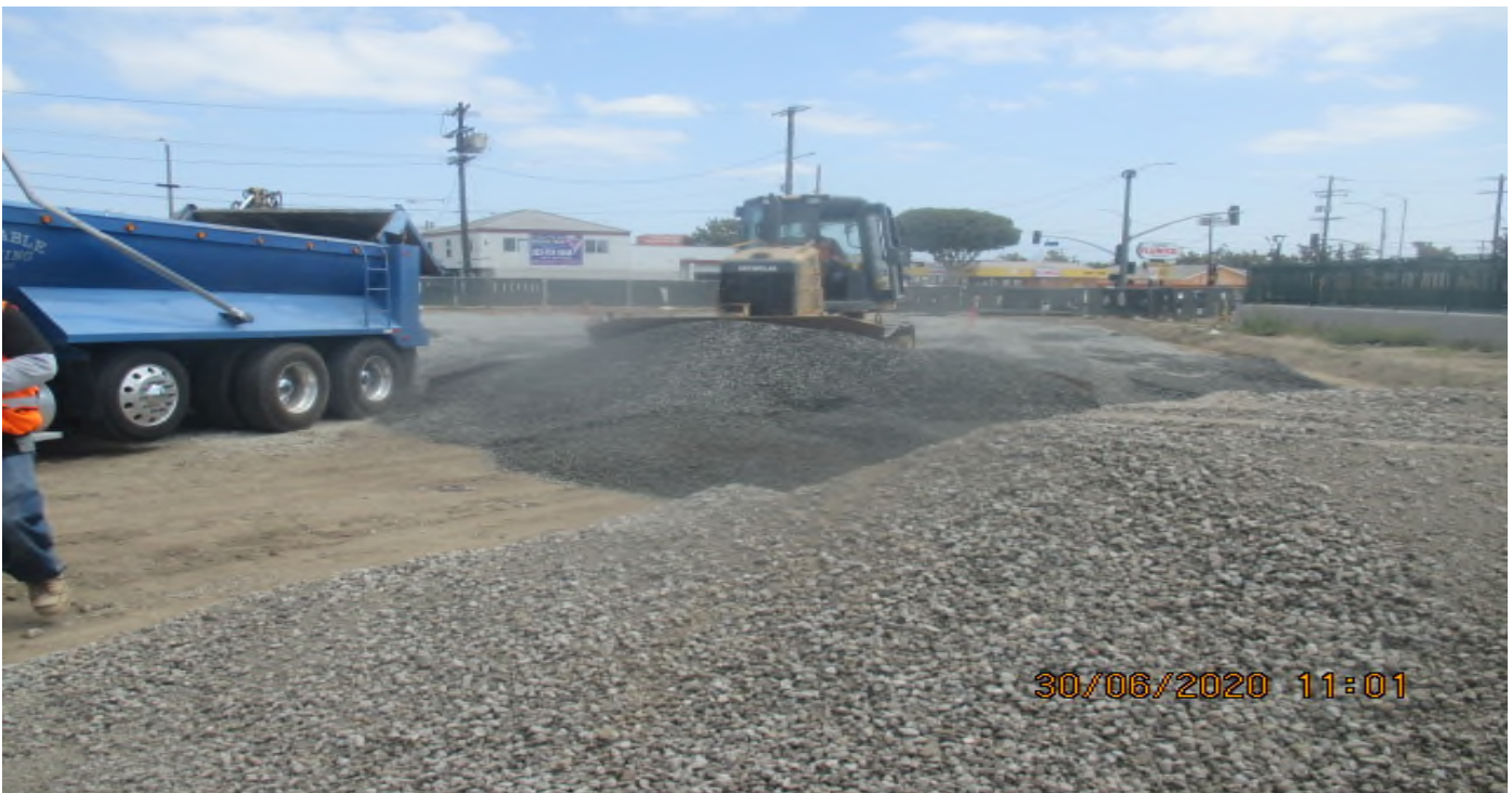
UG3 – Continue placing granite base rock throughout Victoria Yard. 6/30/20
