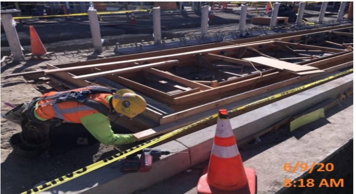
VERNON STATION- WSCC crew building formwork for air exhaust shaft.
