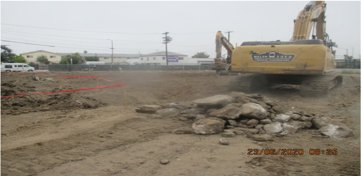
UG3 – Continue excavating/grading the north east section of Victoria Yard. 6/23/20
