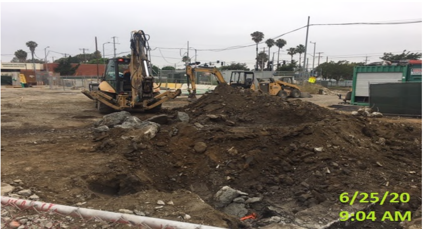
EXPO STATION- WSCC crew demoing slab at north end yard.
