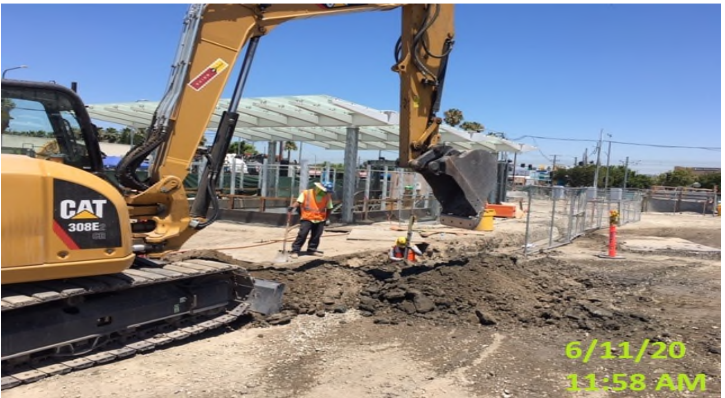
EXPO STATION- WSCC excavating trench for lighting conduit and irrigation.
