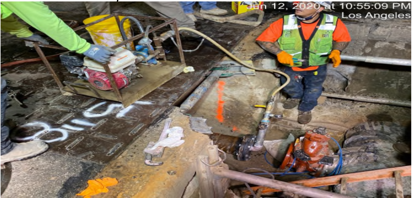
AVIATION/CENTURY- Blois pressurizing the 8" fire line at Aviation & 111th looking south.
