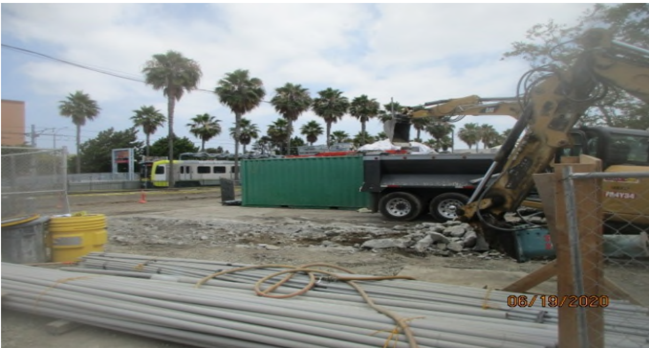
EXPO STATION – Demolishing/clearing the north side section of the plaza.
