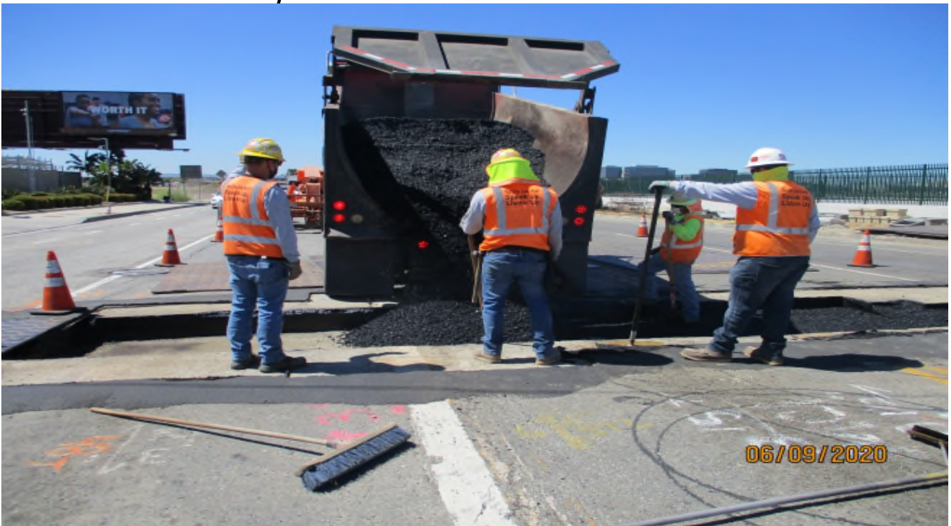
104th Street- Paving the electrical trench at 104th street.
