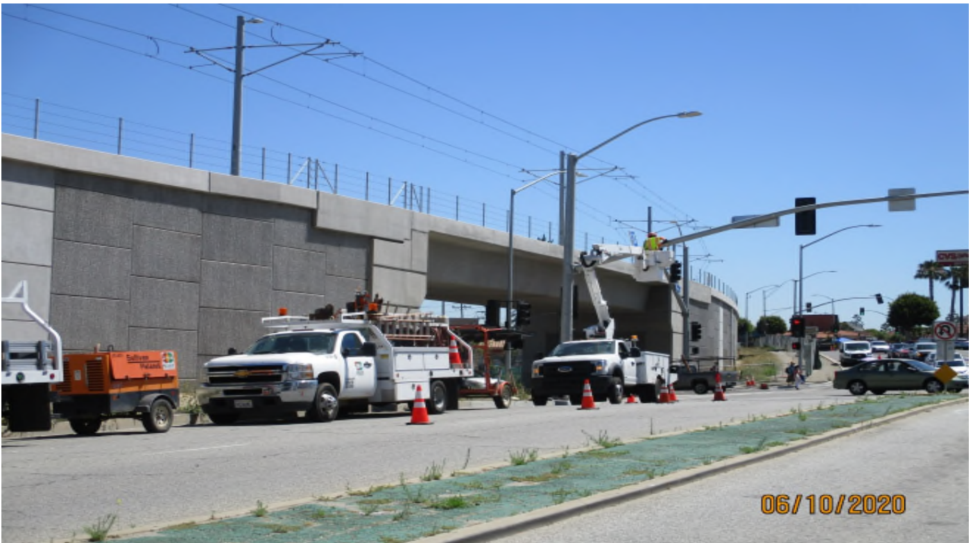
La Brea –Placing street signs on the traffic signal mast arm at La Brea.
