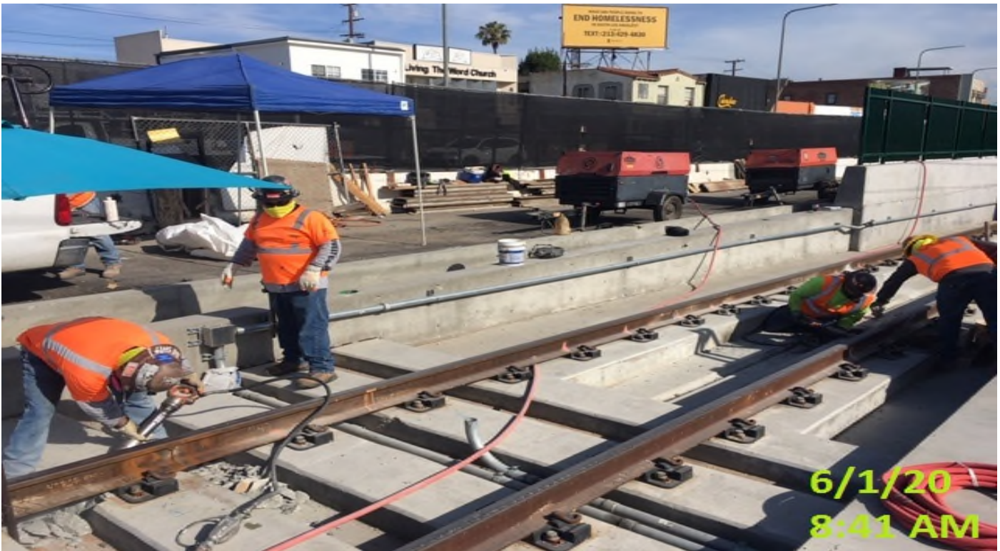
UG4 – Crew demoing sections of plinths blocks.
