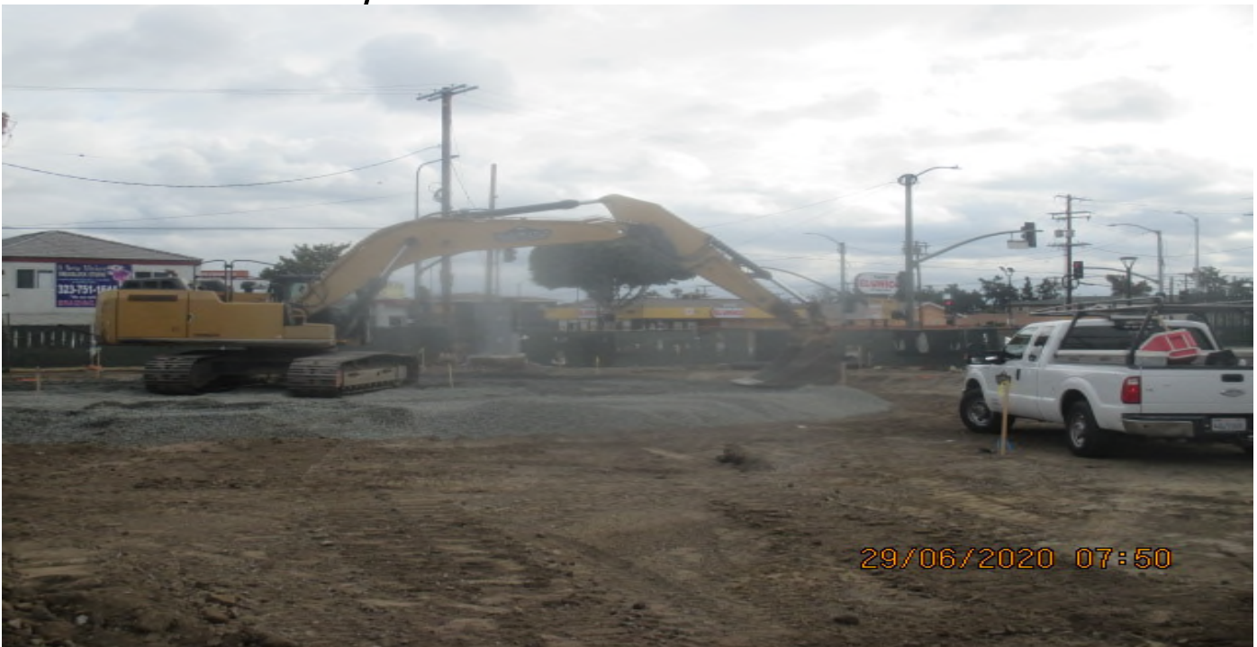
UG3 – Placing granite base rock throughout Victoria Yard. 6/29/20
