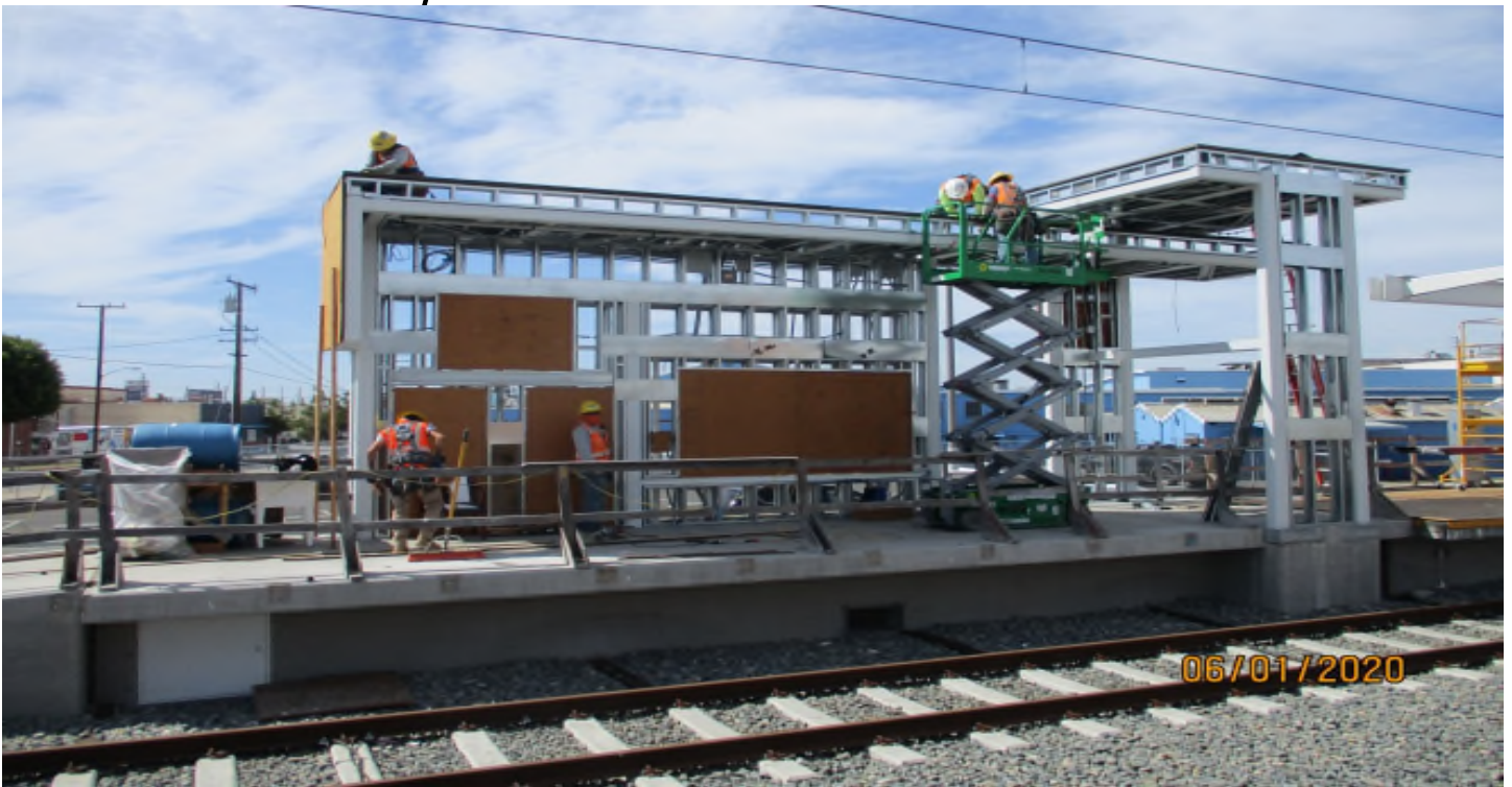
Hindry Station – Framing in the roof block outs at the Hindry Station.
