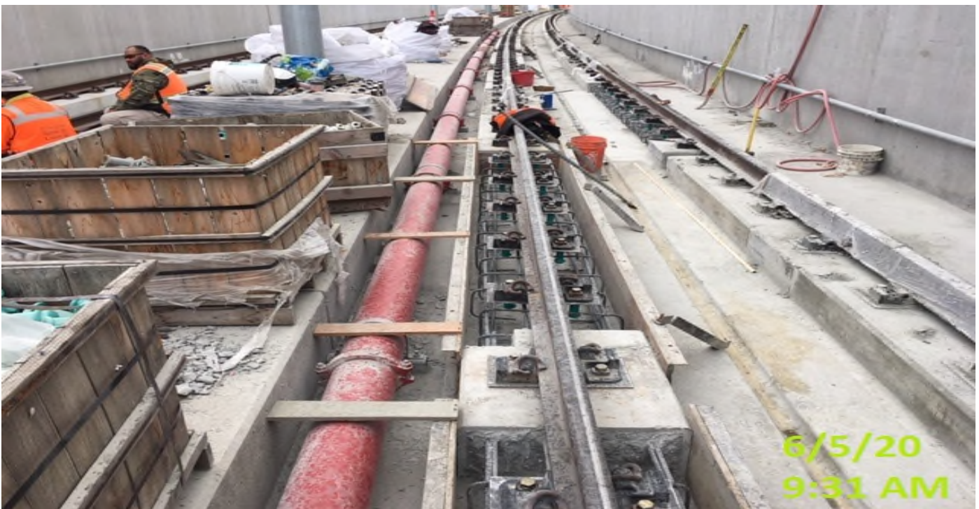
UG4 – WSCC crew continue demoing sections of plinths blocks.
