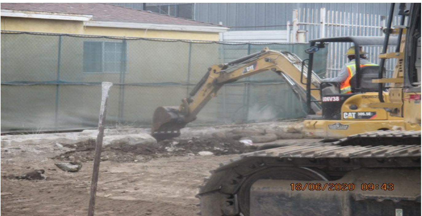
UG3 – Continue excavating/grading the north east section of Victoria Yard. 6/18/20
