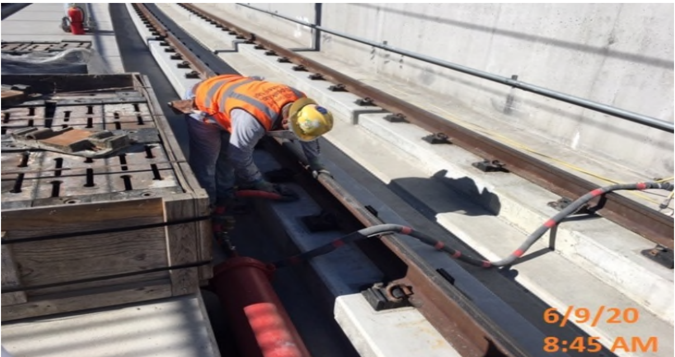
UG4 – WSCC crew resurfacing section of plinths.
