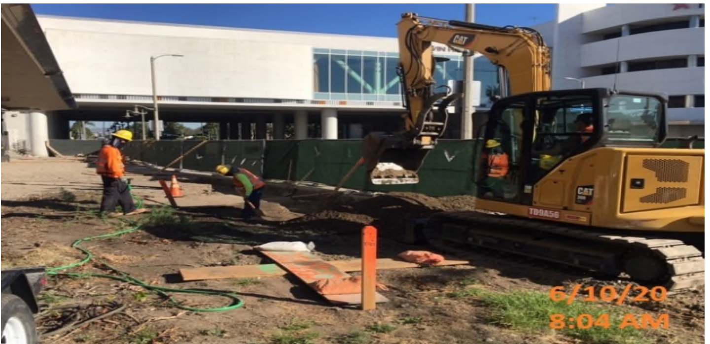
MLK STATION- WSCC crew excavating to subgrade for pavers and sidewalk.
