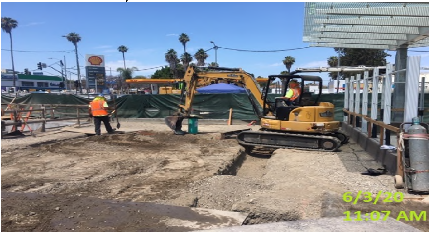
EXPO STATION- WSCC crew excavating trench for mapcase.
