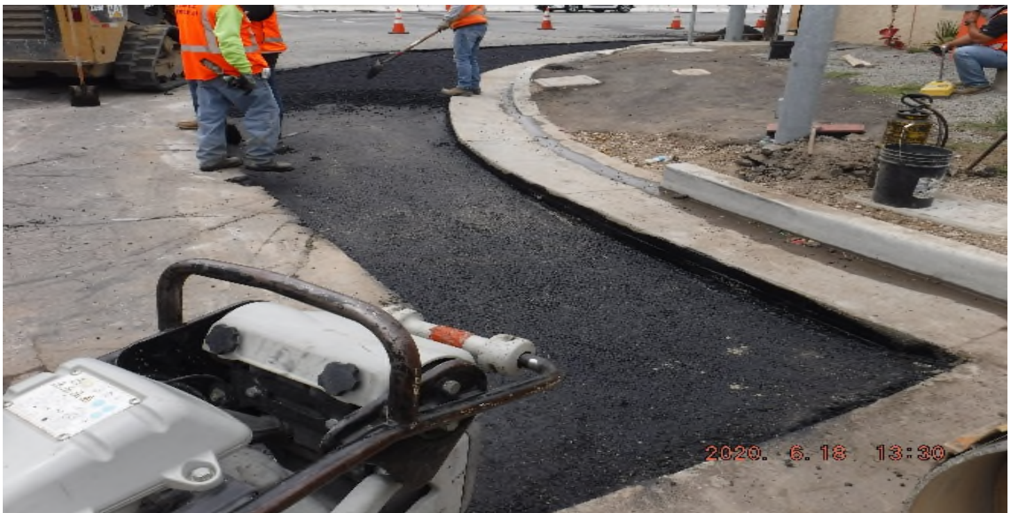
AVIATION/CENTURY- STA 27+00 looking west – 111th St w, Aviation Blvd. road work in front NEC of curb return (slot pave)
