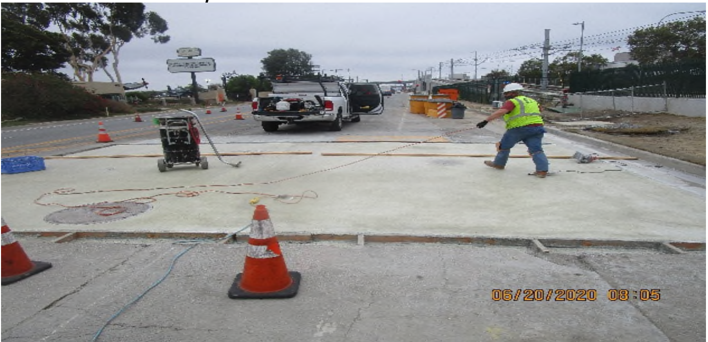
AVIATION/CENTURY- Aviation Blvd south of 111th St. Stationing 28+50 Saw cutting (2) 31`-10" lateral saw cuts (2") deep by 1/8" wide
