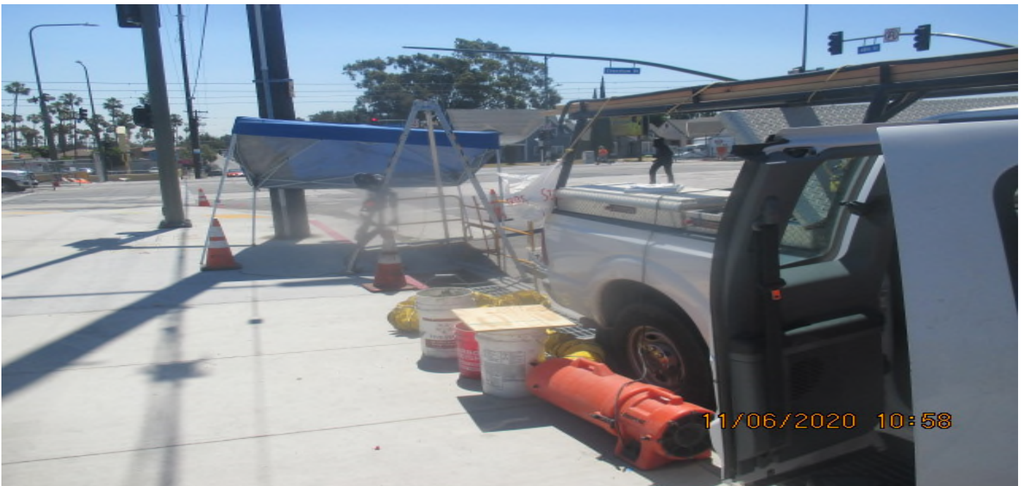
PARK MESA – Sack and patching Catch Basin #29 on southbound Crenshaw Blvd and 48th St. 6/11/20
