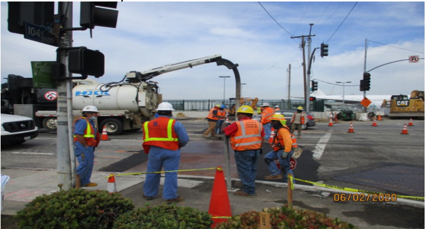
104th Street- Potholing for utilities at 104th street. Facing west.
