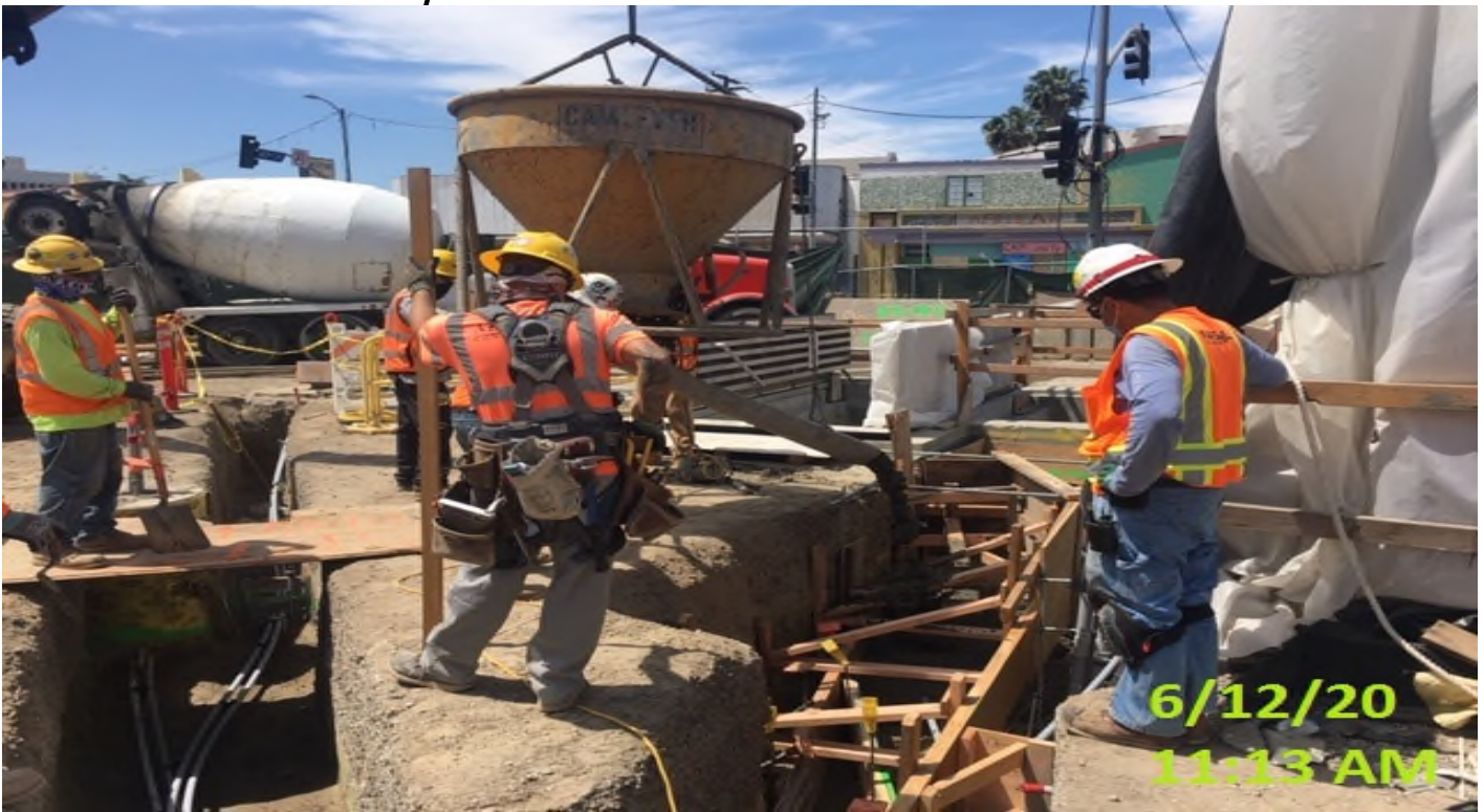
VERNON STATION- WSCC placing concrete in conduit trench.
