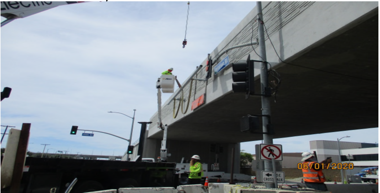
111th Street- Hanging the traffic signal mast arm at 111th street.
