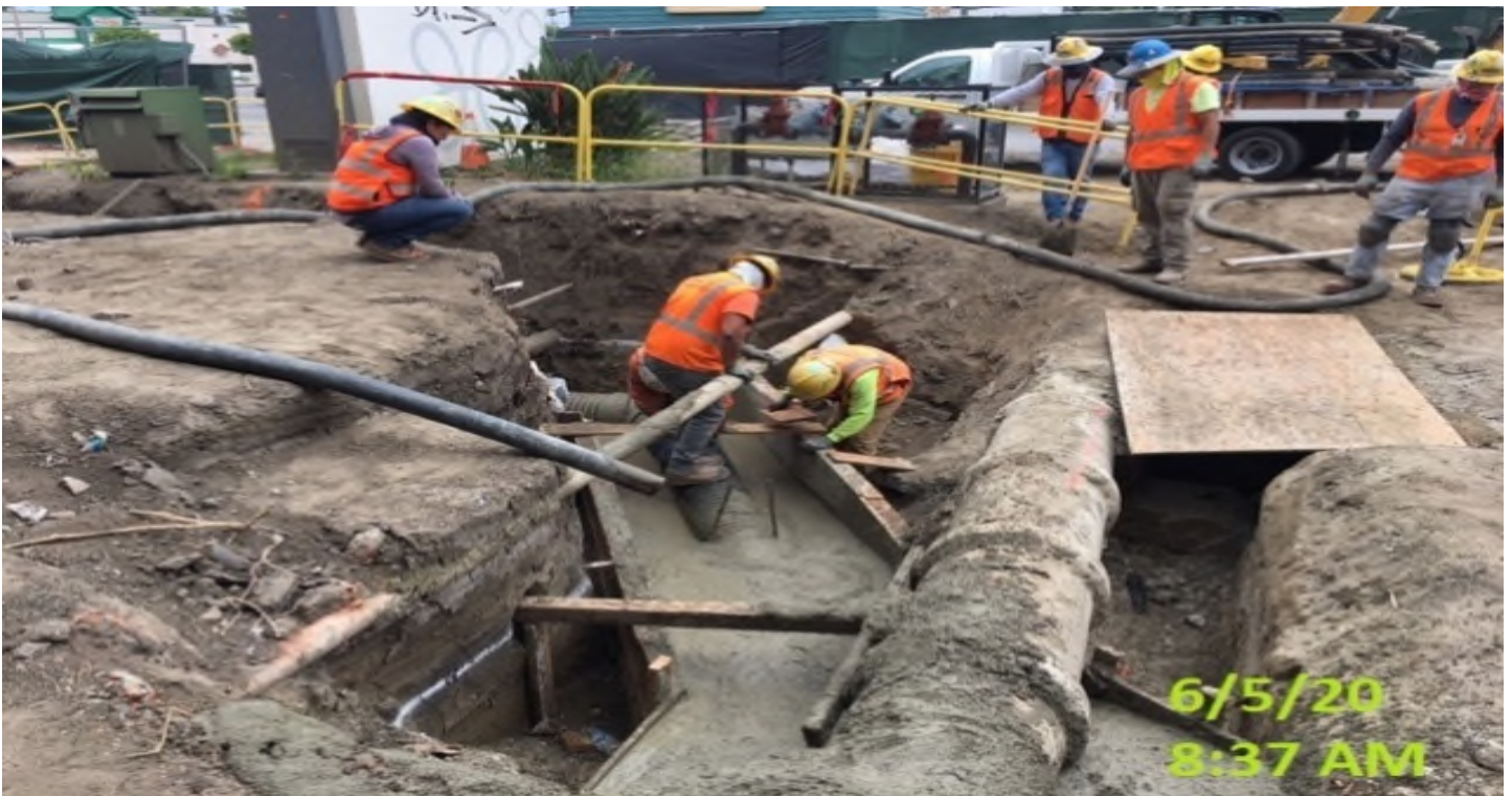
MLK STATION- WSCC crew encasing 12" HDPE drain line in slurry.
