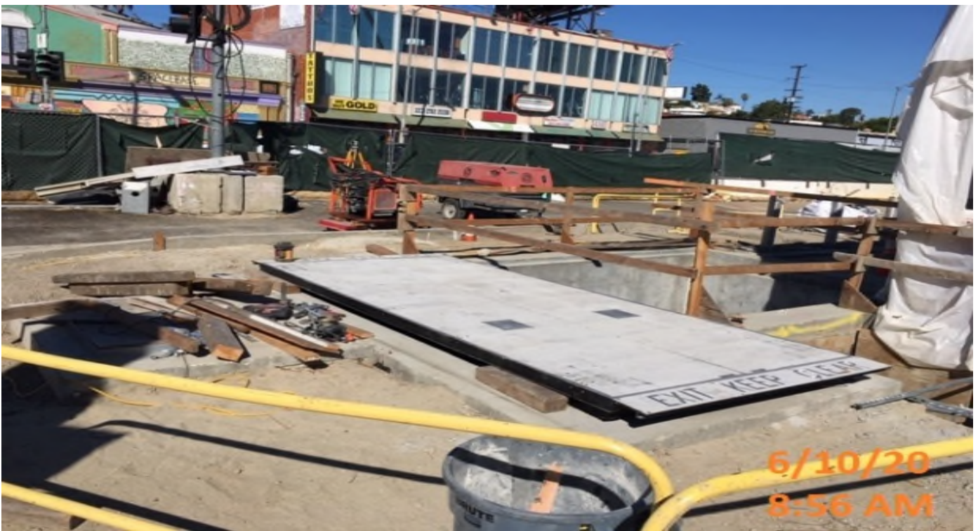
VERNON STATION- WSCC crew installing hatch doors for emergency exit #1.
