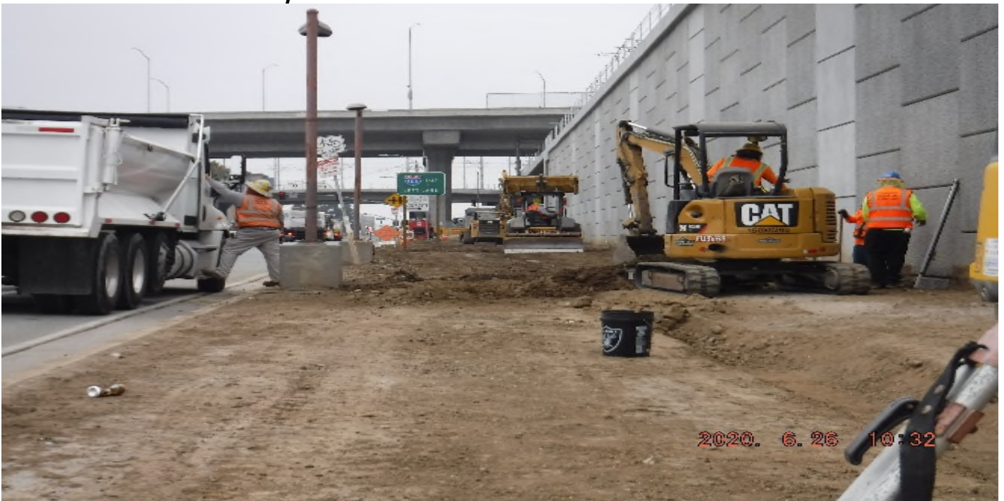
AVIATION/CENTURY- STA 20+00 looking south along RW17R Aviation Blvd. grading work status
