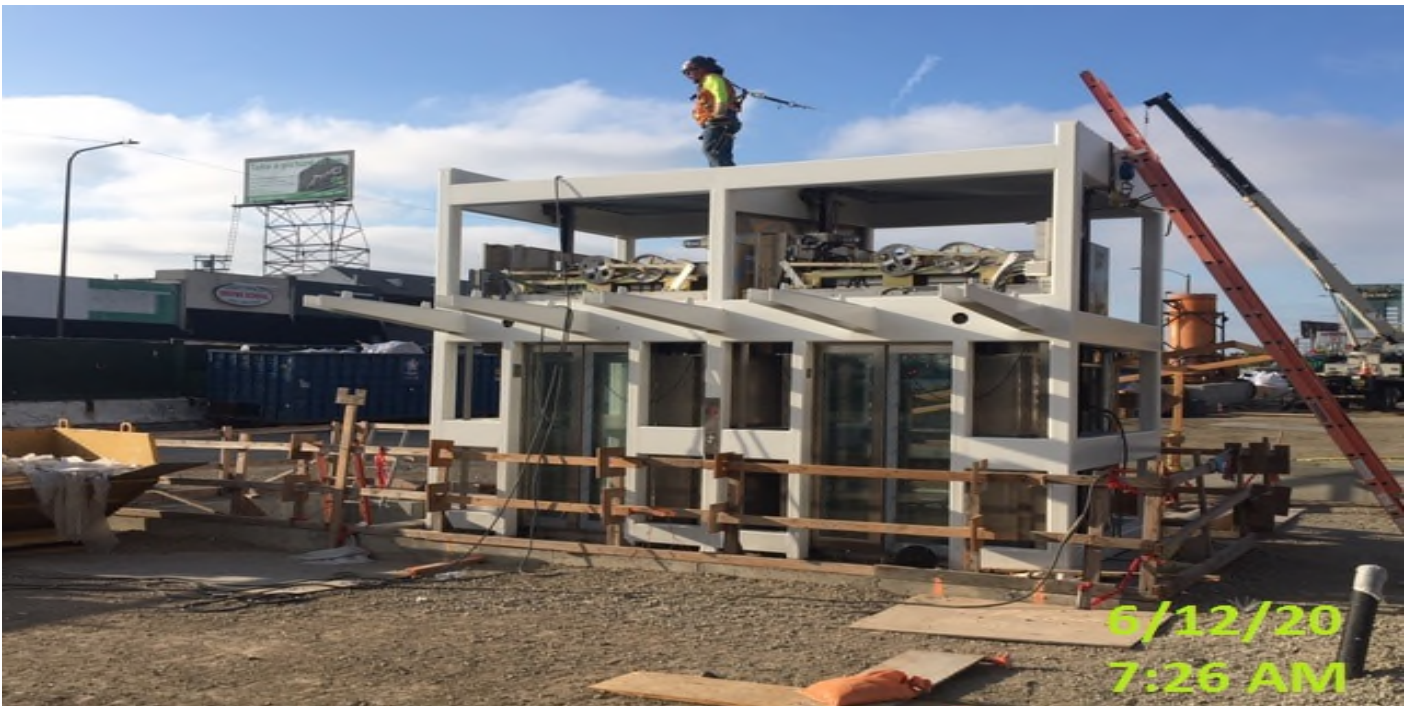
MLK - Continue installing roofing deck for Elevators 1&2 at the plaza level.
