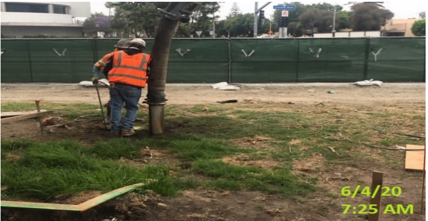
MLK STATION- WSCC crew potholing for tree wells and utility conflicts.
