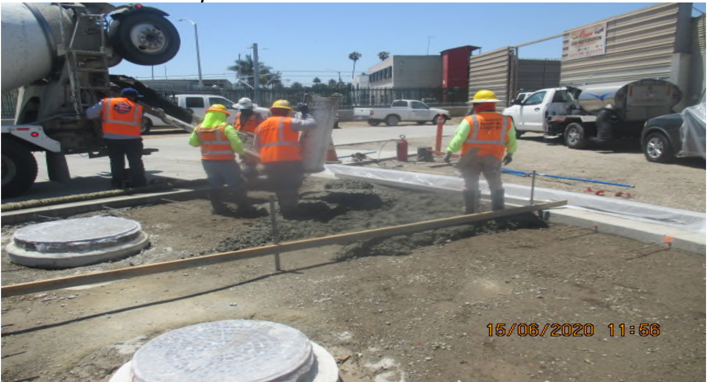
UG3 – Installing rebar and placing concrete for the Victoria Cul-de-sac radius. 6/15/20
