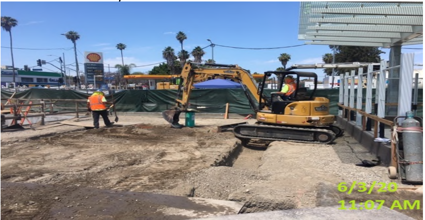
EXPO STATION – Excavating/trenching for map case foundation footing at the plaza.
