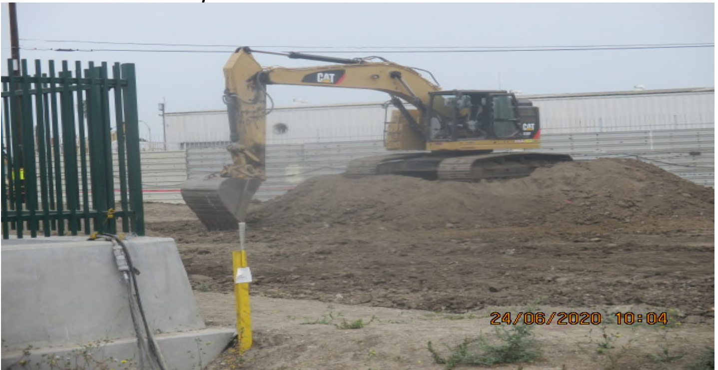
UG3 – Continue excavating/grading the north east section of Victoria Yard. 6/24/20
