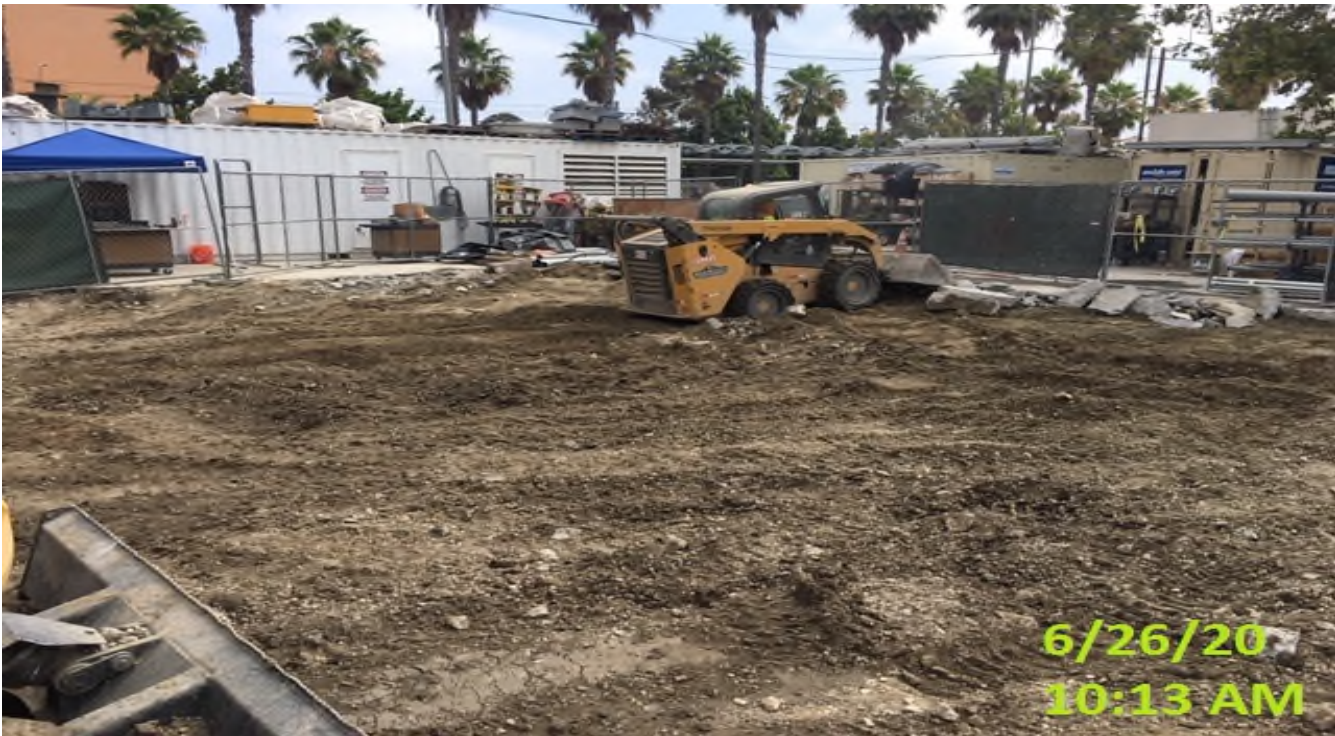
EXPO STATION – Continue demolishing/clearing the north side section of the plaza.
