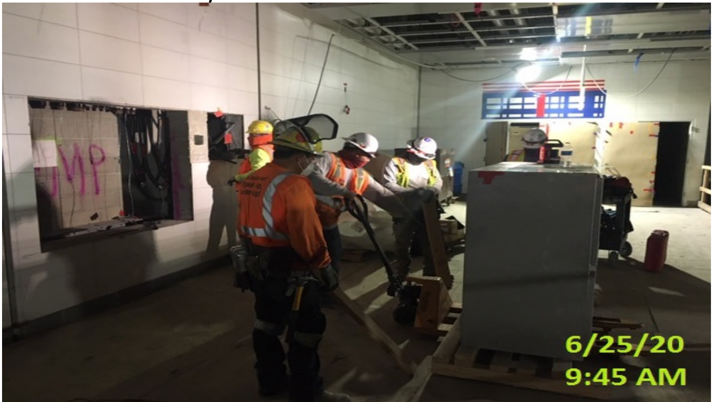
EXPO STATION- WSCC crew sub-support installing EMP unit.
