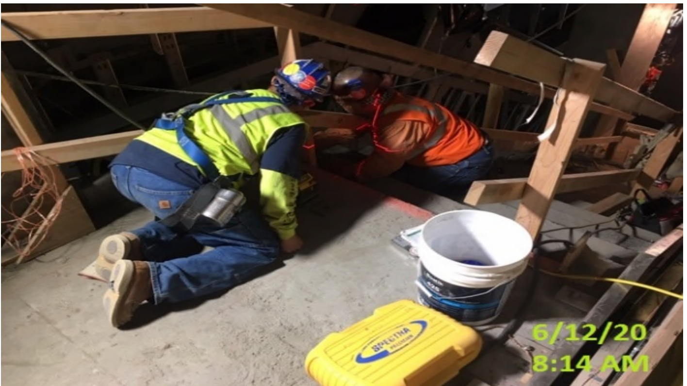
VERNON STATION- McMahon Steel adjusting edge plate height at stair #4.
