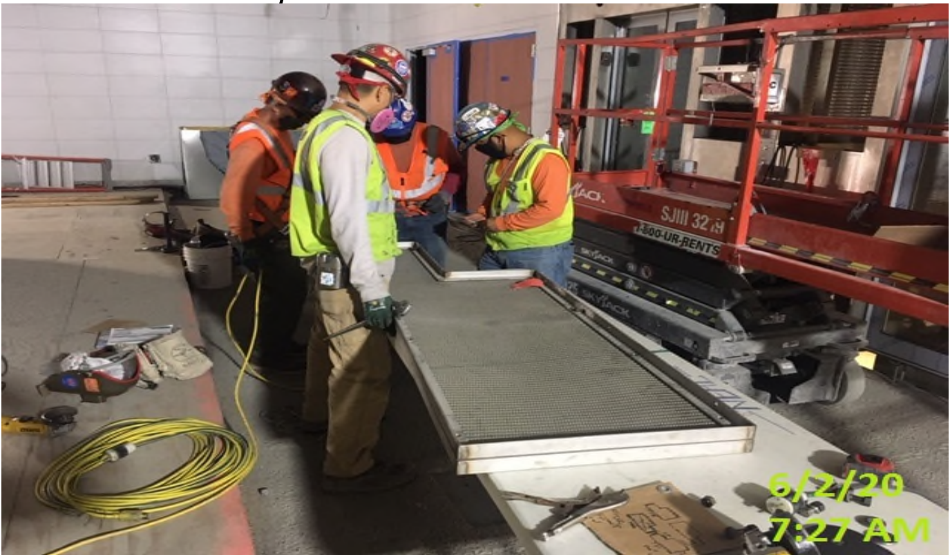
MLK STATION- McMahon installing mesh fascia screens for elevator #3 and #4.
