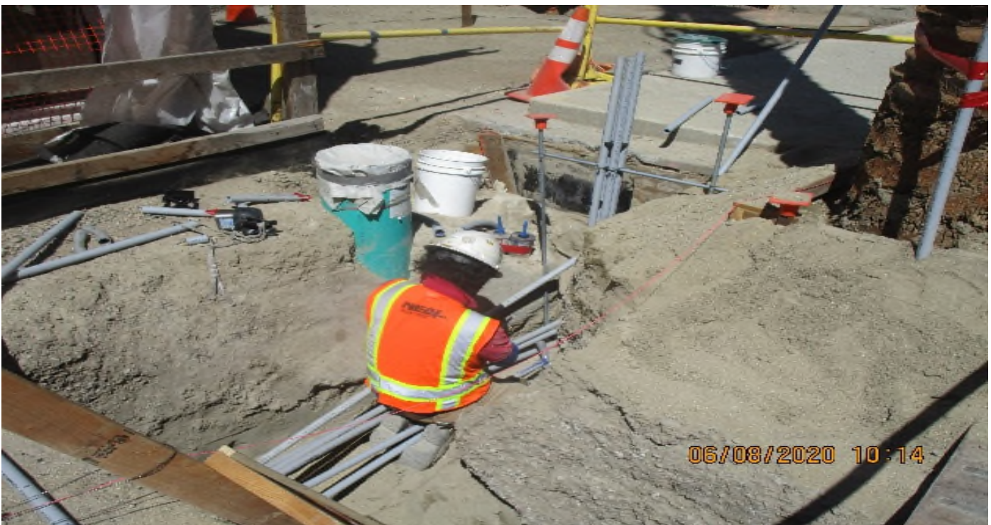
VERNON STATION- Resumed rough in underground Comm, CCTV, Elevator canopy lighting.
