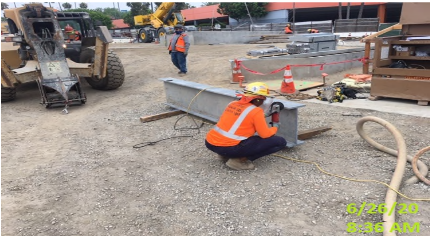
EXPO STATION- Marina Landscaping digging for palm tree placement.
