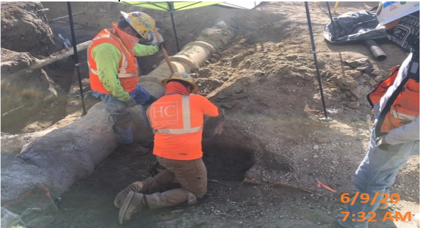
MLK STATION- WSCC crew hand digging for pedestrian light pole foundations.
