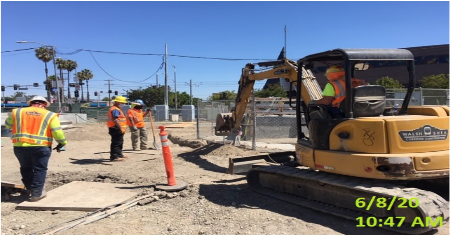
EXPO STATION – Excavating/trenching for irrigation/controller installation at the plaza.
