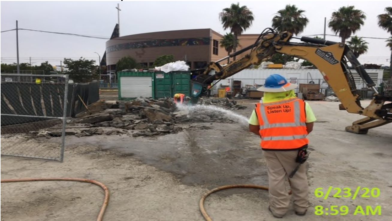
EXPO STATION – Continue demolishing/clearing the north side section of the plaza.
