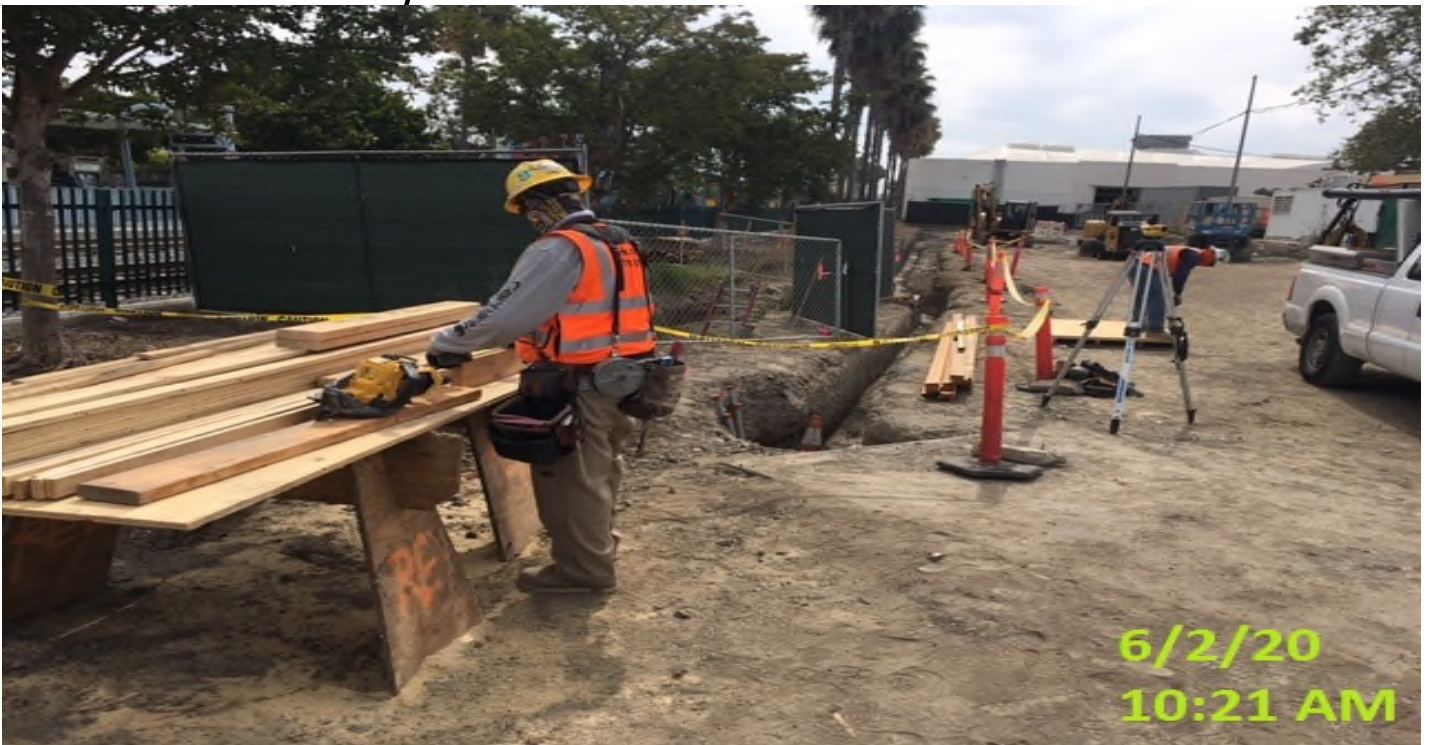
EXPO STATION- WSCC crew building formwork for manhole #1.
