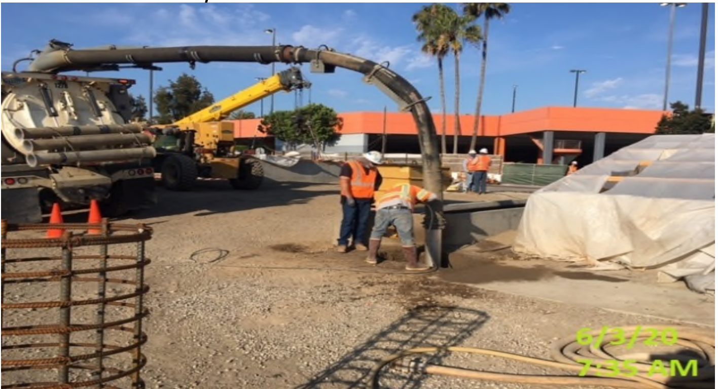
MLK STATION- WSCC crew potholing for light poles.
