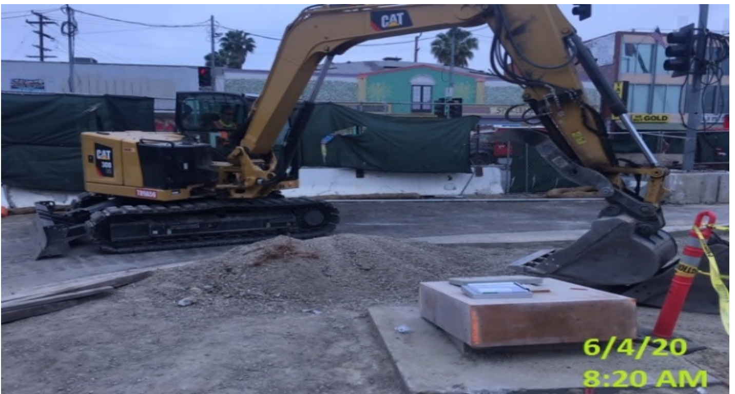
VERNON STATION- WSCC crew grading SW section of station.
