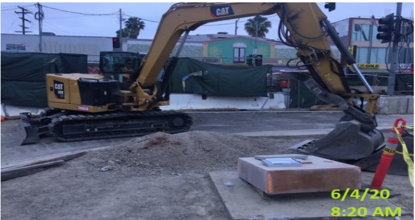
LEIMERT PARK STATION – Excavating/grading at the southwest corner of the plaza level.
