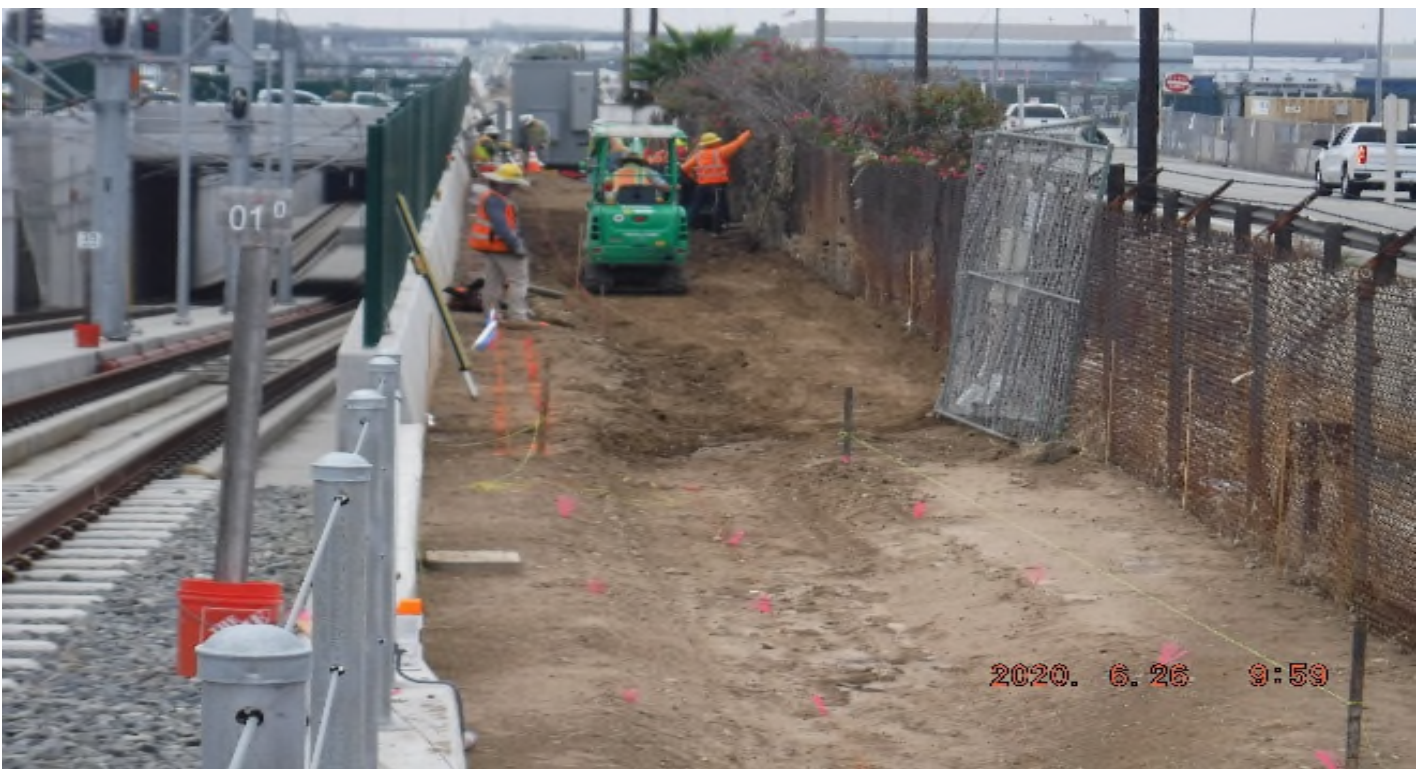
UG1- STA 60+50 looking south V-ditch grading along UG1 wall
