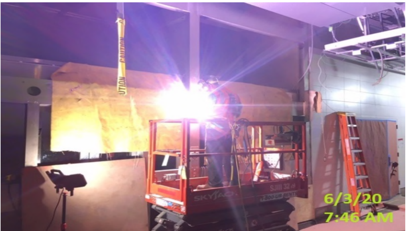
MLK STATION- McMahon Steel welding sections of fascia elevator #3 and #4.
