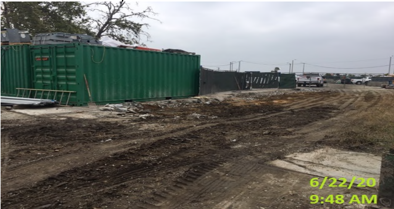
EXPO STATION – Continue demolishing/clearing the north side section of the plaza.
