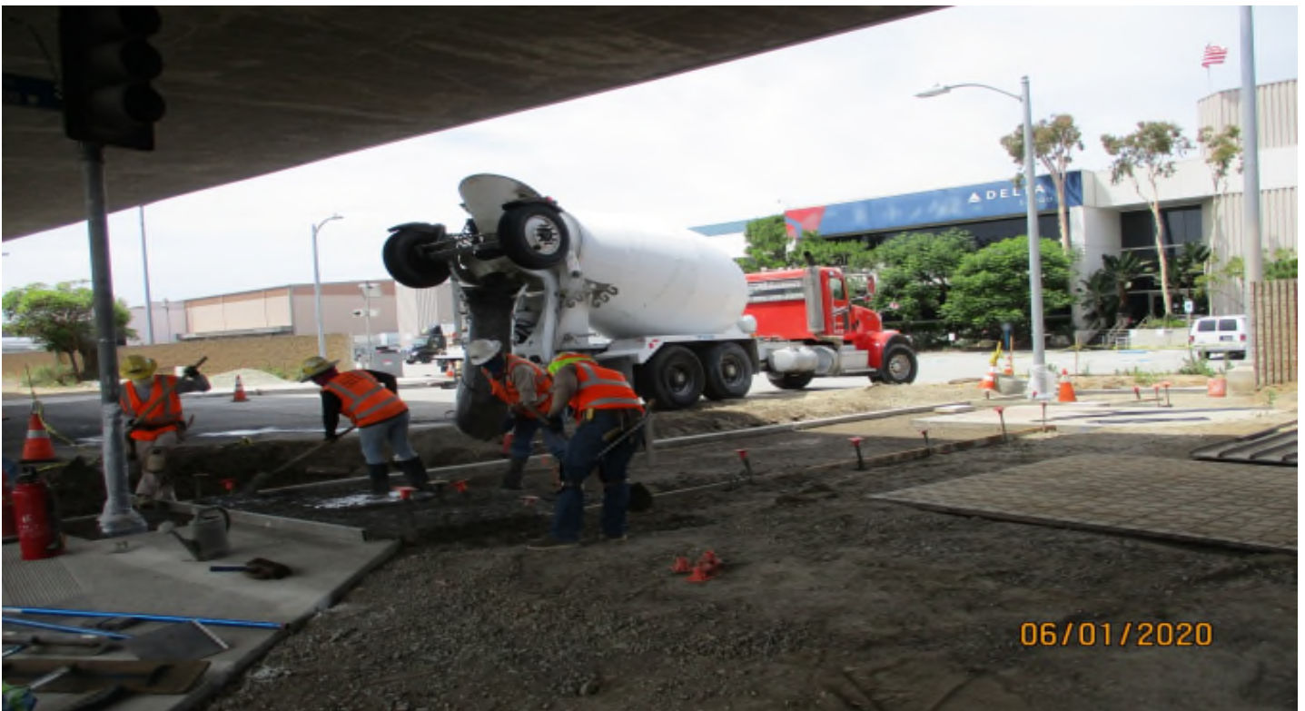
111th Street- Placing concrete for the sidewalk at 111th street.
