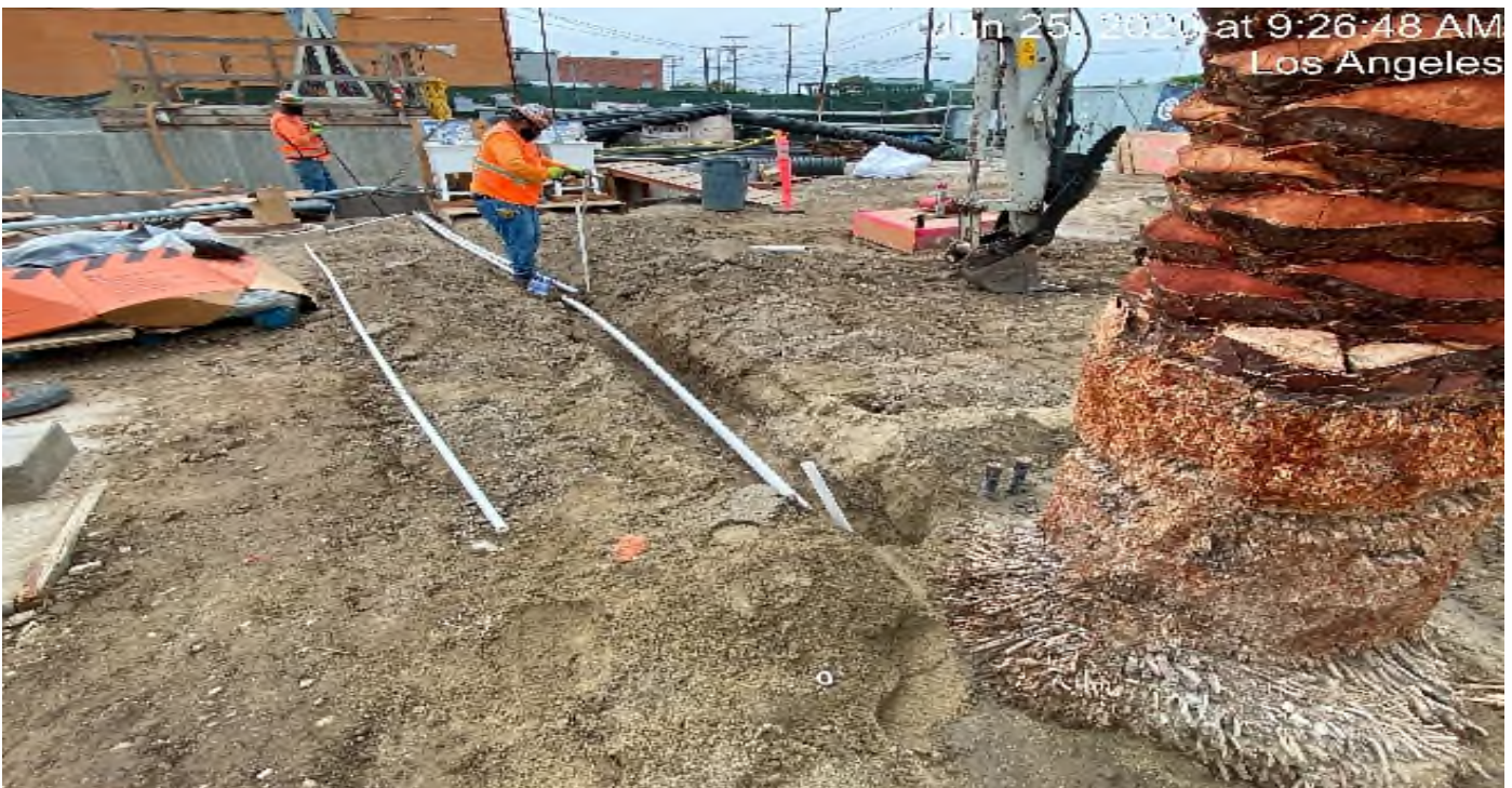
LEIMERT PARK STATION – Installing irrigation lines throughout the plaza level.
