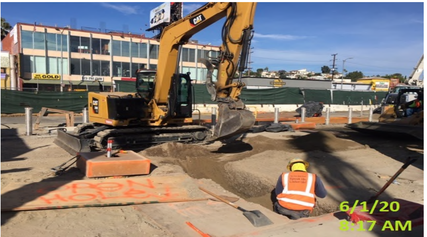
VERNON STATION- WSCC crew excavating for electrical trenches for conduit.
