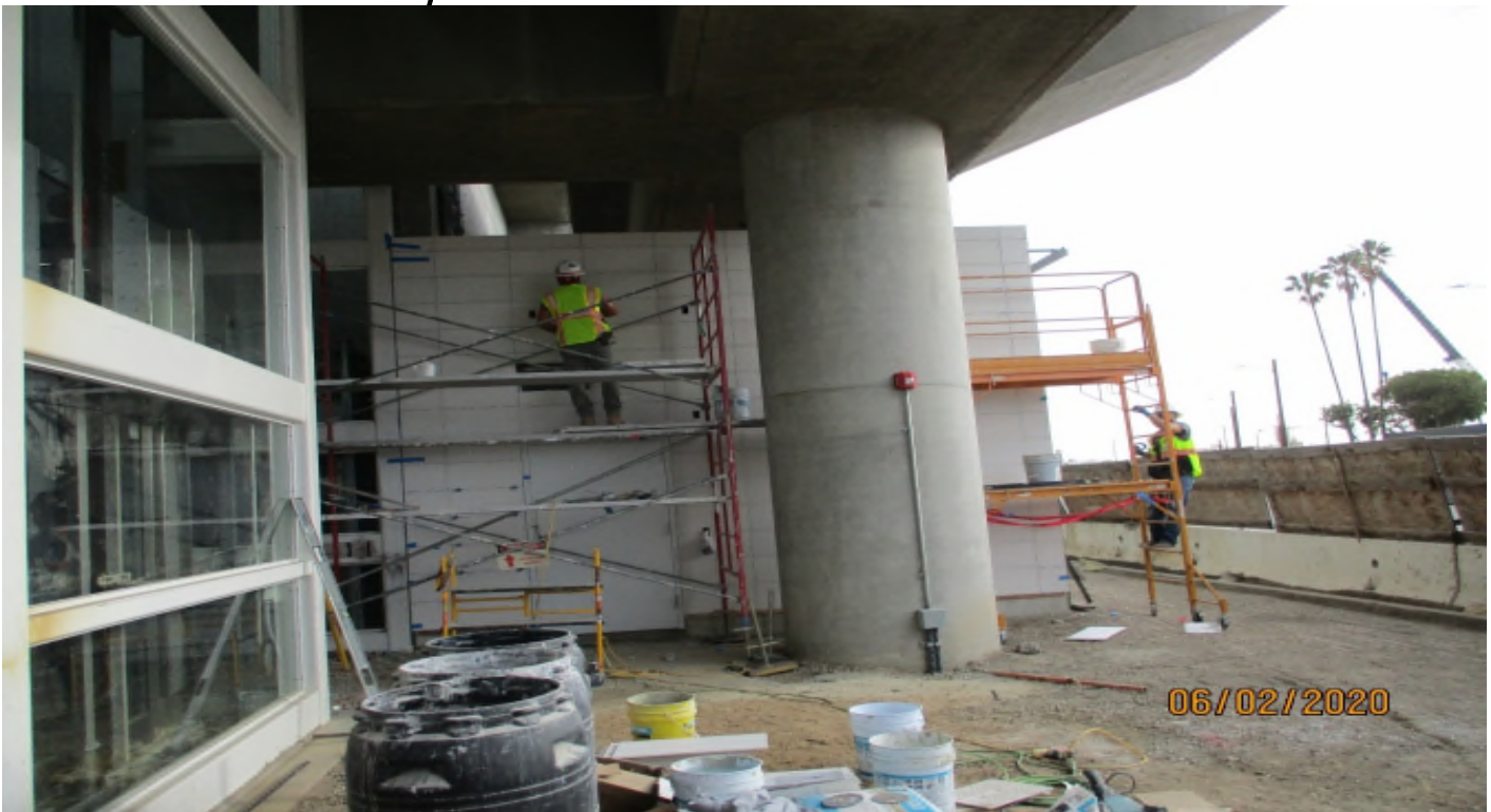
AVIATION/CENTURY- Setting tile for the Aviation Station service building. Facing north.
