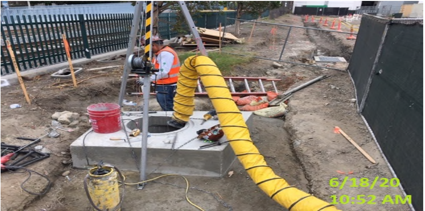
EXPO STATION- WSCC crew chipping and sack & patch inside of manhole #1.
