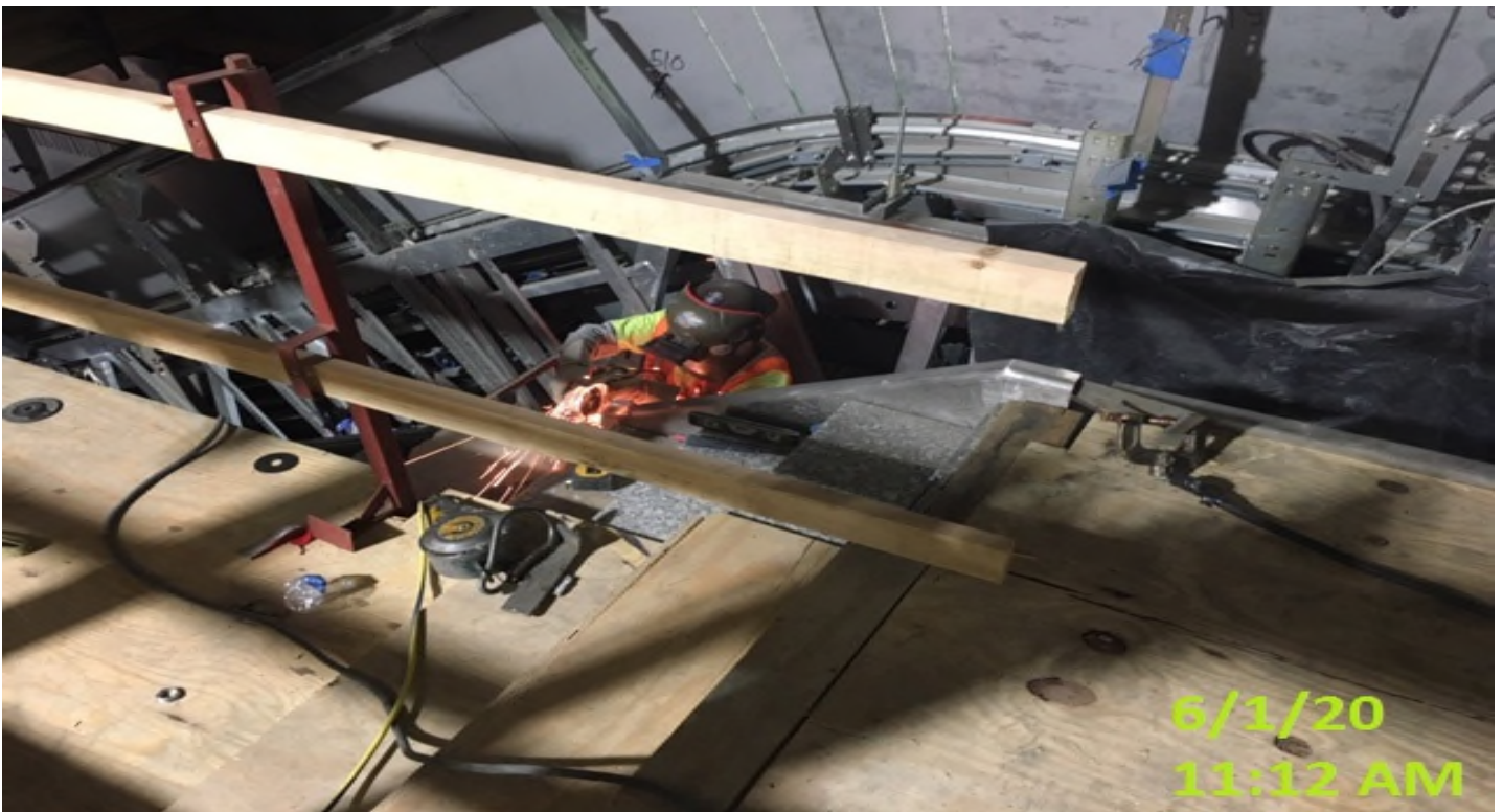
EXPO STATION- McMahon cutting edge plate for hand rail posts.
