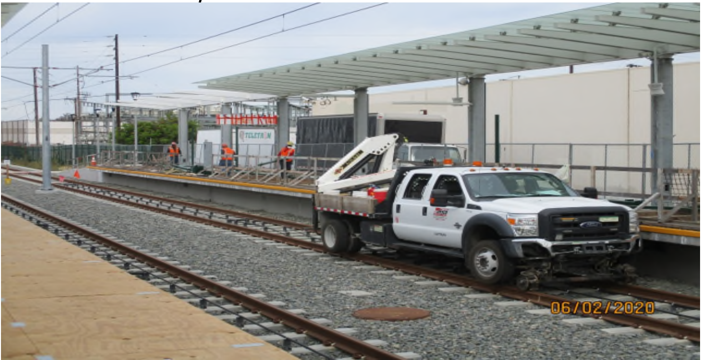
Hindry Station – Setting fence posts at the Hindry Station SB platform.
