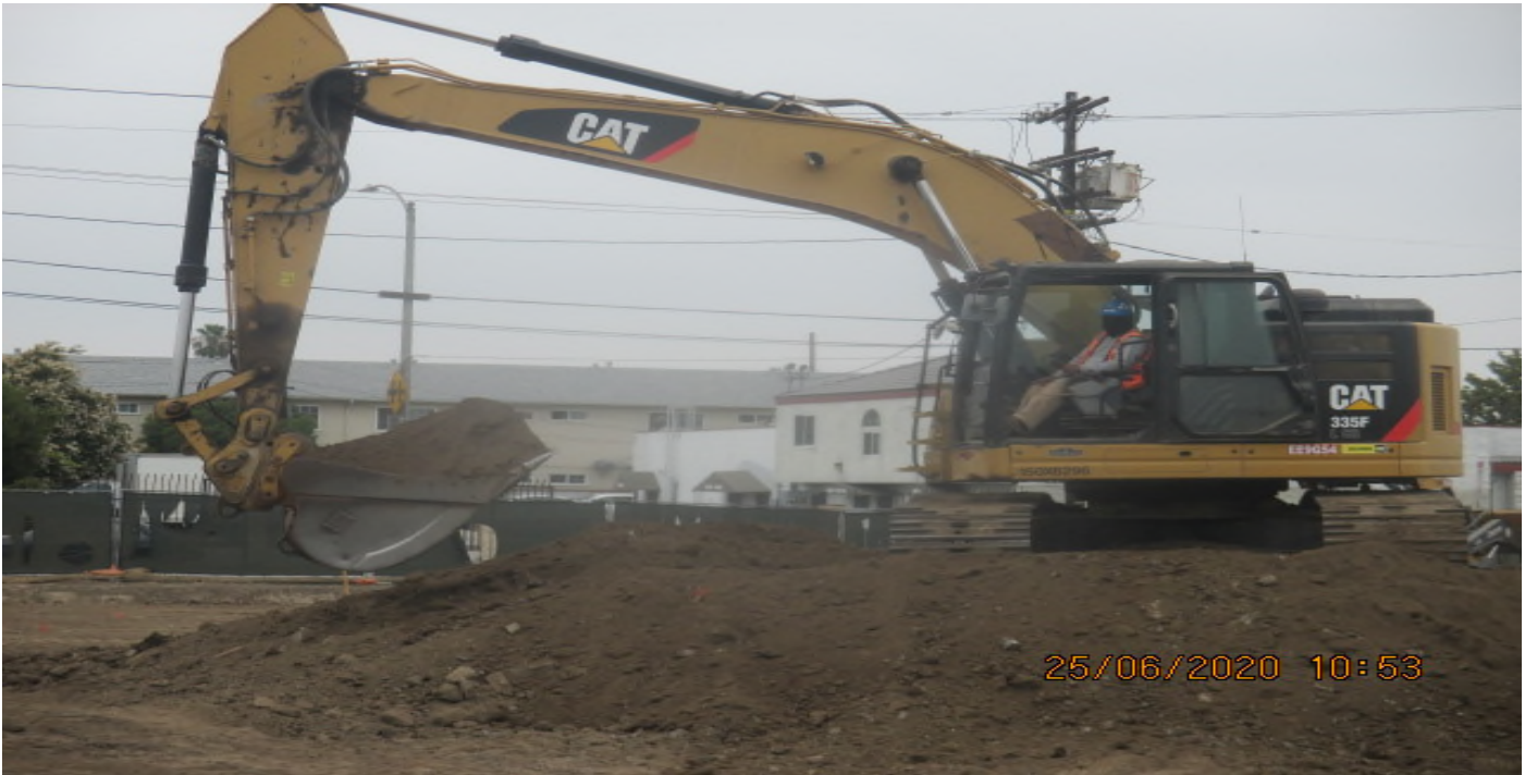
UG3 – Continue excavating/grading the north east section of Victoria Yard. 6/25/20
