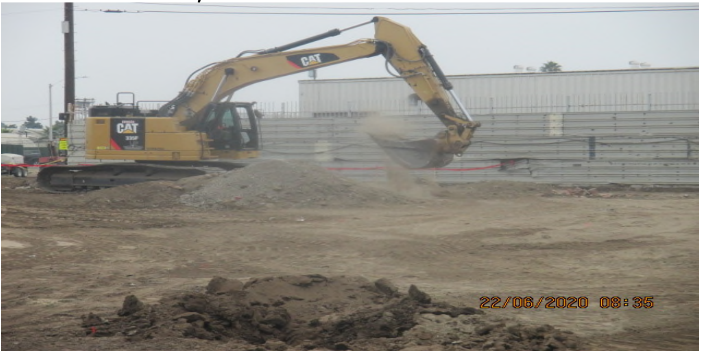
UG3 – Continue excavating/grading the north east section of Victoria Yard. 6/22/20
