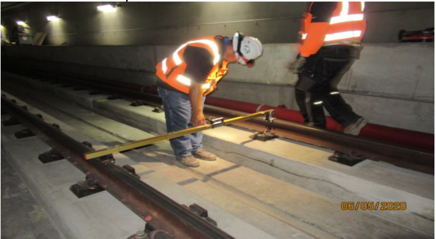
UG4 – WSCC QC inspectors verifying SC on SB-34 UG4 STA 374+32.
