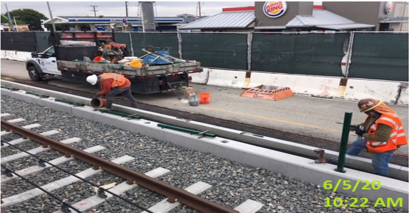
EXPO STATION- Ace Fence installing posts on guardrail curb.
