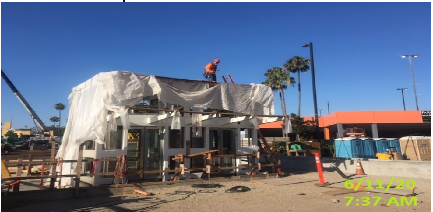
MLK, Installing roofing deck for Elevators 1&2 at the plaza level.
