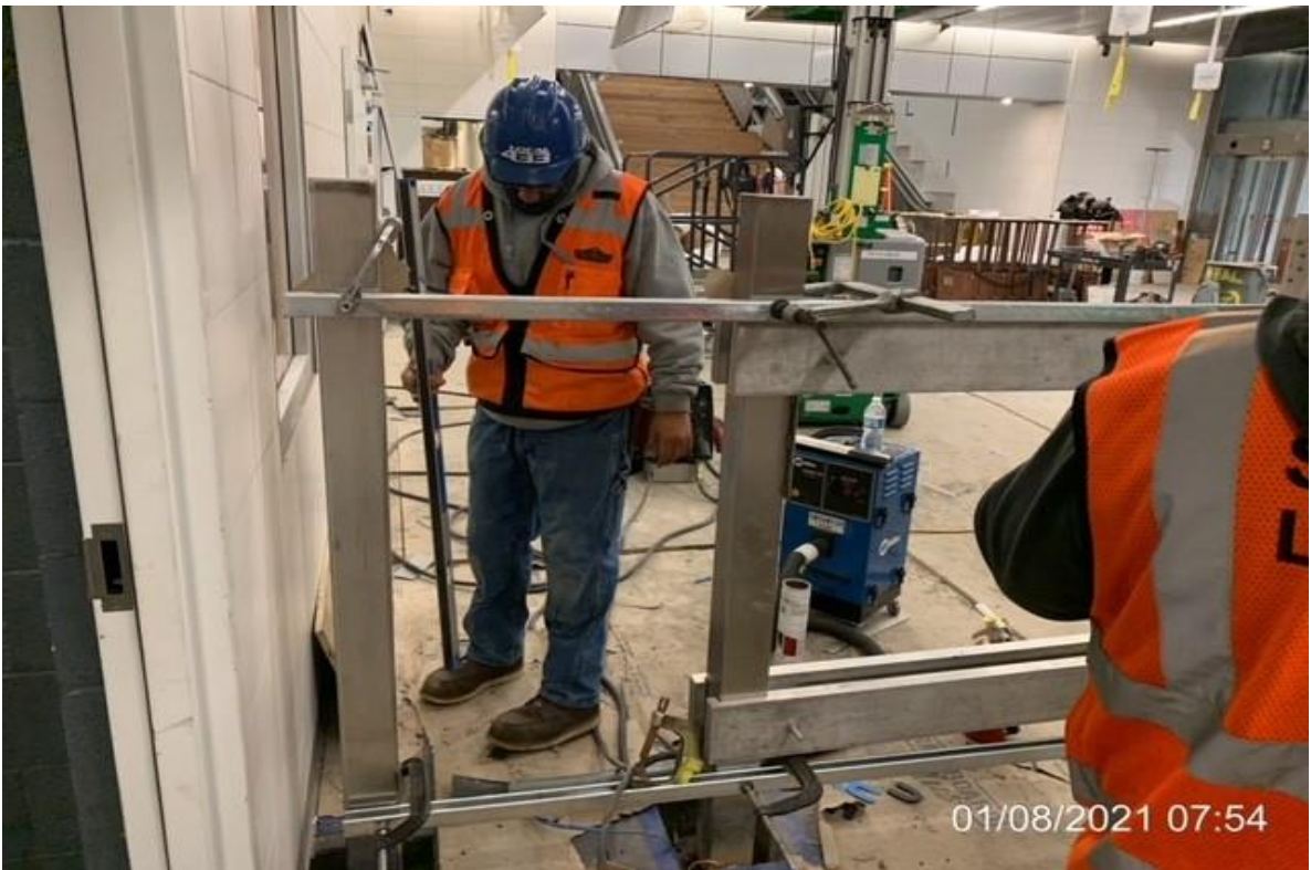
UG3 – Ironworkers installing posts for fare gate picket fence
