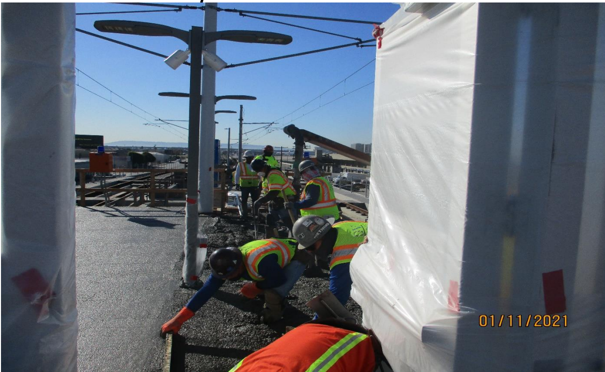
AVIATION/CENTURY- Topping slab concrete placement at the south end of the Aviation Station platform.
