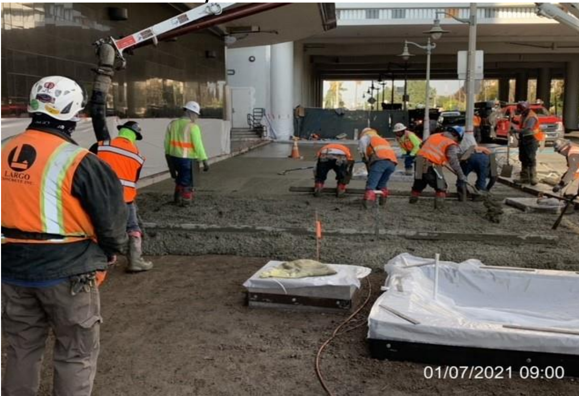
MLK STATION – Griffith placing concrete for sub slab.
