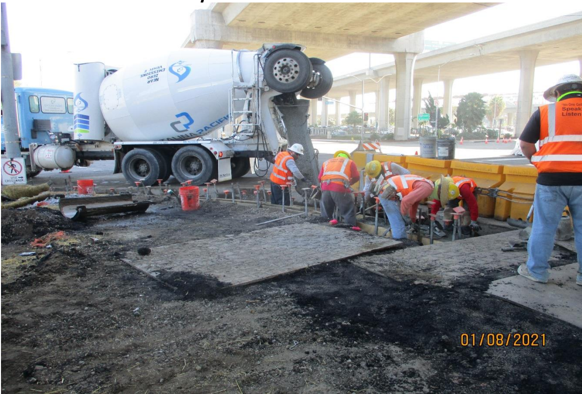
AVIATION/CENTURY- Placing curb and gutter concrete at Aviation and Imperial.
