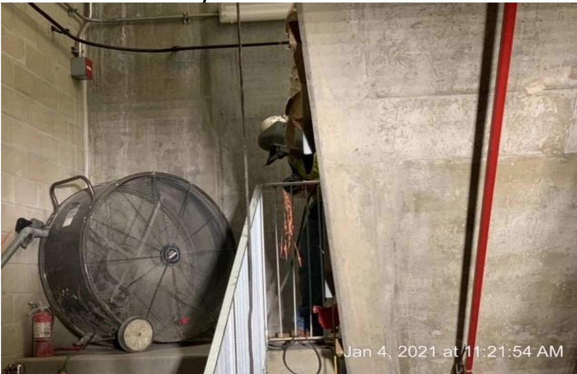
EXPO STATION – McMahon grinding handrails at emergency exit stair #3
