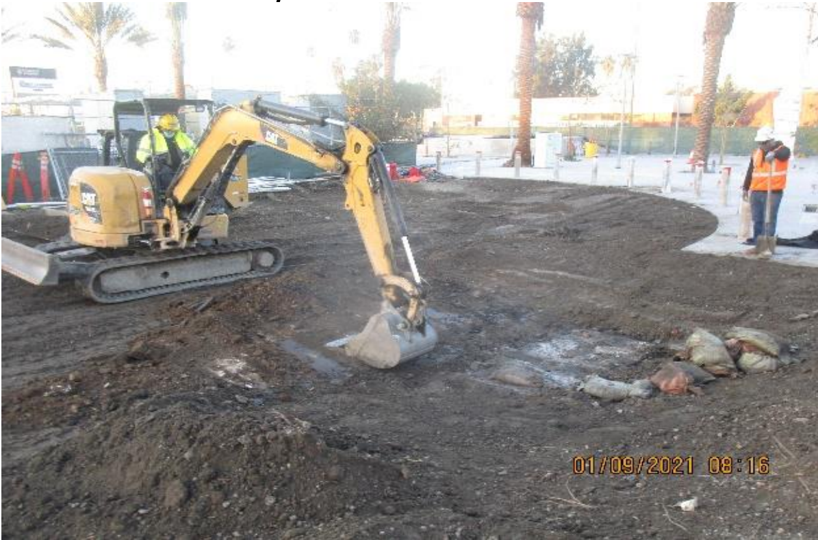
EXPO STATION – continued rough grading slop to drain at beginning of treatment swale #3 & general clean up
