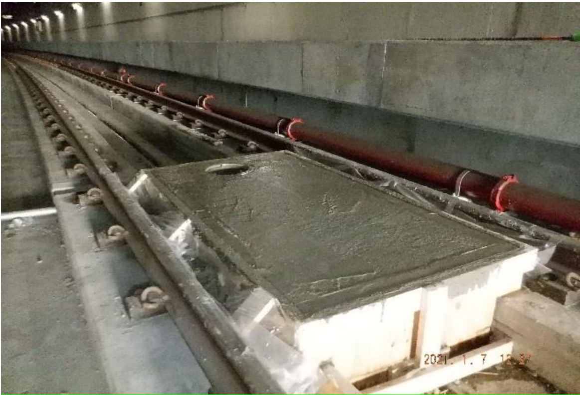
UG4 – STA 372+00 TK#3/SB looking north – UG4 fresh PCC traffic loop detector slab.
