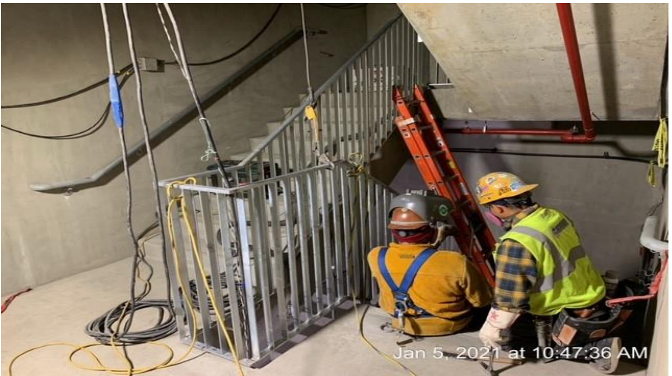
EXPO STATION – Installing and welding guardrails throughout Emergency Exit Stair 4.
