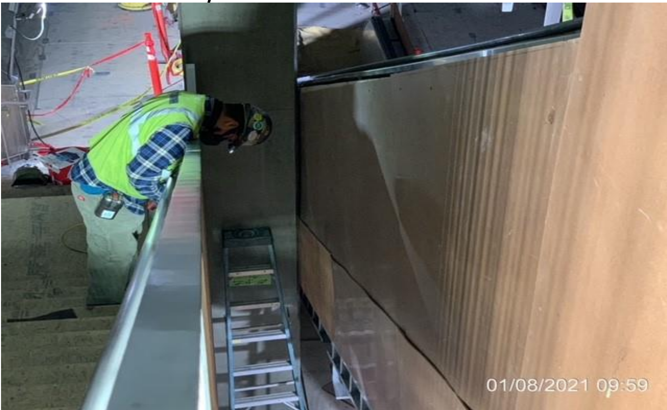
EXPO STATION – Grinding handrail finishes to Staircase 2 from concourse to platform.
