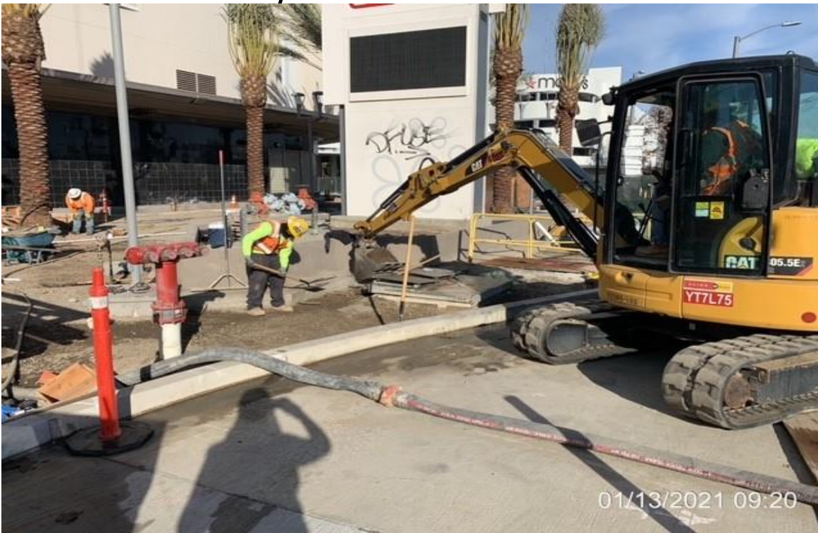
MLK STATION – WSCC crew grading at east side of station.
