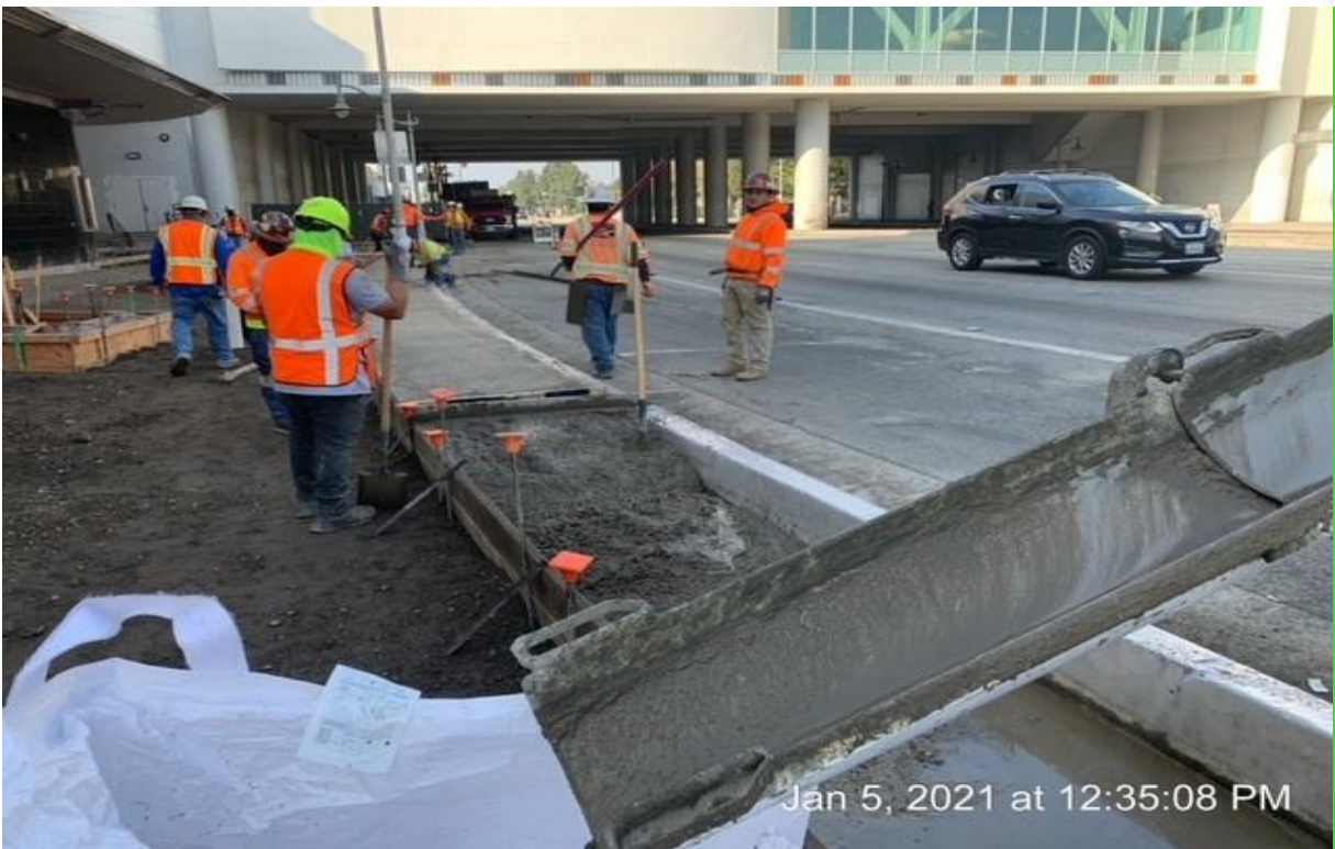
MLK STATION – Griffith placing concrete for sidewalk at north end of station.
