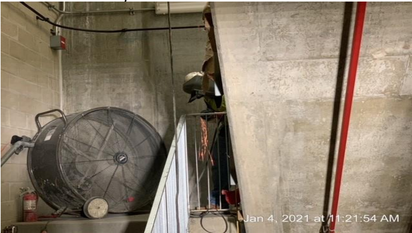
EXPO STATION - Grinding guardrail finishes throughout Emergency Exit Stair 3.
