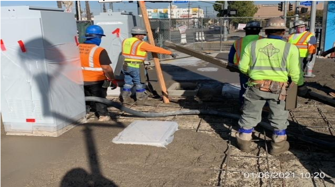
EXPO STATION– Continue placing concrete for the architectural topping slab at the north side of the plaza.
