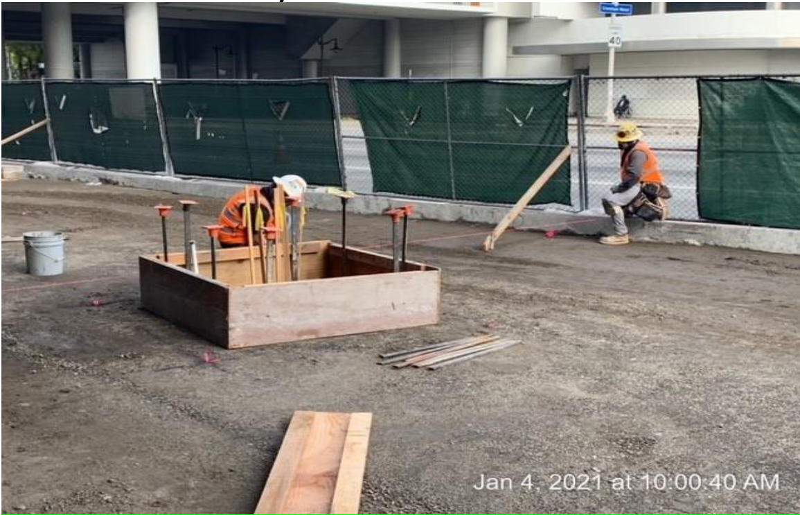
MLK STATION – WSCC carpenters building formwork for concrete tree bases.
