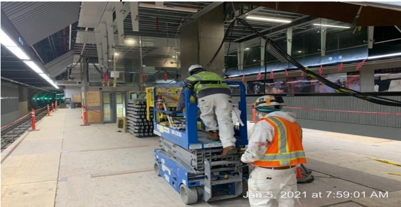
LEIMERT PARK STATION – Preparing to apply primer paint coat to conduits and brackets behind the diagonal screen ceiling panels along the north and southbound side of the platform.
