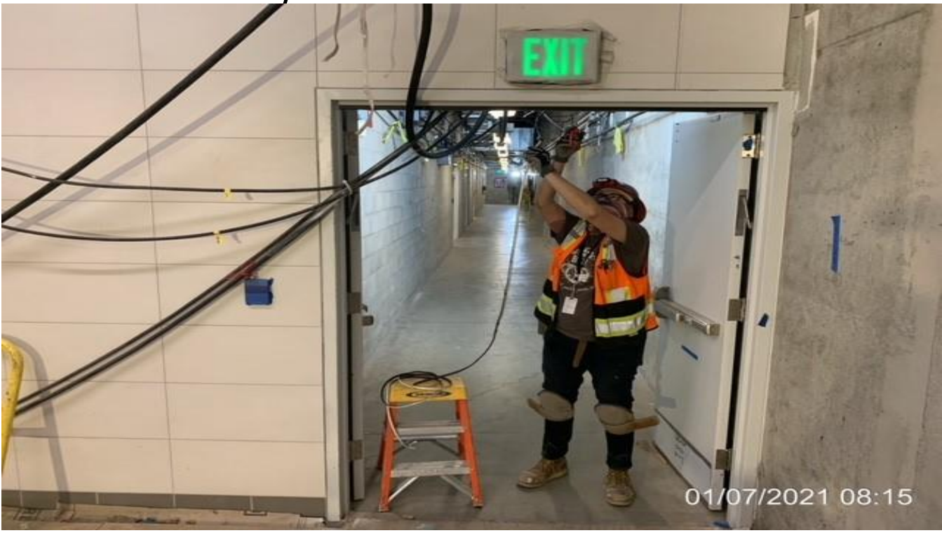
LEIMERT PARK STATION – Continue installing thresholds, fire smoke seals and closures for doors throughout various room at the concourse.
