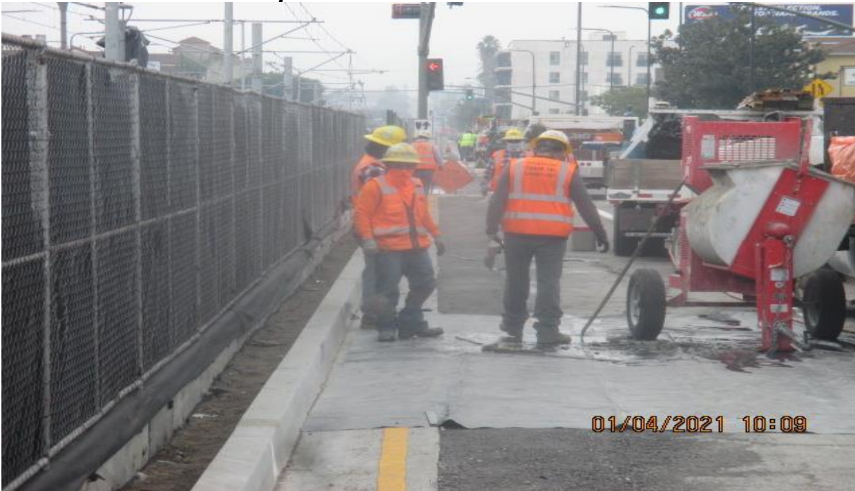
PARK MESA – Mixing and placing mortar base for cobble installation on the southbound median curb on Crenshaw Blvd from 59th St to 58th Pl.
