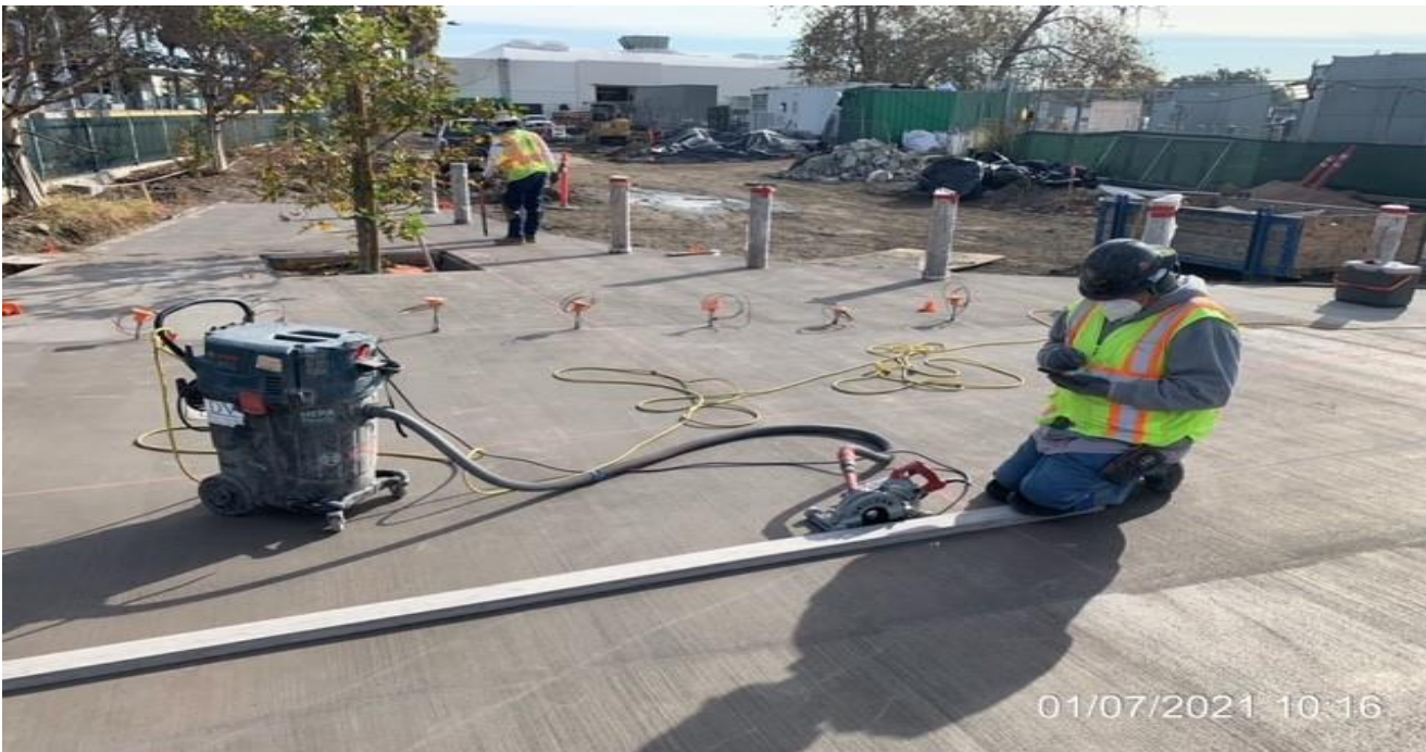
EXPO STATION – Saw cutting control joints to the architectural topping slab at the north side of the plaza.
