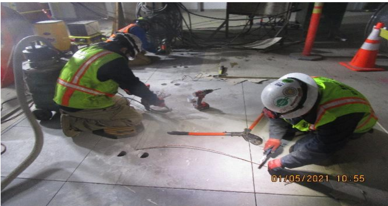
MLK STATION – Continue layout and coring through the walker ducts in preparation for the turnstile fare gate system installation at the Paid & Free Area.
