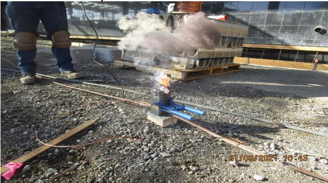
MLK STATION – Continue ground grid installation throughout the plaza.
