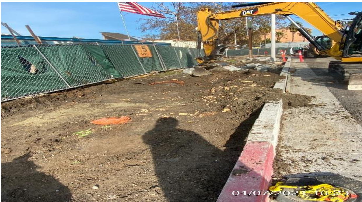
EXPO STATION – Excavating the entire southbound sidewalk along the Bronson Cul-de-sac.
