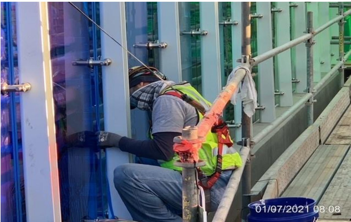
UG3 – Giroux Glass caulking between art wall glass panels
