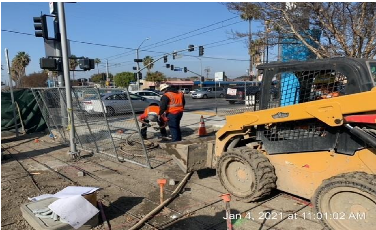
EXPO STATION – WSCC crew demoing sidewalk for plaza slab.
