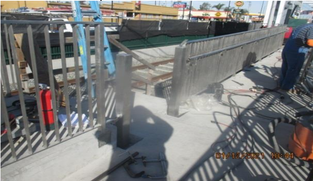
PARK MESA – Installing pedestrian safety gate at the south entrance walkway ramp.
