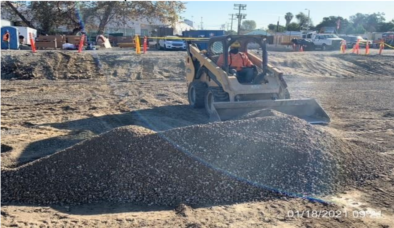
EXPO STATION – Continue rough grading and placing base on the north side of the Park & Ride lot area.
