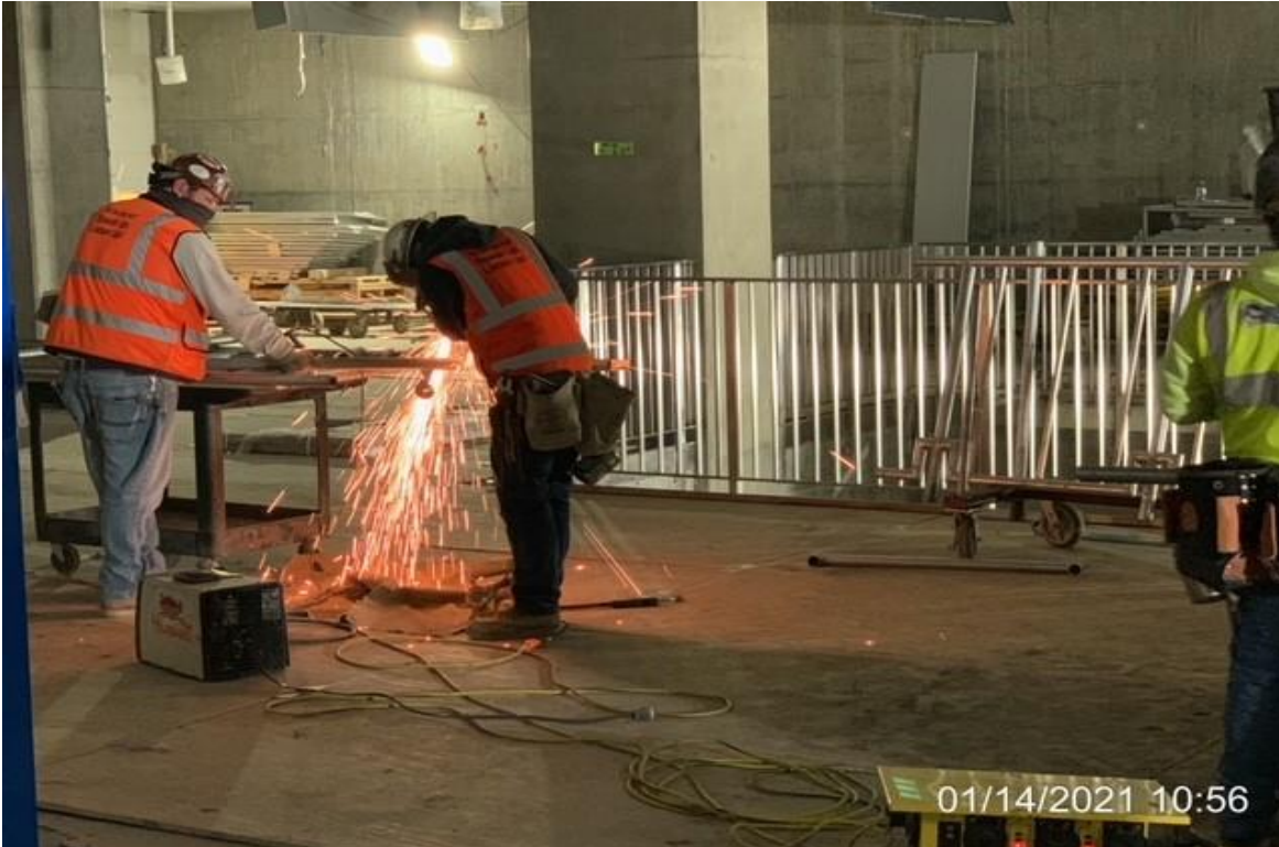
EXPO STATION – McMahon fabricating guard rail for north EVF dampers.
