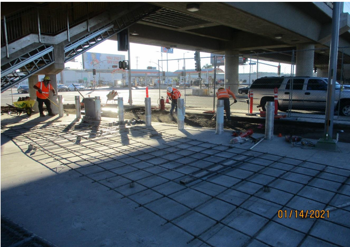
AVIATION/CENTURY- Grading the base for the hardscape at the Aviation Station plaza. Facing SE.
