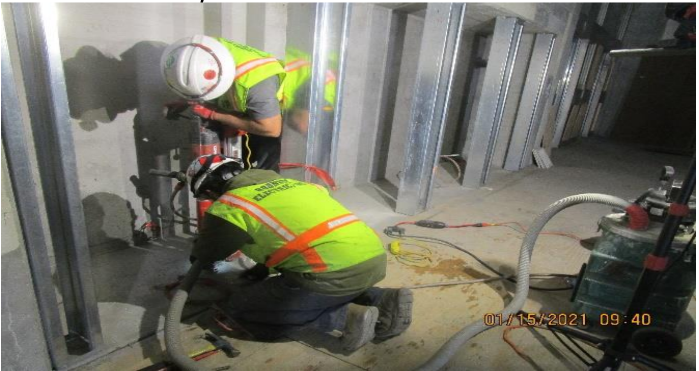
MLK STATION – Performing layout and coring for ticket vending machine installation at the Free Area.
