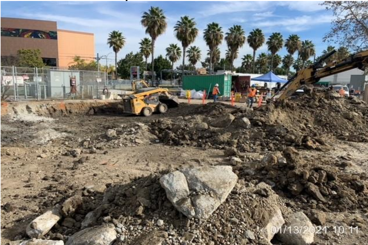
EXPO STATION – WSCC rough grading NW side of park and ride.
