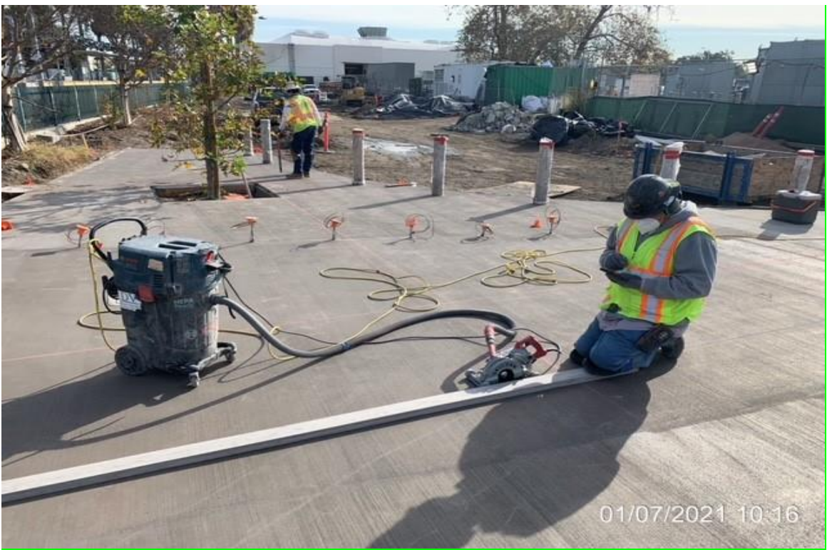
EXPO STATION – McMahon grinding handrails at emergency exit stair #3
