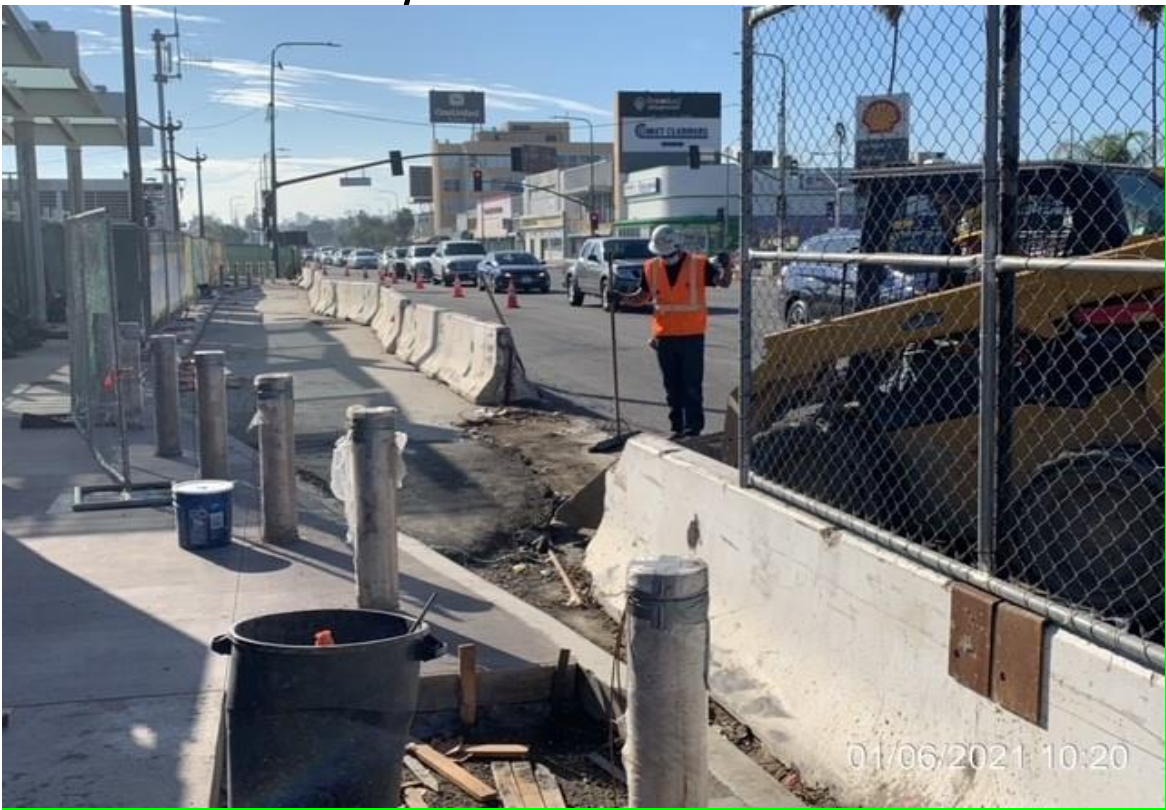
EXPO STATION – WSCC relocating K rail for pedestrian walkway.
