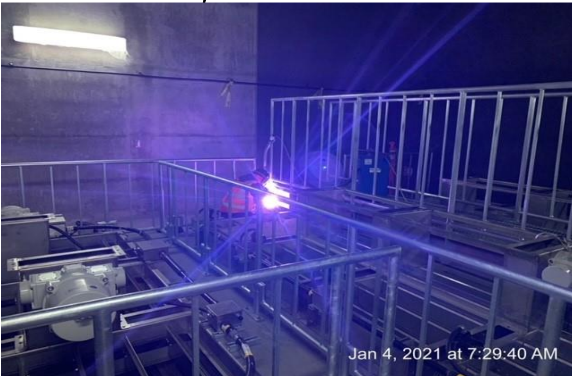
UG3 – WSCC ironworkers welding stiffener plates on cat walk guard rail.
