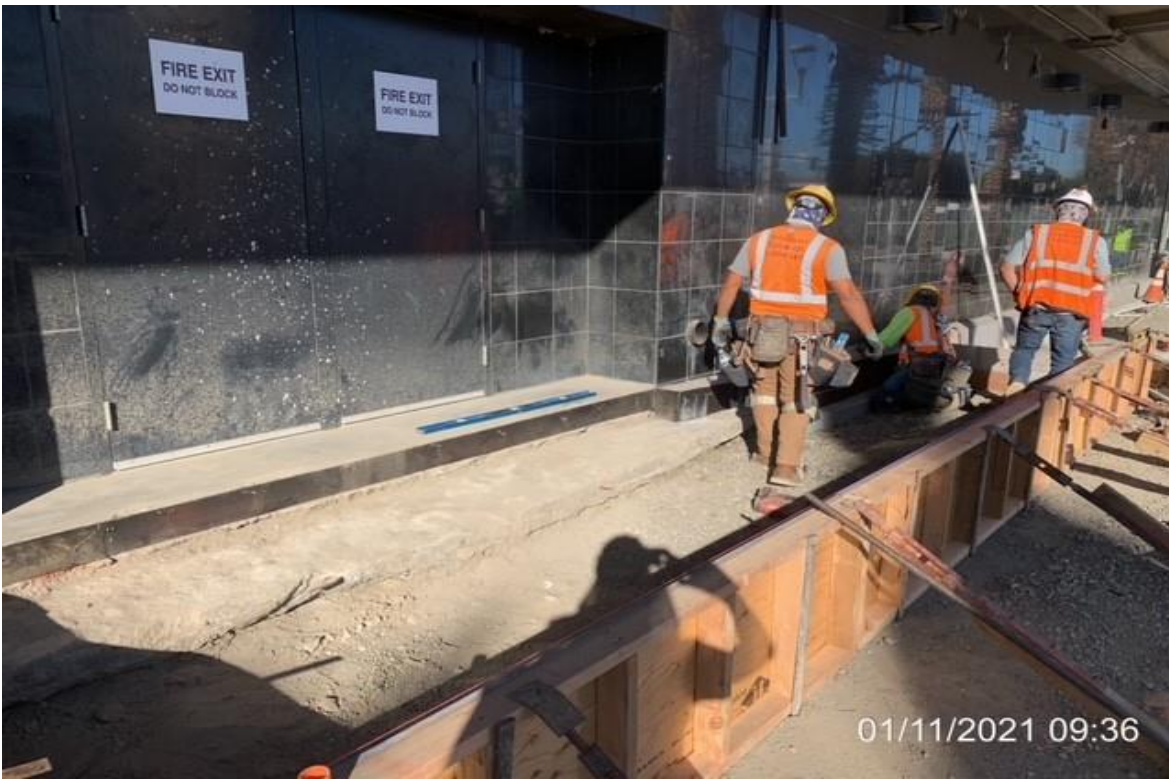
MLK STATION – WSCC crew building formwork for entrance landing.
