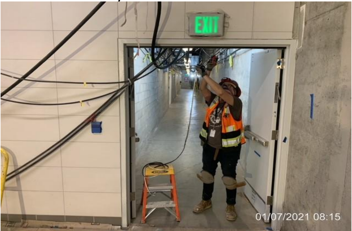
UG3 – Chuck Holland installing fire seals on doorways.
