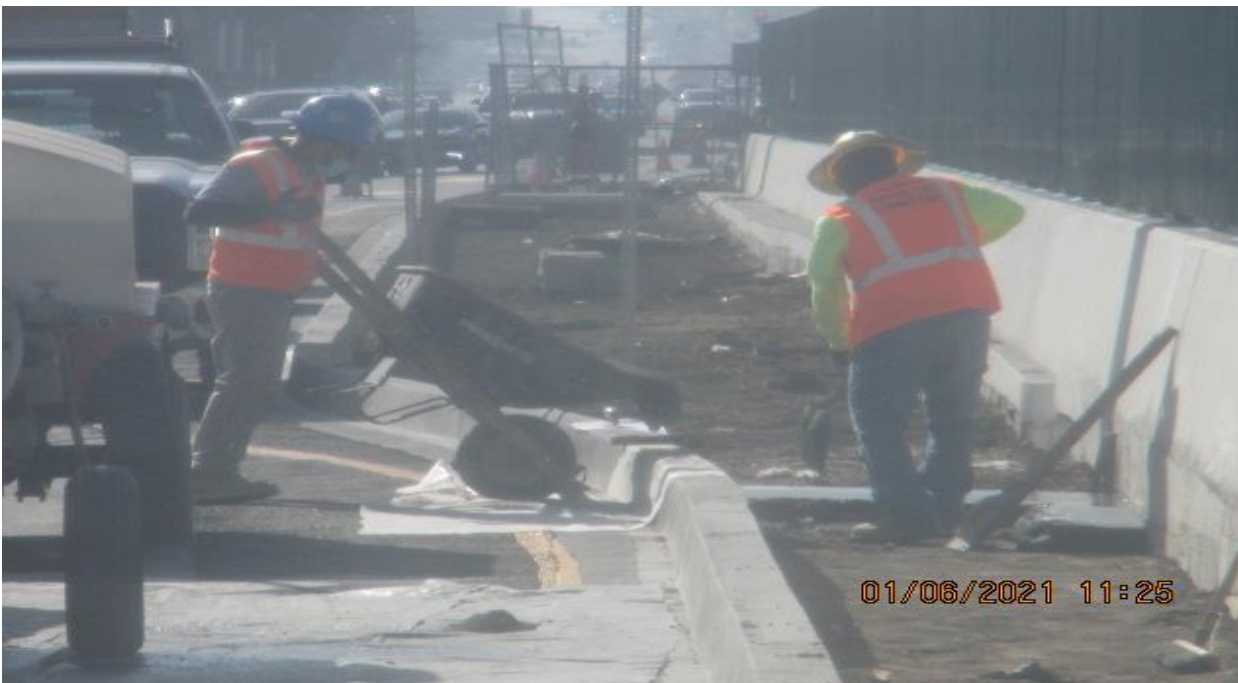
PARK MESA – Continue mixing and placing mortar base for cobble installation on the northbound median curb on Crenshaw Blvd from 59th Pl to 59th St.
