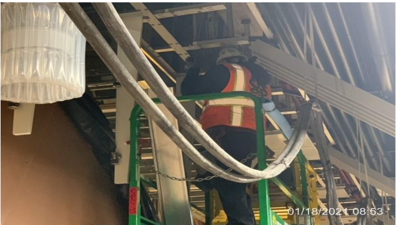
MLK STATION – Installing support framing for stainless steel cladding around the smoke screens of Escalator 4 at the platform.
