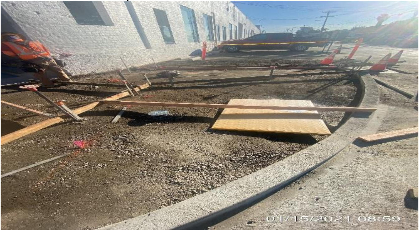
EXPO STATION – Building formwork for new ADA ramp on the northeast side of the Bronson Cul-de-sac.
