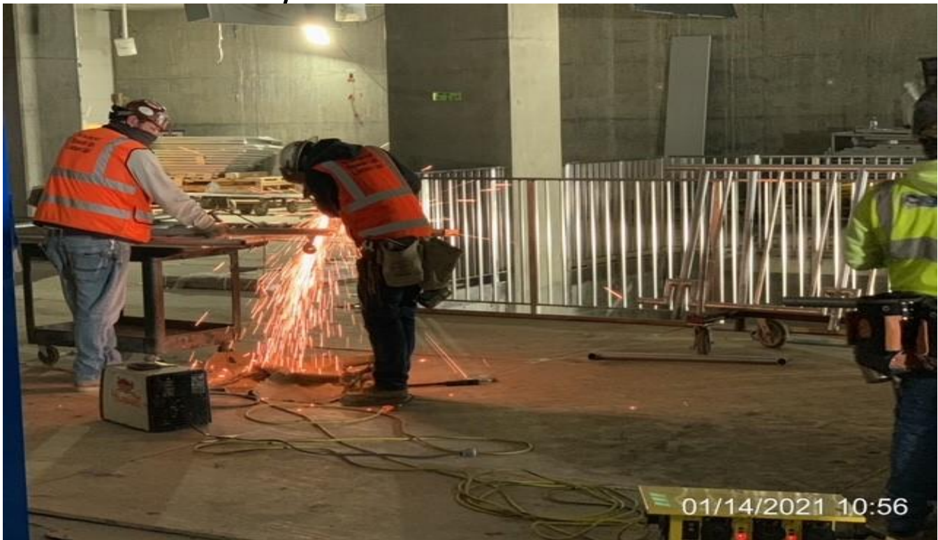
EXPO STATION – Fabricating guardrails for installation inside the Emergency Ventilation Shaft/OTE Plenum North C-126.
