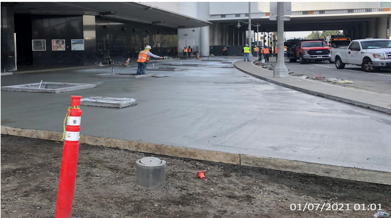
MLK STATION – Spraying curing compound to the entire concrete slab on the northwest section area.
