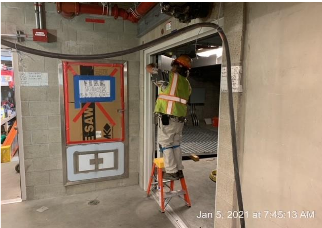
UG3 – Chuck Holland crew installing fire seal on doors
