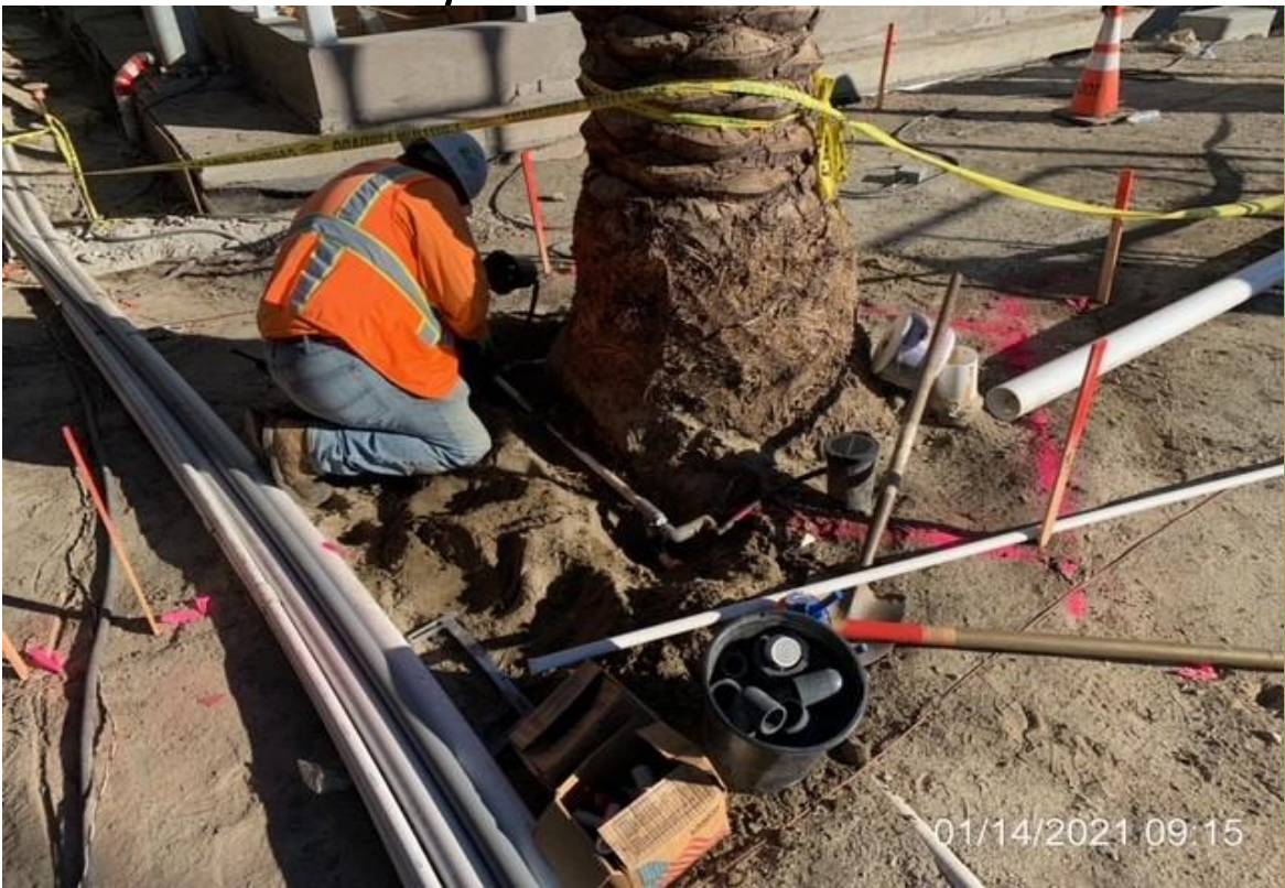
MLK STATION – Marina Landscaping setting irrigation lines within tree well.
