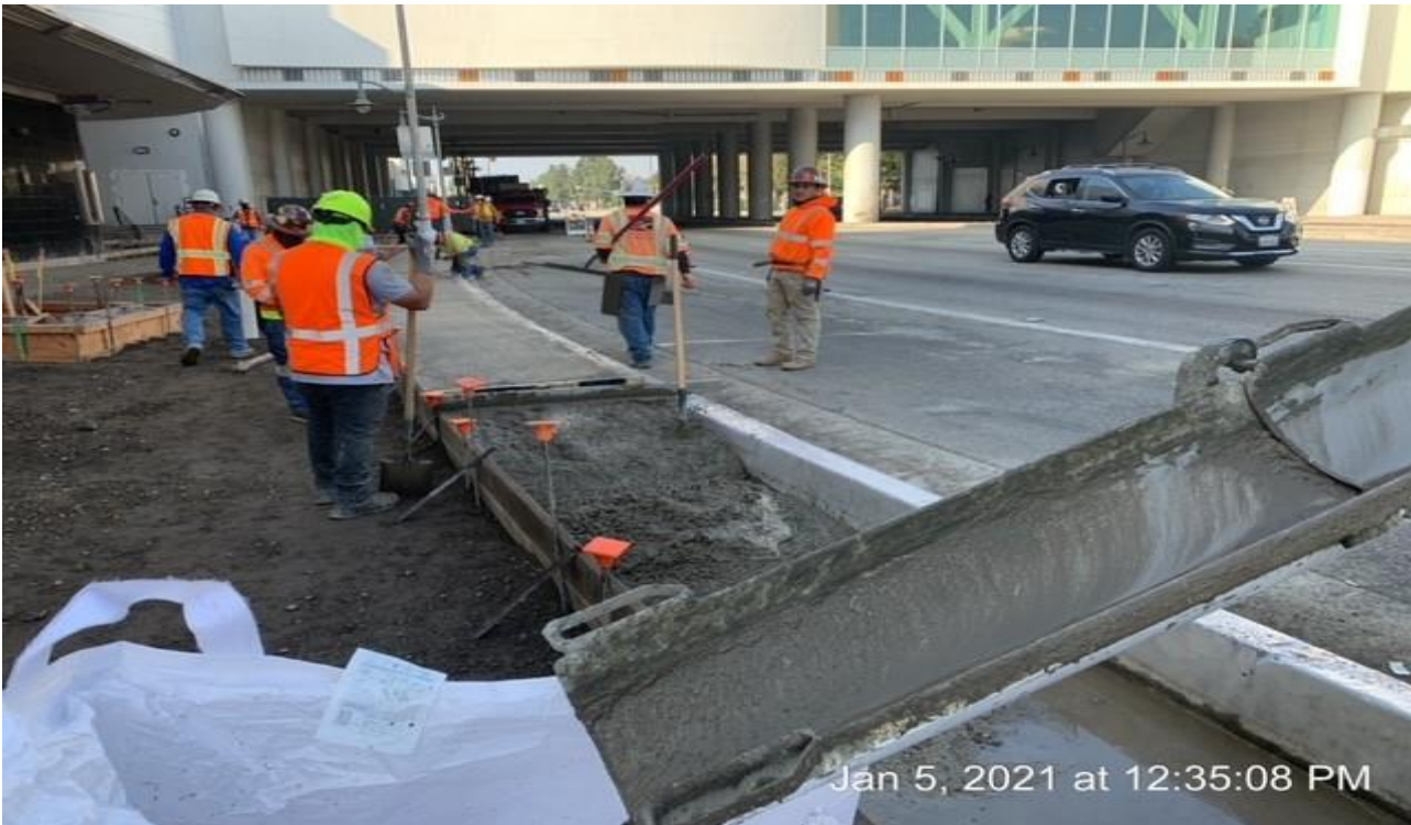
MLK STATION – Placing concrete for new sidewalk installation along the north side of the plaza.
