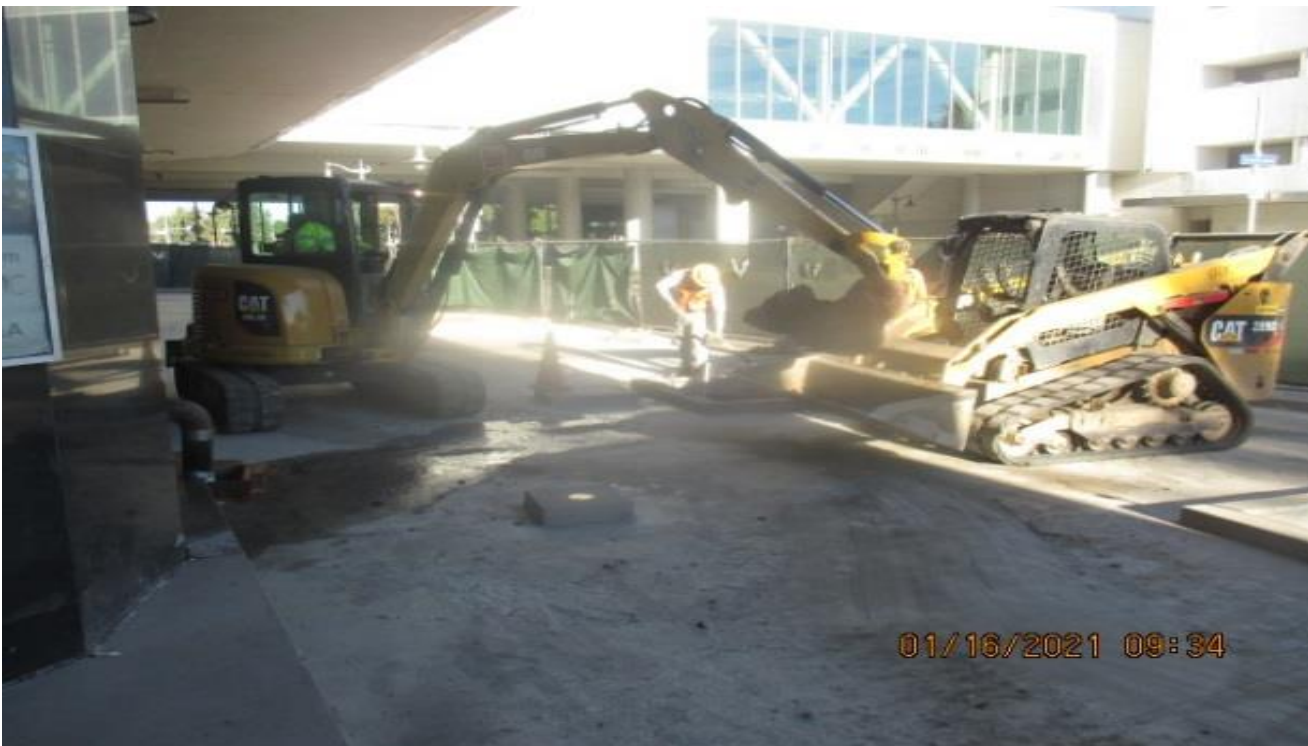
MLK STATION – WSCC crew removing forms from short curb wall along north mall wall.
