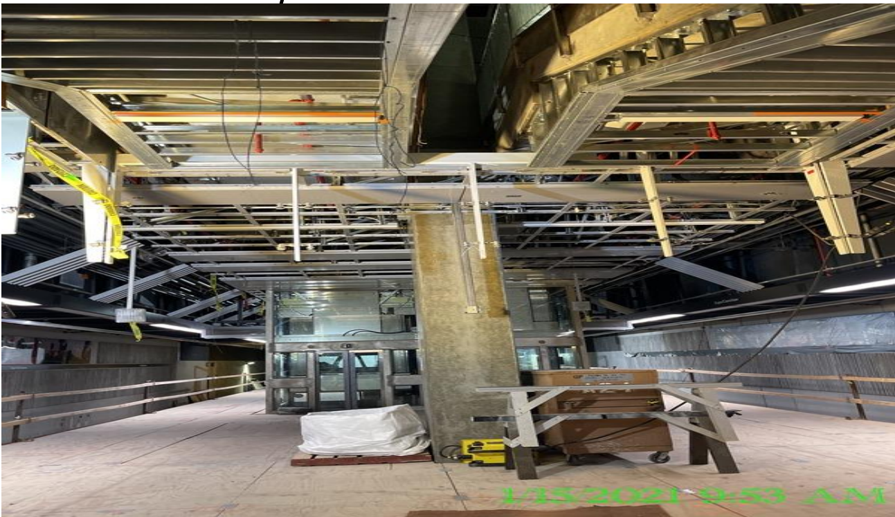
EXPO STATION – Continue installing LED light fixtures to the platform ceiling.
