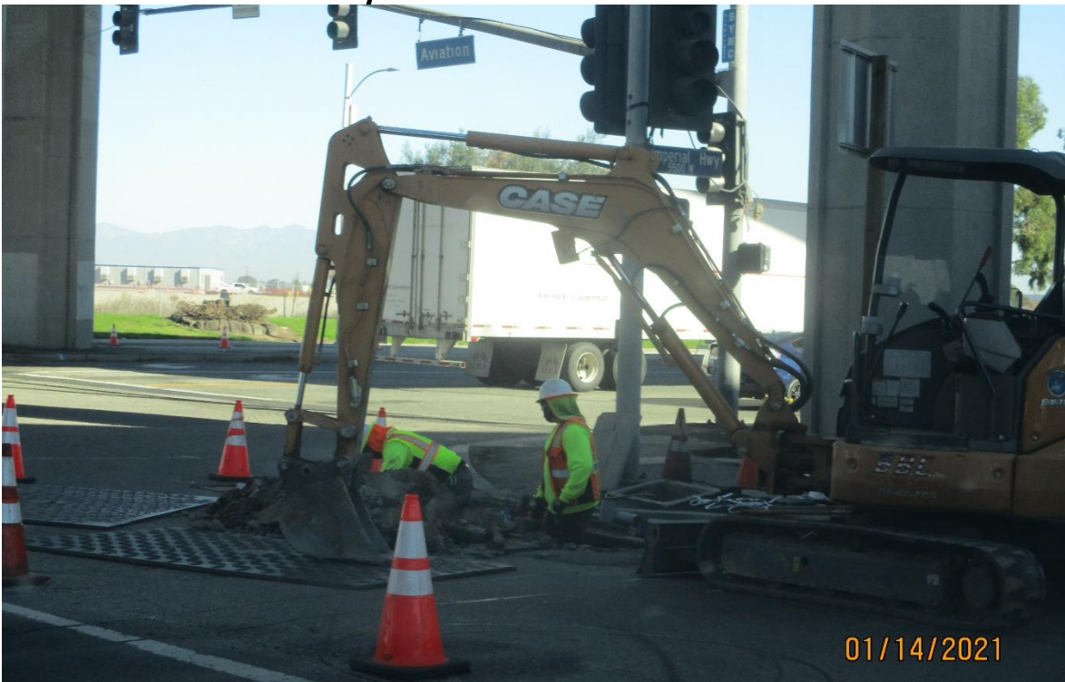
AVIATION/CENTURY- Traffic signal conduit installation at Aviation and Imperial.
