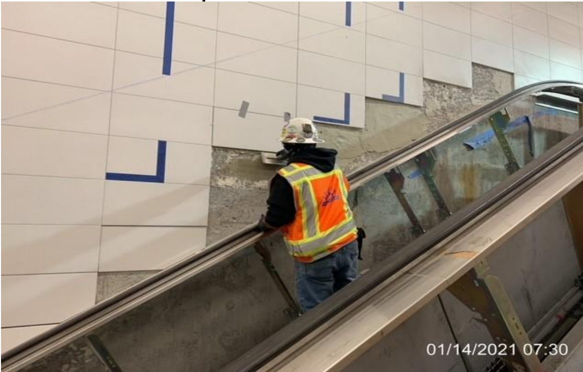
UG3 – Premier Tile & Marble installing missing tiles.
