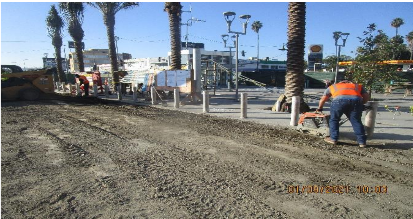
EXPO STATION – Graded/backfilled and compacted the east side of the plaza for drainage swale installation.
