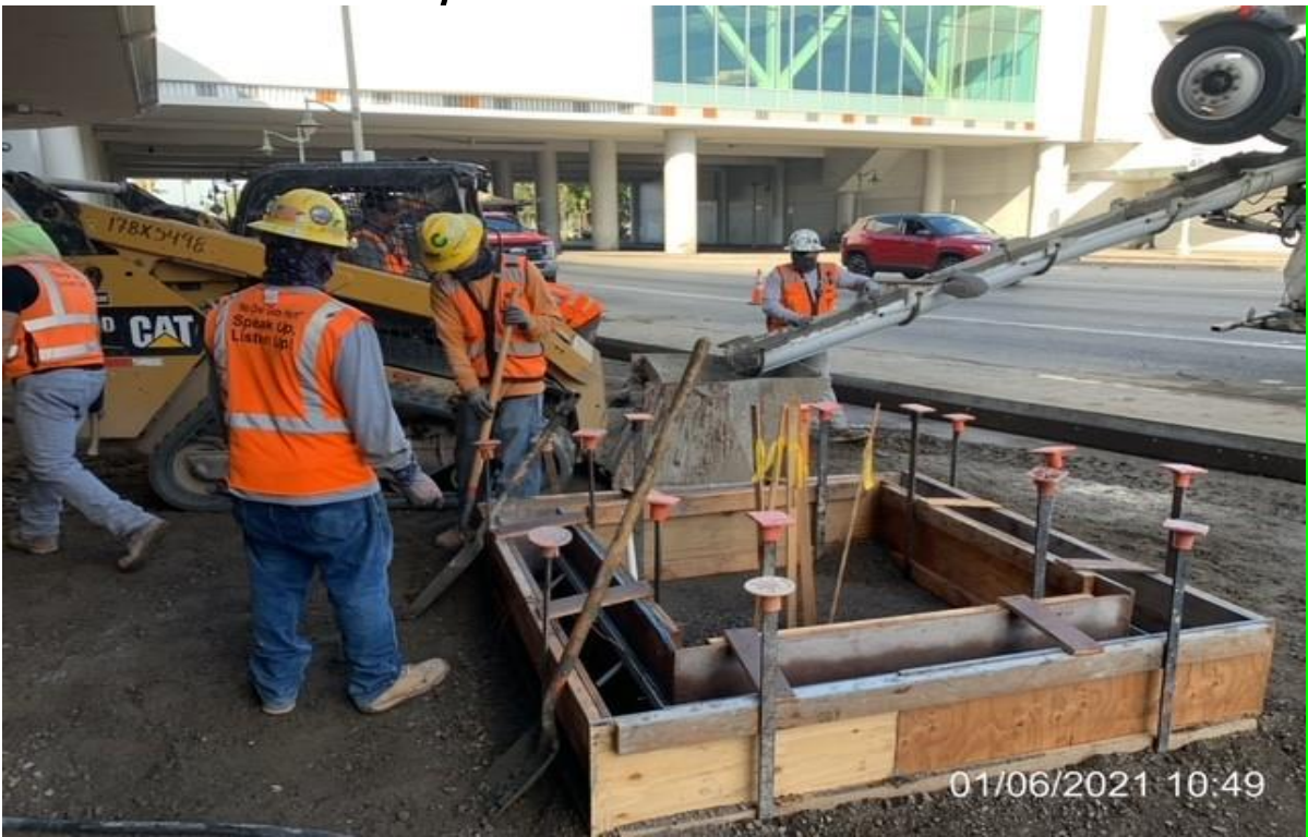
MLK STATION – WSCC crew placing concrete for tree well curbs
