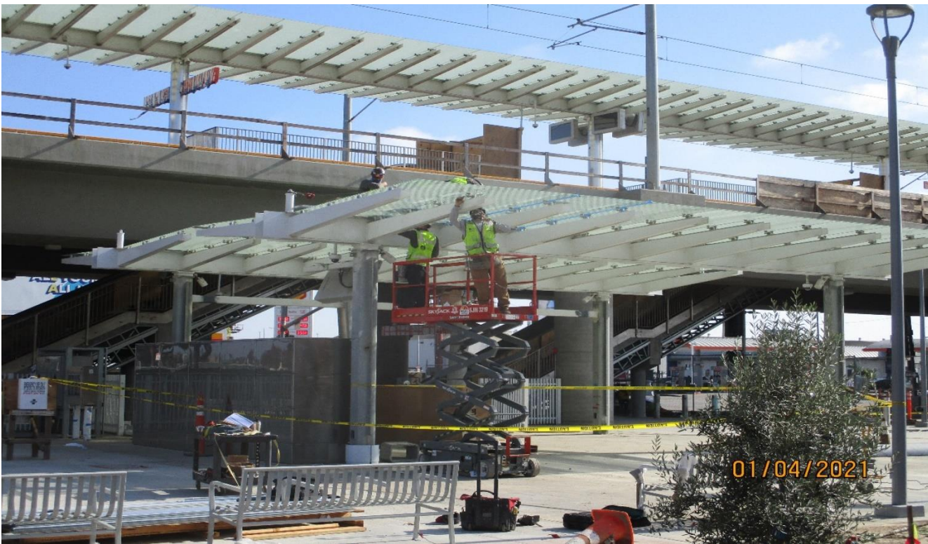
AVIATION/CENTURY- Glass replacement at the Aviation Station TVM structure
