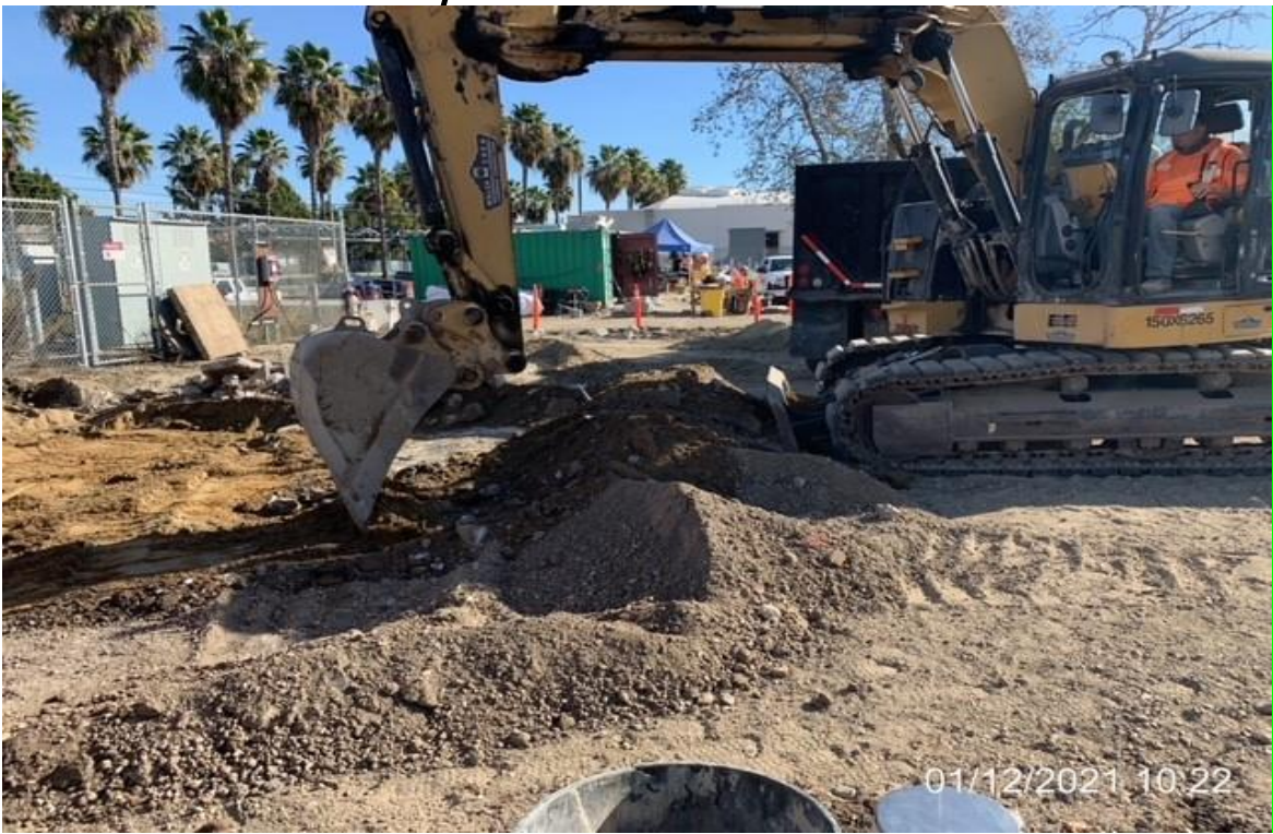
EXPO STATION – WSCC rough grading west side of park and ride.
