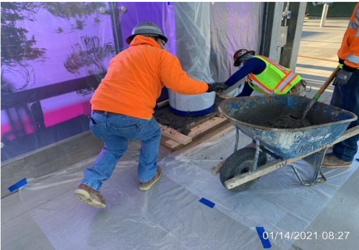
UG3 – Dean Visosky placing concrete for canopy column base.
