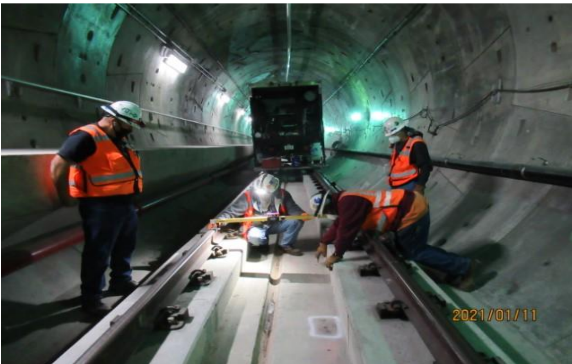
UG4 – HCC using plum bob for SB track at UG4 alignment on open issues log 000253 log status update to reflect “closed” Rework
