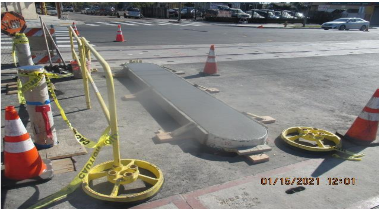
PARK MESA – Placed concrete for safety curb footings on both the north and south end crosswalks at Slauson Ave and 59th St.
