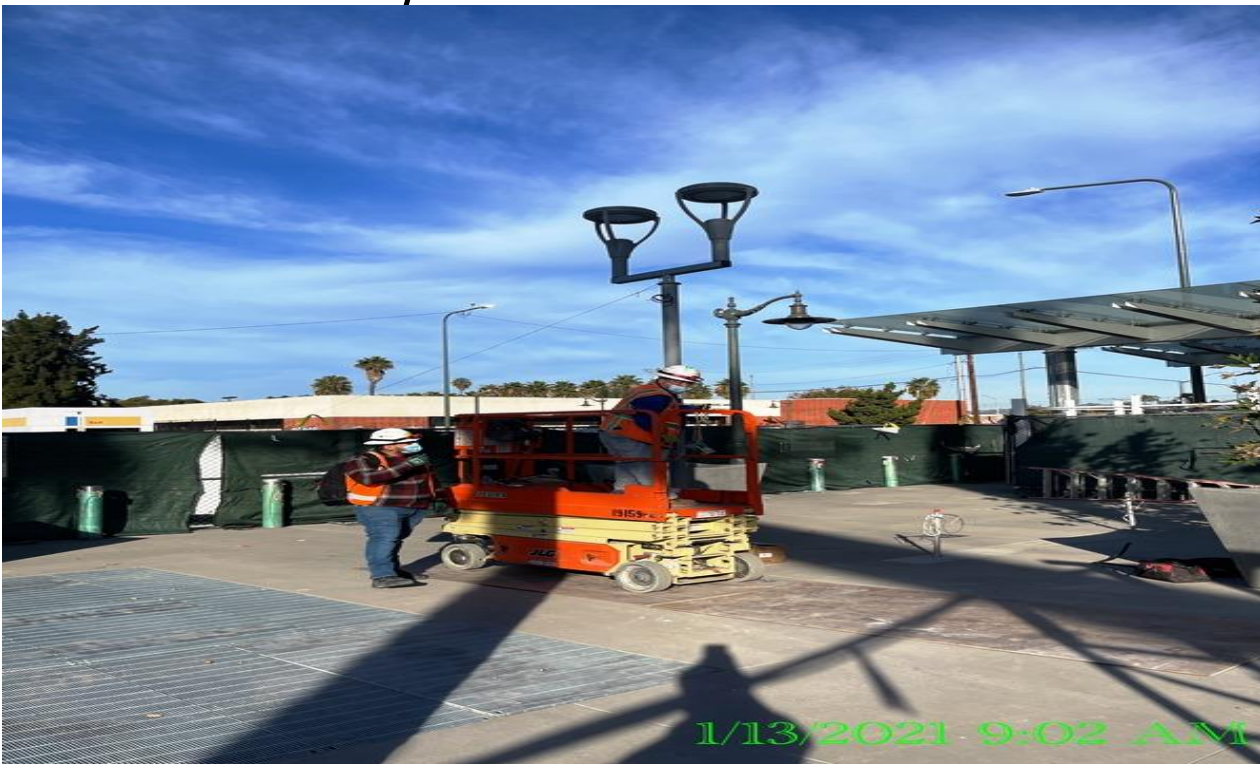
EXPO STATION – Installing CCTV camera supports to all the pedestrian light poles at the plaza.
