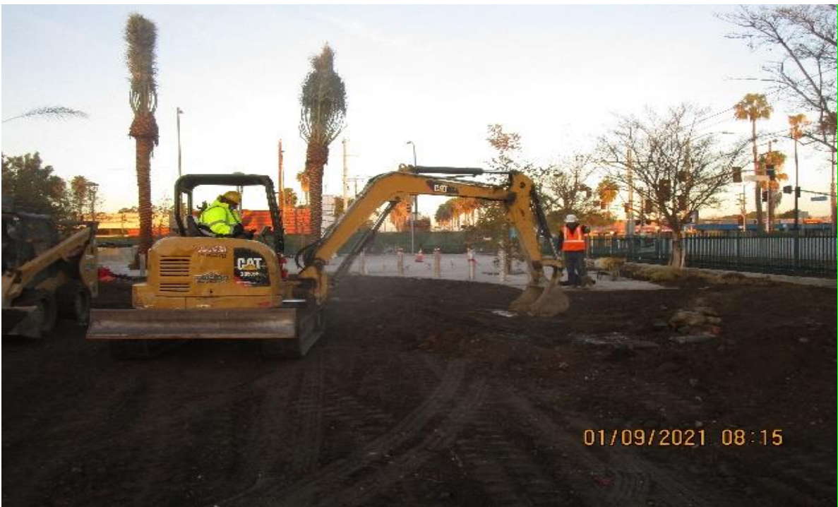
EXPO STATION – begin rough grading slop to drain at beginning of treatment swale #3 east of bollards.
