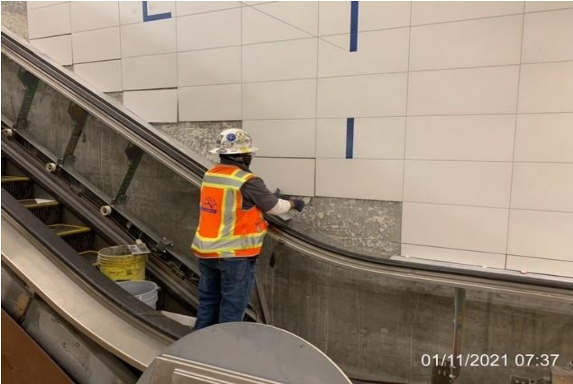
UG3 – Premier Tile & Marble installing wall tiles between escalator #4
