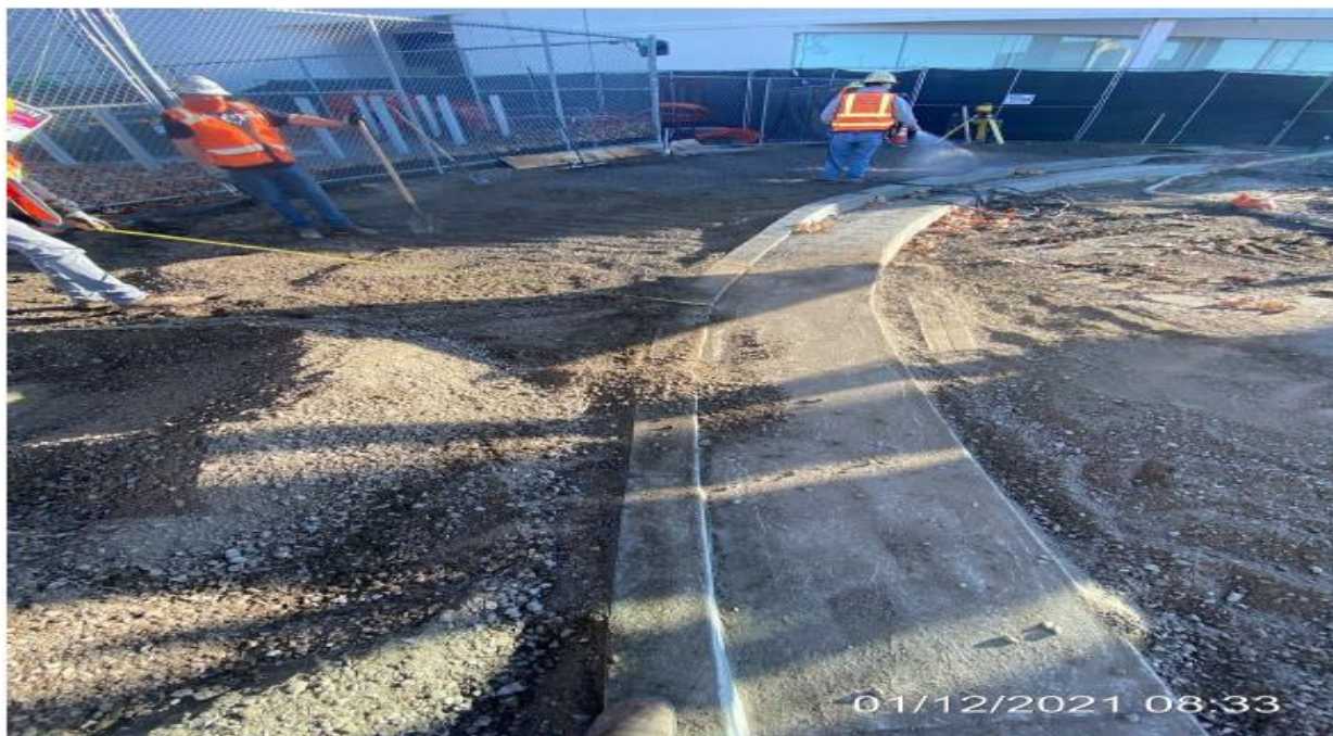
EXPO STATION– Continue excavating to final grade at the northbound sidewalk along the Bronson Cul-de-sac.
