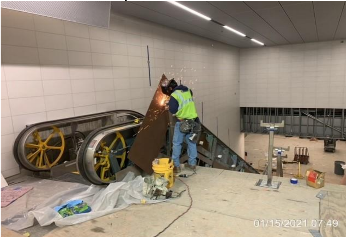
UG3 – McMahon Steel fabricating and welding center posts for stair #2.
