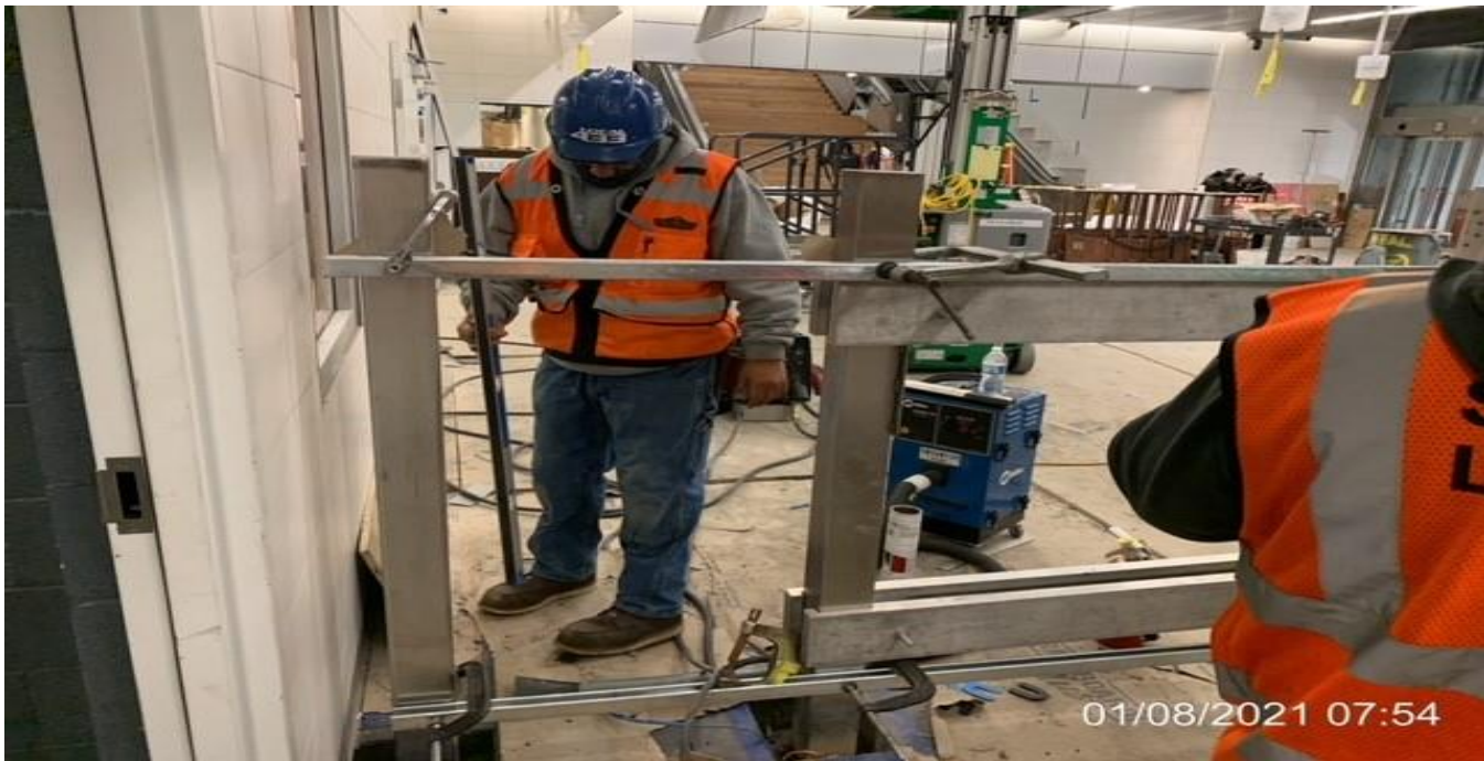
LEIMERT PARK STATION – Installing posts for the Fare Gate picket fence at the Paid & Free Area.
