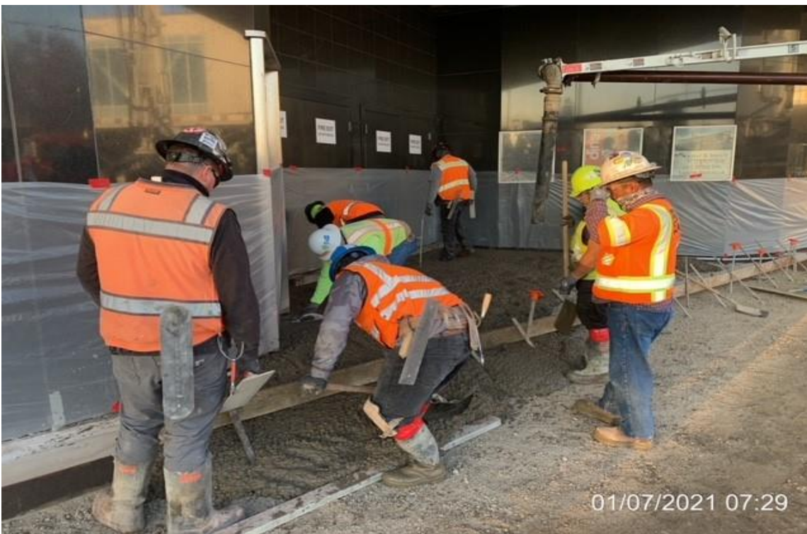
MLK STATION – Griffith placing concrete for mall entrance coves.
