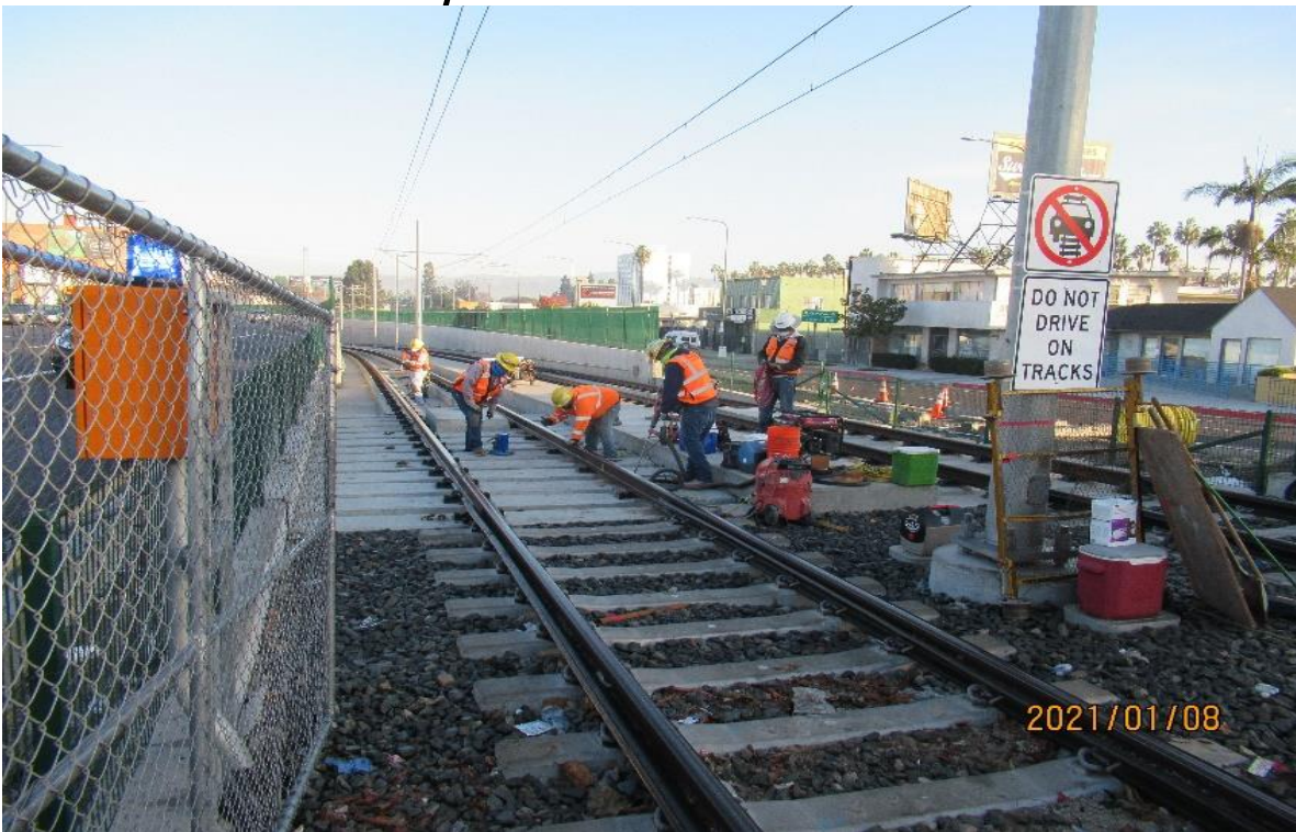
48 th Street – 48th Street SB track WSCC repair crew removing & demoing out loose DF fastener inserts STA 364+48 (looking northeast) Rework for NCR-129 revision-2
