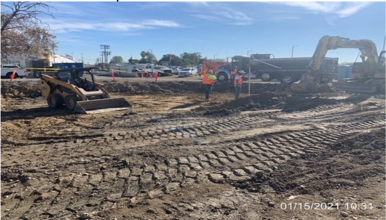
EXPO STATION – Continue rough grading and removing existing concrete on the east side of the Park & Ride lot area.
