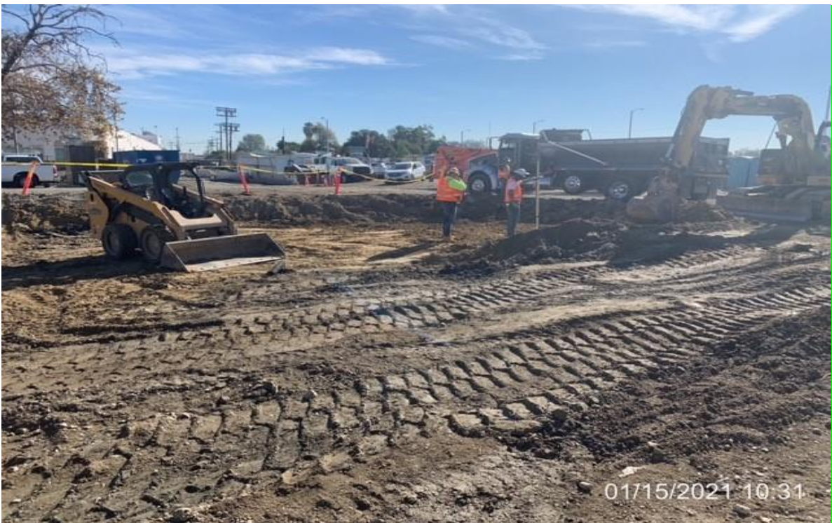
EXPO STATION – WSCC crew rough grading and removing with super 10.
