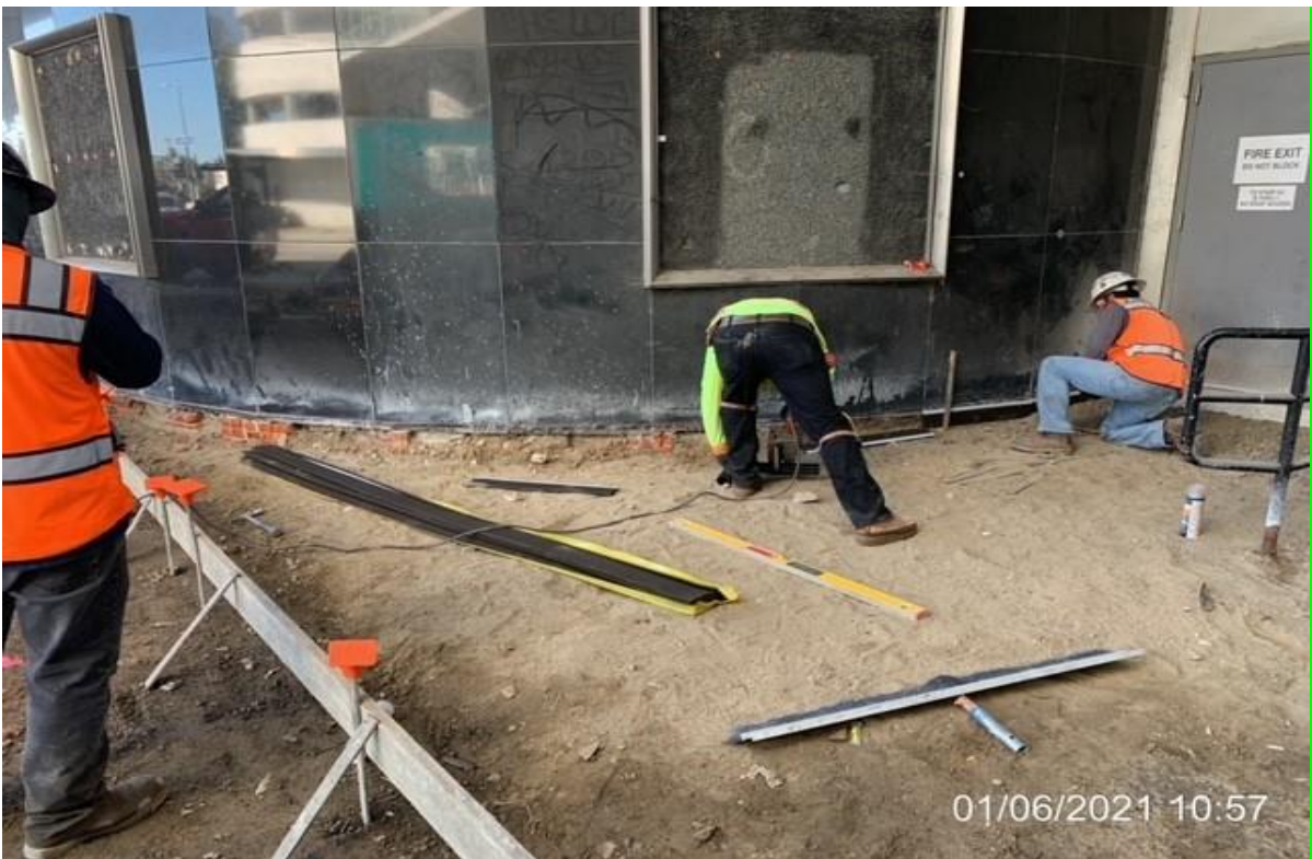
MLK STATION – Griffith installing expansion board prior to concrete slab placement.
