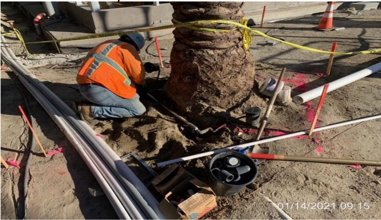
MLK STATION – Setting irrigation lines near tree wells at the plaza.
