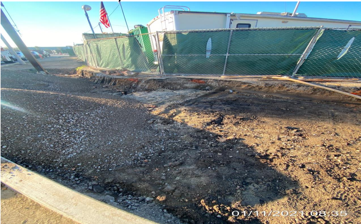
EXPO STATION– Continue excavating to final grade at the southbound sidewalk along the Bronson Cul-de-sac.
