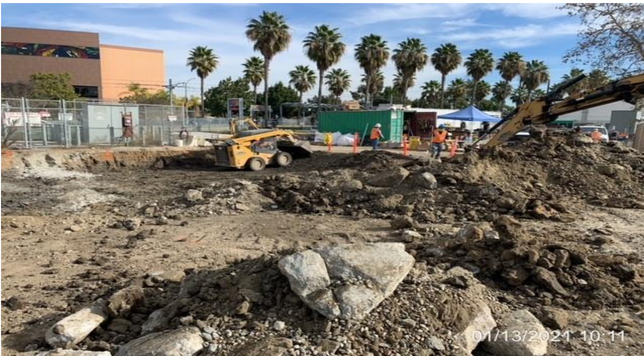
EXPO STATION SITE– Continue rough grading the northwest side of the Park & Ride lot area.
