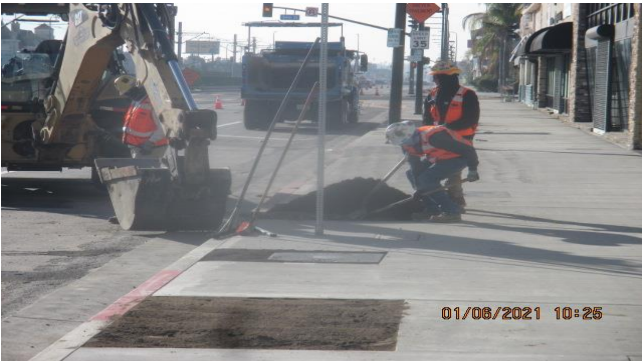
PARK MESA – Continue placing top soil to tree wells along southbound Crenshaw Blvd between 52nd St. and 54th St.
