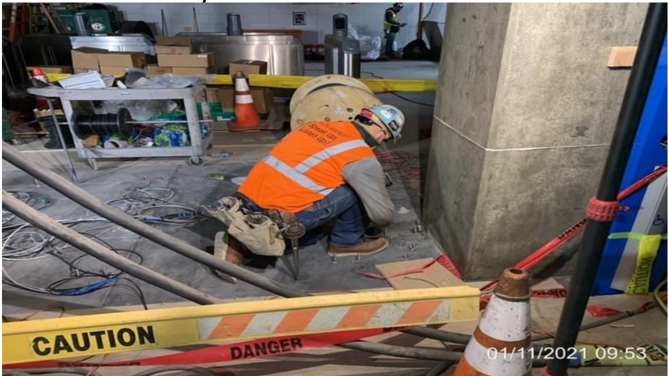
MLK STATION – Anchoring plates for Fare Gate System picket fence posts at the Paid & Free Area.
