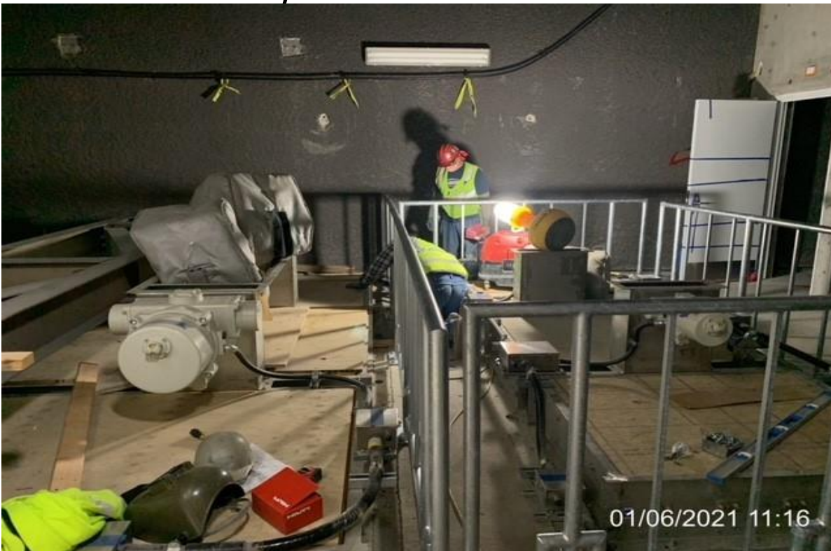
MLK STATION – McMahon installing guardrails around north EVF dampers.
