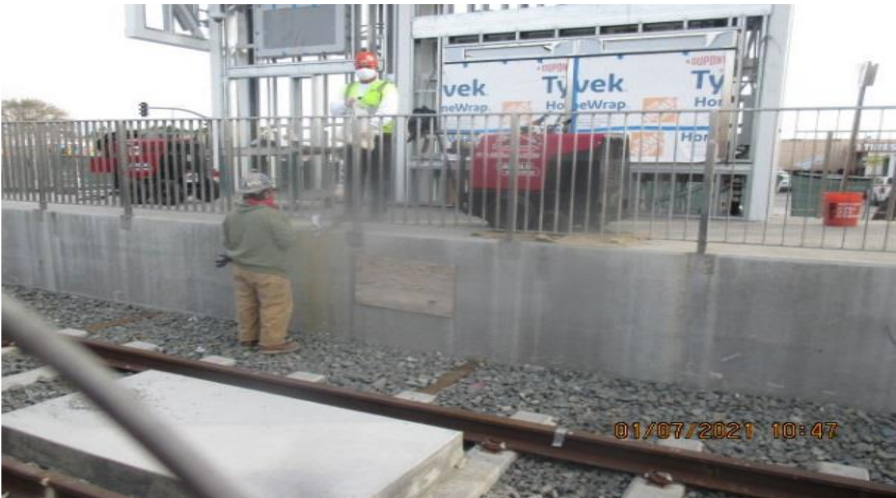
PARK MESA – Grinding and polishing handrail and guardrail finishes at the north entrance walkway ramp.
