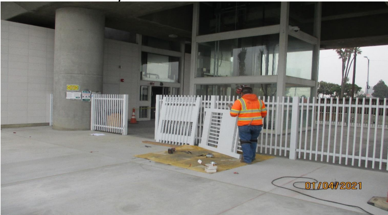
AVIATION/CENTURY - Welding fence gates at the Aviation Station.
