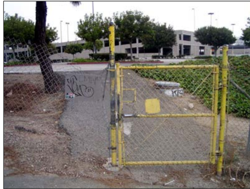
Looking at transit center from Rio Hondo Bike Path. Gate is locked.
