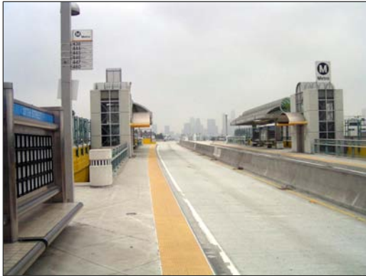
Harborway Transit Center at freeway grade
