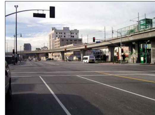
Alameda Street facing south across College Avenue
