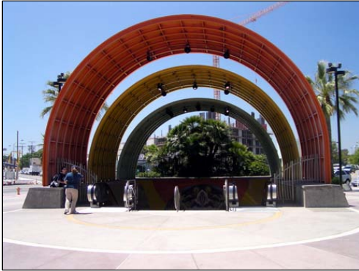
North Hollywood Metro Red Line station
