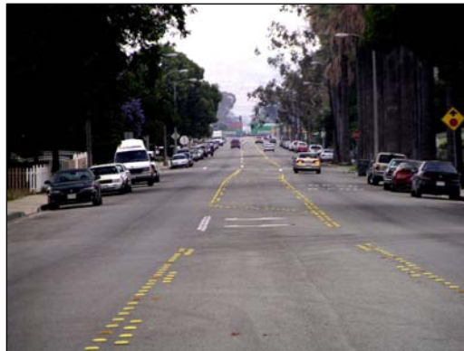
Alvarado Street and Park Avenue looking southbound
