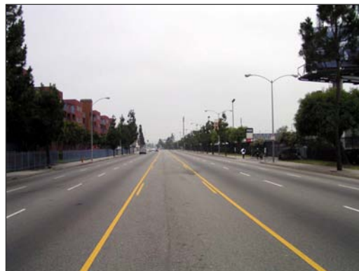
Martin Luther King Boulevard, facing west
