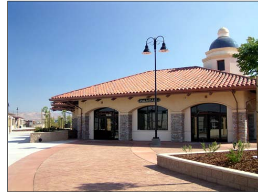
Palmdale Transportation Center
