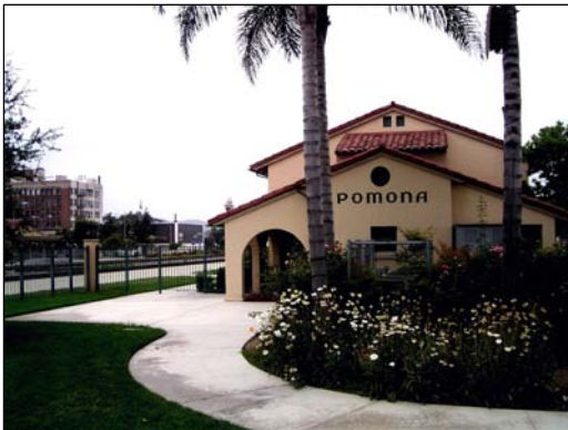
Pomona Metrolink Station
