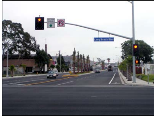
Spring Street at Long Beach Boulevard
