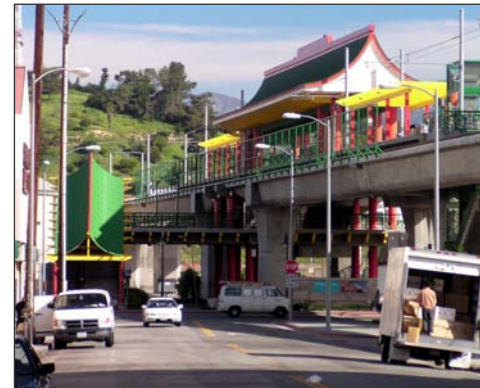
Spring Street facing north towards station
