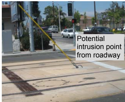
Figure 3 – Unprotected Guy Wire
