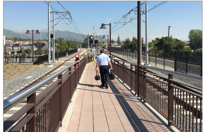
Convenient Paths At-Grade Stations are typically located near intersections for easy connections between street crossings and Station entrance pathways (Gold Line APU/Citrus College Station, Azusa)
