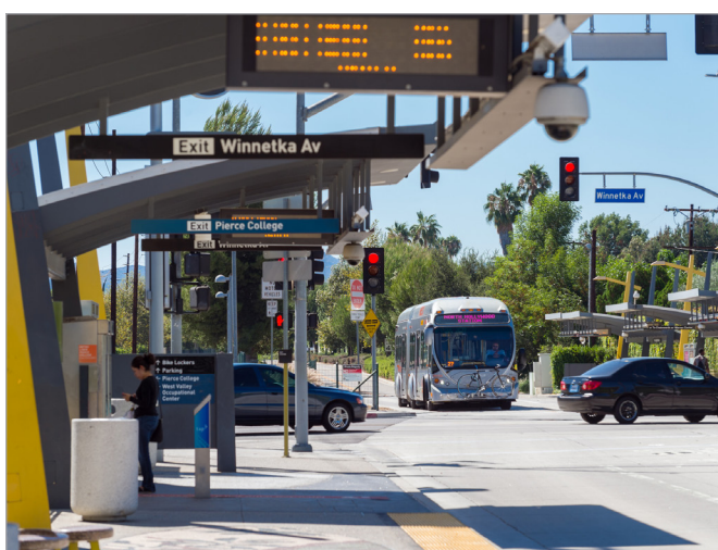
Design Design of paths and boarding areas should create a consistent rider experience (Orange Line Pierce College Station, San Fernando Valley)
