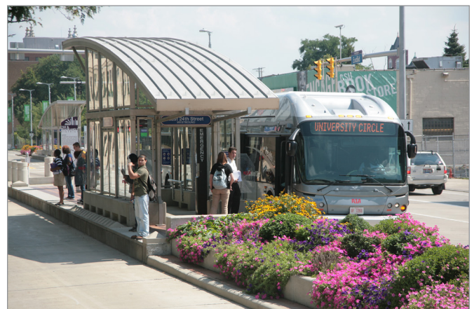
Median Station Stations may be located in the medians of streets, increasing the number of street crossings customers must cross between transfer points (Regional Transit Authority, Cleveland)
