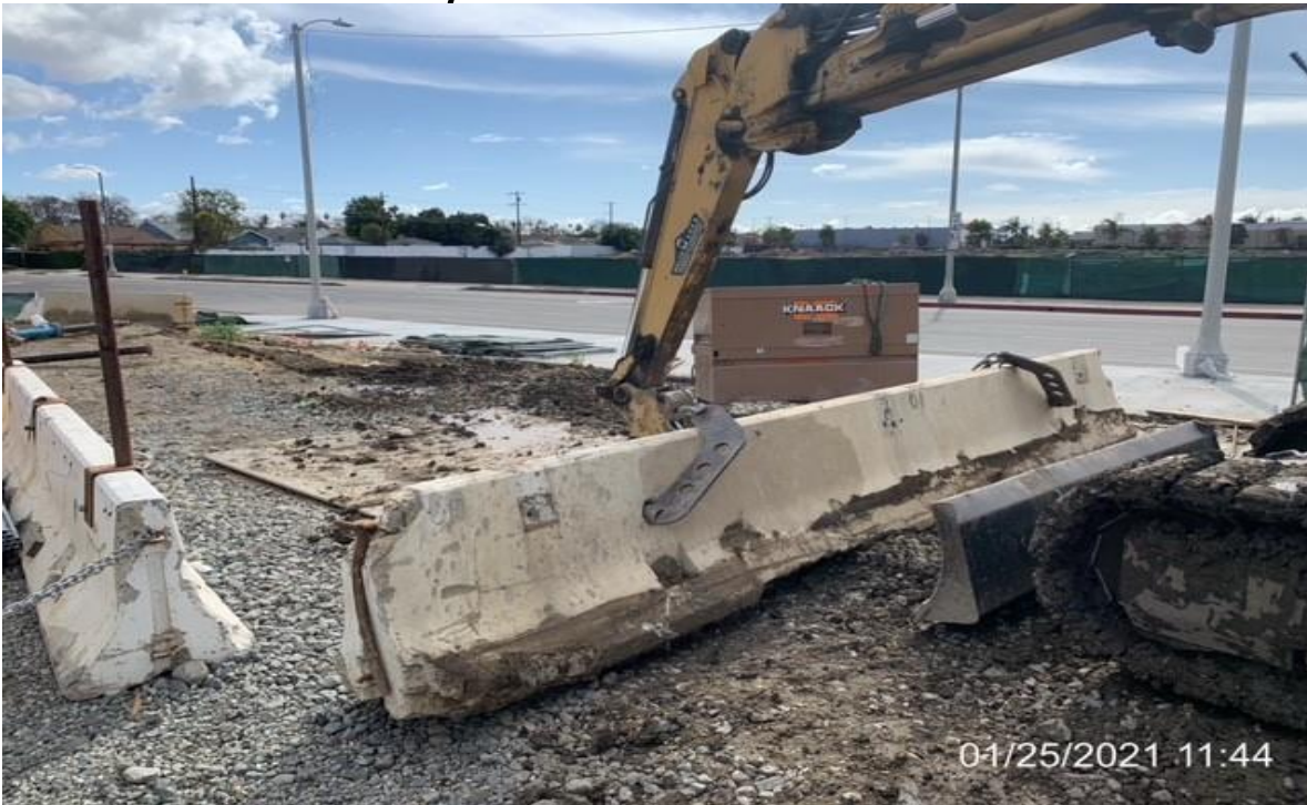
MLK STATION – WSCC crew replacing K rail with temporary fencing.
