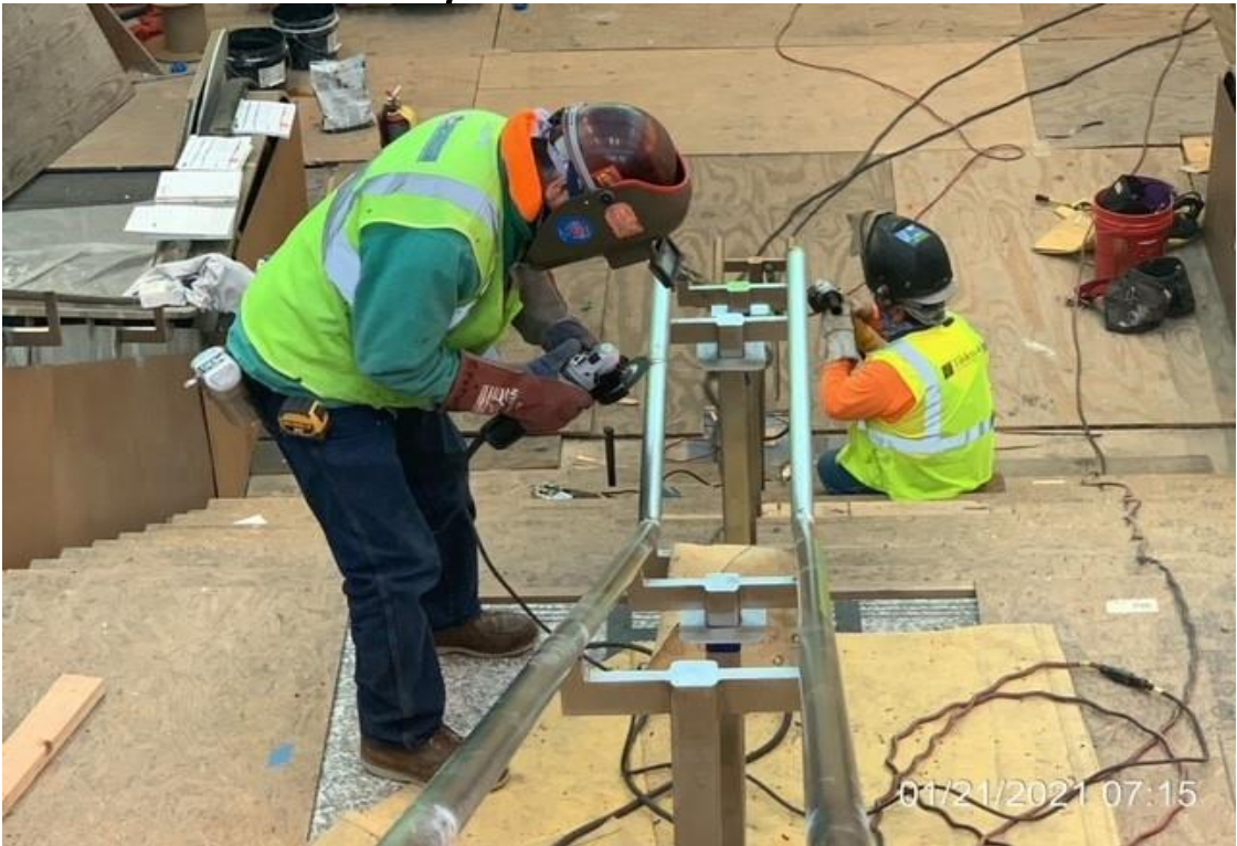
UG4 – McMahon grinding to finish handrail at stair #2
