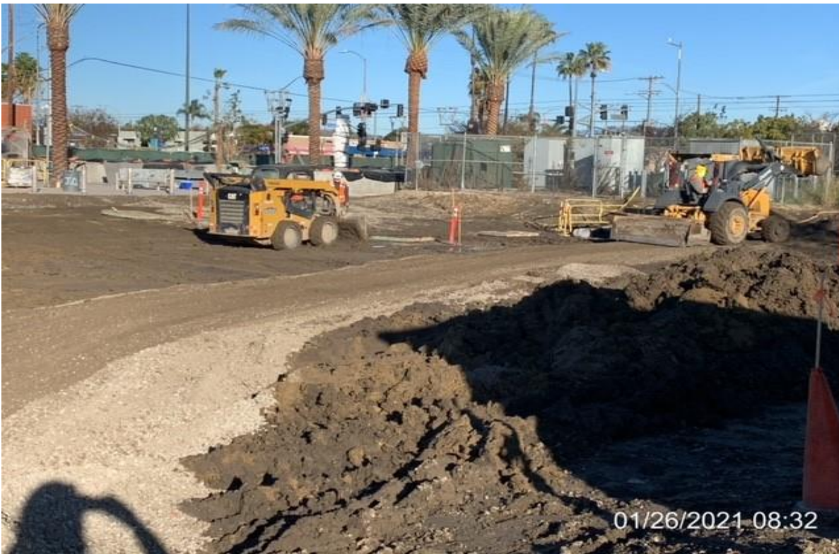
MLK STATION – WSCC crew distributing base and gravel in preparation for rainfall
