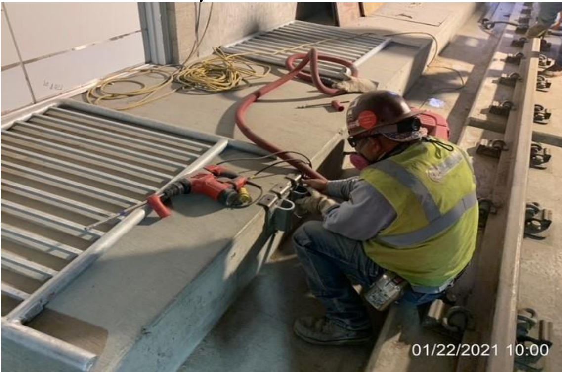
MLK STATION – WSCC crew scanning ceiling for seismic bracing anchors.
