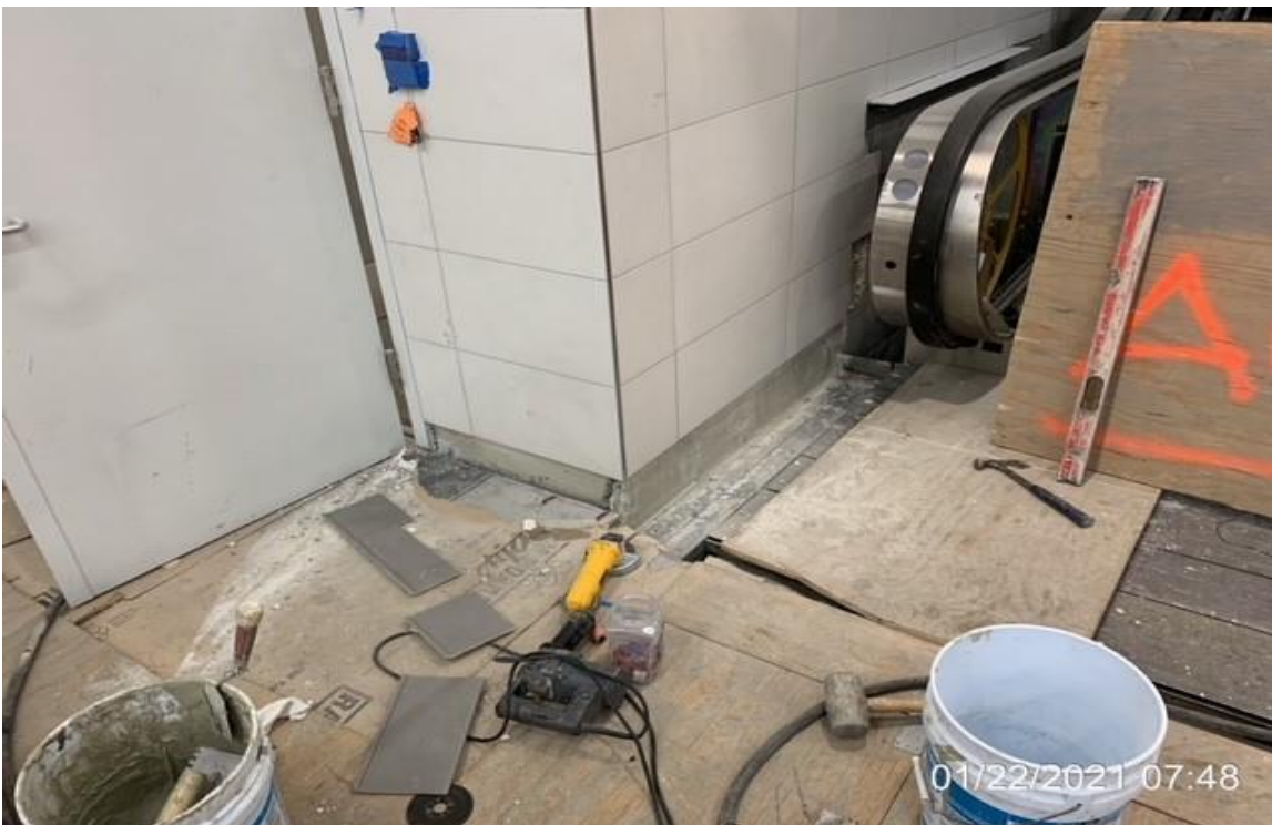
UG4 – Premier Tile & Marble installing base cove at concourse.
