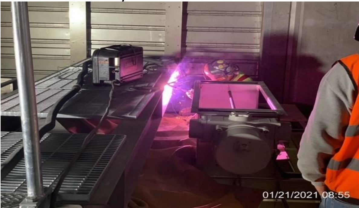
MLK STATION – WSCC ironworkers welding stiffener plates for cat walk.
