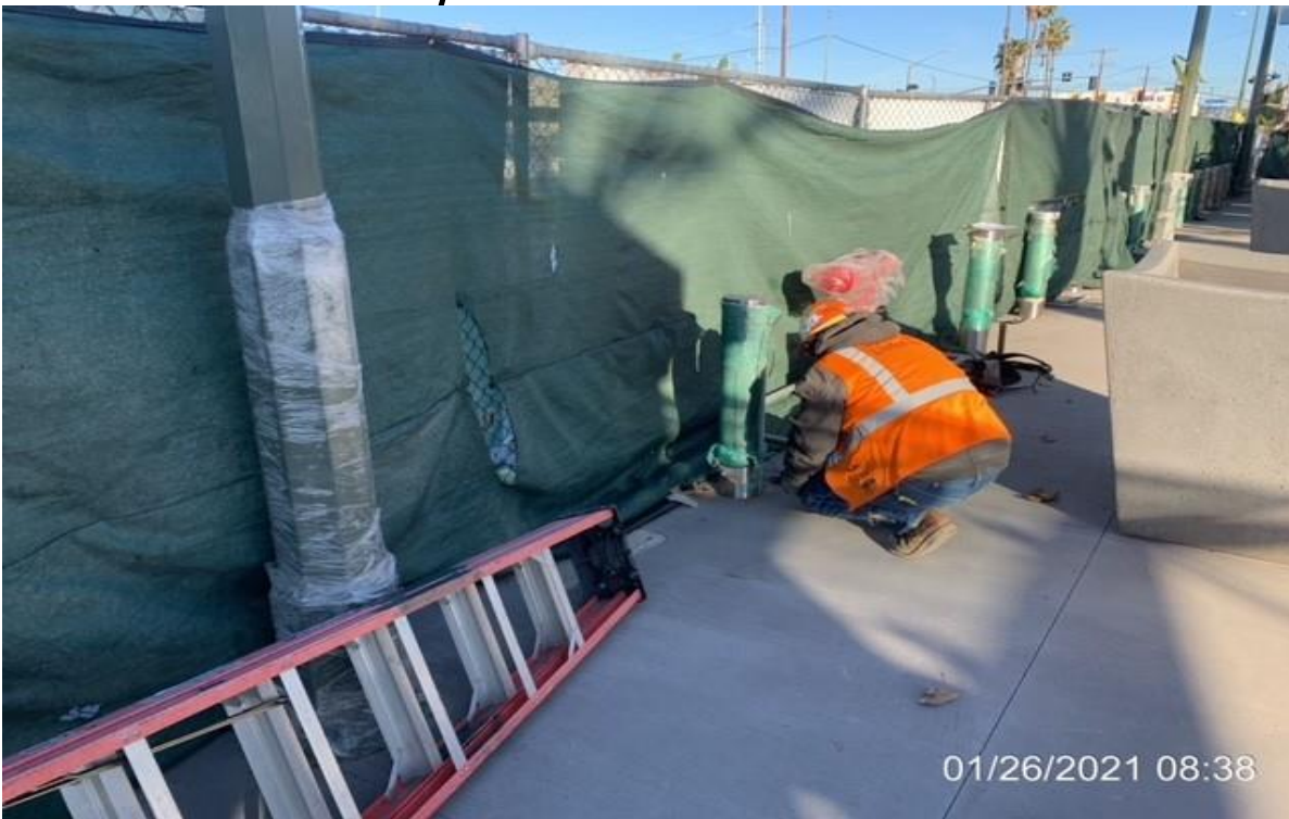
MLK STATION – WSCC ironworkers drilling holes into ballasts for ground wire.
