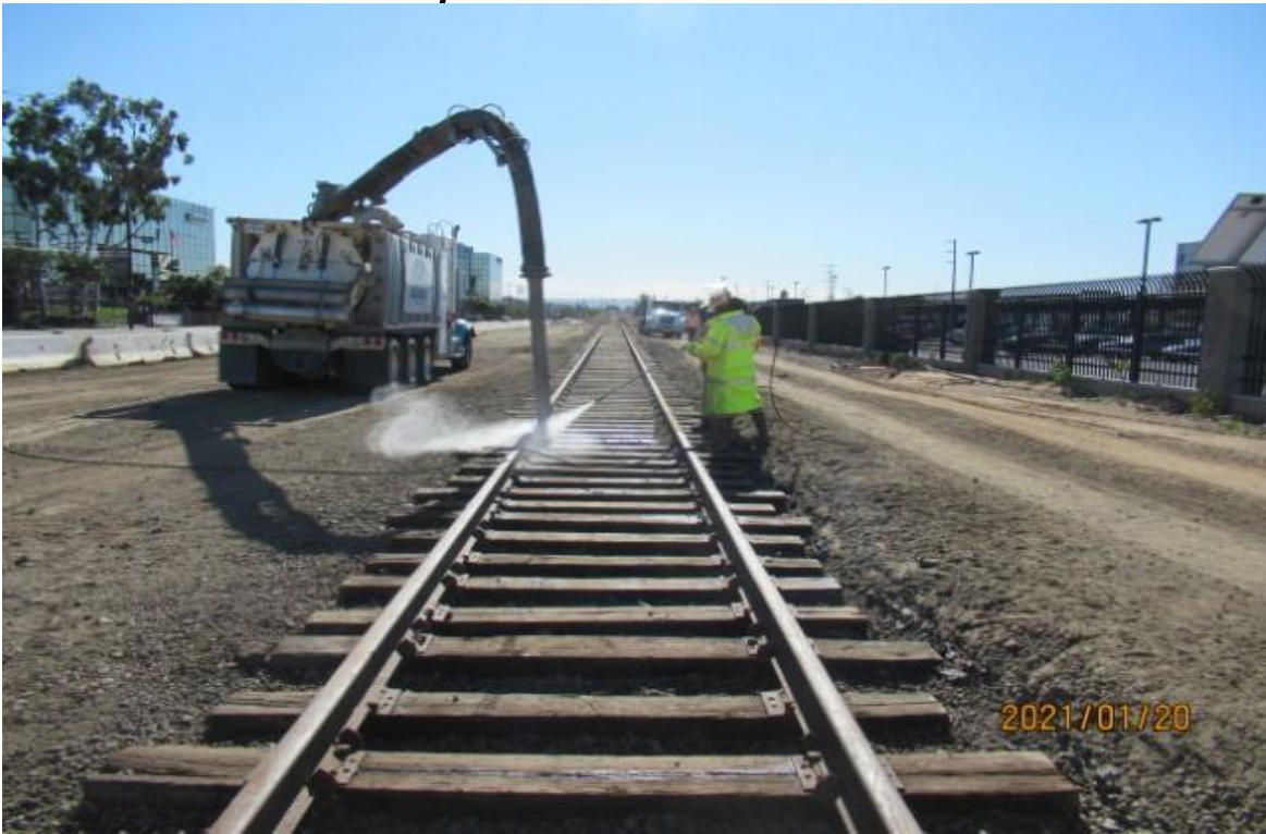
124 th - WSCC Sub-contractor Badger Day lighting using vacuum truck & hi pressure water to remove contaminated ballast on BNSF track near 124th Street outside of CLAX project limits (looking south)
