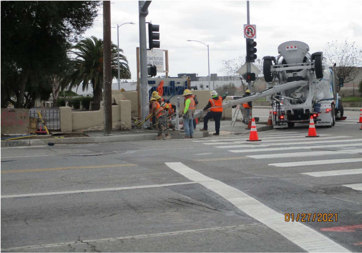
AVIATION/CENTURY- Placing sidewalk concrete at Aviation and 111th.
