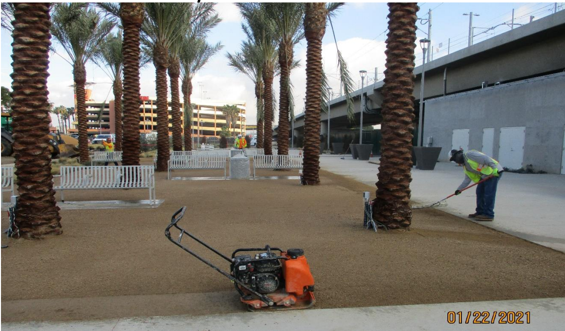
AVIATION/CENTURY - Placing decomposed granite at the Aviation Station plaza.
