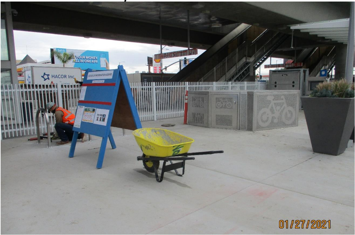
AVIATION/CENTURY- Bike rack installation at the Aviation Station plaza.
