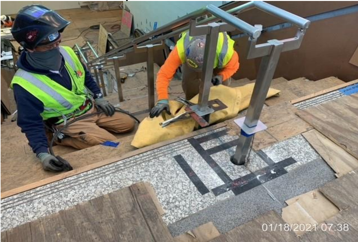
UG4 – McMahon Steel fabricating and welding post cover plates for stair #1.
