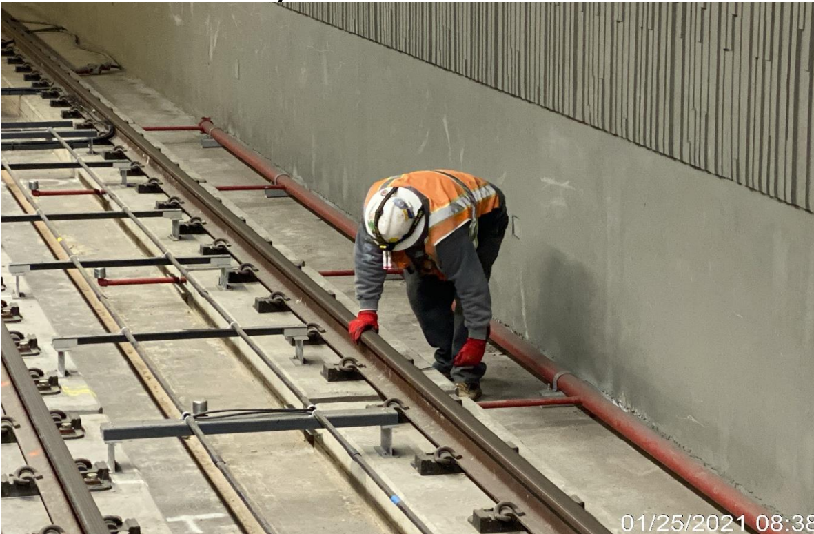
UG4 – RMA checking track fastener gaps at UG-4.
