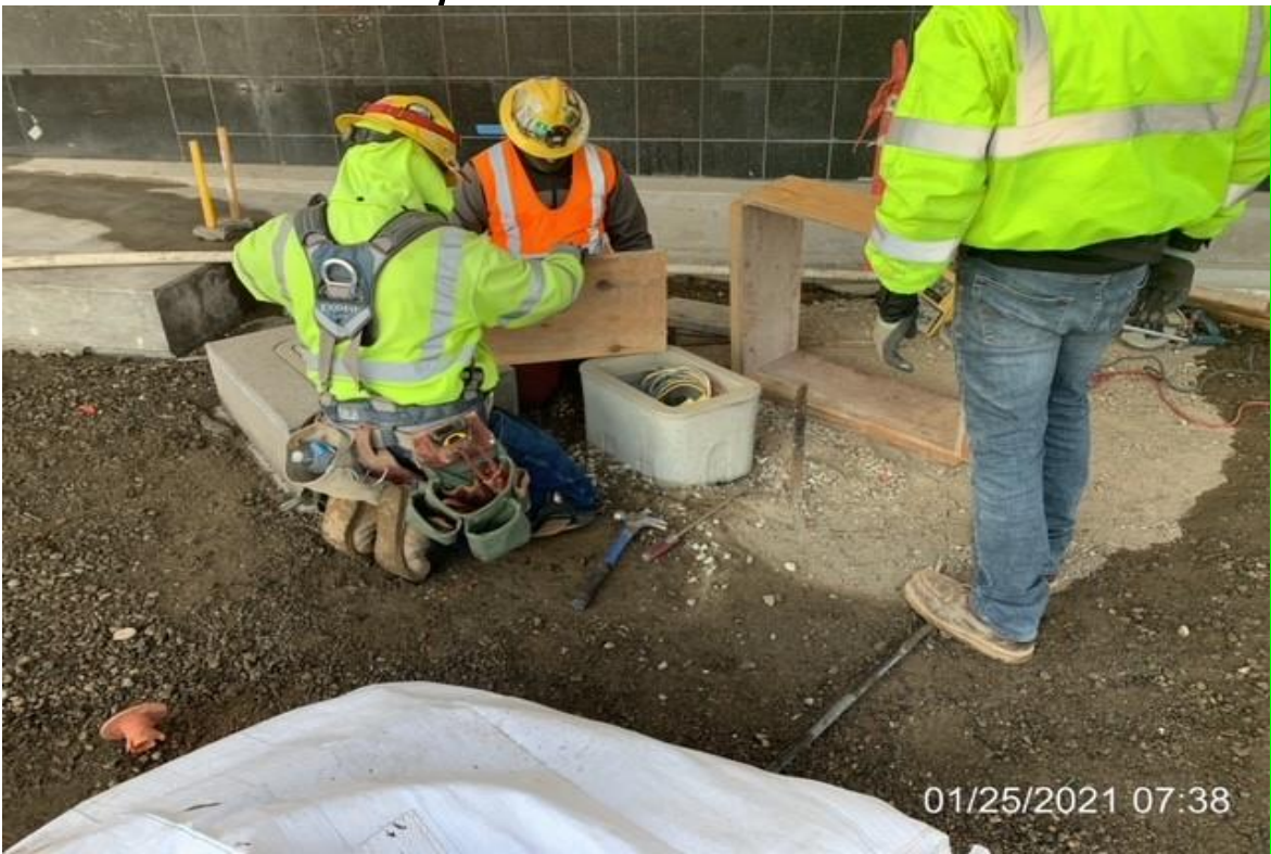
MLK STATION – WSCC carpenters building formwork for pull boxes.
