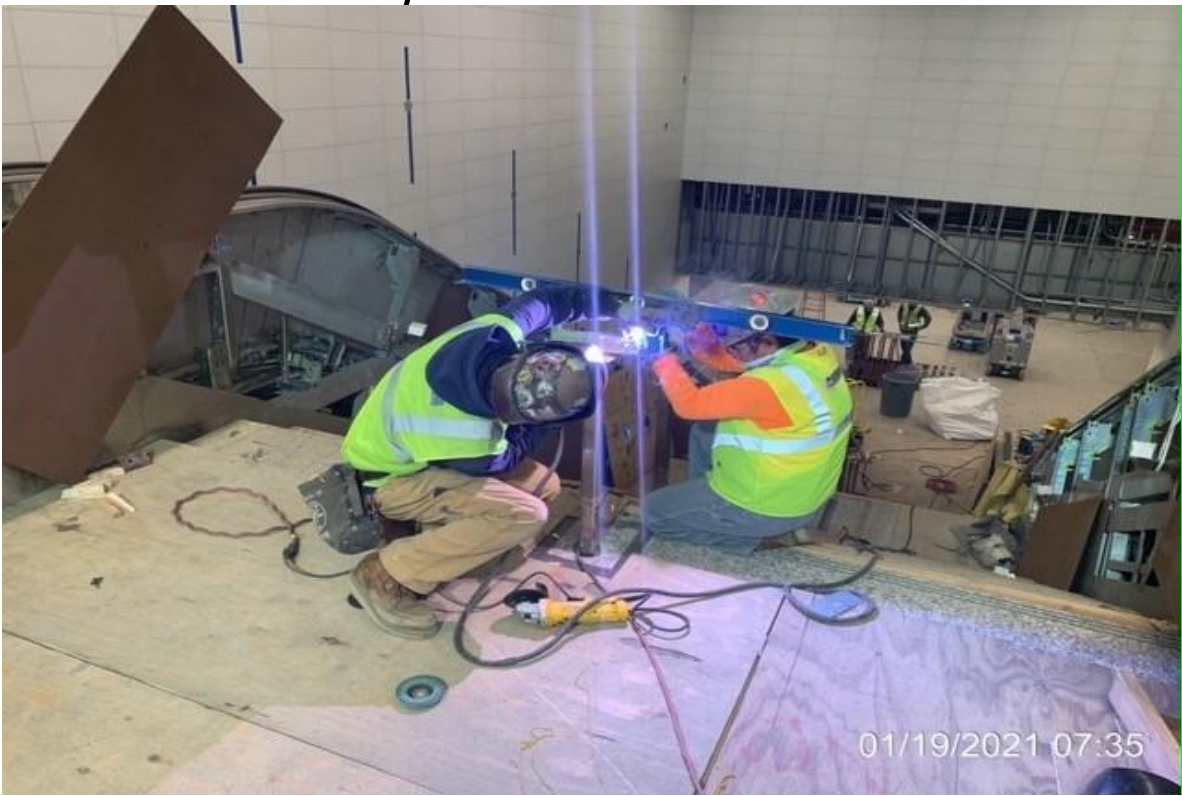
UG4 – McMahon Steel tack welding handrail to center posts at stair #2.
