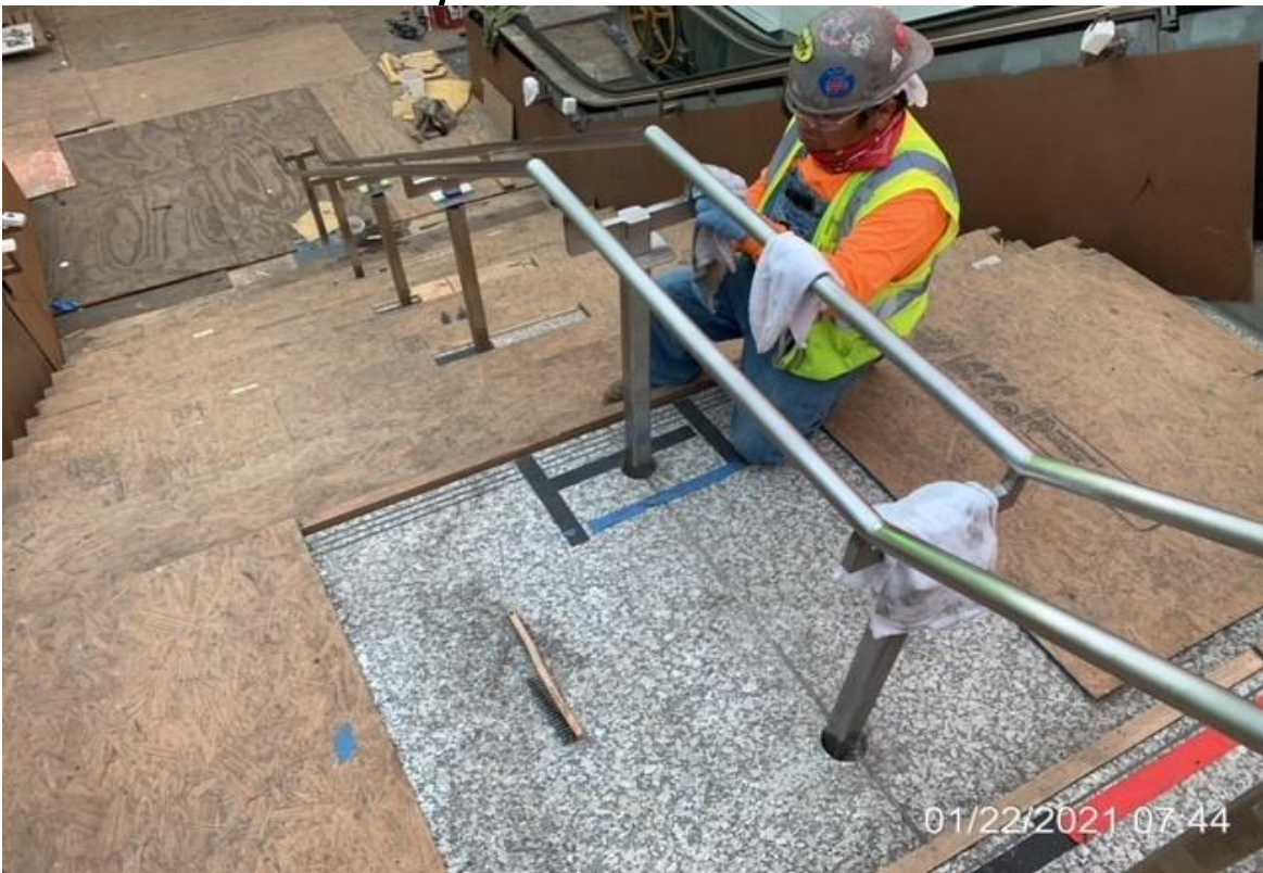
UG4 – McMahon polishing handrail at stair #1 and #2.
