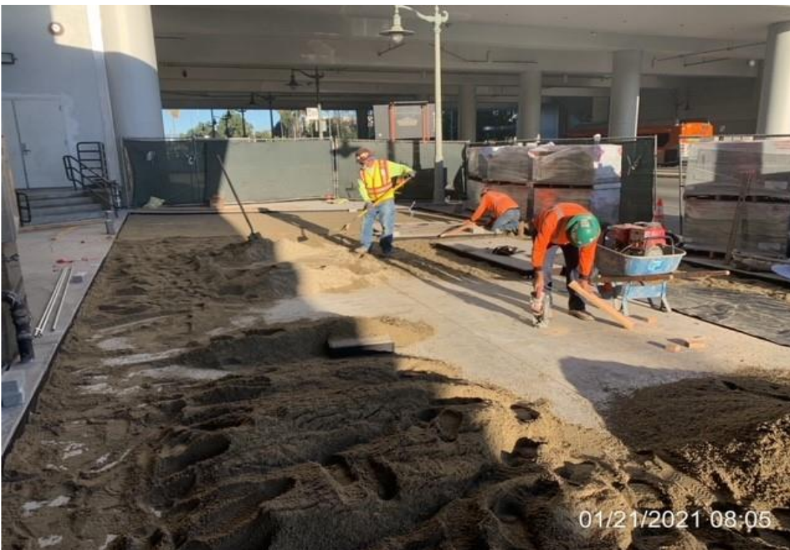
MLK STATION – Grandstorm Masonry laying bedding sand for pavers.
