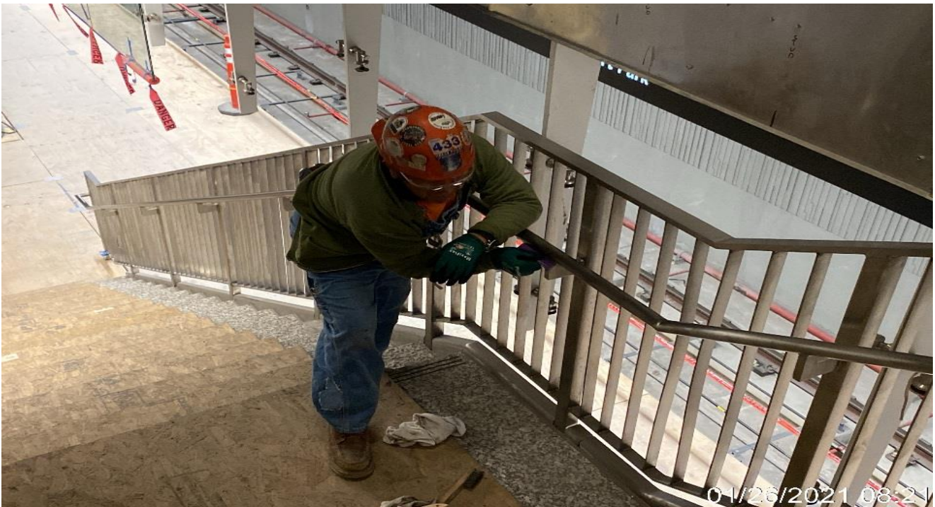
LEIMERT PARK STATION – Polishing handrails for Staircases 3&4 from concourse to platform.
