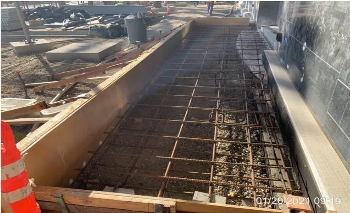
MLK STATION – IRP installing #5 rebar for pedestrian entrance ADA ramp.
