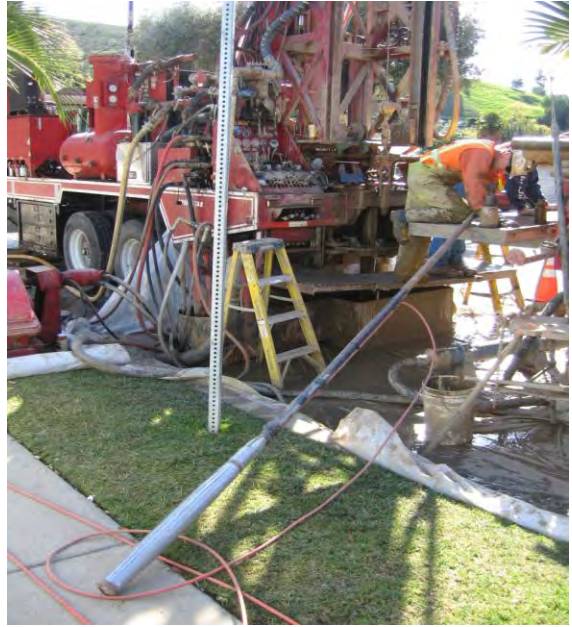
Figure 3-2. Pressuremeter set up at Boring Location R-09-Z1B5.
