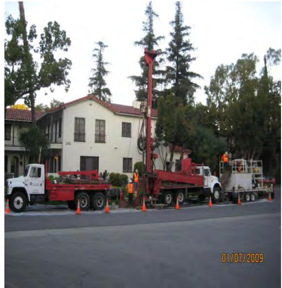
Figure 3-1. Drilling Operation at Boring Location R-09-Z3B12.
