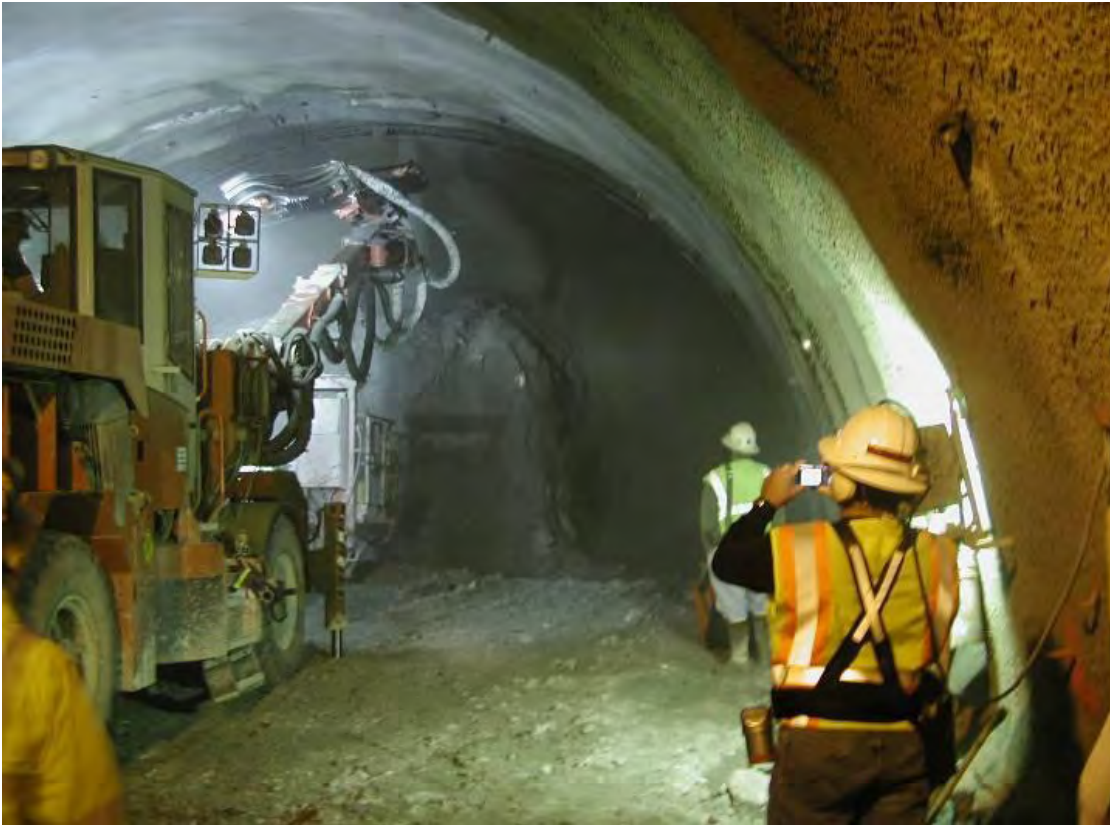
Figure 12-7. Shotcreting in the Devil's Slide Tunnel.
