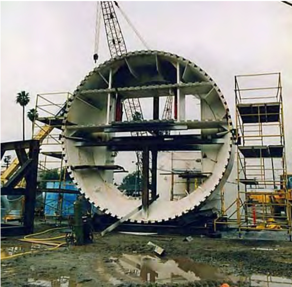
Figure 12-4. Digger Shield used in Los Angeles Metro Red Line Tunnel.
