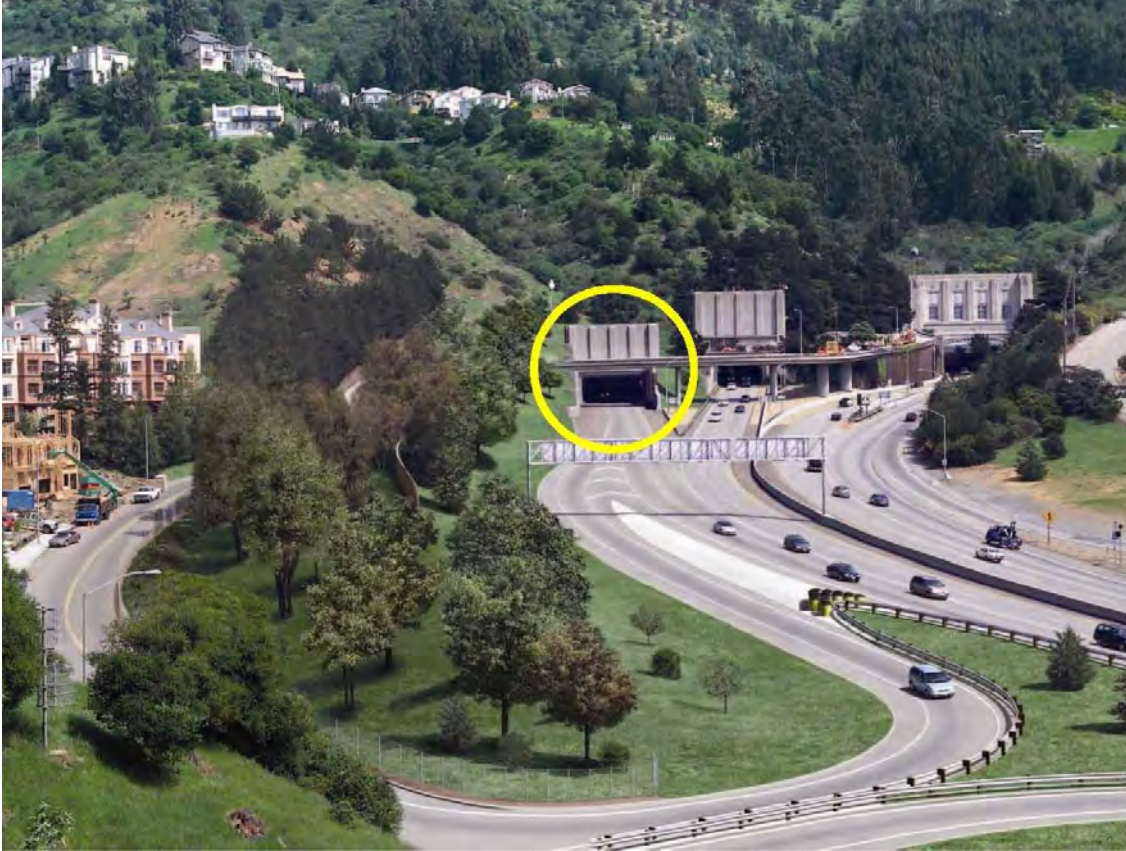
Figure 12-6. The Caldecott Fourth Bore Tunnel portal showing the existing tunnels and simulation of the proposed tunnel (highlighted with yellow circle).
