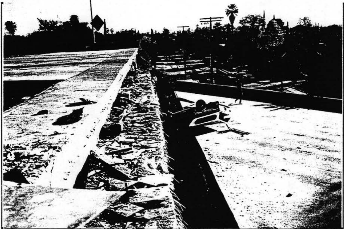
Mission Gothic Abutment 5R. looking south.
