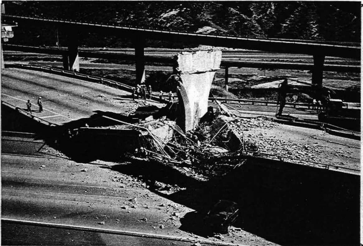
14/5 Conn. Sep. & OH 53-1960F 7-LA-14/5-R14.73/R45.62 3-36-JSM Pier #3 from above, looking East
