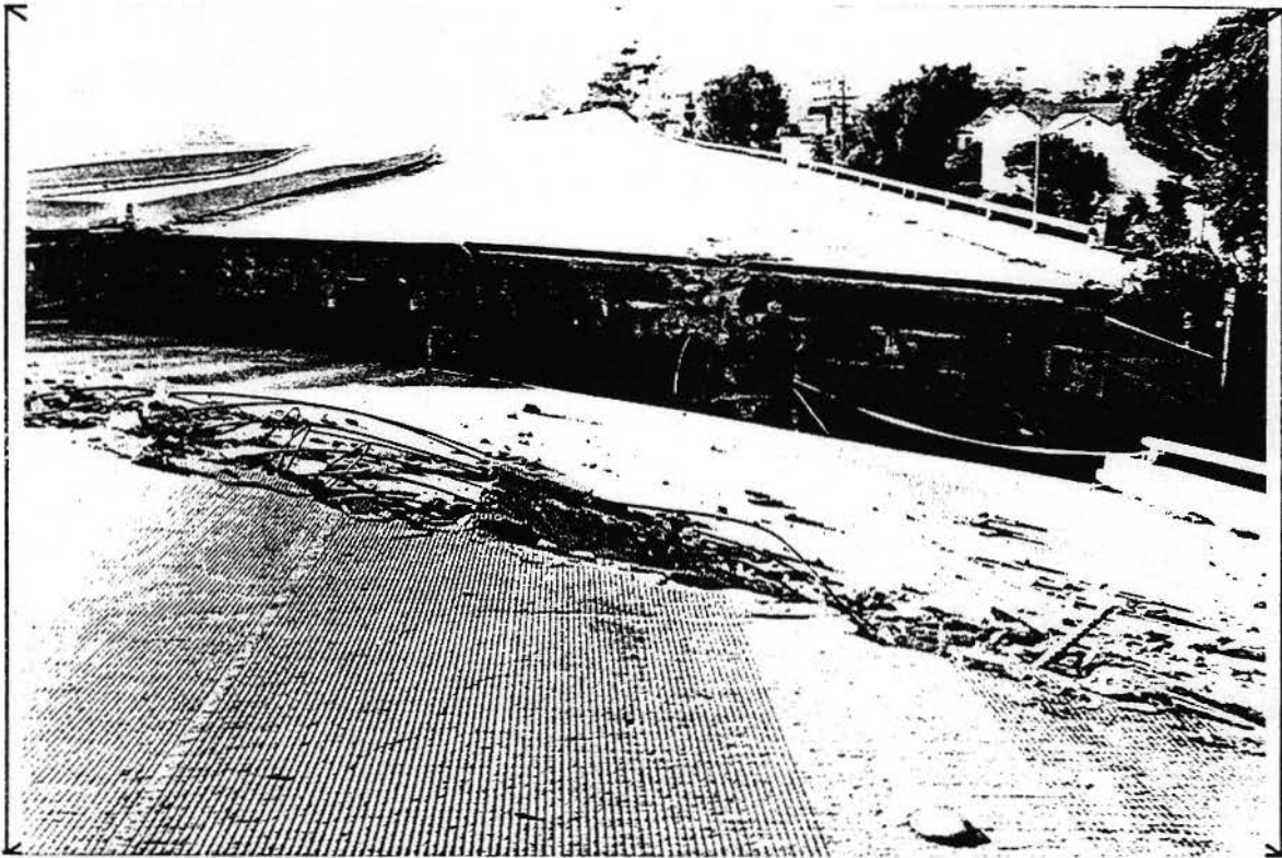
La Cienega-Venice U.C. 53-1609 7-LA-10-R8.83 C-31-BKT Span 6 Collapse at Hinge. WB Struc., Looking West.
