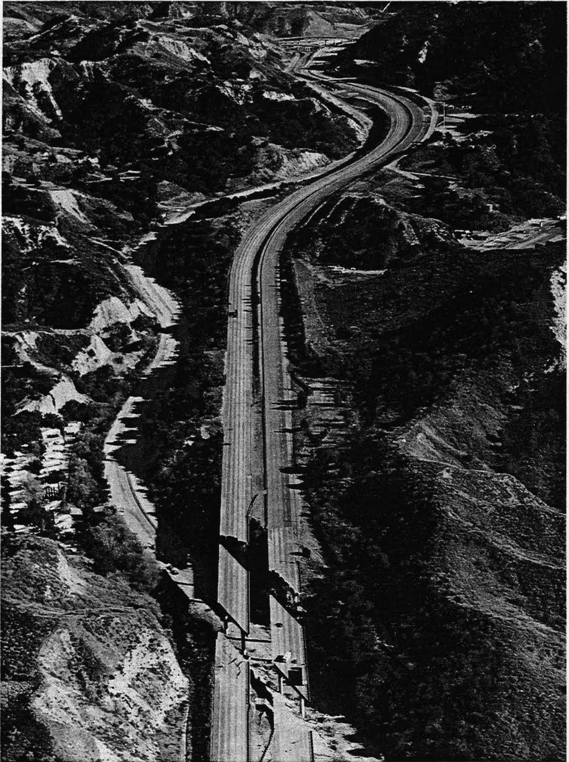
Overview of Gavin Canyon Road (53-1797R/L), with Route 14/Interstate 5 Interchange in distance.
