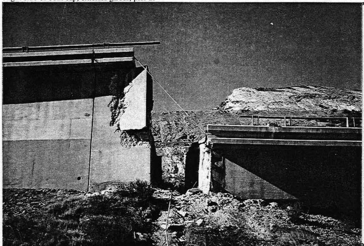
14/5 Conn. Sep. & OH Abutment #1.
