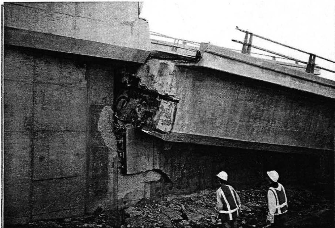
North Conn. OC Abutment #1
