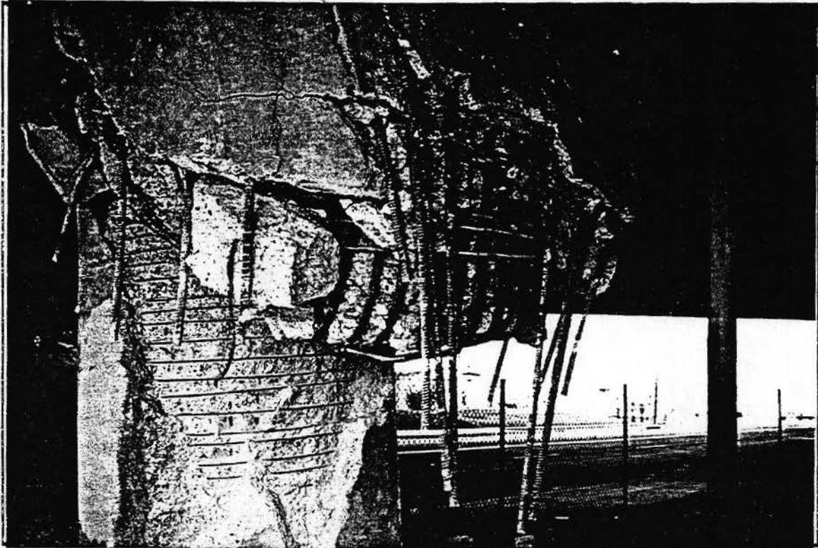
Mission Gothic 53-2205 7-LA-118-R8.63 9-3-TES Bent 2R, left column, looking north.
