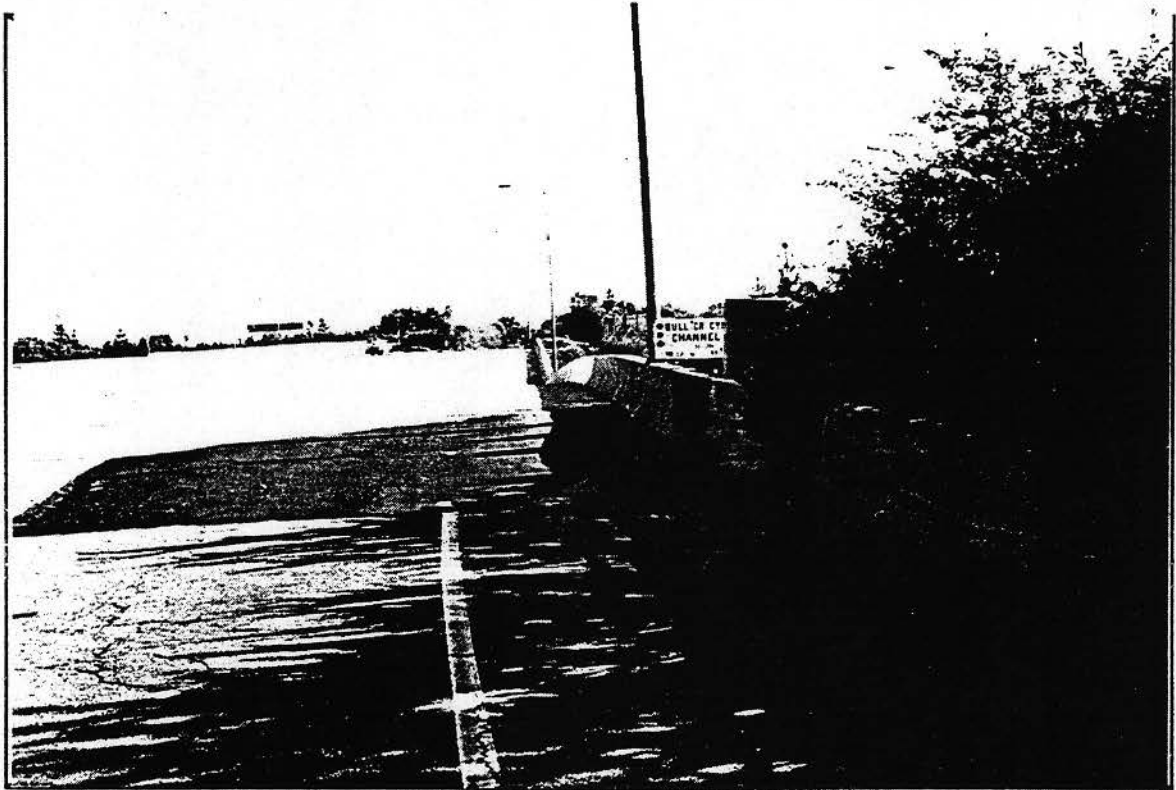
Bull Creek Canyon Channel 53-2206 7-LA-118-R8.84 14-1-TES Abutment 1, southside, looking east.
