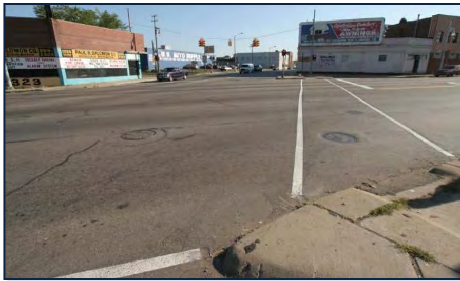
Long crossing distance can be especially challenging for bicyclists and pedestrians.
