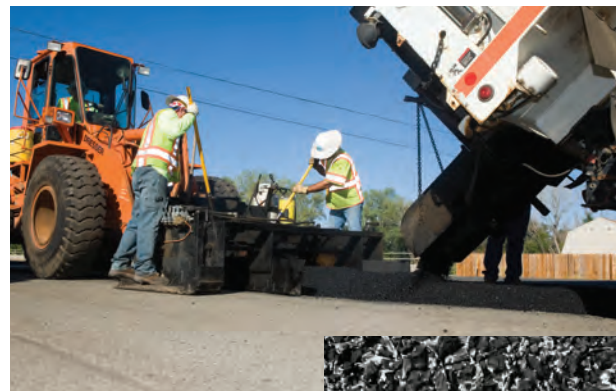
Above: Caltrans workers laying down rubberized hot-mix asphalt. Right: Closeup of shredded recycled tires used in RHMA.
