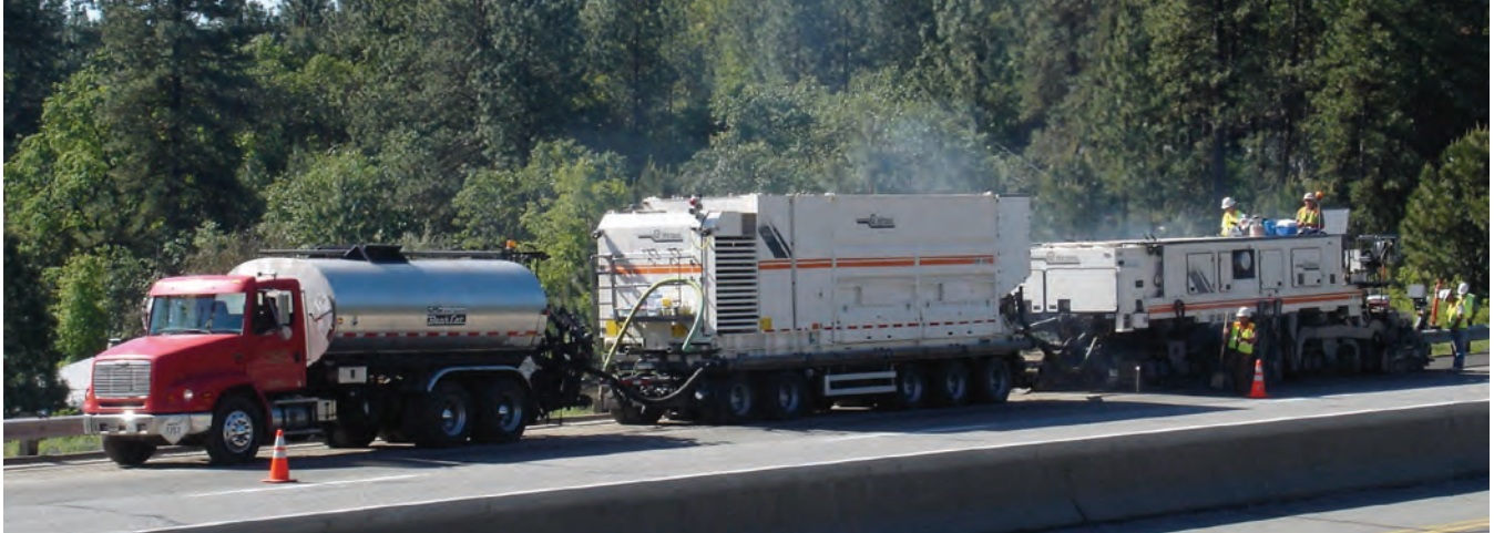
Cold-in-place recycling train.
