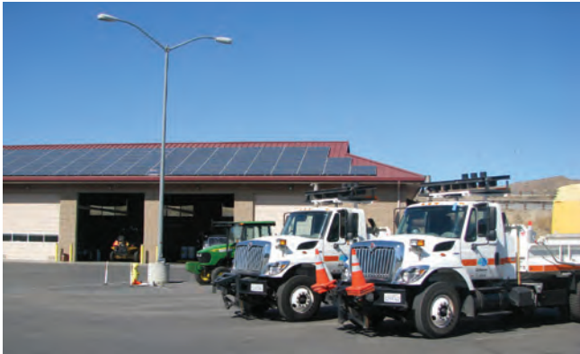
Solar panels at a maintenance facility in District 7.
