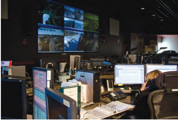
Operations at a Caltrans Traffic Management Center.
