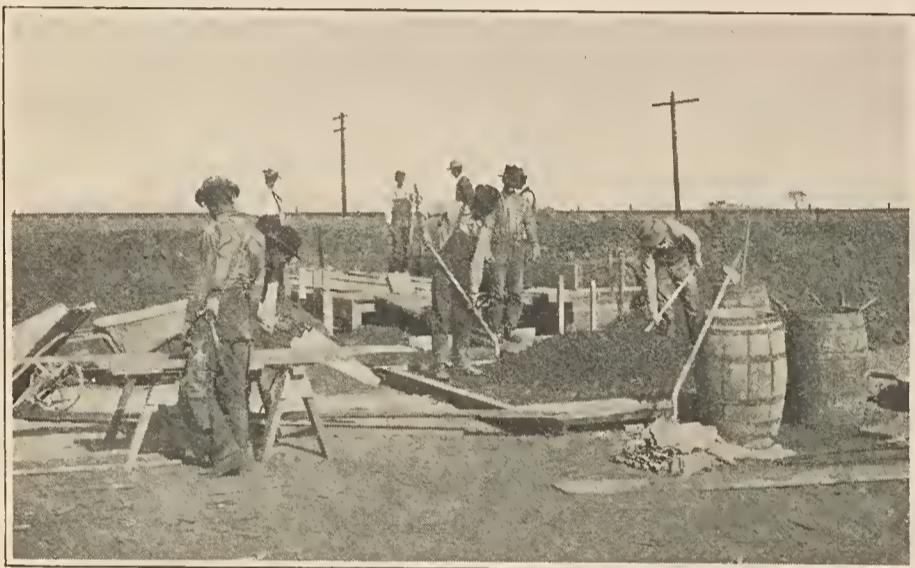
Making Reinforced Concrete Culvert on State Highway Near Marysville.
