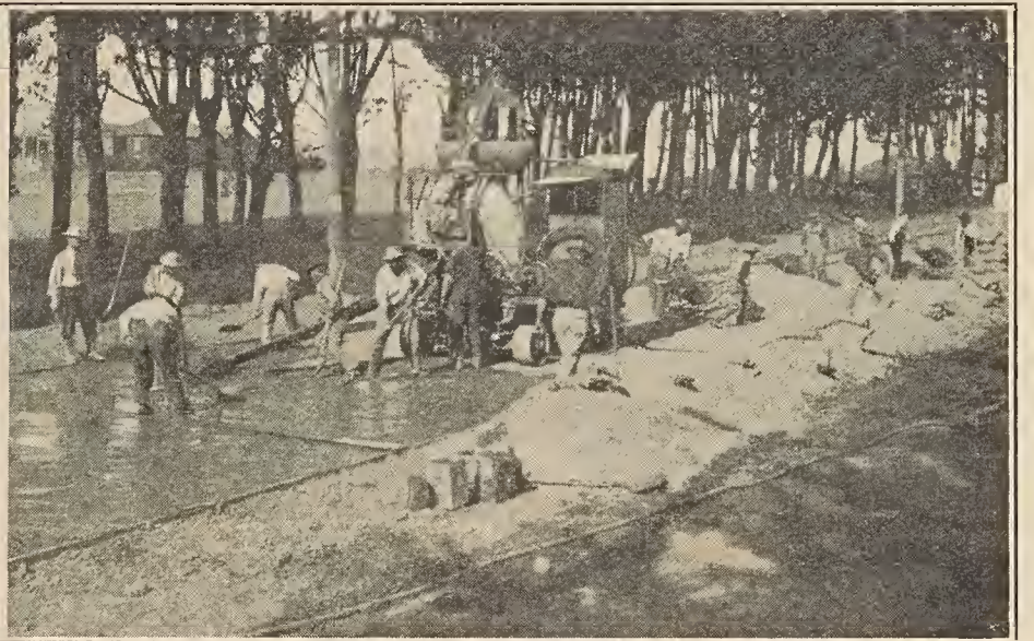
Work on the State Highway Near Burlingame, San Mateo County.
