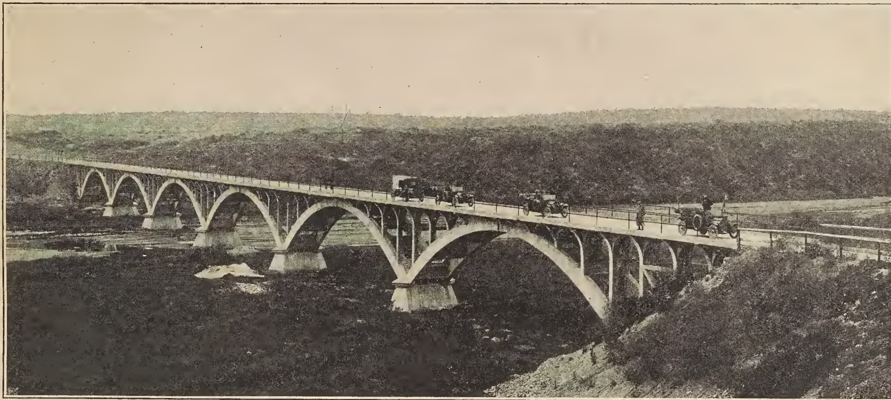
Reinforced Concrete Bridge Over San Luis Rey River. Length, 690 Feet. Built by San Diego County Highway Commission. On Route of State Highway.
