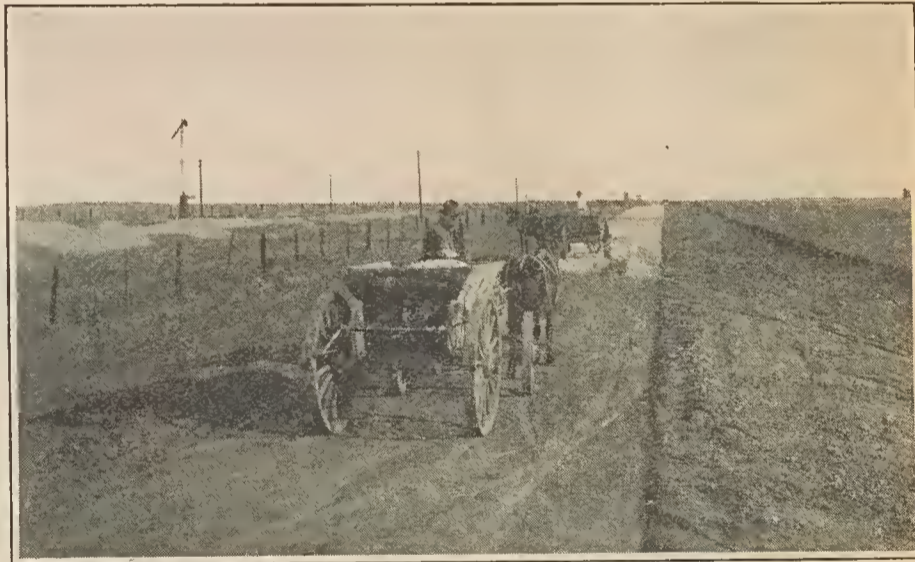
Building the State Highway Near Marysville.
