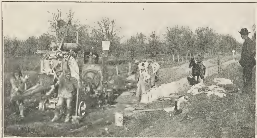
Concrete Mixer, State Highway, near Roseville.
