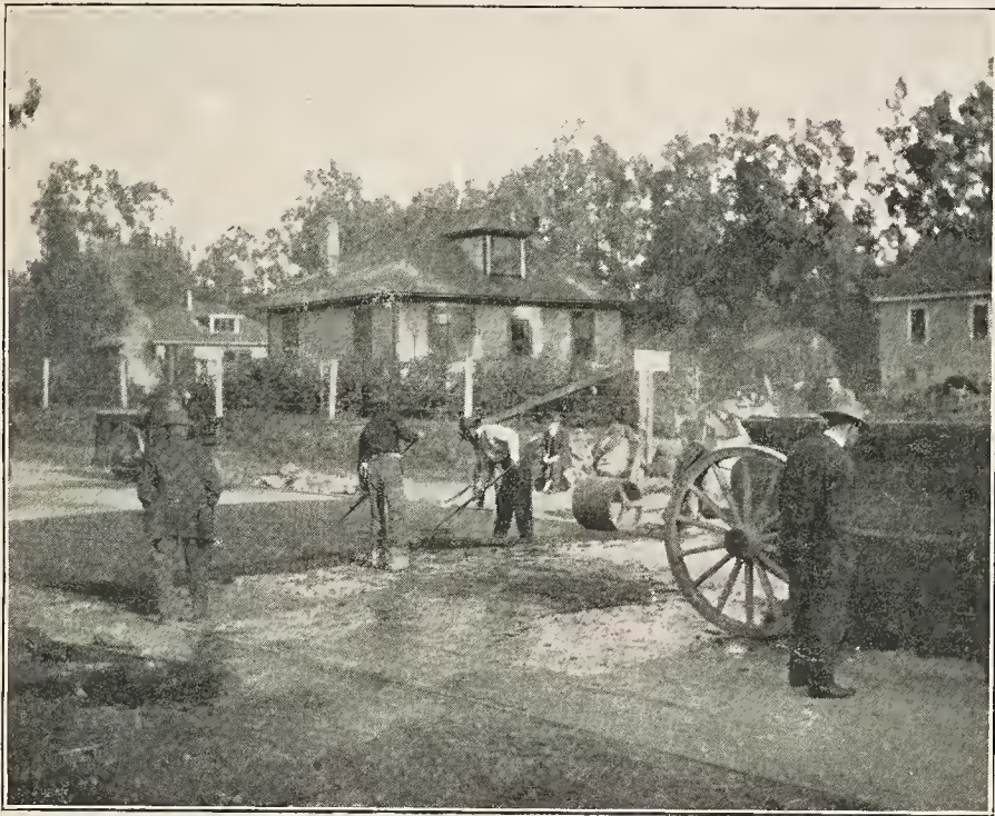
Raking Asphalt Surface, State Highway, San Mateo County.
