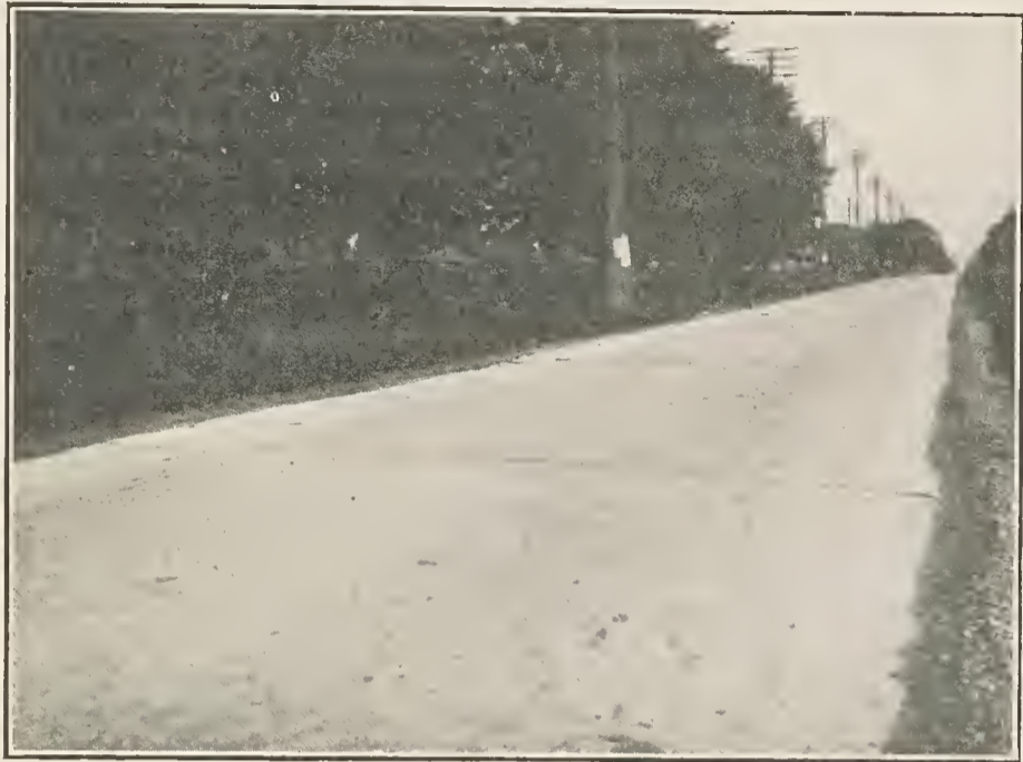
Concrete Road, Armored Joints, No Wearing Surface, Wayne County, Mich.
