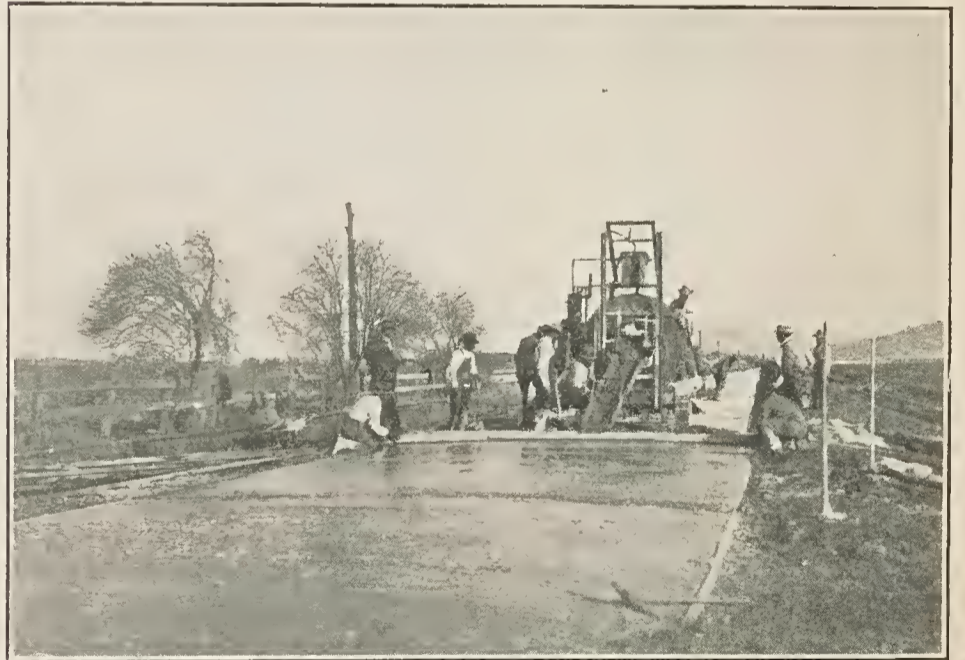
Placing Concrete Base, State Highway, Los Angeles County.
