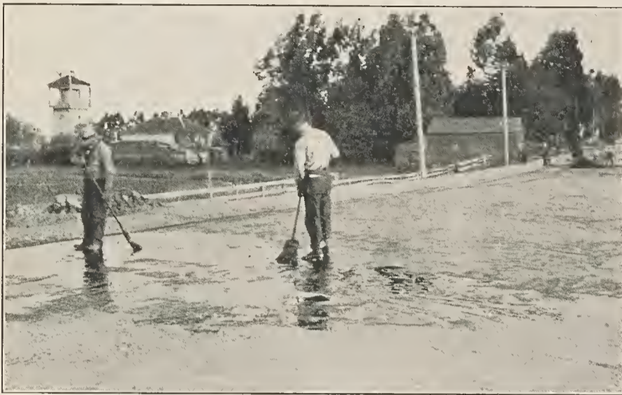
Spreading Asphalt Paint Coat, State Highway, San Mateo County.
