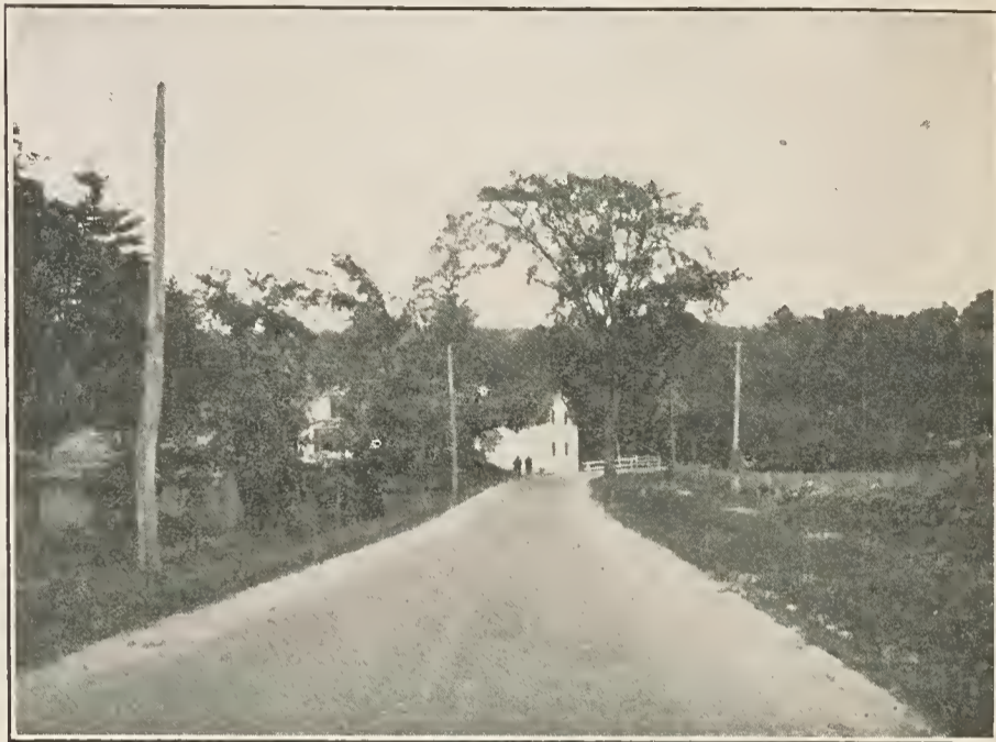
Concrete Road, Thin Bituminous Top, State Highway, Spencer, Mass.
