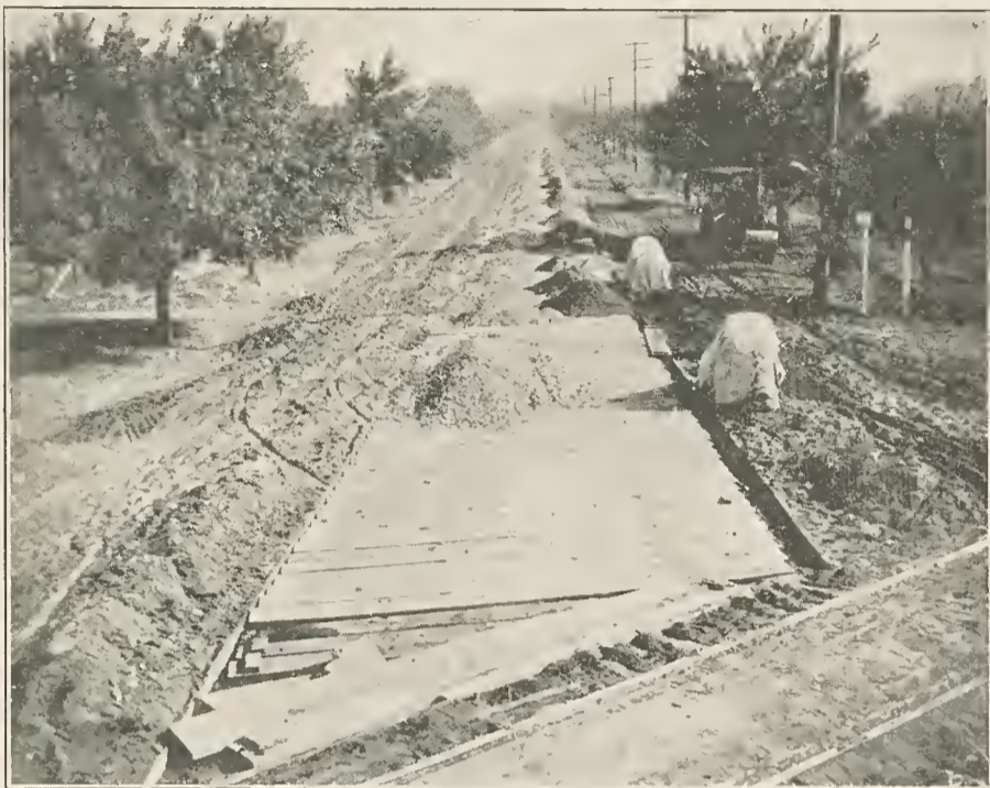
Ready for Concrete, State Highway, near Fresno.
