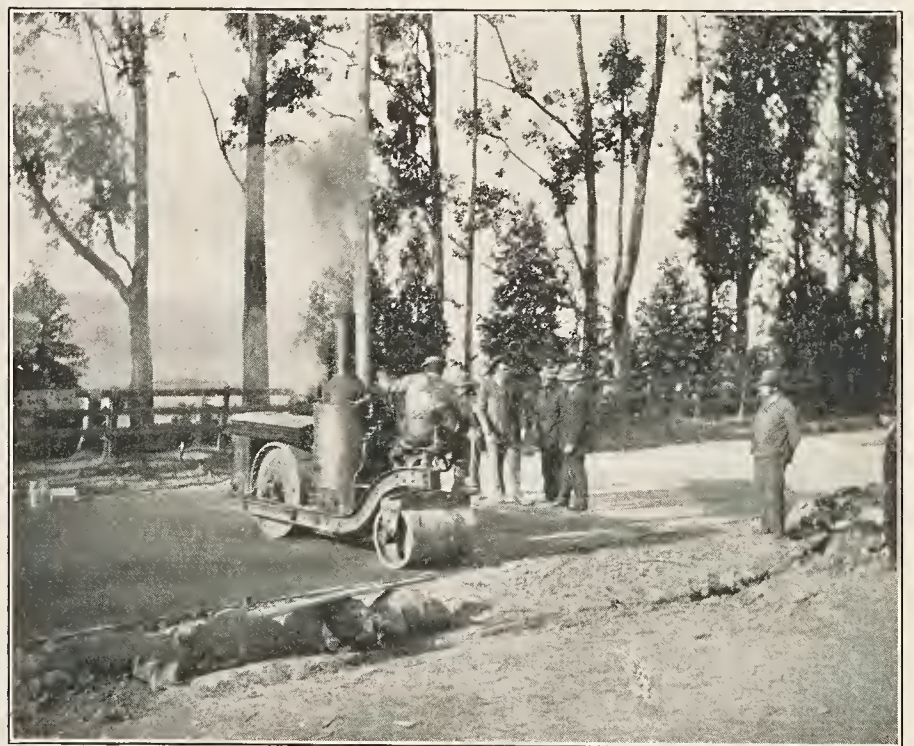
Rolling Asphalt Surface, State Highway, San Mateo County, Near Lomita Park.
