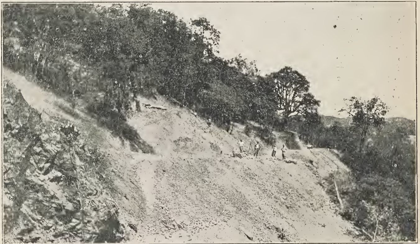
Grading State Highway Near Hopland, Mendocino County.
