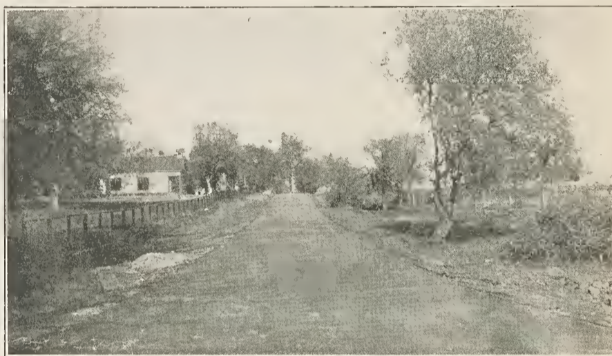
Concrete Base, Bituminous Surface, State Highway, near Roseville.
