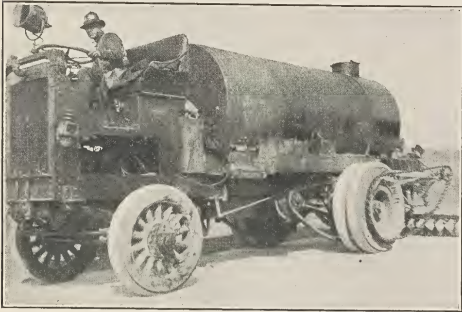
Motor Spraying Machine on State Highway, Los Angeles County.
