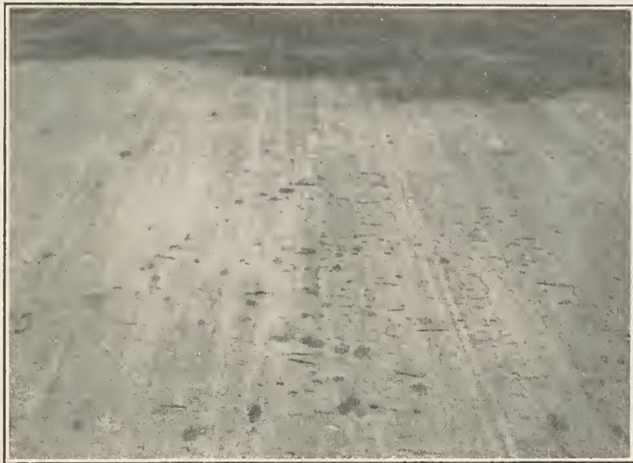
Concrete Base with Bituminized Top, Ann Arbor, Michigan.
