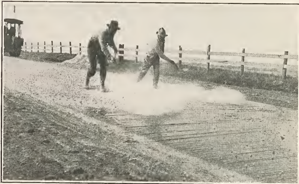
Spreading Screenings for Thin Bituminous Top, State Highway.
