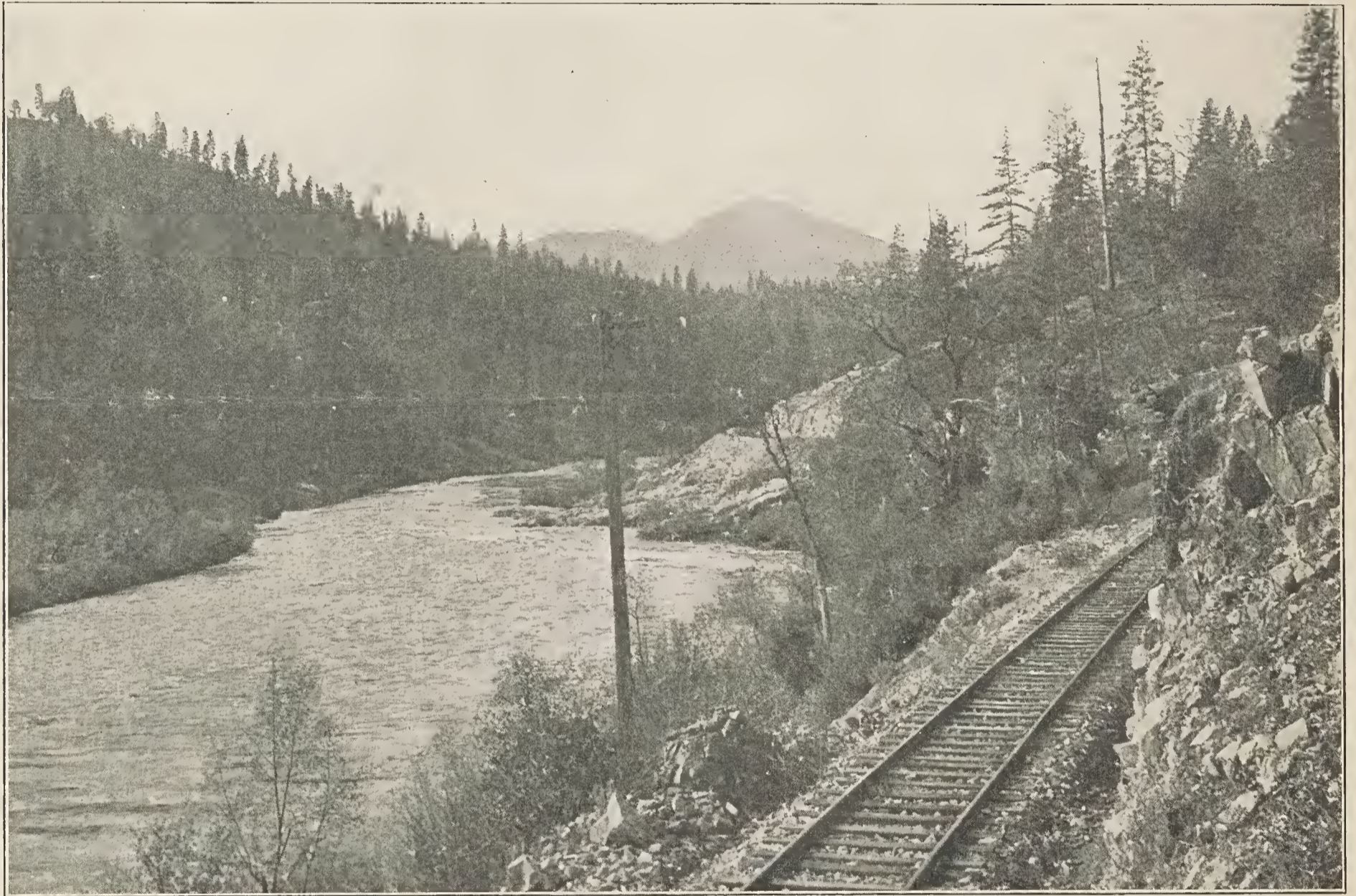
Pit River Bridge Site, Shasta County, State Highway Survey.
