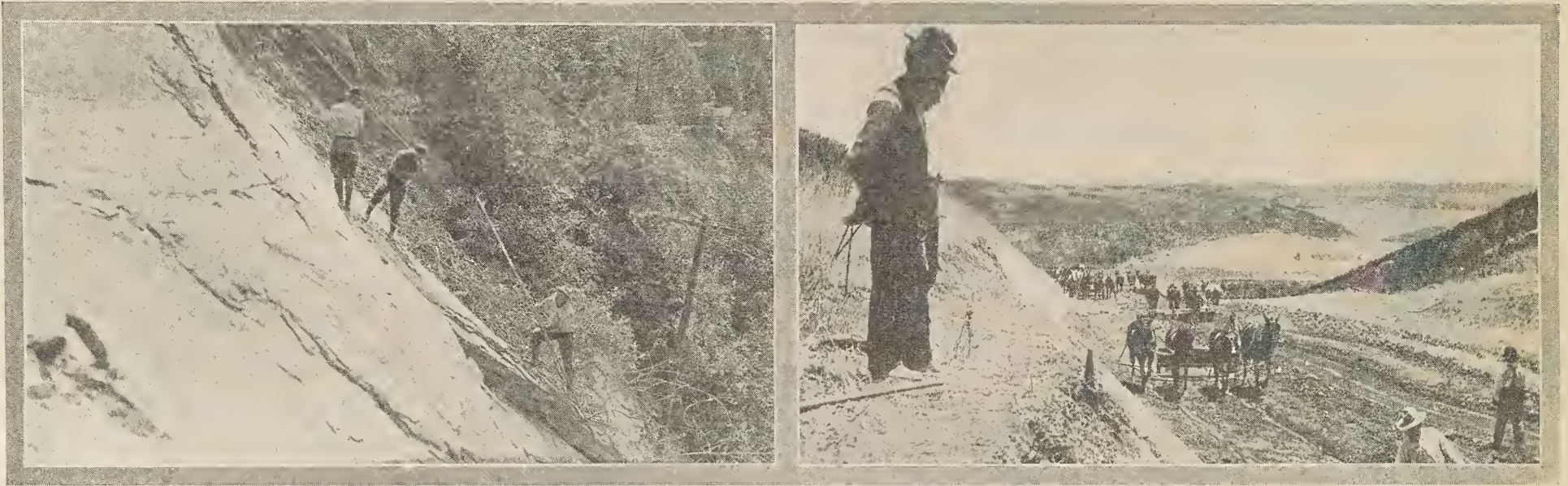
Surveying and Building Mountain Roads of State Highway
