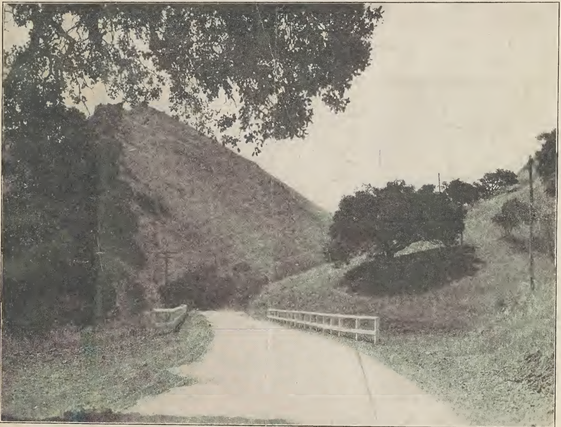
ON THE COAST ROUTE OF CALIFORNIA STATE HIGHWAY
