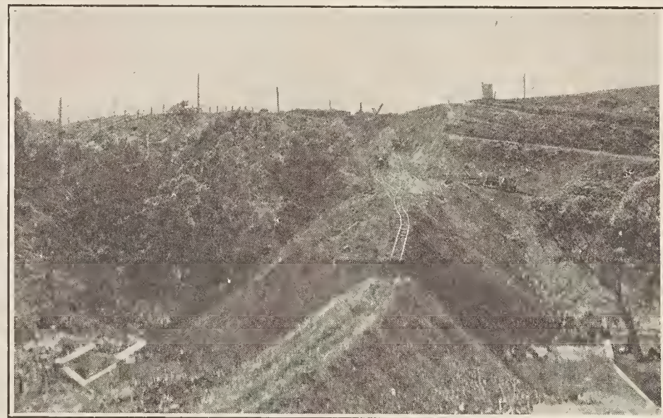
Cuts, Fills, and Culverts—State Highway Construction, Santa Barbara County.
