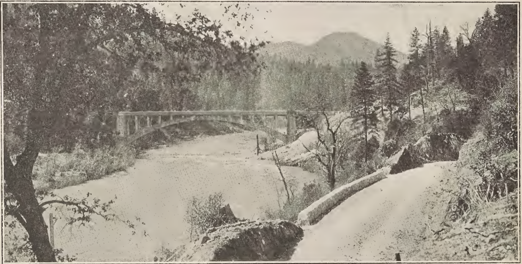
The Pit River Bridge near Baird, Shasta County. It lacks only a few feet of having the longest concrete arch west of the Rockies.
