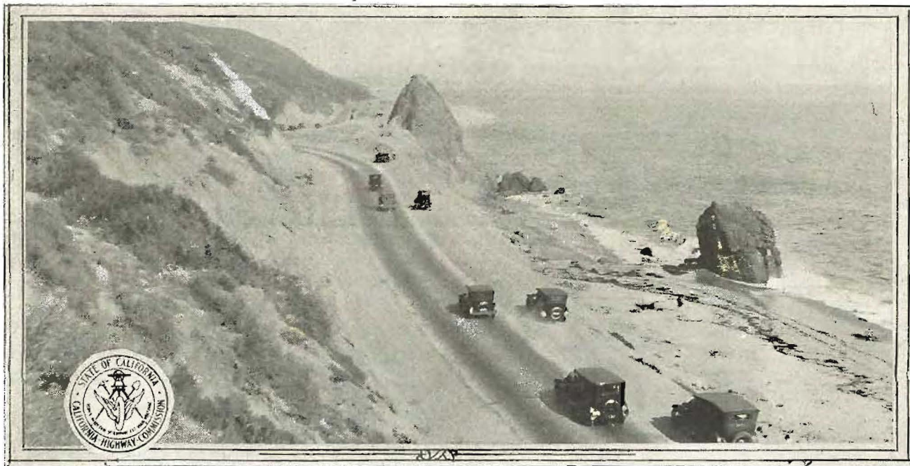
ALONG THE SOUTHERN COAST—View of the state highway north of Santa Monica, Los Angeles County, a part of the Oxnard-San Juan Capistrano route. This wonderfully scenic road is planned to relieve traffic in the congested section around Los Angeles. Its construction is going steadily forward.
