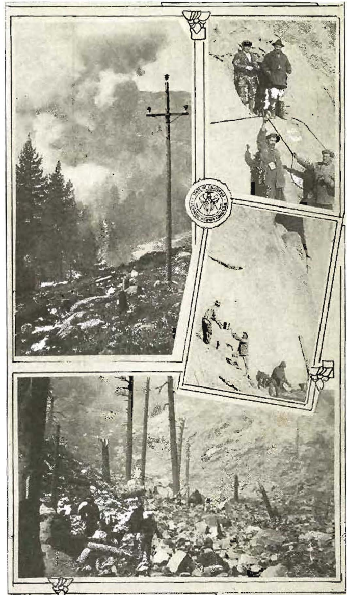
Within hearing of the graves of members of the famous Donner Party, who perished amid Sierra snows for lack of a road, the state is now building an improved highway. Thirty-three tons of powder recently were used to blast away a granite cliff. The pictures show powder being placed in the tunnels, fuses connected up, the blast, and some of the results. The new location will eliminate steep grades between Donner Lake and Donner Summit on the Victory highway.
