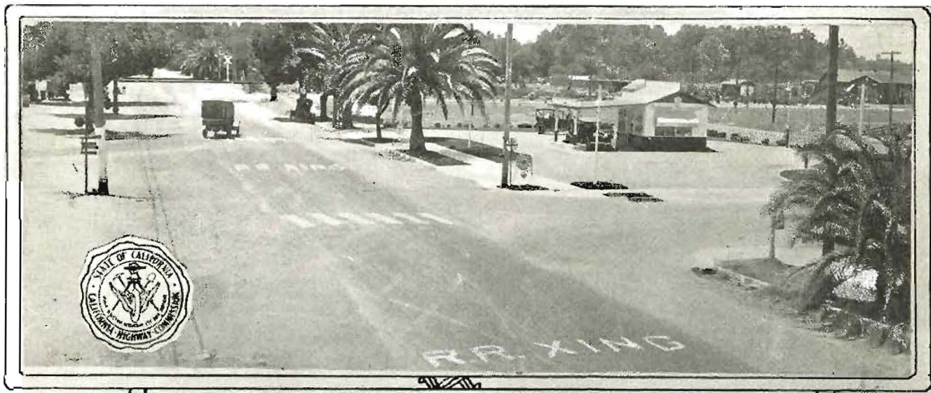
NEW GRADE CROSSING WARNING —Plan being tried out in Division VI. Approaching a grade crossing at the northern entrance to Fresno, the warning is painted on the pavement at intervals for several hundred feet. Similar experiments are under way near Modesto, Division X. See story on Page Six.
