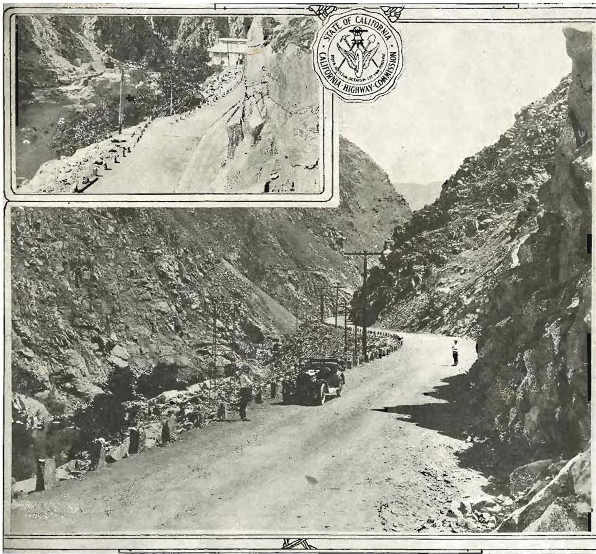
NATURAL ROCK GUARD RAIL IN THE KERN RIVER CANYON—Views on the Walker Pass route, east of Bakersfield, showing Division Engineer Woodson's natural rock guard rail. This guard rail is not costly and harmonizes with the rugged canyon.
