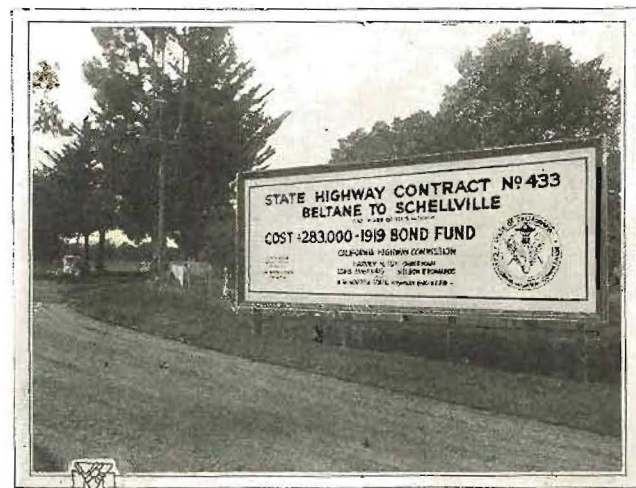
"THAT THE PUBLIC MAY KNOW"—One of the signs erected in Division IV to inform the public concerning highway construction under way in Sonoma County.
