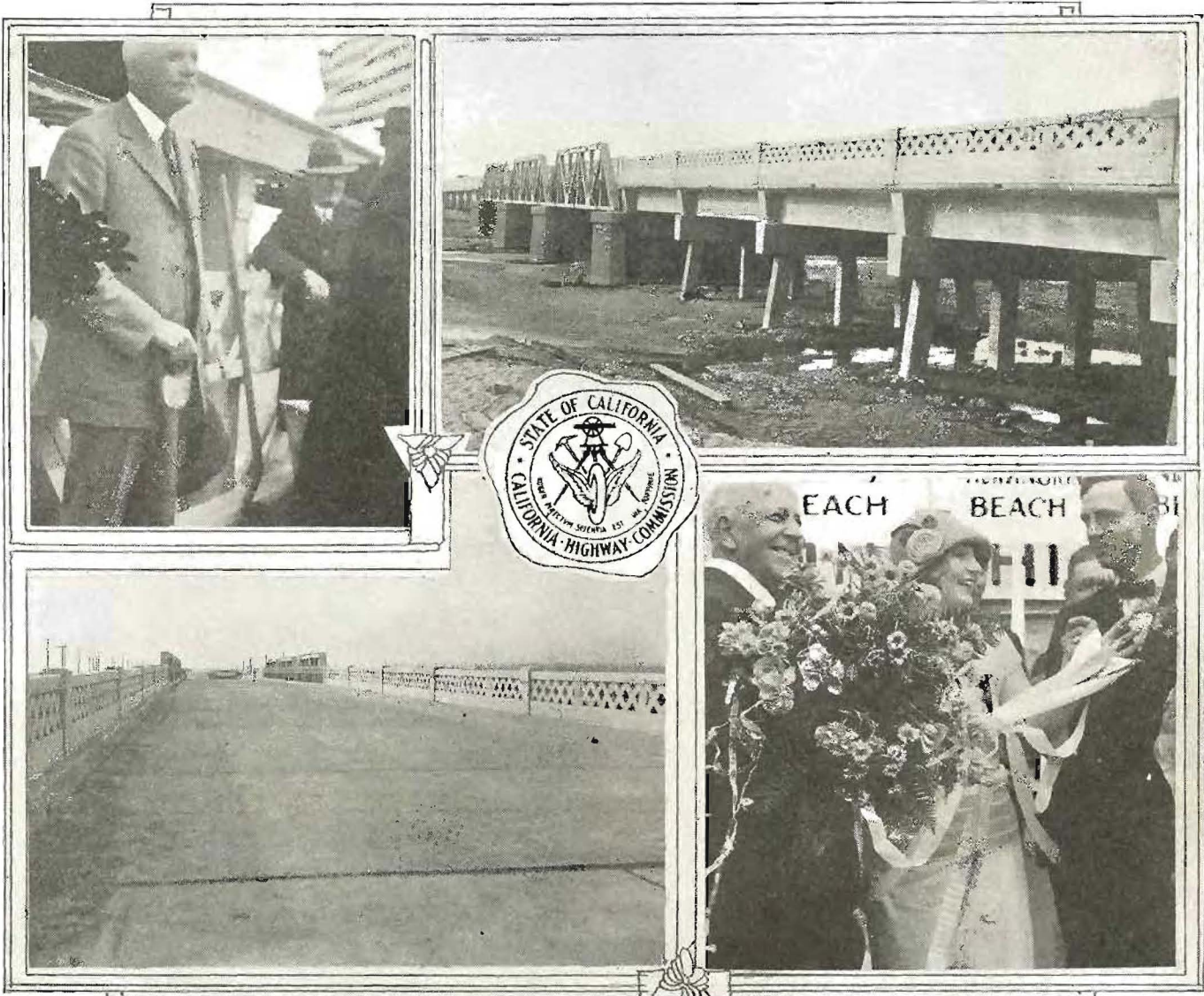
NEW SANTA ANA RIVER BRIDGE LINKS BEACH CITIES IN SOUTH—Scenes at the recent dedication of the Santa Ana River bridge on the Coast boulevard, Orange County. UPPER LEFT, Commissioner N. T. Edwards with silver plated shovel just after he had removed the last barrier of earth; UPPER RIGHT, the new bridge built by the county under joint state and county inspection; LOWER LEFT, another view of the bridge showing wide roadway; LOWER RIGHT, Miss Belle Bennett, screen star, and officials of beach chambers of commerce who took part in the ceremonies.
