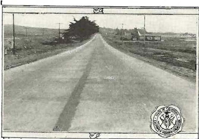
New cement concrete pavement on the Jahn and Bressi contract, in San Diego County, showing center expansion joint. A gasoline tax job.
