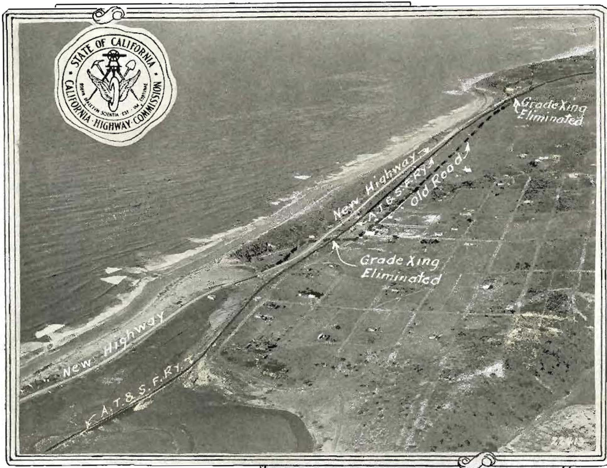
MAKING THE HIGHWAYS SAFE—AERIAL PHOTOGRAPH OF GRADE CROSSING ELIMINATIONS ON THE SAN DIEGO COAST—The new pavement between Encinitas and Cardiff has been constructed on the west side of the Santa Fe railroad, doing away with both crossings and reducing the number of curves from eleven to four and lowering the maximum grade from 7.10 per cent to 4.75 per cent. Distance shortened 350 feet. A gasoline tax job. (Div. VII.) Photo by U. S. Air Service.
