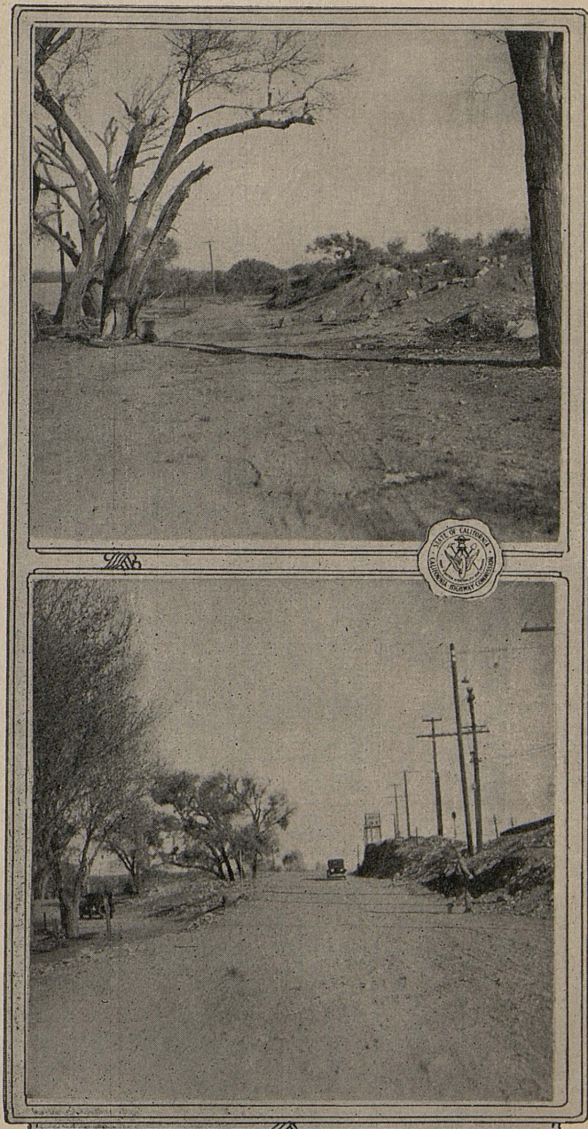
IMPROVEMENTS ON THE NATIONAL OLD TRAILS, SAN BERNARDINO COUNTY—Above, old county road near Oro Grande, between Victorville and Barstow; below, recently completed state highway grade, same point. This improvement was financed with state highway funds.
