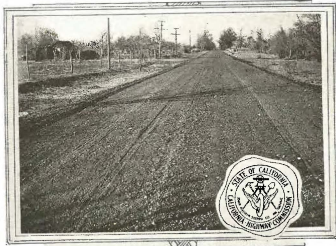
VOLCANIC CINDERS—The state highway near Independence, Inyo County, surfaced with crushed volcanic cinders. (Division IX.)
