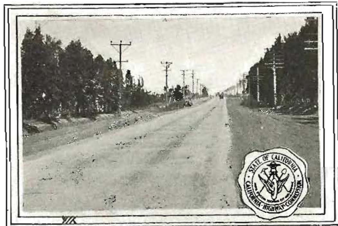
New twenty-foot concrete pavement in Sacramento County placed on an oil macadam sub-base. A gasoline tax job.
