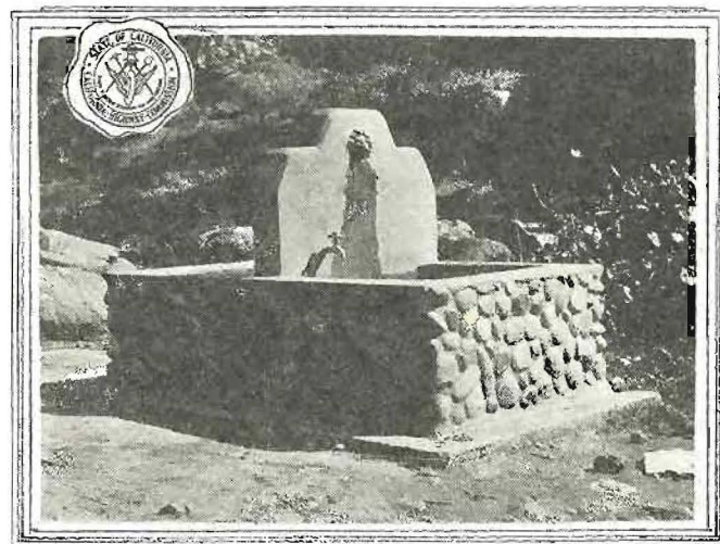
ROADSIDE WATERING PLACE—Fountain built on the highway right of way near Sonora, Tuolumne County, with funds furnished by the Lions Club of that community. Its water supply comes from a nearby spring. Plans were furnished and the work supervised by Division X.
