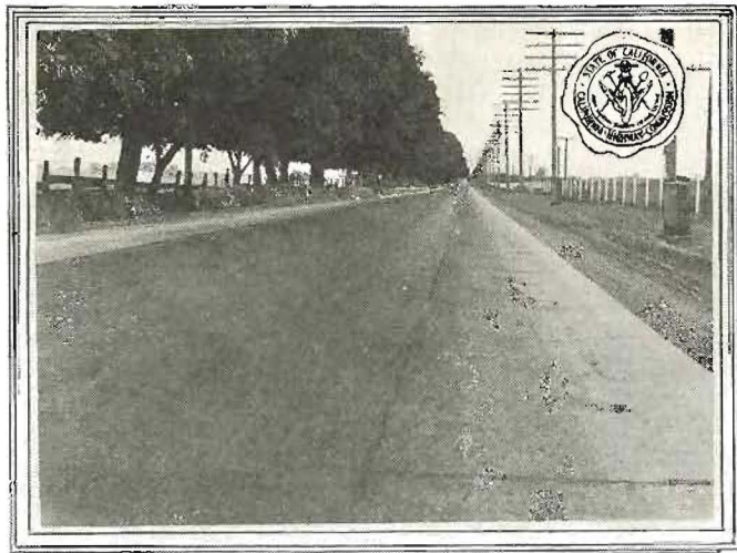
NEW SHOULDERS IN YOLO COUNTY —View of new six-foot flush cement concrete shoulders recently placed on the state highway between Davis and the Woodland Wye, Yolo County. This section now has a twenty-seven-foot width of pavement and, in addition, a two-foot rock shoulder at either edge, making a thirty-one-foot roadway. The county cooperated with the state in financing the improvement. (Photo by Div. X.)
