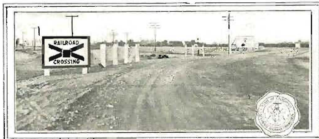
Type of railroad crossing warning in use in Division VI. The center is a Reflex lens.
