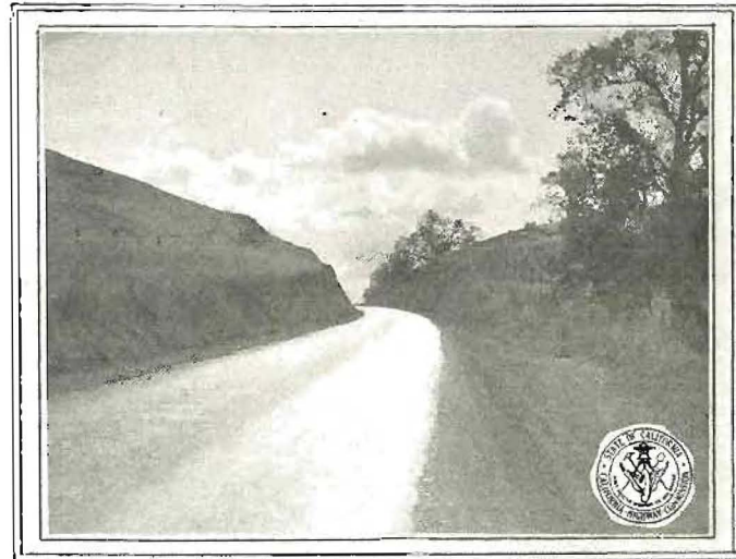
A section of oiled highway on Redwood route, Division I. The public is now demanding more improvements of this kind on this route.
