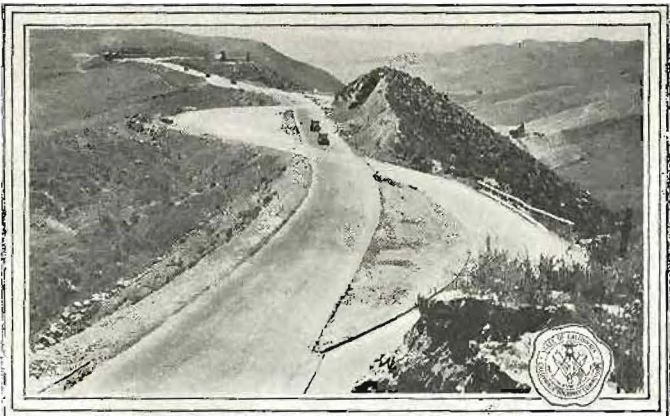
RIDGE ROUTE LINE CHANGE—Callahan line change as it looks today. New line eliminating curves has been paved with oiled macadam. Photo by Division VII.
