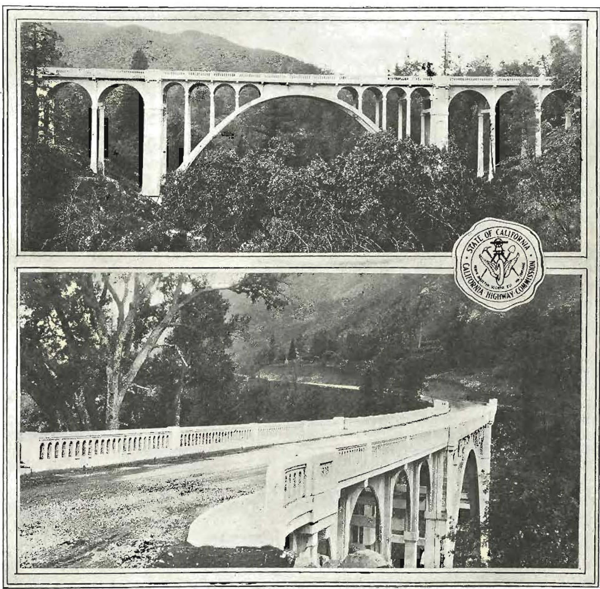
PACIFIC HIGHWAY ARCH—Bridge across Charley Creek in northern Shasta County. This structure, 120 feet from creek bed to bridge floor, shortens distance nearly a half mile and greatly improves alignment. Plans for two other similar structures have been completed by Bridge Department. (See article on page eleven.)
