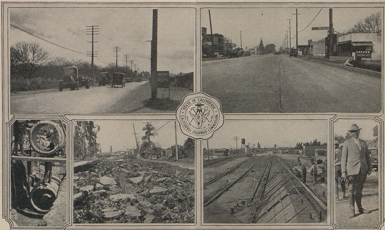
RECONSTRUCTION OF WHITTIER BOULEVARD—The state highway between Los Angeles and Whittier is now a fifty-six-foot street surfaced with heavy pavement for the entire distance. Left, above , Old oil macadam surfacing twenty-two feet wide; (note extreme crown, dangerous to motor vehicle traffic); Right , New state highway through Pico, paved with concrete for full width of street. Left to right, below , Rebuilding pipe line to care for irrigation; oil macadam scarified to provide base for new pavement; paving approaches and retaining walls at Montebello subway; A. N. George, resident engineer. Reconstruction with gasoline tax funds. (Photos by Div. VII.)
