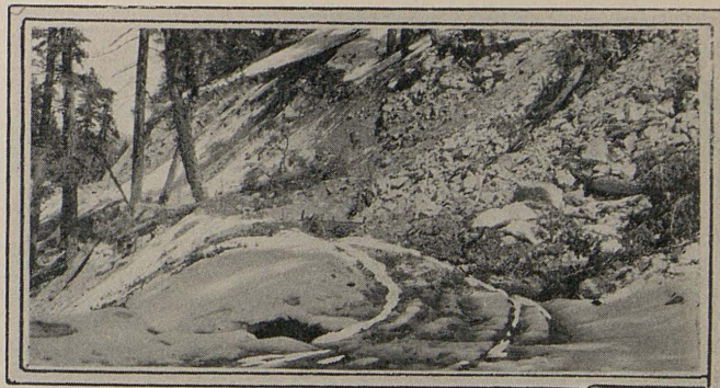
ON THE CREST ROUTE—A typical slide on the state highway in the San Bernardino Mountains where Division VIII is being forced to make large expenditures of maintenance funds because of heavy storms during recent weeks.
