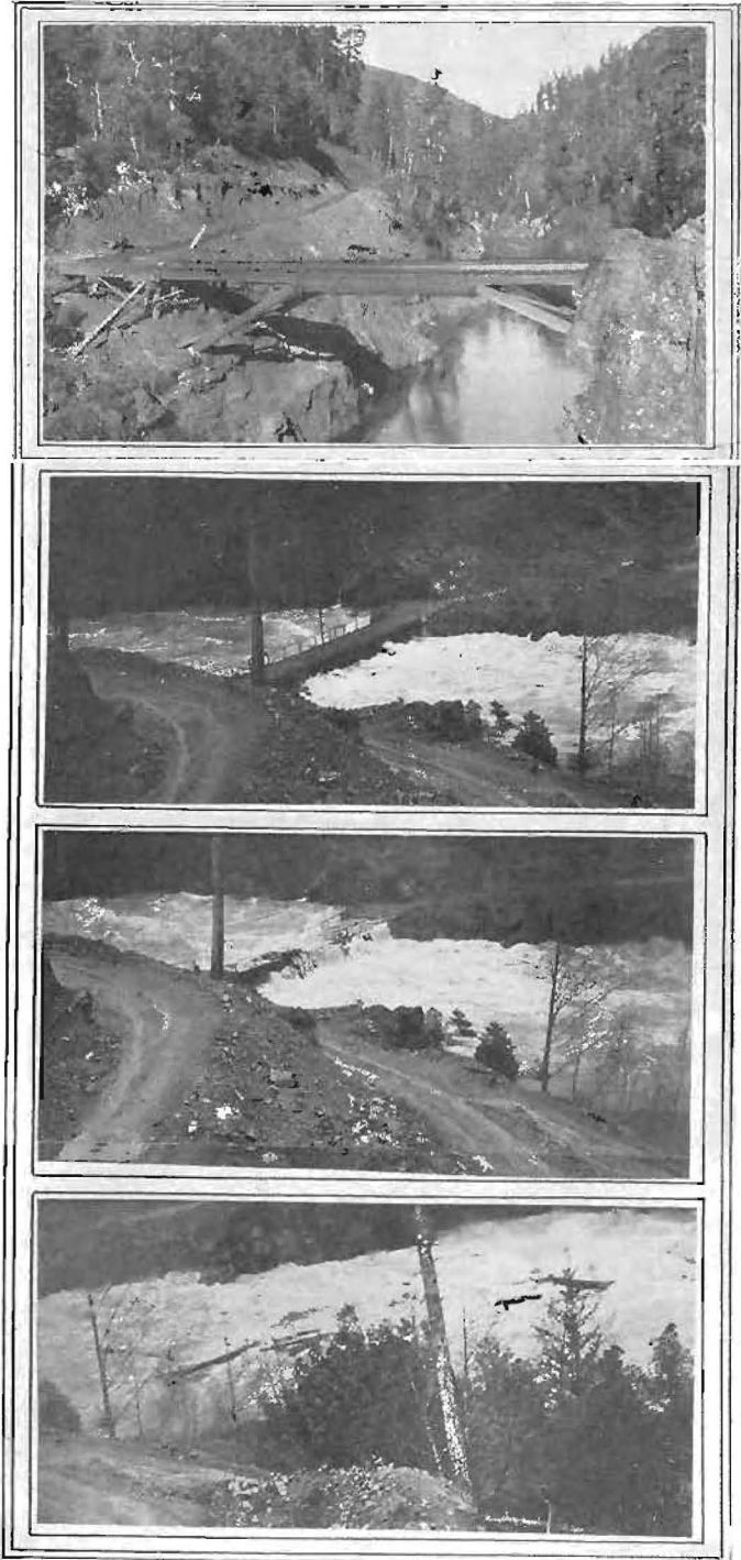
RIVER ON RAMPAGE—Above, summer level of Smith River, Del Norte County; temporary bridge in use while Redwood highway is under construction; below, three views taken within an hour showing destruction of bridge during recent storm; heavy wire cable anchors were of no avail. (Views taken near prison road camp.)
