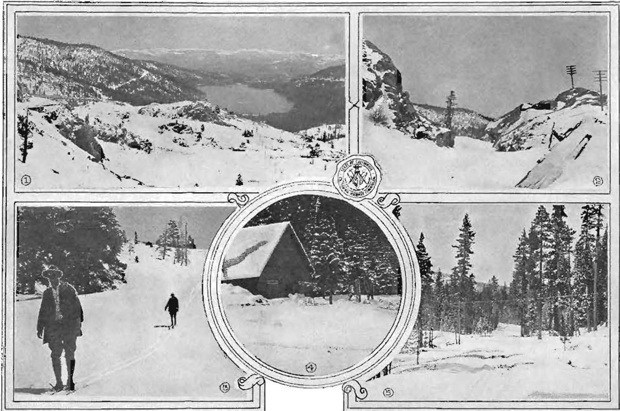
SCENES ON THE CALIFORNIA STATE HIGHWAY IN THE HIGH SIERRAS—(1) Donner Lake from Donner Summit; note Donner Summit Bridge to the left. (2) A 20-foot cut on the highway nearly level with snow. (3) State highway looking towards Donner Summit. (4) Camp at Tahoe City. (5) State highway looking east towards Tahoe City from Tahoe Tavern.
