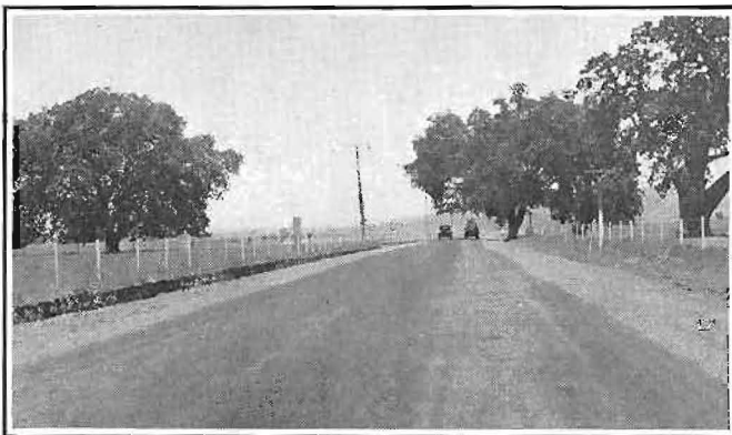
AFTER OILING.—A portion of the Cholame Lateral following oiling by the "mixing" method.
