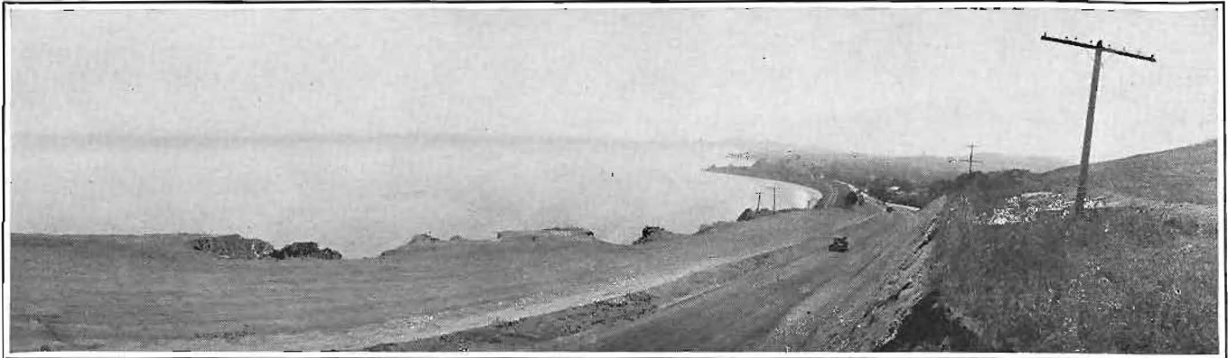
COAST ROUTE HILL CONQUERED.—View of recently graded State highway along Santa Barbara channel, over Ortega Hill, near Summerland, Santa Barbara County. The roadway was daylighted giving motorists a view of the majestic Pacific.
